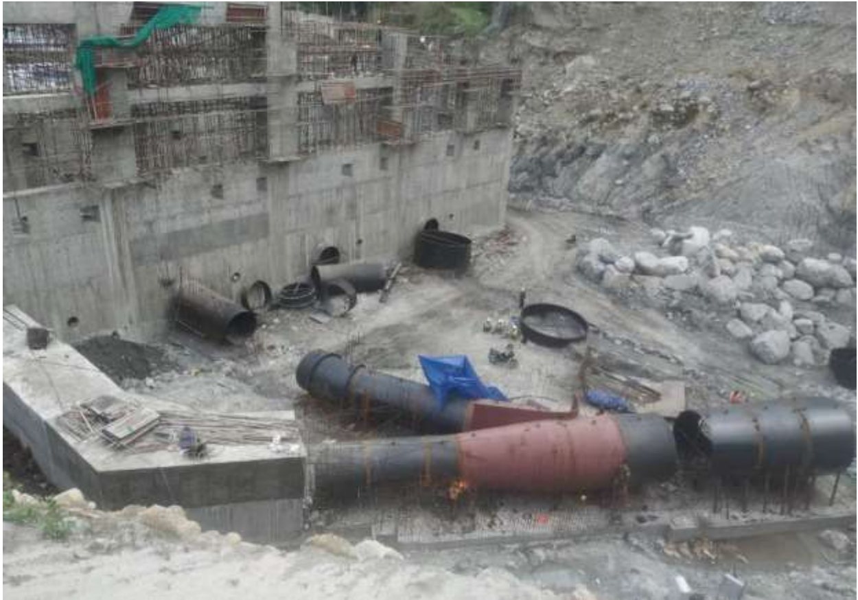
Figure 27: Concreting works at the manifold
