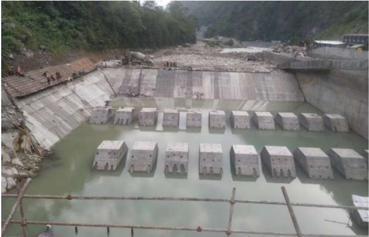
Figure 12: Aerial view of concreting works at stilling basin along with baffle blocks
