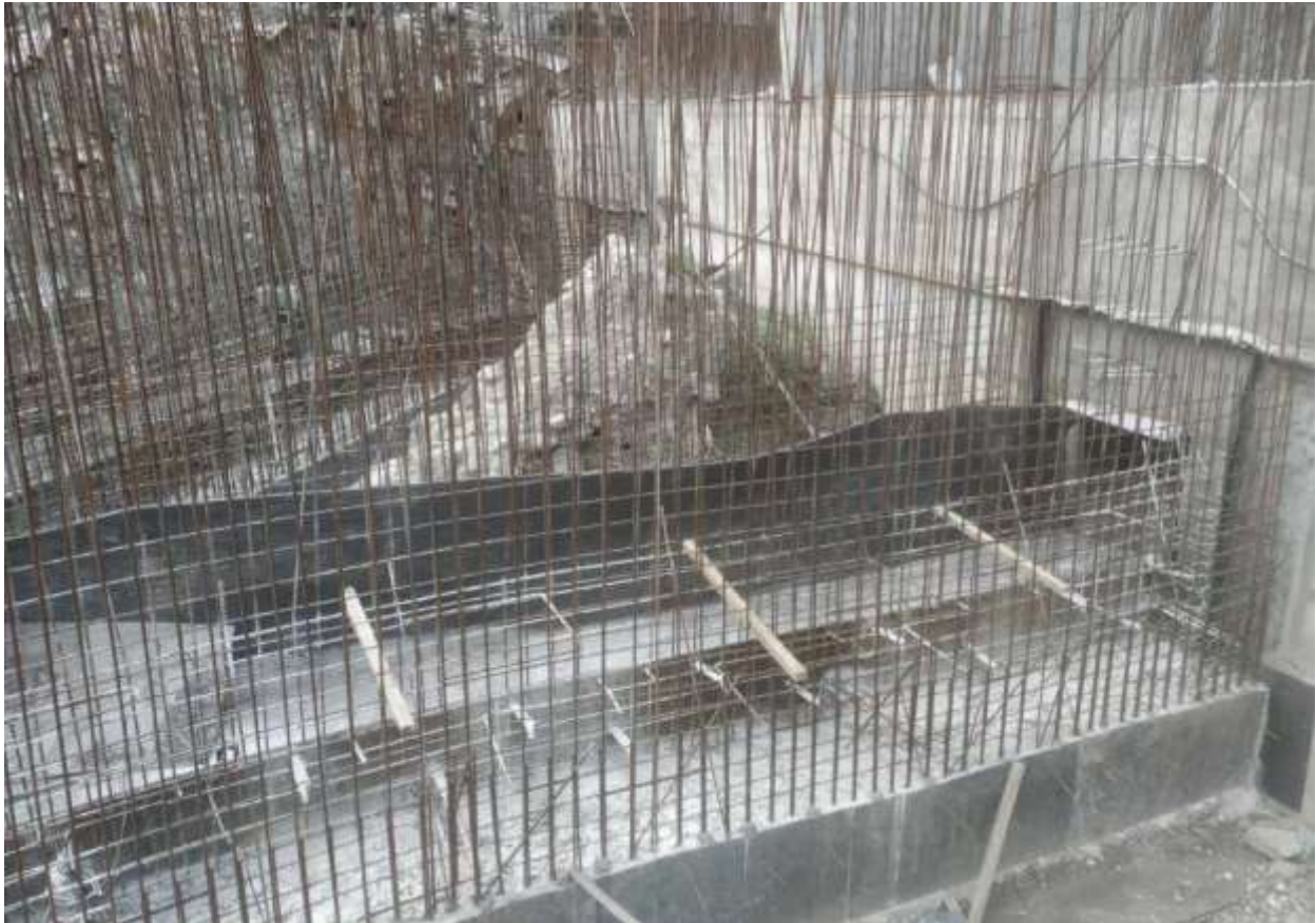
Figure 39: Steel lining works at gravel flushing culvert
