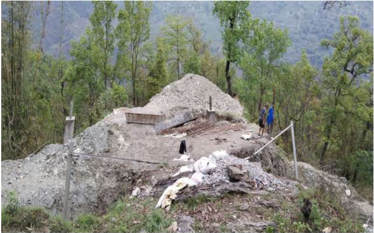
Figure 50: Stubs erection in AP-18
