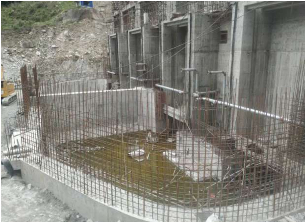
Figure 31: Reinforcement works at Tailrace culvert Panel 01 & 02
