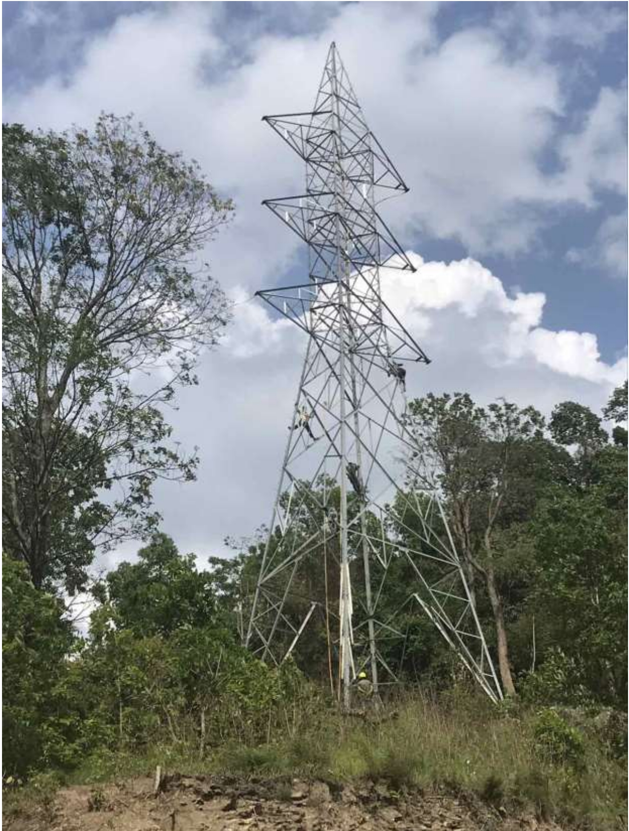
Figure 56: Tower erection works ongoing at AP16
