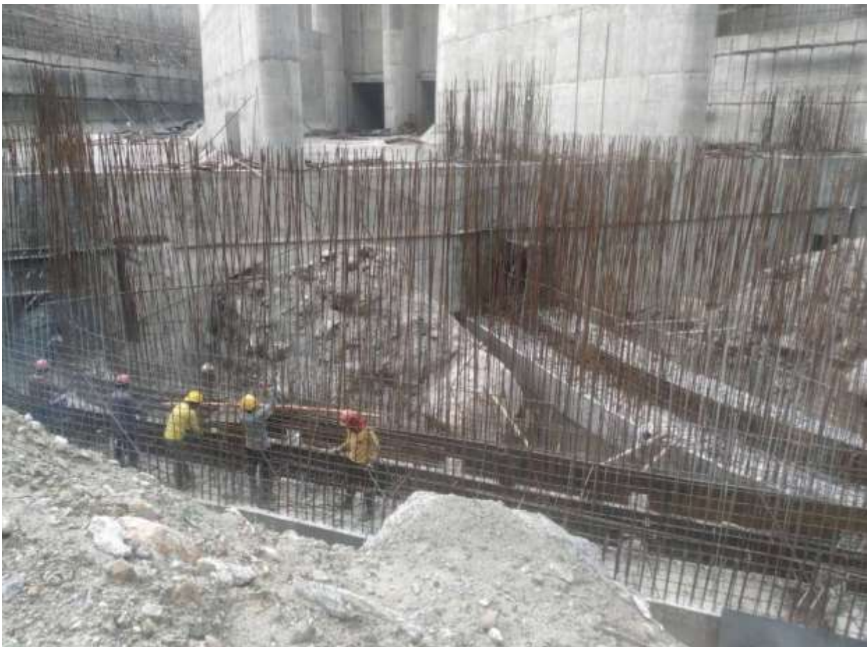
Figure 10: Rebar and steel plate installation in gravel flushing culvert
