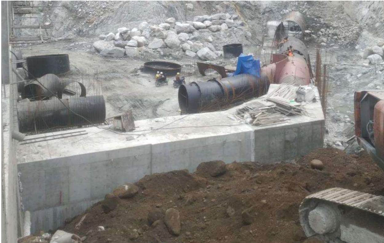
Figure 32: Backfilling works at Penstock manifold
