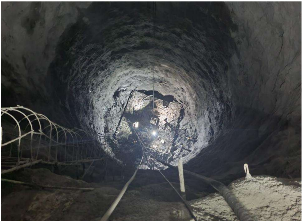
Figure 26: Excavation of Surge Shaft
