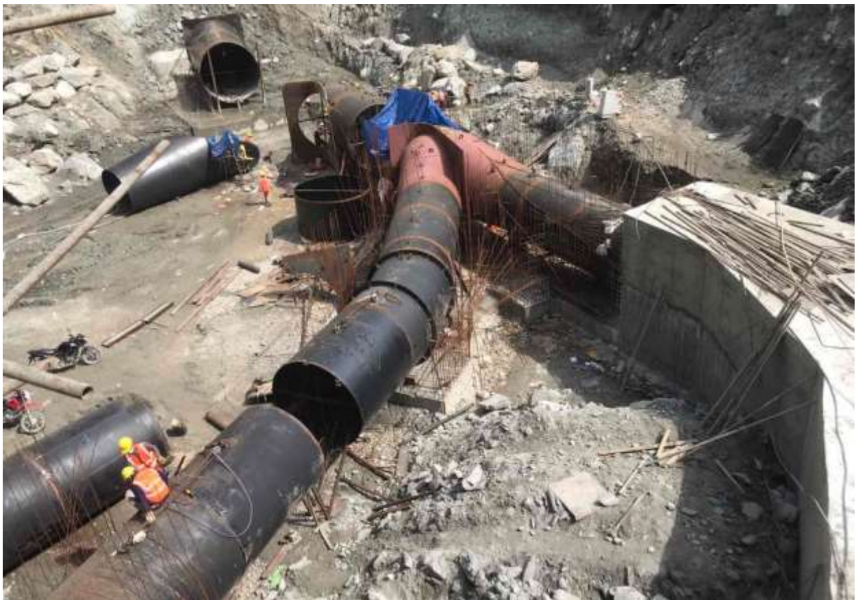
Figure 36: Bifurcation Unit 3 ( Inlet Dia: 3.18 m, Outlet Dia: 2.25 m , thk: 25 mm)
