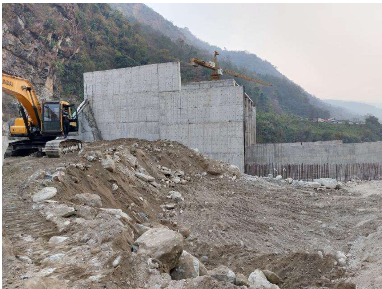
Figure 16: Backfilling works at u/s floodwall region
