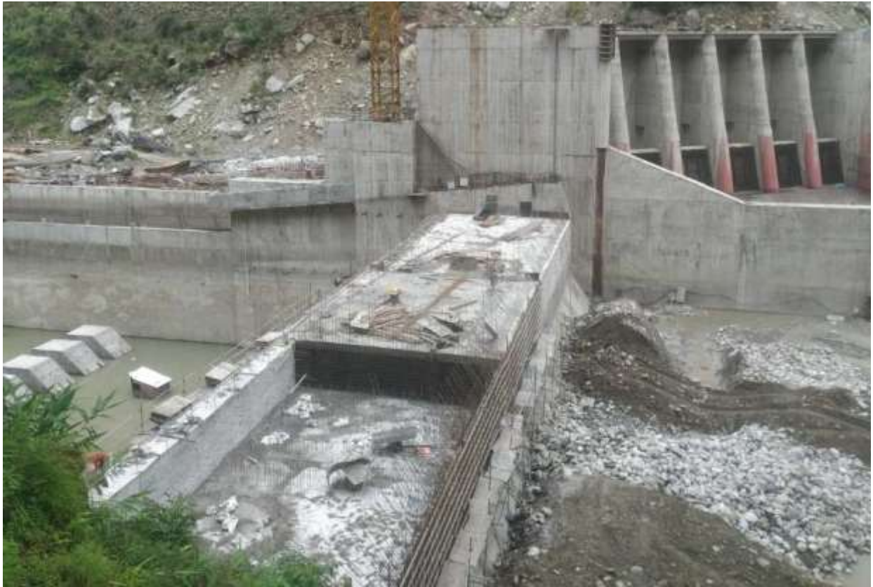
Figure 14: Concreting works at weir main body
