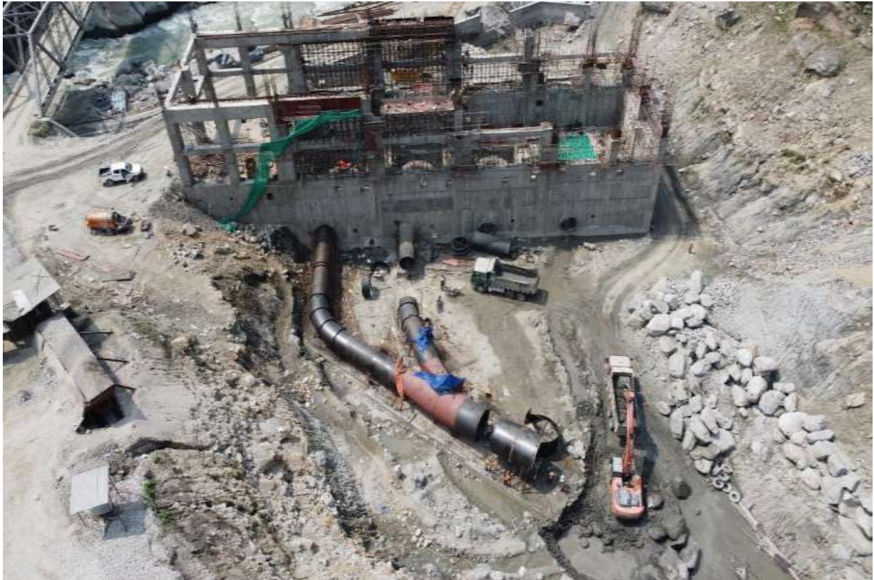
Figure 37: View of excavation works and installation works of penstock
