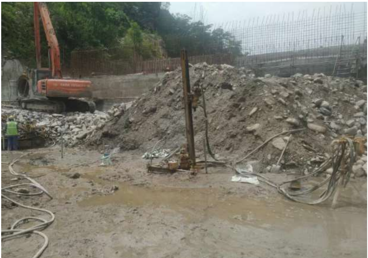
Figure 15: Curtain grouting works at U/s slab of weir
