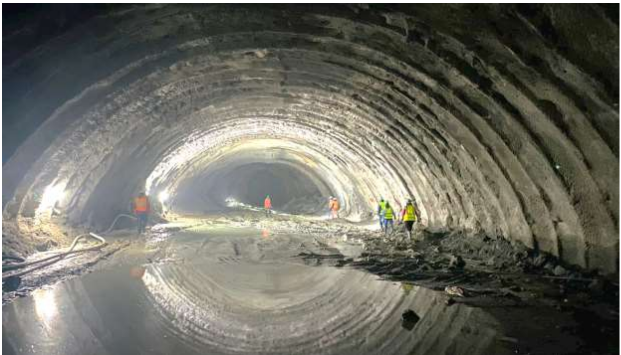
Figure 22: Breakthrough at Connecting Tunnel junction (SB-02)
