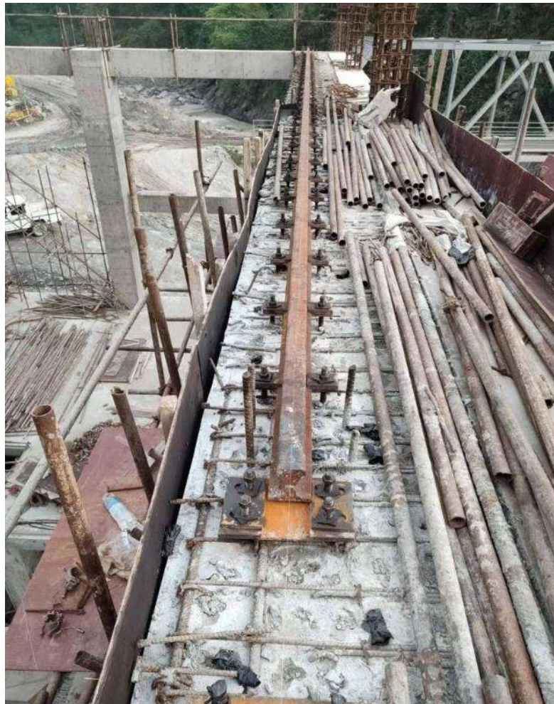
Figure 41: Ongoing Installation of rail track in Bay 1 downstream's crane beam
