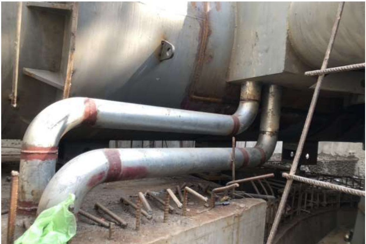
Figure 54: Nose drain of Spiral case
