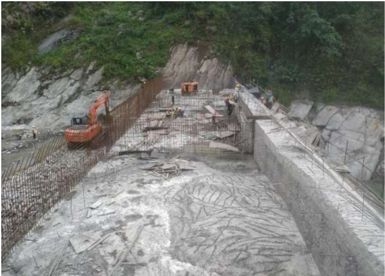
Figure 13: Rebar Installation works at Panel 02 and 03 of main weir body
