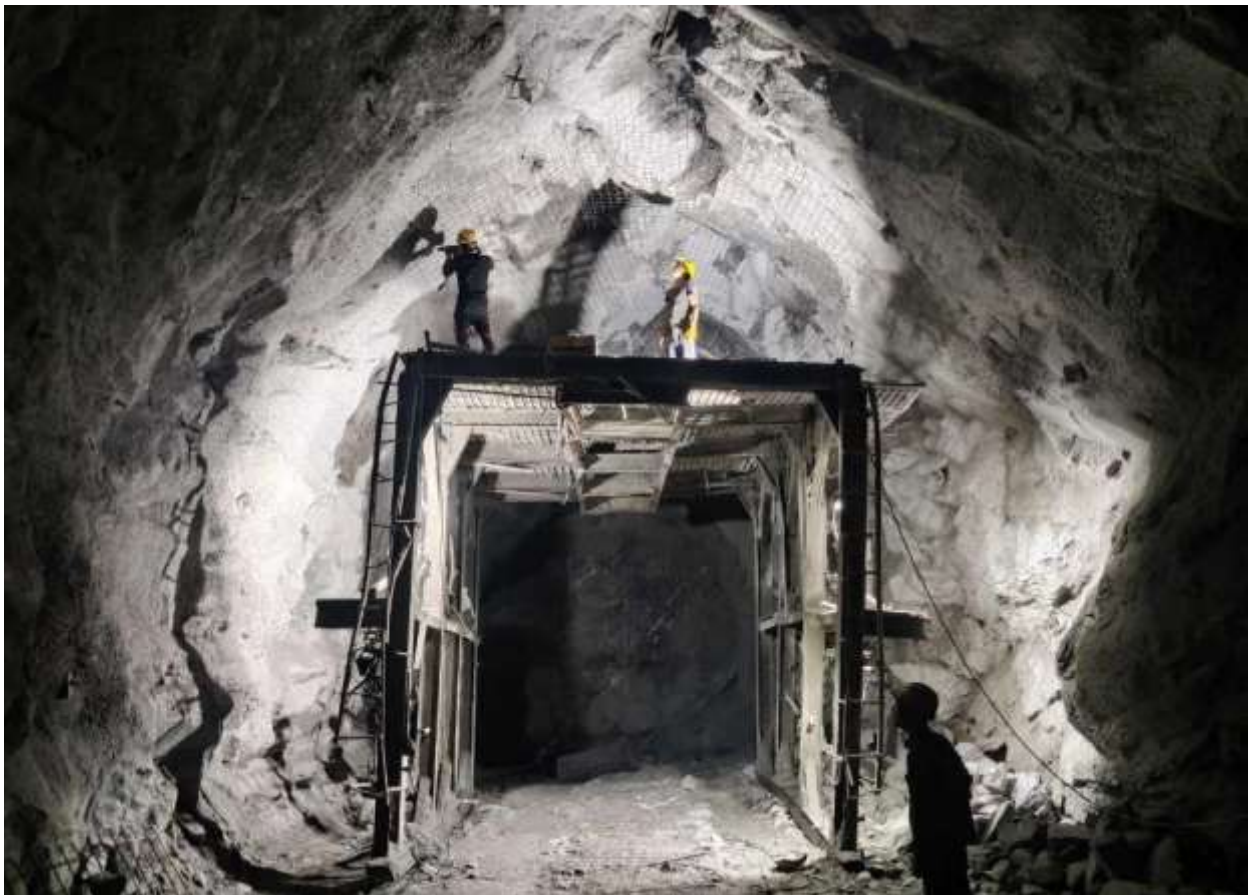
Figure 20: Rock support works at HRT from adit
