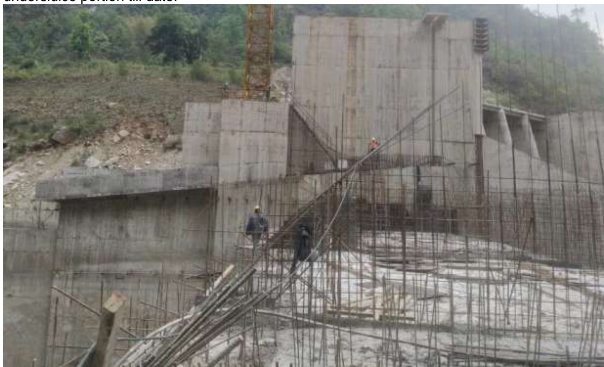
Figure 11: Reinforcement works at weir main body
