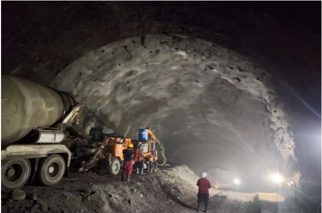
Figure 21: A view of application of shotcrete with robotic shotcrete machine at SB-02
