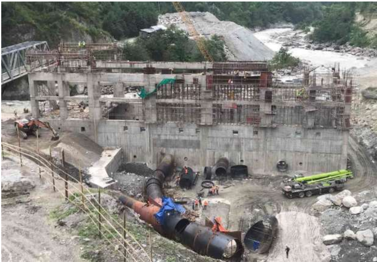
Figure 33: Interface works at manifold
