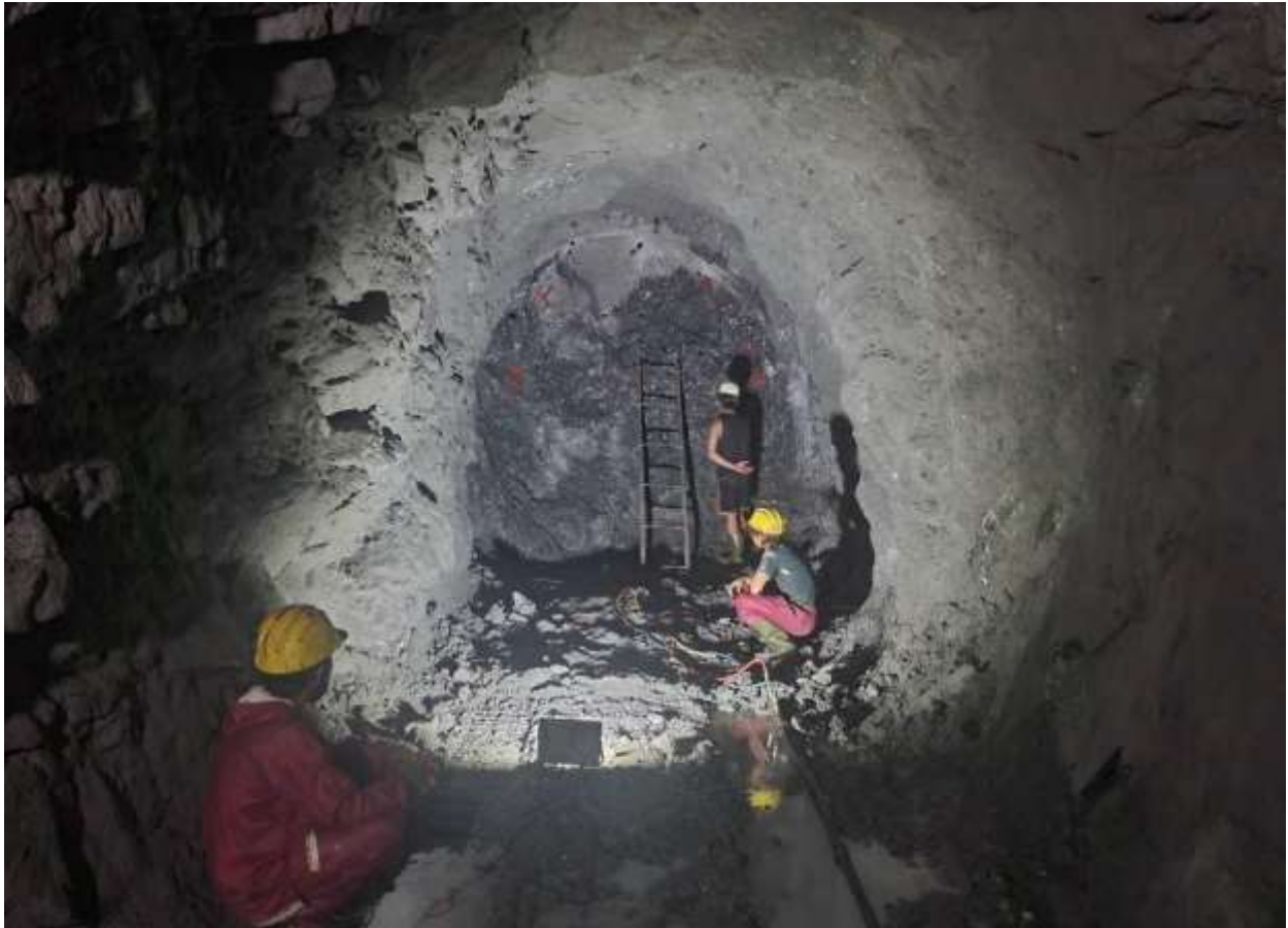
Figure 23: Excavation works at flushing tunnel
