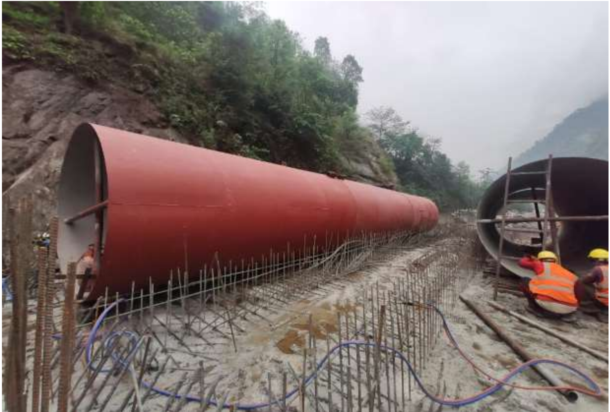
Figure 35: Erection of weir flushing pipe (ID: 2.25 m , thk: 12 mm)p
