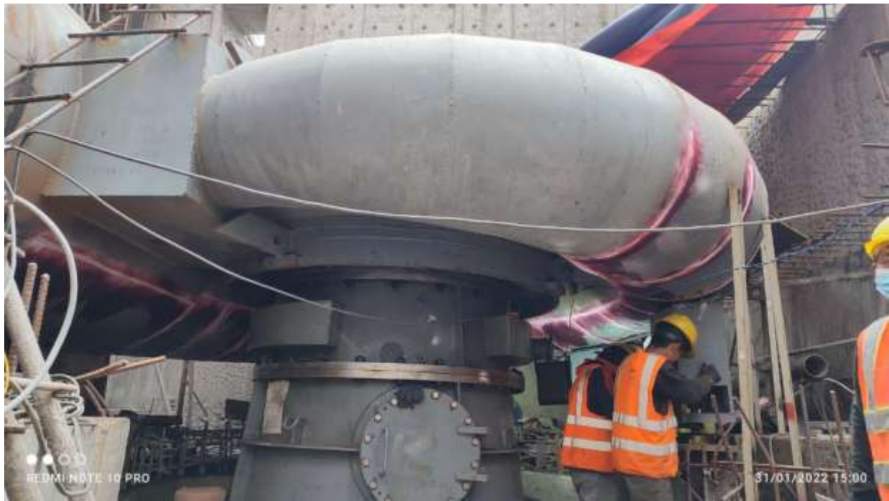
Figure 51: DPT test of welded segments of Spiral case
