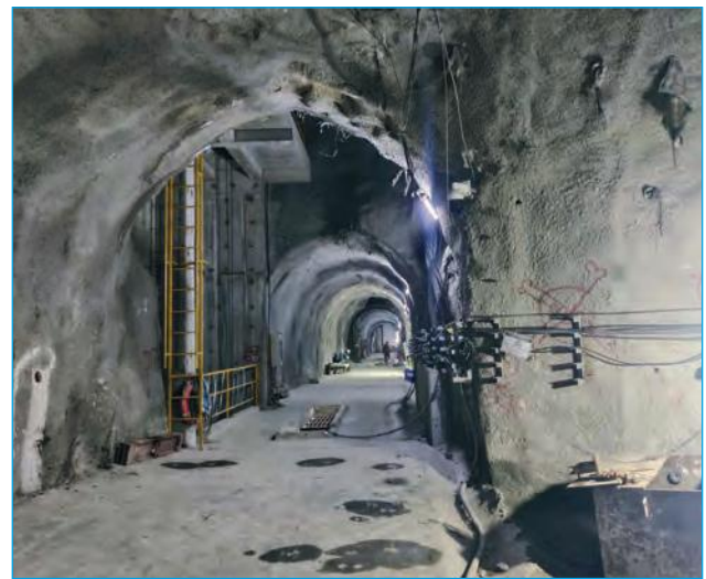
Underground Inspection Tunnel
