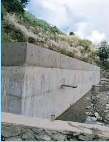
Fire Fighting Water Tank
