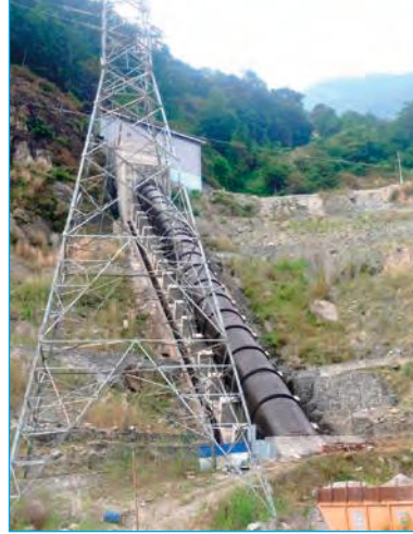
Penstock Slope Protection Works
