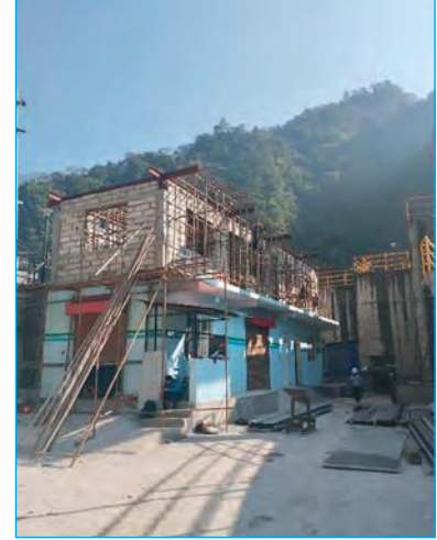
Headwork's Control Building
