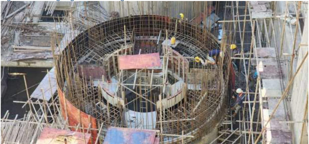
Figure 33: Rebar installation for generator casing at unit 02
