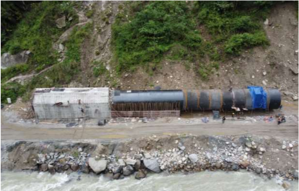
Figure 14: Erection of concrete encased approach pipe
