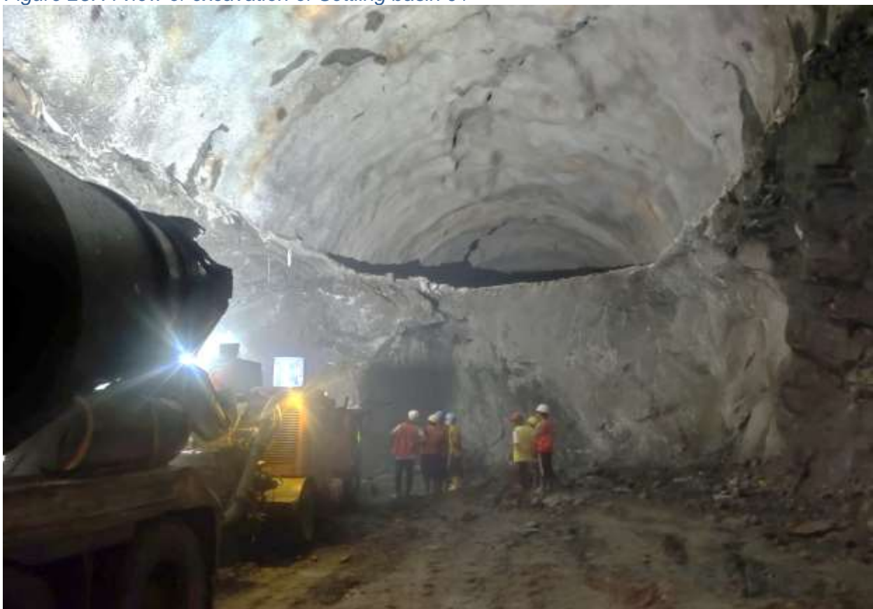
Figure 26: A view of excavation of Settling basin 02
