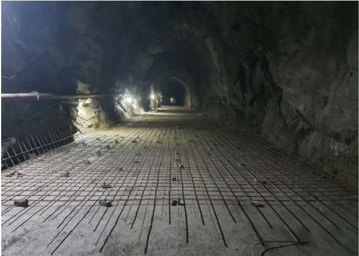
Figure 21: Rebar layout at the HRT invert
