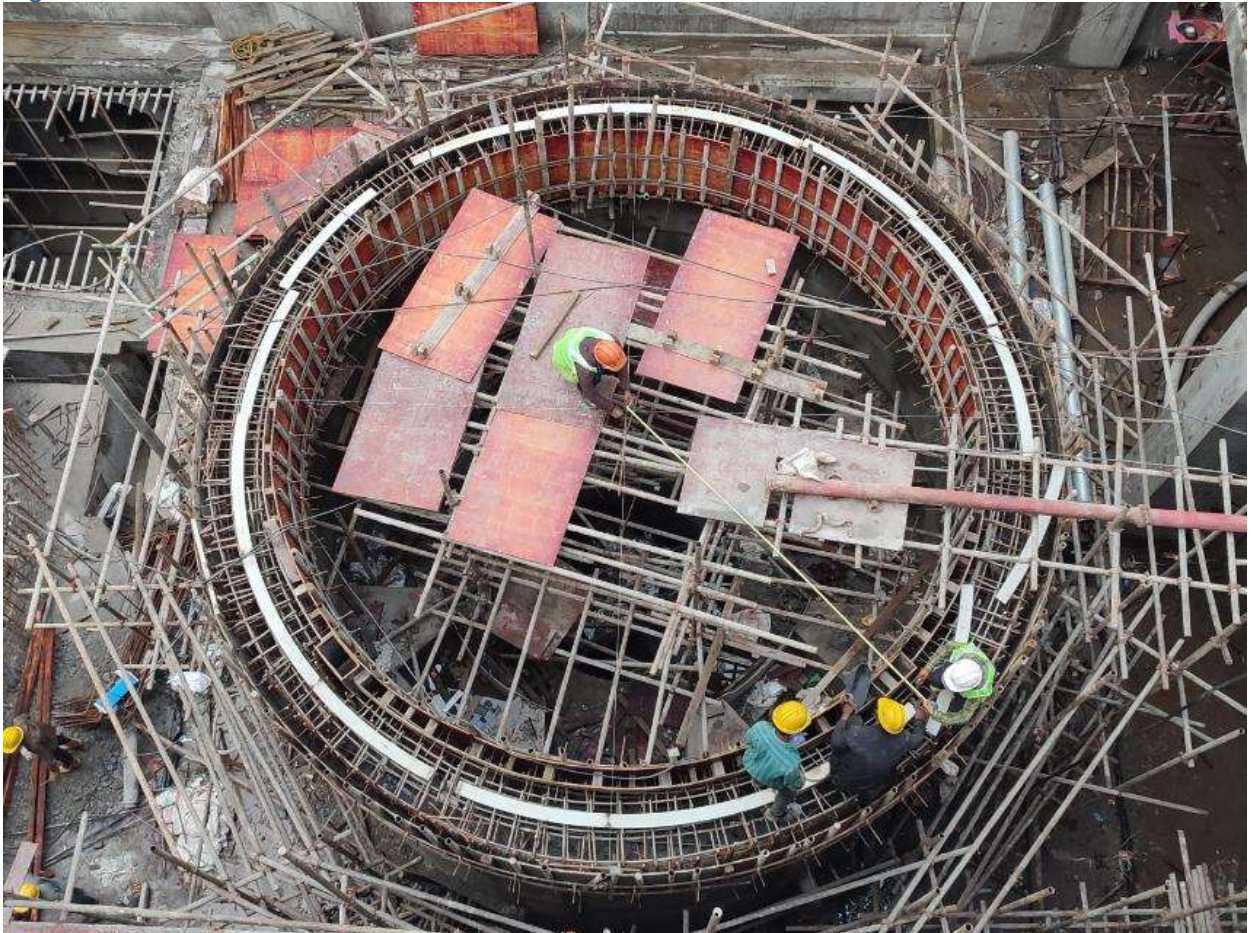
Figure 63: View of Unit 1 generator Pit ready for concreting
