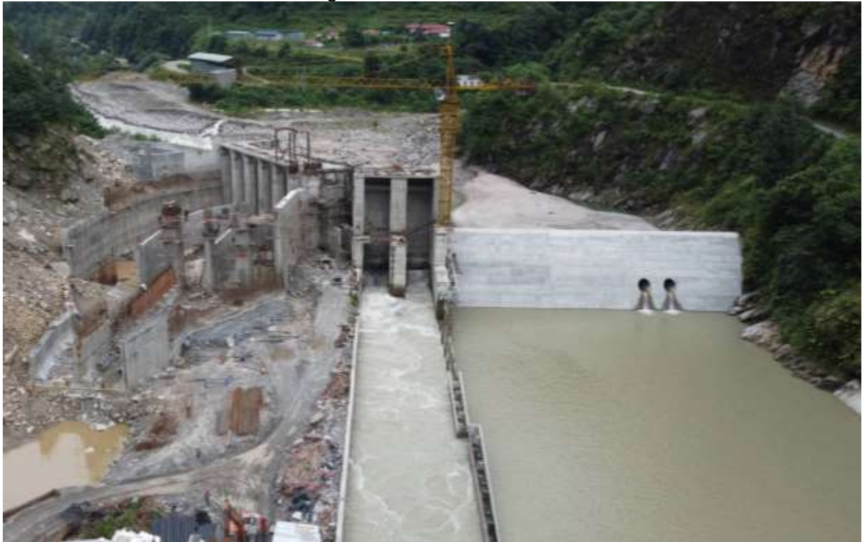
Figure 11: Aerial view of headworks with completed weir to the right
