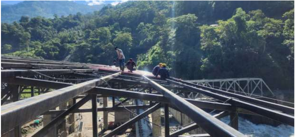
Figure 35: Roof installation works
