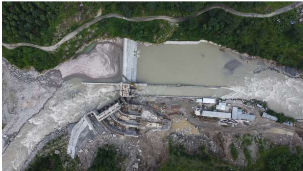
Figure 7: Aerial view of Headworks
