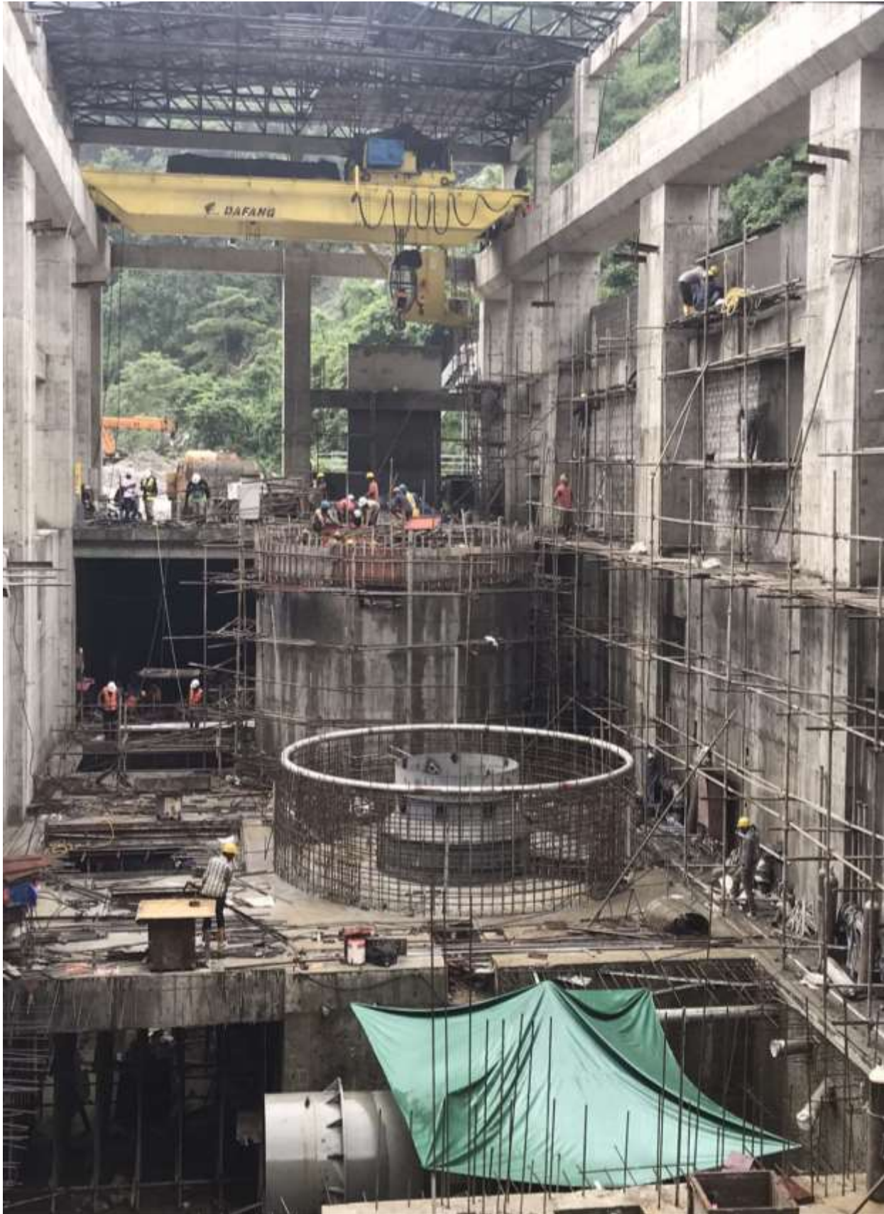
Figure 61: Installation of embedded plates of generator
