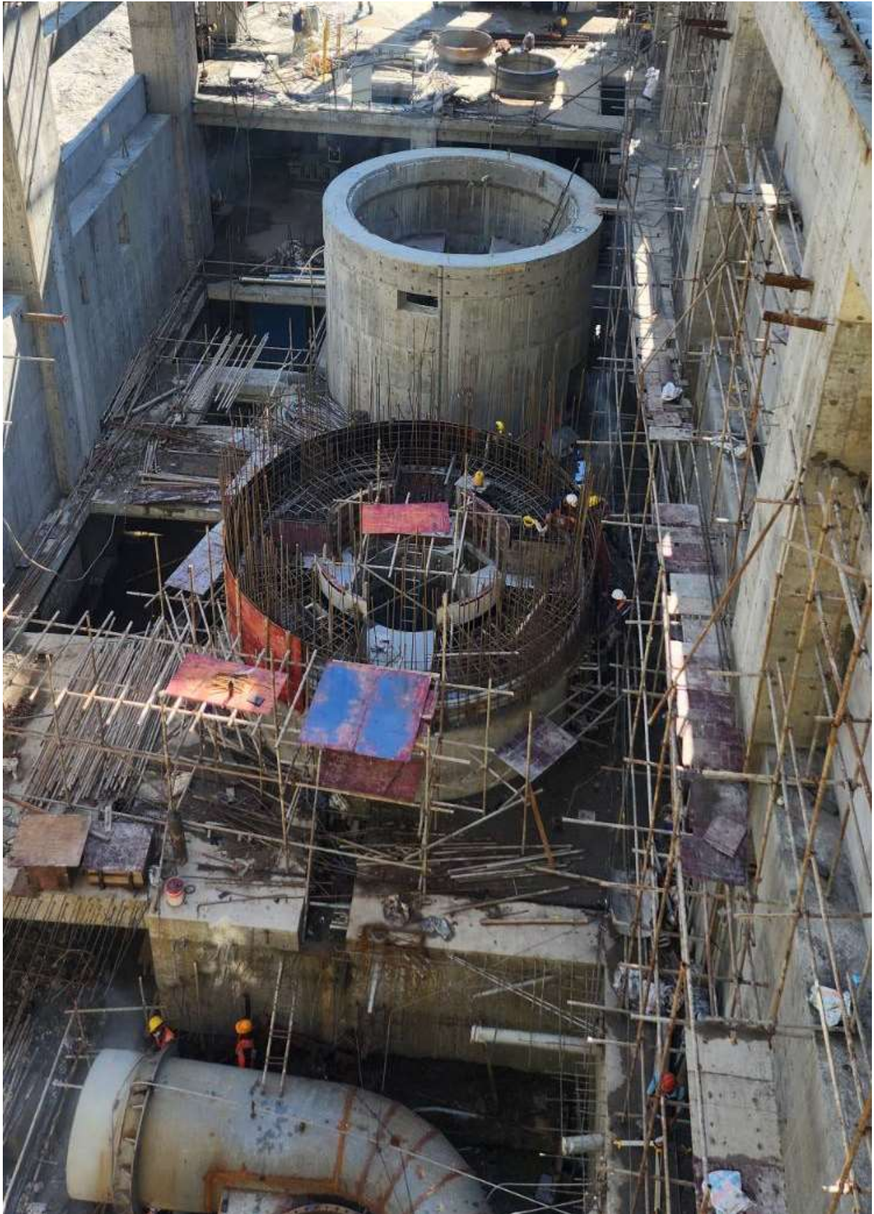
Figure 49: Installation of spiral case using EOT crane after cone installation
