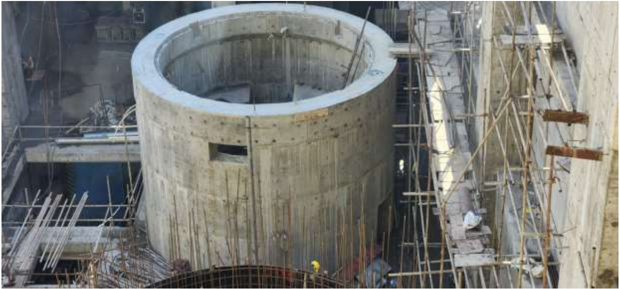
Figure 32: Casting of generator casing at unit 01
