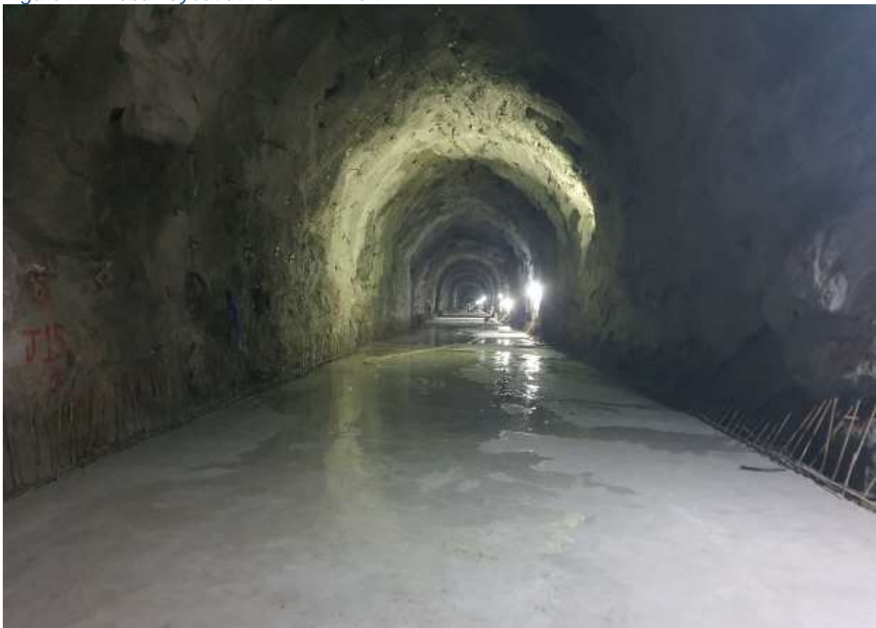
Figure 22: Concreting works at HRT invert
