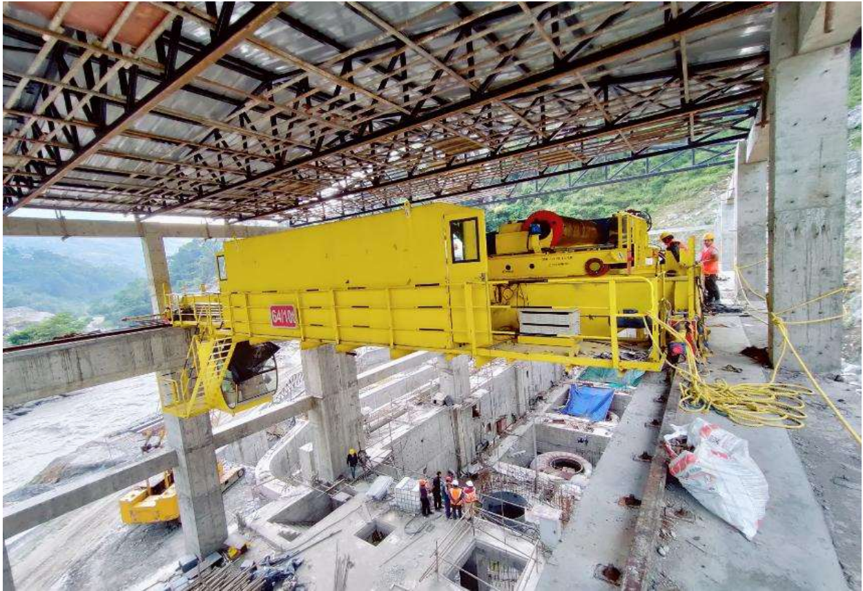
Figure 54: Electrical connection works of EOT crane
