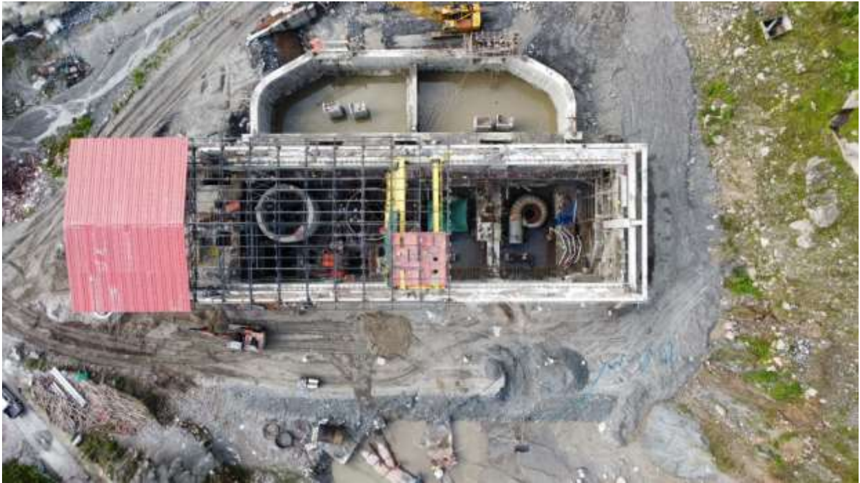
Figure 30: Top view of powerhouse
