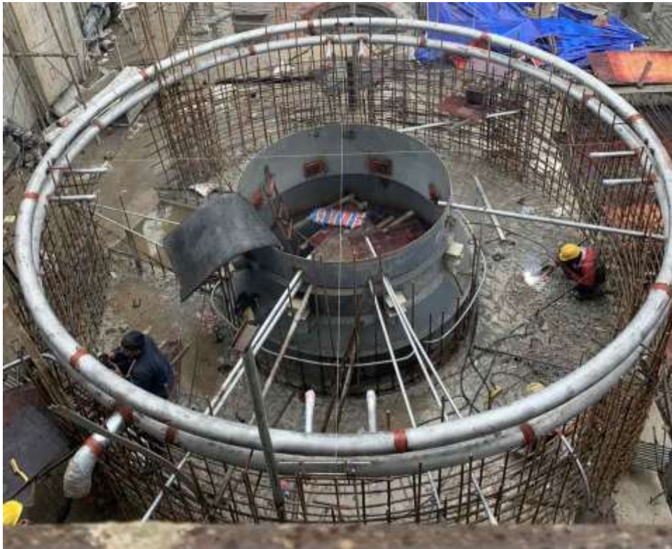
Figure 58: Installation of colling pipes for stator
