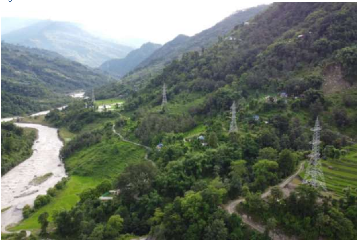
Figure 66: View of erected towers from right bank of Tamor
