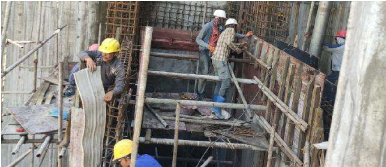
Figure 37: Installation of steel plates at trash passage
