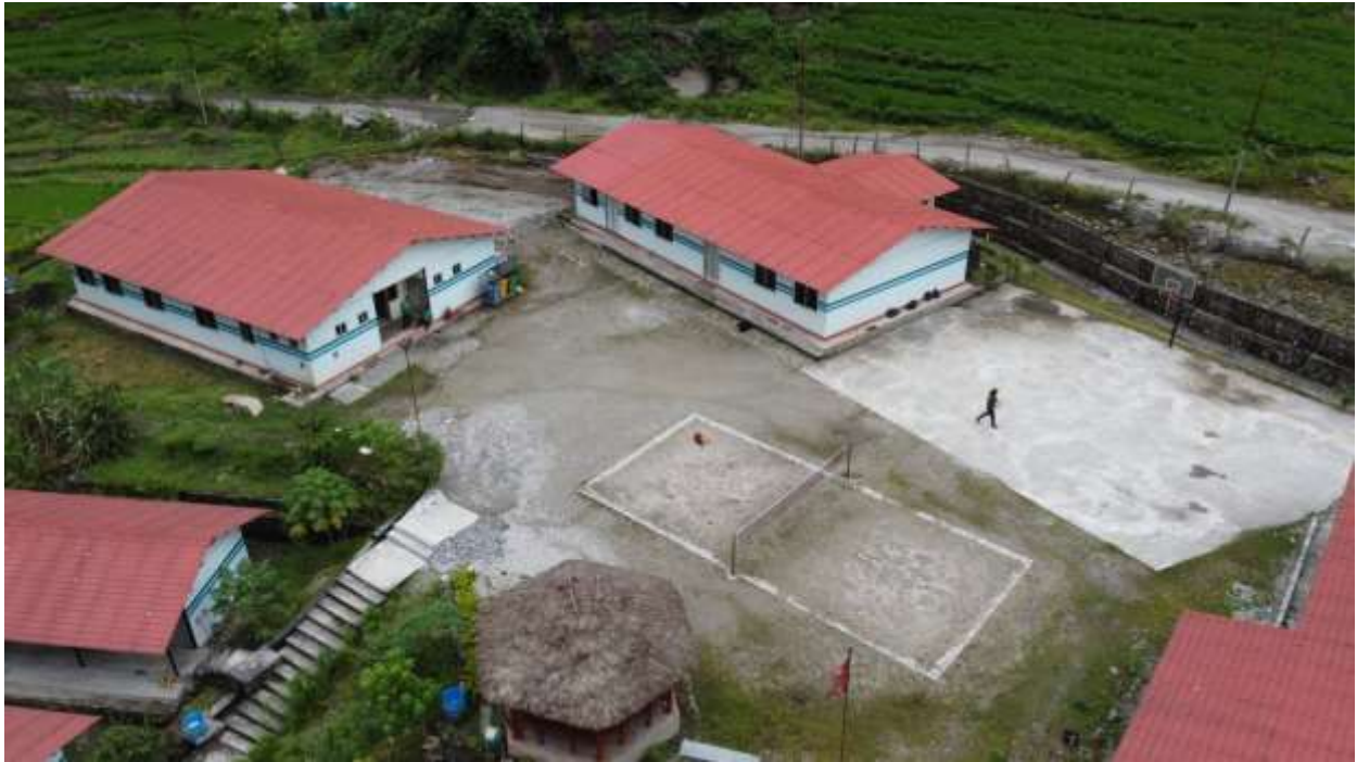
Figure 5: Employer's residential camp at Headworks (Simle)
