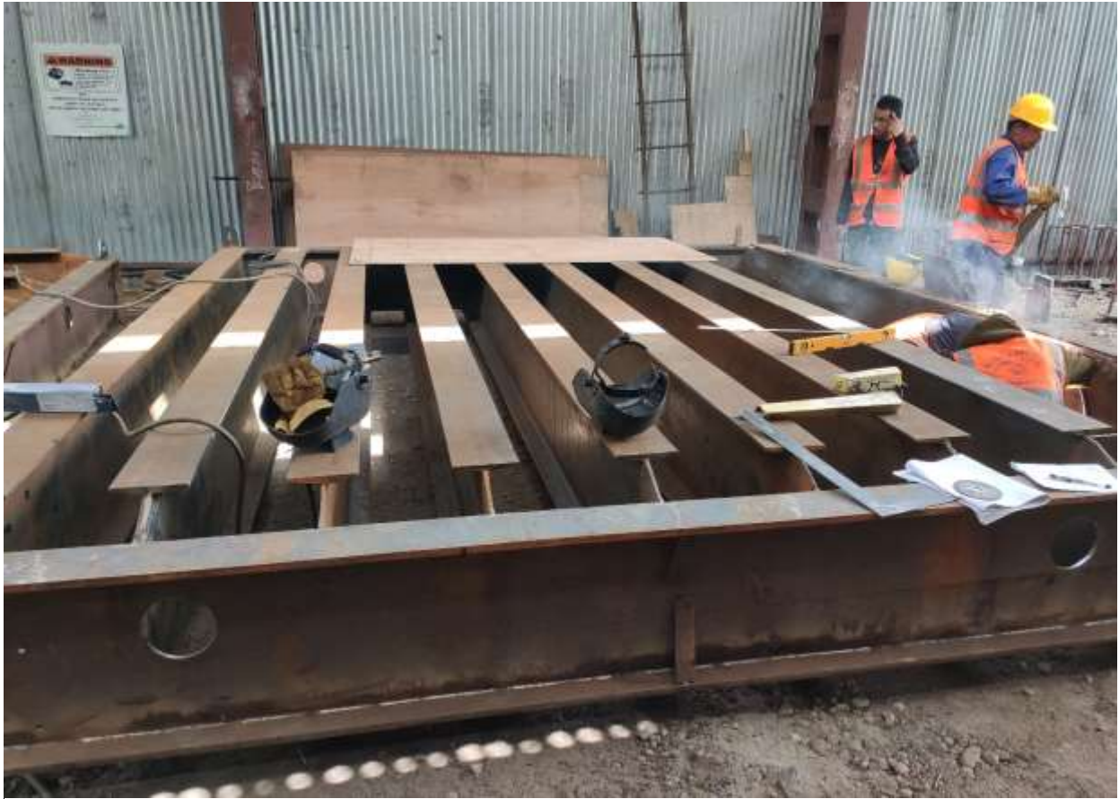
Figure 42: Fabrication of intake gate
