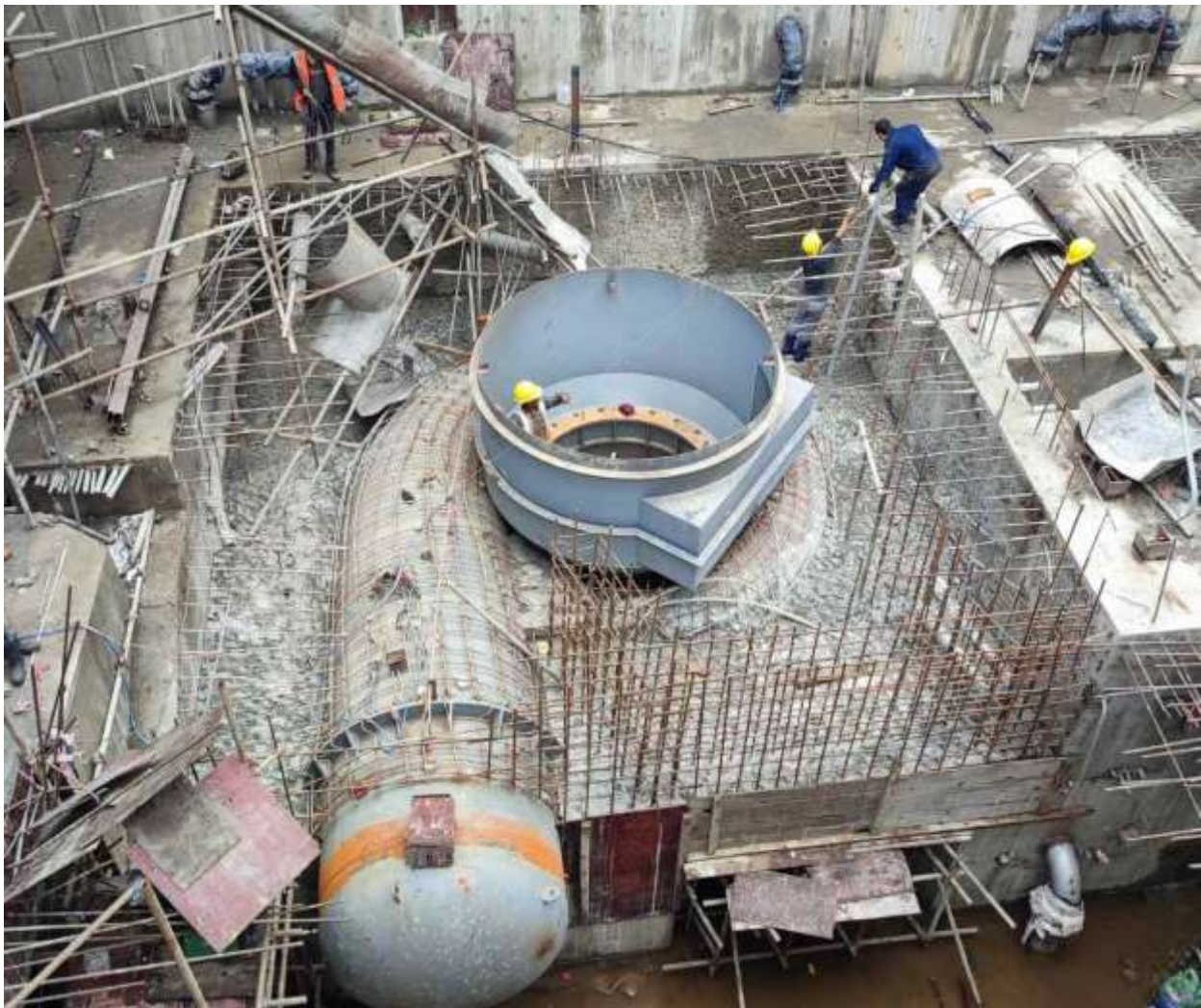
Figure 56: Installation of bottom part of Pit Liner at Unit 1
