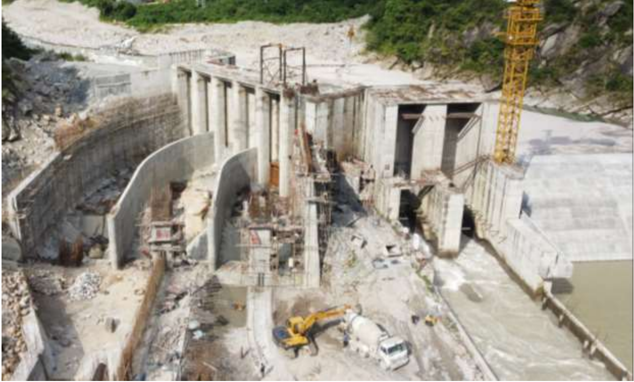
Figure 8: Intake and Undersluice section from downstream
