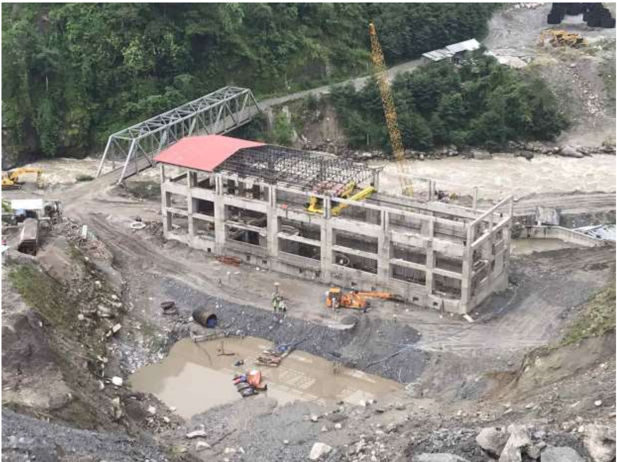
Figure 31: An aerial view of Powerhouse
