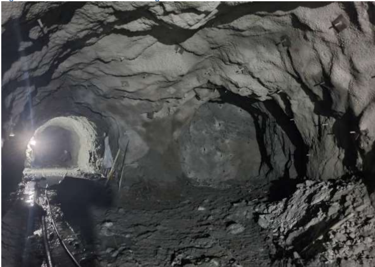
Figure 24: A view of Main Flushing Tunnel and first branch towards SB-01
