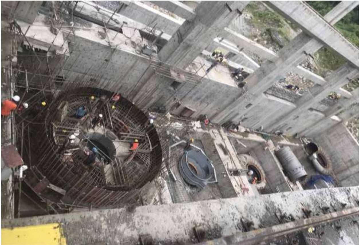
Figure 59: Installation of Pit liner at Unit 2
