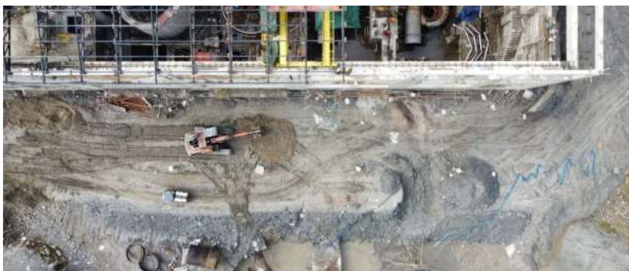
Figure 29: Backfilling works at manifold
