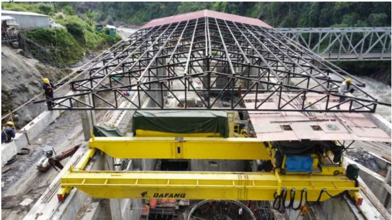
Figure 36: A view of truss installation works
