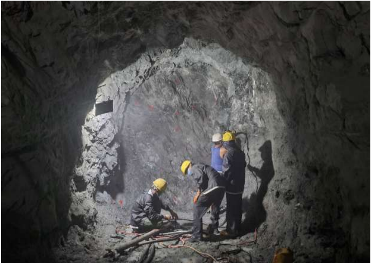
Figure 23: Excavation works at flushing tunnel
