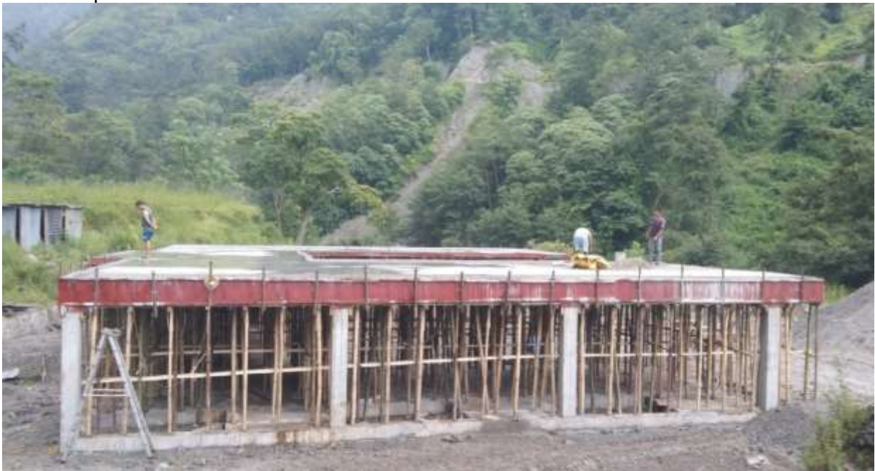
Figure 2: Concreting of first floor slab
