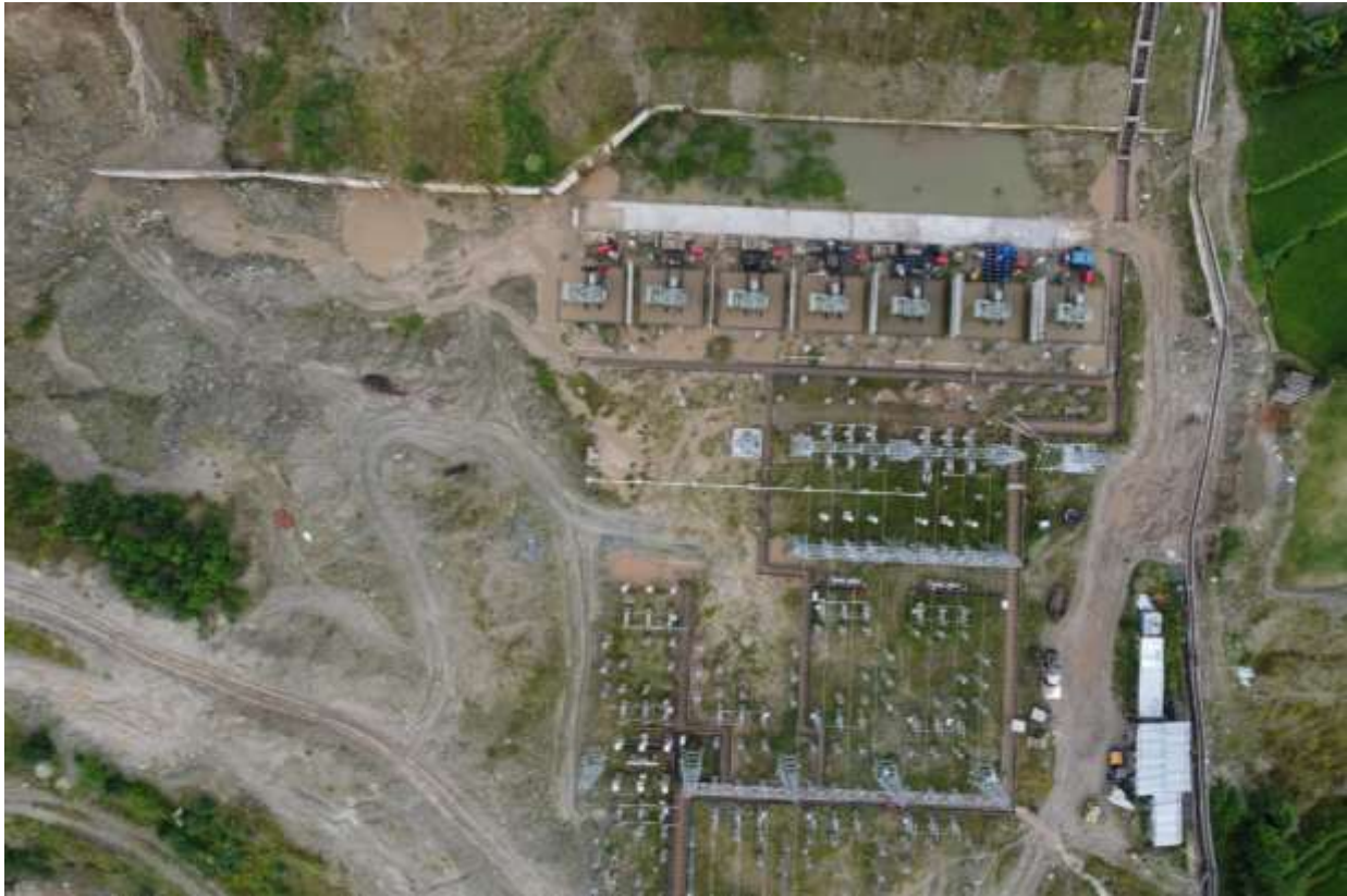
Figure 71: Interconnection bay at Dhunge-sanghu substation (NEA Project)
