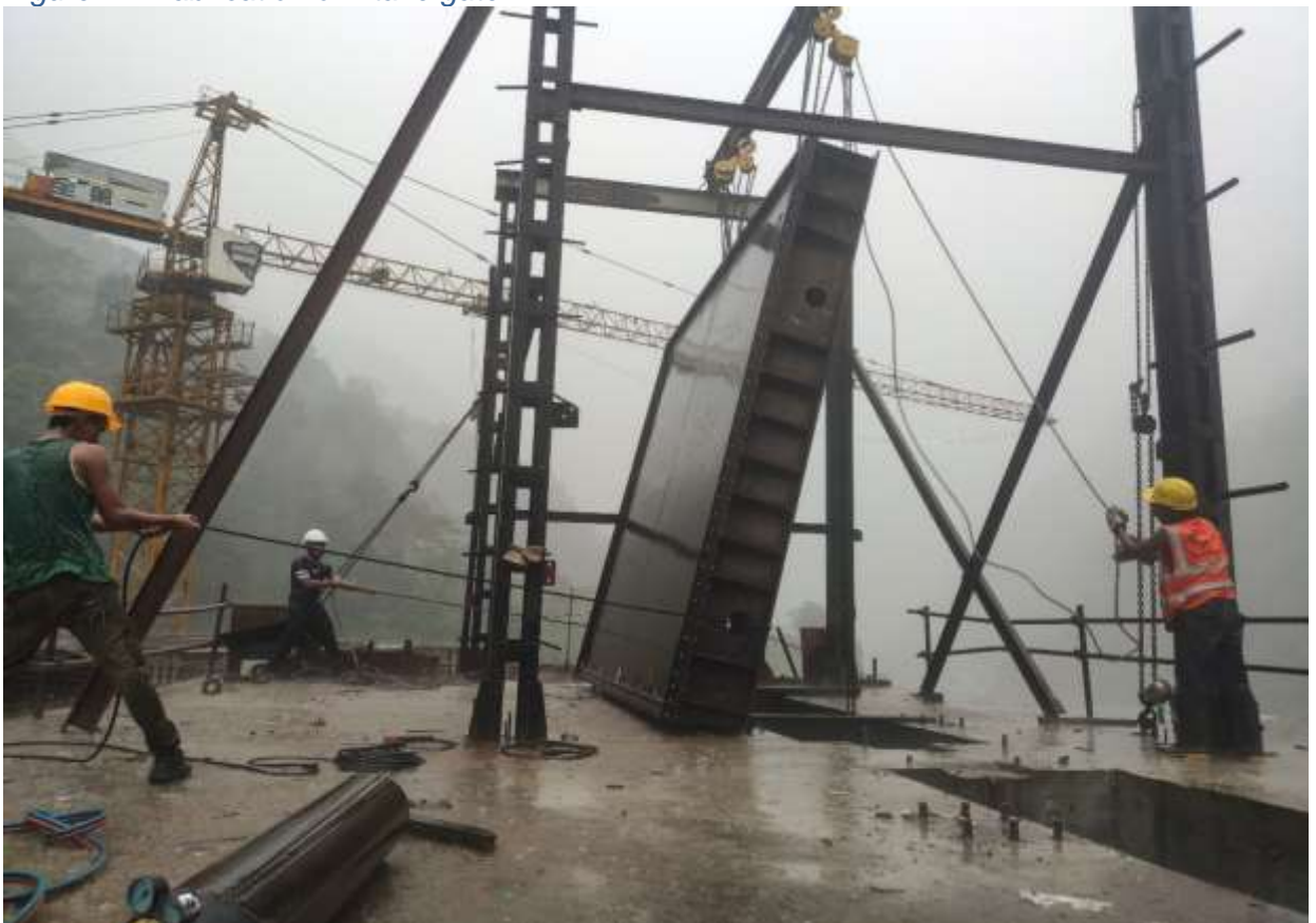
Figure 43: Lifting of intake gate Unit 2 for erection
