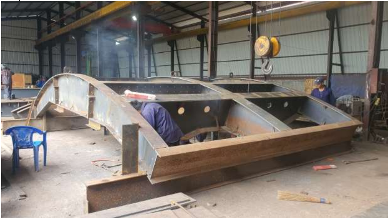
Figure 41: Fabrication of radial gates
