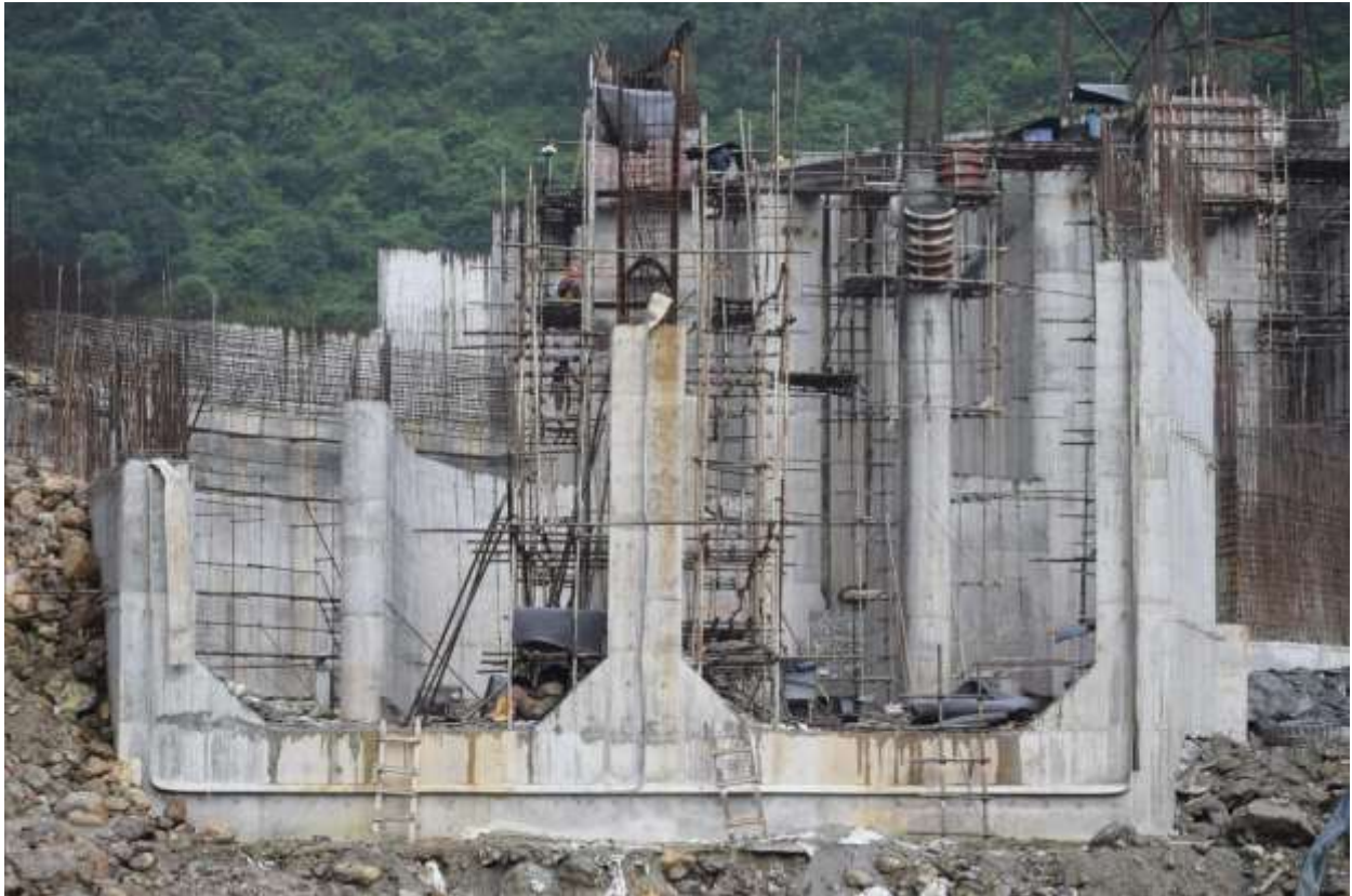
Figure 12: A view of conveyance tank from downstream
