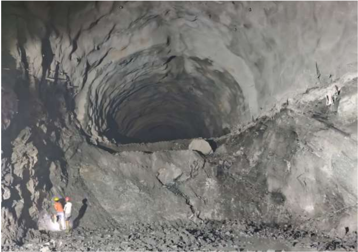
Figure 25: A view of excavation of Settling basin 01
