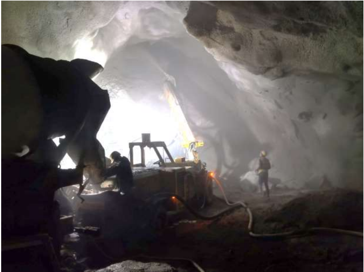
Figure 27: Shotcreting works at Settling Basin 03
