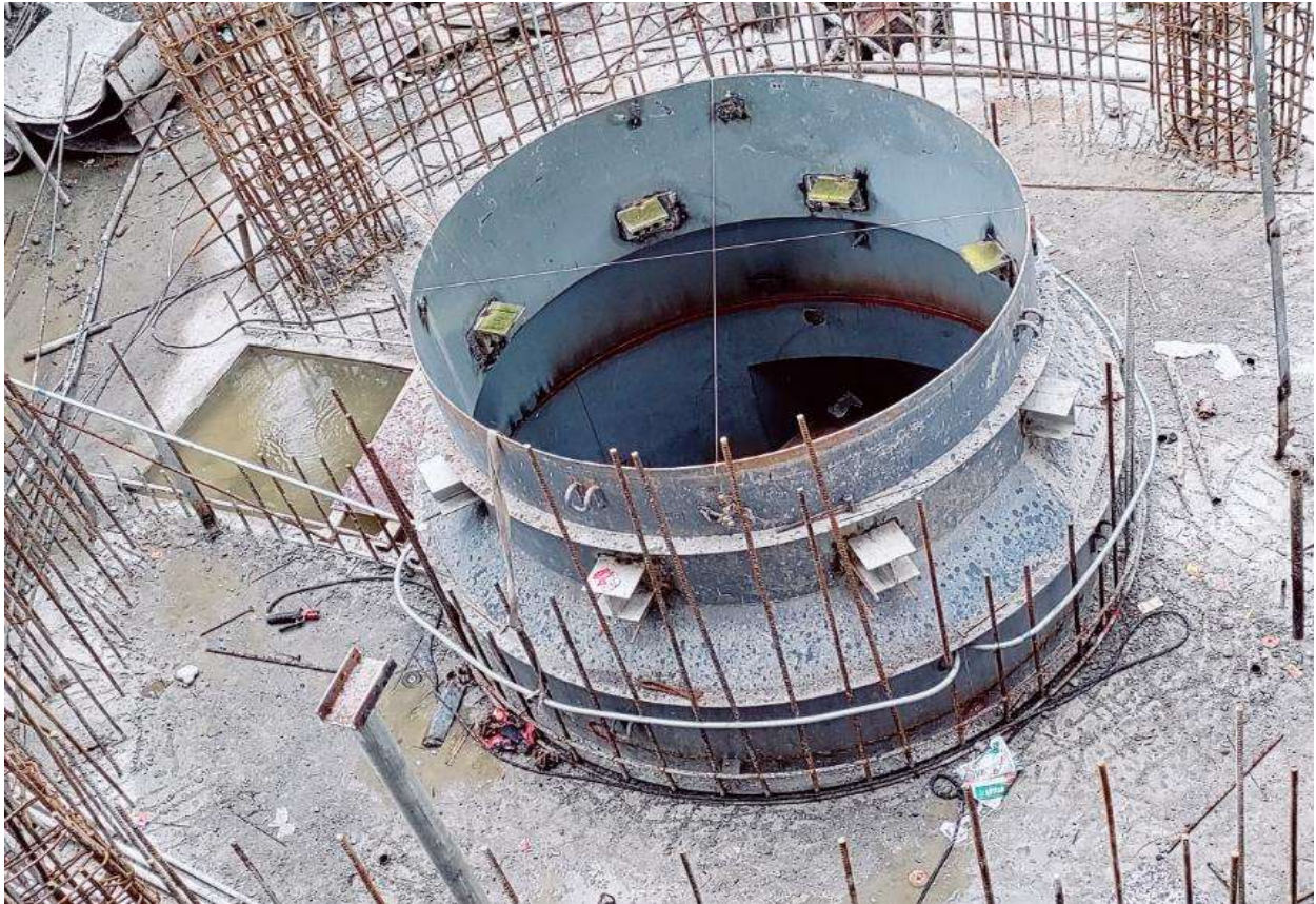
Figure 57: View of Pitliner after third lift concrete
