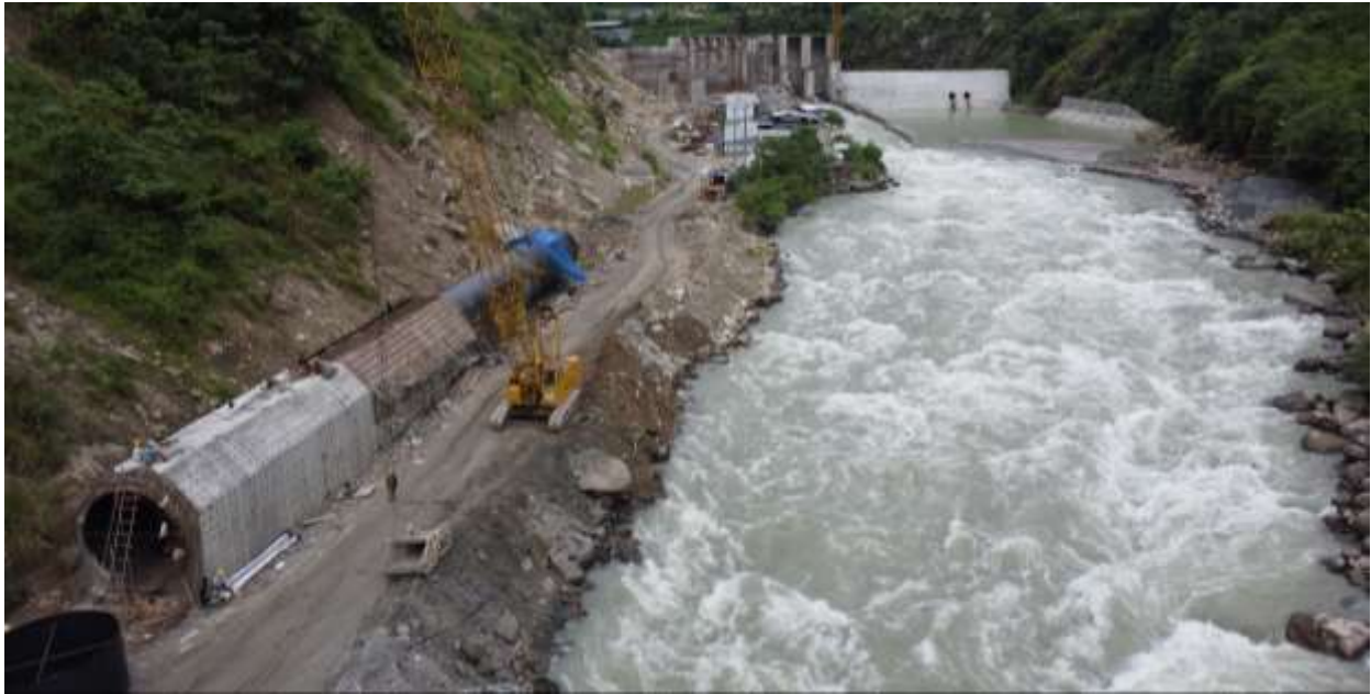
Figure 38: Installation of approach pipe
