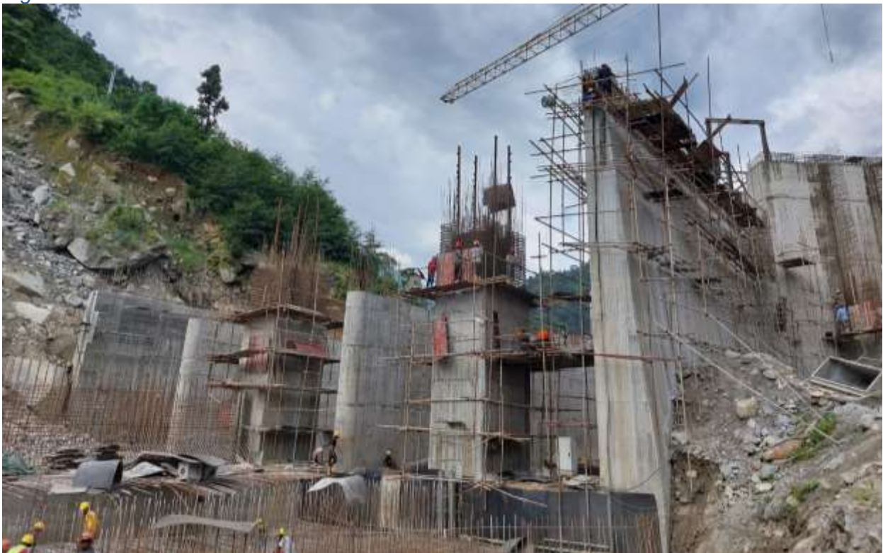
Figure 9: Rebar and concrete works in gravel trap exit piers
