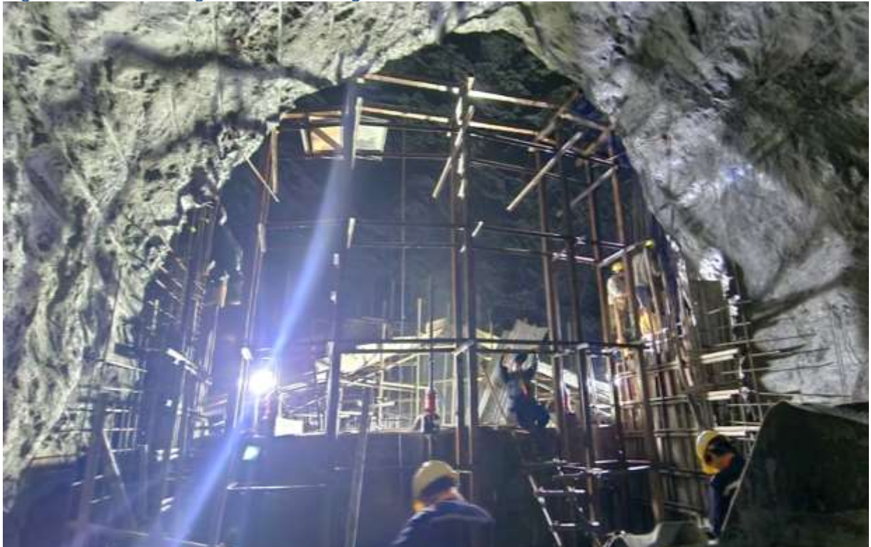
Figure 28: Formwork instalation for the concreting of surge shaft
