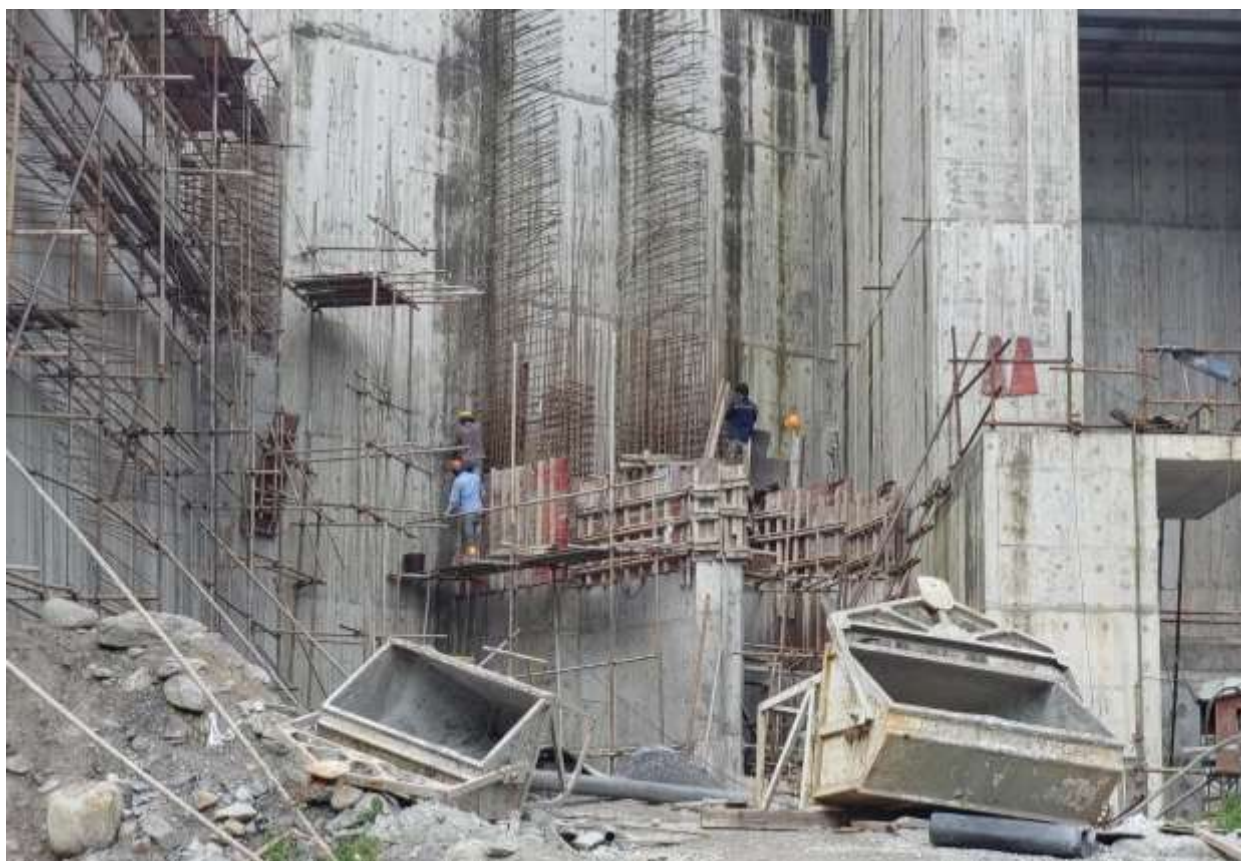
Figure 10: A view of concreting works at trash passage
