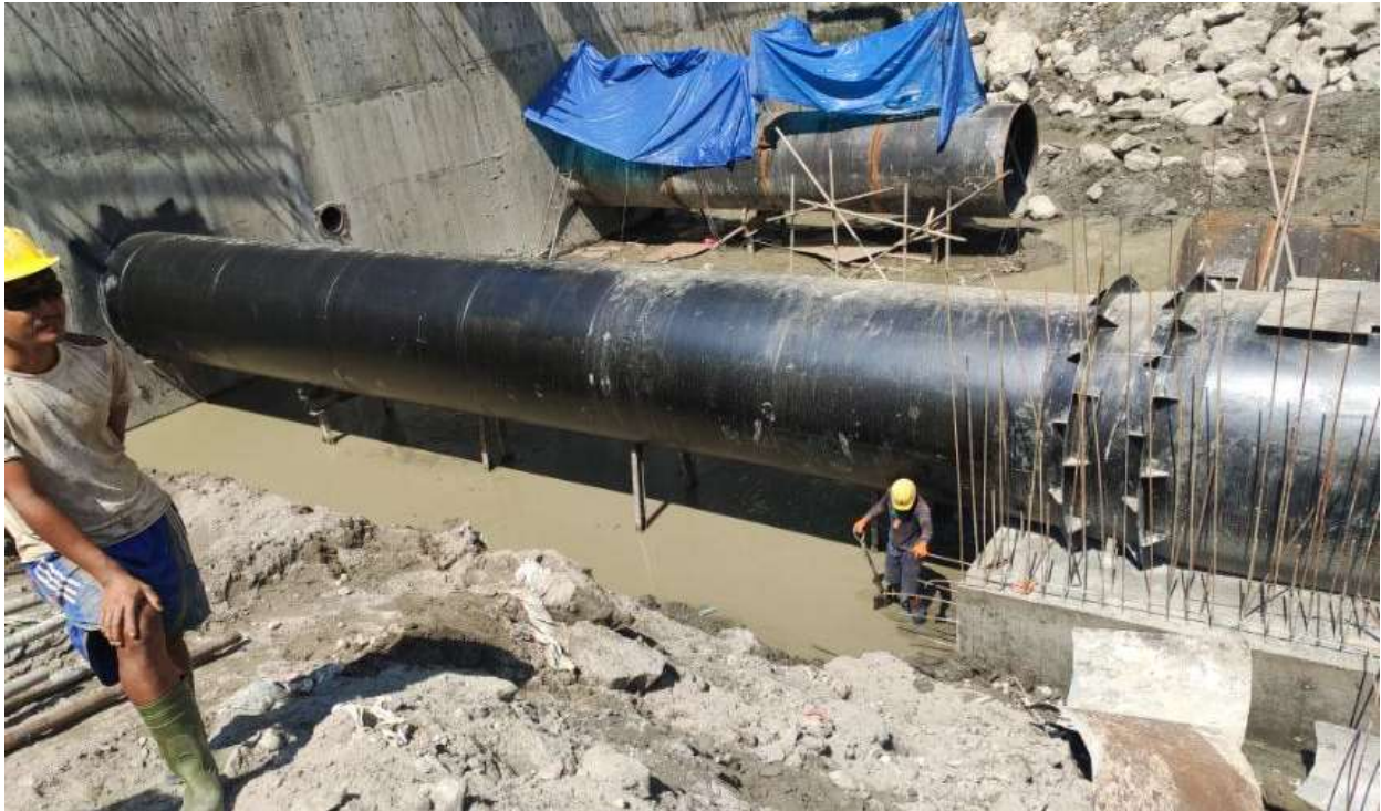
Figure 40: A view of brach pipe of penstock installation
