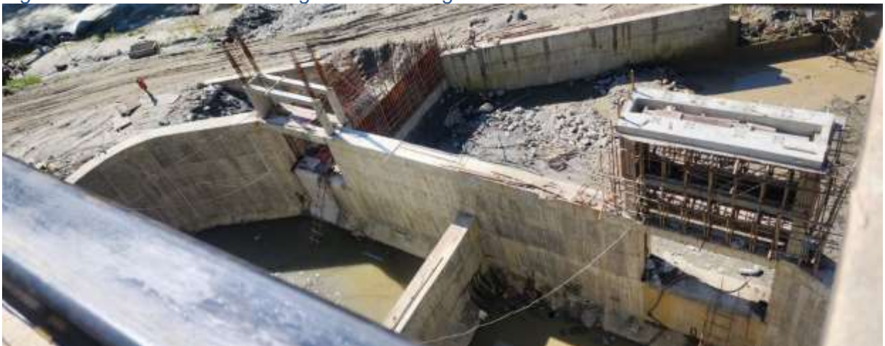
Figure 34: Concreting works for tailrace culvert
