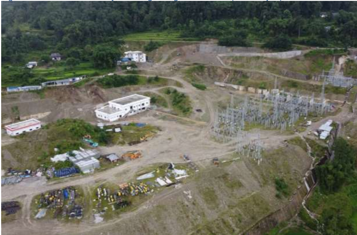
Figure 72: An aerial view of Dhunge-sanghu substation (NEA Project)
