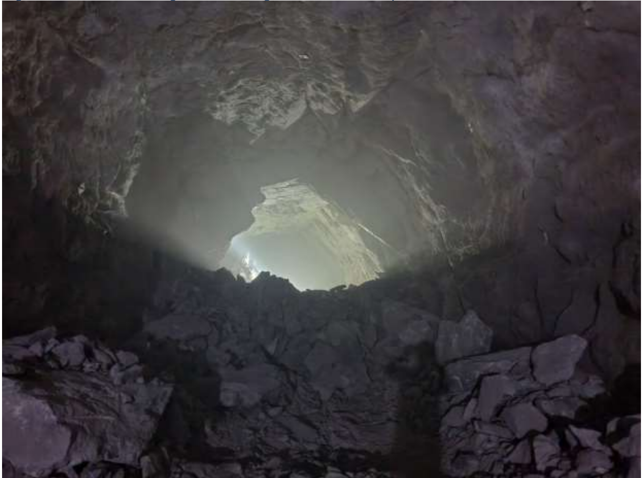
Figure 18: A view of HRT breakthrough at chainage 1+545.37
