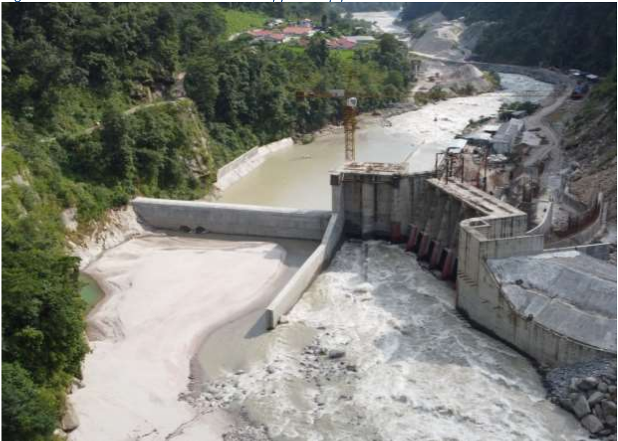
Figure 15: Main weir body (Completed)
