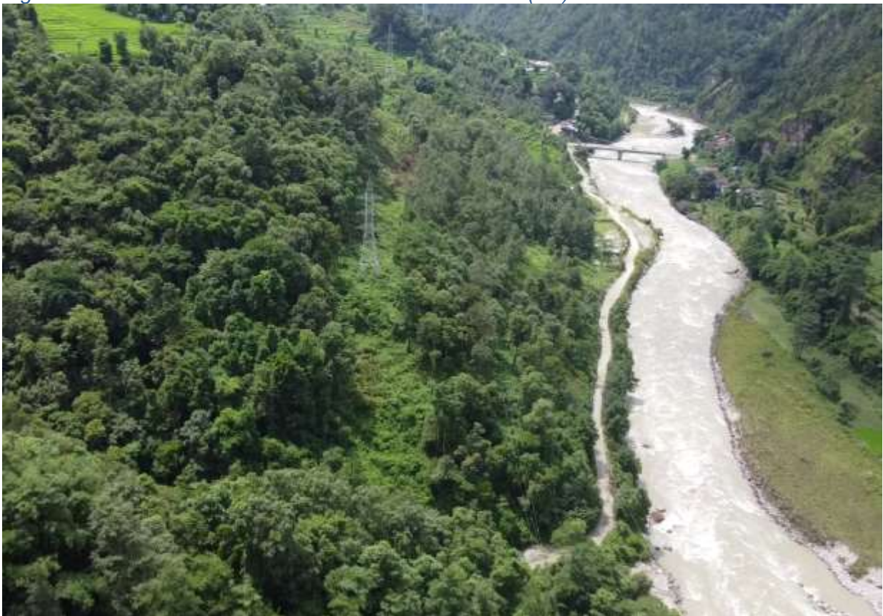
Figure 70: A view of RoW clearance
