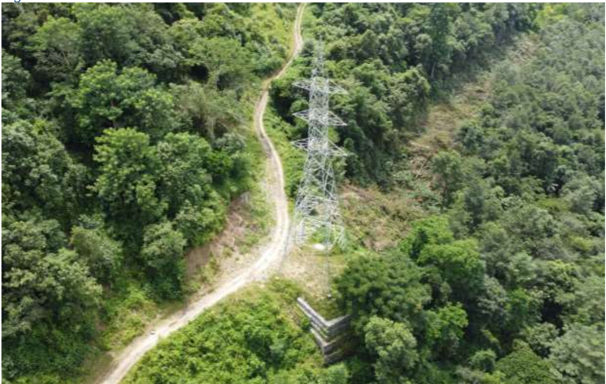
Figure 68: A view of AP10 along with protection works
