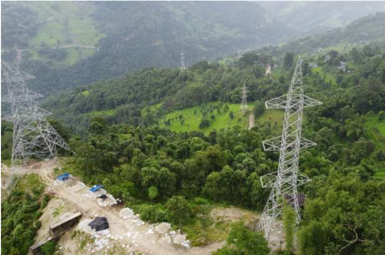
Figure 69: Erected last tower at AP24 and tower of NEA (left)
