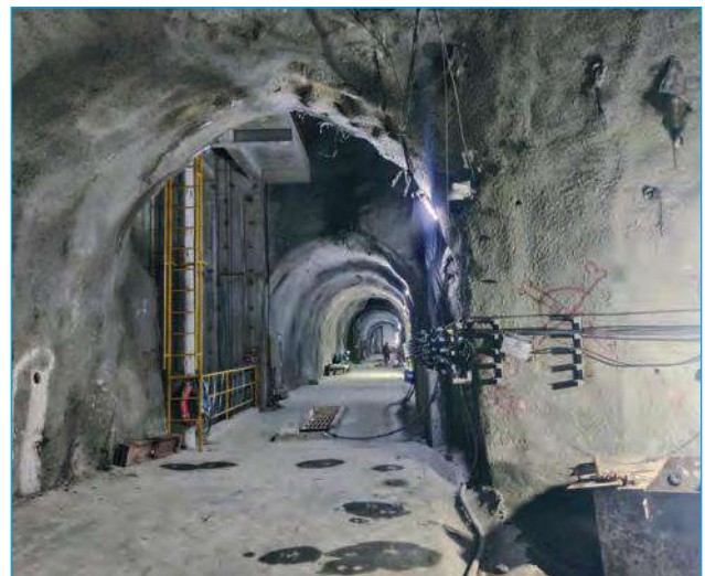
Underground Inspection Tunnel
