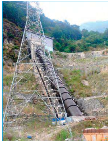
Penstock Slope Protection Works
