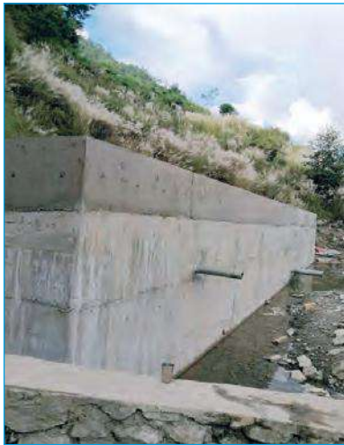
Fire Fighting Water Tank
