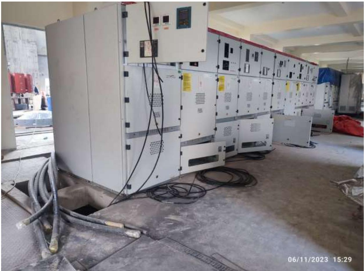
Figure 2-68: Laying of power and control cables in 11kV switchgear room
