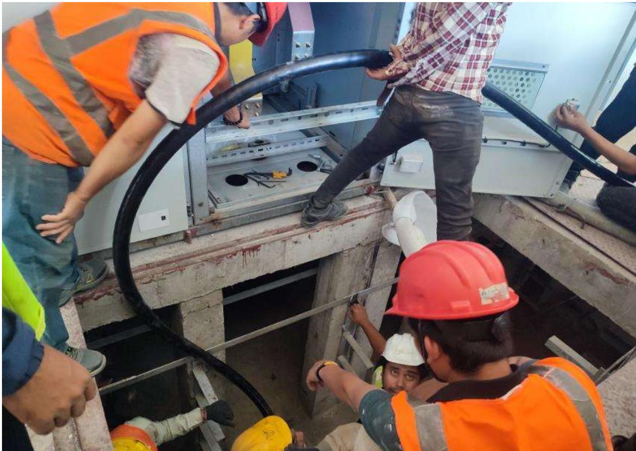
Figure 2-64: Laying of power cables in 11KV switch gear room
