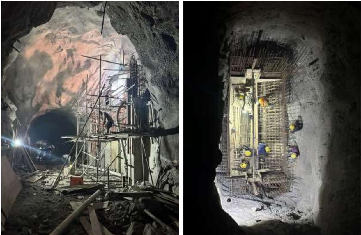
Figure 2-18: Concreting at Inlet gate shaft 01 (left) and Inlet gate shaft 02 (right)
