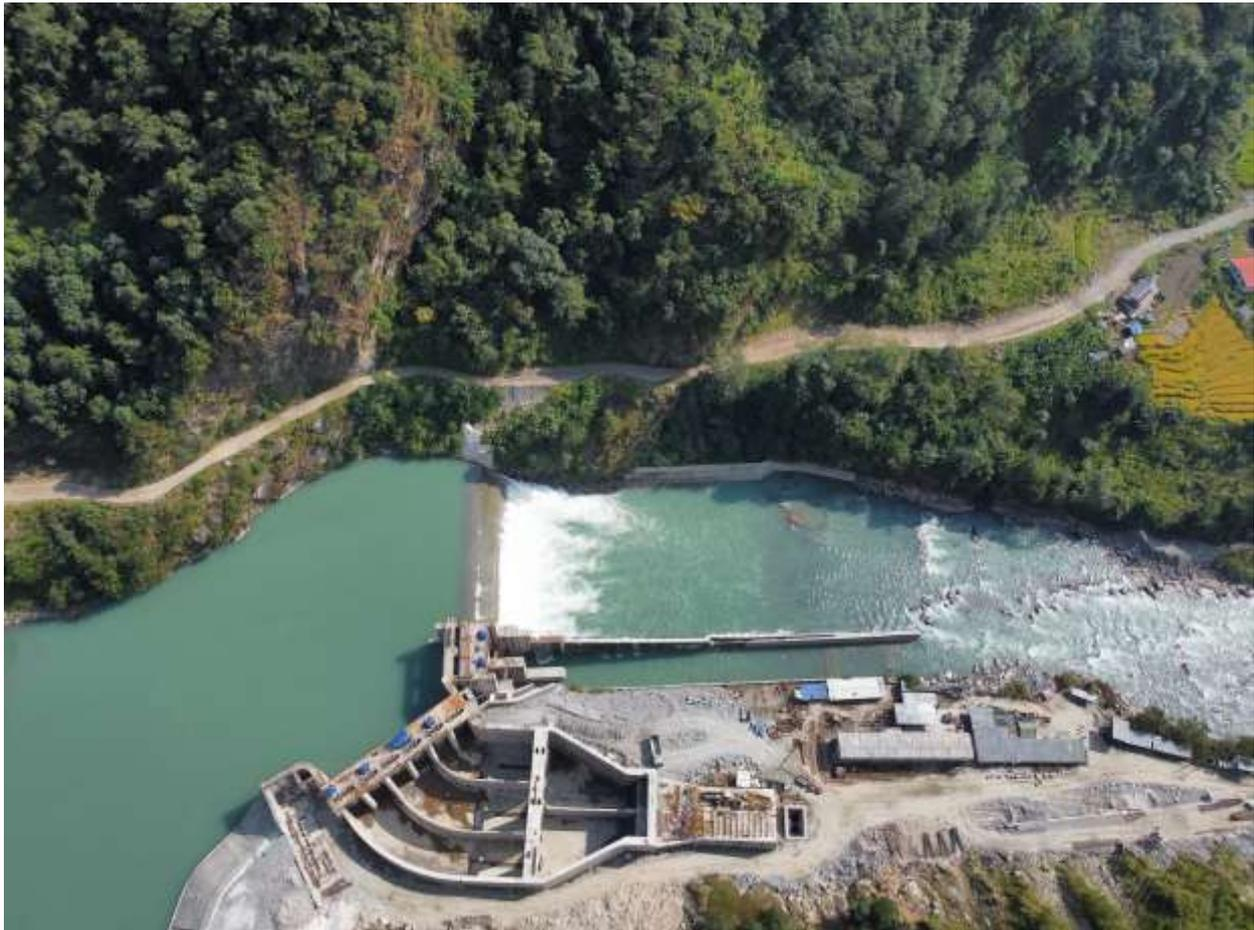
Figure 2-6: An aerial view of weir during monsoon water flow over the ogee crest
