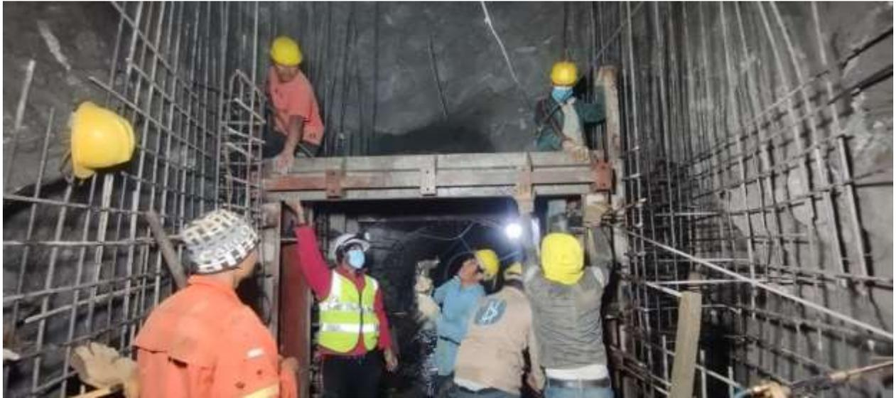
Figure 2-34: Erection of embedded parts of settling basin flushing gate and stoplog at SBF-5
