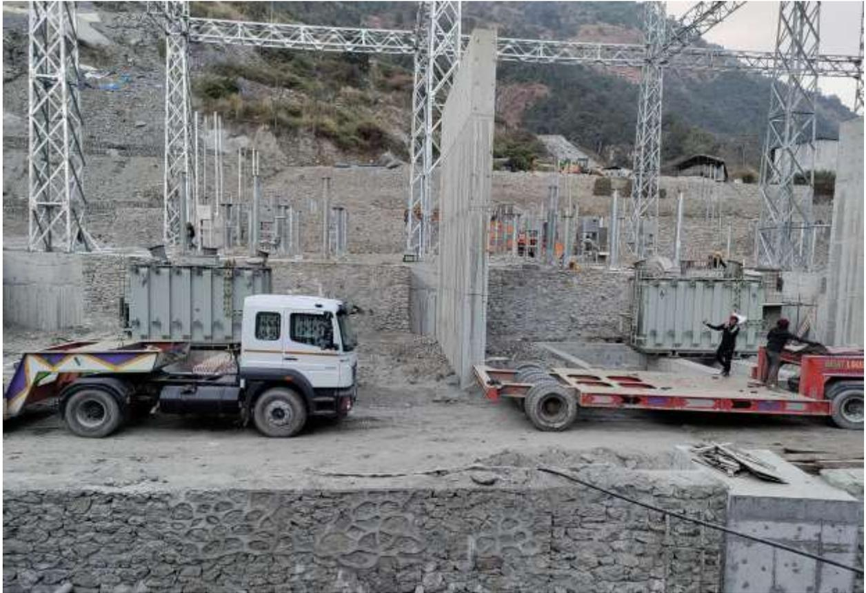
Figure 2-71: Unloading of power transformers at the switchyard region
