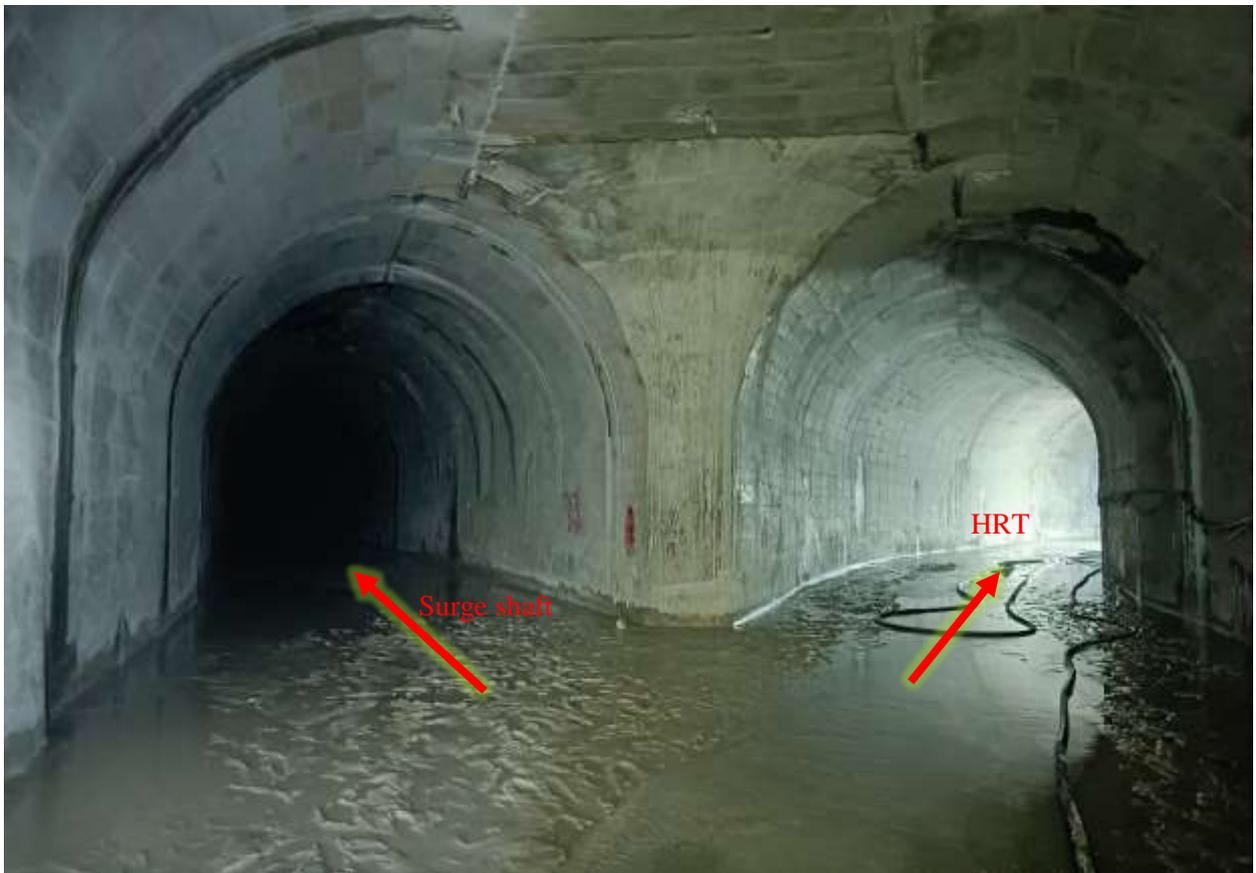
Figure 2-27: Full concrete lining at the junction of connecting tunnel and HRT
