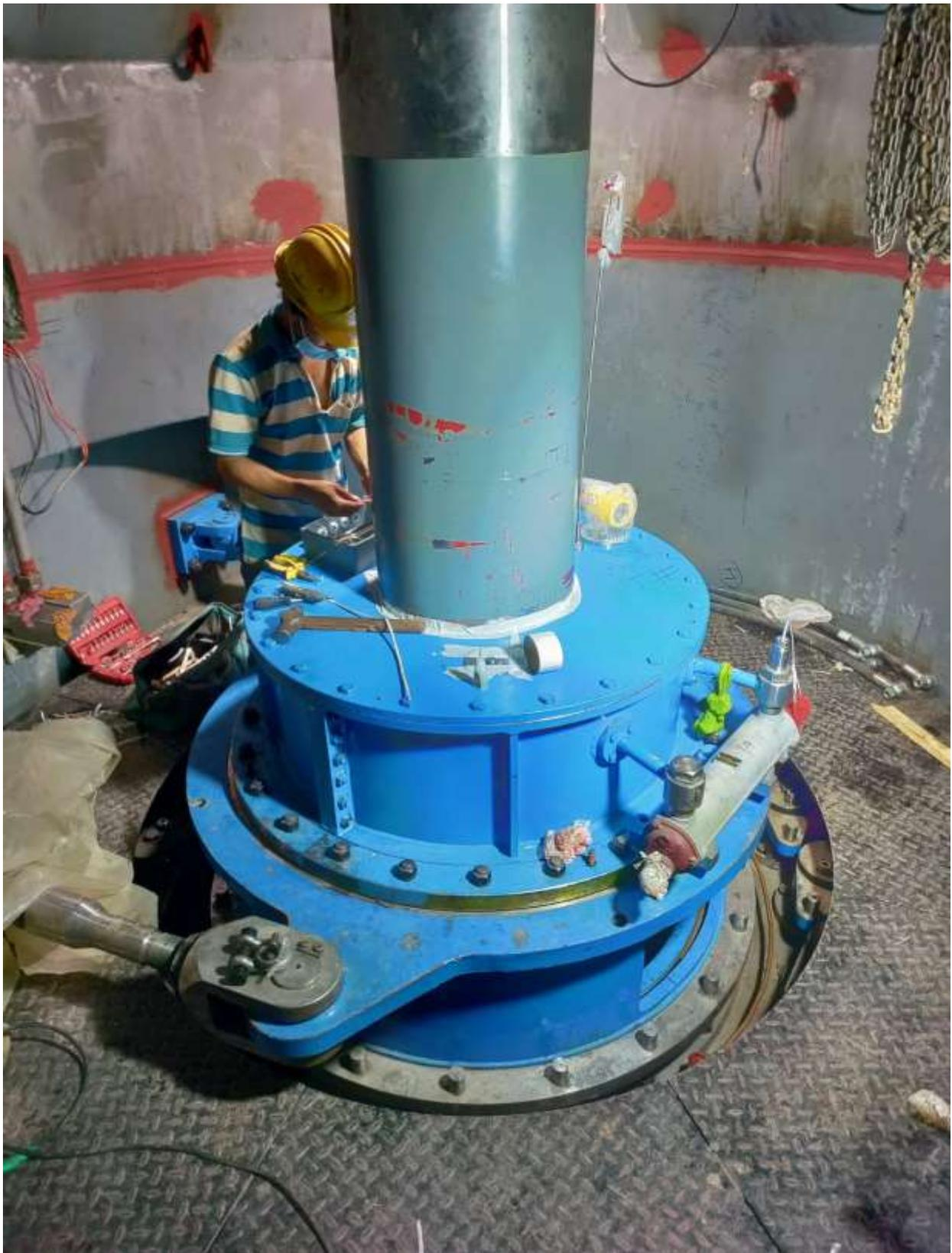
Figure 2-52: Final installation of turbine guide bearing and water regulating mechanism
