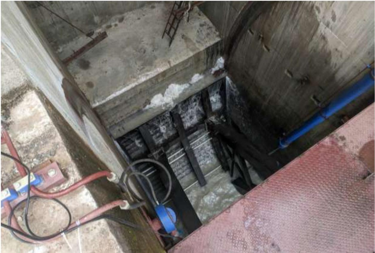
Figure 2-41: Erection of radial gate at unders luice
