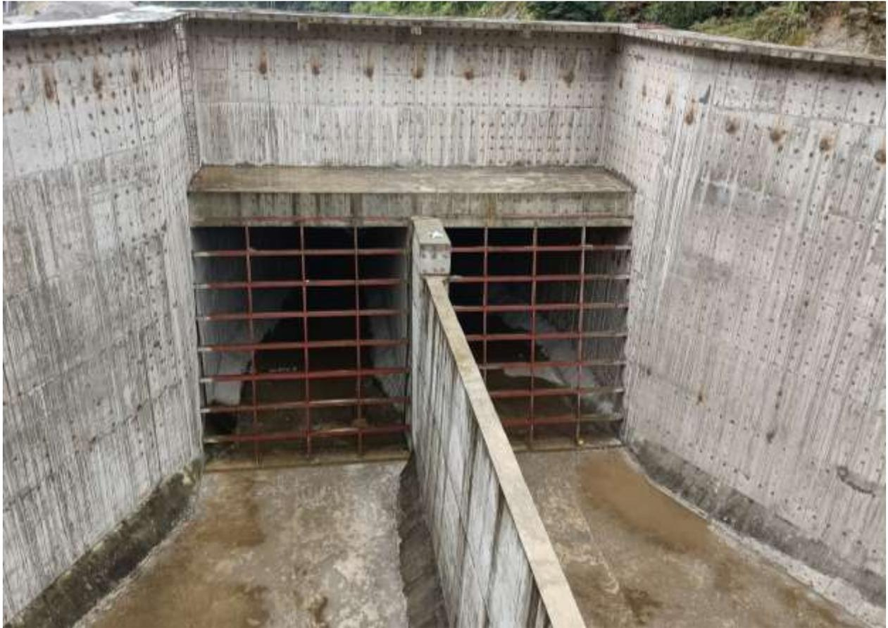
Figure 2-36: Installation of trash rack at the conveyance tank region
