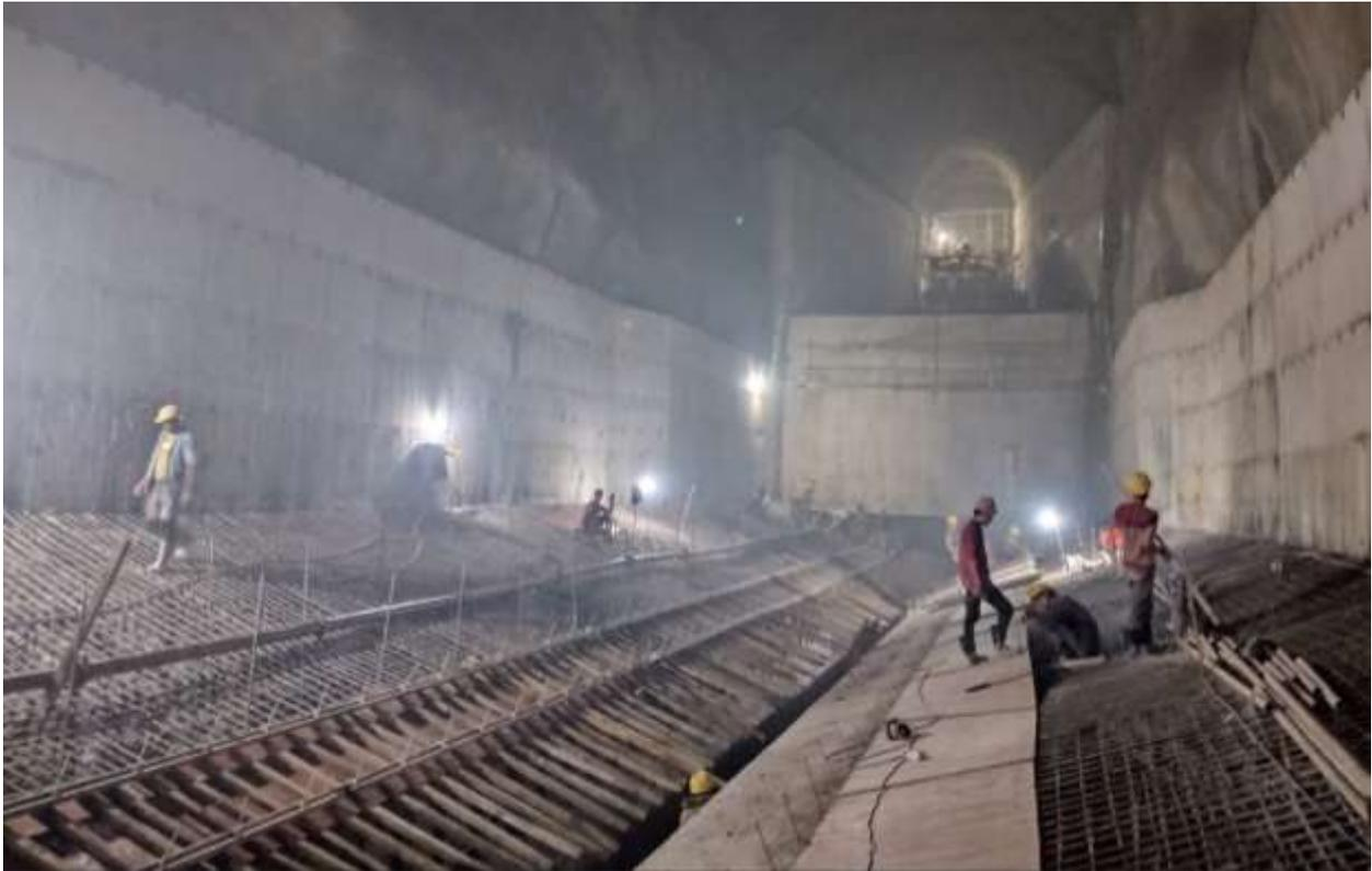
Figure 2-15: A view of SB 03 during installation of final lining wiremesh shotcrete
