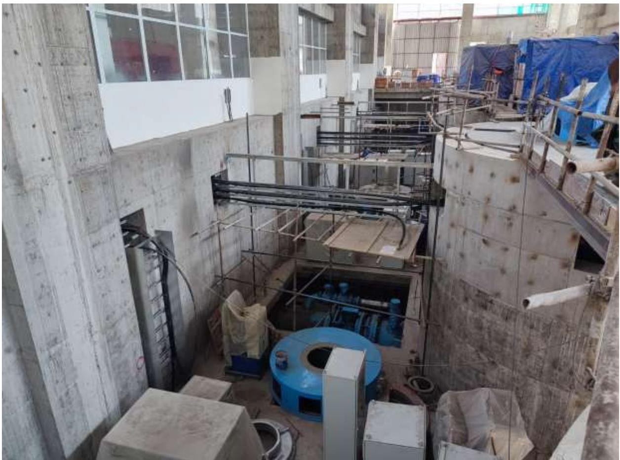
Figure 2-66: Laying of power and control cables in main powerhouse
