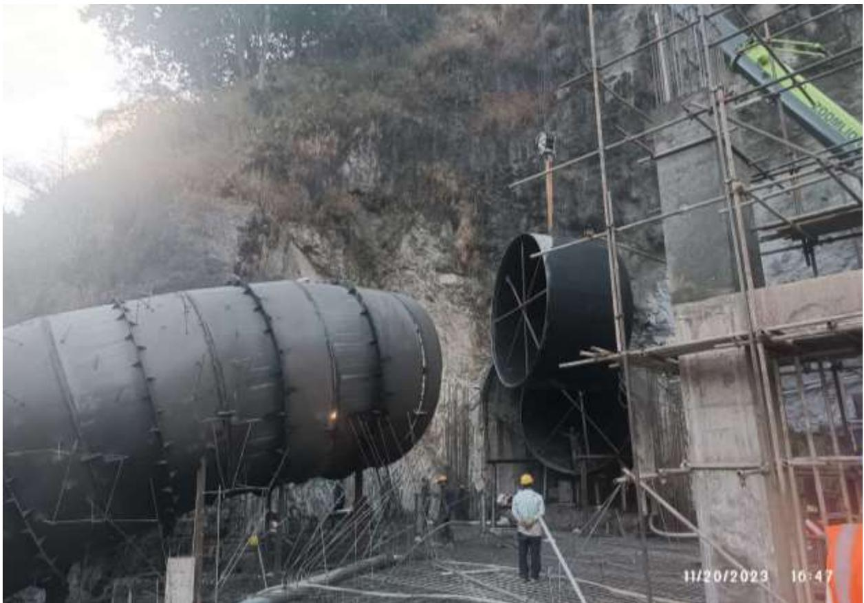
Figure 2-40: Erection of final piece of penstock pipe from HRT outlet region
