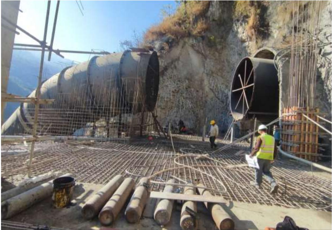
Figure 2-73: Earthing plates and drainage pipes embedded of valve house
