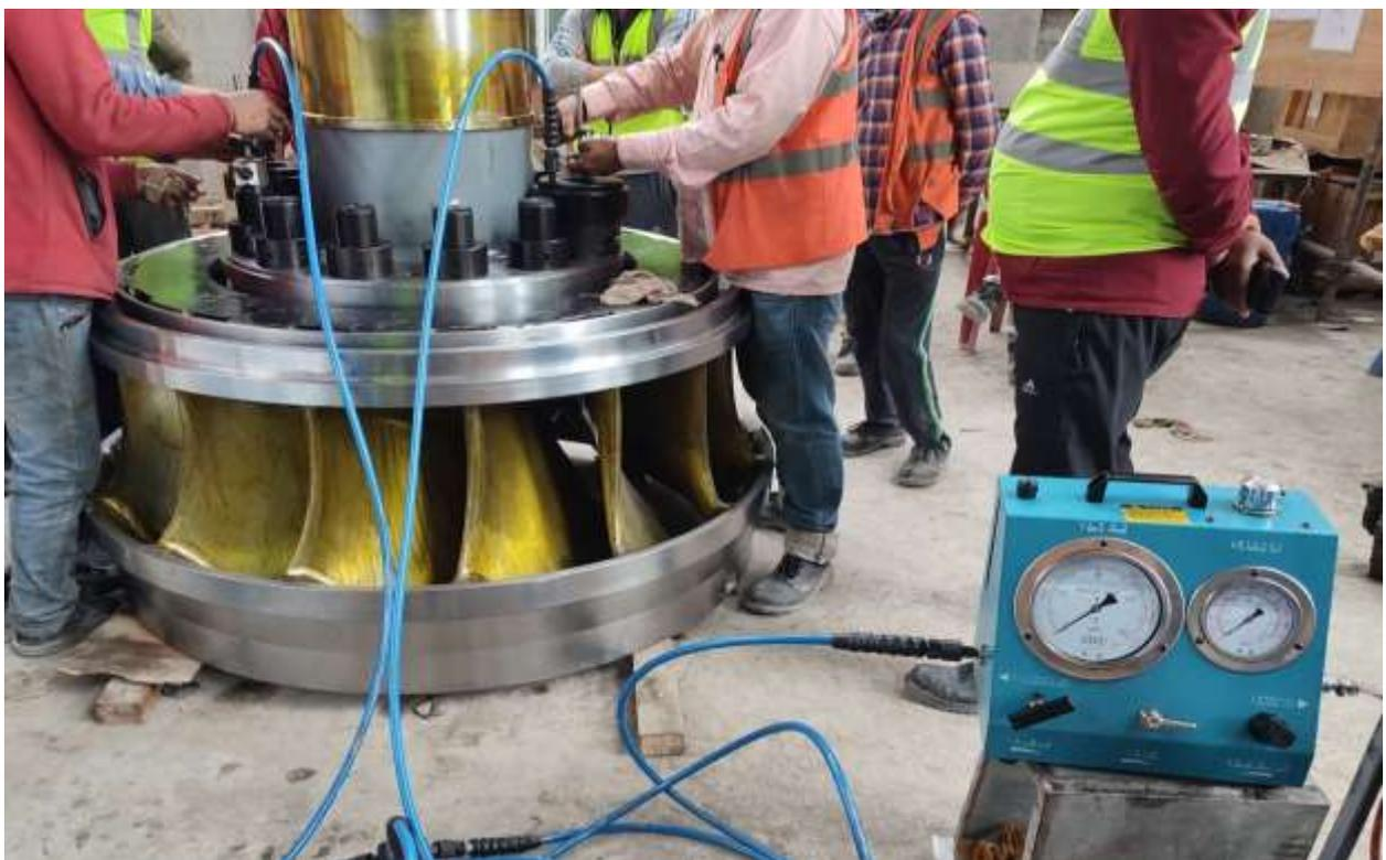
Figure 2-54: Assembly of runner with main shaft
