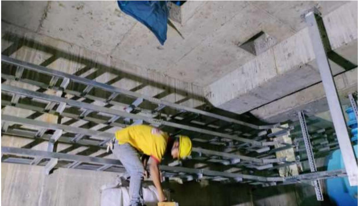
Figure 2-67: Cable tray work under the floor slab of turbine floor
