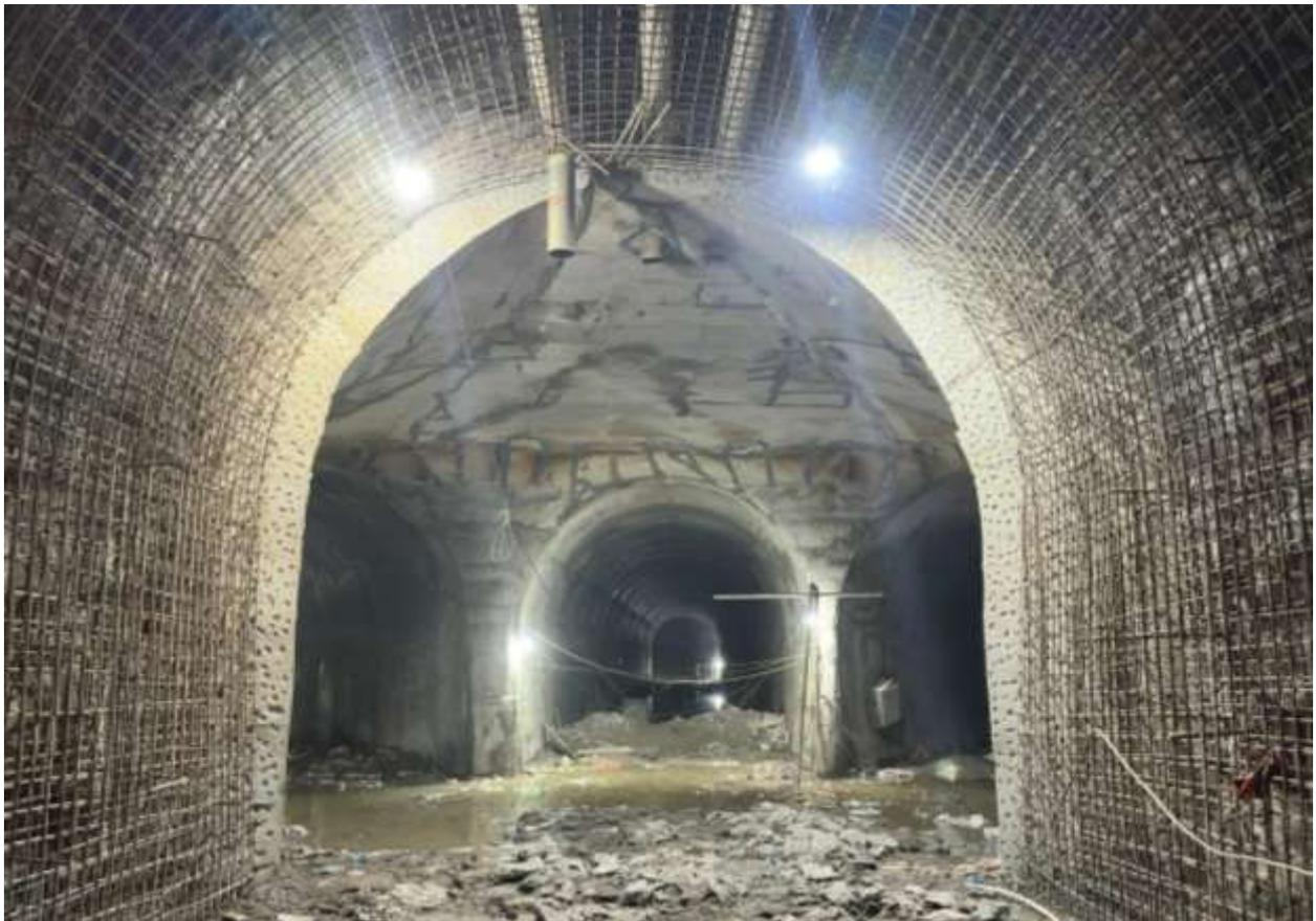
Figure 2-18: Rebar installation at the HRT region
