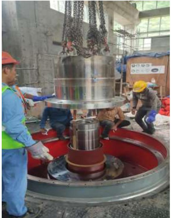
Figure 2-51: Different stages of thrust bearing installation
