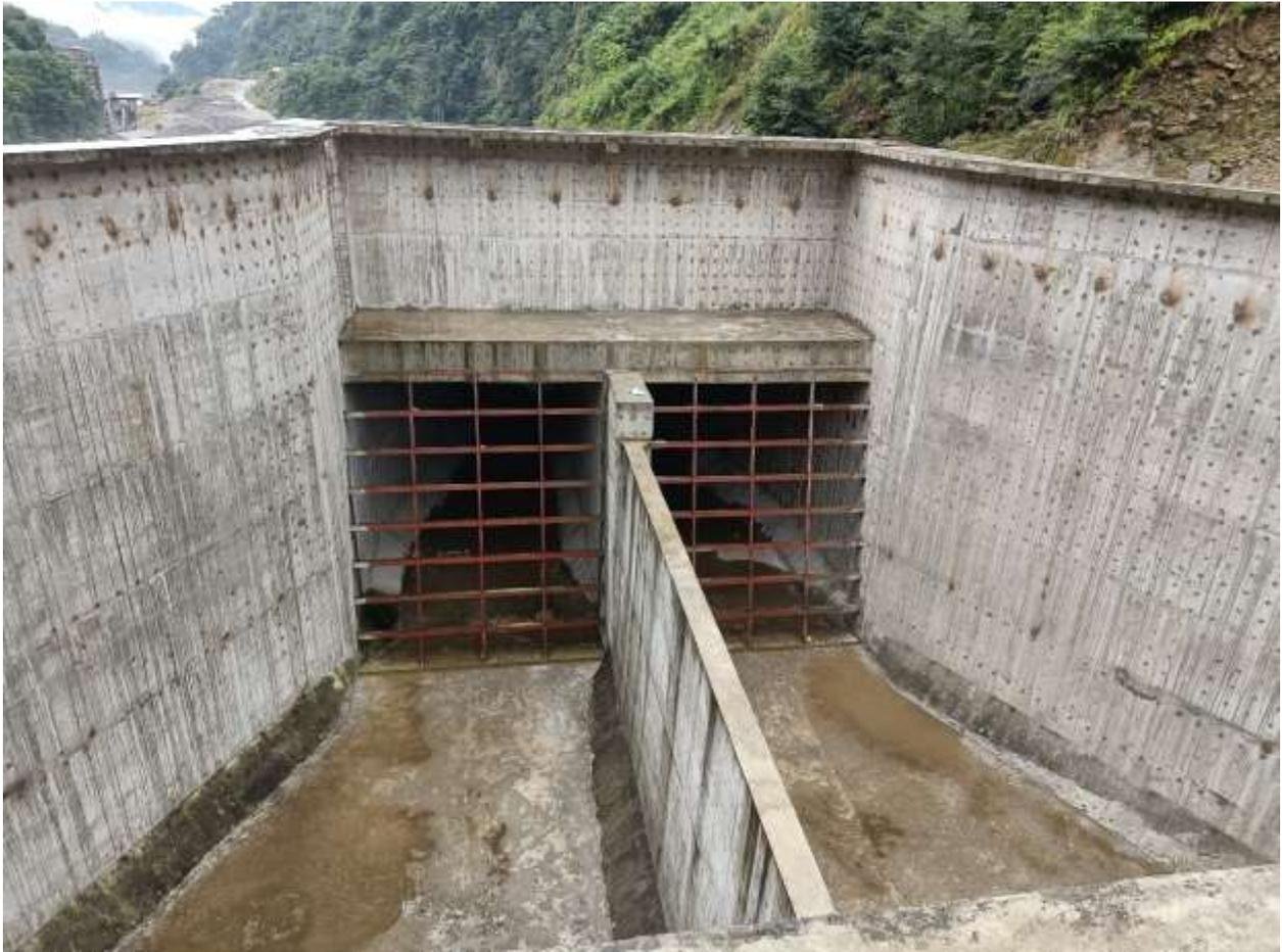
Figure 2-8: A view of conveyance tank
