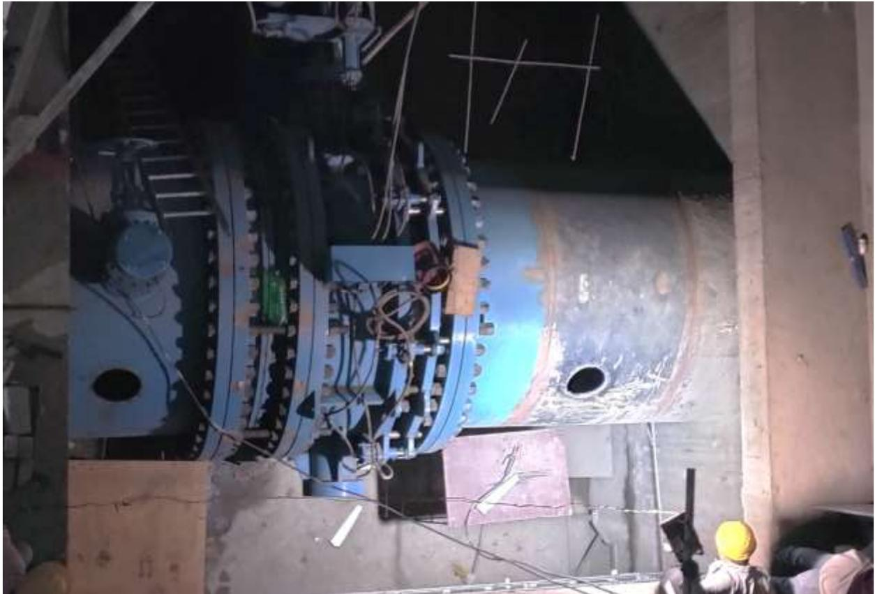
Figure 2-60: Unit 03 preparation for bypass valve erection
