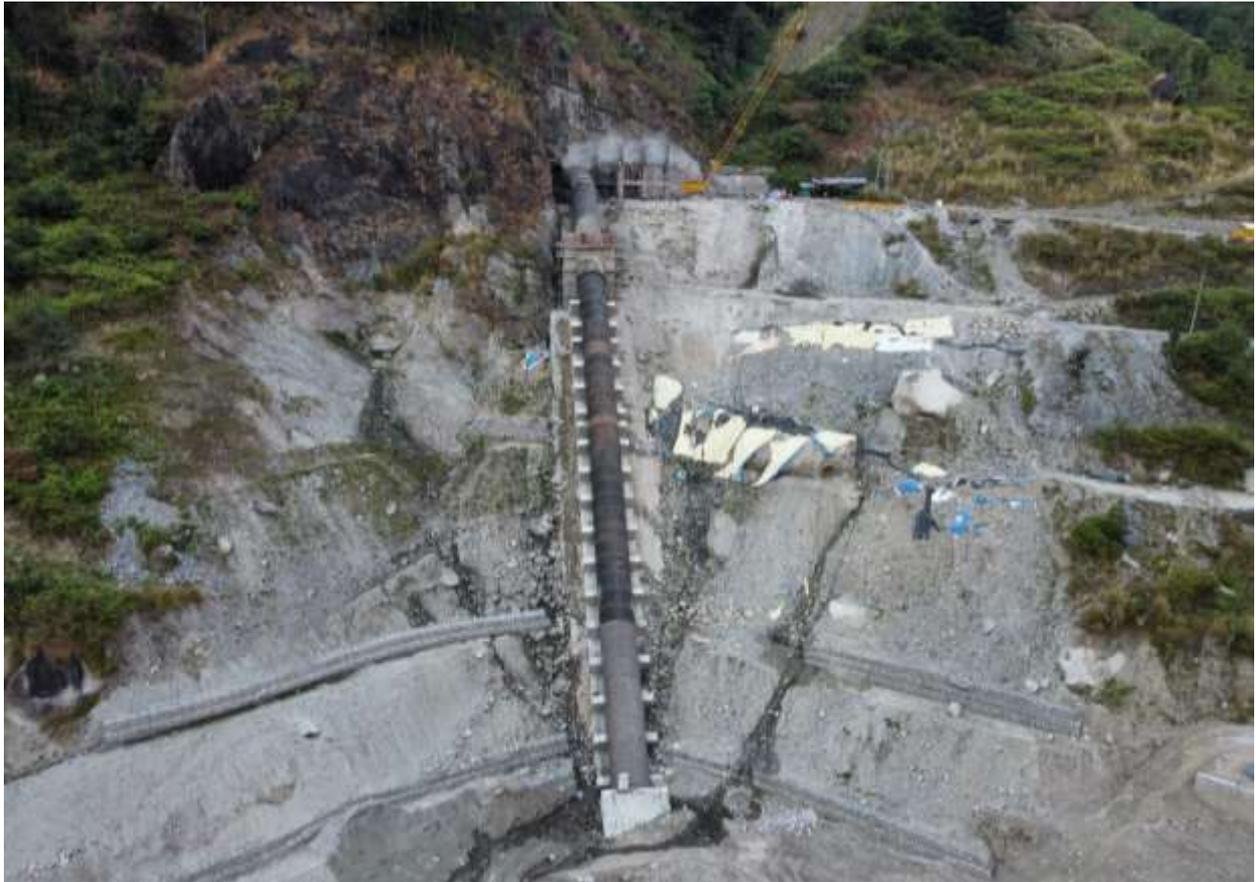
Figure 2-39: Erection of penstock pipes
