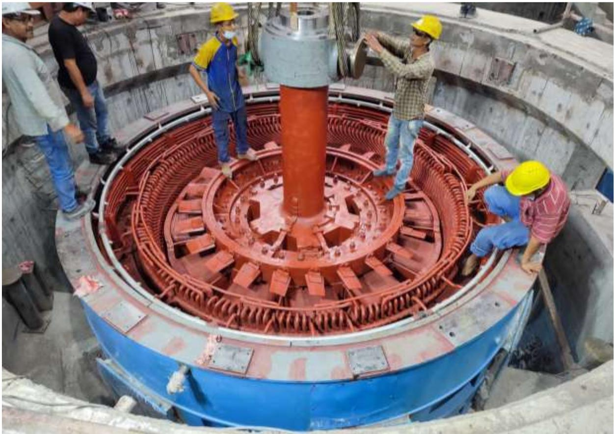
Figure 2-45: Rotor and stator coupling in unit 01
