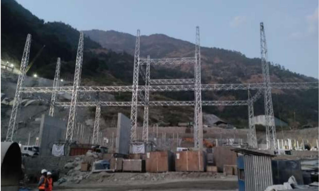
Figure 2-69: Overview of gantry tower erection
