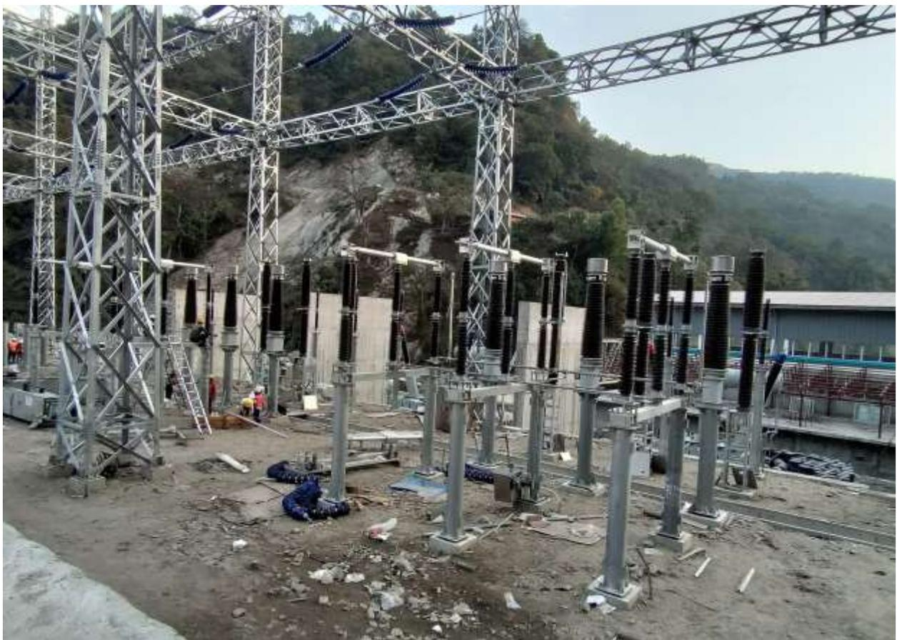
Figure 2-72: Erection of gantry towers at switchyard
