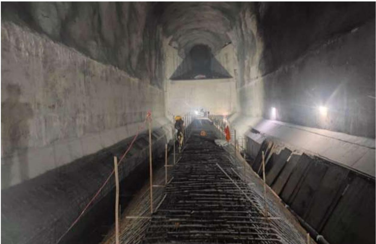
Figure 2-11: A view of SB 01 with completed wall lining and hopper concreting
