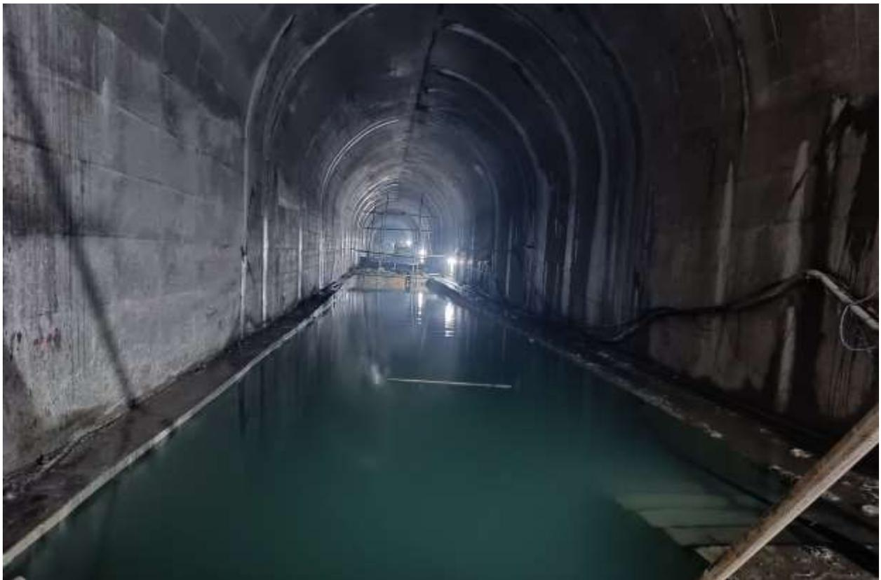
Figure 2-20: A completed section of concrete lining works at rock trap
