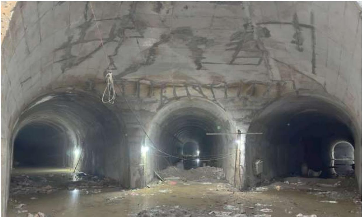
Figure 2-16: Full lining concrete at connecting tunnel junction
