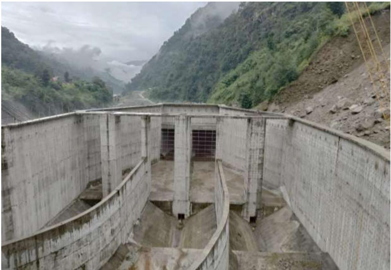
Figure 2-5: A view of gravel trap and conveyance tank from upstream
