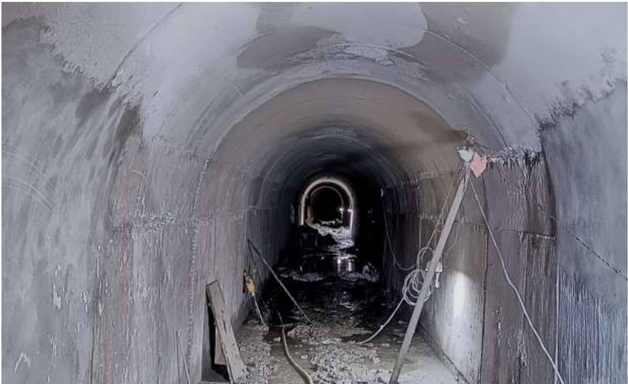
Figure 2-22: A view of full concrete lining at the flushing tunnel
