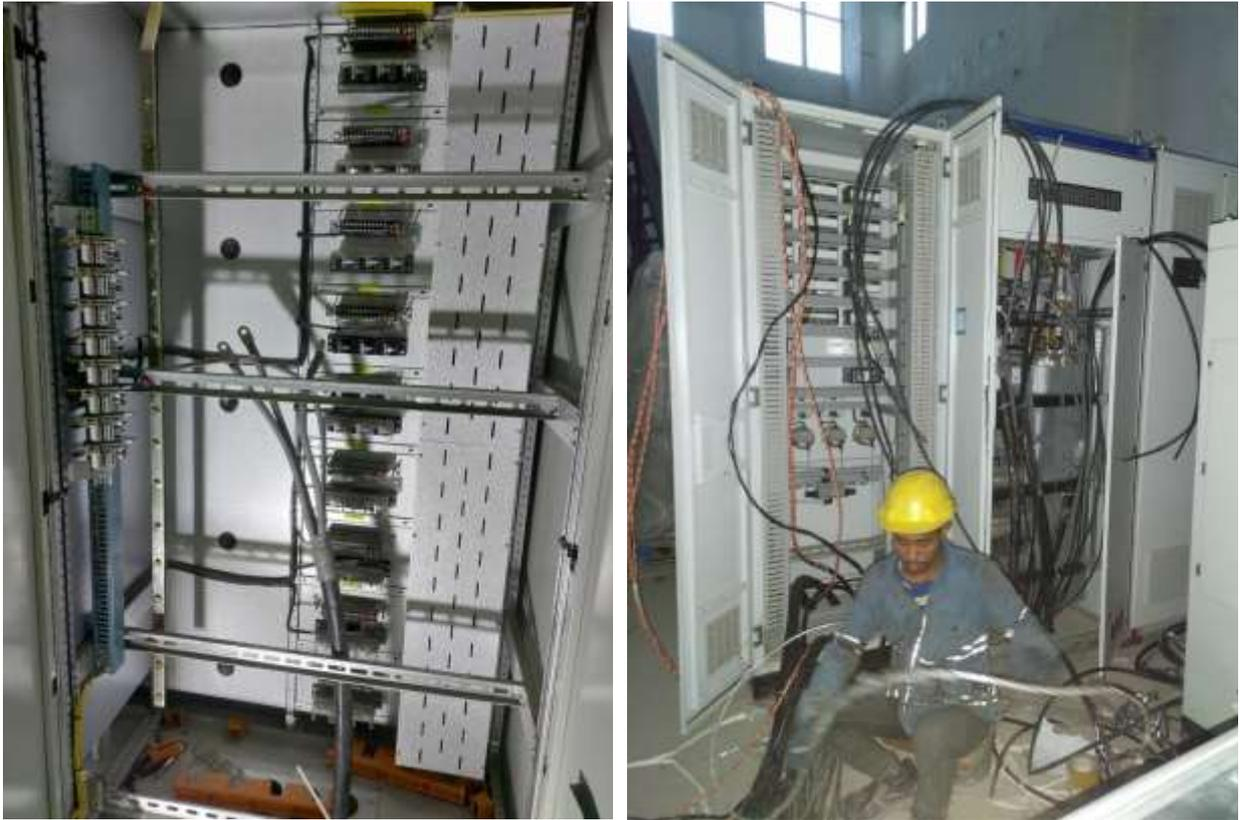
Figure 2-63: Cable shoe crimping (left) and cable termination work (right)
