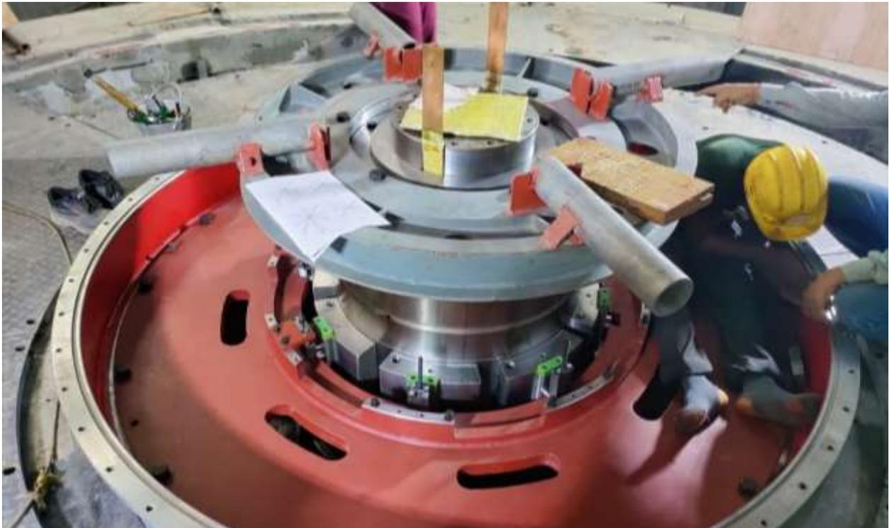
Figure 2-56: Run-out check of shaft
