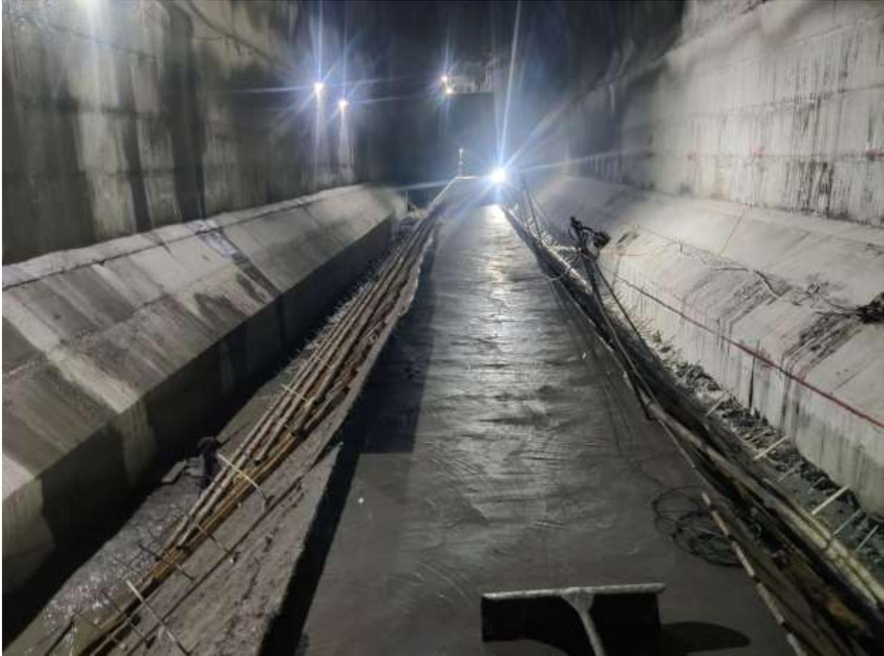
Figure 2-14: Concreting works at the middle pier of hoppers of settling basin bay 02
