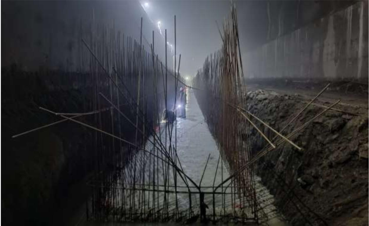
Figure 2-10: A view of concreting at the left hopper of Settling Basin 01
