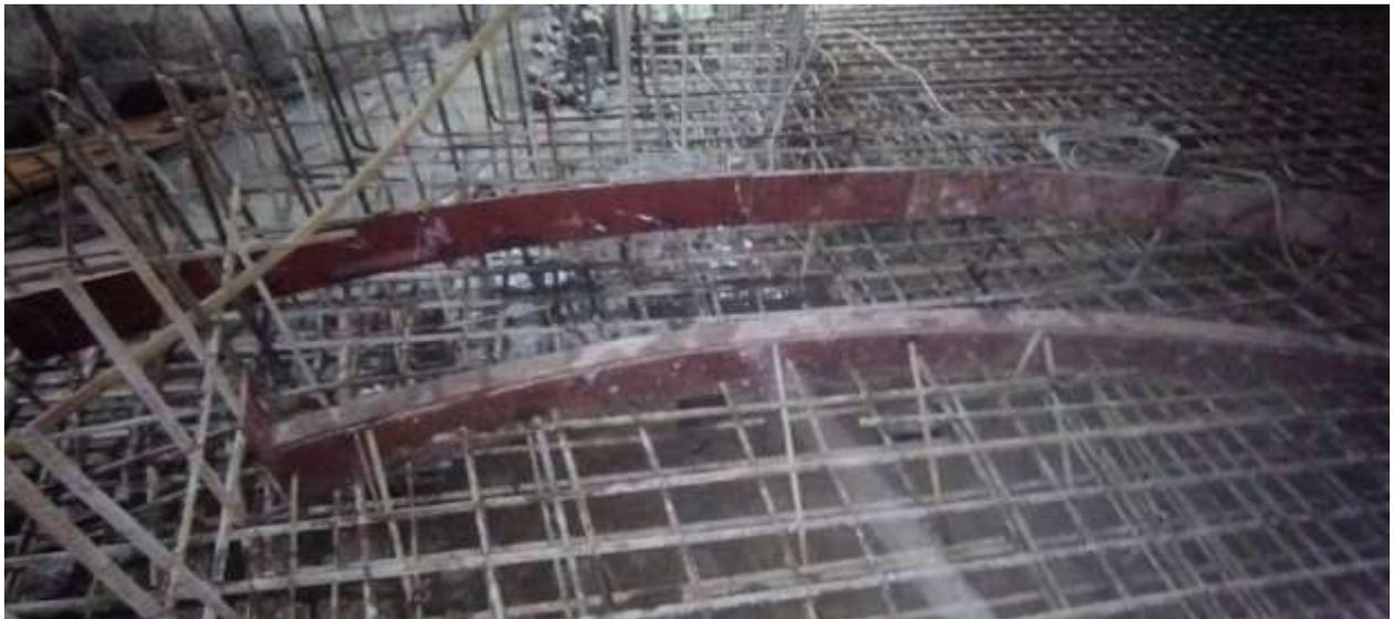
Figure 2-35: Erection of track for Adit Bulk Head gate
