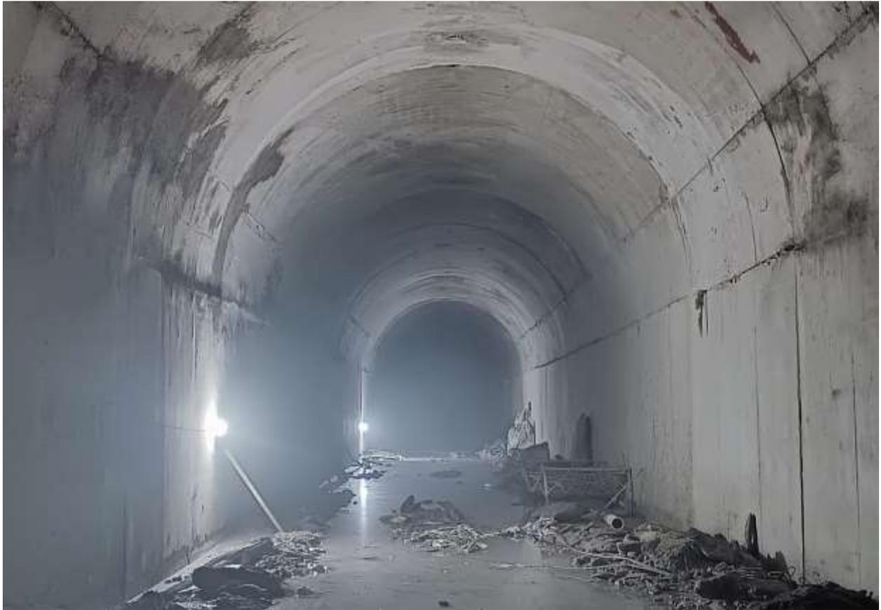
Figure 2-17: A section of HRT with concrete full lining from the adit region
