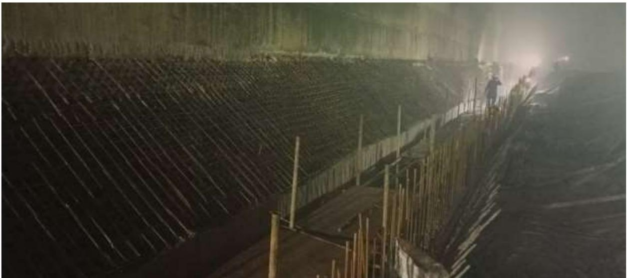
Figure 2-13: Rebar layout of hopper of SB 02
