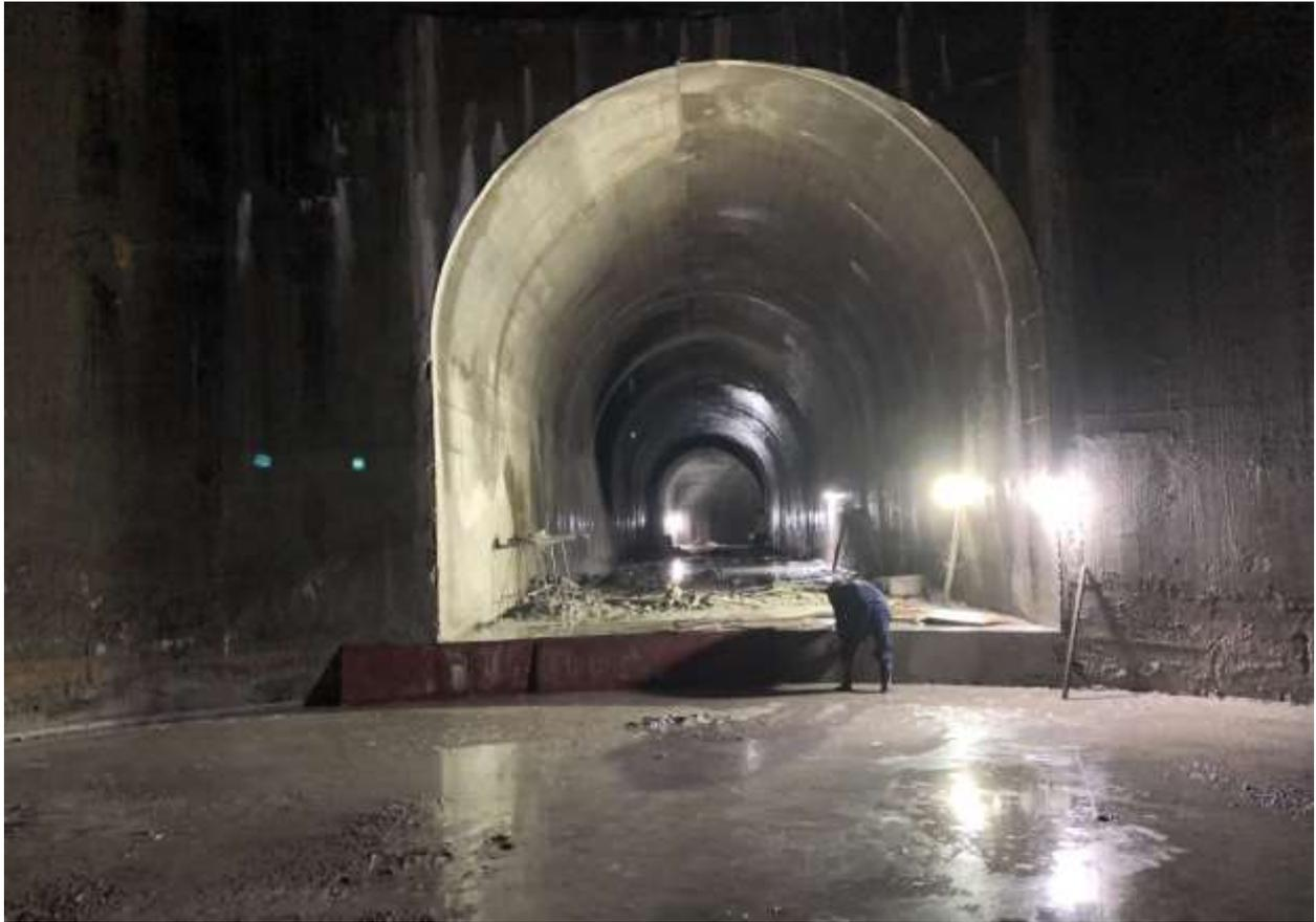
Figure 2-26: A view of full lining concrete at connecting tunnel of Surge Shaft
