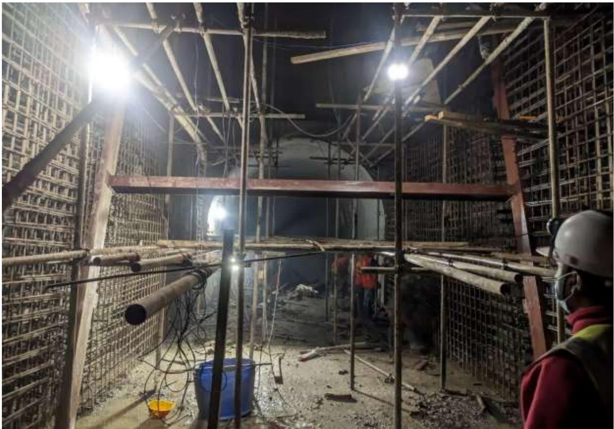
Figure 2-37: Erection of trashrack frame and gate embedded parts at Settling Basin Outlet Gate-3
