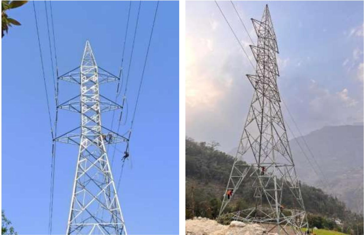
Figure 2-78: Conductor stringing works at various angle points
