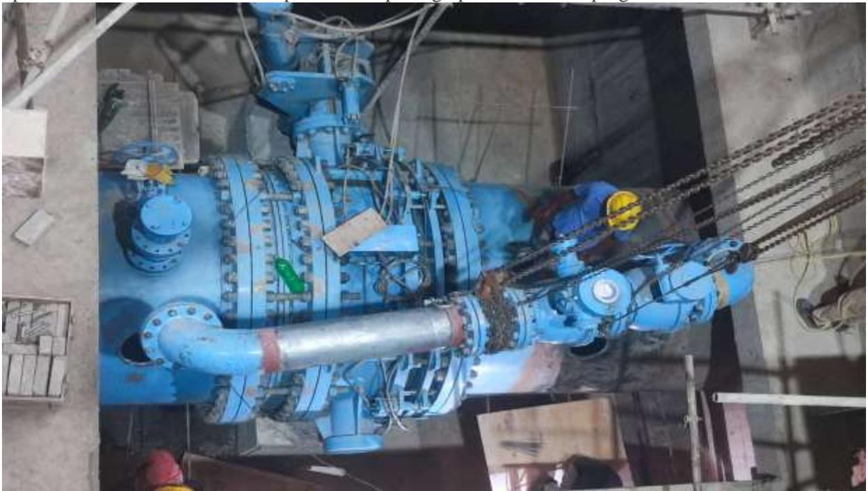
Figure 2-58: Unit 02 bypass valve assembly and erection
