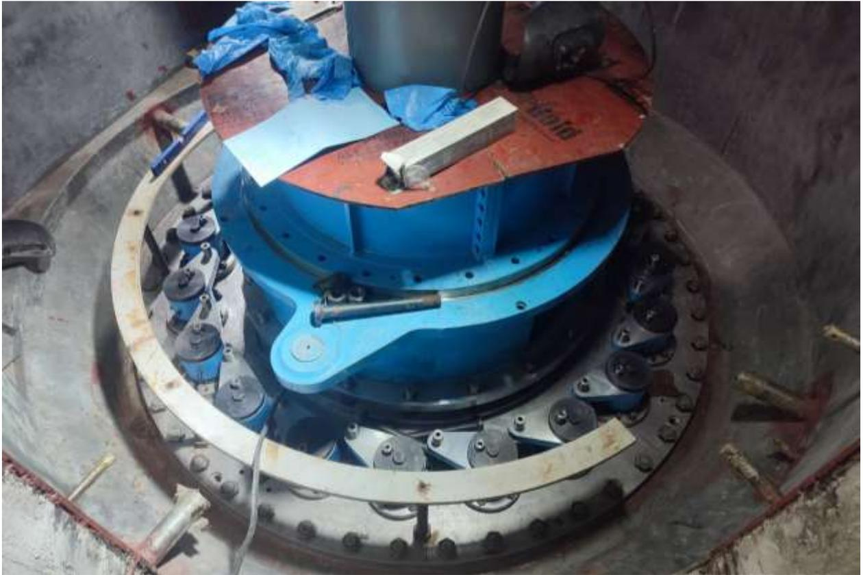
Figure 2-57: Final assembly of water regulating mechanism
