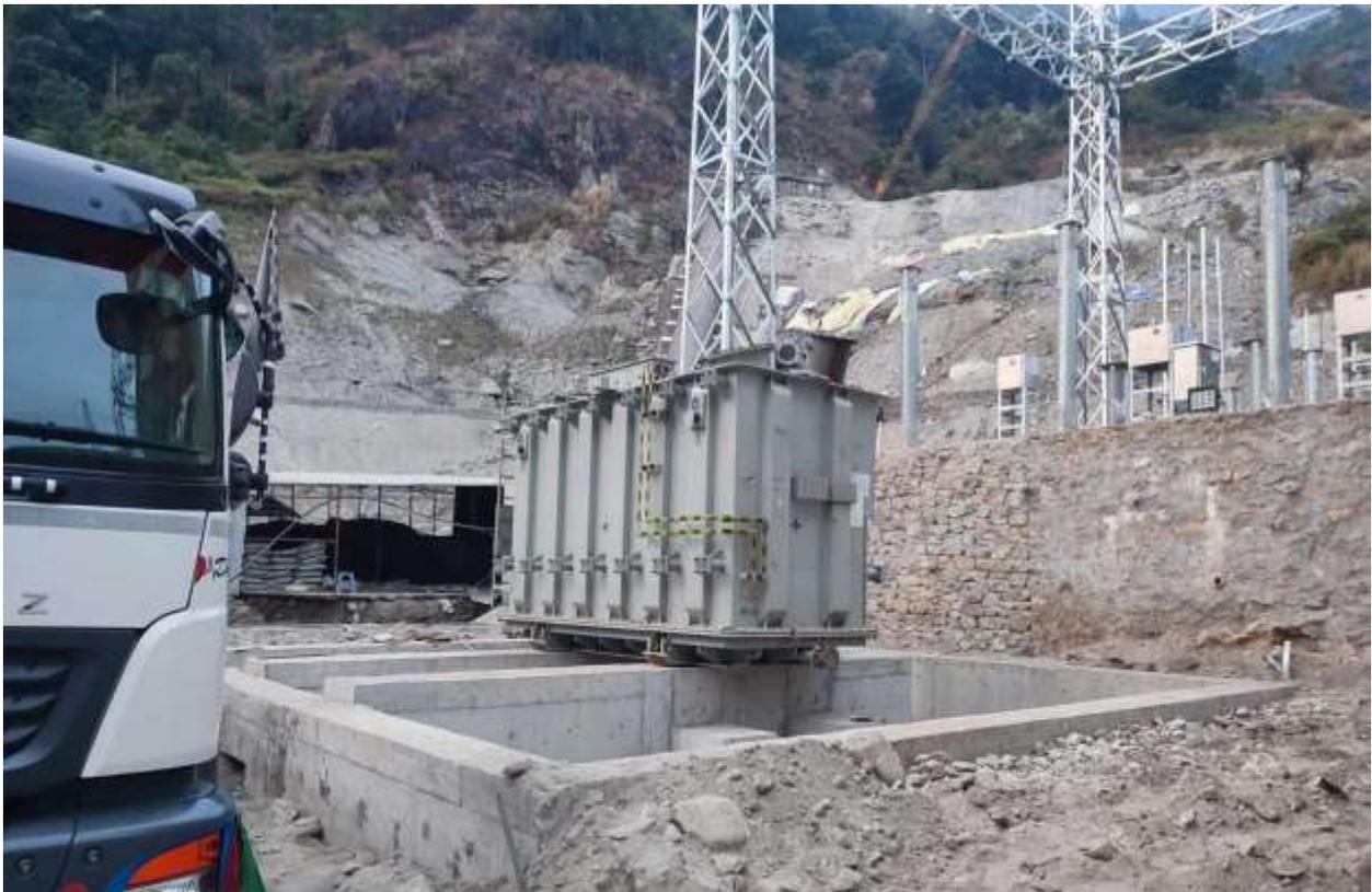
Figure 2-70: Power transformers placed at its position
