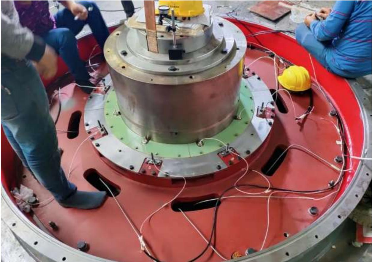
Figure 2-44: Installation of temperature and resistance measuring sensors at thrust bearing
