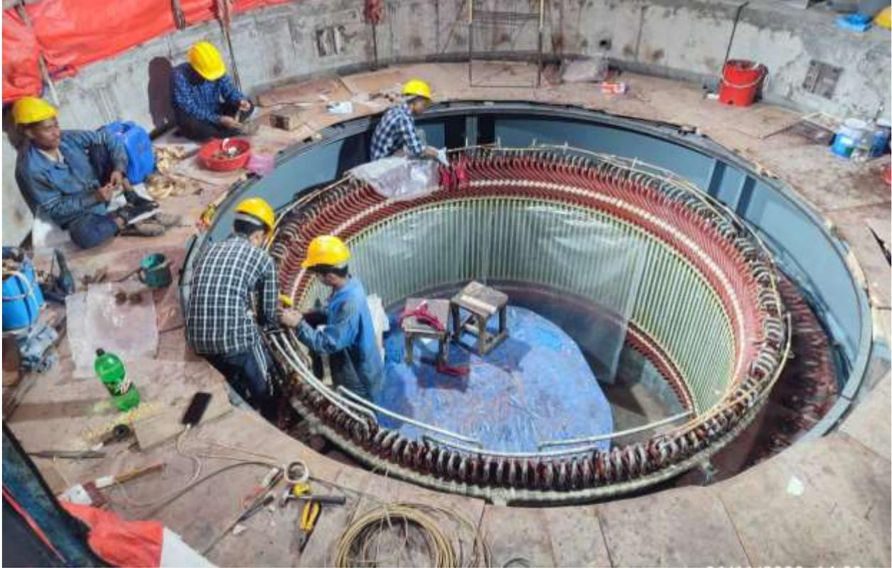
Figure 2-47: Brazing and lacing work of stator coils
