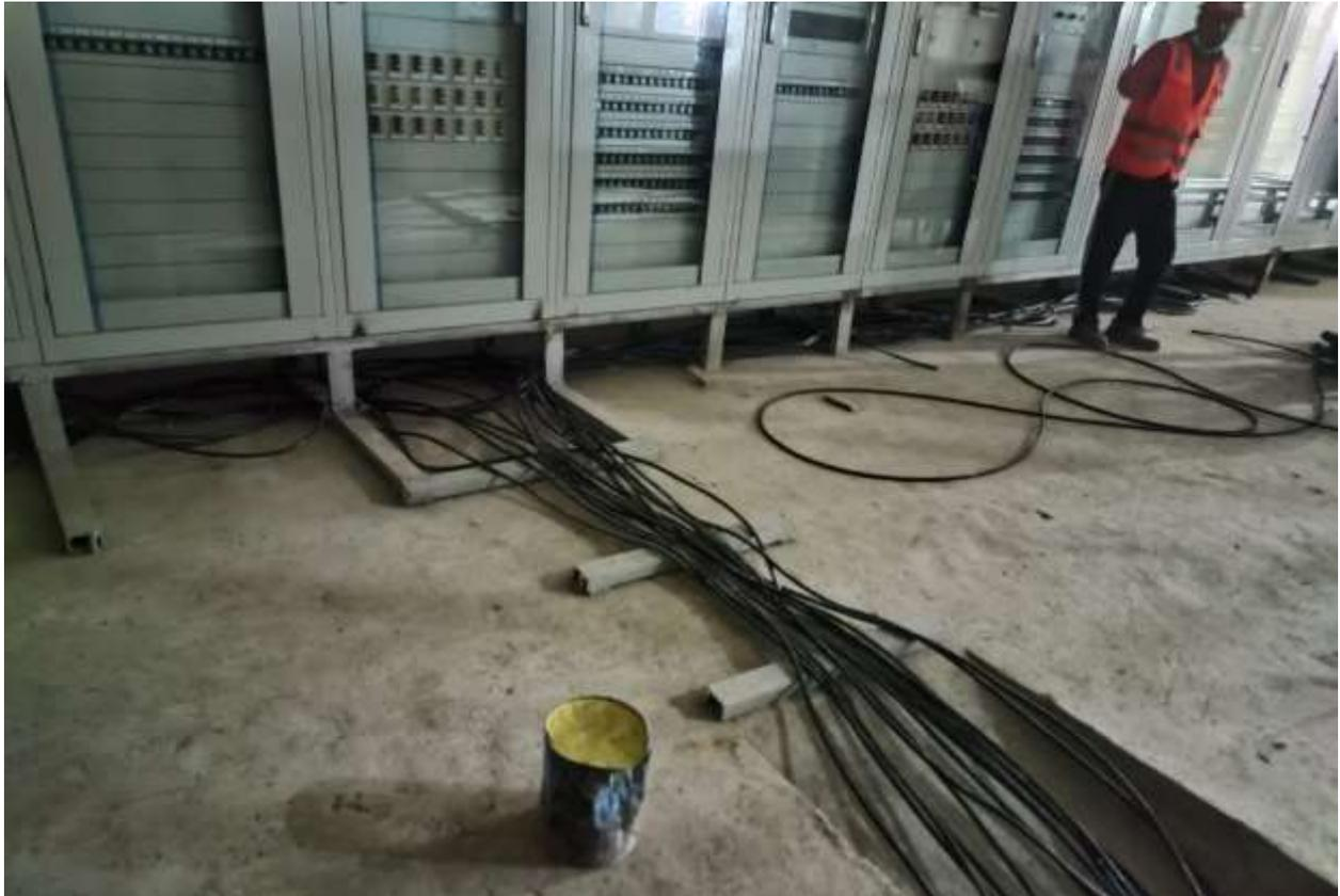
Figure 2-65: Laying of control cables
