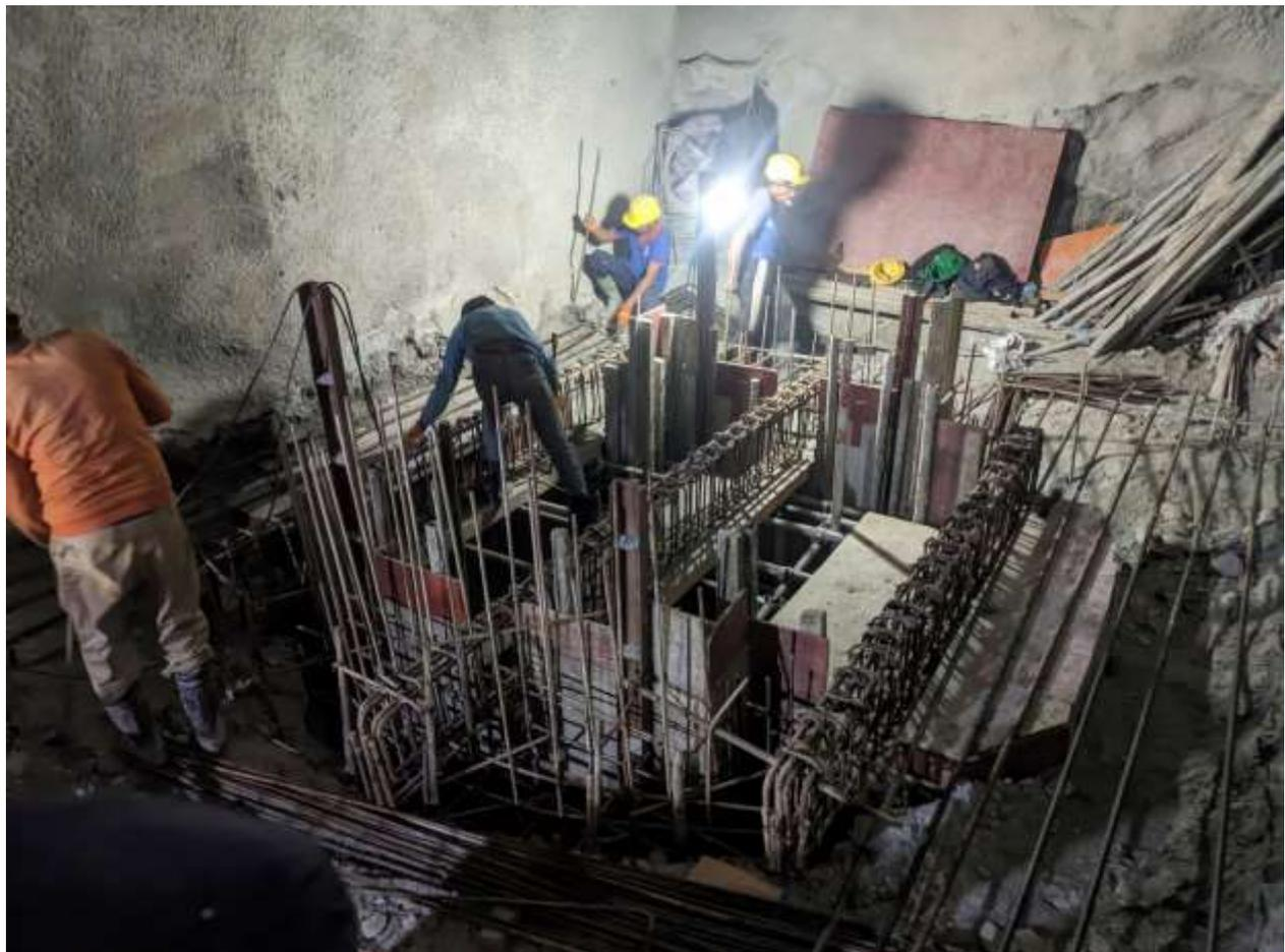
Figure 2-33: Erection of embedded part of gate and stoplog at SBF-3
