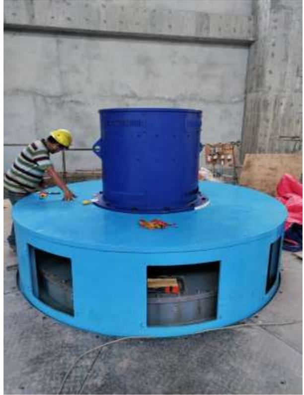
Figure 2-50: Excitation system installation
