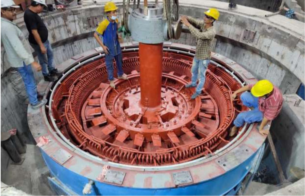
Figure 2-55: Rotor lowering of unit 04
