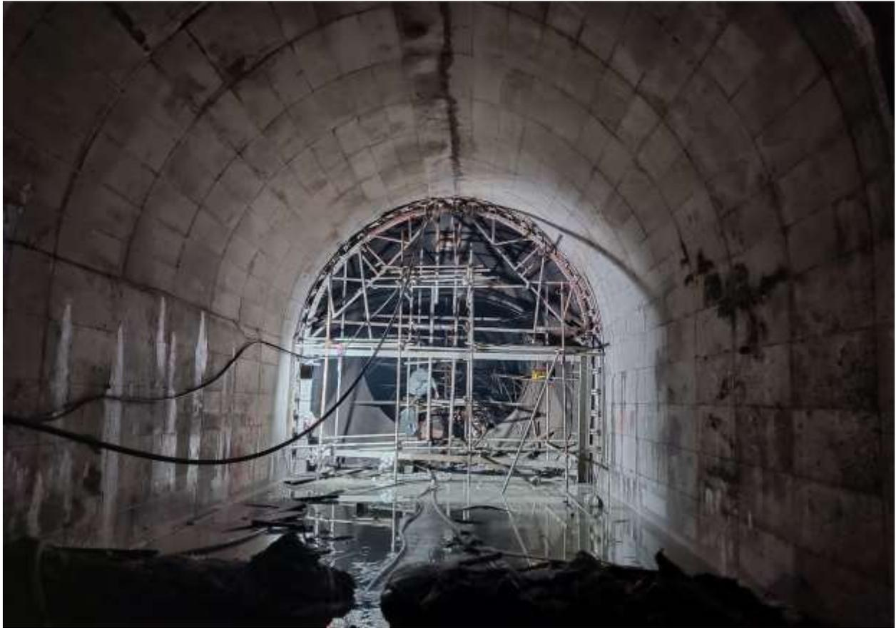
Figure 2-19: A section of HRT with concrete full lining from the outlet region
