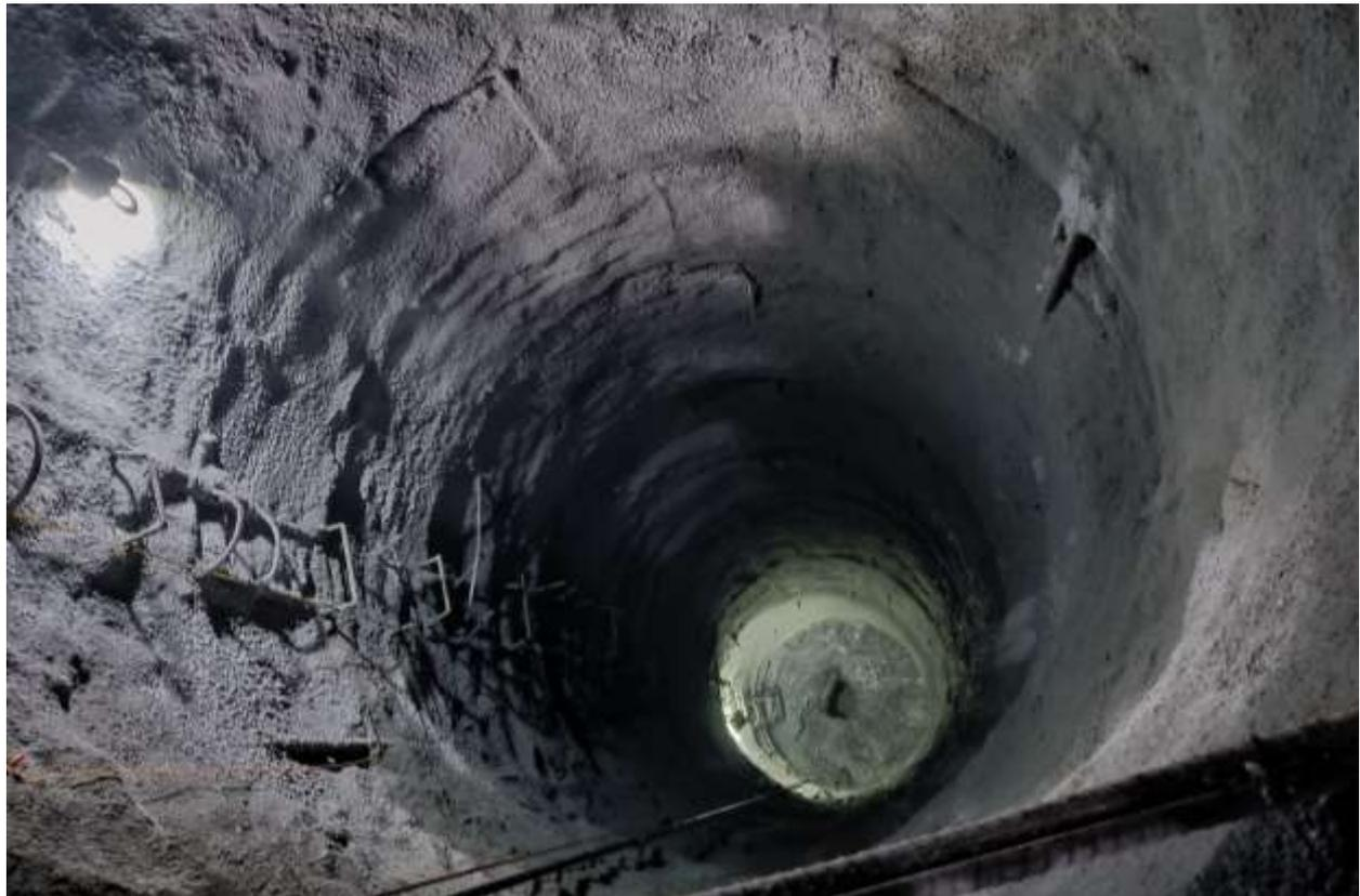
Figure 2-23: Breakthrough of flushing tunnel 04
