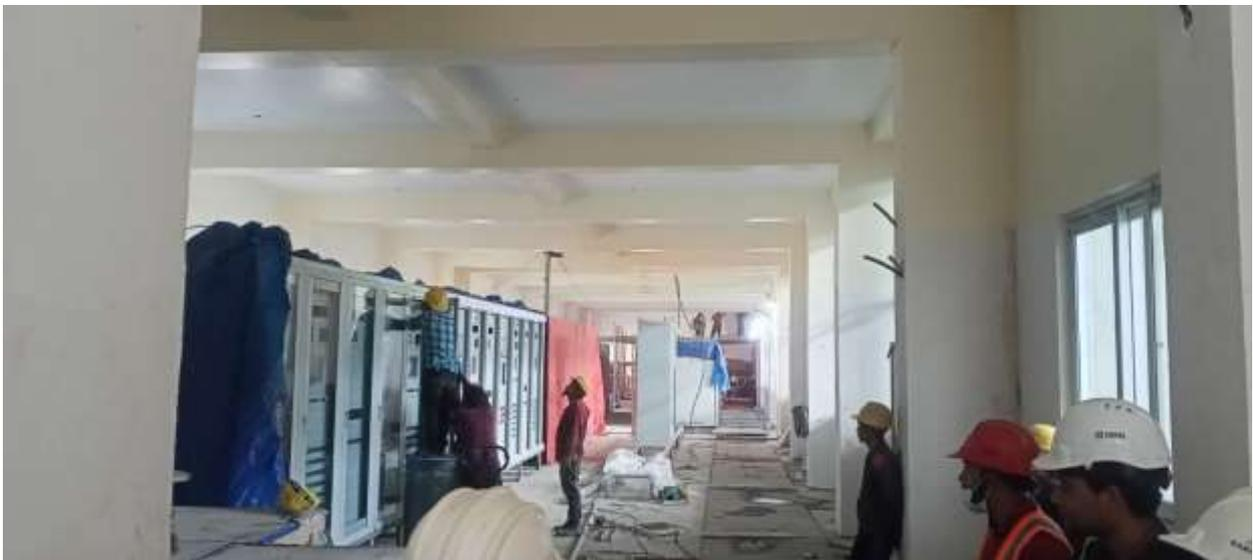
Figure 2-62: Installation of control panels
