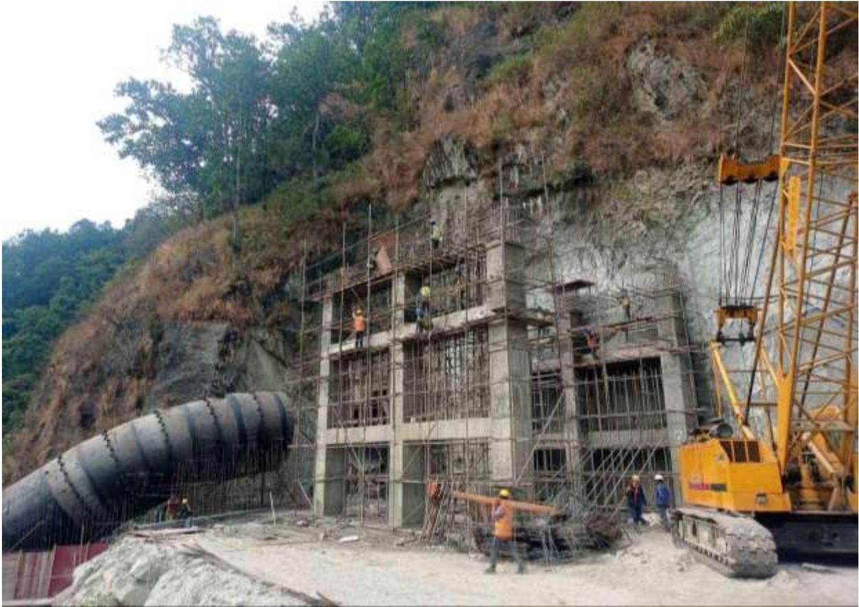
Figure 2-31: Construction of valve house
