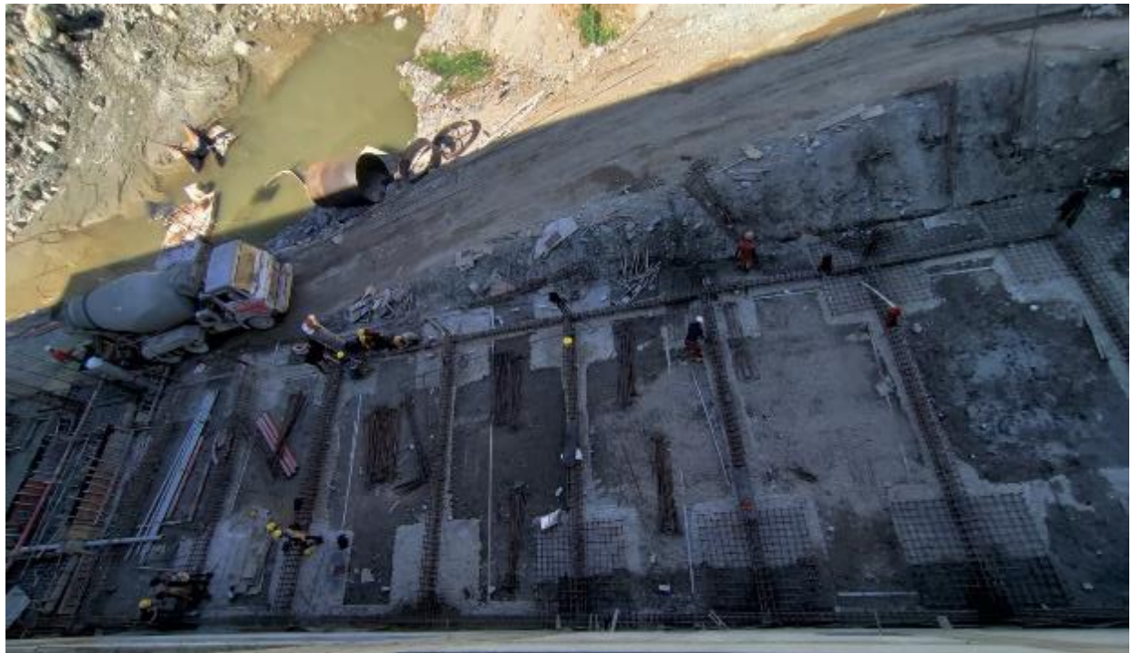
Figure 46: PCC done after earth mat installtion in auxiliary power house
