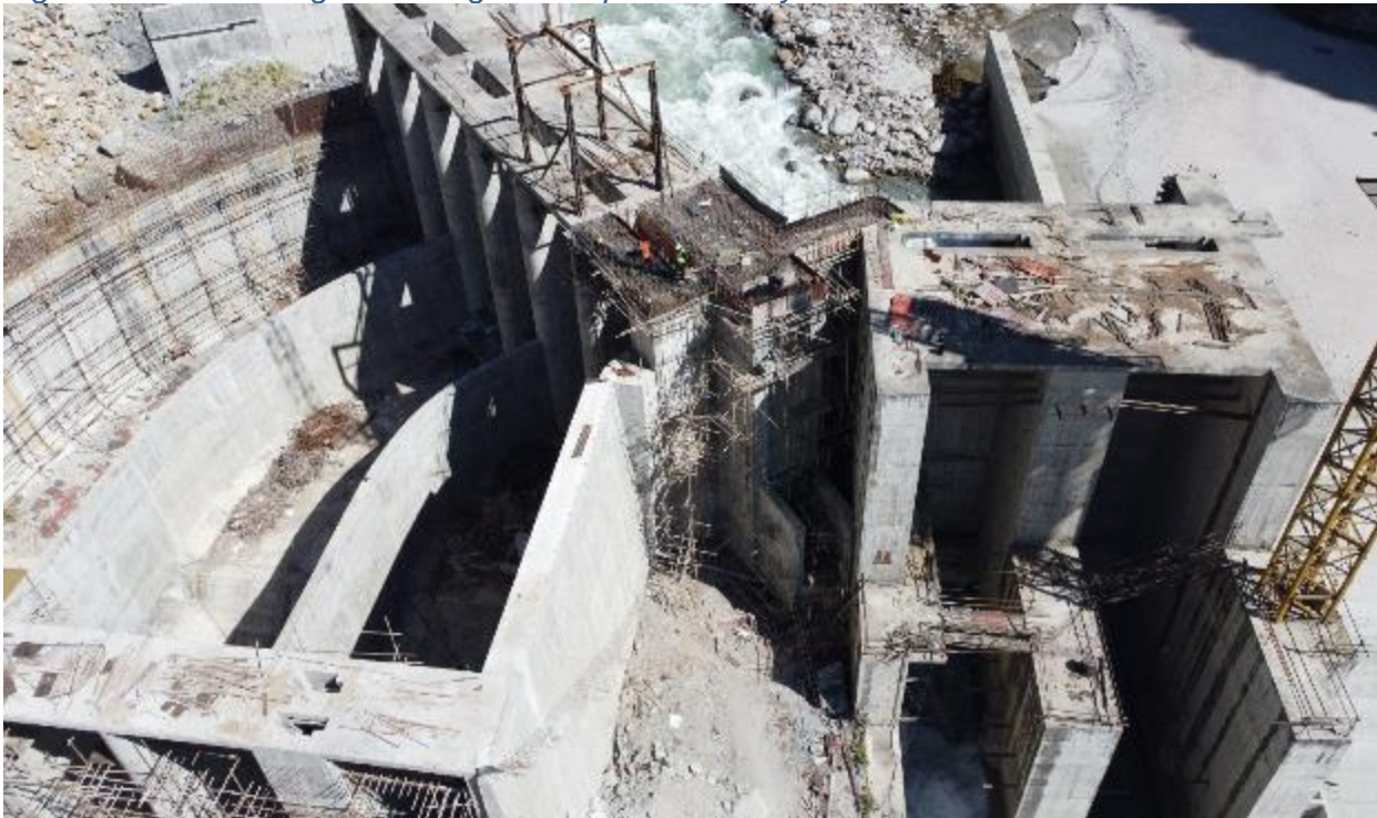
Figure 2-8: Rebar and concrete works at the top slab of intake
