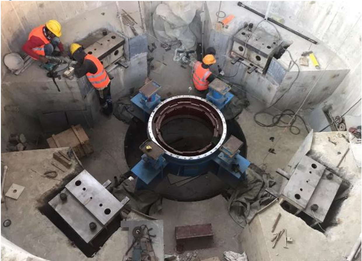
Figure 2-31: Stator foundation inside generator casing of Unit 01
