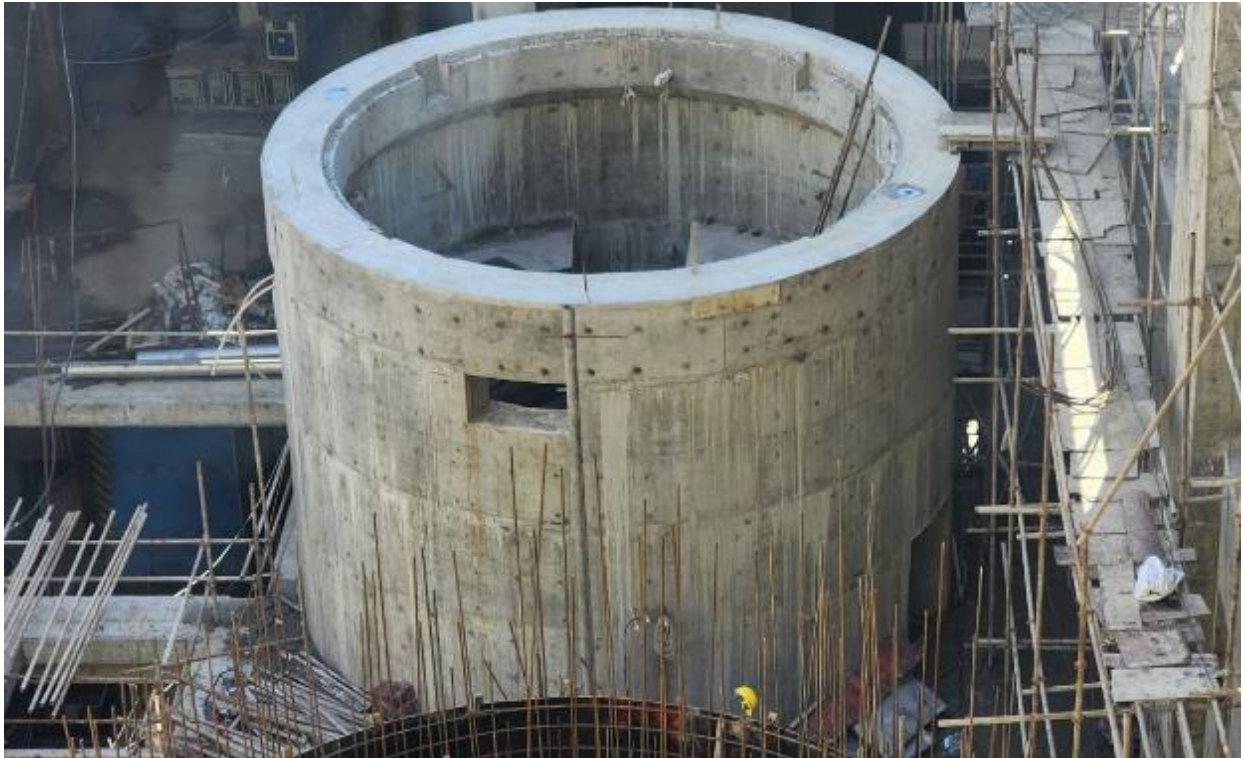
Figure 2-28: Casting of generator casing at unit 01
