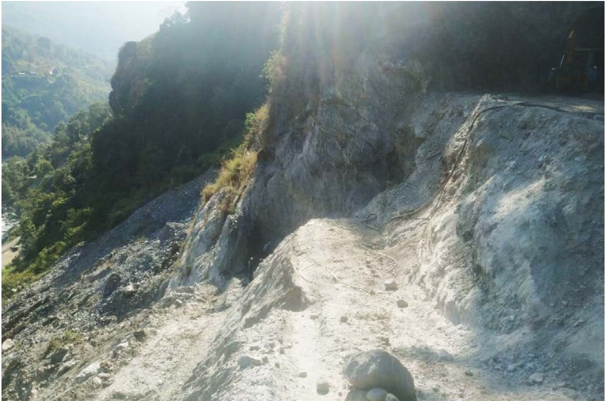
Figure 2-30: Rock excavation for anchor block
