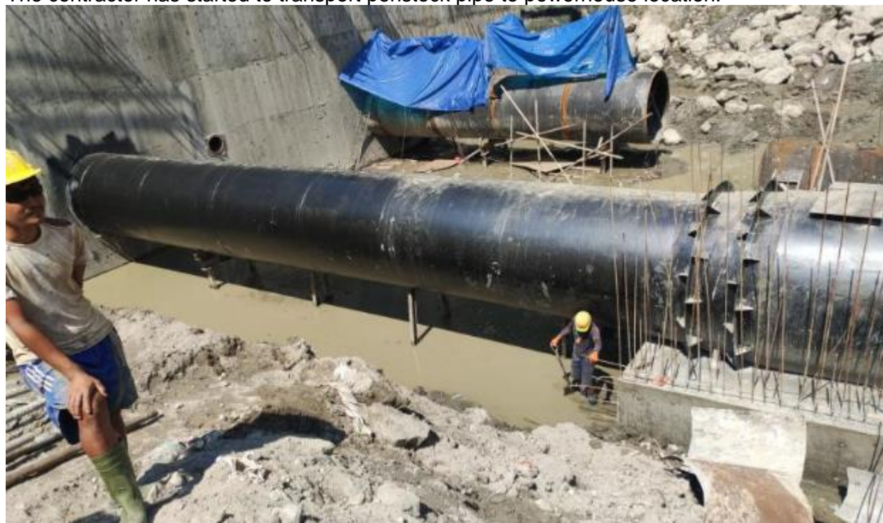
Figure 2-36: A view of brach pipe of penstock installation (during installation)
