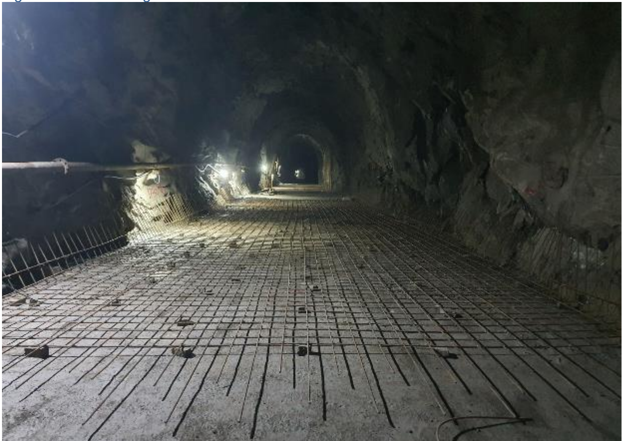
Figure 2-17: Rebar layout at the HRT invert
