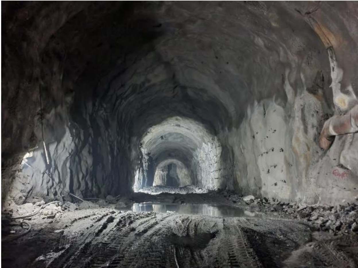
Figure 2-22: A view of SB 02 after 1 layer of benching
