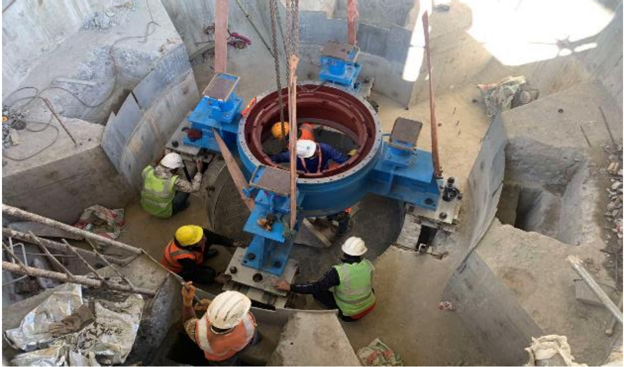
Figure 2-46: Installation of lower bracket in unit 1
