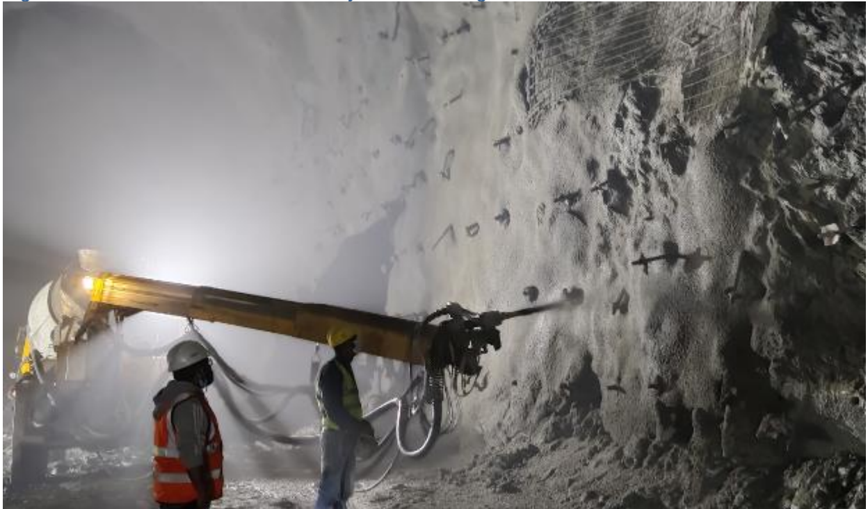
Figure 2-23: Application of rock supports on the side walls
