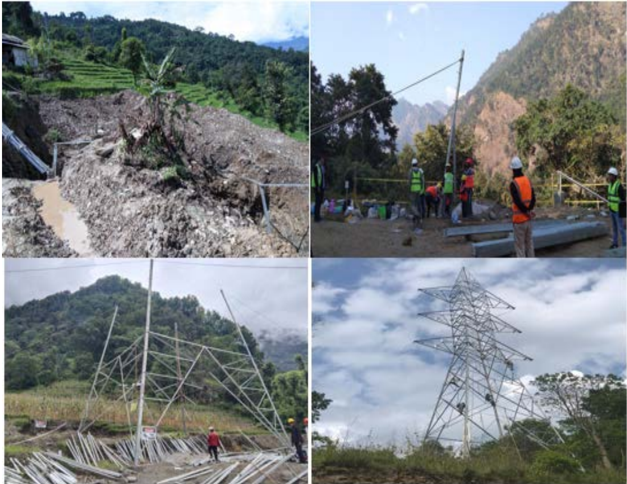
Figure 2-52: Various stages of transmission line works
