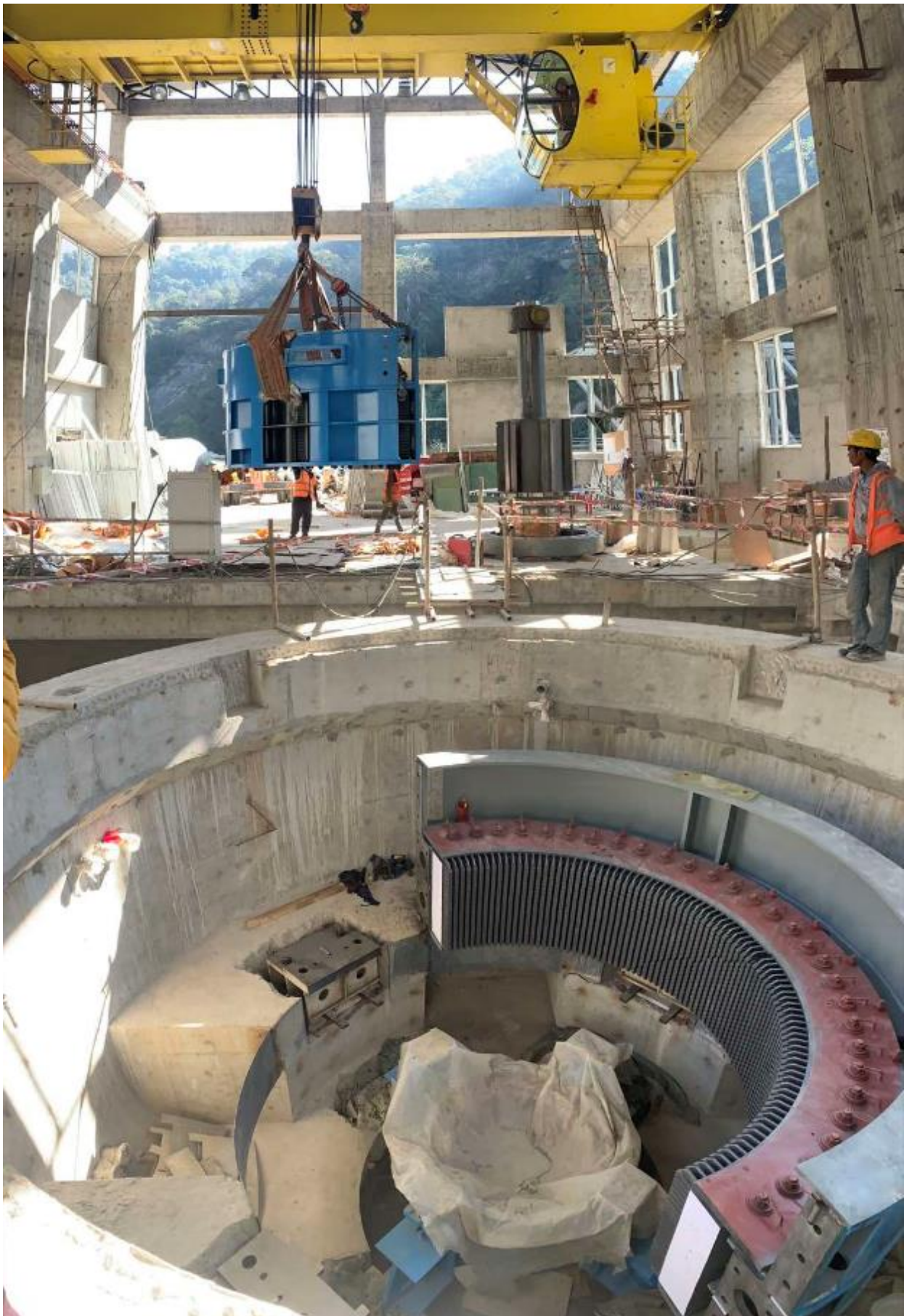
Figure 2-49: Lowering of stator into unit pit 1
