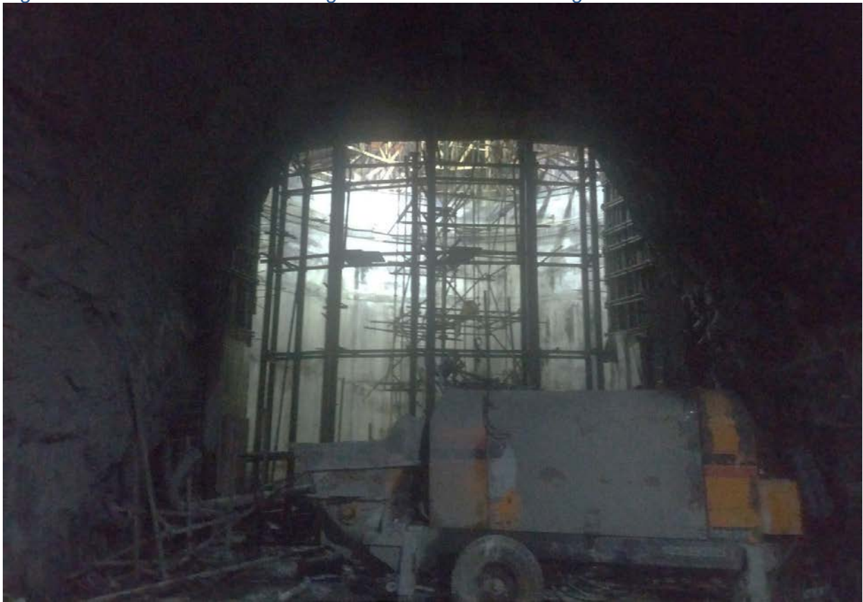
Figure 2-25: Concreting of surge shaft walls
