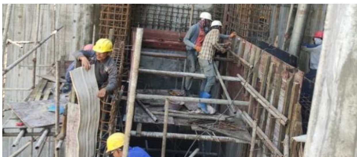
Figure 2-33: Installation of steel plates at trash passage
