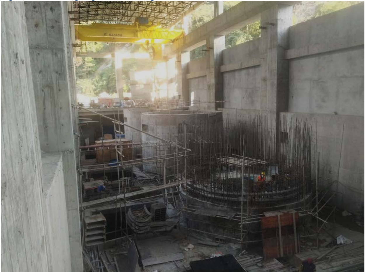
Figure 2-29: Rebar installation for generator casing at unit 03
