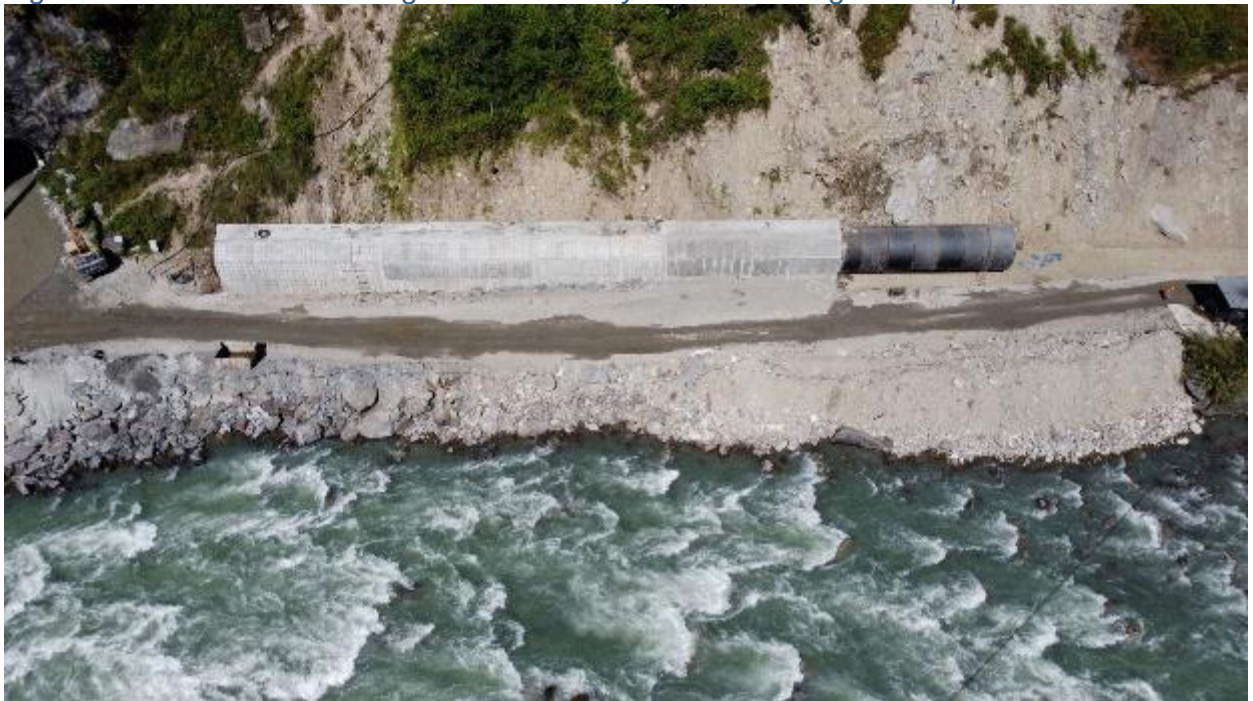
Figure 2-10: Erection of concrete encased approach pipe
