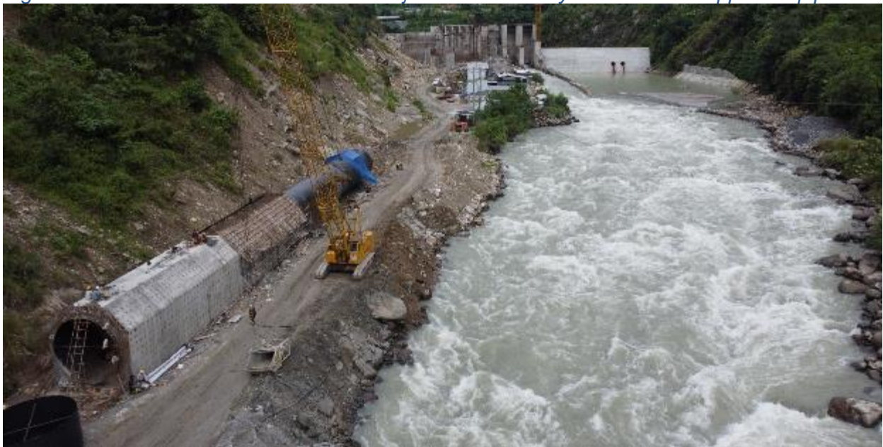
Figure 2-35: Installation of approach pipe
