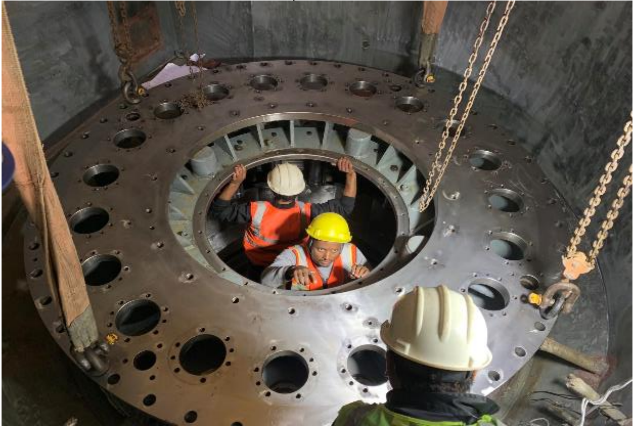
Figure 47: Lowering of headcover in unit 2
