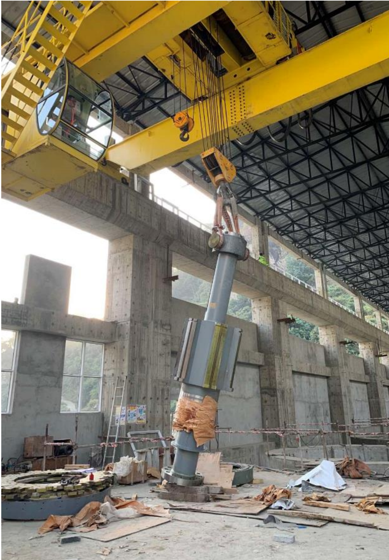
Figure 2-48: Erecting rotor of unit 1 in service bay
