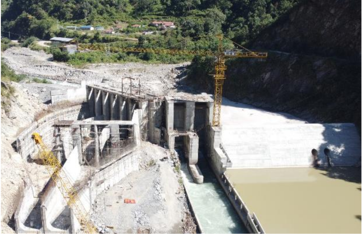
Figure 2-7: Concreting works at gravel trap and conveyance tank
