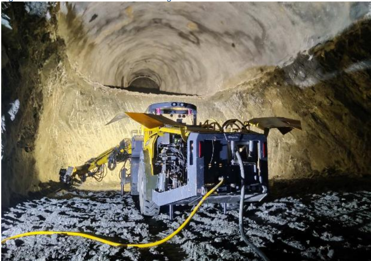
Figure 2-21: A view of drilling and rockbolt installation works at Settling basin 02
