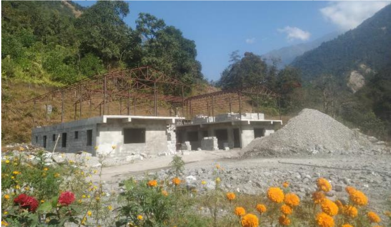
Figure 2-1: Installation of truss at first floor
