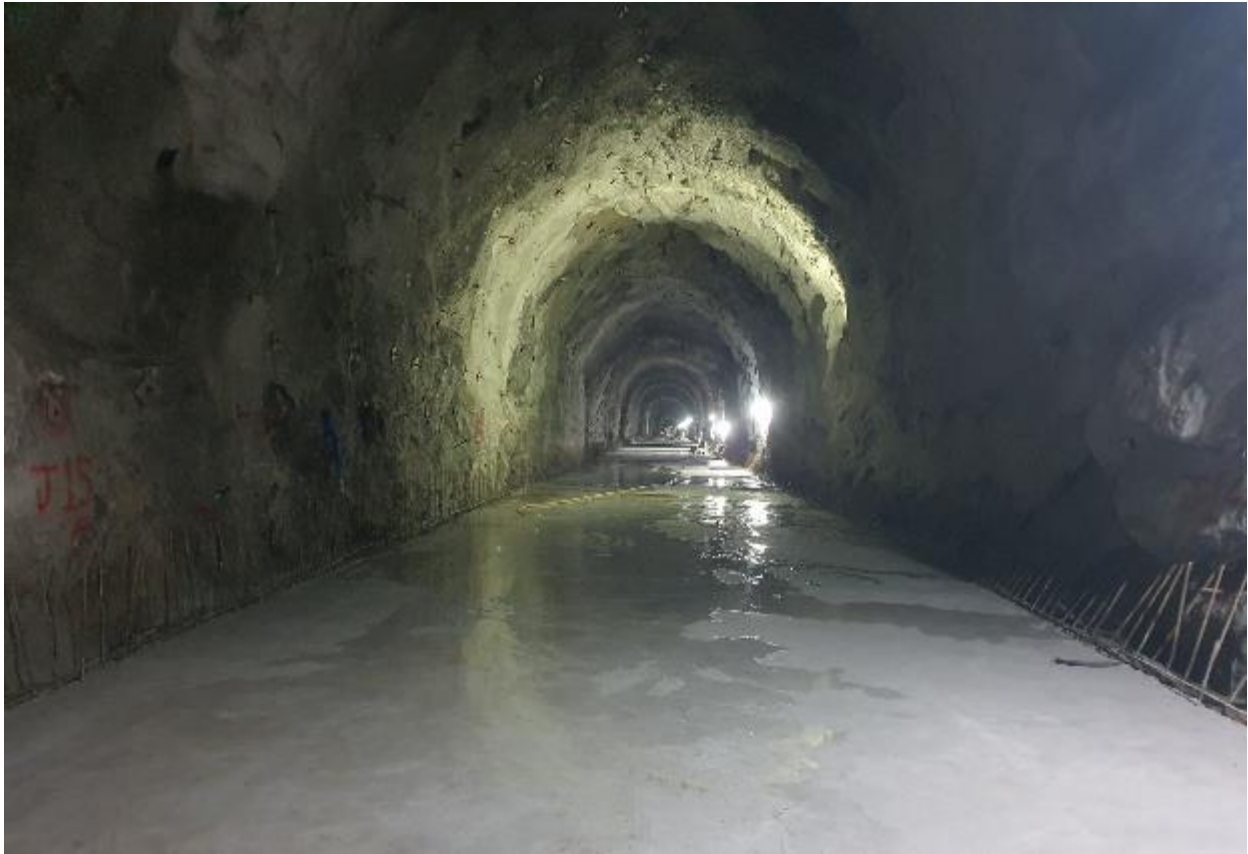
Figure 2-18: Concreting works at HRT invert
