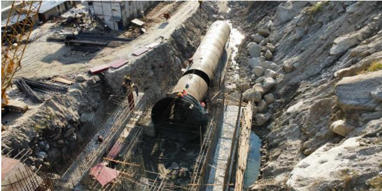
Figure 2-34: Installation of bellmouth at the junction of conveyance tank and approach pipe
