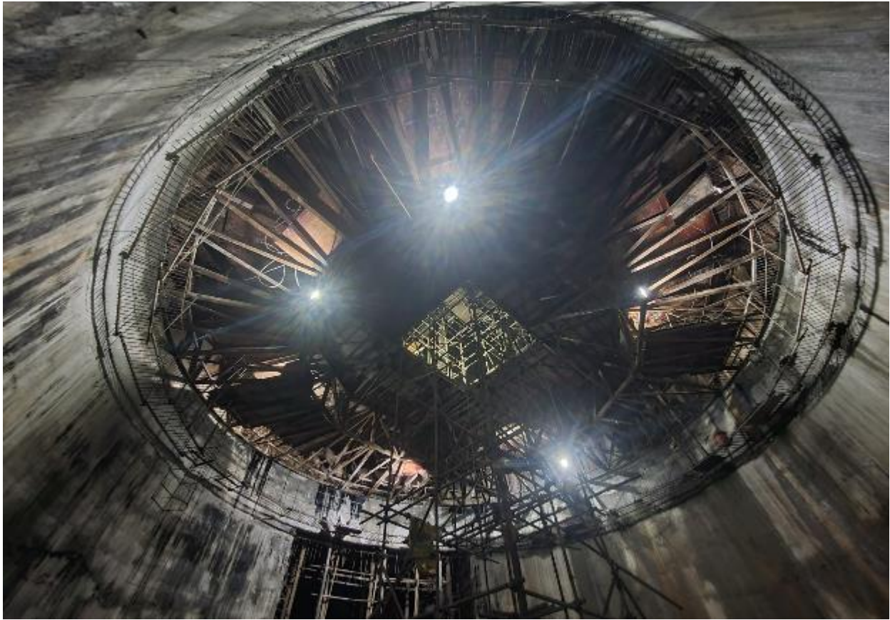
Figure 2-24: Formwork for concreting works of side walls of Surge shaft
