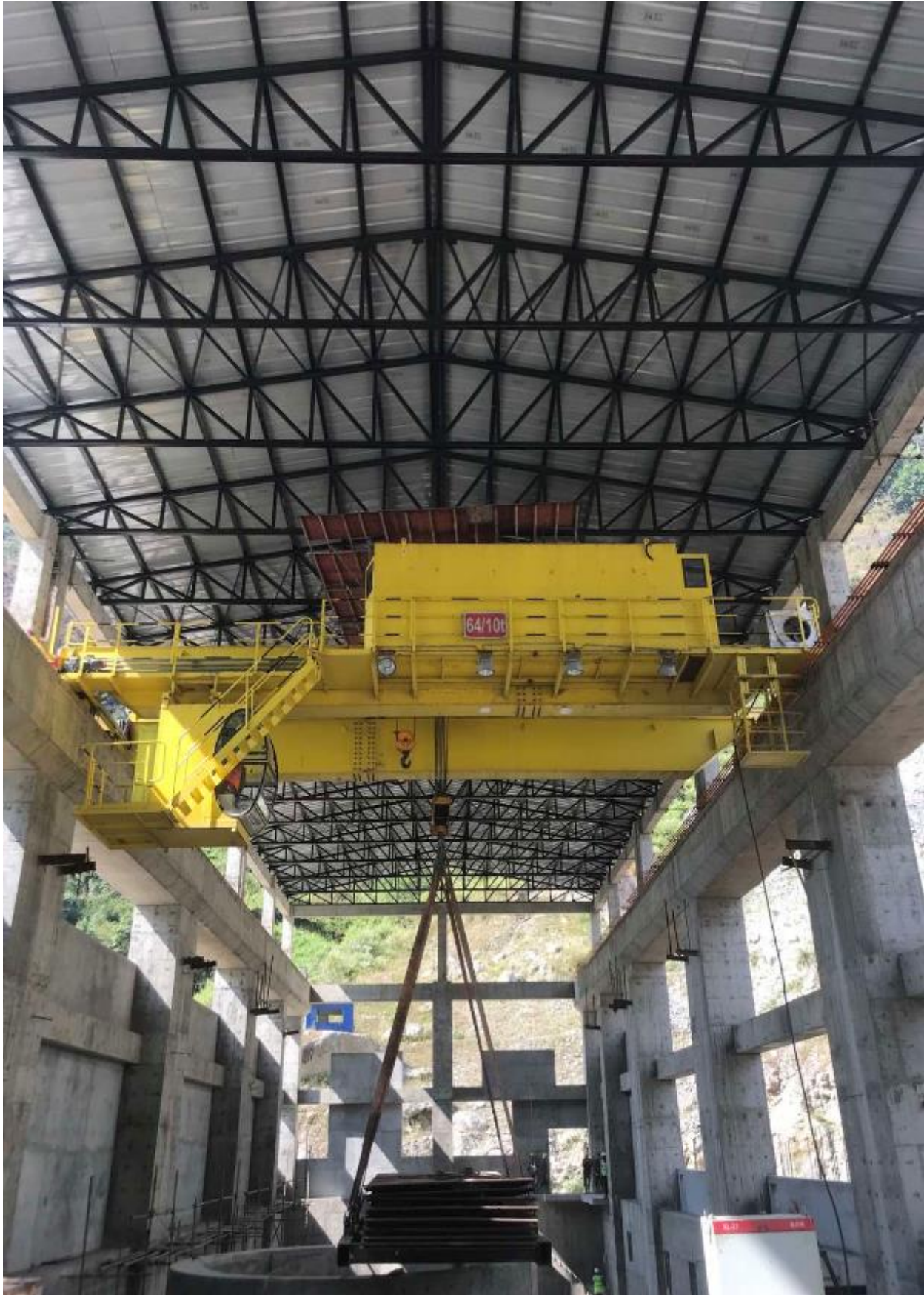
Figure 2-44: Load test of EOT lifting 66 ton and travelling across unit 2
