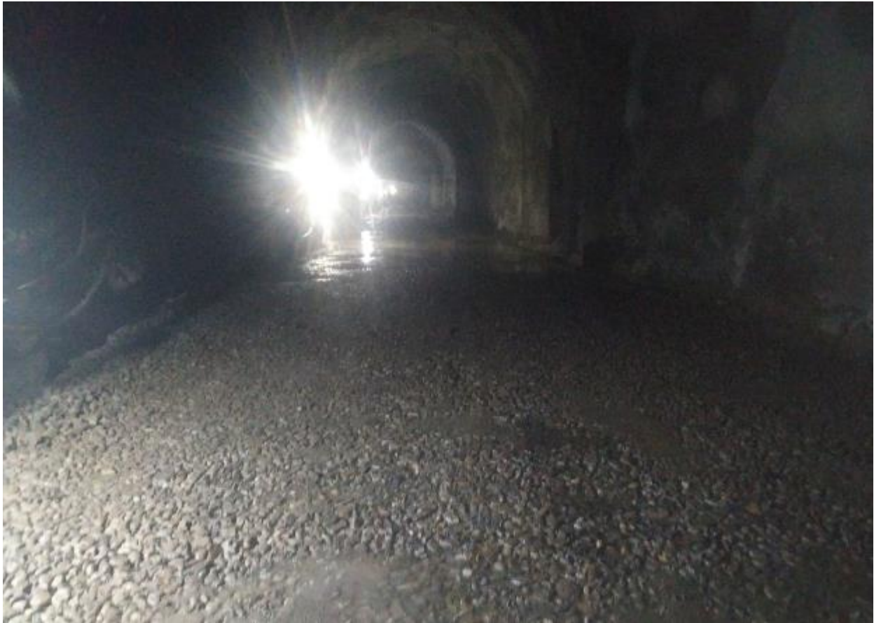
Figure 2-16: Backfilling works at the invert of HRT
