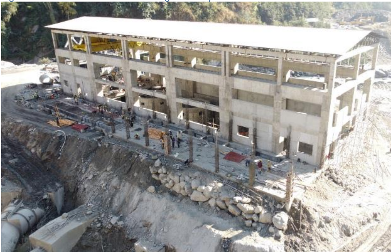
Figure 2-27: An aerial view of Powerhouse and construction of foundation of control bay
