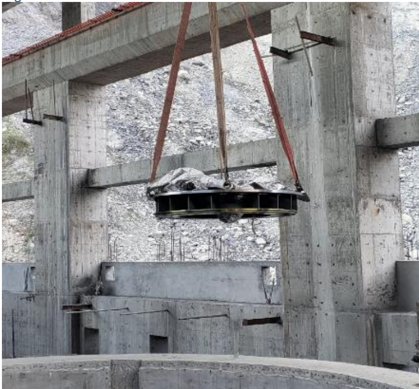
Figure 2-47: Lowering of headcover in unit 1 pit
