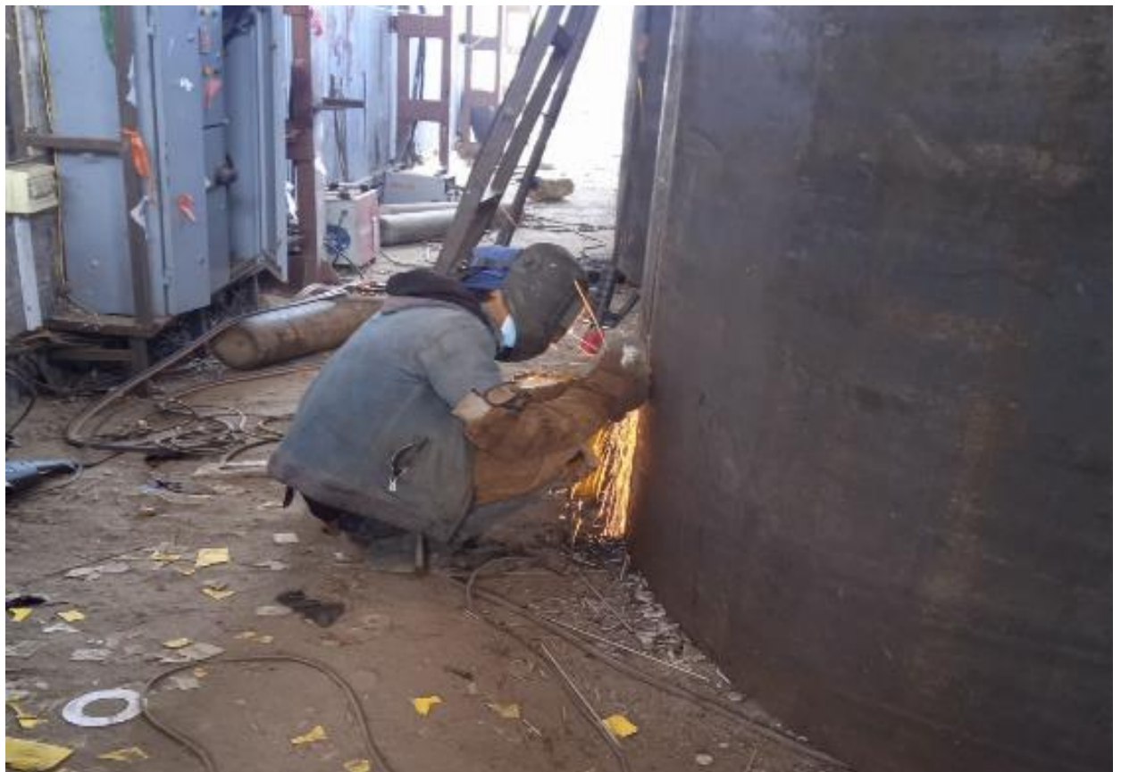
Figure 37: Grinding works before welding
