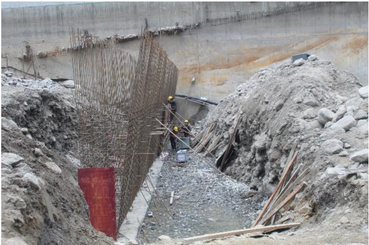
Figure 19: Reinforcement works at weir downstream cutoff wall
