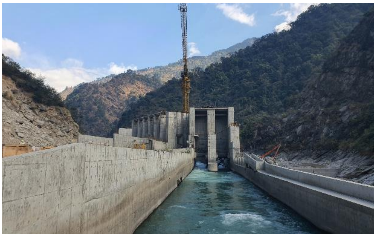
Figure 20: A view of Undersluice from downstream
