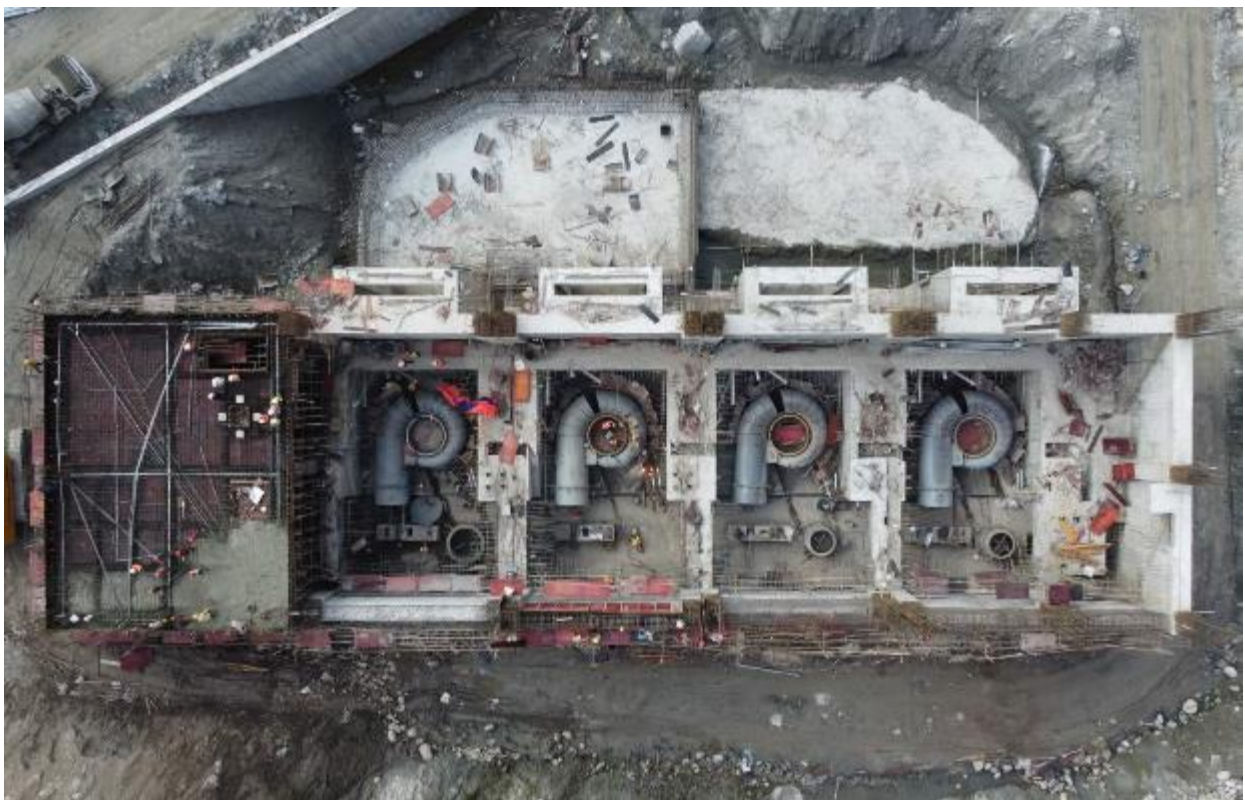
Figure 30: Reinforcement and formwork work at column in Powerhouse Bay 01
