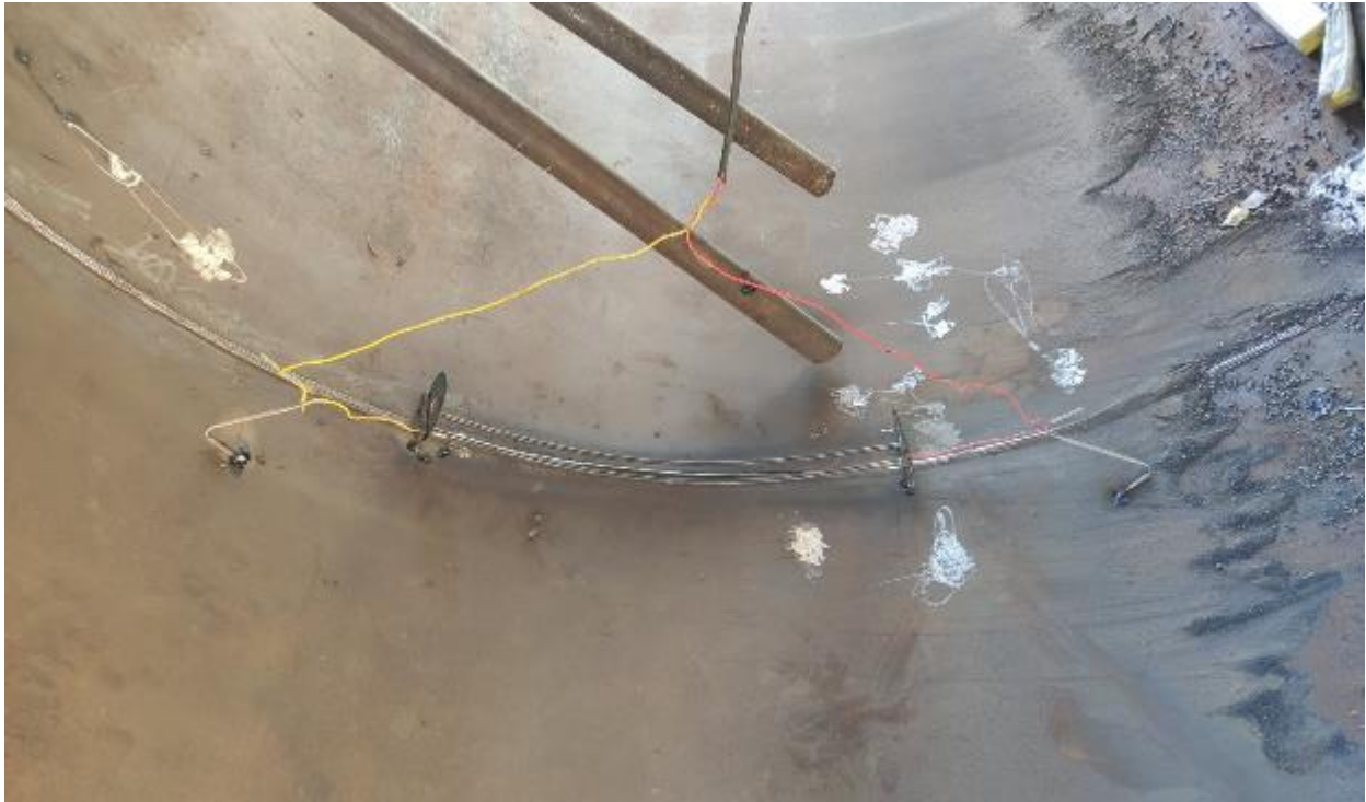
Figure 42: Pre-heating of joint before welding work using heating rod.
