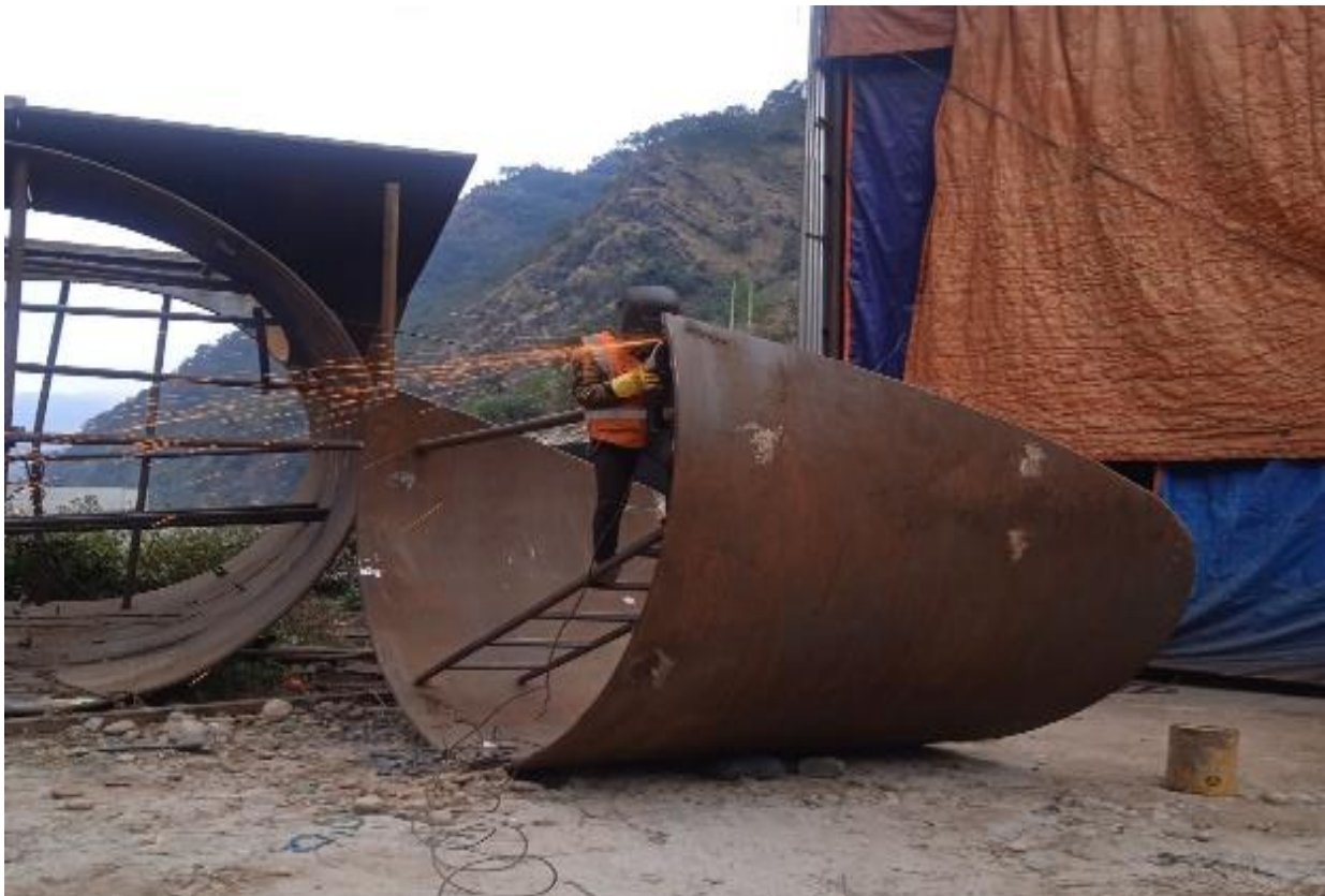
Figure 39: Bifurcation Unit 2 before grit blasting preparation work
