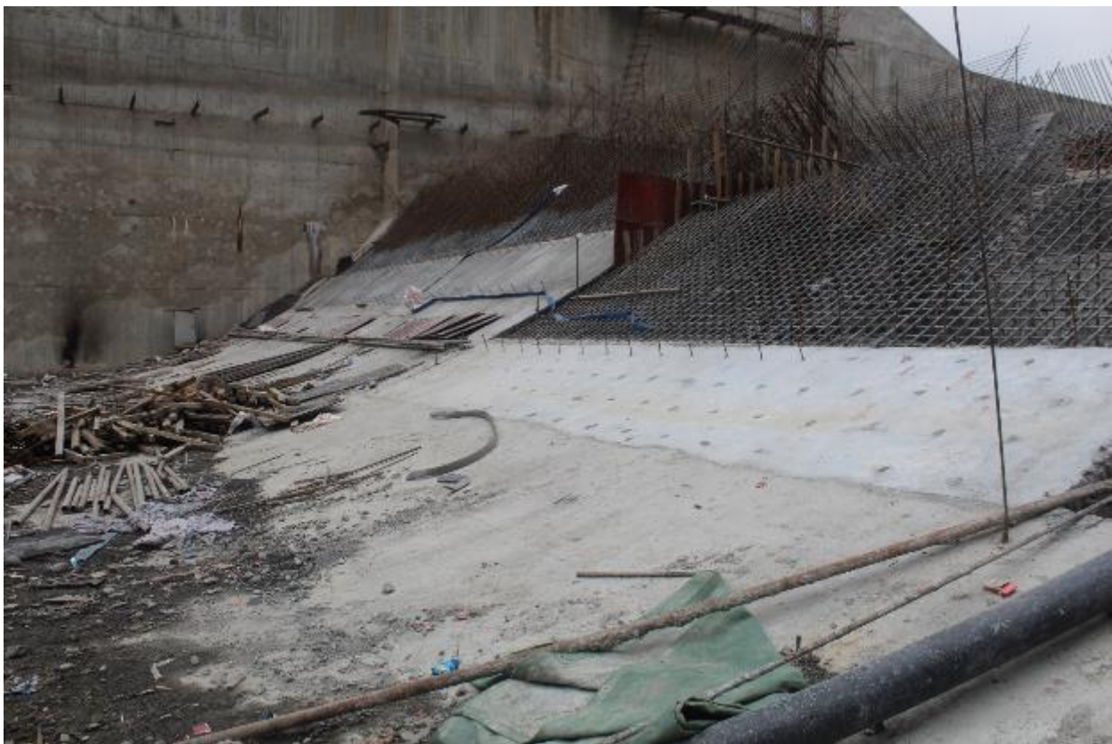
Figure 15: Ongoing reinforcement works of downstream slope of weir body
