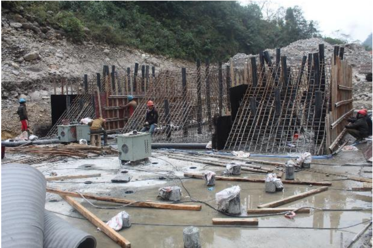
Figure 18: Ongoing Reinforcement works at baffle blocks of panel 08
