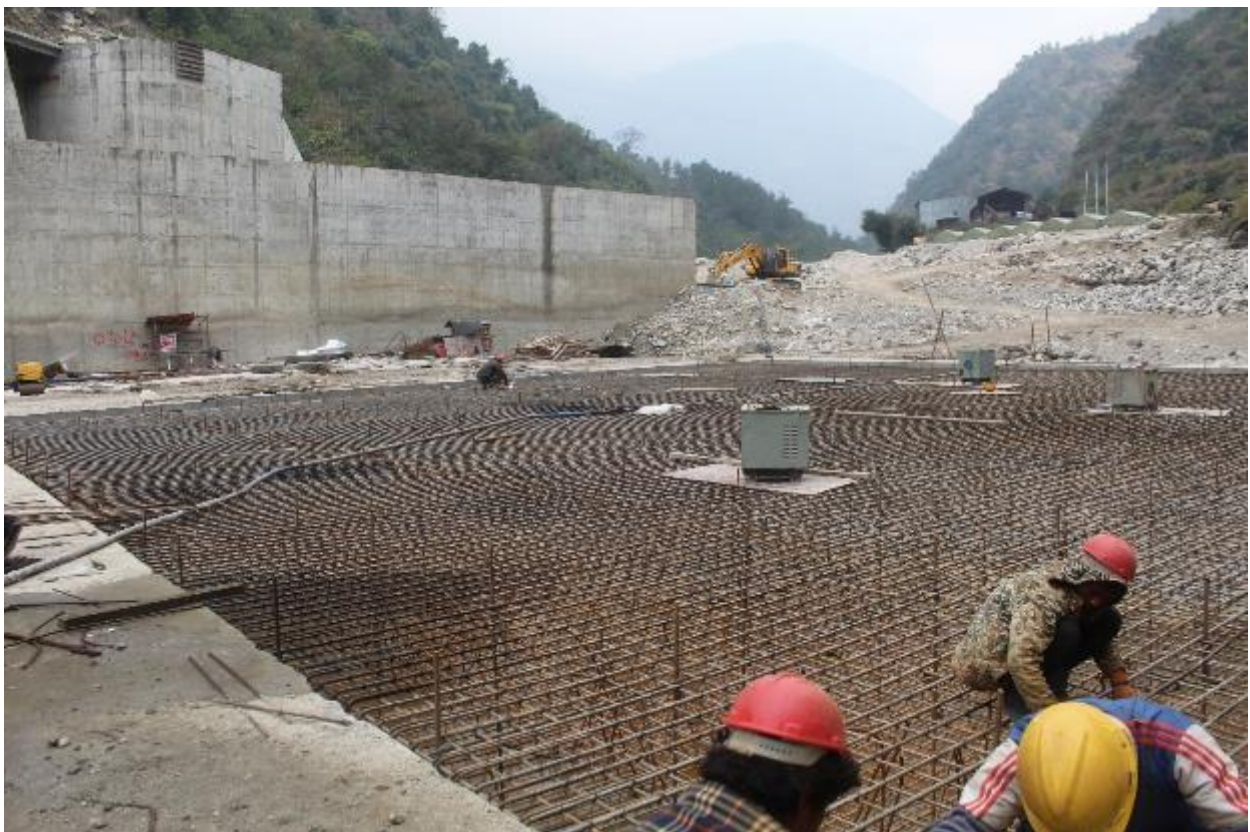
Figure 13: Reinforcement works at weir Upstream slab panel 02
