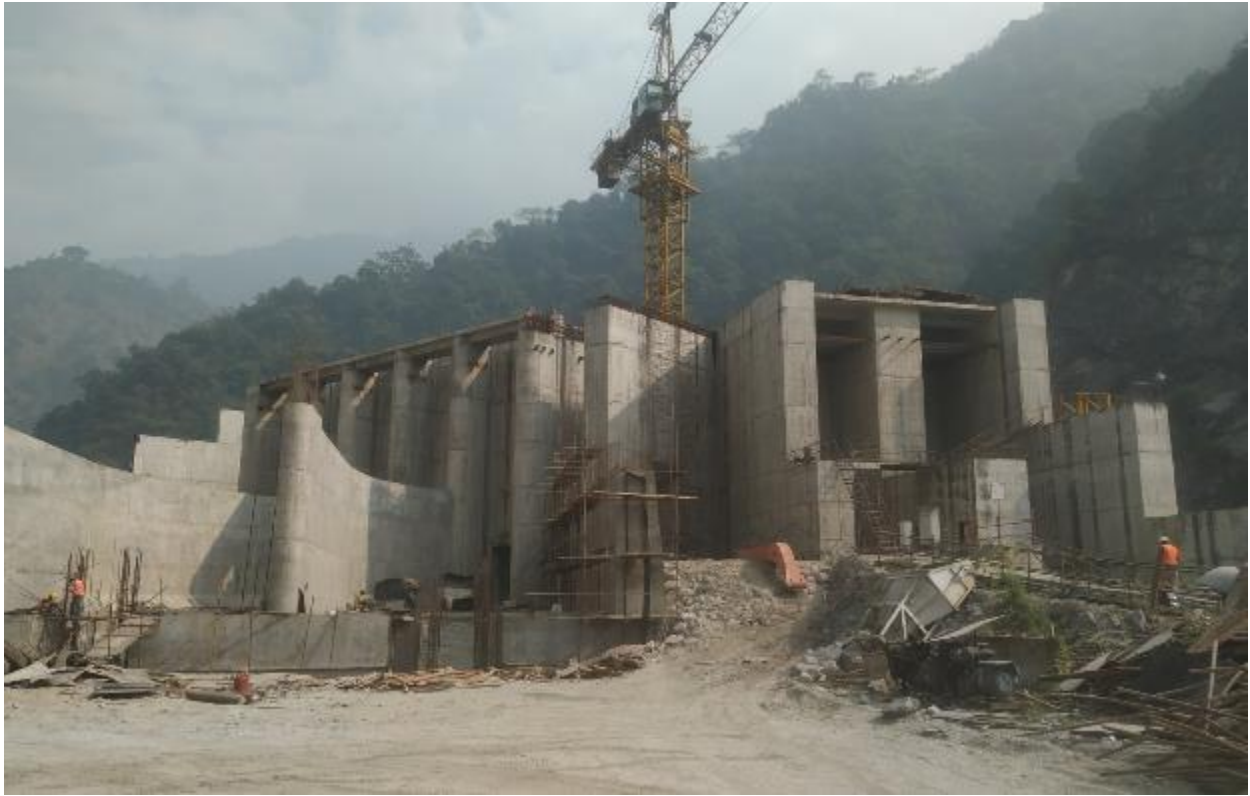
Figure 9: Intake and Undersluice section from downstream
