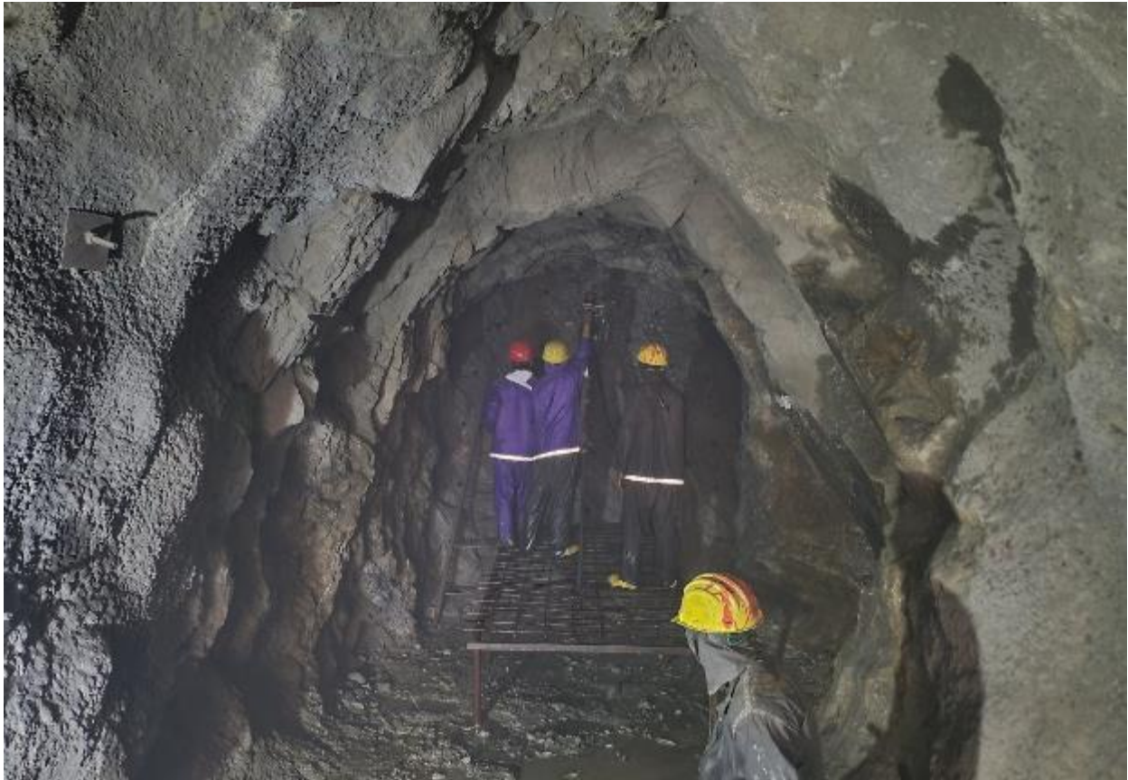
Figure 26: Face Drilling at Sediment flushing Tunnel
