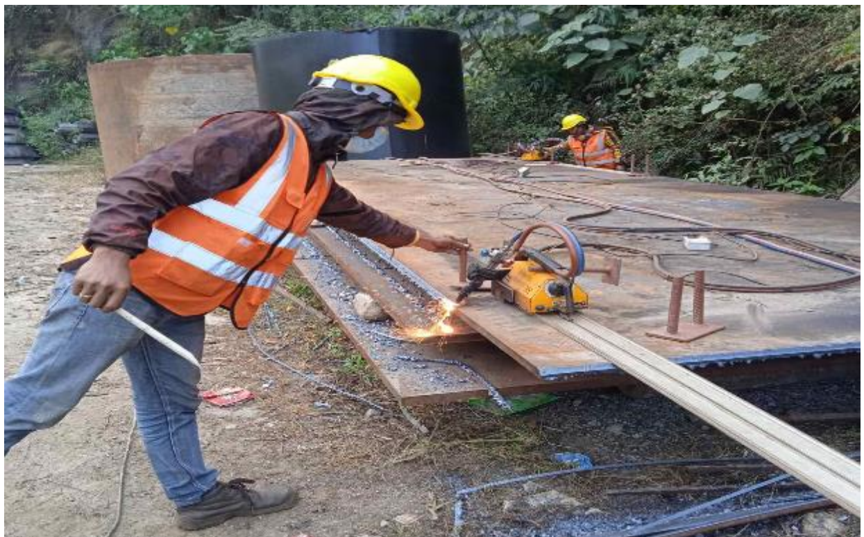
Figure 41: Cutting of plate for penstock pipe.
