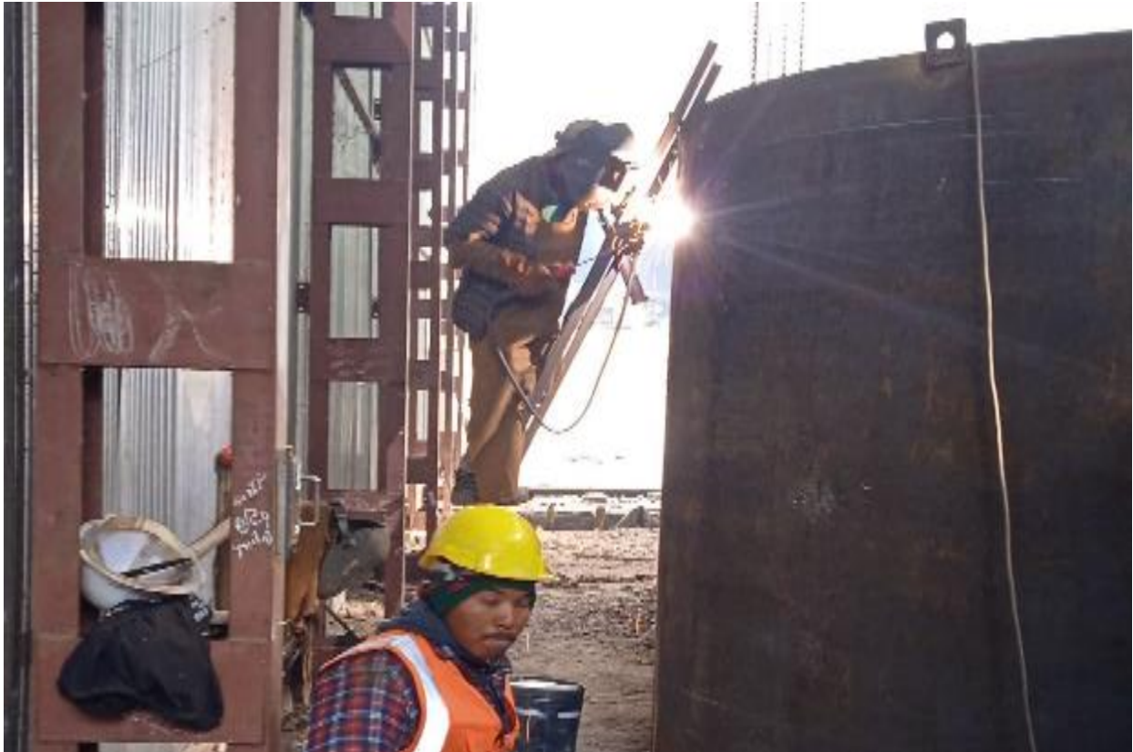
Figure 38: Welding work on penstock pipe
