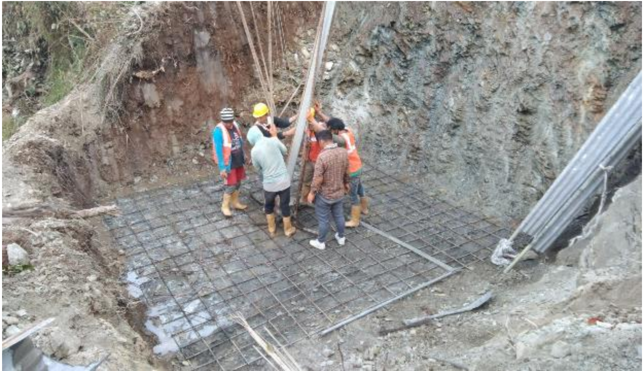
Figure 52: Rebar installation work of leg at AP24
