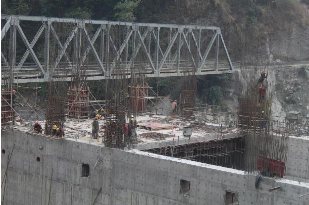
Figure 30: Reinforcement and formwork work at column in Powerhouse Bay 01
