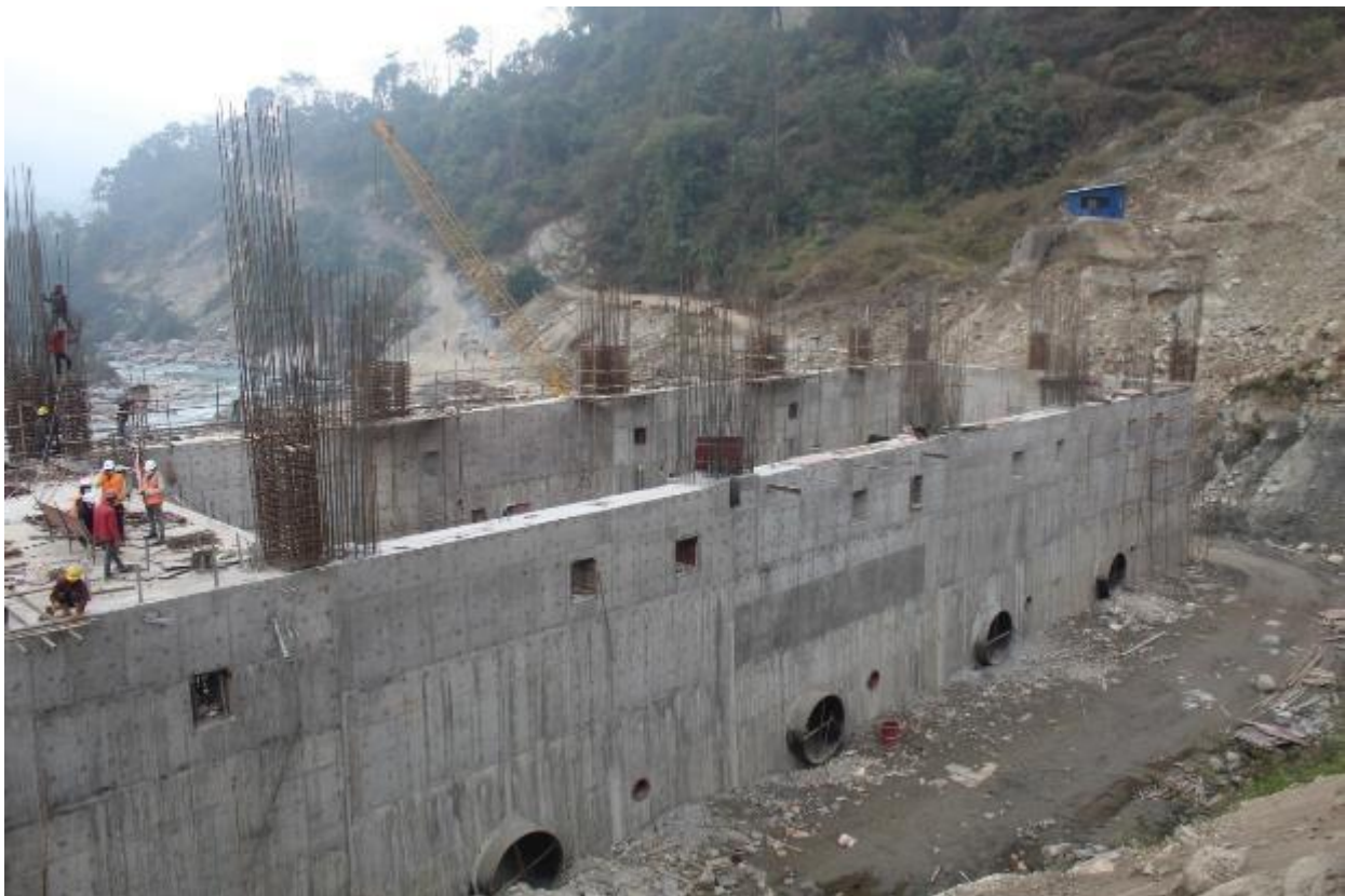
Figure 29: View of powerhouse from the upstream face
