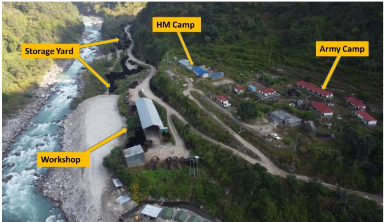
Figure 36: Aerial view of HM Camp, storage yard, workshop and Army camp
