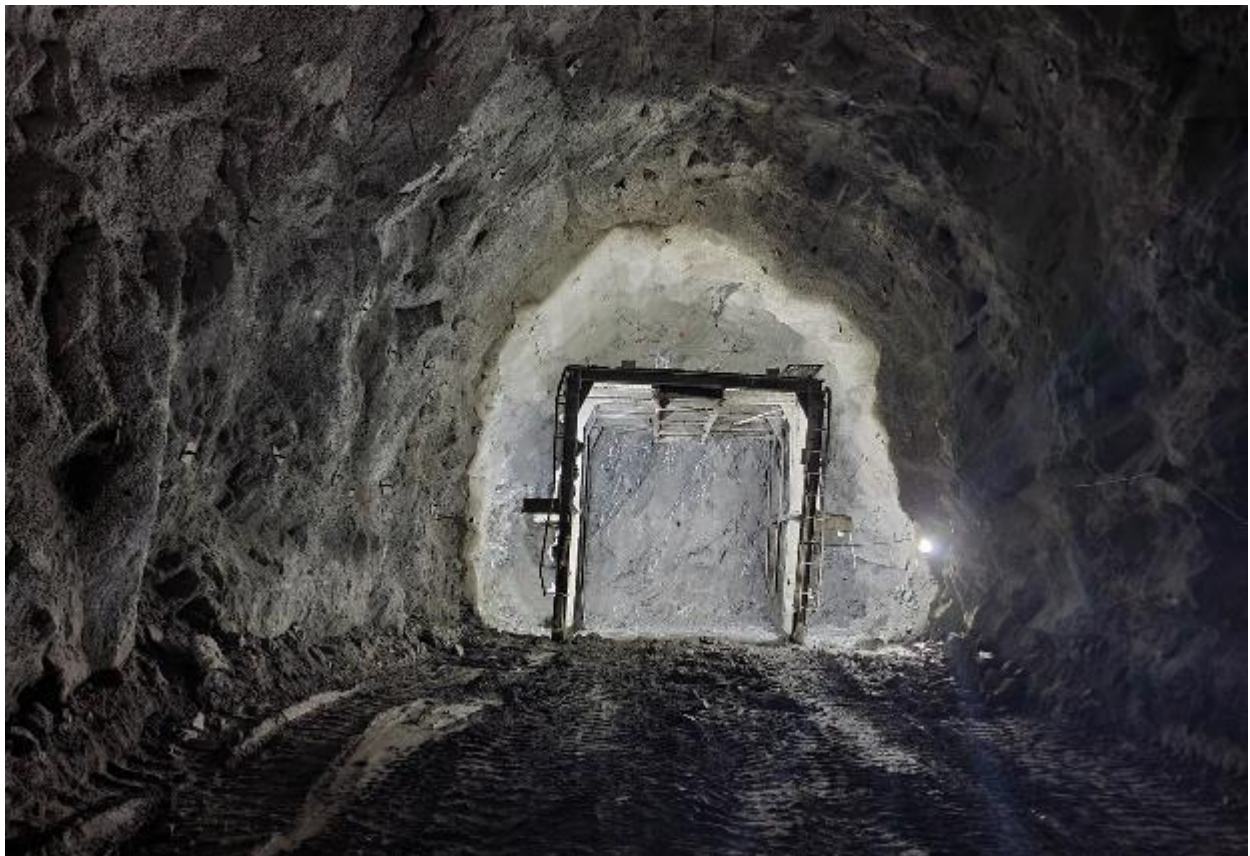
Figure 25: Scaling works at HRT from Outlet
