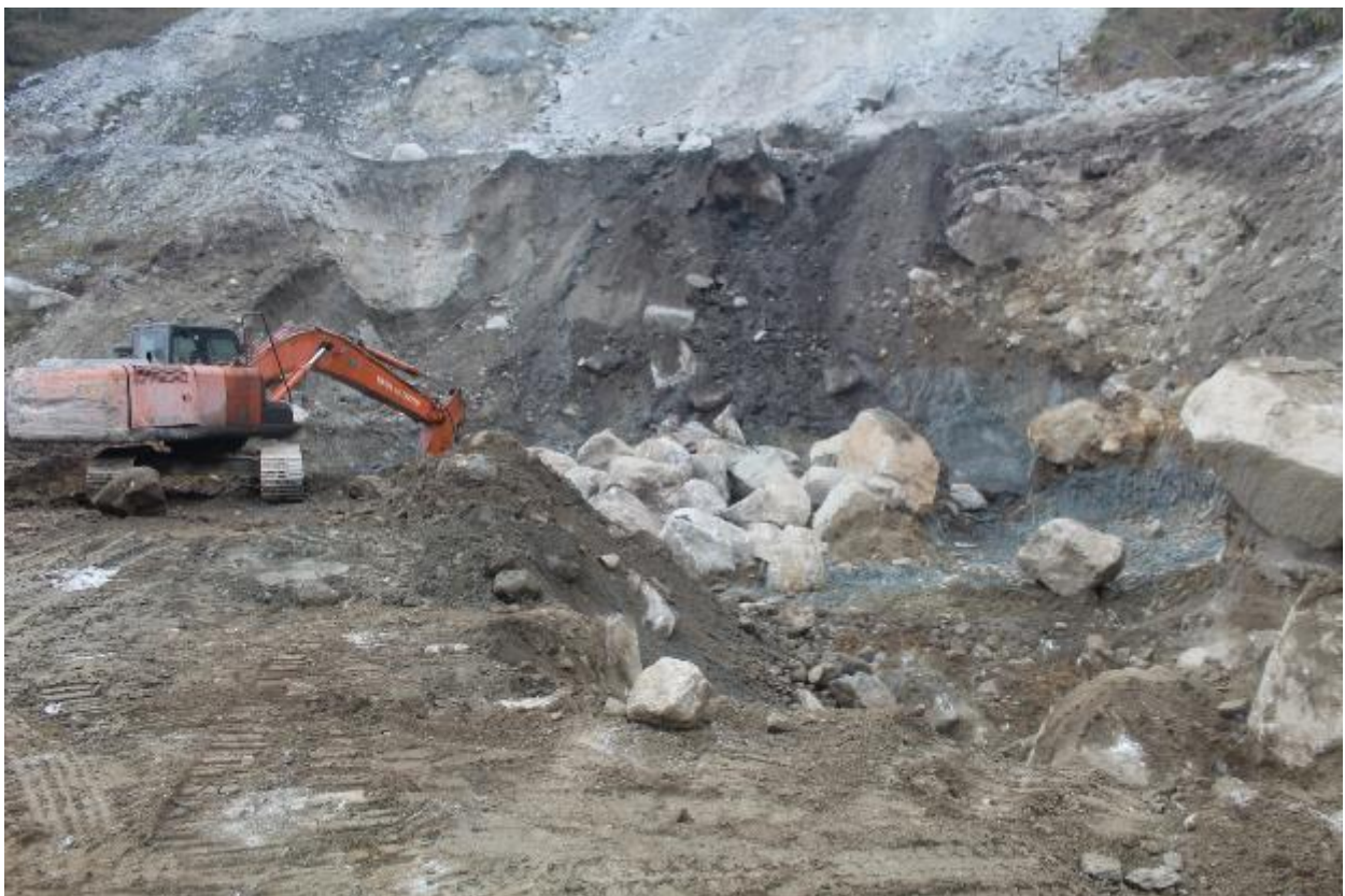
Figure 35: Excavation work ongoing at Penstock area
