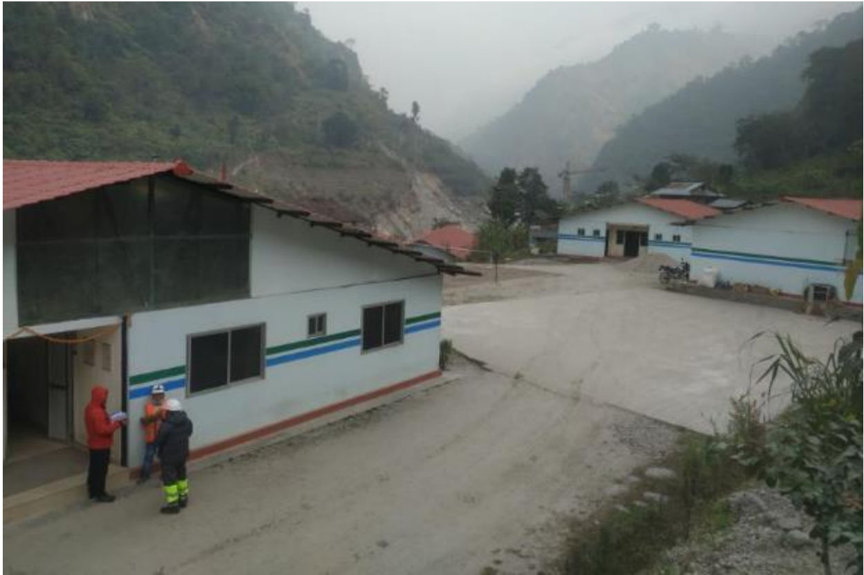
Figure 6: Employer's residential camp at Headworks (Simle)
