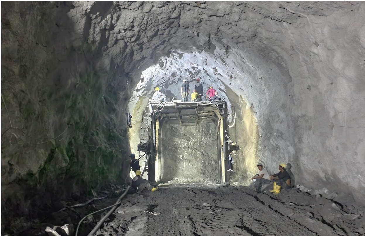
Figure 21: A view from HRT from adit
