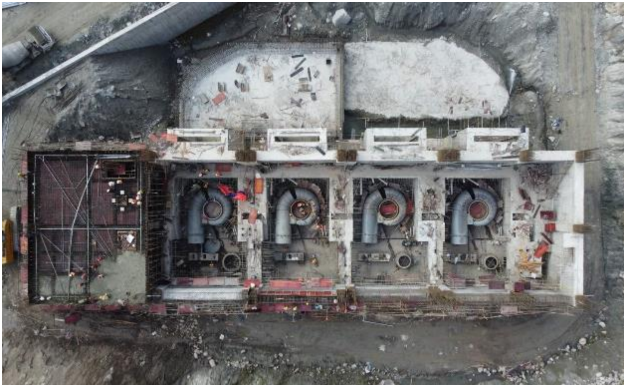
Figure 49: Aerial view of Powerhouse showing all 4 units Spiral case assembly
