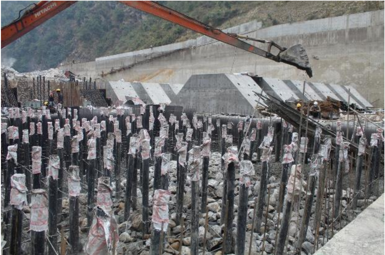
Figure 16: Installation of uplift pressure releasing pipes at stilling basin panel 03
