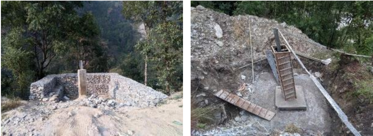
Figure 49: Stub erection and foundation works
