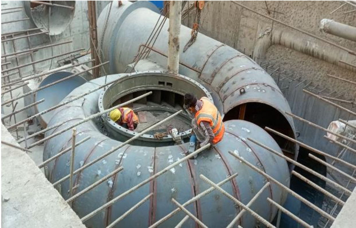
Figure 46: Unit 1 Spiral case segment being assembled and Tack Welding being done
