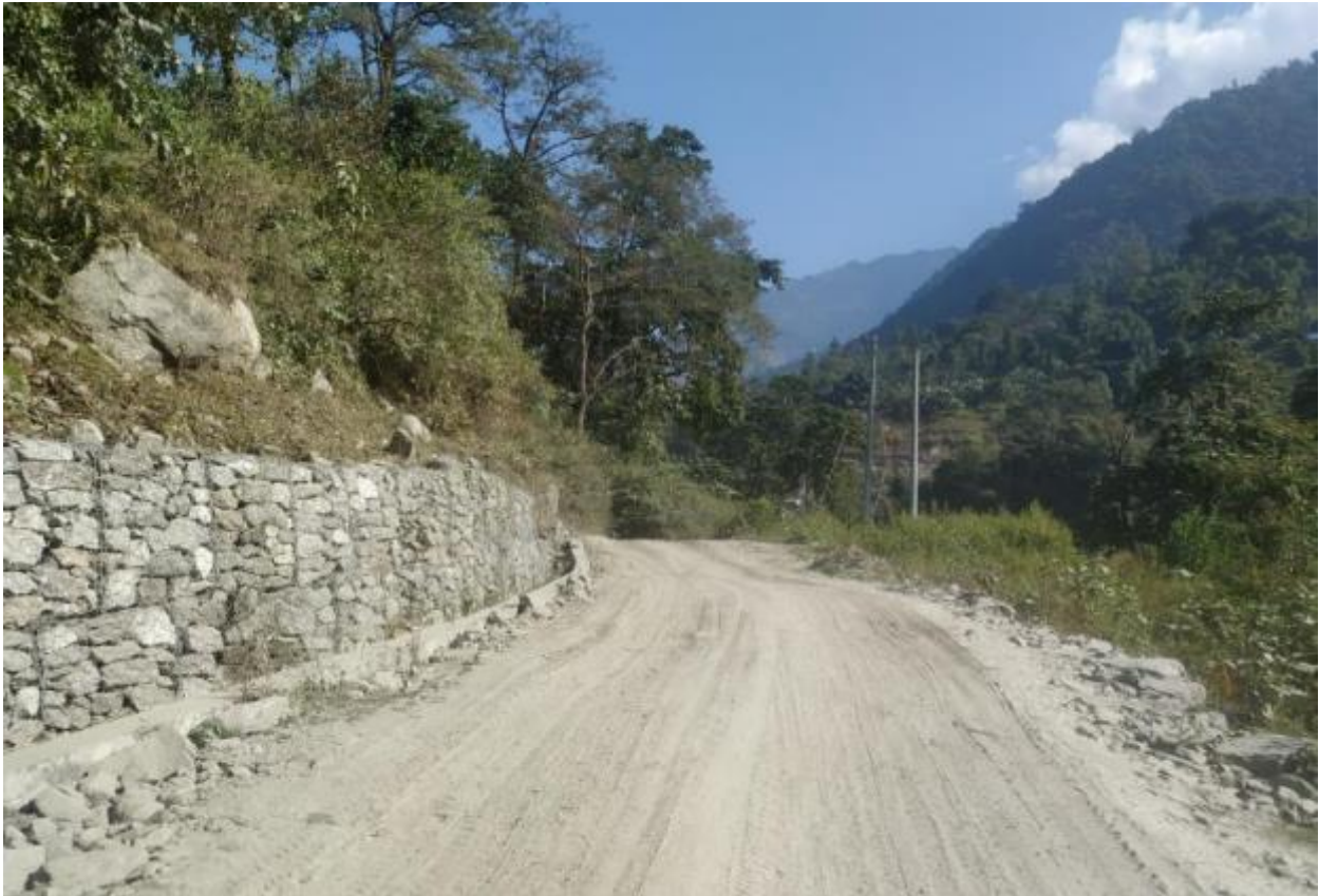
Figure 4: Gabion wall construction at new access road from Mitlung to Thumba
