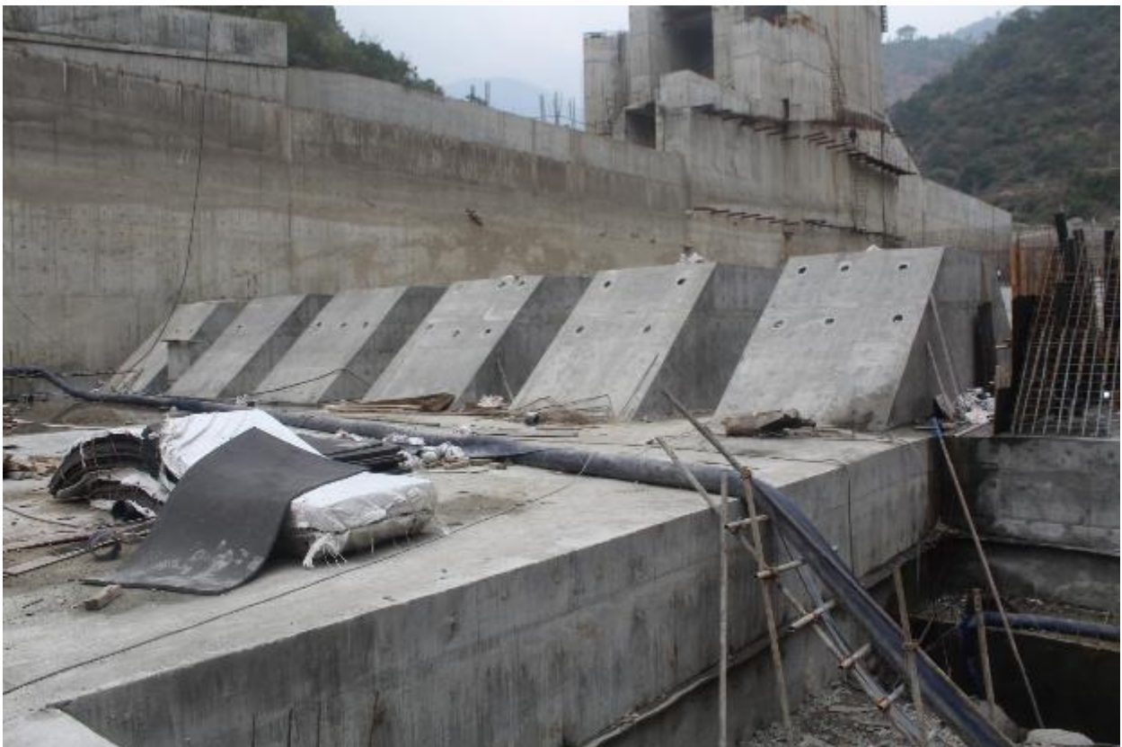
Figure 17: Completed concreting works at baffle blocks Weir stilling basin Panel 06 & 07
