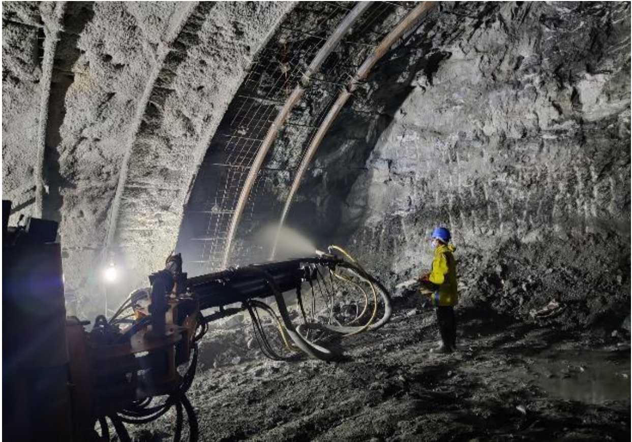
Figure 24: Shotcreting at SB 01
