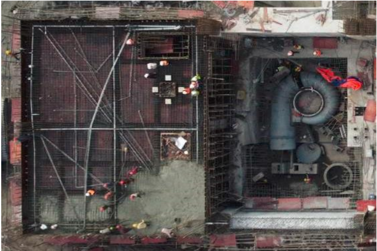
Figure 48: Imbedded pipes installation at service bay
