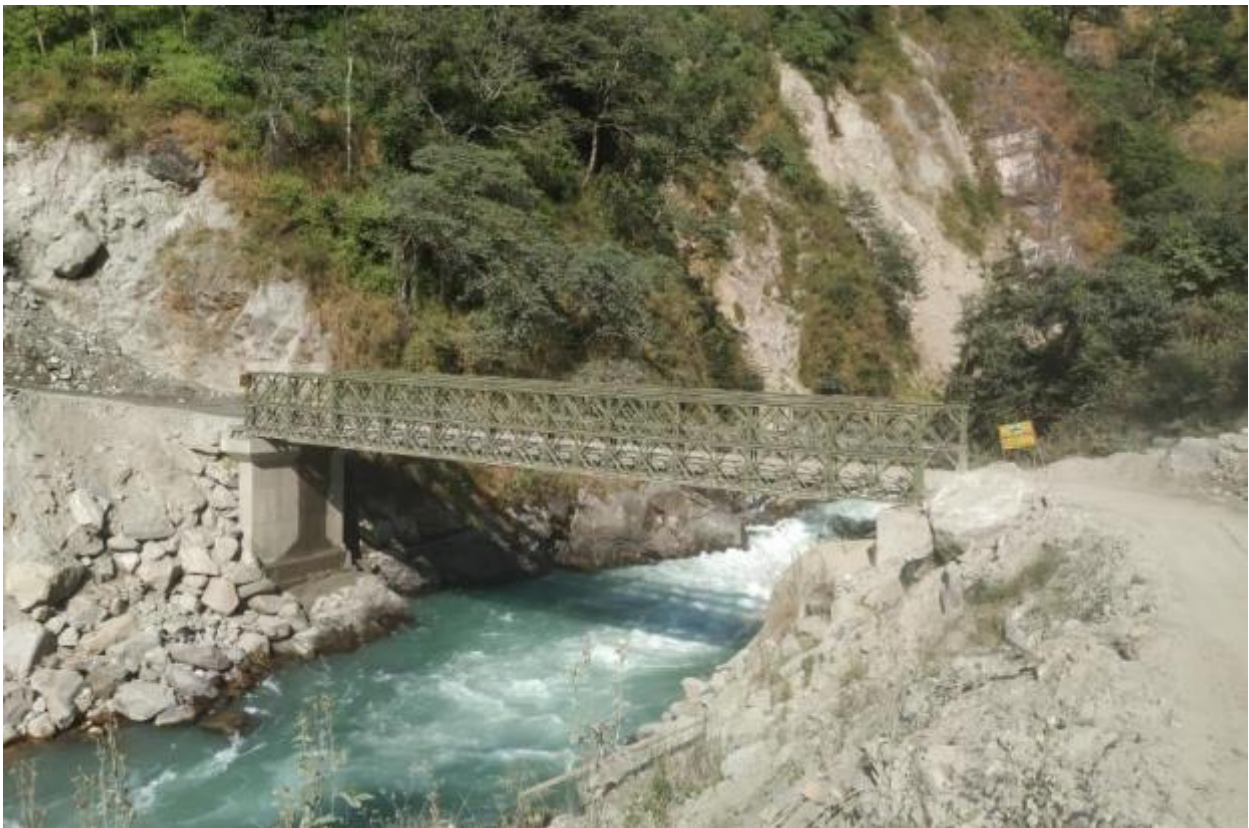
Figure 5: Bailey Bridge at Budidaha section
