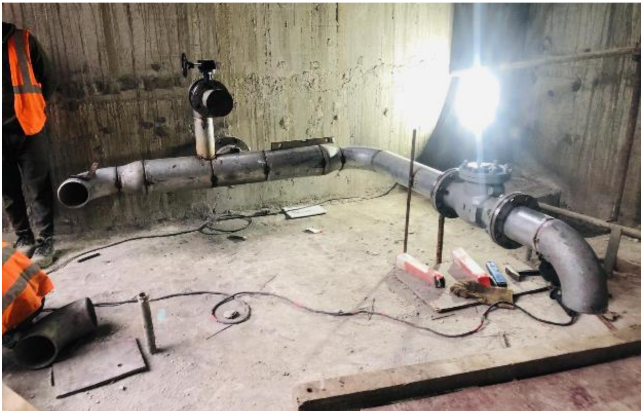
Figure 45: Installation of Butterfly valves/Check valves of Leakage drainage system
