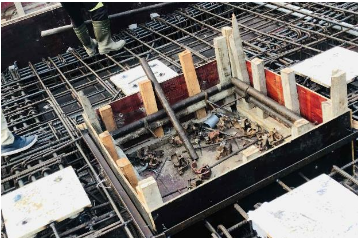
Figure 47: Installation of Support plate for Rotor maintenance pier
