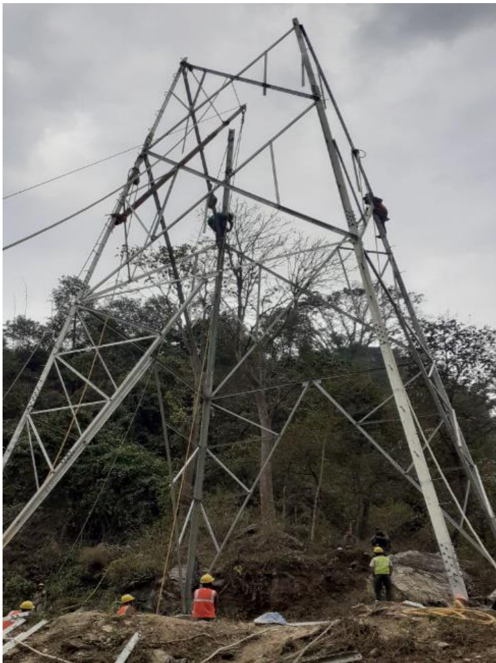
Figure 51: Tower erection works ongoing at AP16
