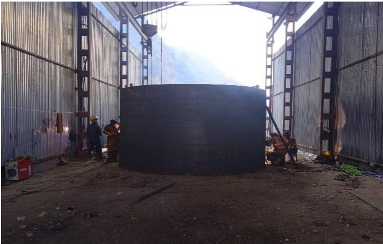
Figure 43: Welding works on penstock pipe
