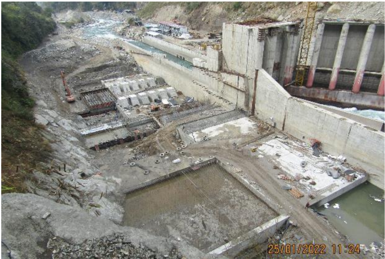
Figure 14: Aerial view of concreting works at stilling basin
