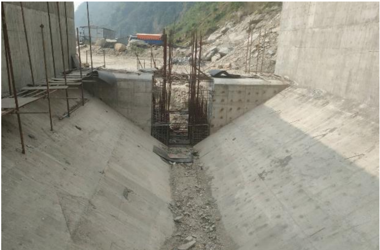
Figure 10: A view of Gravel trap
