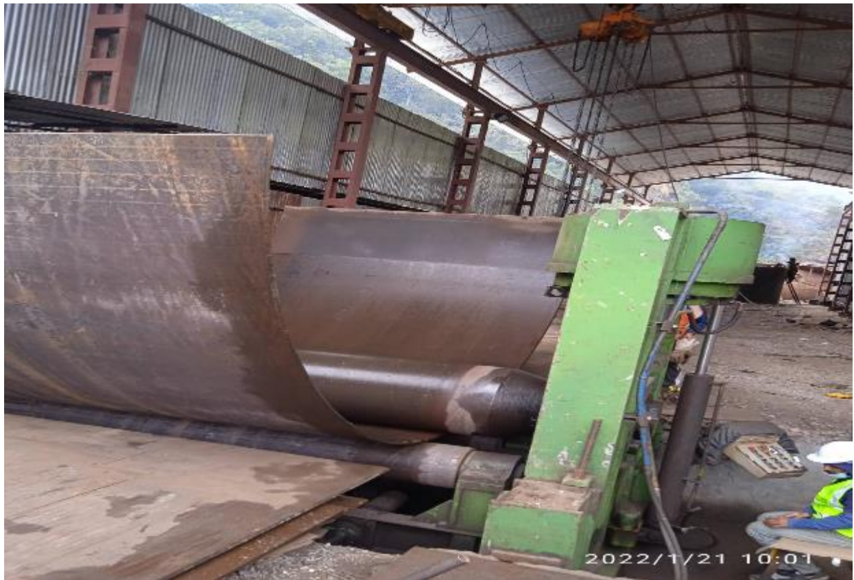
Figure 40: Rolling of penstock pipe
