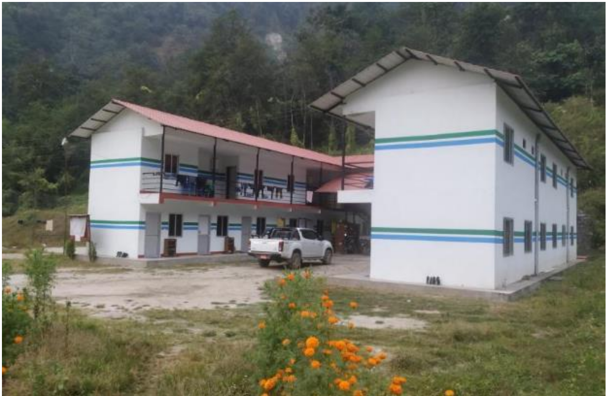
Figure 7: Employer's residential camp at Powerhouse (Lorindin)
