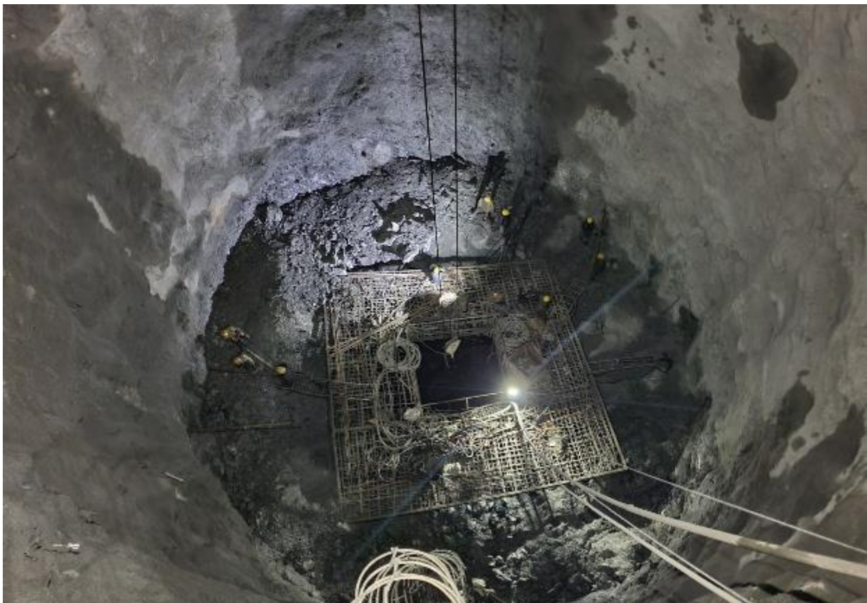
Figure 26: Face Drilling at Sediment flushing Tunnel
