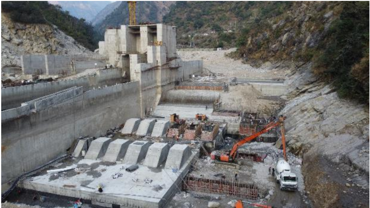
Figure 12: Headworks (A view of Undersluice and weir stilling basin from downstream)
