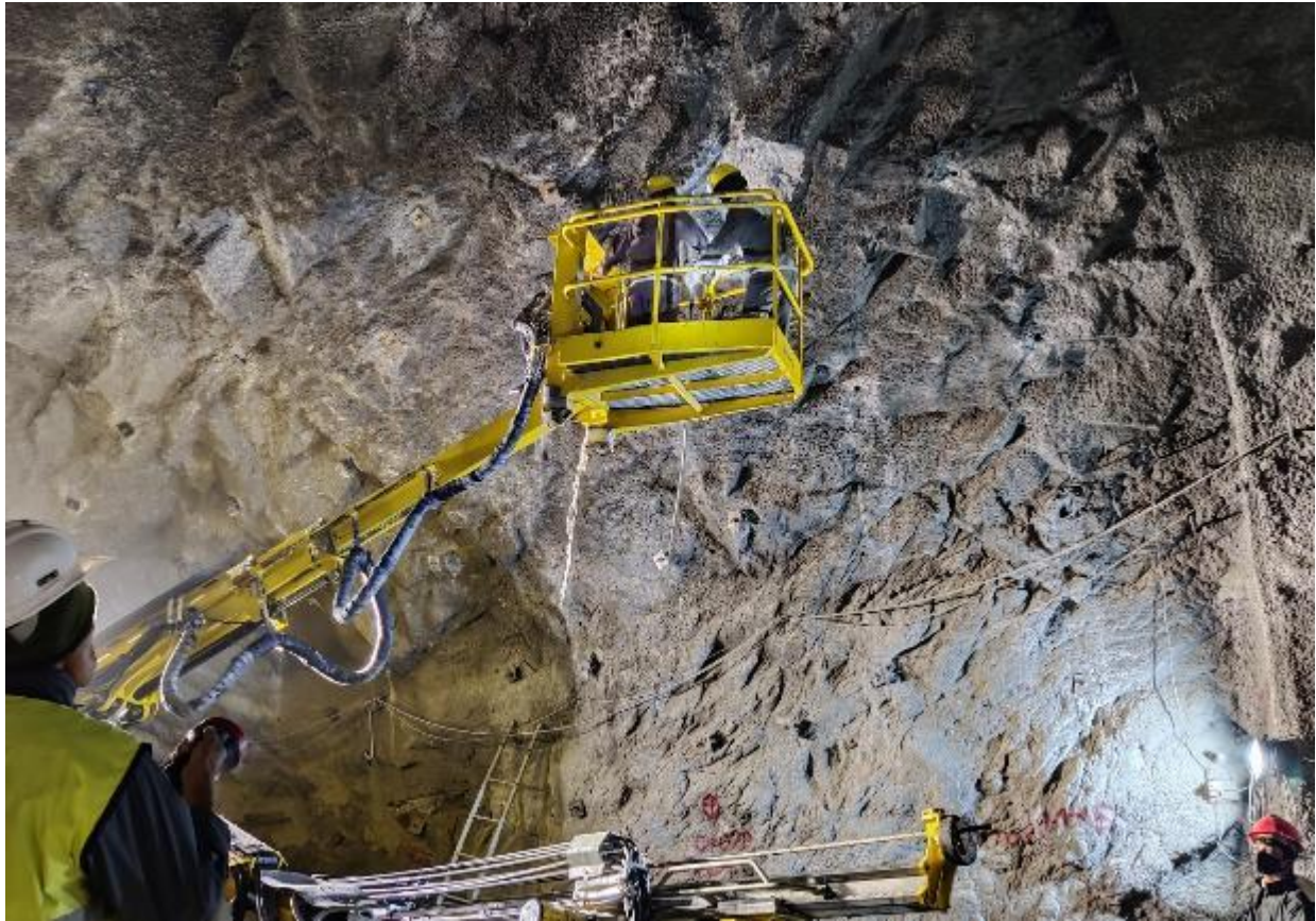
Figure 22: Face drilled by Boomer at SB 01
