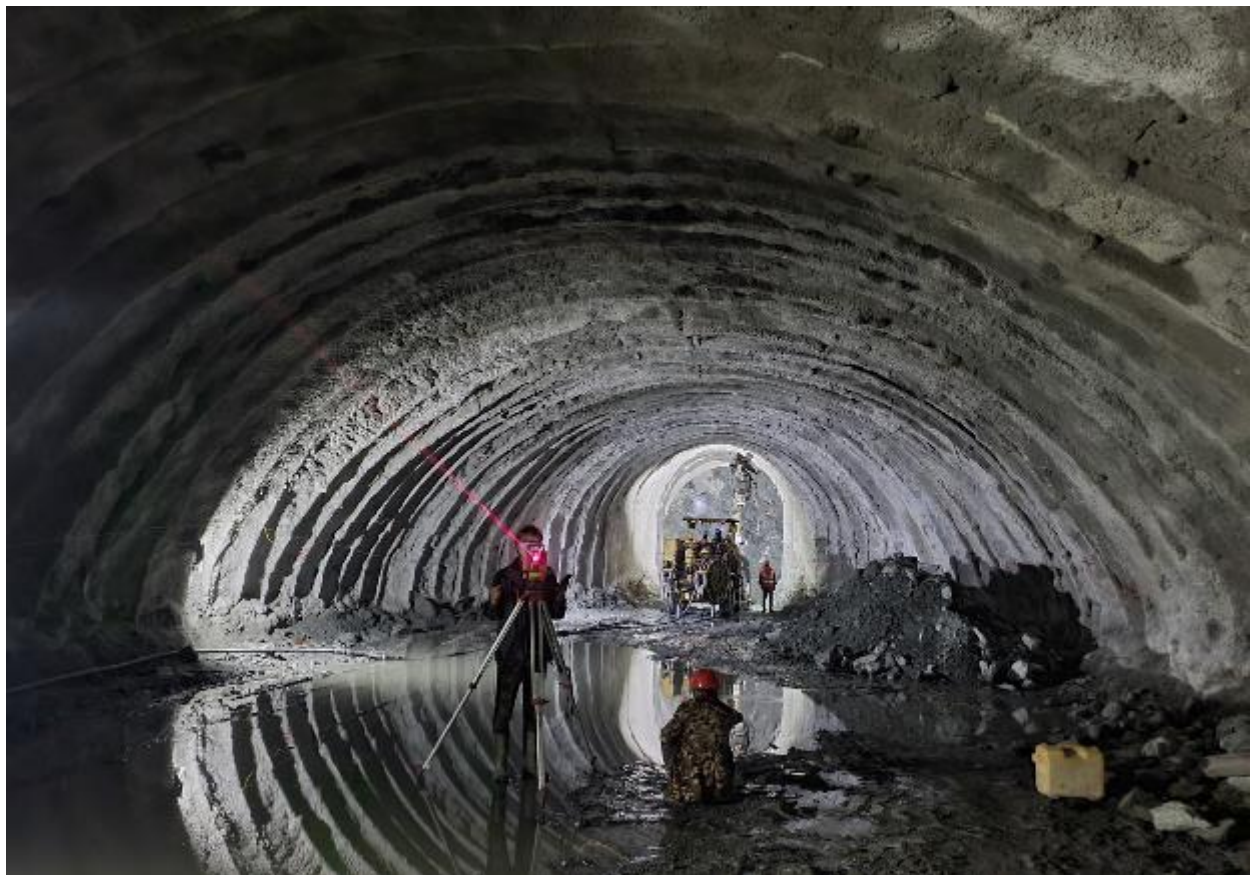
Figure 23: Excavation works at Connecting Tunnel junction (SB-02) using Boomer
