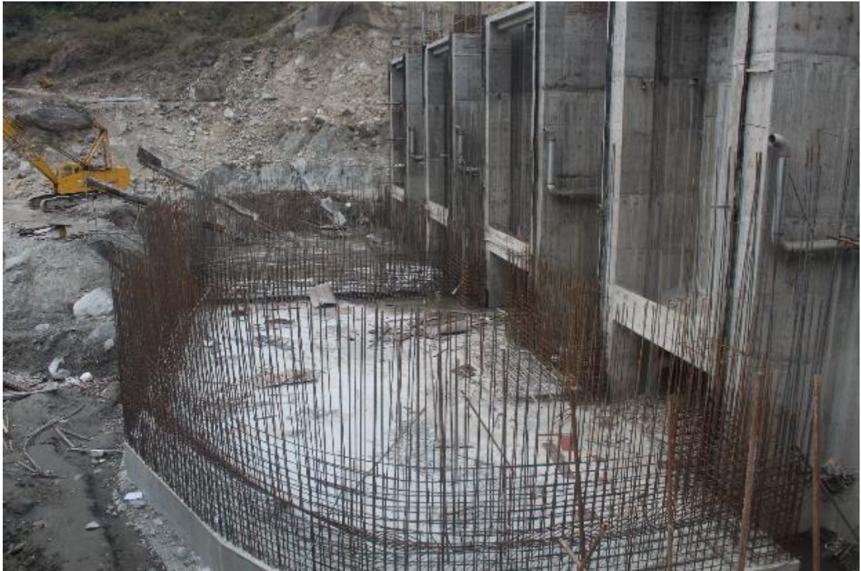
Figure 34: Reinforcement works at Tailrace culvert Panel 01 & 02
