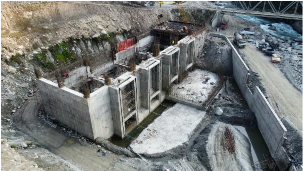
Figure 33: An aerial view of Powerhouse
