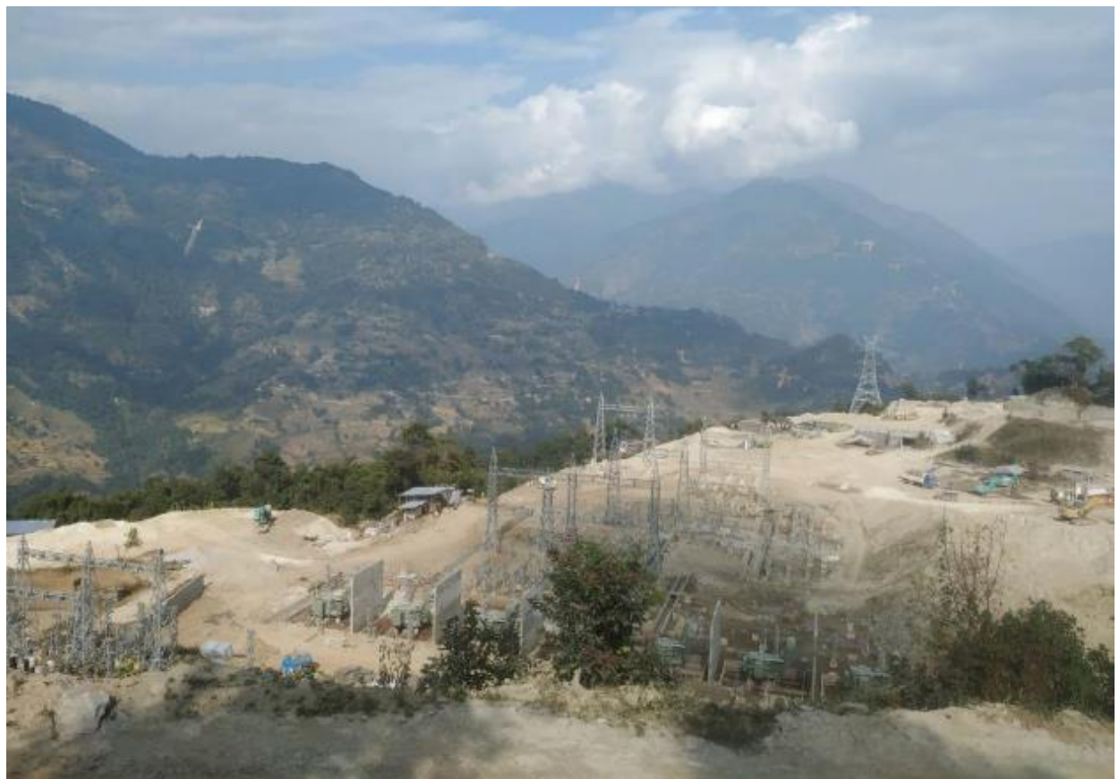
Figure 50: Dhunge-Sanghu substation (NEA Project)
