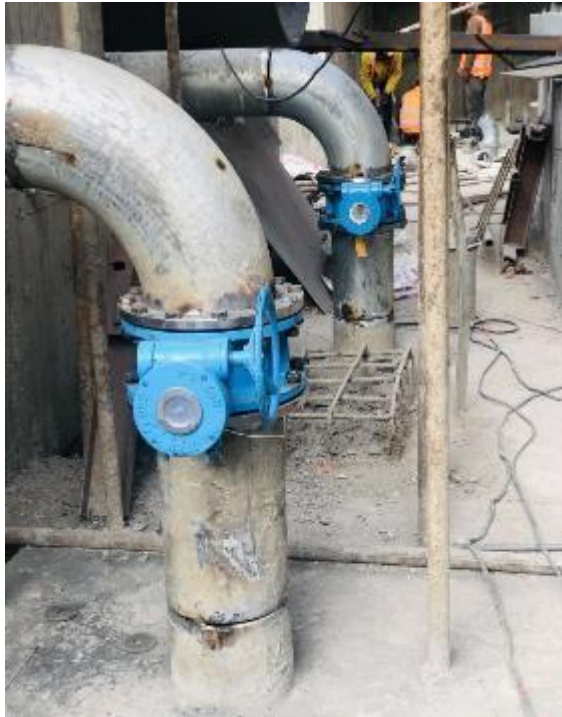
Figure 46: Installation of Butterfly valves (left) and tailrace measurement pipes (right)
