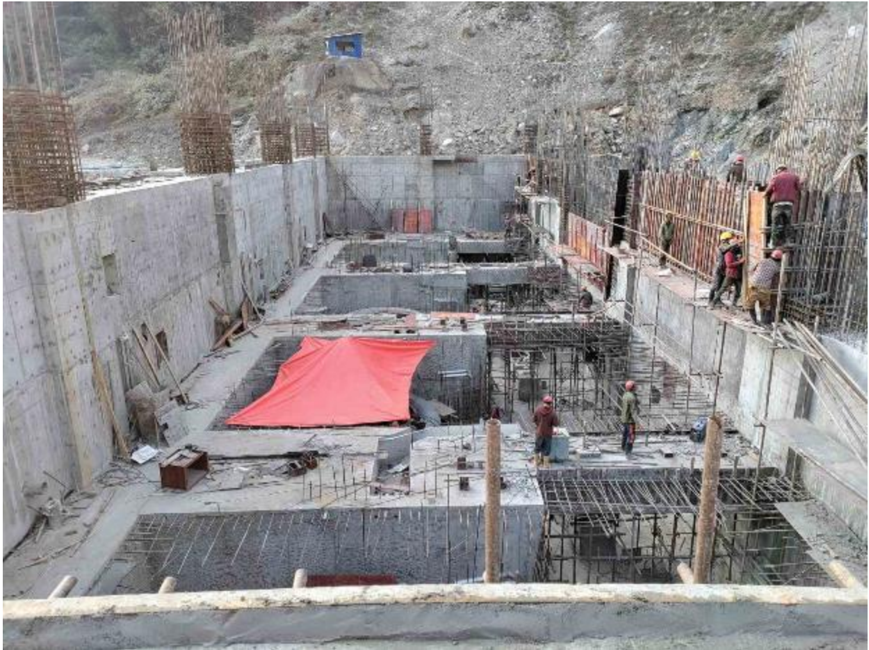
Figure 32: Side view of Powerhouse MTHP 73 MW
