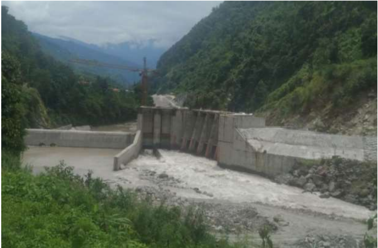
Figure 12: Aerial view of headworks with completed weir to the left
