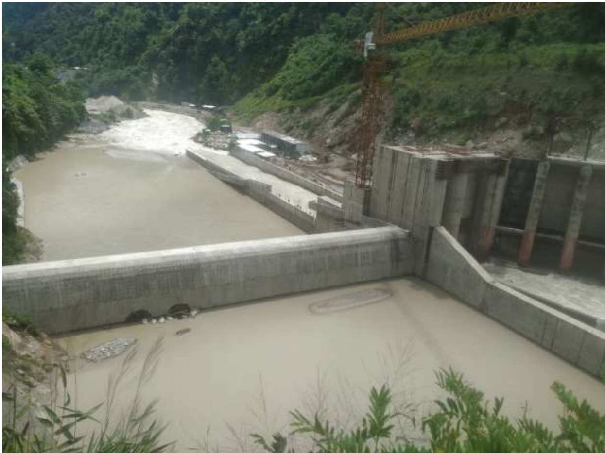
Figure 13: Main weir body (Completed)
