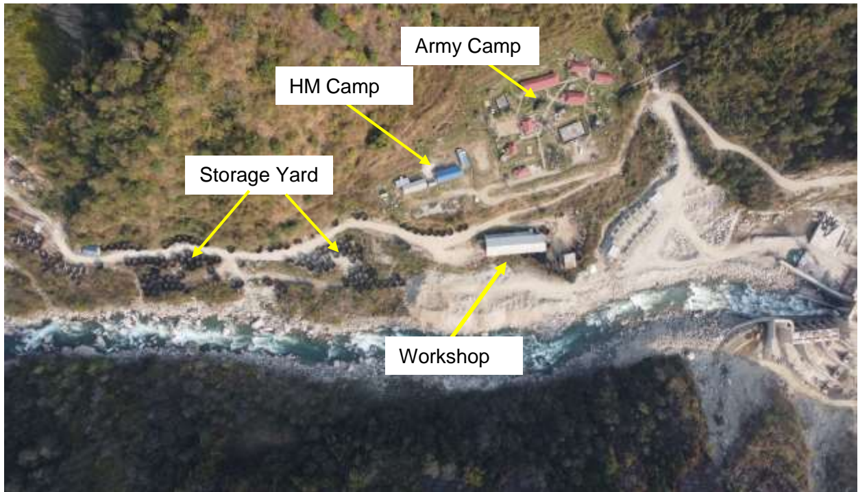
Figure 30: Aerial view of HM Camp, storage yard, workshop and Army camp
