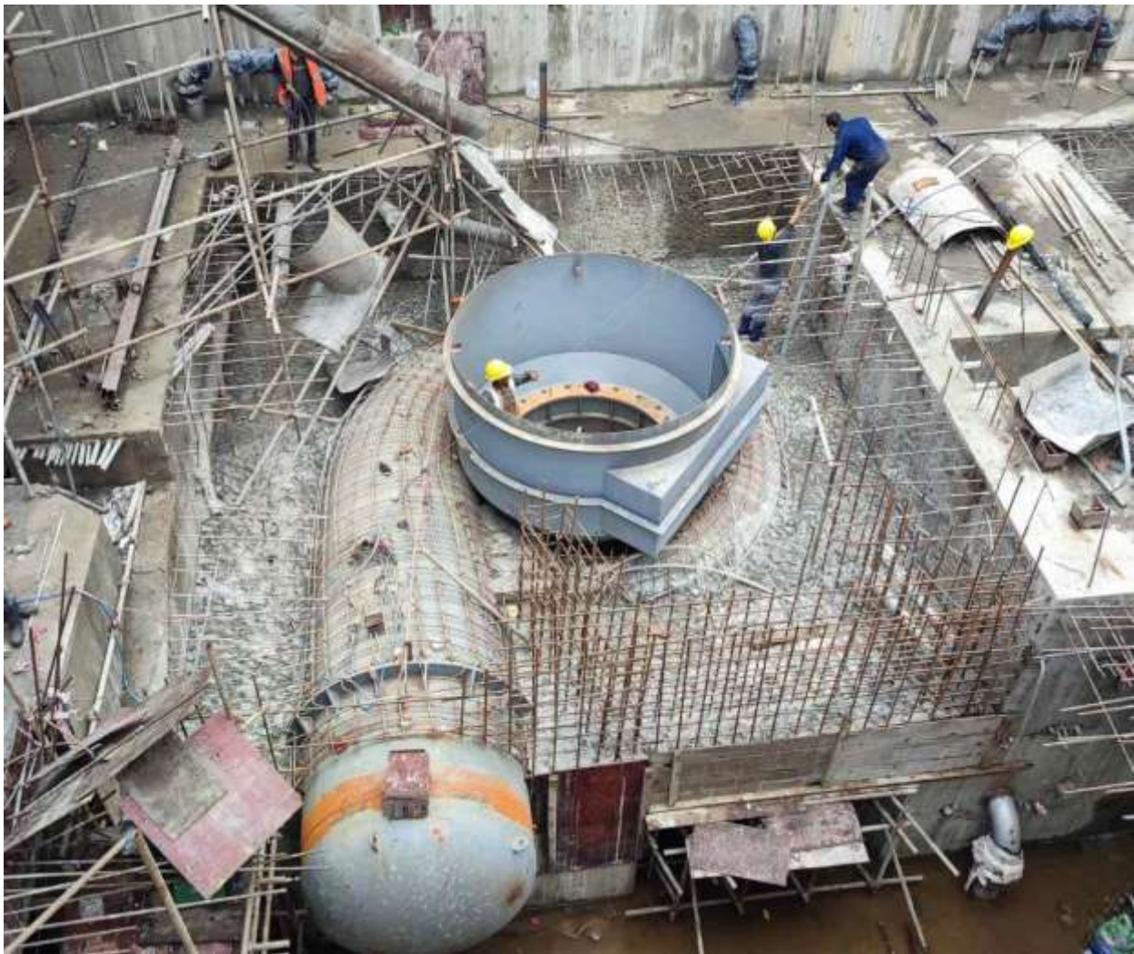
Figure 51: Installation of bottom part of Pit Liner at Unit 1
