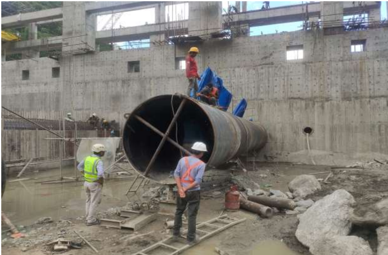
Figure 33: Erection work(Unit 1) (Dia: 2.0 m and thk: 20 mm)
