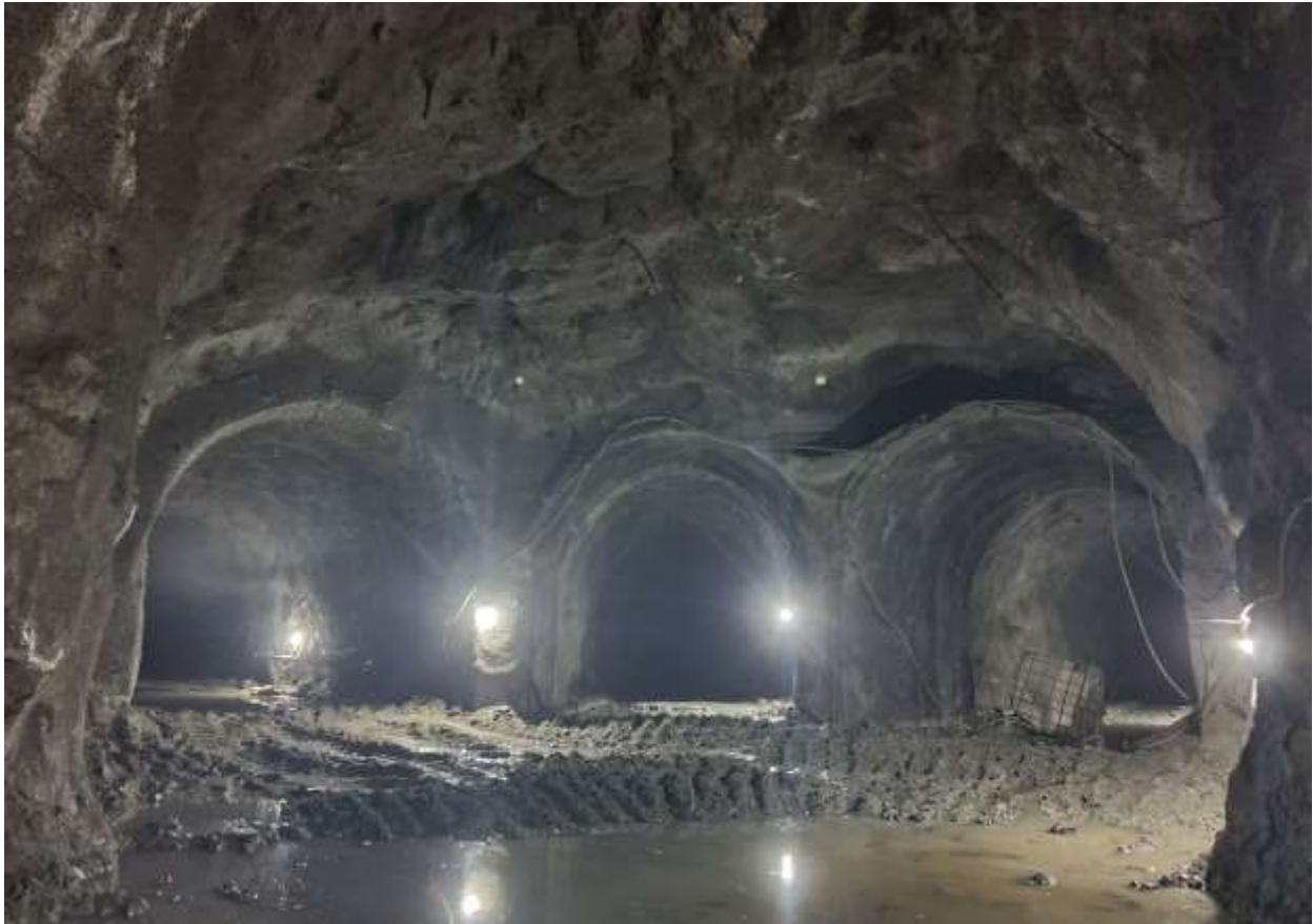
Figure 21: Connecting tunnel junction point
