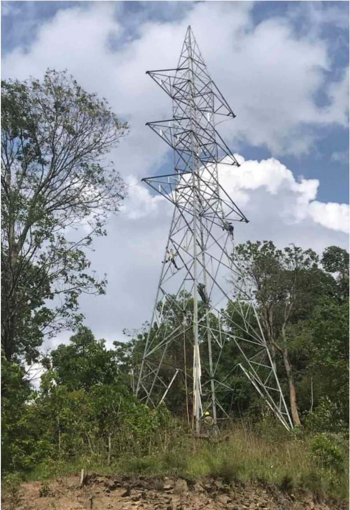
Figure 59: Tower erection works completed at AP16
