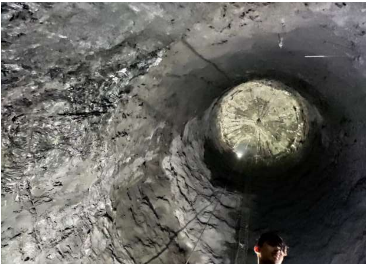
Figure 24: A view of Surge Shaft from invert
