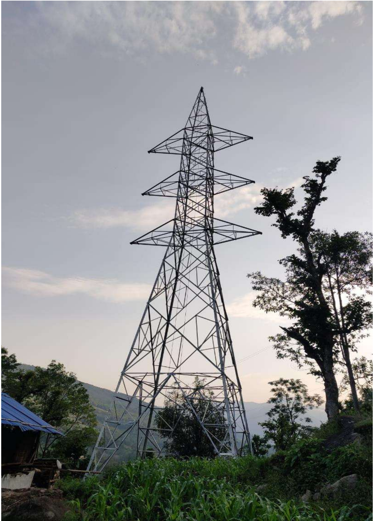
Figure 60: Tower erection works completed at AP03
