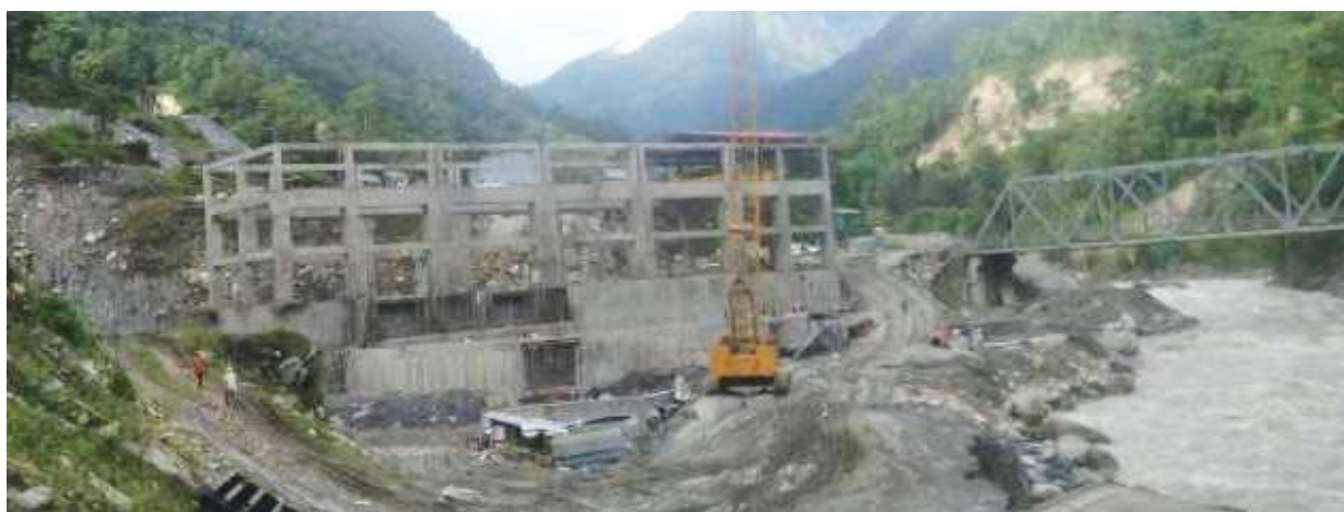
Figure 25: A view of powerhouse from downstream
