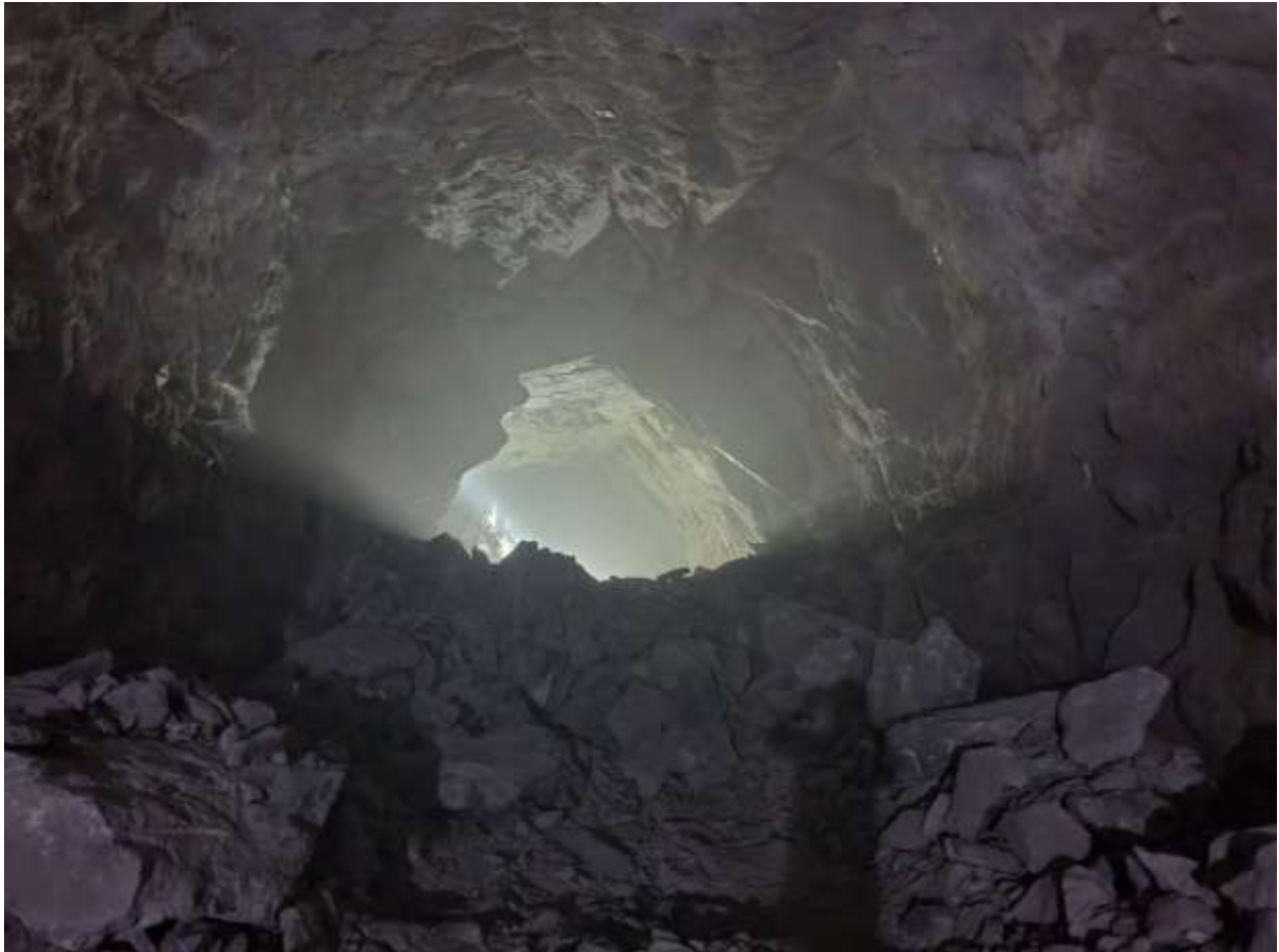
Figure 16: A view of HRT breakthrough at chainage 1+545.37
