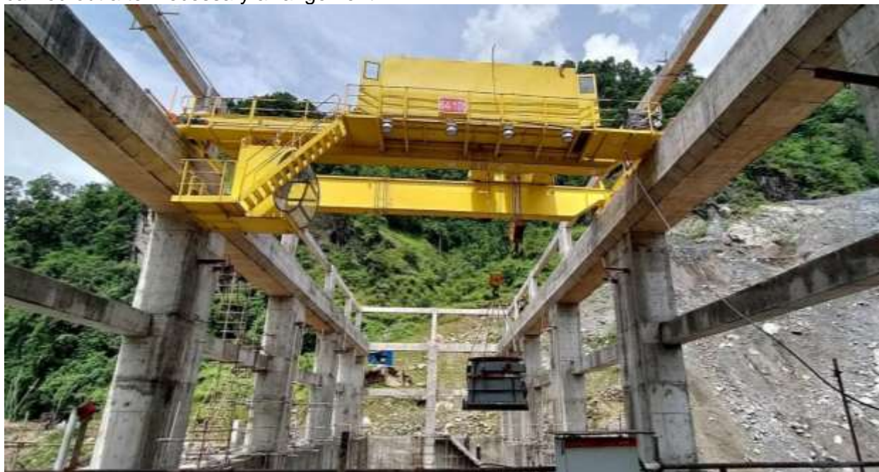
Figure 48: EOT crane being commissioned with small load
