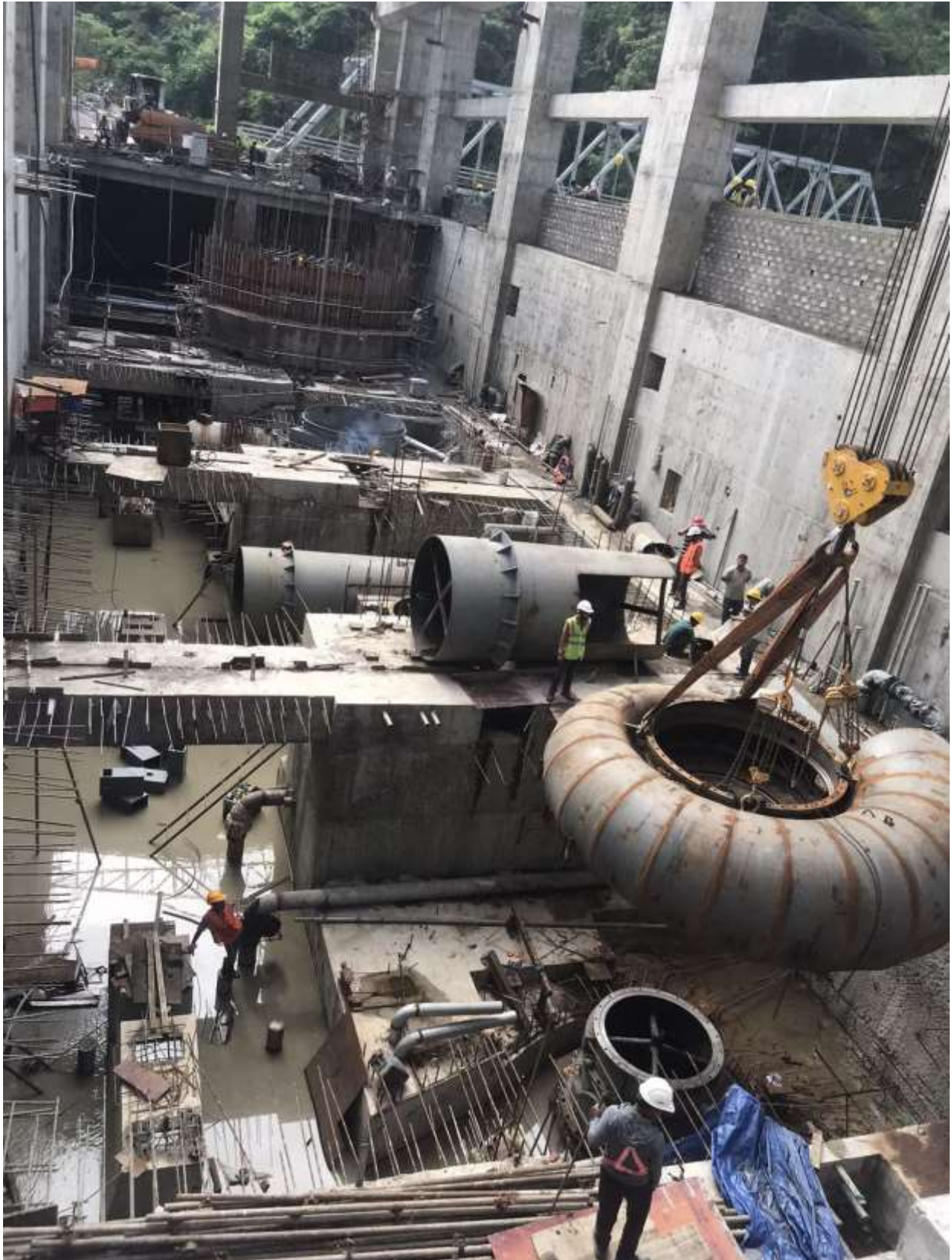
Figure 46: Installation of spiral case using EOT crane after cone installation
