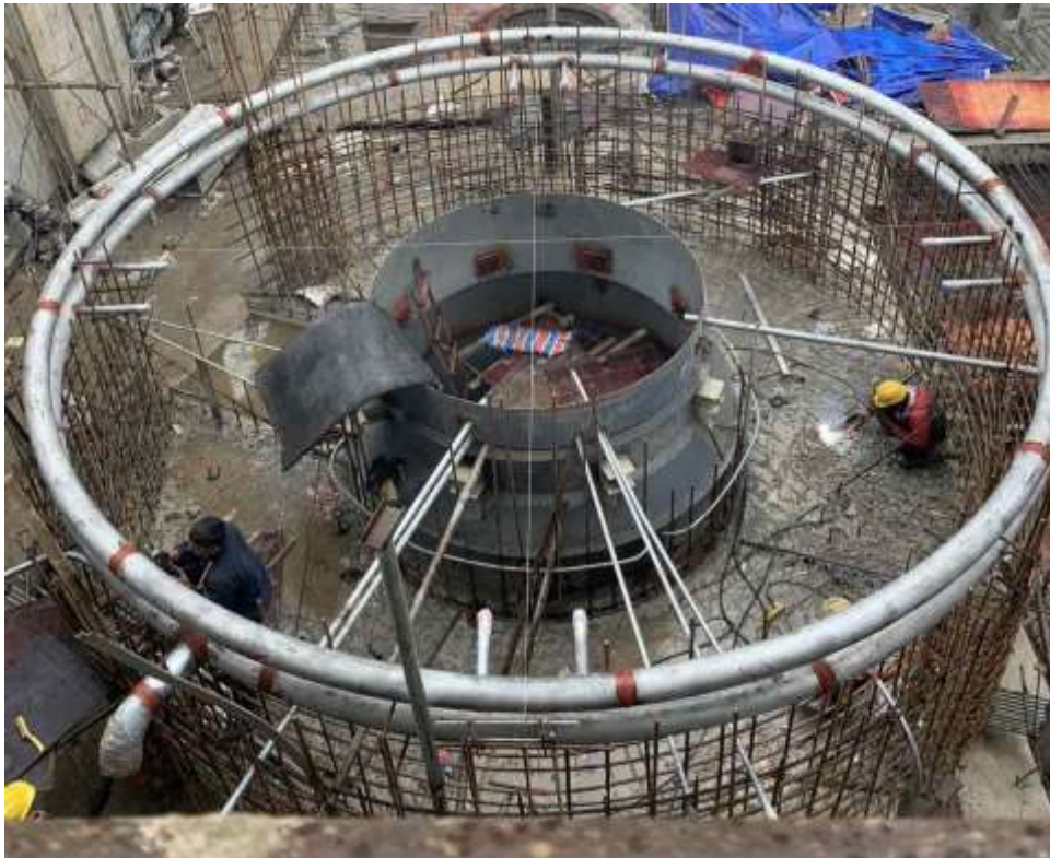
Figure 53: Installation of colling pipes for stator
