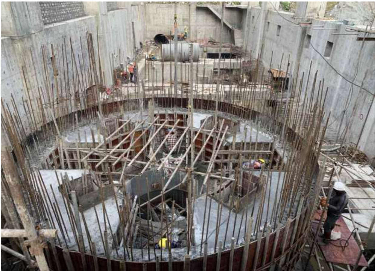
Figure 55: View of Pit Liner after fourth lift concreting
