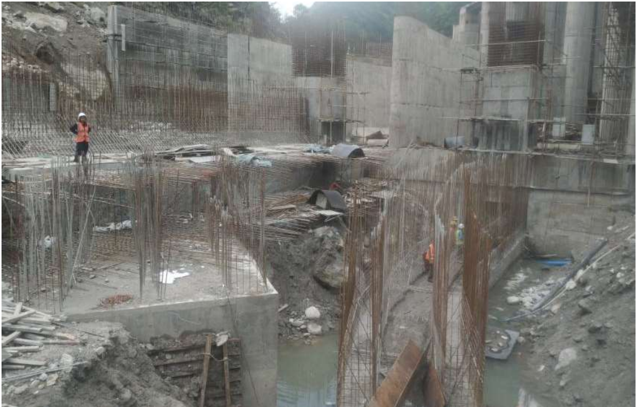
Figure 9: Rebar and concrete works in gravel flushing culvert
