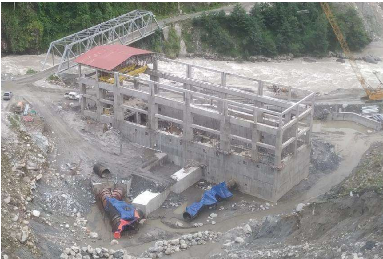
Figure 27: An aerial view of Powerhouse
