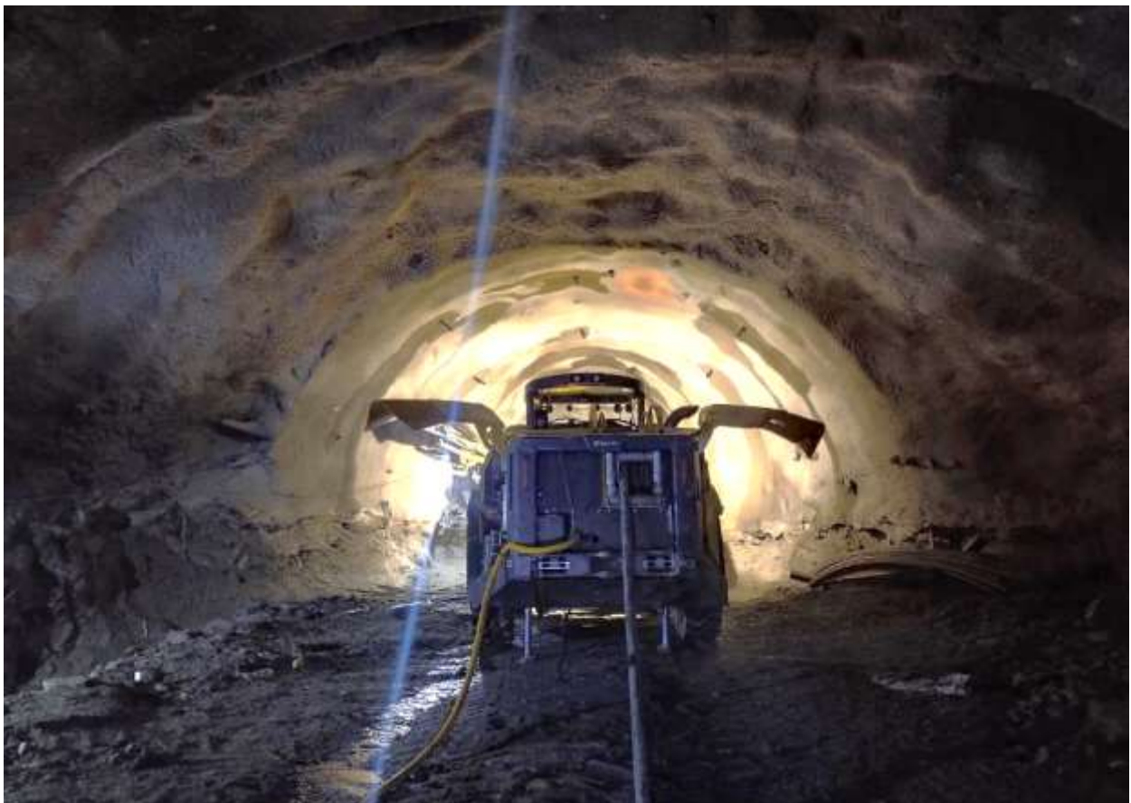
Figure 20: A view of drilling at the crown at SB-02 using Boomer
