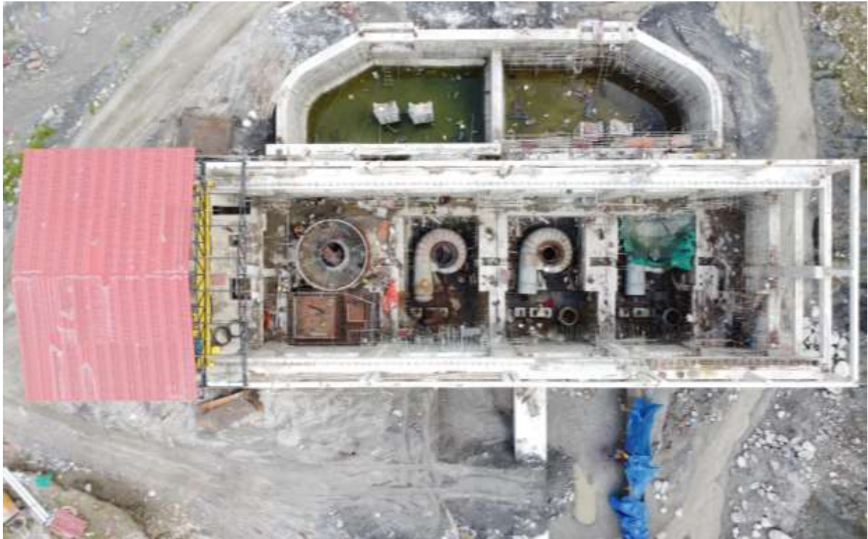
Figure 26: Top view of powerhouse
