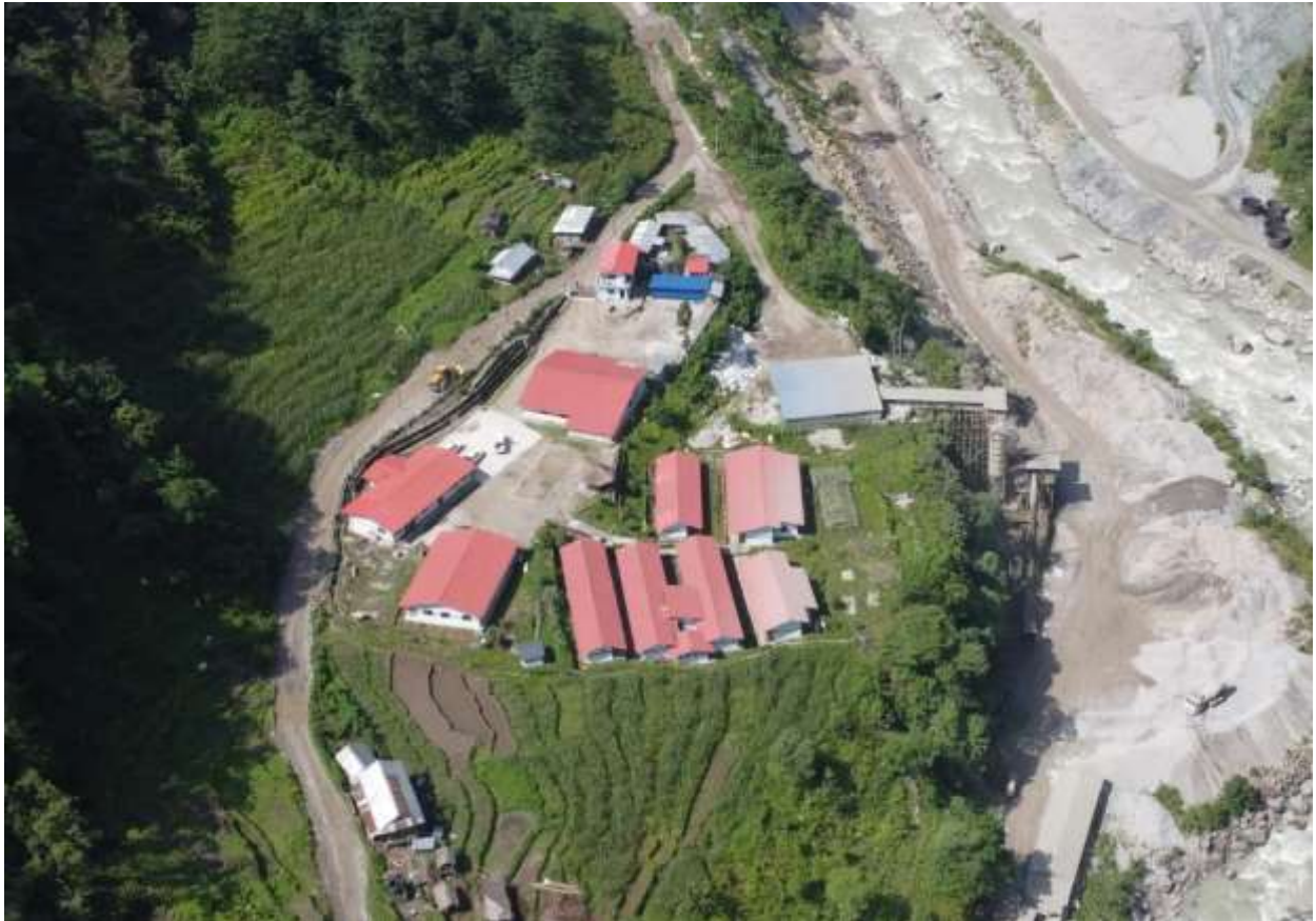
Figure 5: Employer's residential camp at Headworks (Simle)
