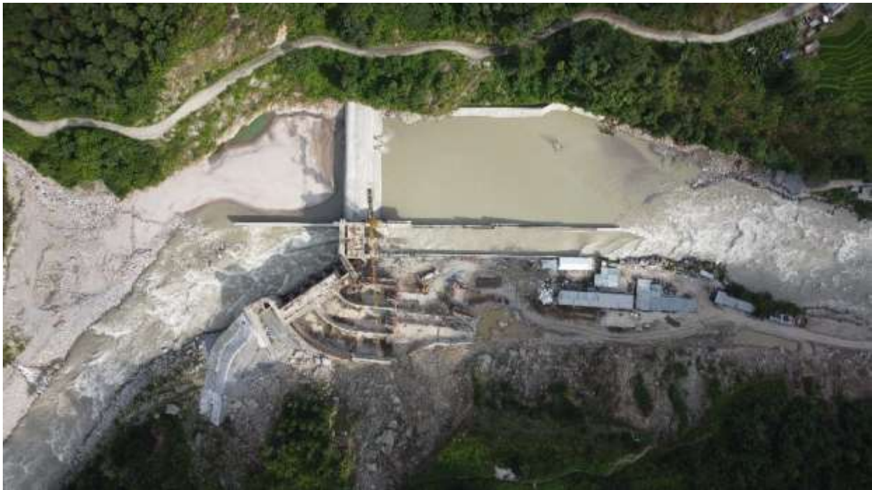
Figure 7: Aerial view of Headworks
