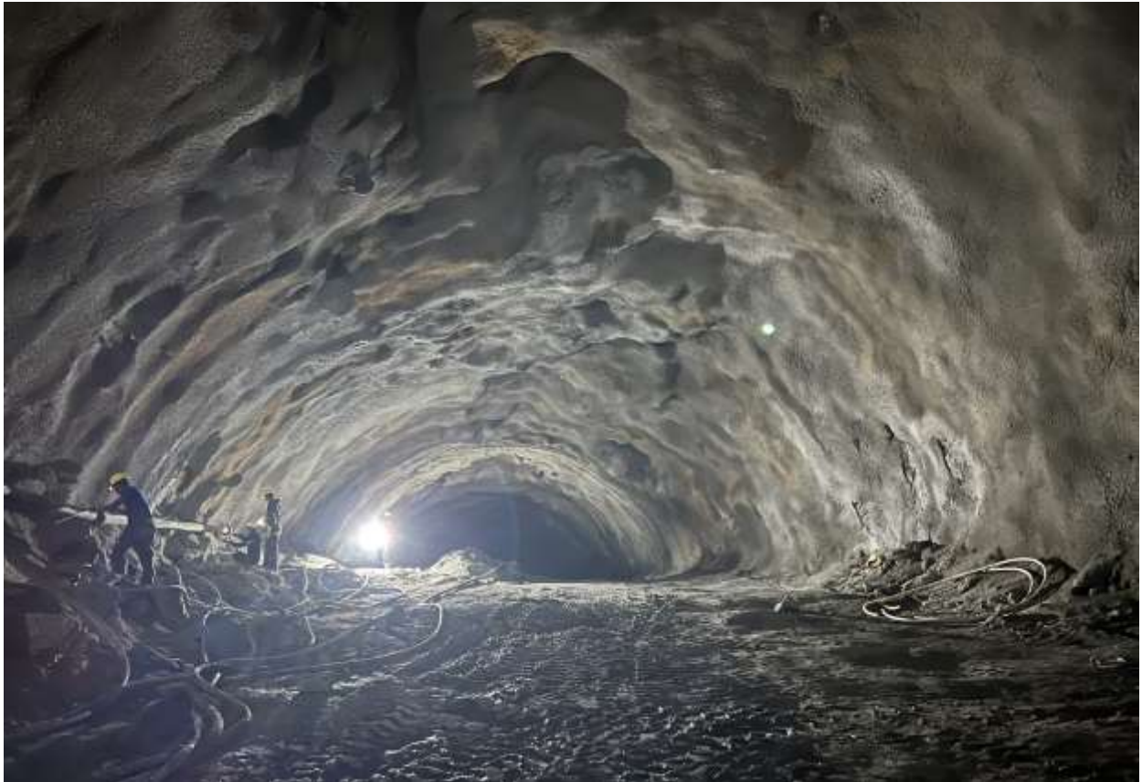
Figure 23: A view of Settling Basin 02
