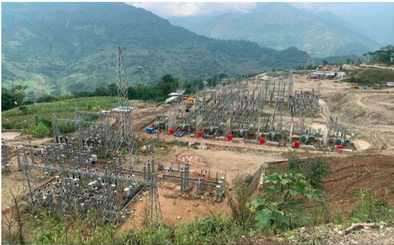
Figure 58: View of Interconnecting substation at Dhungesaghu
