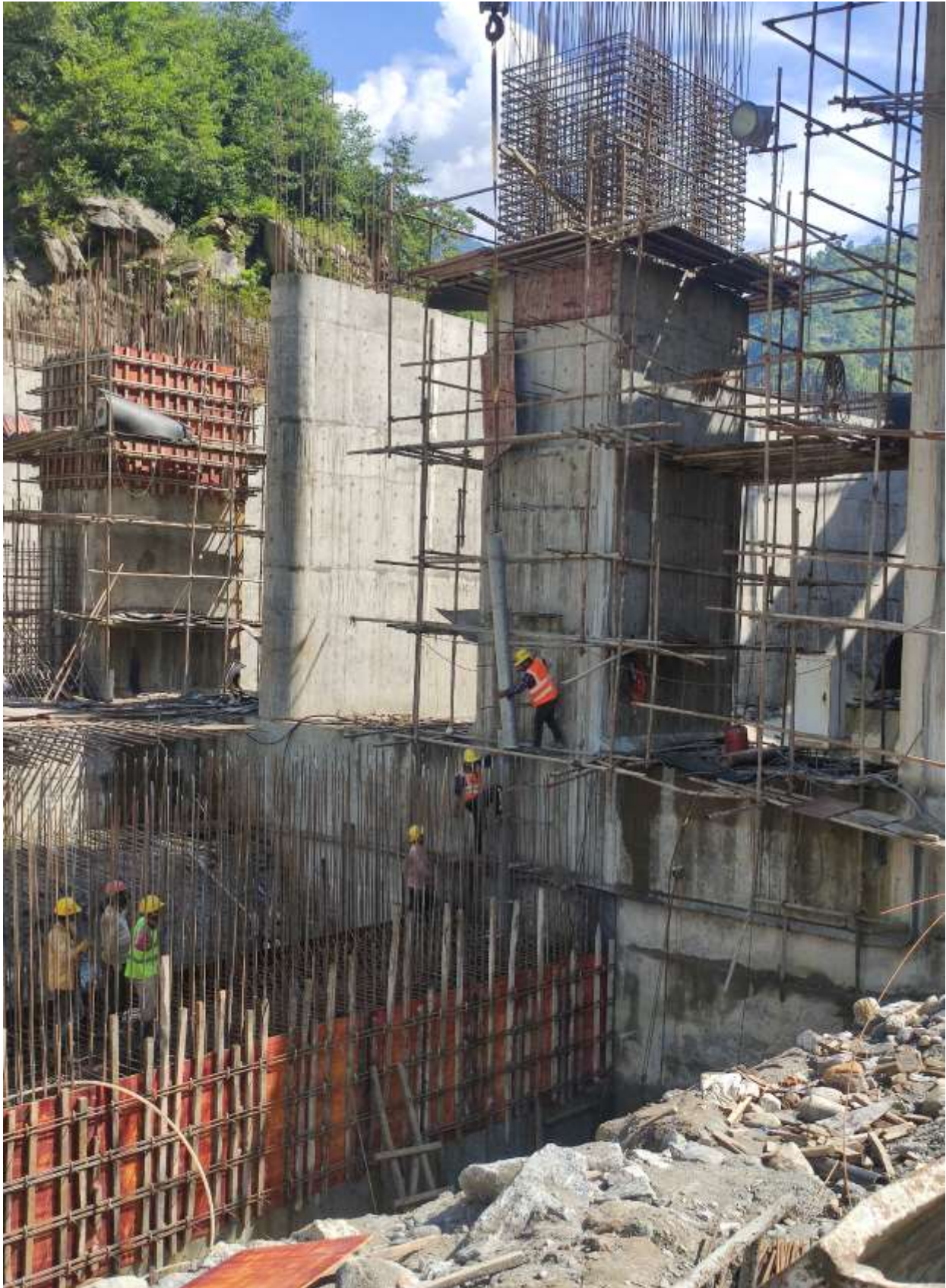
Figure 40: Erection of air vent pipe at gravel flushing Unit 3 (Dia 200 mm)
