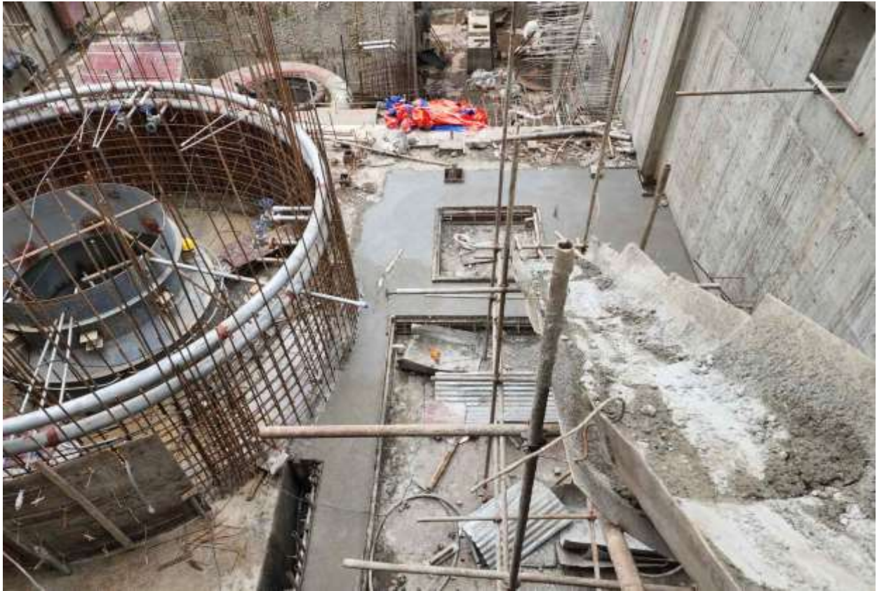
Figure 28: Casting of side slab at unit 01
