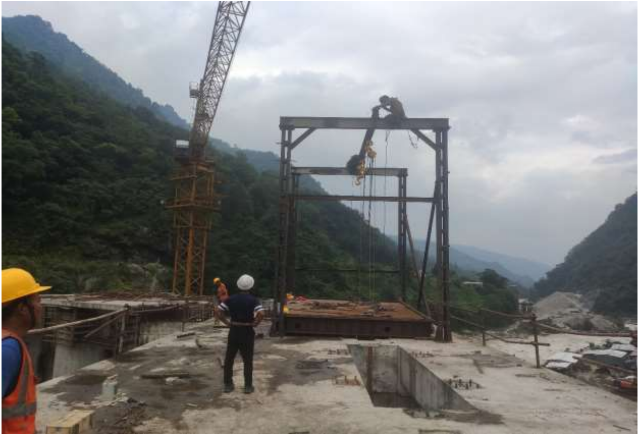
Figure 38: Hoisting mechanism for erection of Intake Gate Unit 2
