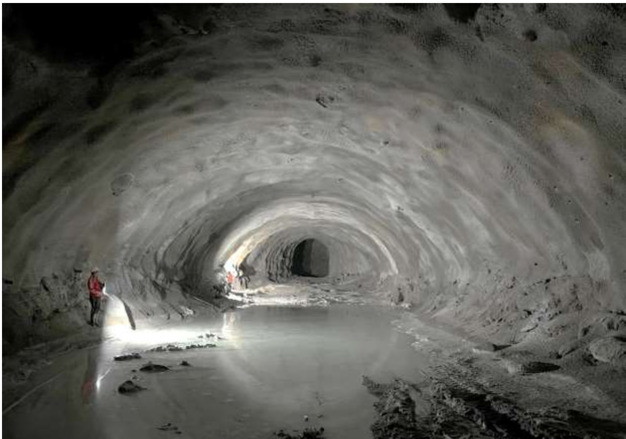
Figure 22: A view of Settling Basin 01 after crown support
