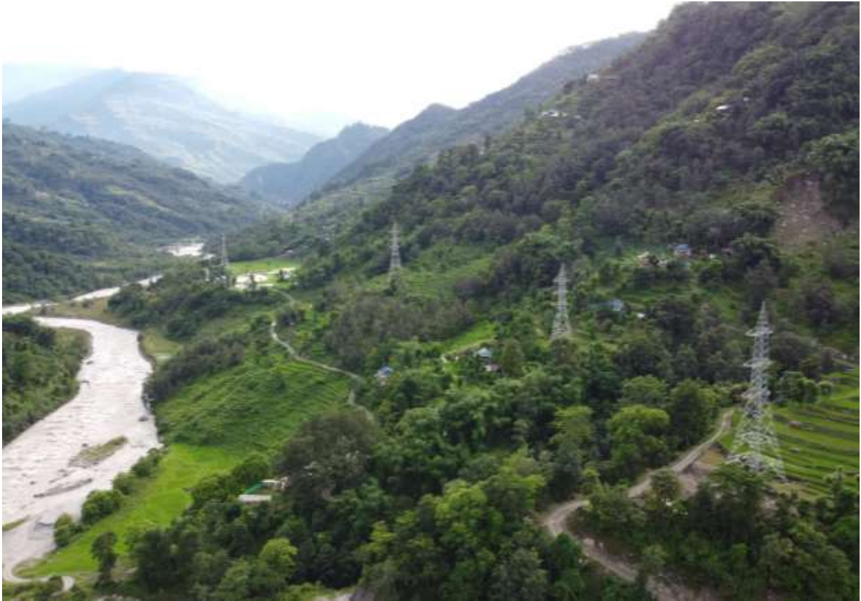
Figure 61: View of erected towers from right bank of Tamor
