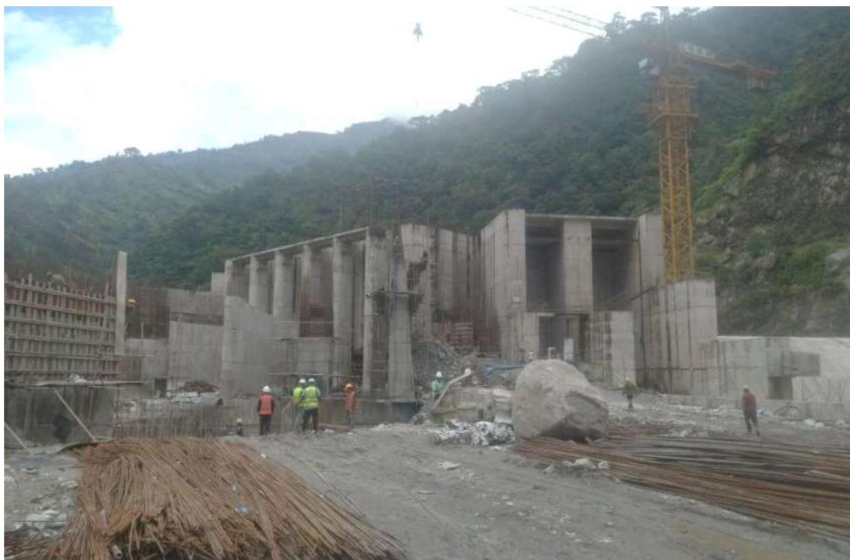
Figure 10: A view of the intake and gravel trap section from the downstream
