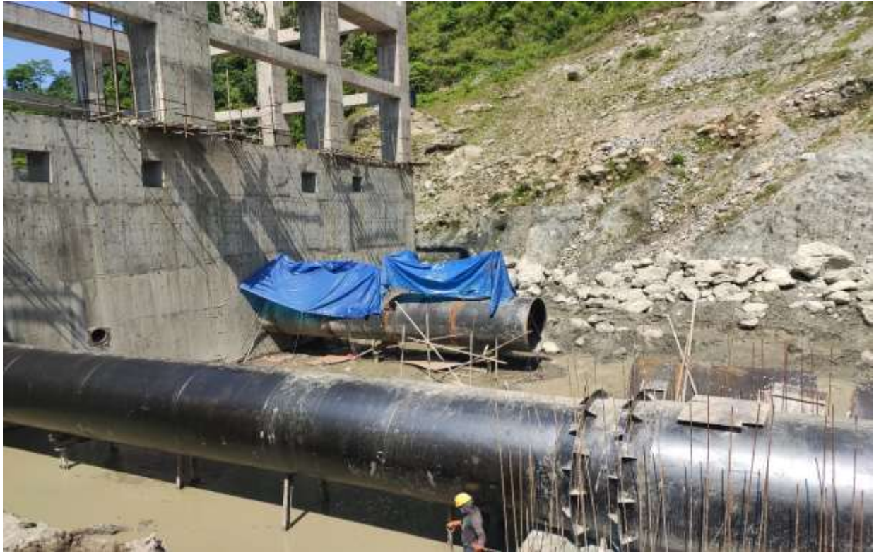
Figure 32: Erection work Unit 2 (Complete) and Unit 1 (Ongoing)
