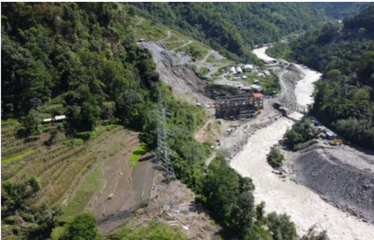
Figure 62: Aerial view of AP 02 near Powerhouse
