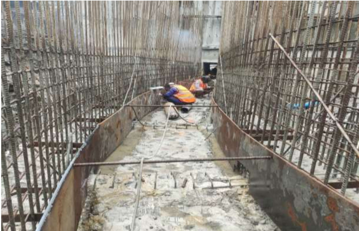
Figure 34: Steel lining works at gravel flushing culvert (thk: 12 mm)
