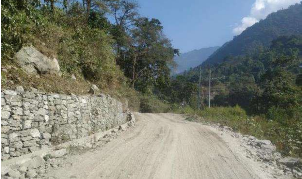
Figure 3: Gabion wall construction at new access road from Mitlung to Thumba
