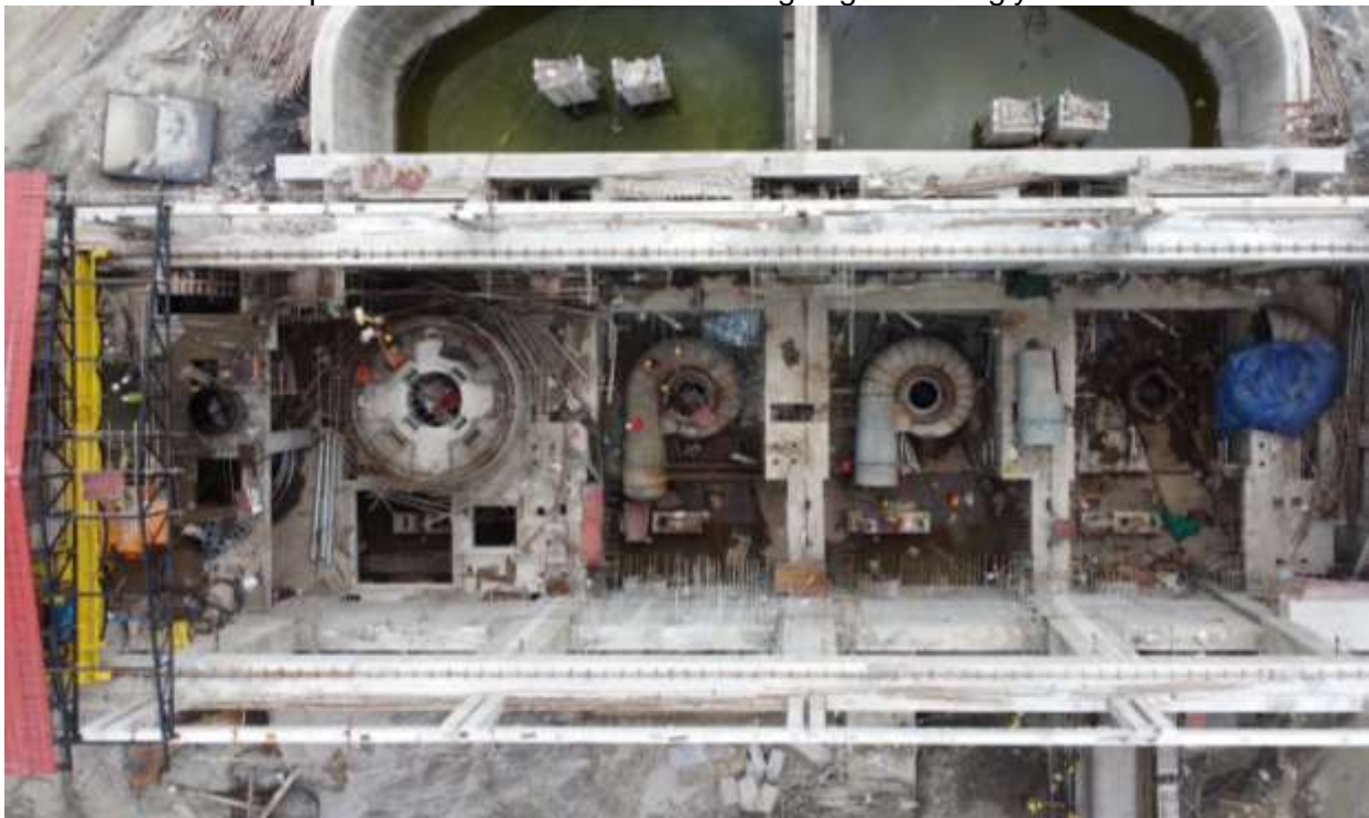
Figure 45: Aerial View showing all four spiral cases and EOT crane
