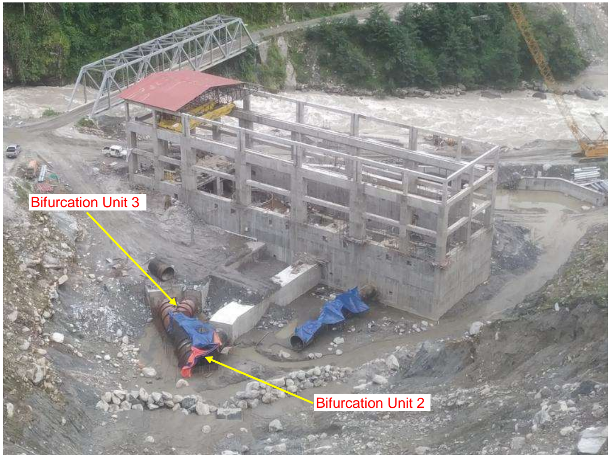
Figure 31: Aerial View of Powehouse Penstock Pipe Erection
