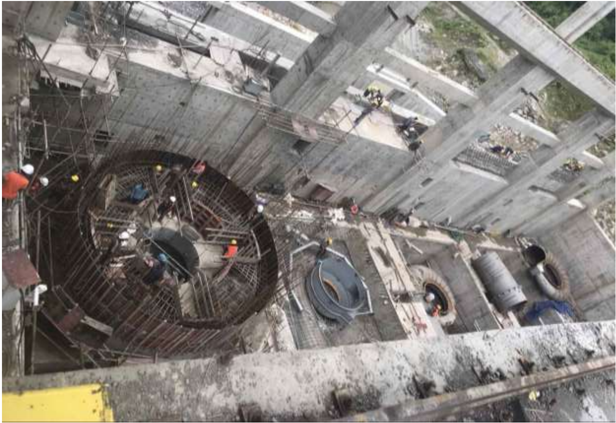
Figure 54: Installation of Pit liner at Unit 2
