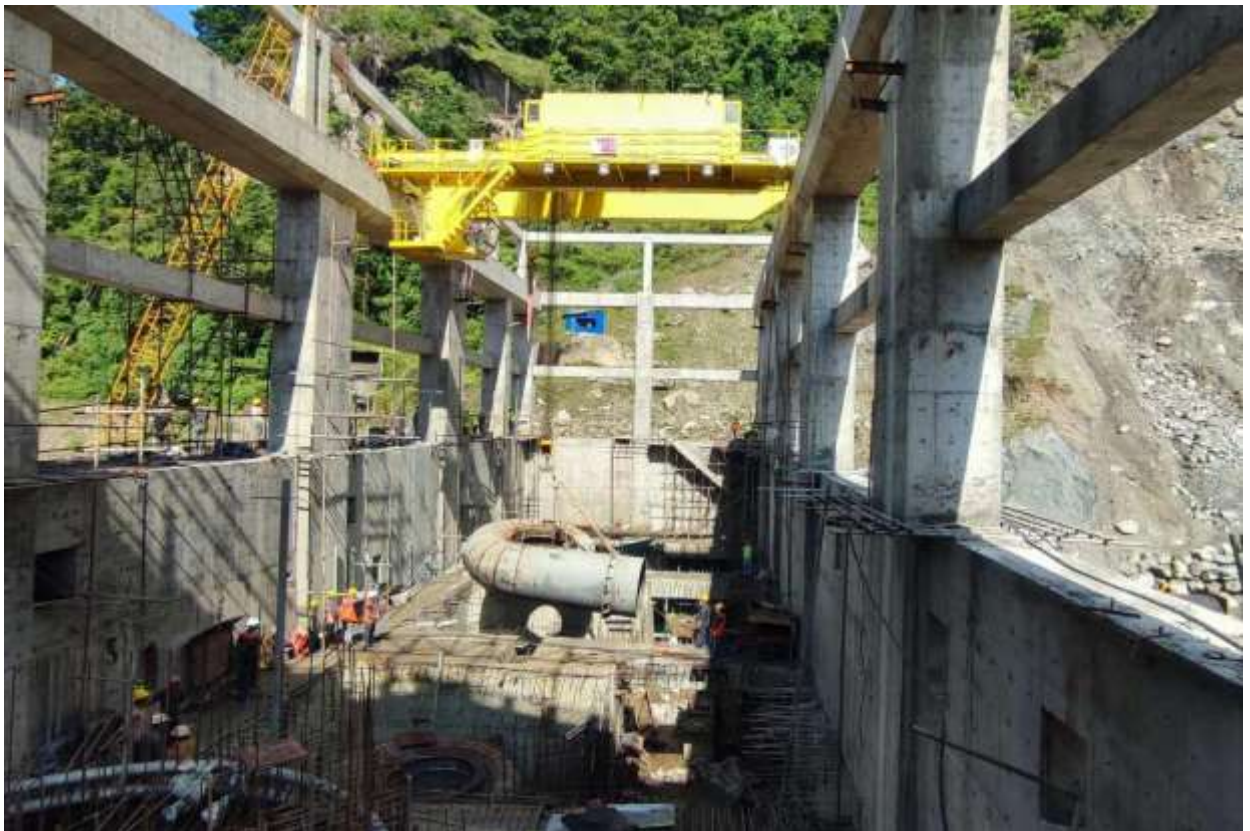
Figure 50: EOT crane being commissioned with the medium load
