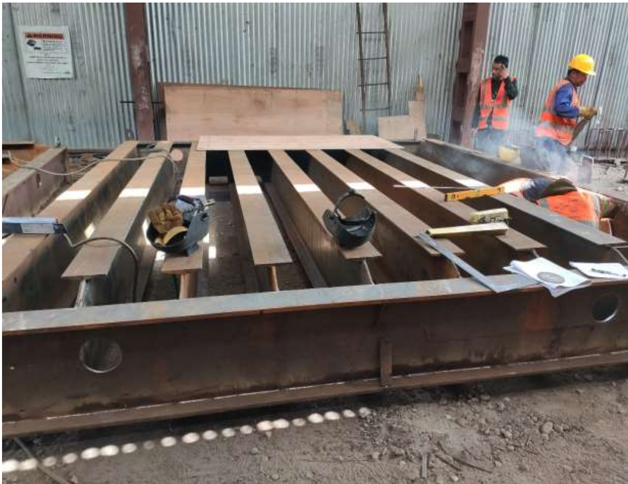
Figure 35: Fabrication of intake gate
