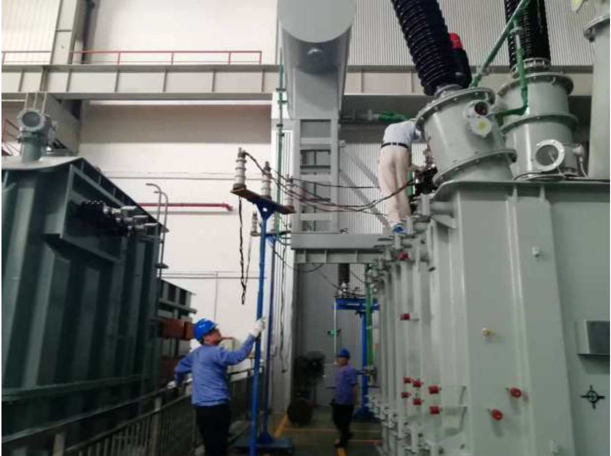
Figure 41: Transformer being factory tested(Contractor's factory in China)
