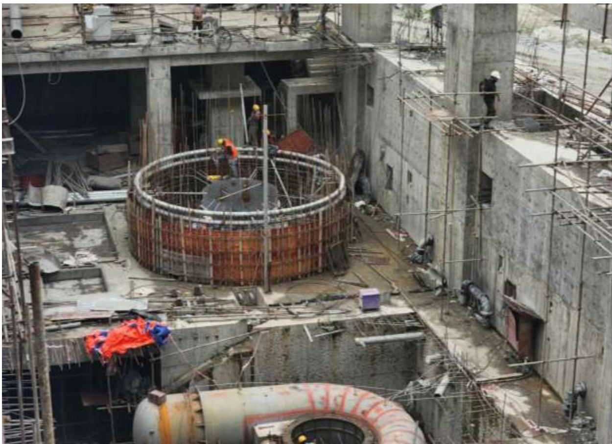
Figure 29: Rebar installation for generator casing at unit 01
