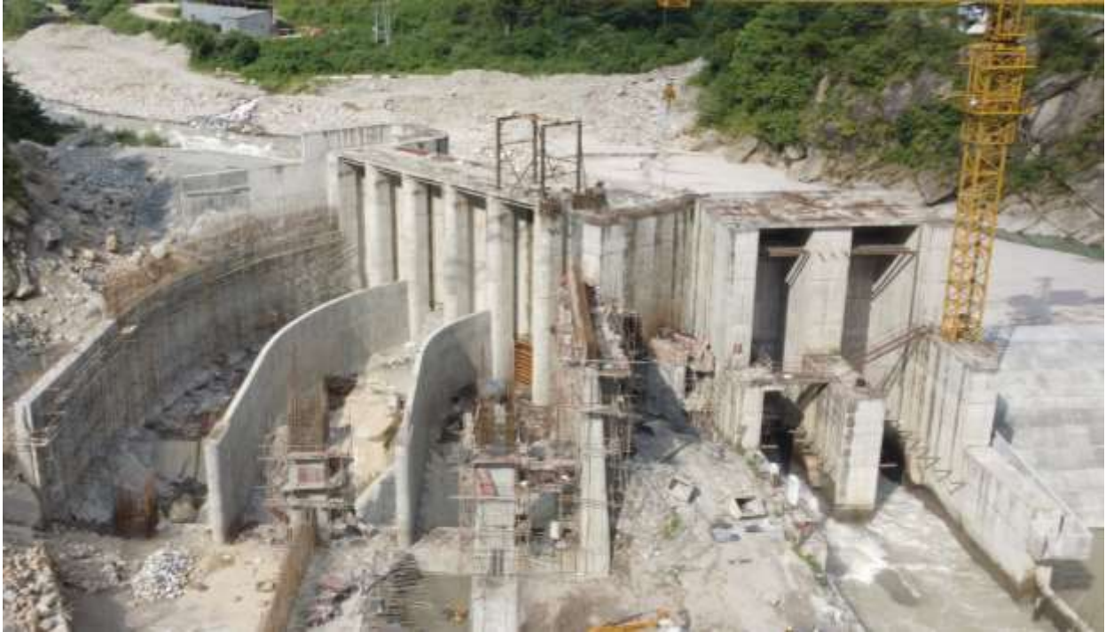
Figure 8: Intake and Undersluice section from downstream
