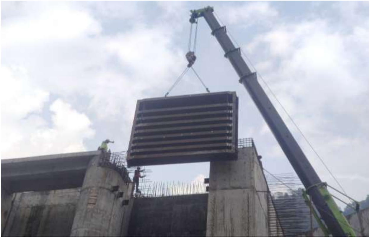
Figure 36: Erection of Intake gate
