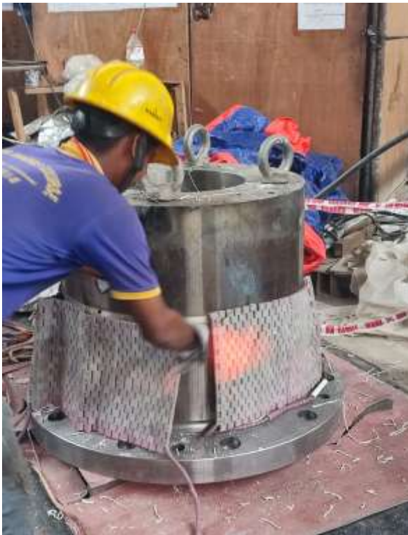
Figure 2-65: Different stages of thrust bearing installation
