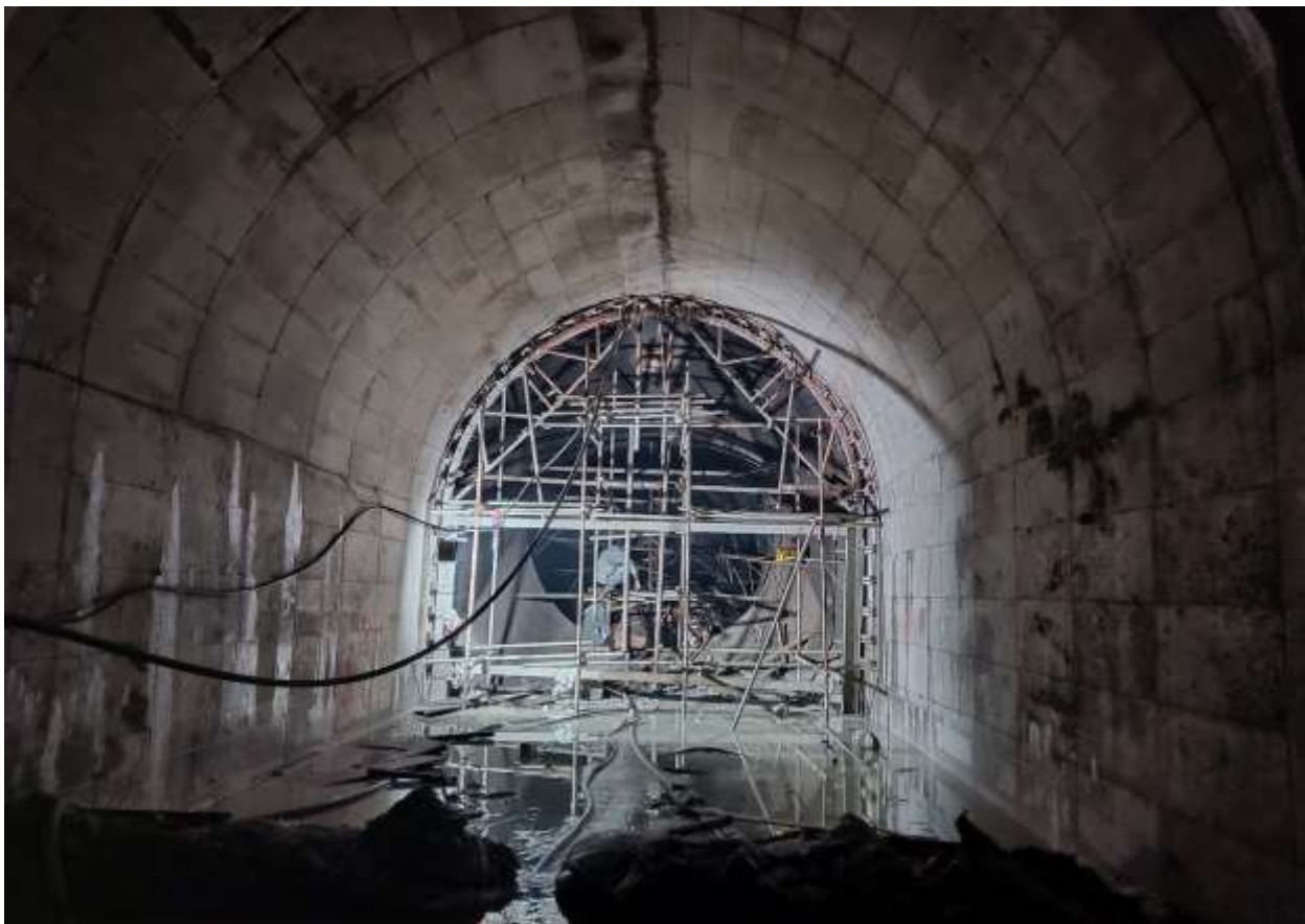
Figure 2-23: A section of HRT with concrete full lining from the outlet region
