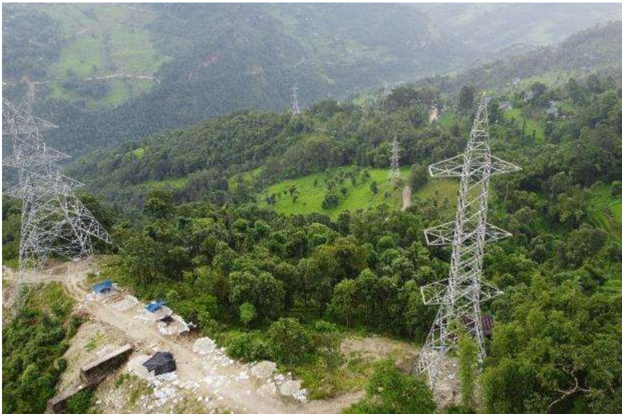
Figure 2-88: Erected last tower at AP24 and tower of NEA (left)
