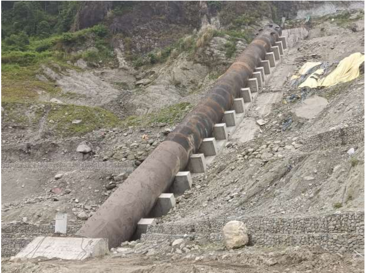
Figure 2-41: Erection of penstock pipes
