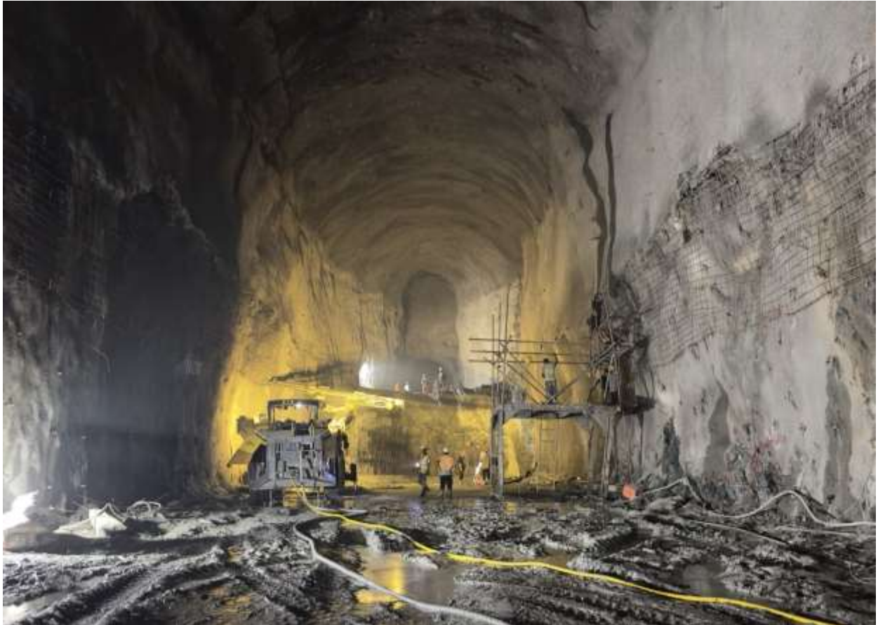
Figure 2-18: Final stage of rock bolt installation works using Boomer at SB 03
