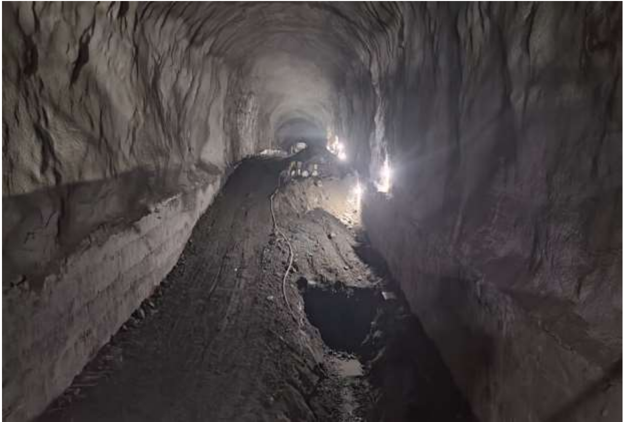
Figure 2-14: A view of SB 01 with completed wall lining and shotcrete on the walls
