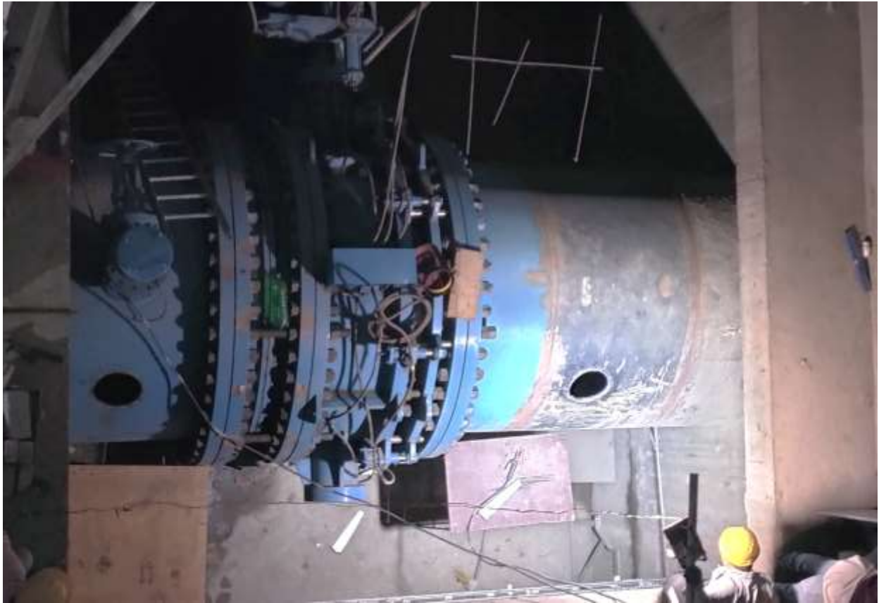
Figure 2-74: Unit 03 preparation for bypass valve erection
