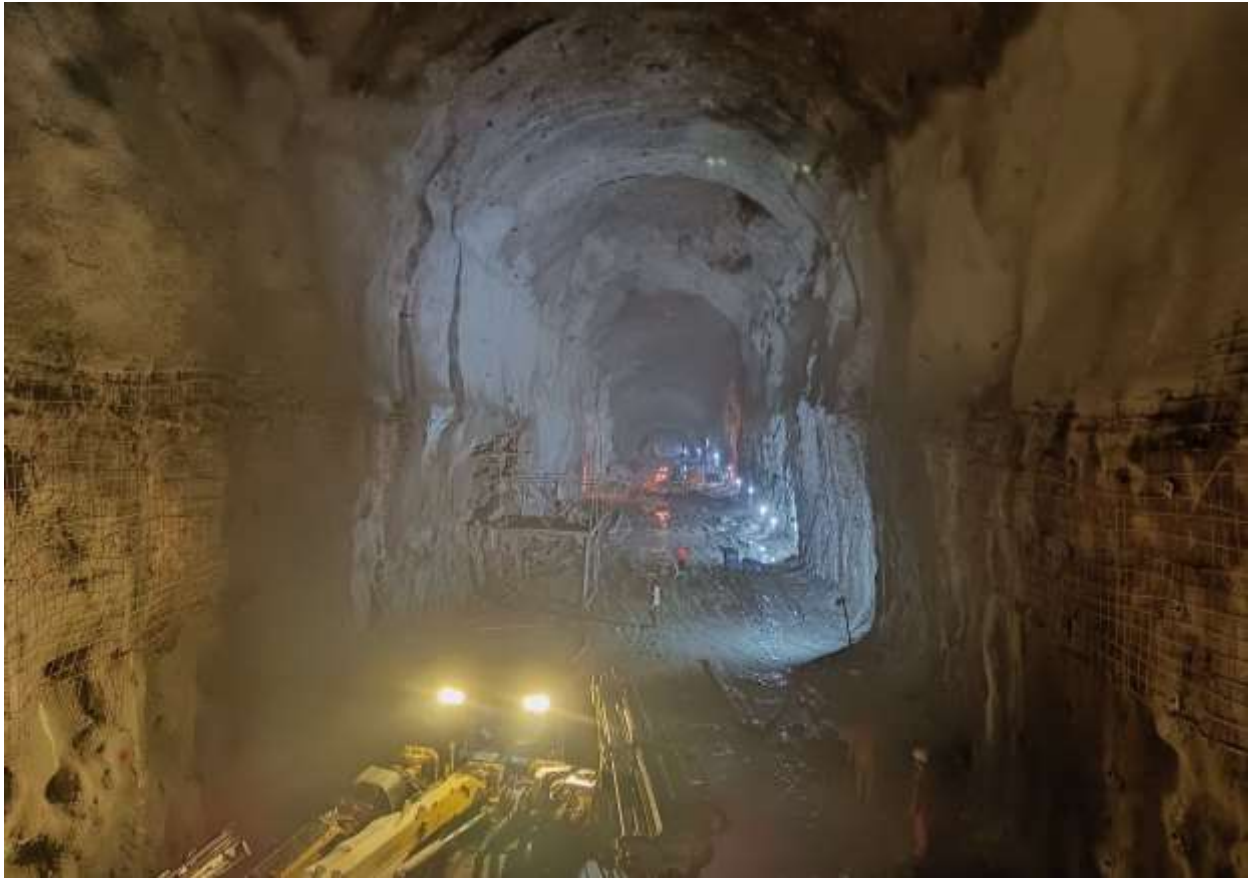
Figure 2-17: A view of SB 03 during installation of final lining wiremesh shotcrete
