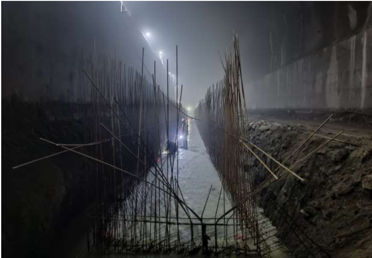
Figure 2-15: A view of concreting at the left hopper of Settling Basin 01
