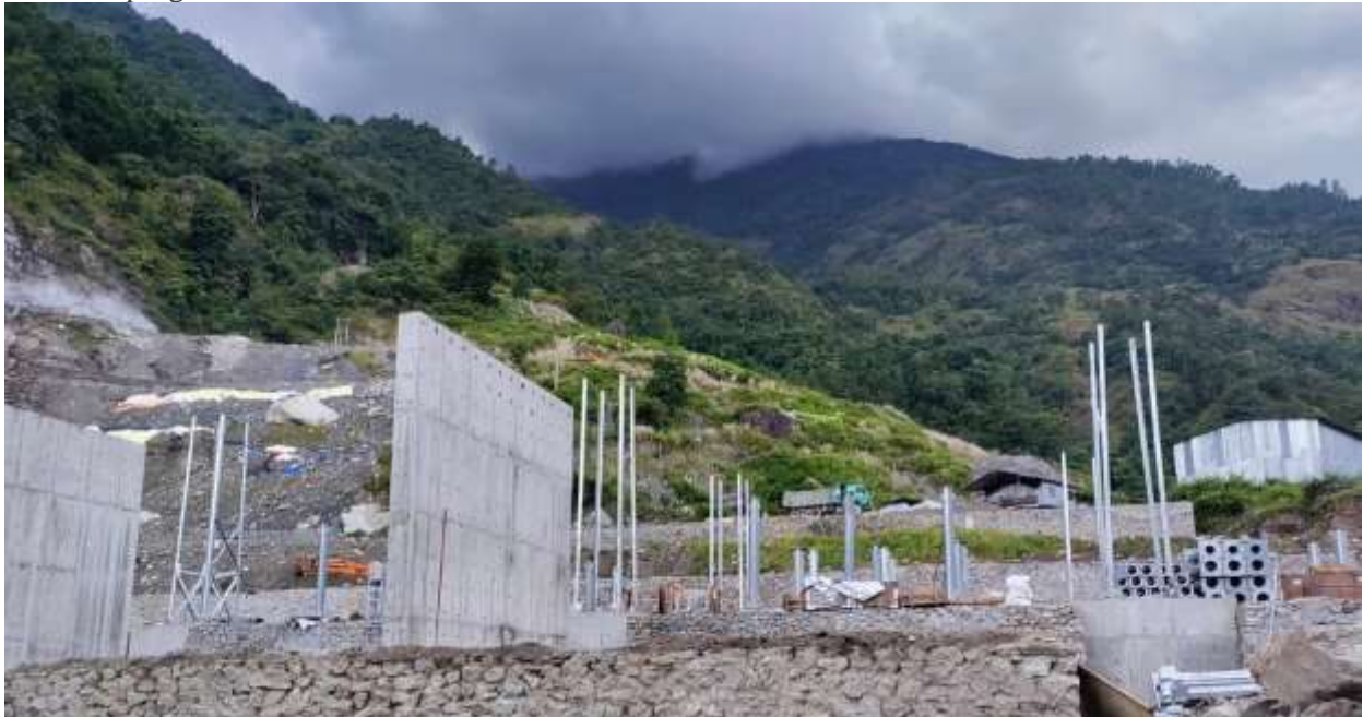
Figure 2-80: Erection of gantry tower and other supporting posts
