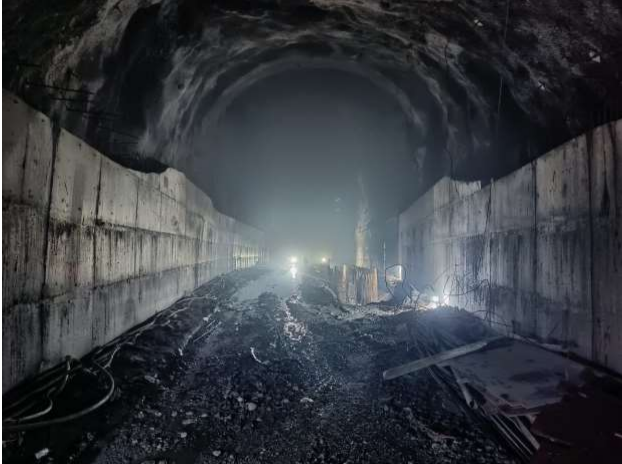
Figure 2-16: Concreting works at the right hopper of settling basin bay 02
