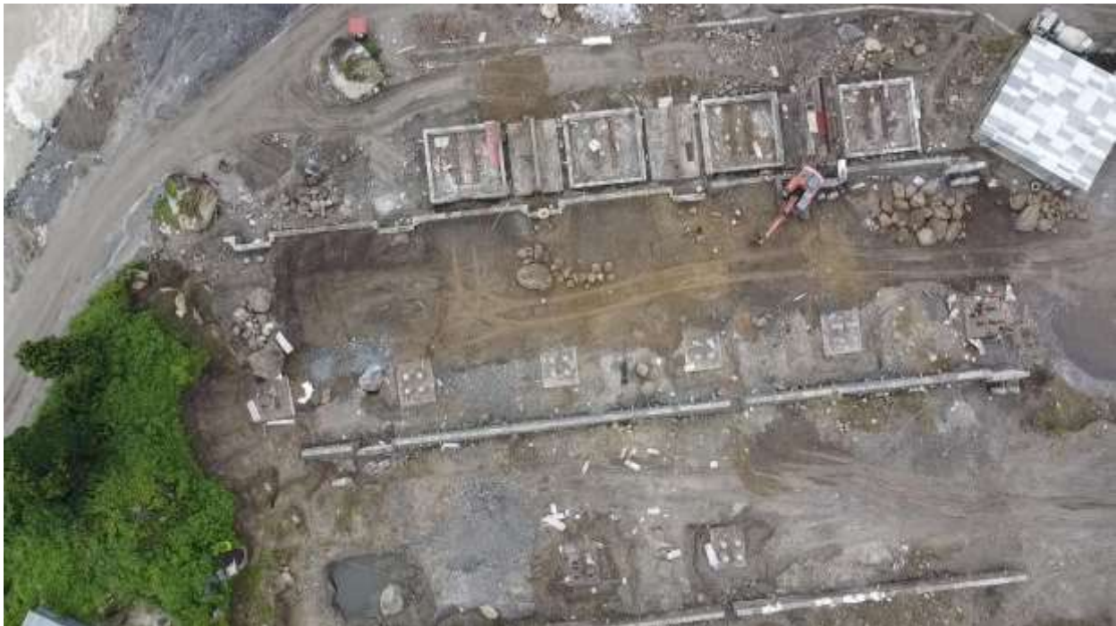
Figure 2-32: A view of the construction works of transformer foundation at switchyard region
