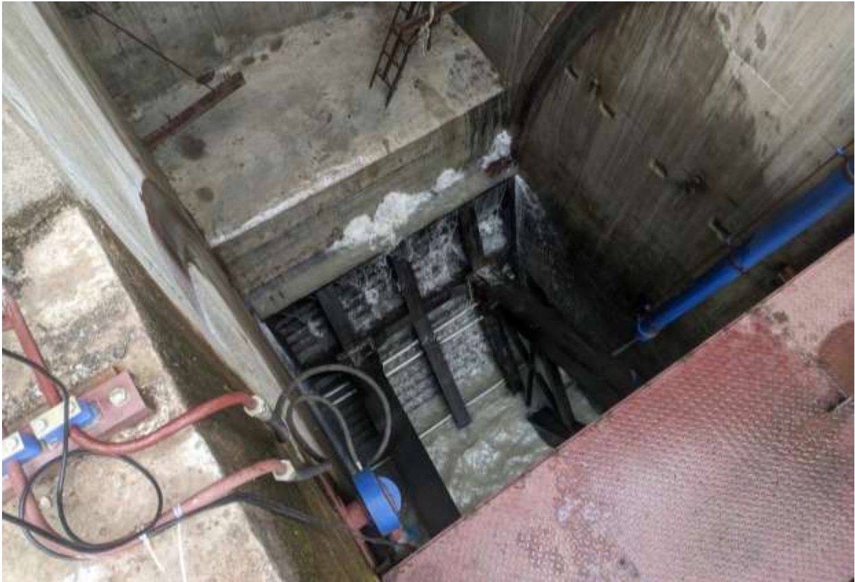
Figure 2-46: Erection of radial gate at undersluice
