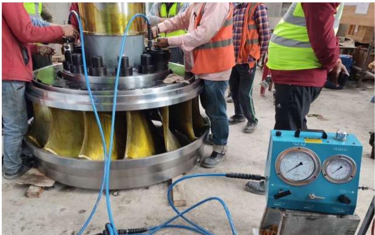
Figure 2-68: Assembly of runner with main shaft
