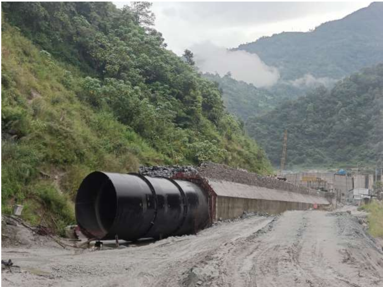
Figure 2-40: Installation of head race bend at the approach pipe section
