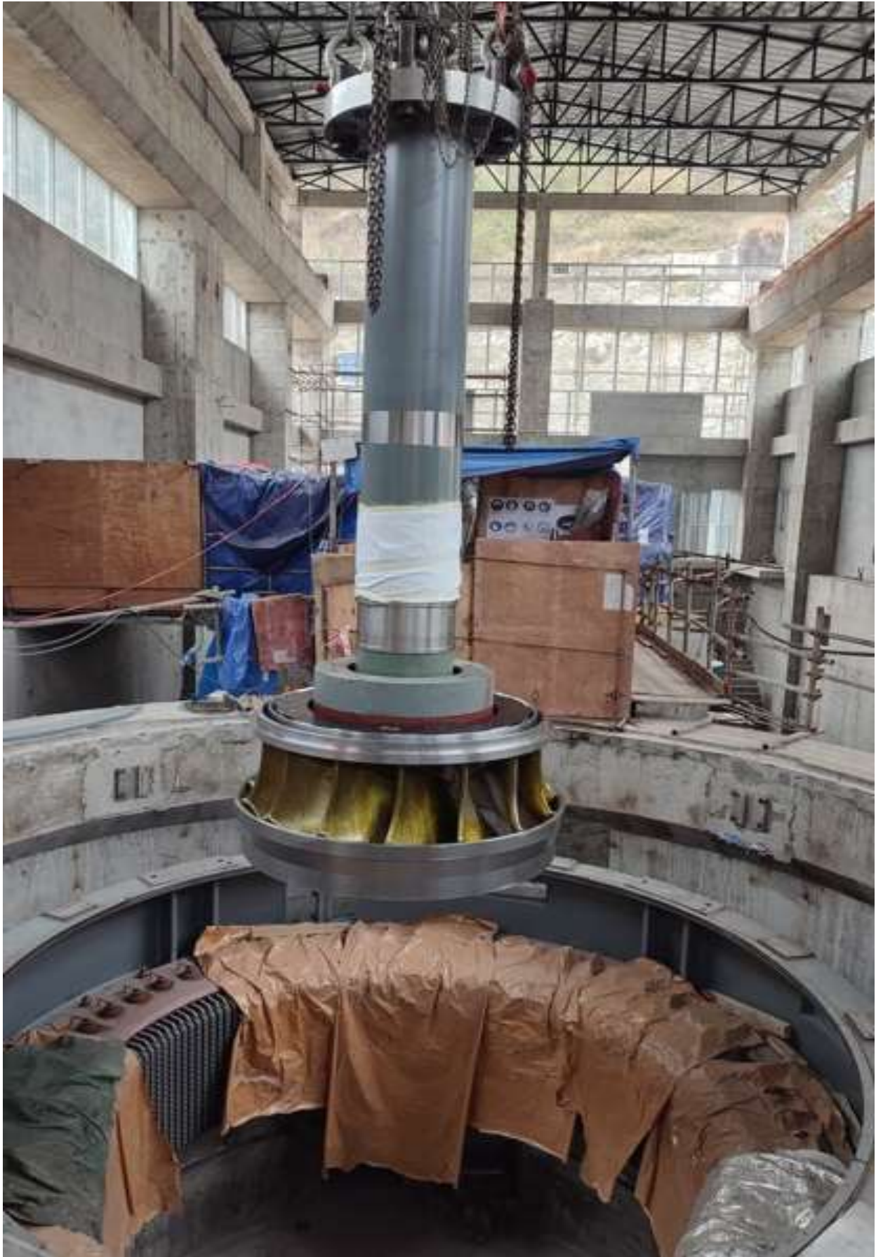
Figure 2-62: Final assembly and lowering of runner with main shaft in unit 2
