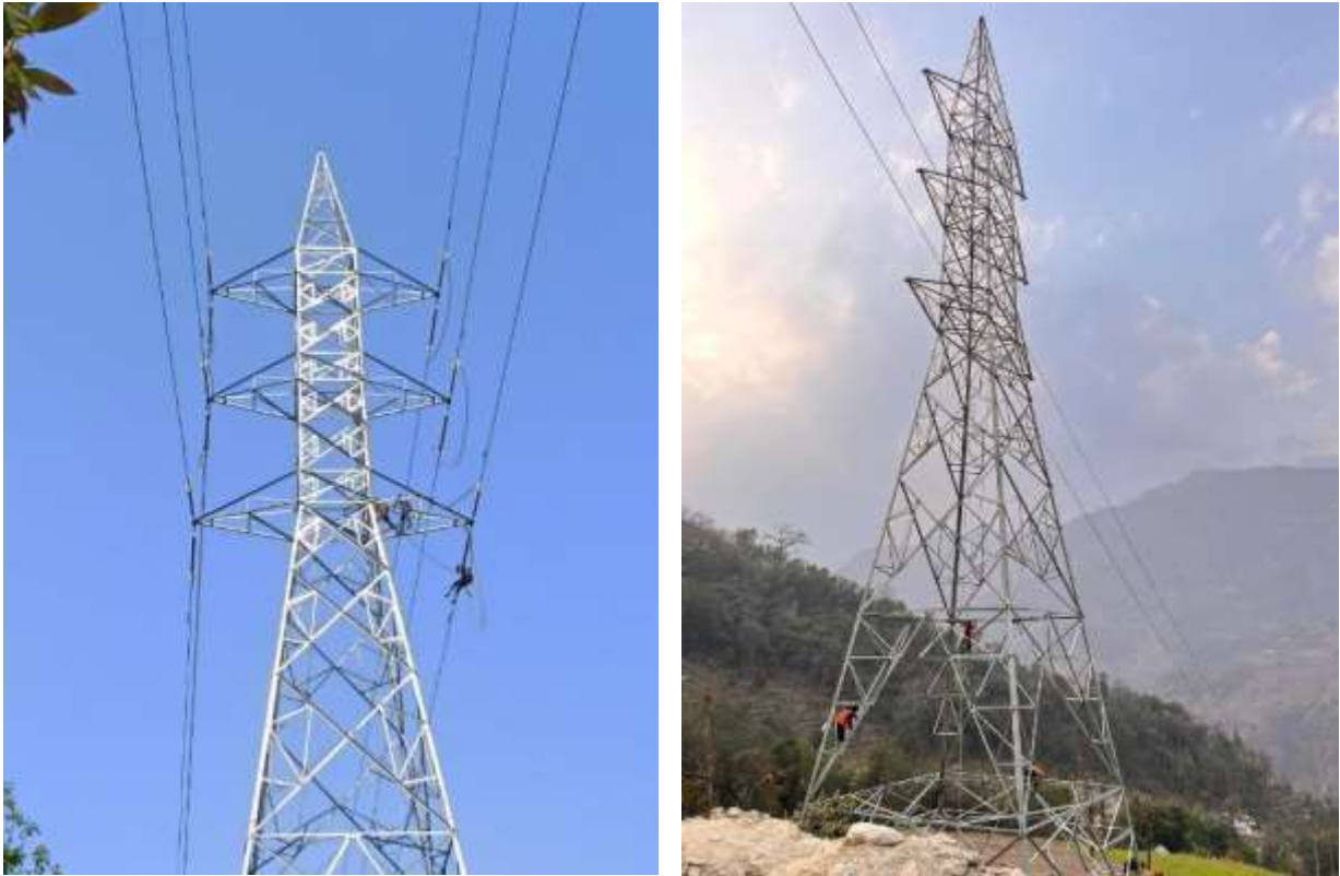
Figure 2-87: Conductor stringing works at various angle points
