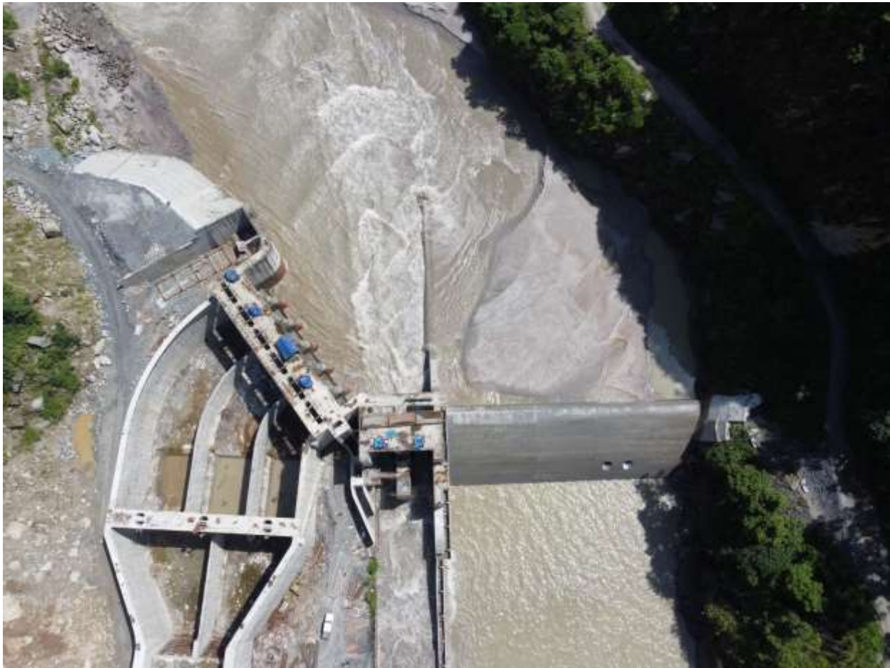
Figure 2-10: From left, Intake canal, Intake, Undersluice and weir
