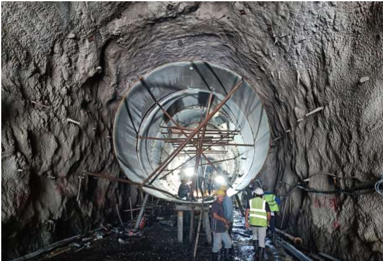
Figure 2-44: Installation of penstock pipes inside HRT from outlet region
