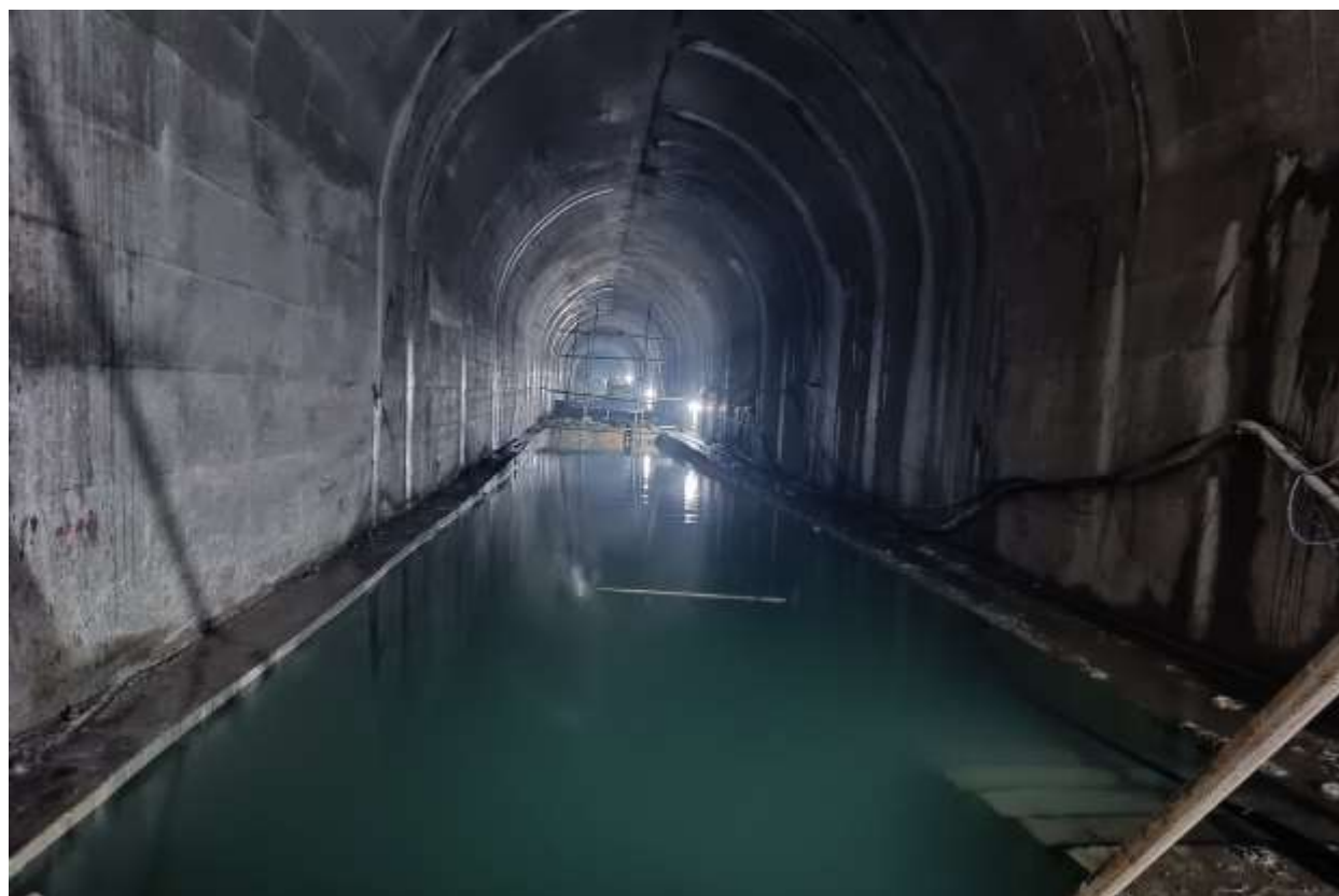
Figure 2-24: A completed section of concrete lining works at rock trap
