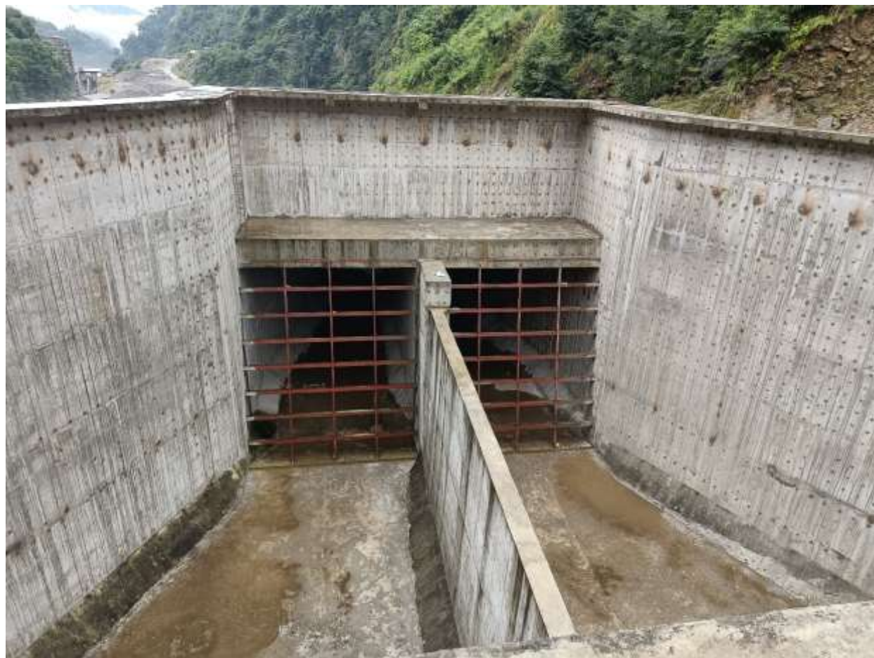
Figure 2-11: A view of conveyance tank
