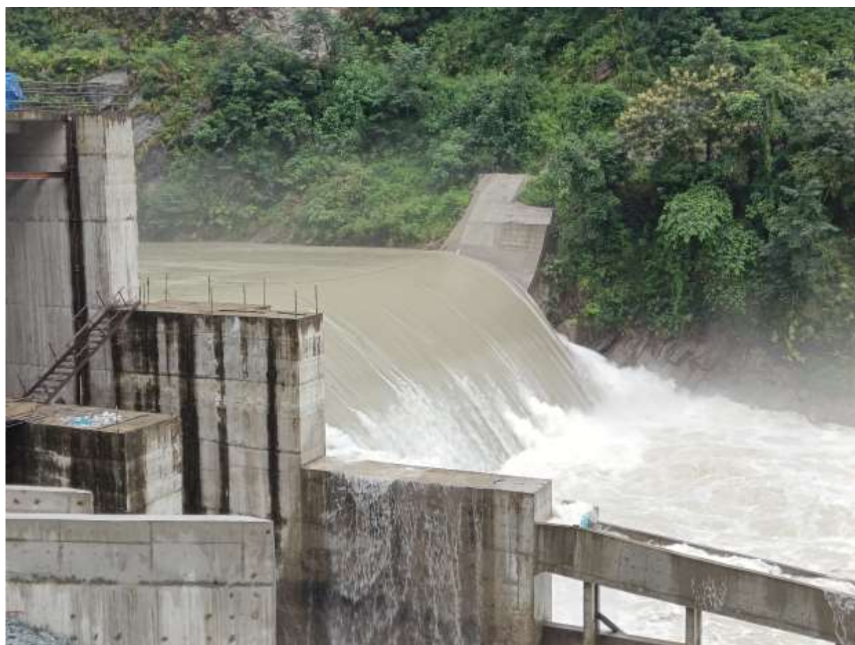
Figure 2-6: A view of weir during monsoon water flow over the ogee crest
