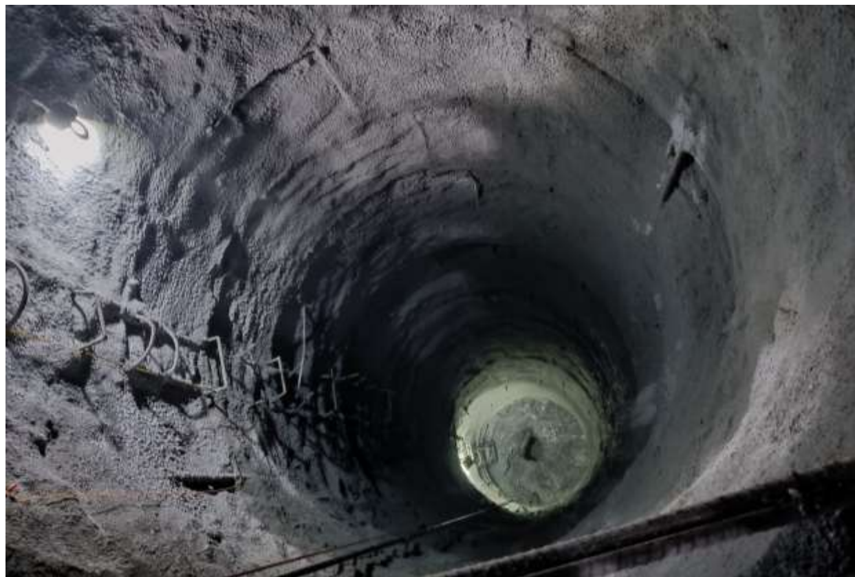
Figure 2-27: Breakthrough of flushing tunnel 04
