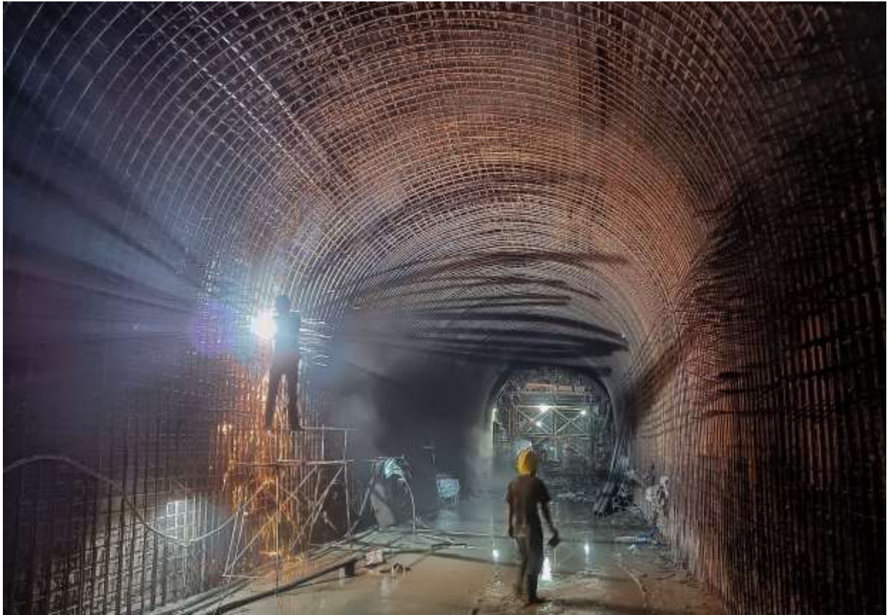
Figure 2-22: Rebar installation at the HRT region
