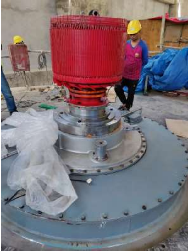
Figure 2-64: Pressure test of upper bracket bearings oil cooler
