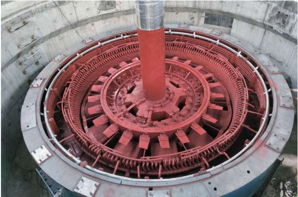
Figure 2-58: Rotor and stator coupling in unit 01
