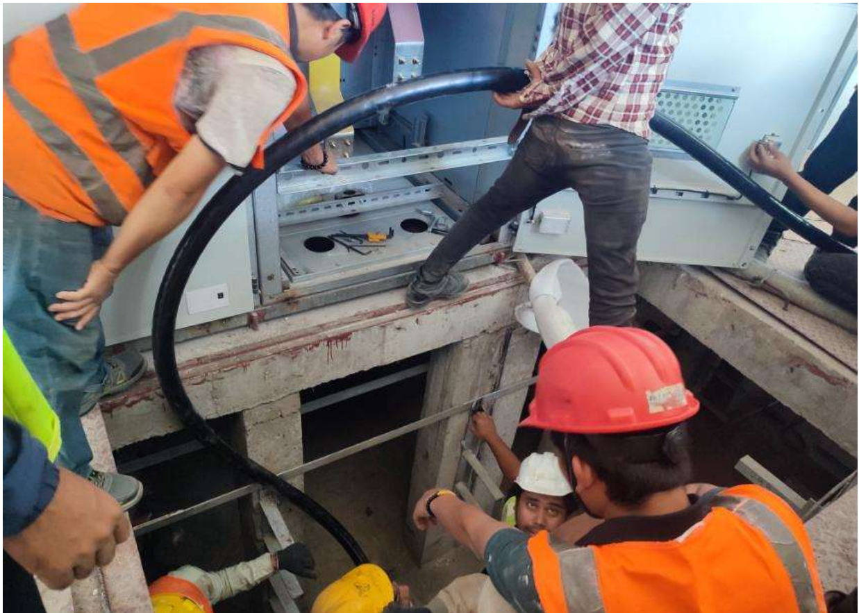
Figure 2-77: Laying of power cables in 11KV switch gear room
