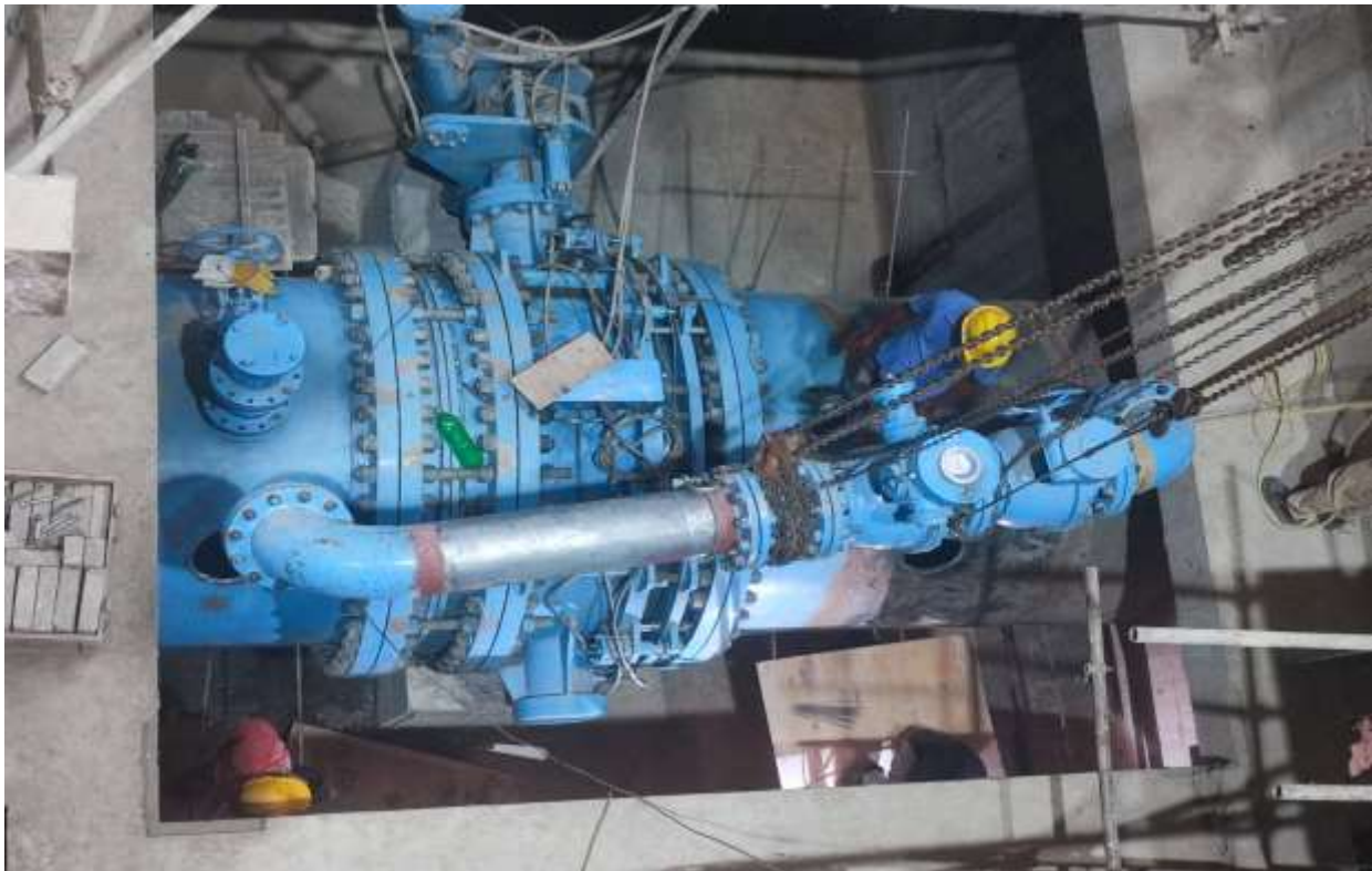
Figure 2-73: Unit 02 bypass valve assembly and erection
