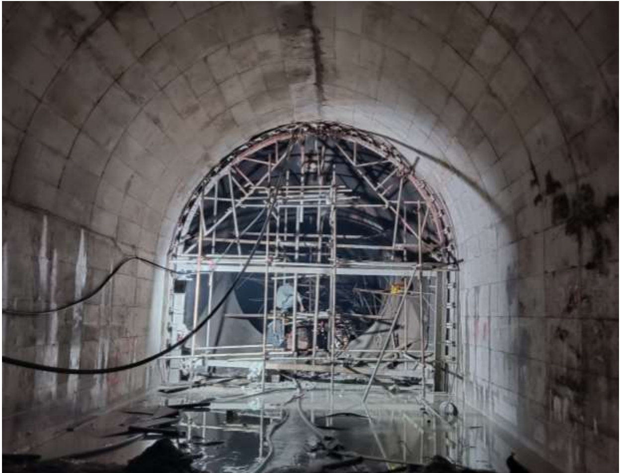
Figure 2-45: Installation of transition pipe at the plug block 01 region
