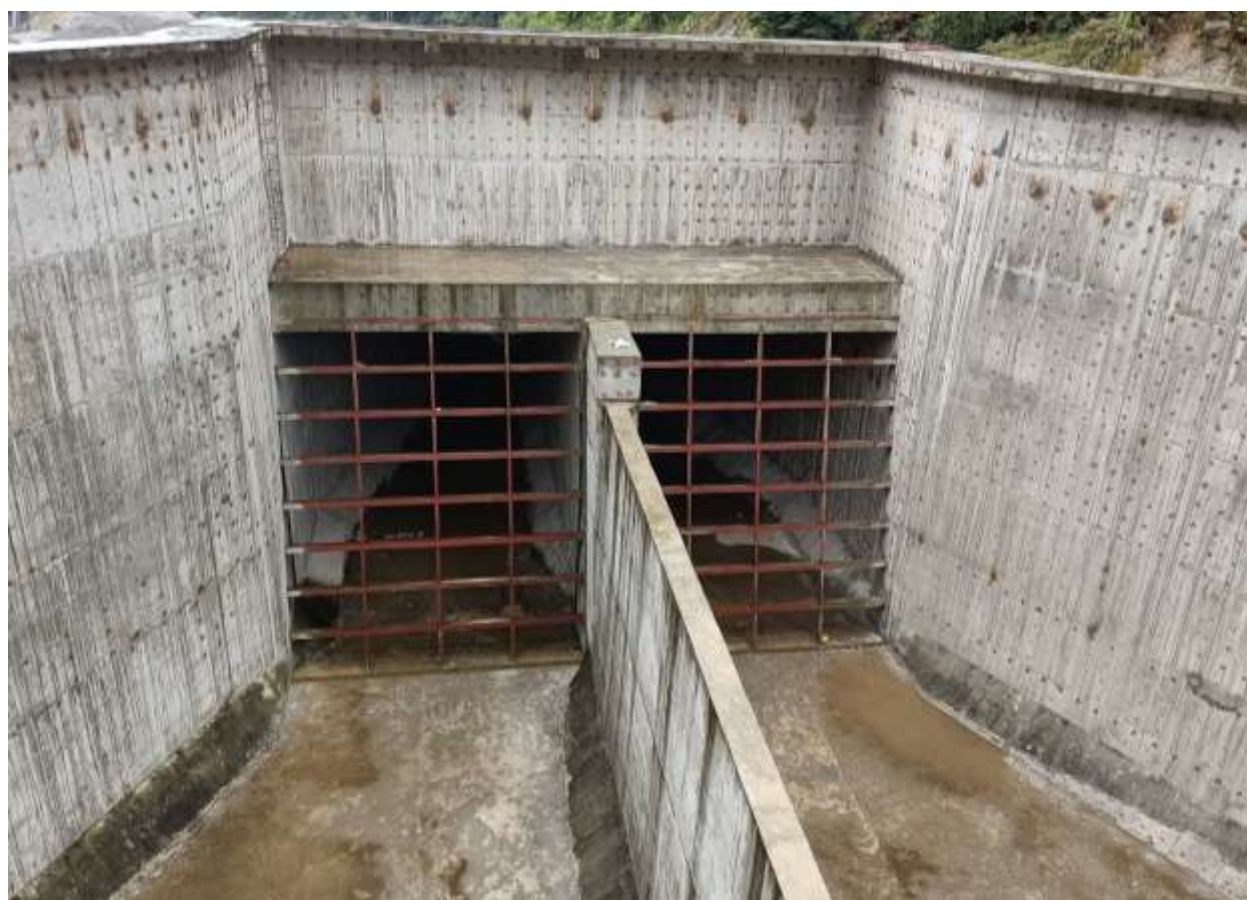
Figure 2-39: Installation of trash rack at the conveyance tank region
