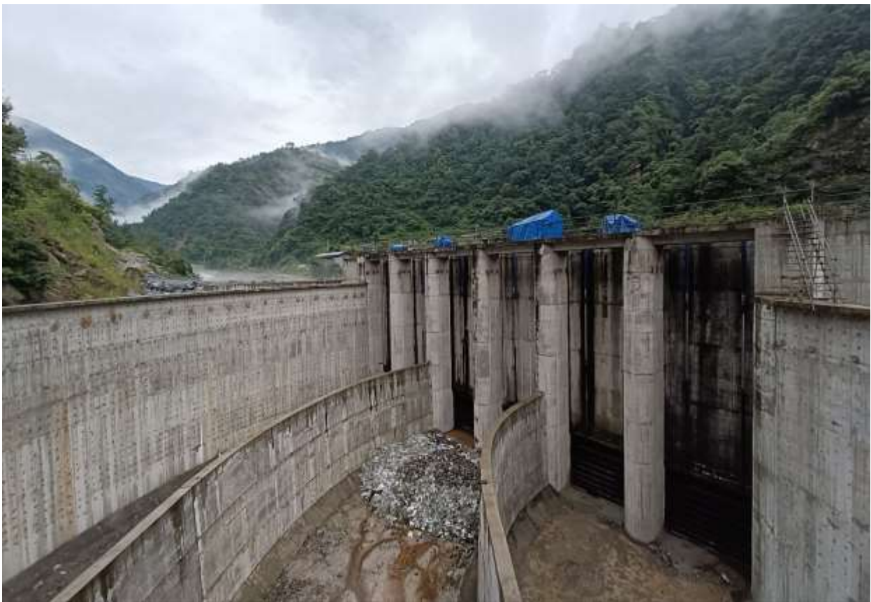
Figure 2-47: Intake gates installation completed
