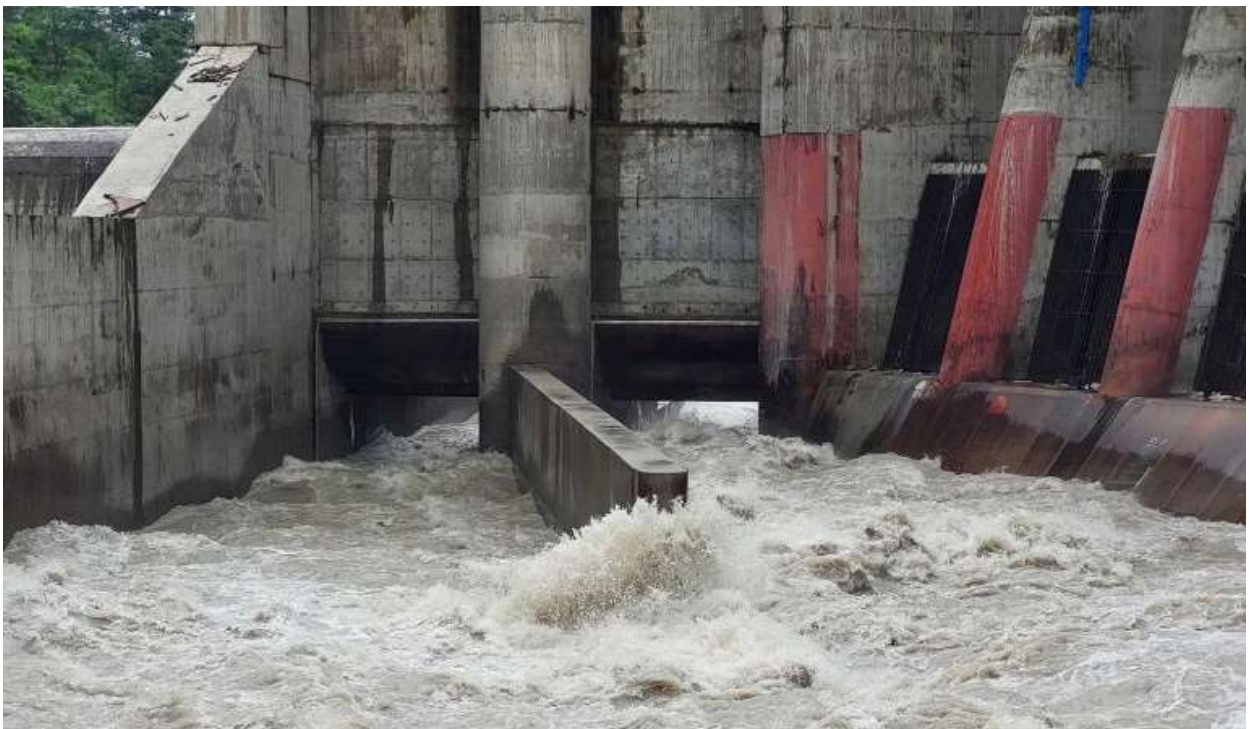
Figure 2-8: A view of undersluice during gate opening condition
