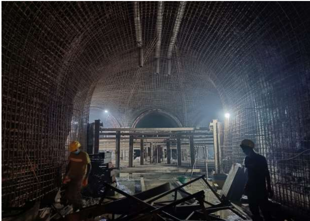
Figure 2-19: Preparation for full lining at the connecting tunnel junction
