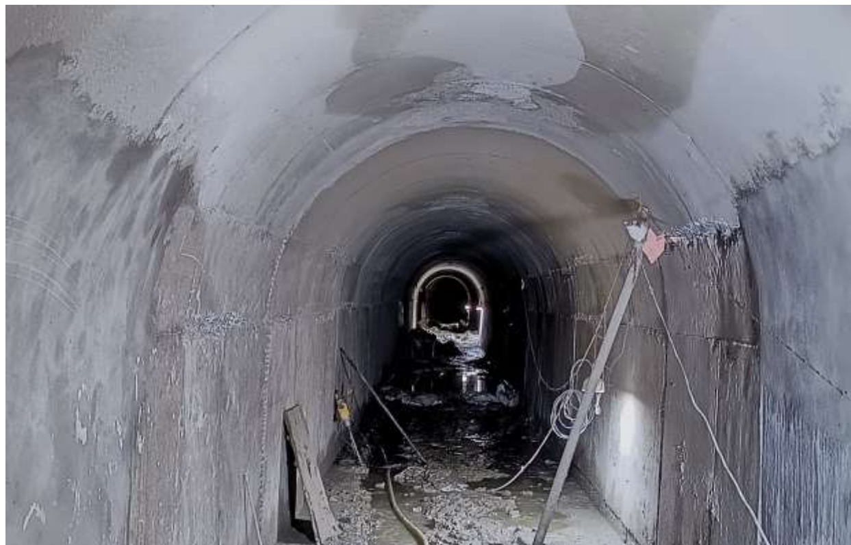
Figure 2-26: A view of full concrete lining at the flushing tunnel
