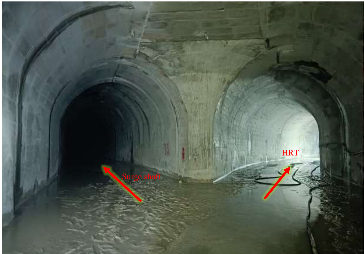
Figure 2-30: Full concrete lining at the junction of connecting tunnel and HRT
