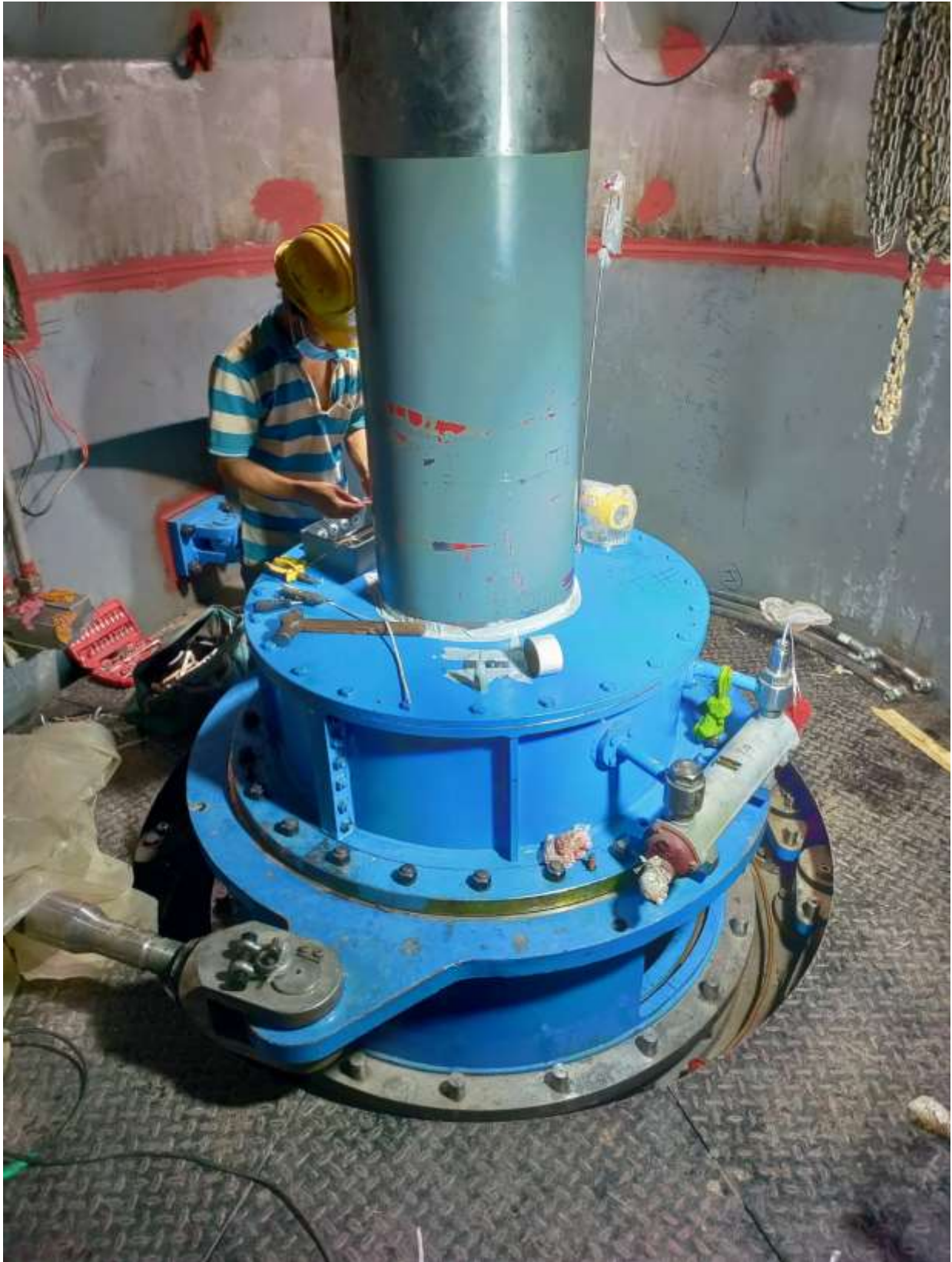
Figure 2-66: Final installation of turbine guide bearing and water regulating mechanism
