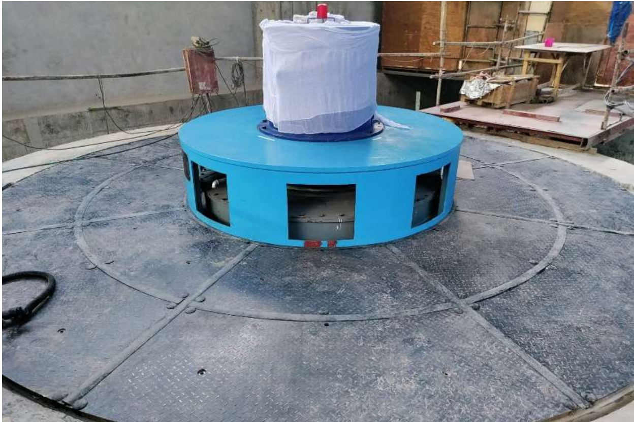
Figure 54: Final installation of excitation system
