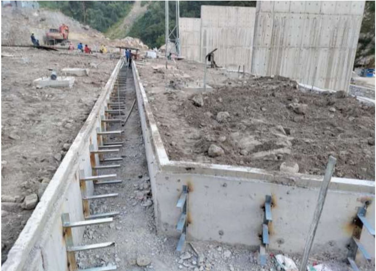
Figure 2-82: Cable tray support inside cable trench of switchyard
