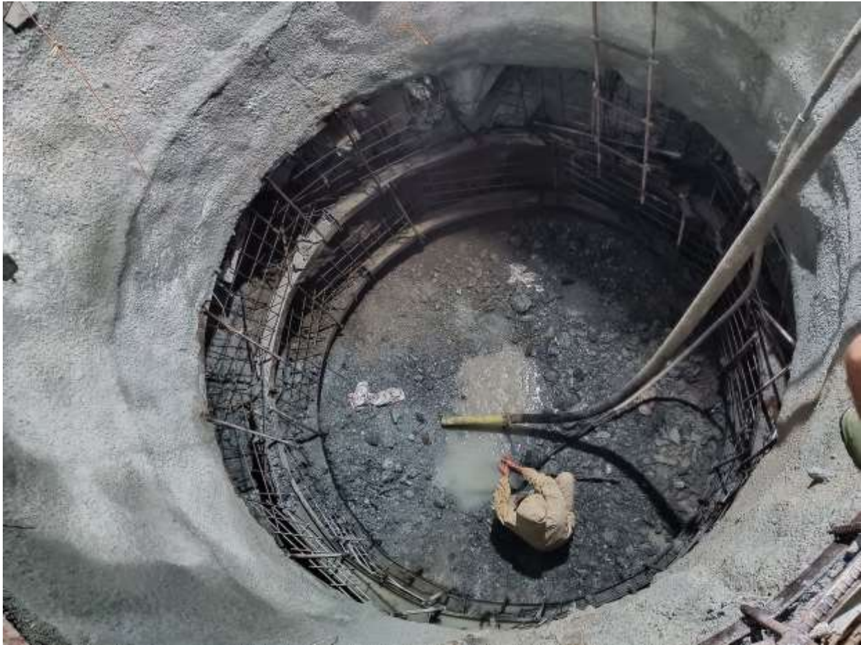
Figure 2-28: Excavation of flushing tunnel 03 in progress
