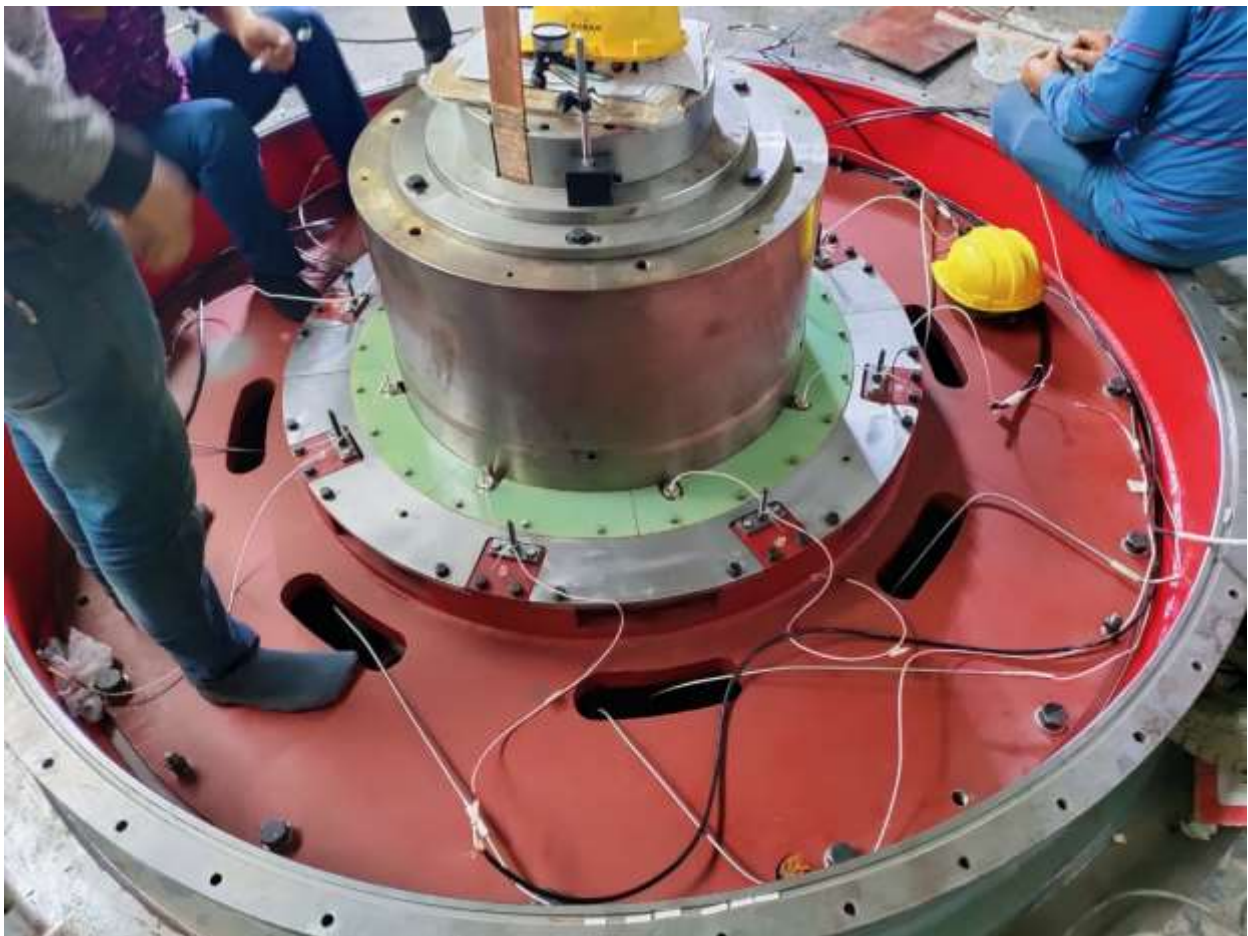
Figure 2-57: Installation of temperature and resistance measuring sensors at thrust bearing
