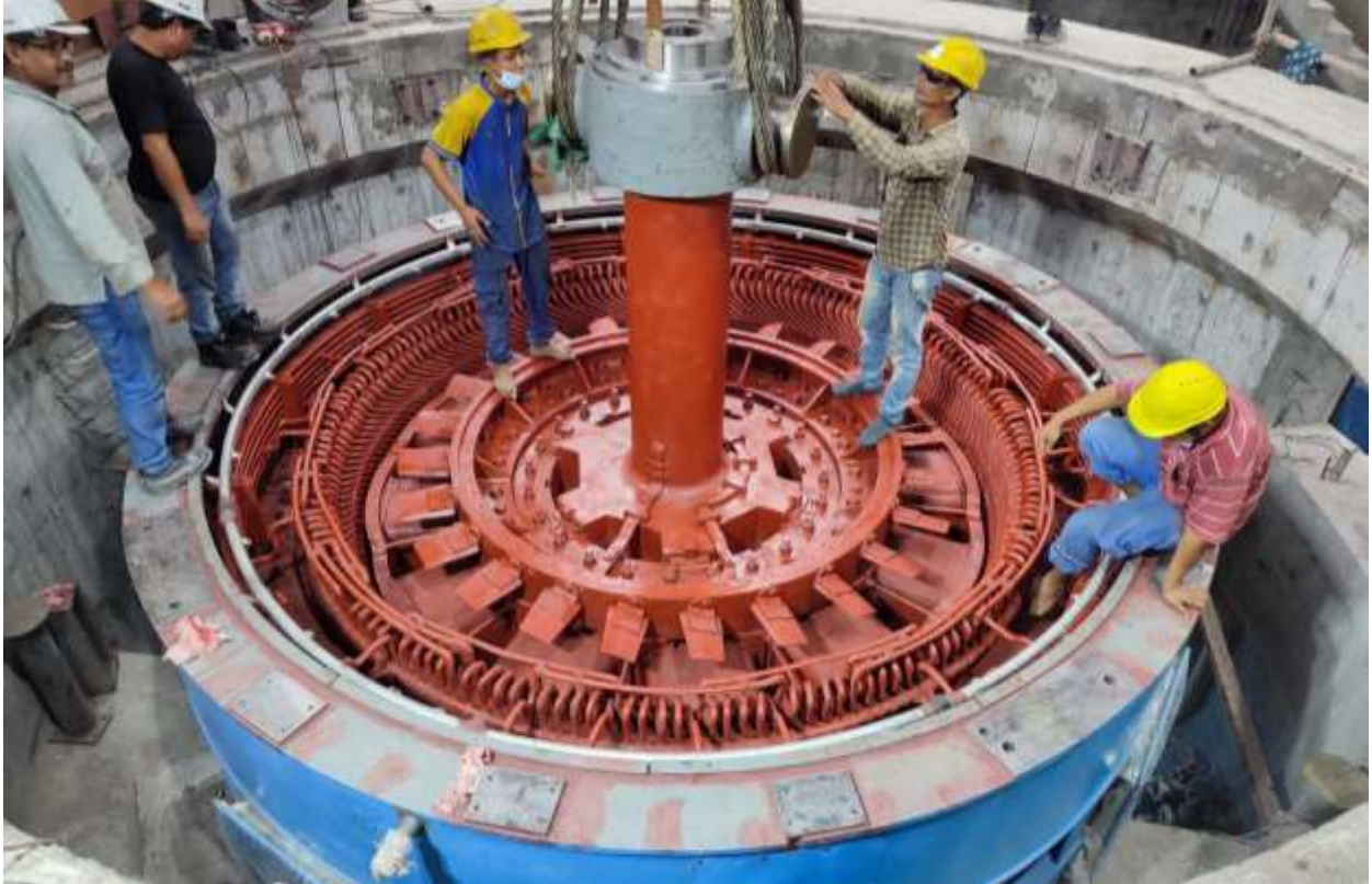
Figure 2-69: Rotor lowering of unit 04
