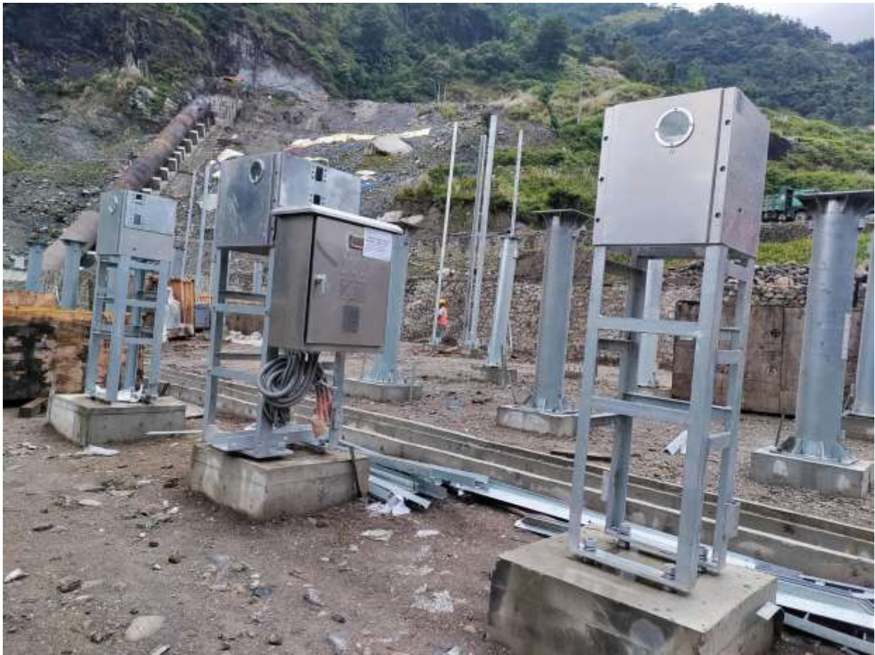
Figure 2-81: Erection of circuit breaker posts
