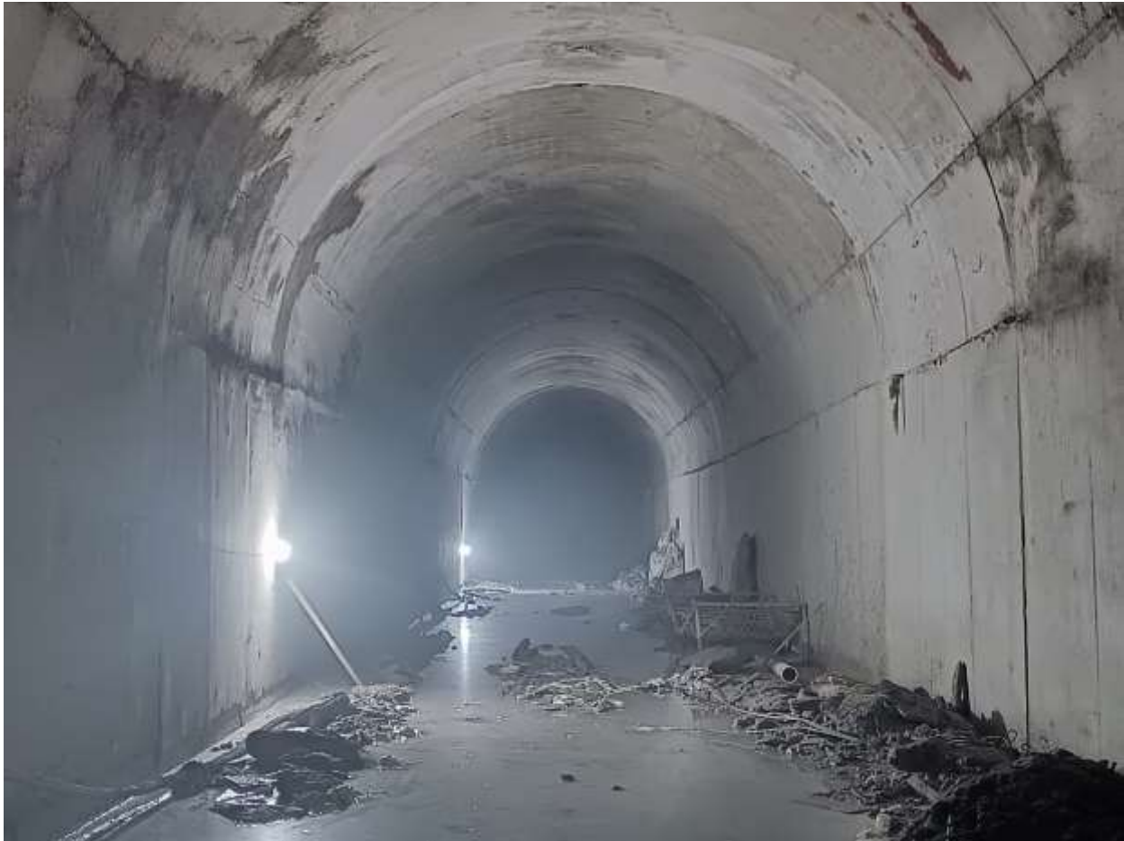
Figure 2-21: A section of HRT with concrete full lining from the adit region
