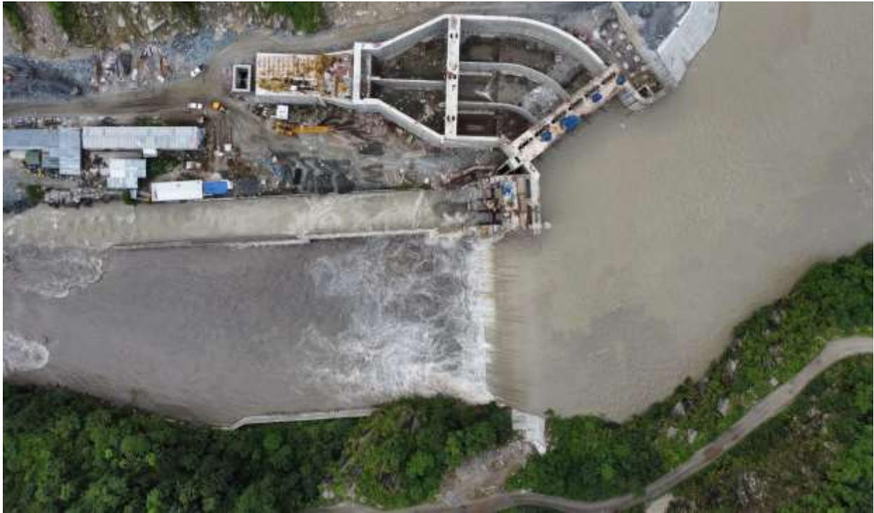
Figure 2-9: Flowing of water over the weir during water filling test
