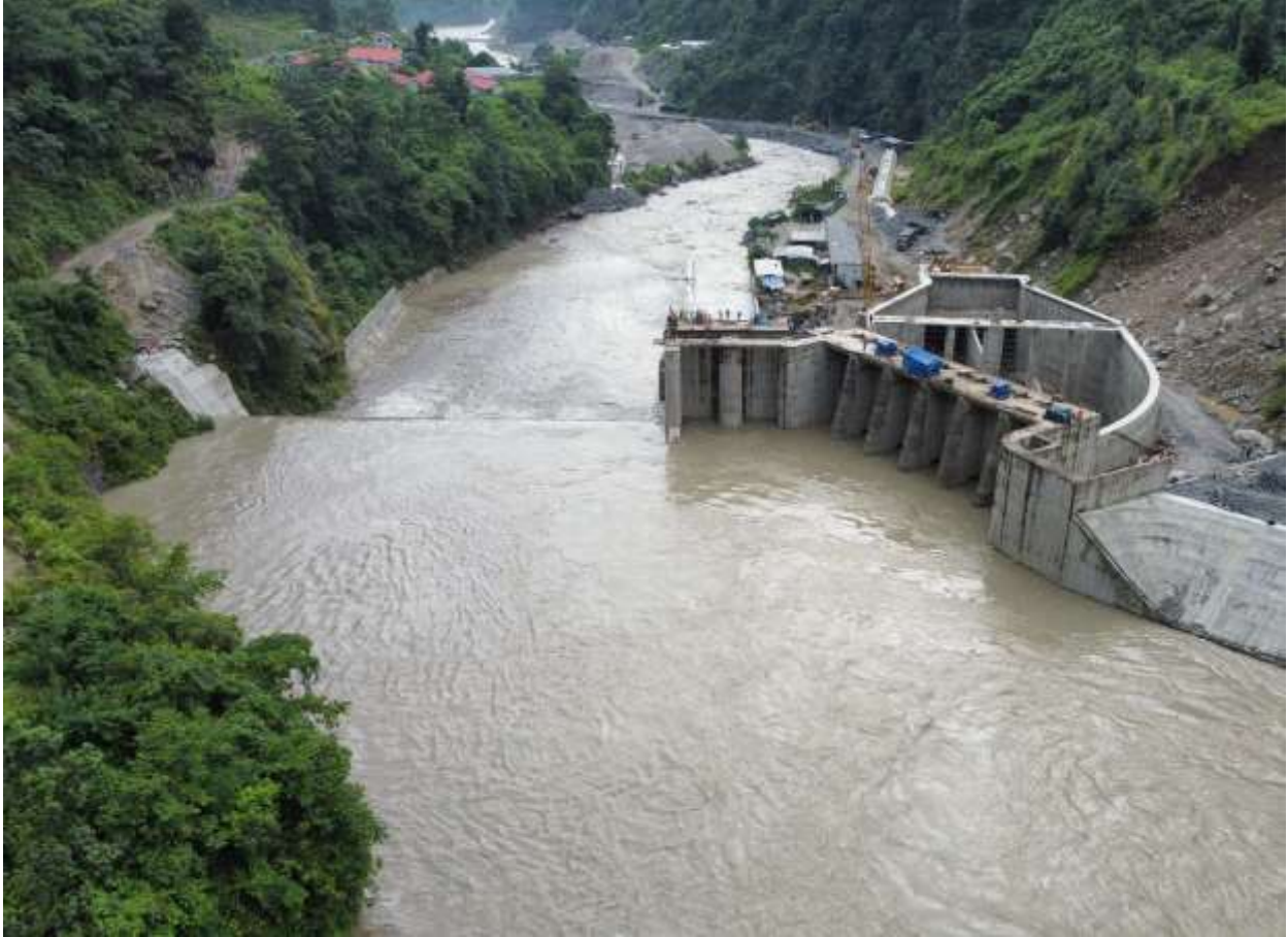
Figure 2-7: A view of headworks during water filling test
