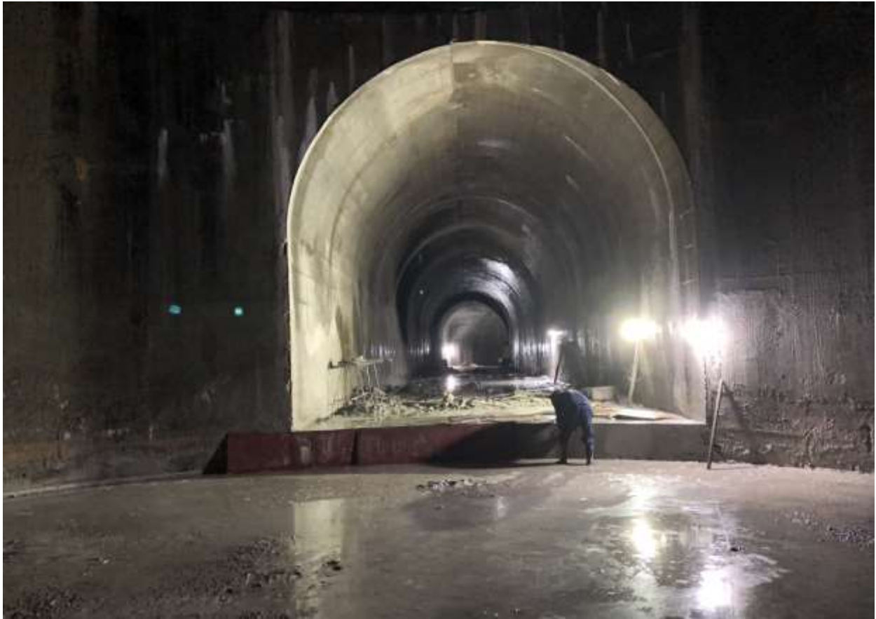
Figure 2-29: A view of full lining concrete at connecting tunnel of Surge Shaft
