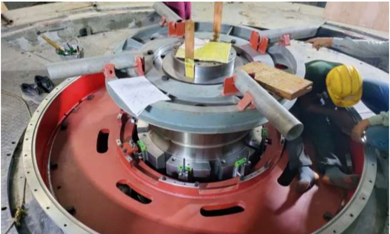
Figure 2-70: Run-out check of shaft
