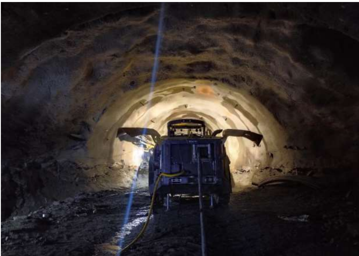
Figure 19: A view of drilling at the crown at SB-02 using Boomer
