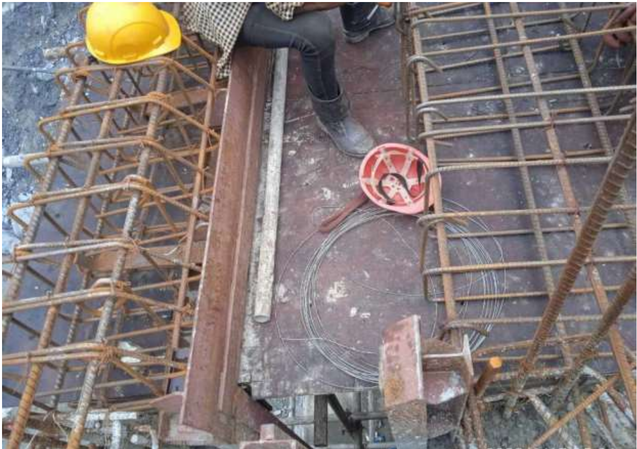
Figure 34: Embedded parts in Tailrace culvert gate
