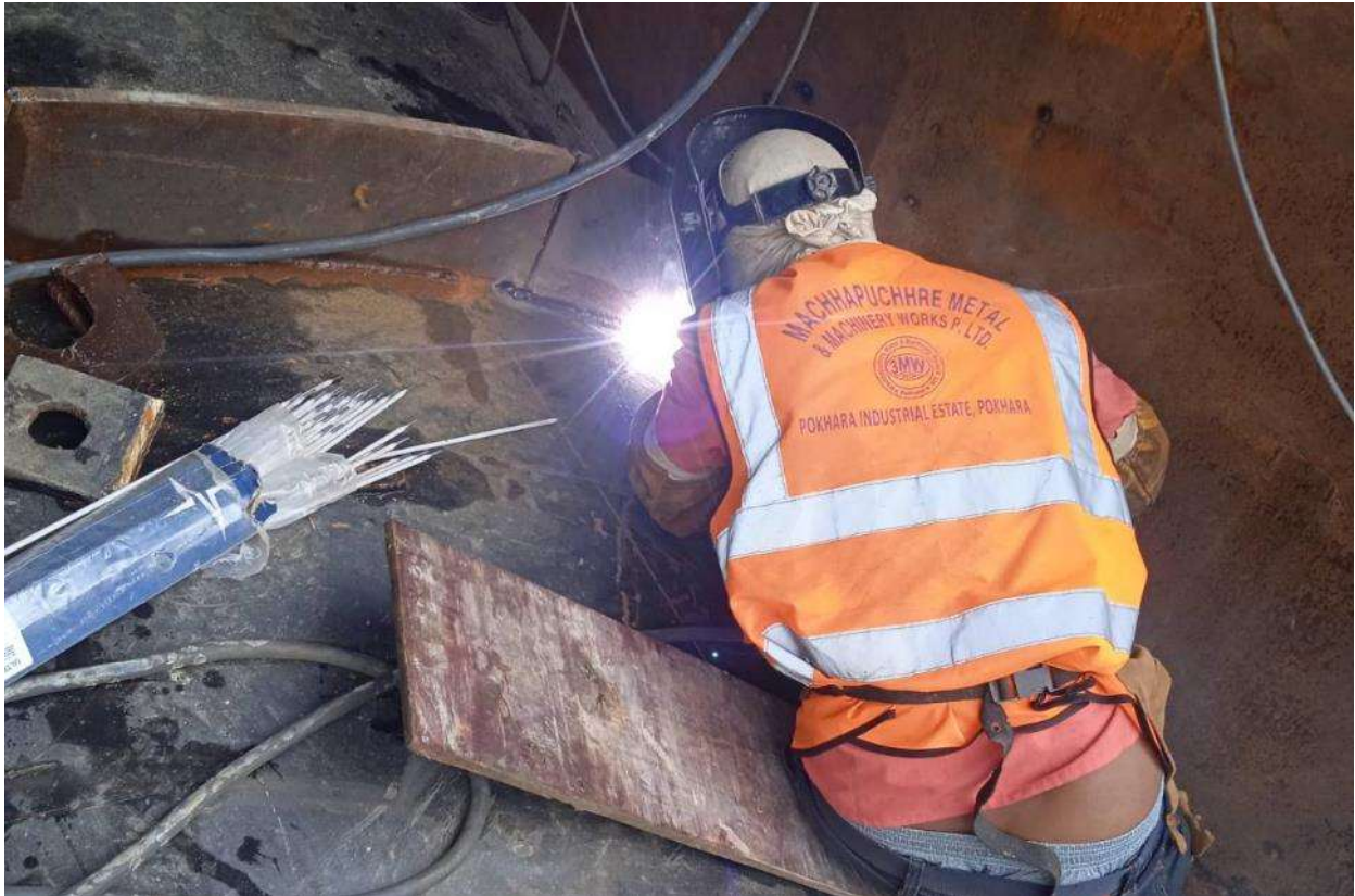
Figure 33: Welding of sickle plate of Unit 2 bifurcation
