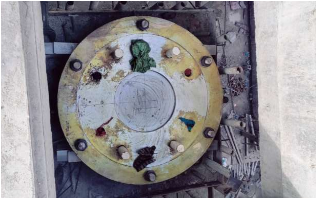
Figure 48: Installation of imbedded parts of Rotor pier
