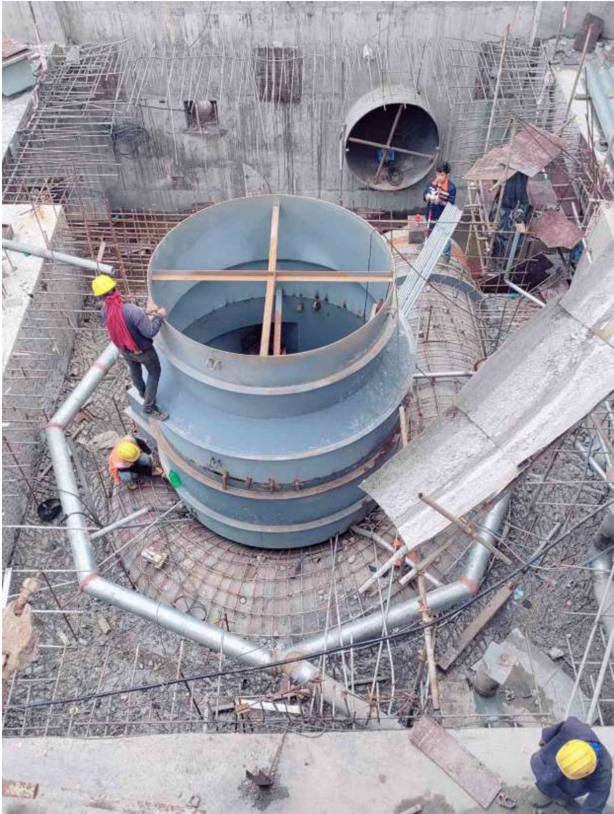
Figure 49: Installation of top part of Pit Liner and imbedded pipes
