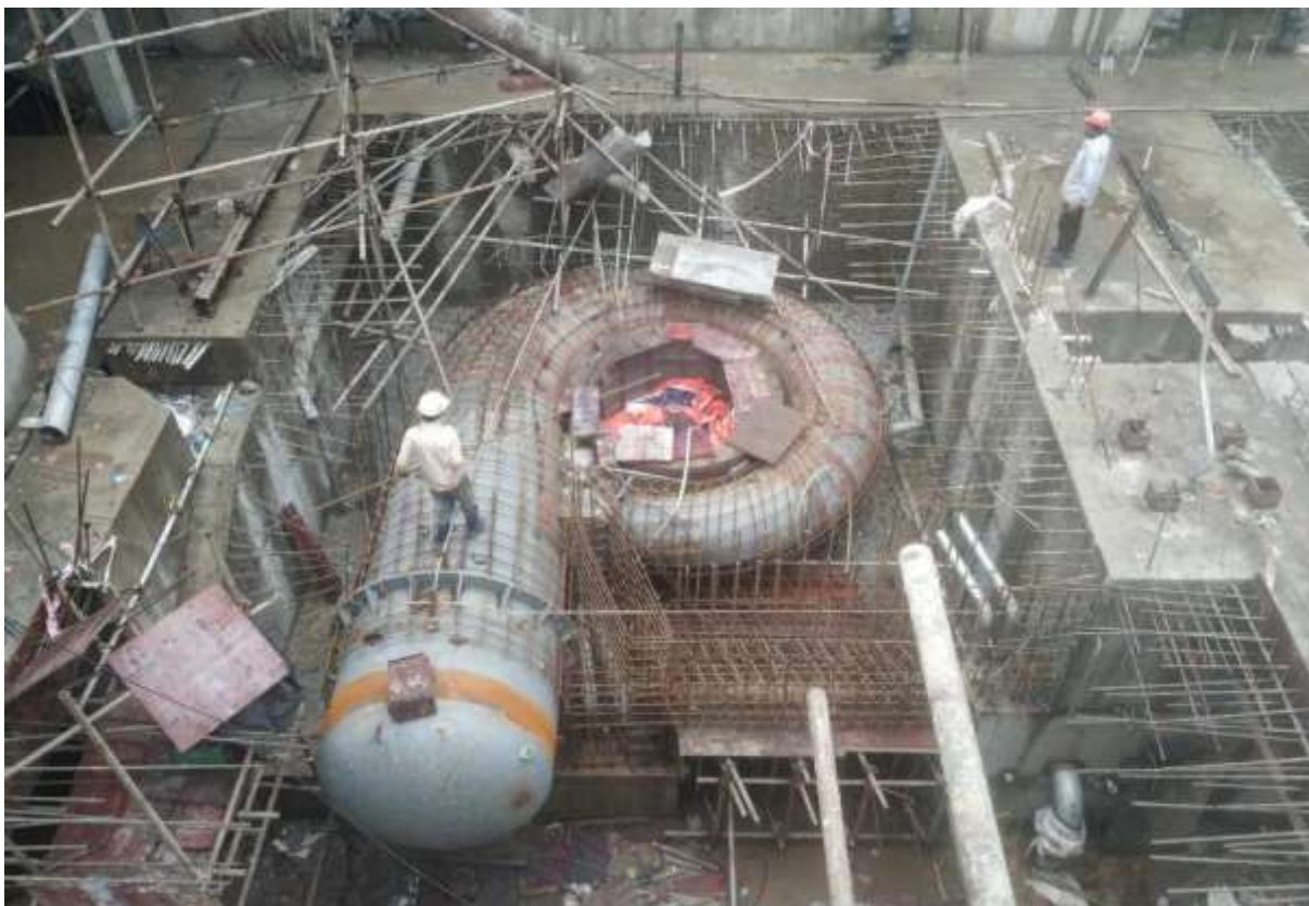
Figure 46: A view of spiral case unit 1 ready for 2nd stage embedding concrete
