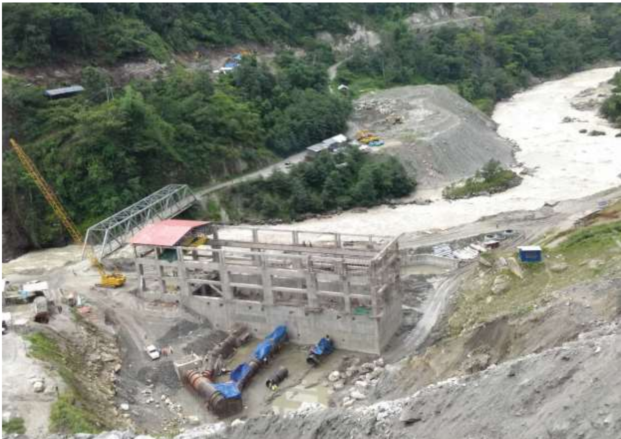
Figure 43: View of powerhouse with roofing works completed at Bay01
