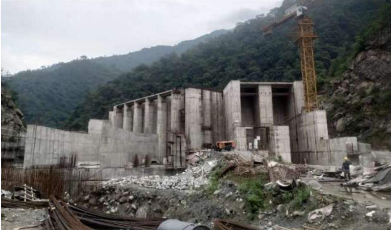
Figure 8: Intake and Undersluice section from downstream
