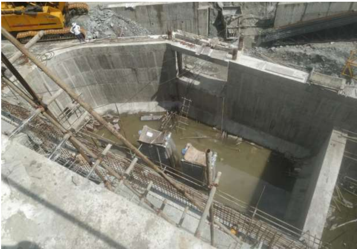
Figure 30: Concrete works at tailrace culvert
