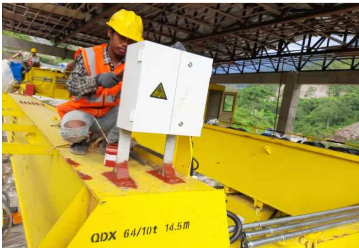
Figure 44: Electrical wiring works of EOT crane
