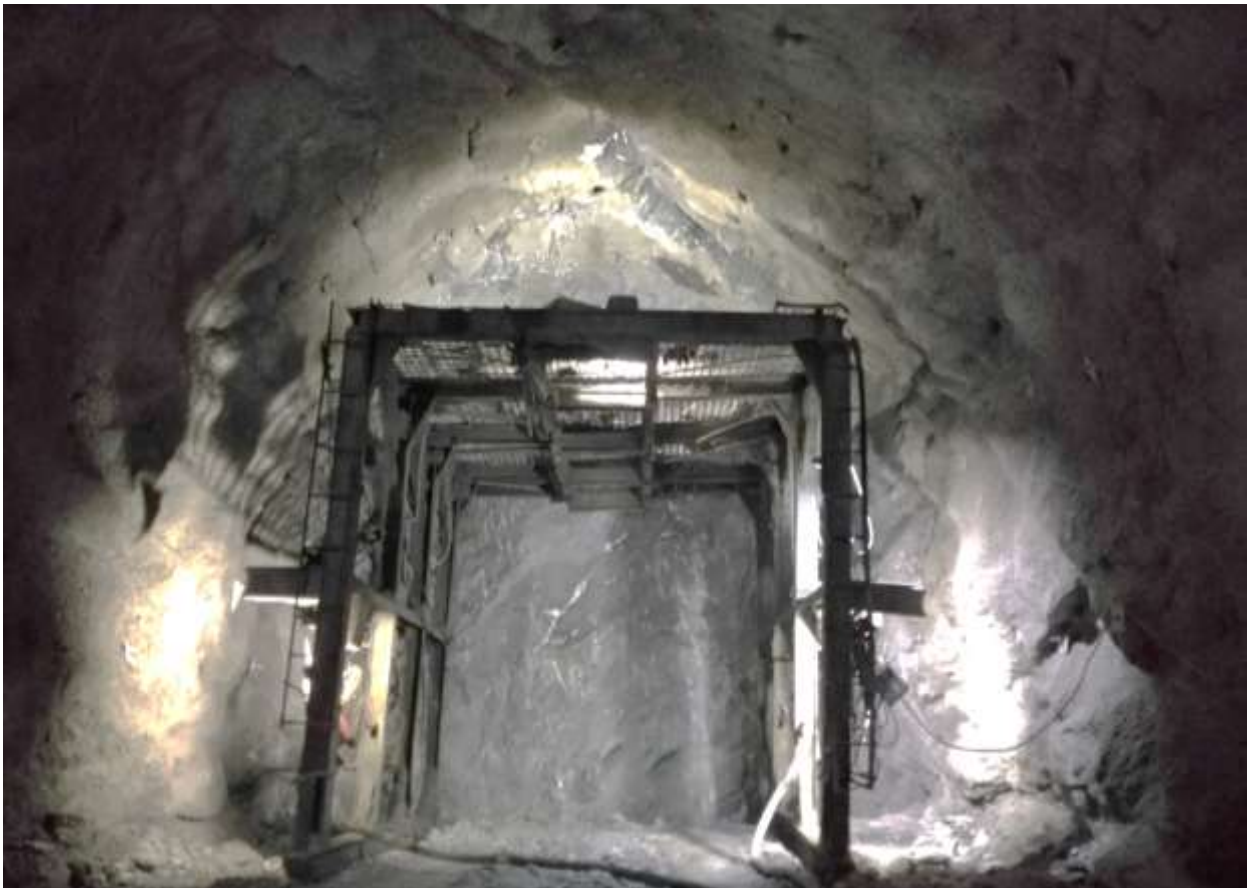
Figure 23: A view of face drilling works of HRT from Outlet
