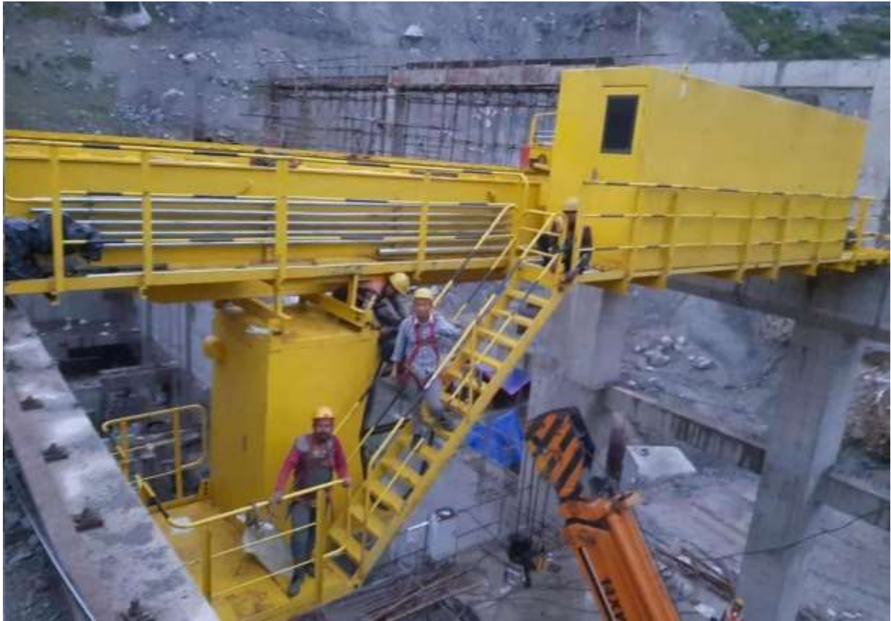
Figure 42: EOT crane after installation
