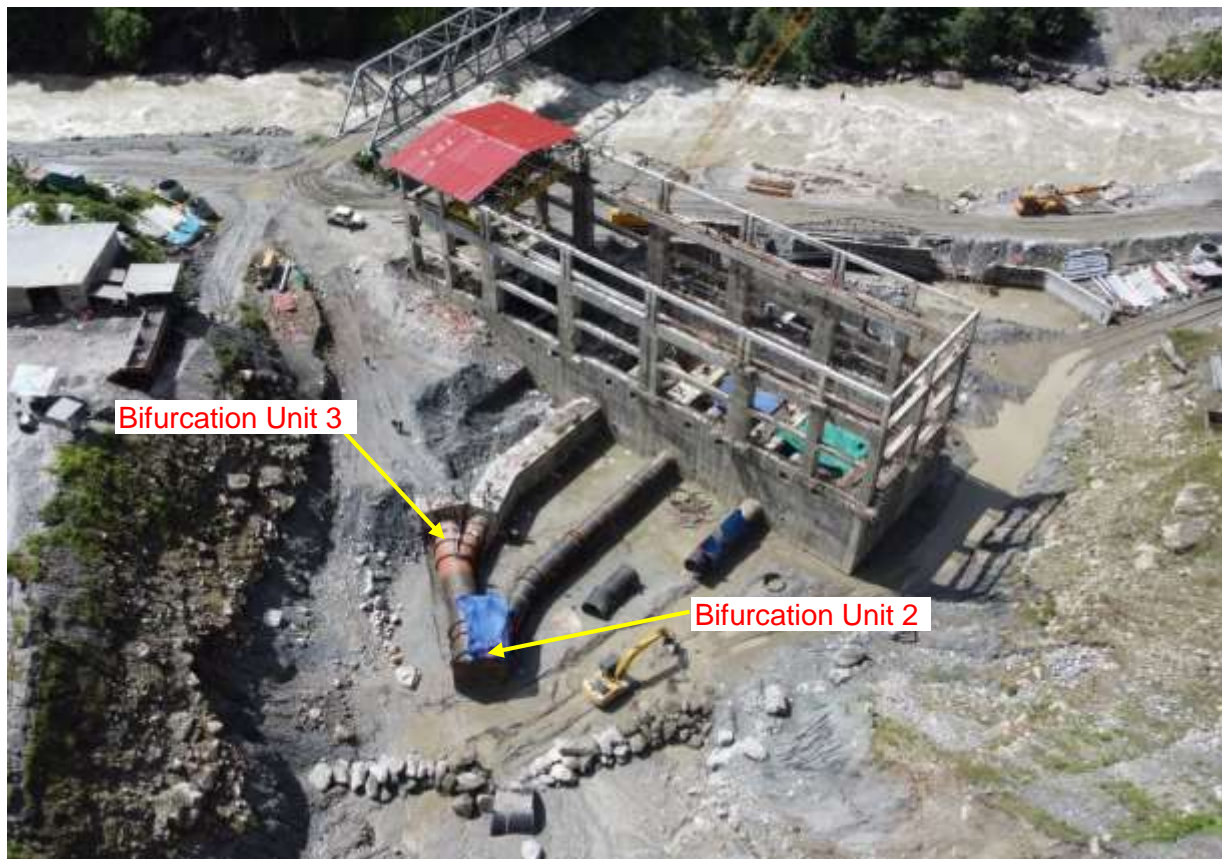
Figure 31: Aerial View of Powehouse Penstock Pipe Erection
