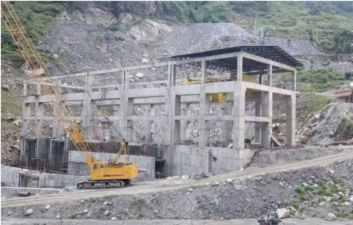
Figure 28: Concreting works at Crane beam at Bay 04
