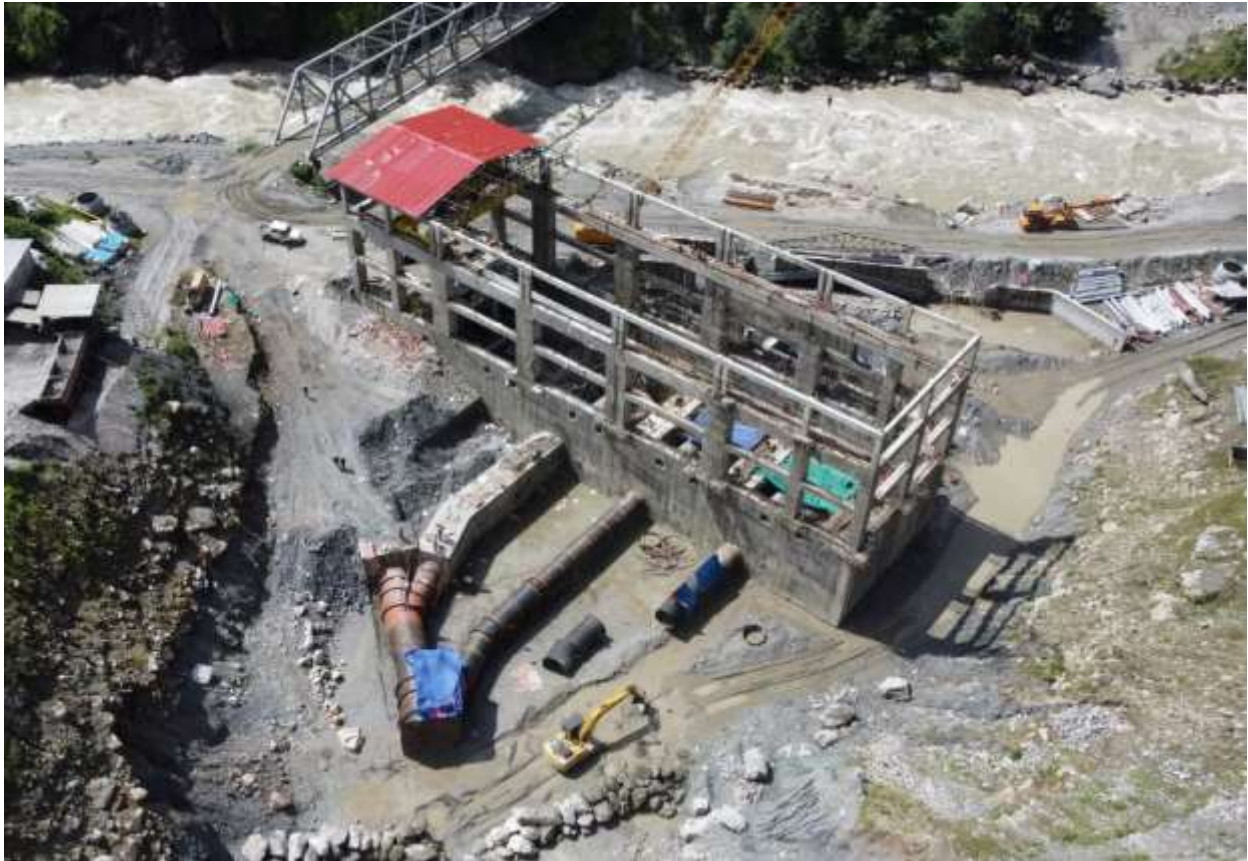
Figure 29: A view of Powerhouse and manifold section
