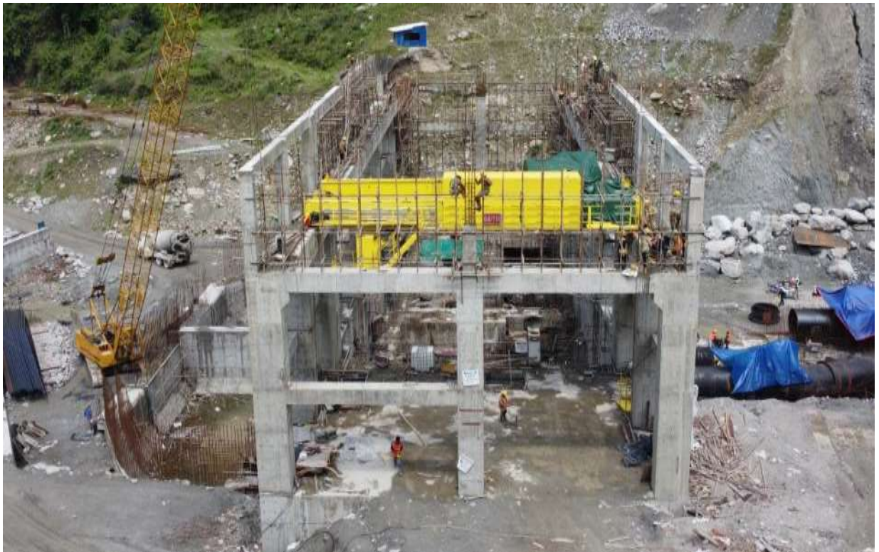
Figure 41: A view of EOT crane and penstock manifold
