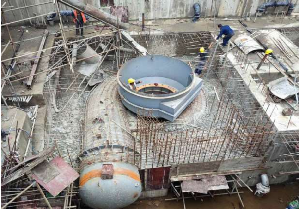
Figure 47: Installation of bottom part of Pit Liner
