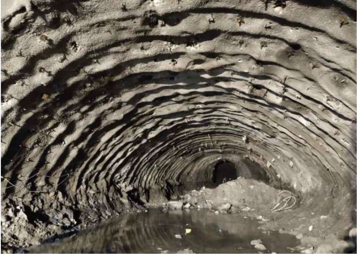
Figure 22: Grouting works in the crown of Settling Basin
