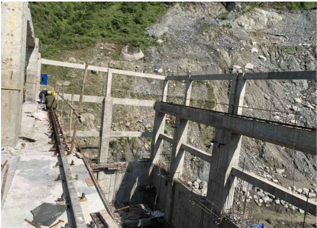
Figure 52: Installation of rail track along the Powerhouse corbell beam
