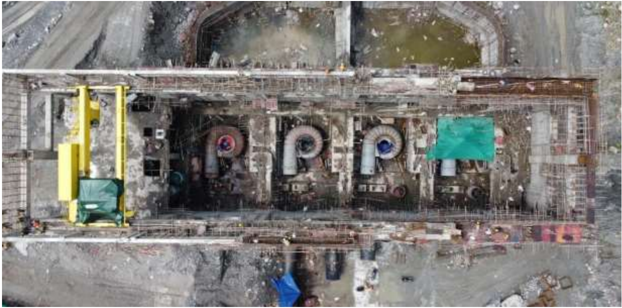
Figure 40: Aerial View showing all four spiral cases and EOT crane
