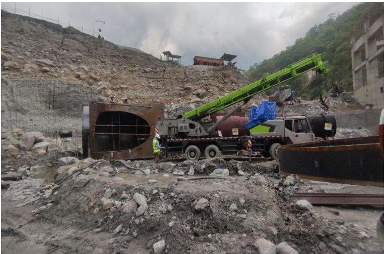
Figure 32: Erection of Bifurcation Unit 2 (Dia: 3.9 m to 2.25m and 3.18 m, thk: 30mm)
