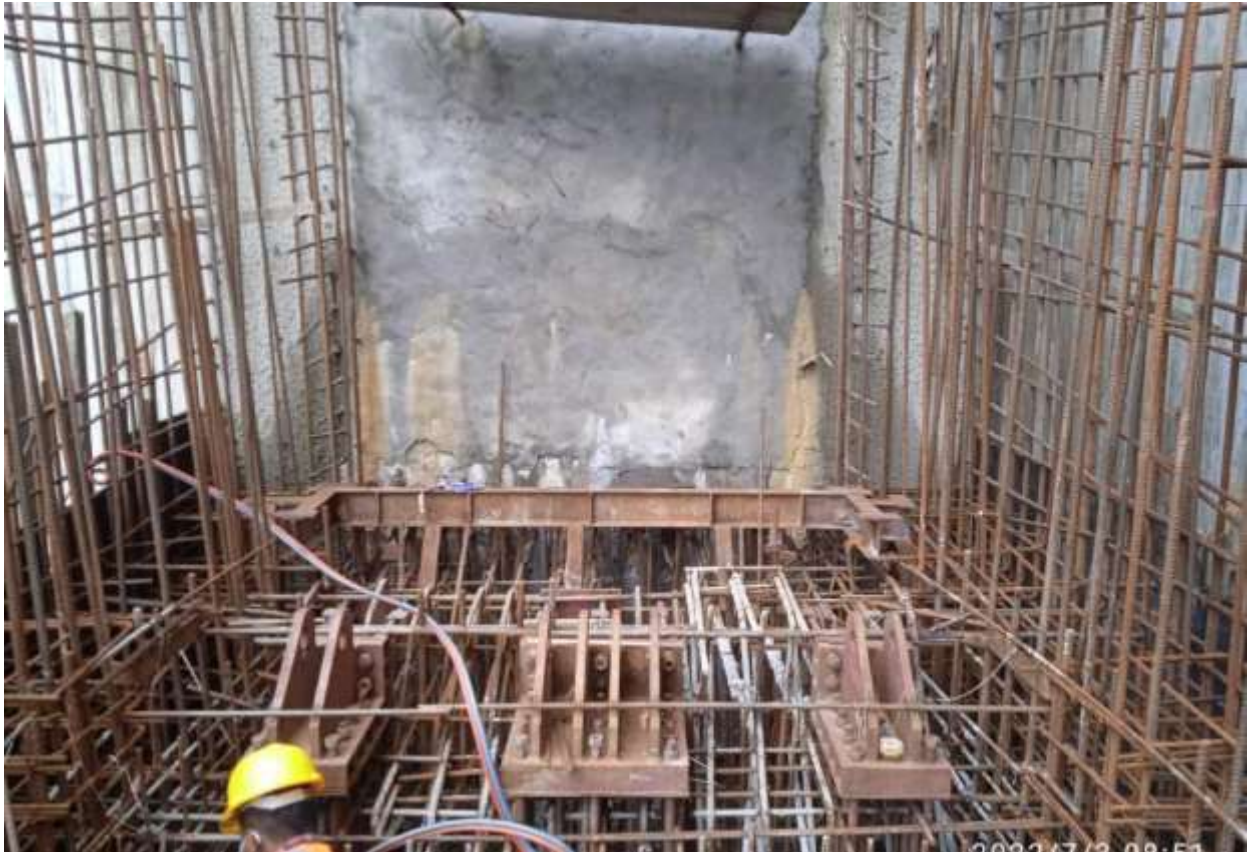
Figure 35: Embedded parts in trash passage
