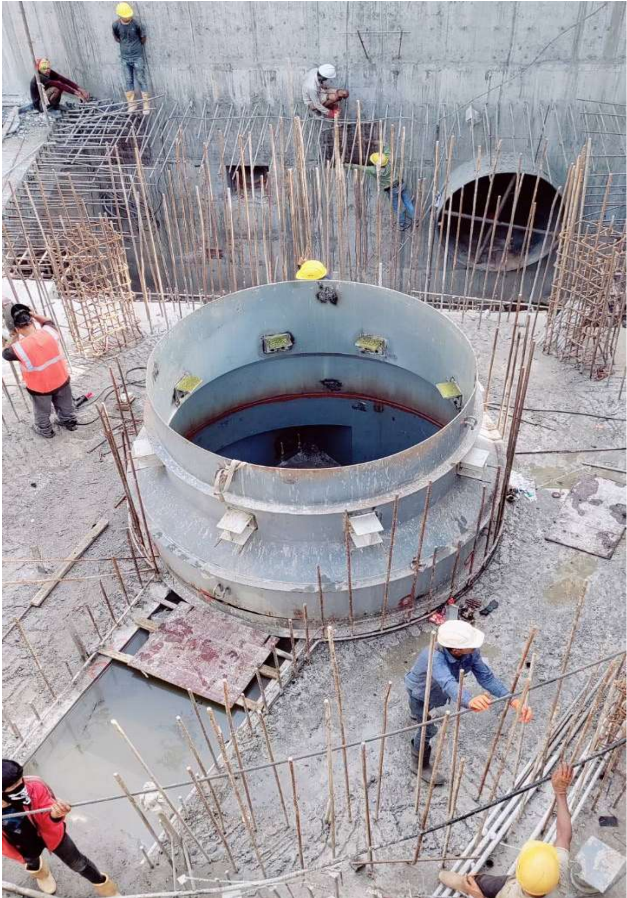
Figure 50: View of Pit Liner after second stage concreting
