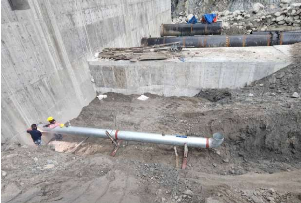
Figure 51: Installation of Ventilation pipes under the control room
