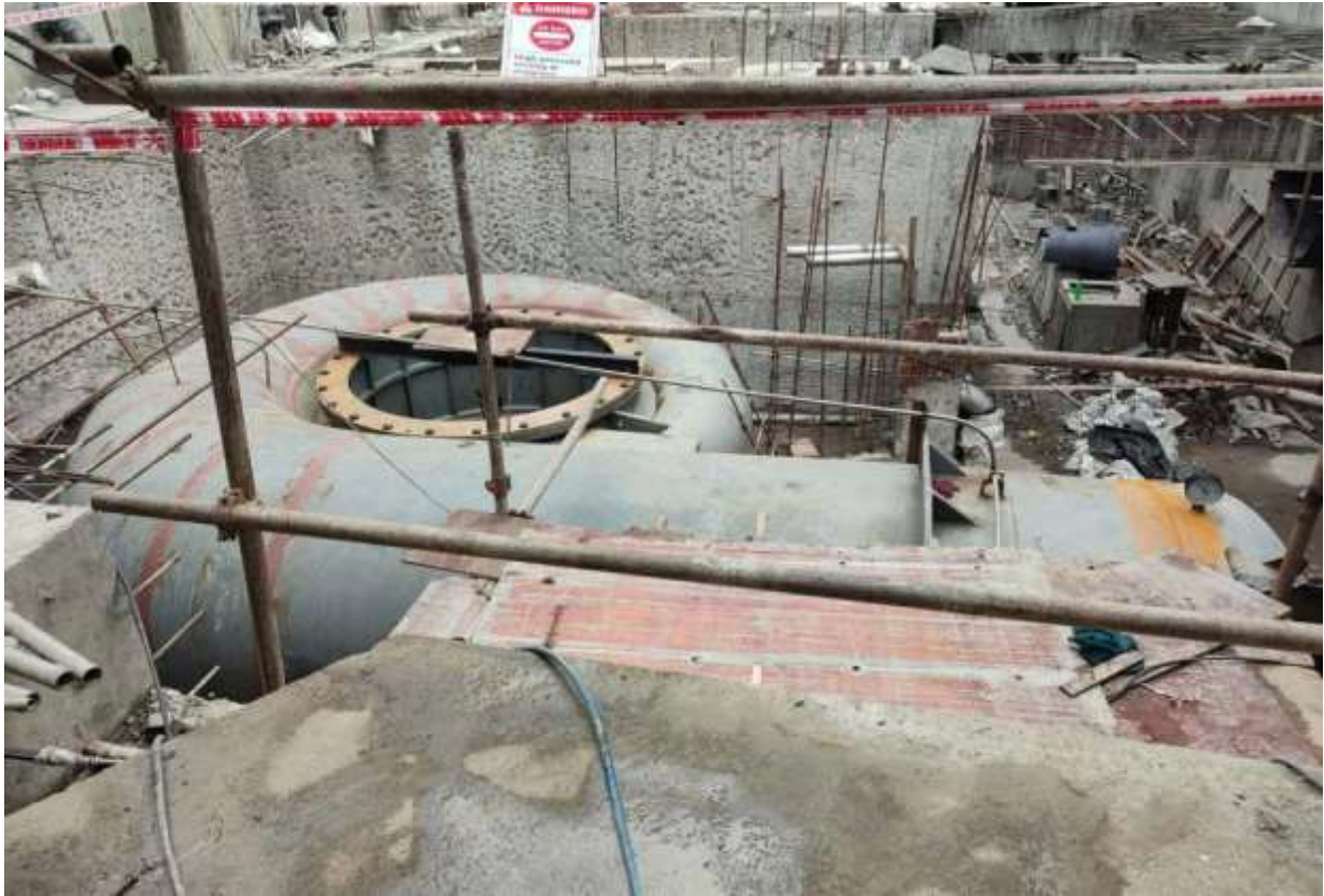
Figure 45: Hydrostatic Pressure test at Spiral case unit 01
