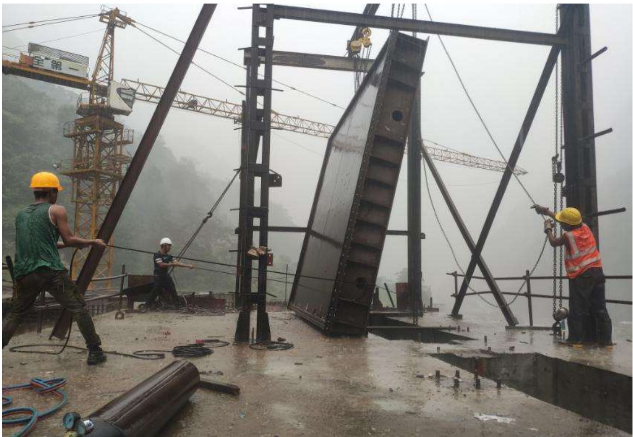
Figure 36: Installation of intake gates
