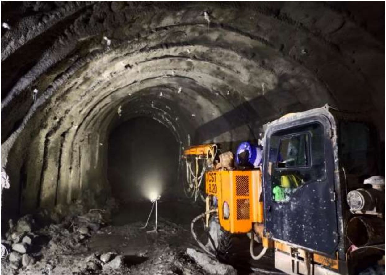
Figure 20: Application of shotcrete using Robotic shotcrete machine
