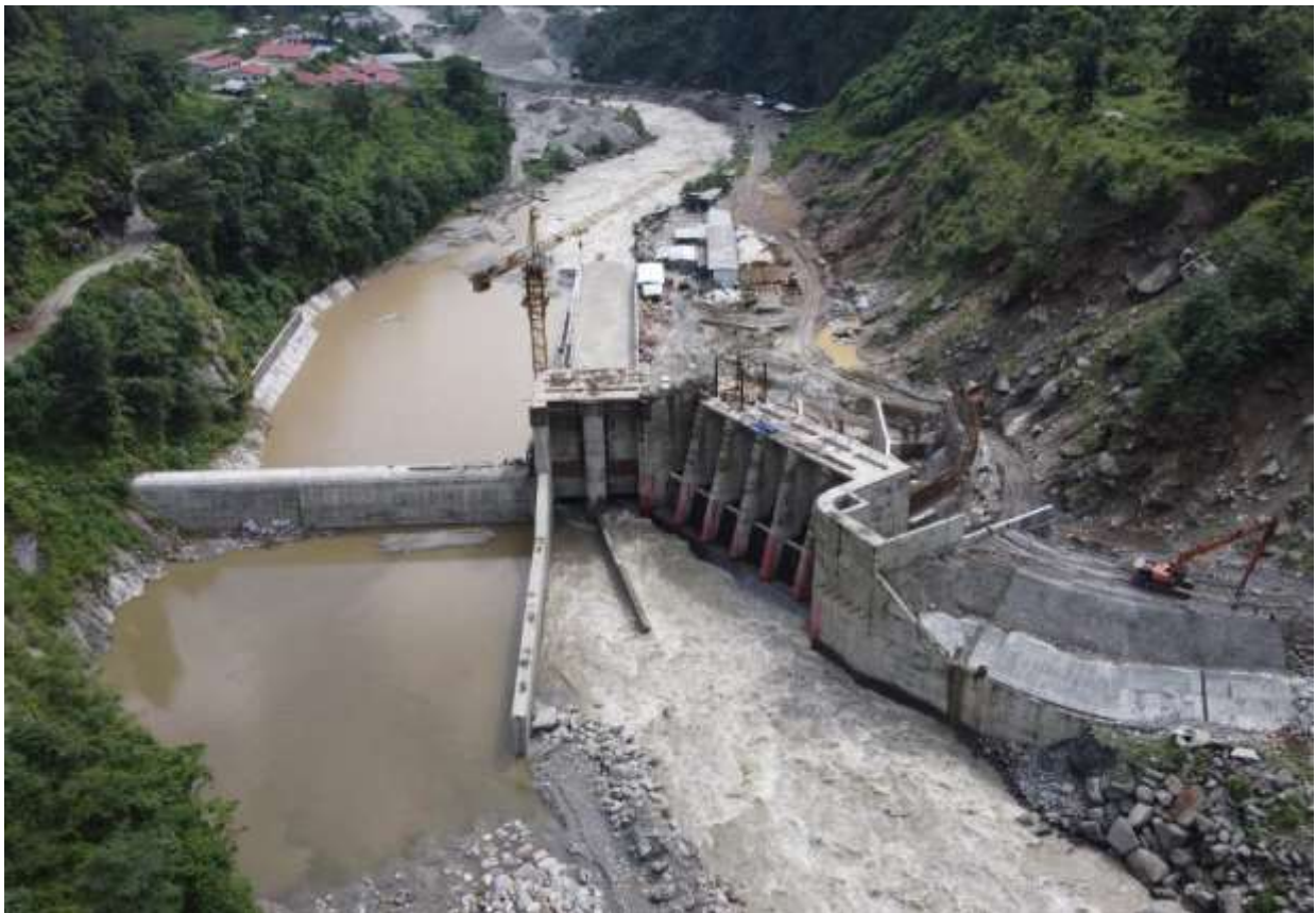
Figure 11: Aerial view of headworks with completed weir to the left
