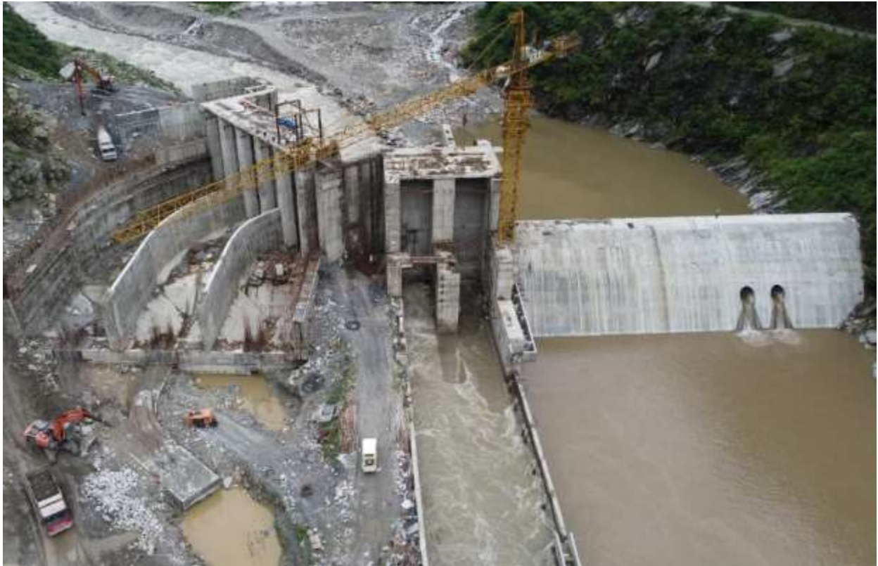
Figure 10: Aerial view of headworks with completed weir to the right
