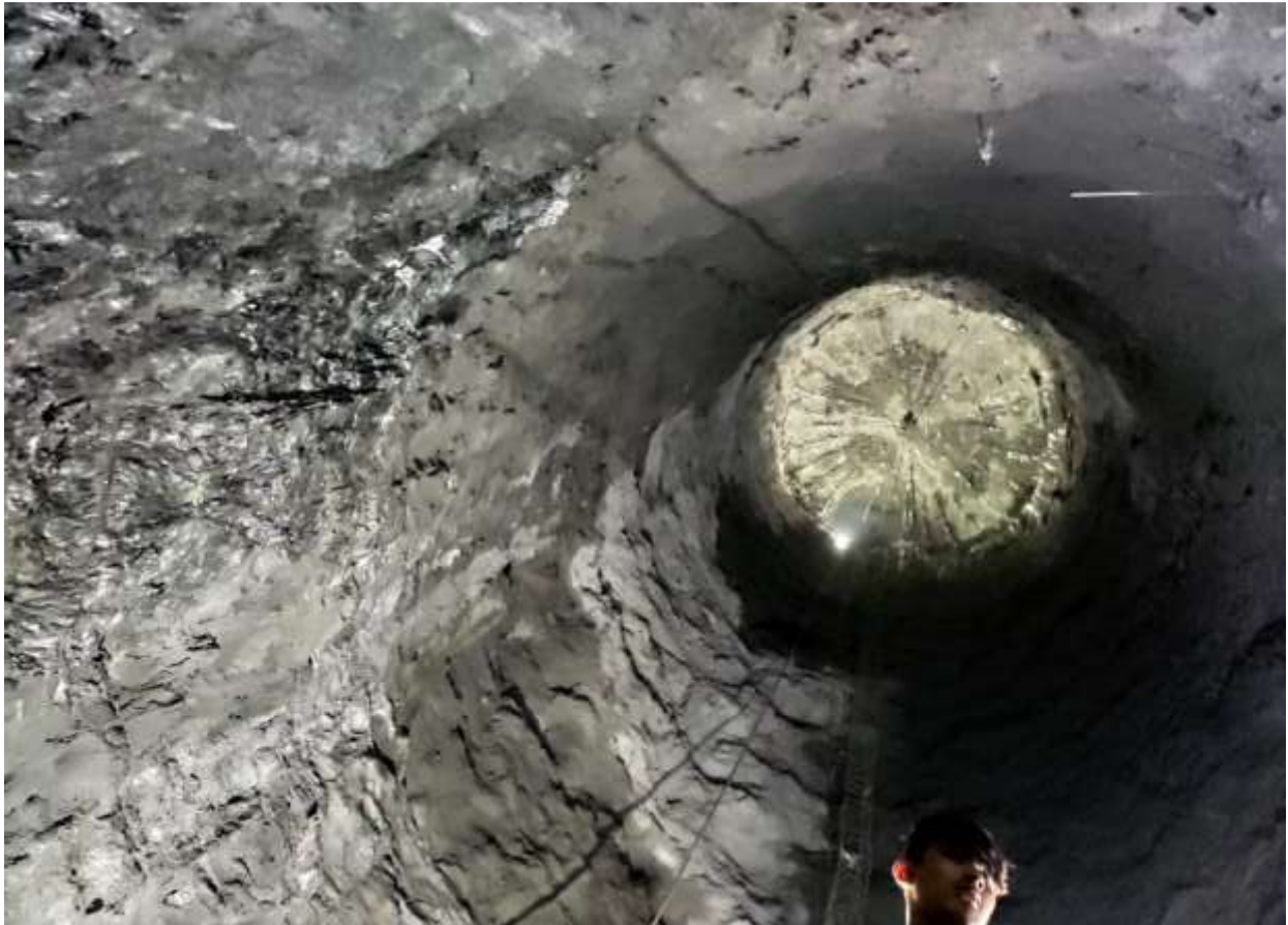
Figure 24: A view of Surge Shaft from invert
