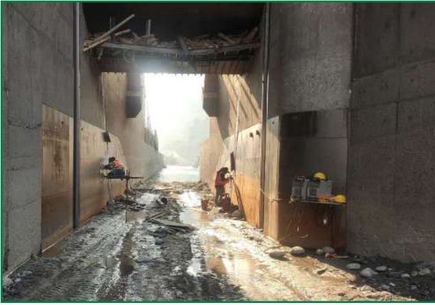
Preparation work for radial gate installation at undersluice (left) and fabrication of bends (right)
