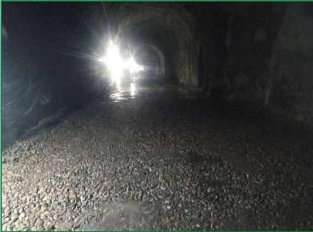
Placement of base material for backfill of HRT invert (left) and rebar layout at HRT invert (right)
