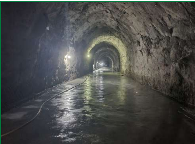
A view of concreting works at HRT invert (left) and rock support works at SB (right)
