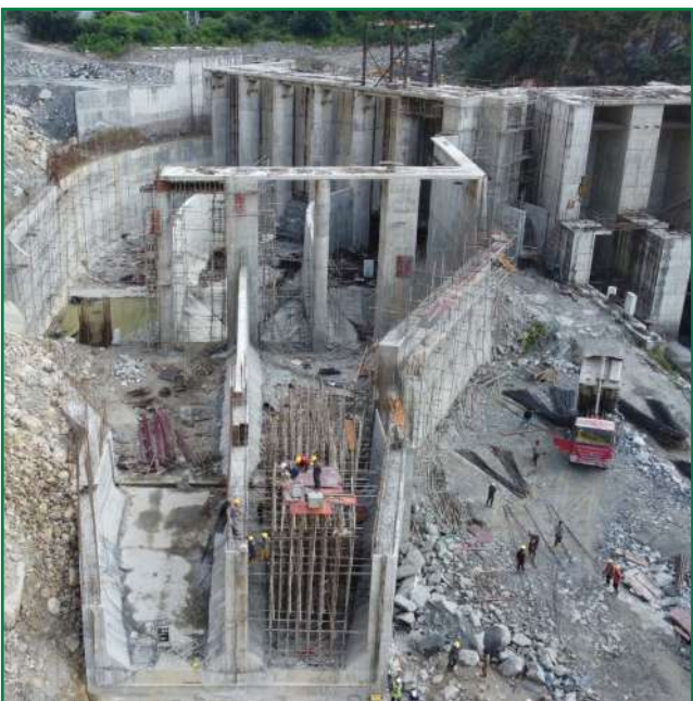
Construction of conveyance tank
