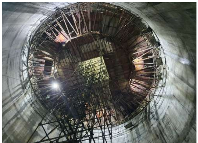
A view of concreting works at surge shaft from ventilation tunnel (left) and invert (right)
