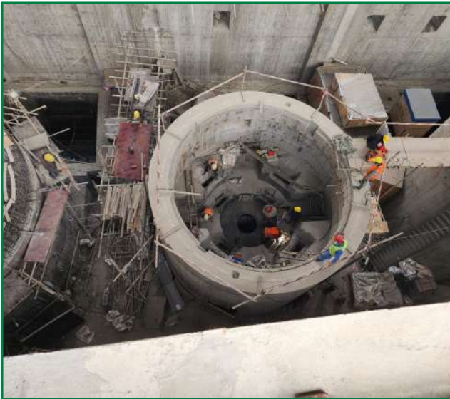
Preparation of installation of stator foundation at unit 02 (left) and assembly of rotor at rotor pier (right)
