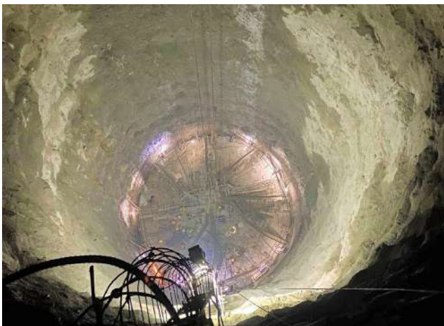
A view of concreting works at surge shaft from ventilation tunnel (left) and invert (right)
