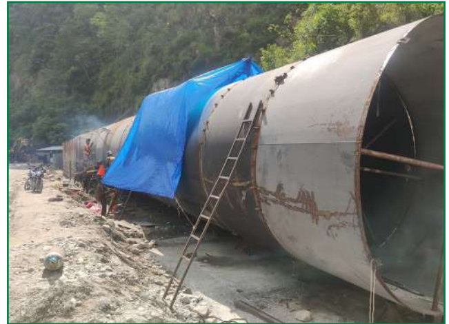
Approach pipe erection
