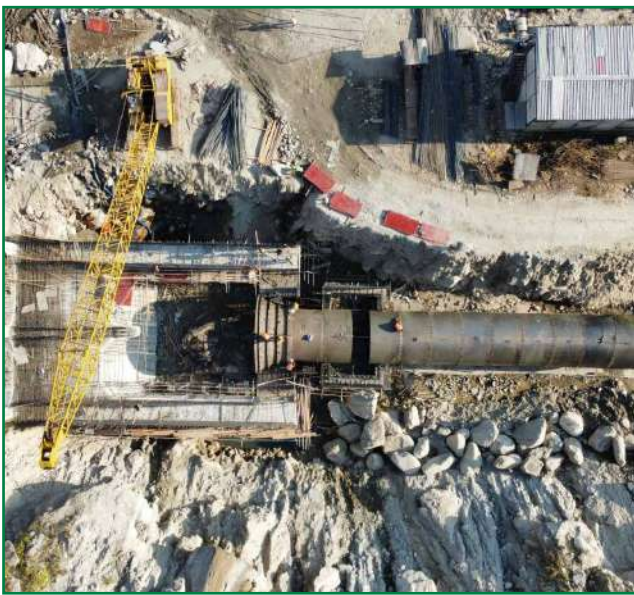
Installation and bellmouth (left) and approach pipe (right)
