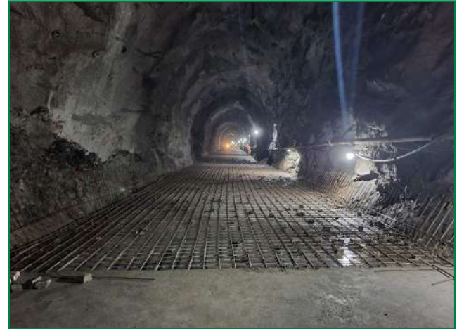
Placement of base material for backfill of HRT invert (left) and rebar layout at HRT invert (right)
