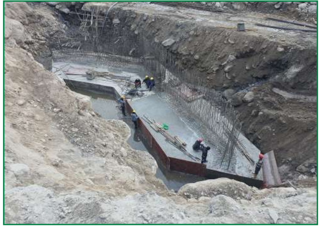
Down stream floodwall
