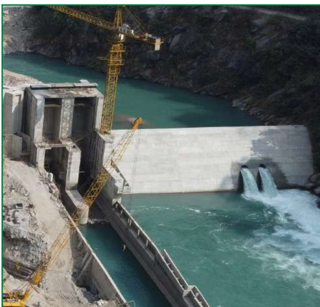
Aerial view of weir and under sluice
