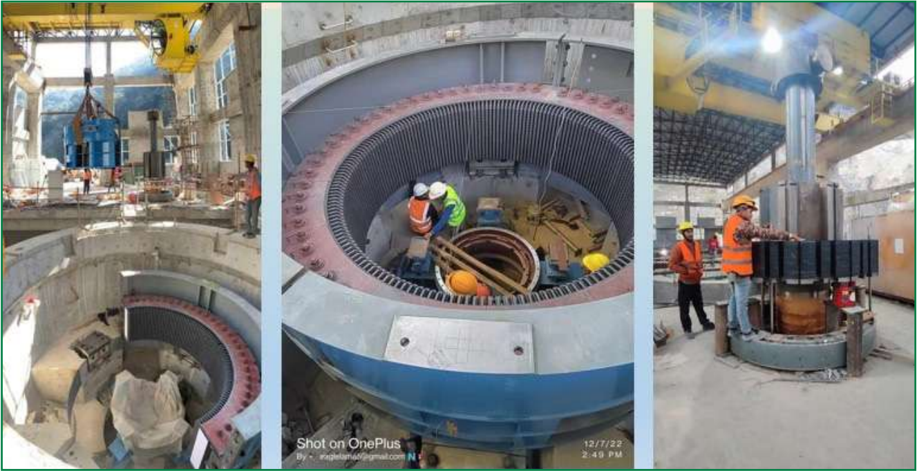
Preassembly of stator and rotor (generator parts) at the site
