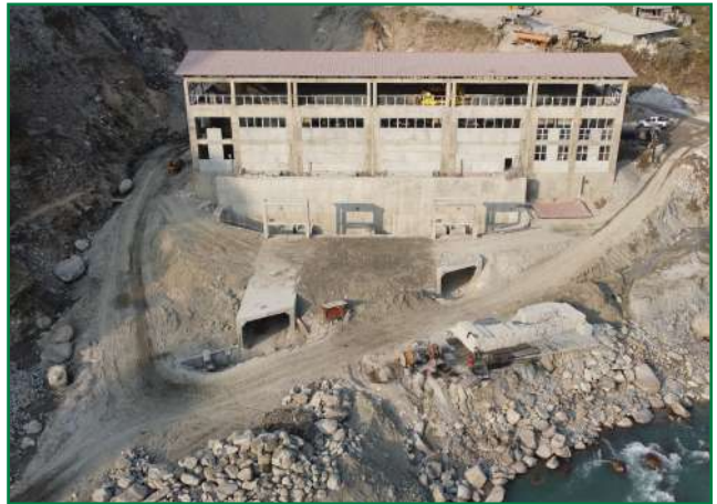
Aerial view of Powerhouse and tailrace section
