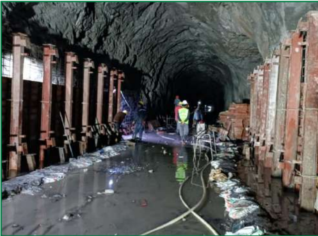
Formwork placement for wall concreting of HRT
