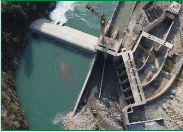
Final stage river diversion at head works
