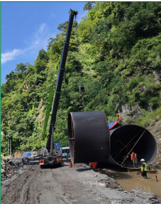
Erection of approach pipes (left) and installation of trashrack frame in conveyance tank (right)
