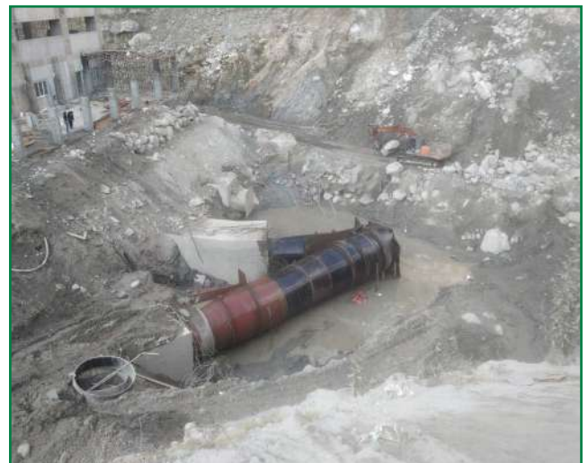
Rock excavation of anchor block completed (left) and muck clearing at penstock manifold region (right)
