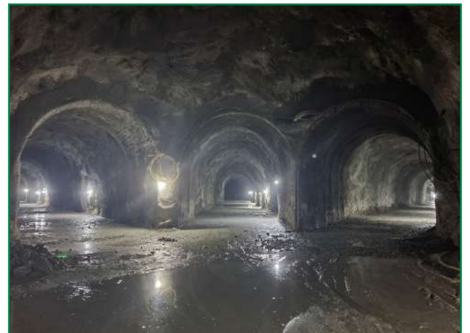
A view of flushing tunnel (left) and connecting tunnel junction (right)
