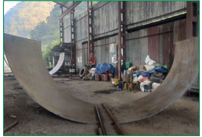
Preparation work for radial gate installation at undersluice (left) and fabrication of bends (right)
