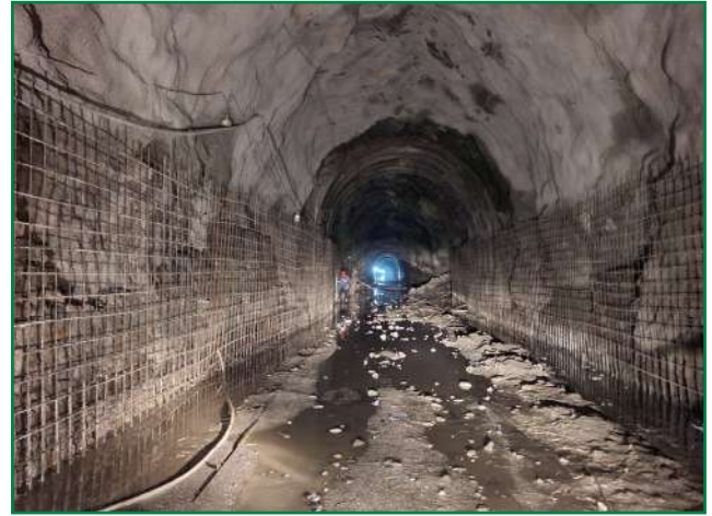
Rebar layout for wall concreting of HRT
