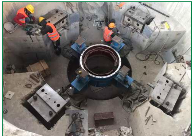
Stator foundation at unit 1
