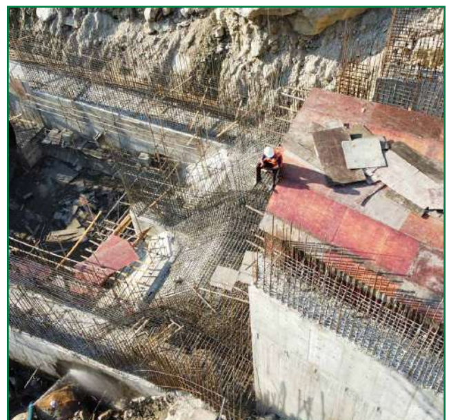
Conveyance Tank rebar layout
