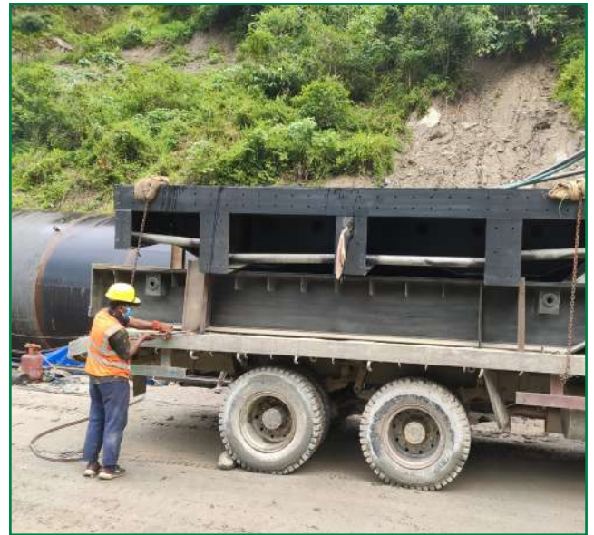
Erection of approach pipes (left) and delivery of radial gate parts at the site (right)
