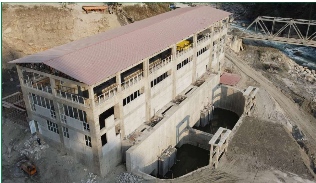
A view of completed powerhouse superstructure and tailrace section
