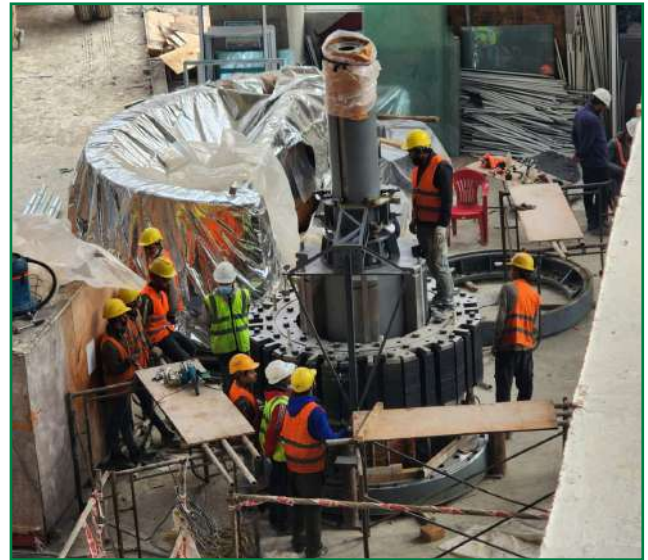
Preparation of installation of stator foundation at unit 02 (left) and assembly of rotor at rotor pier (right)
