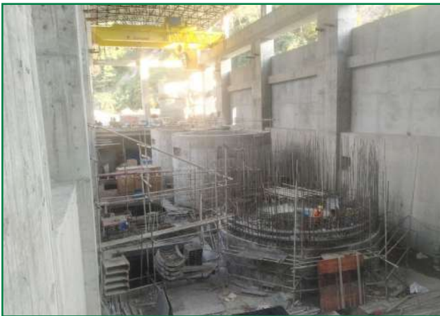
Concrete works at Generator Casing at Unit 3
