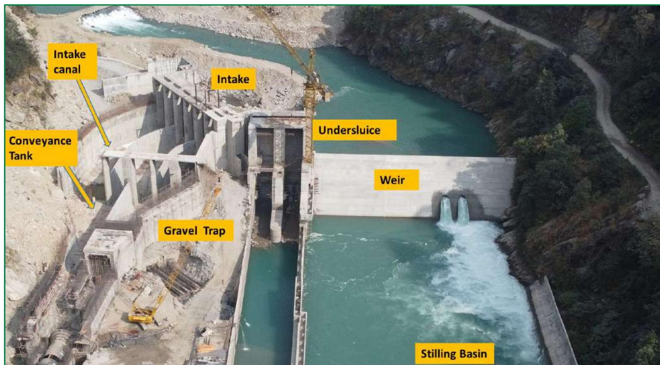
Bird's eye view of Heaworks under construction
