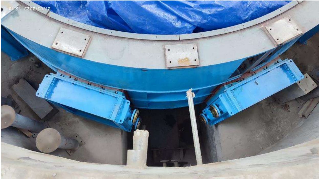
Figure 2-45: Final assembly of stator air cooler
