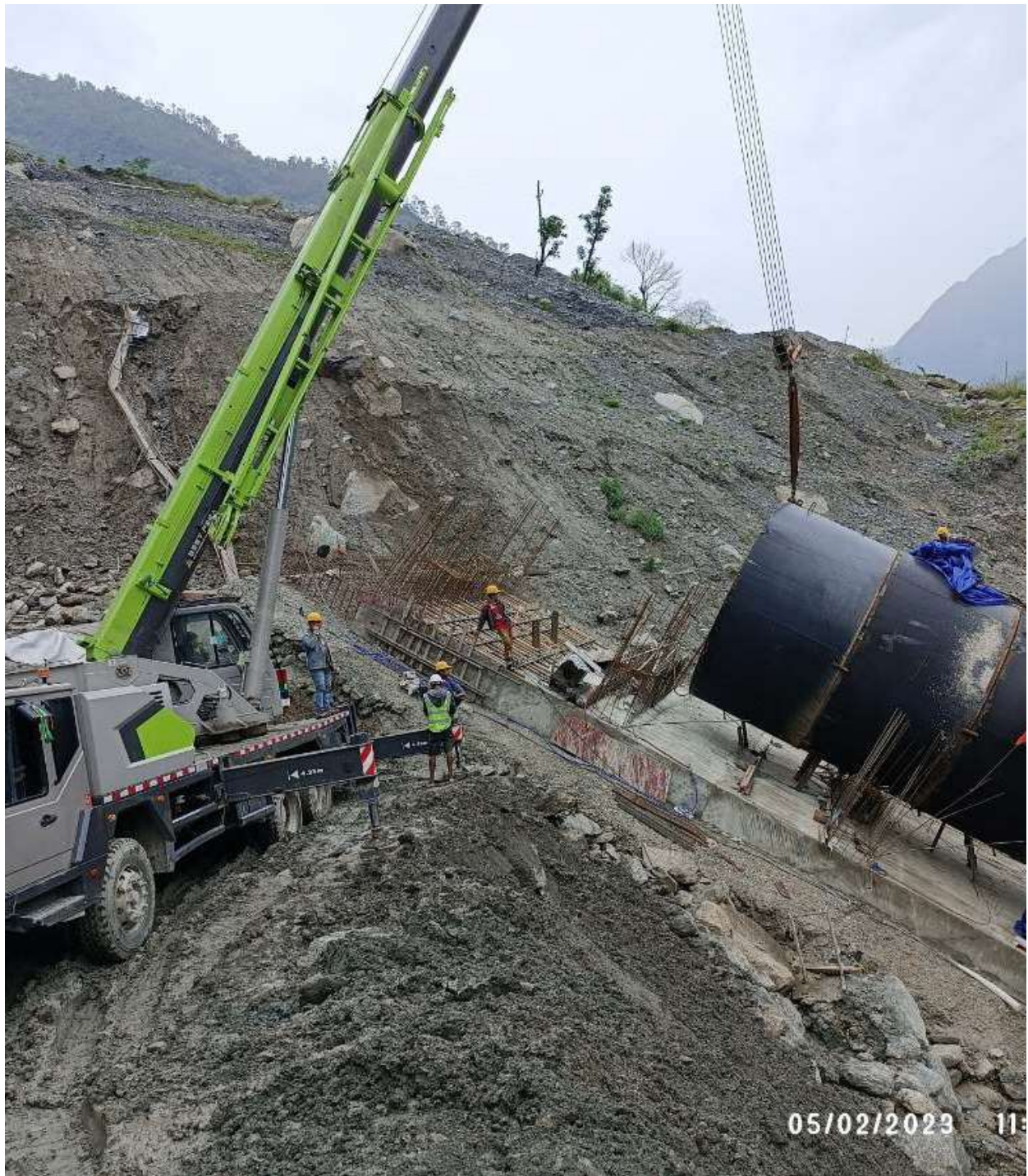
Figure 2-27: Installation of penstock pipe of thickness 28 mm.
