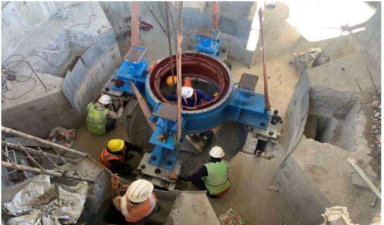
Figure 55: Installation of lower bracket in unit 1
