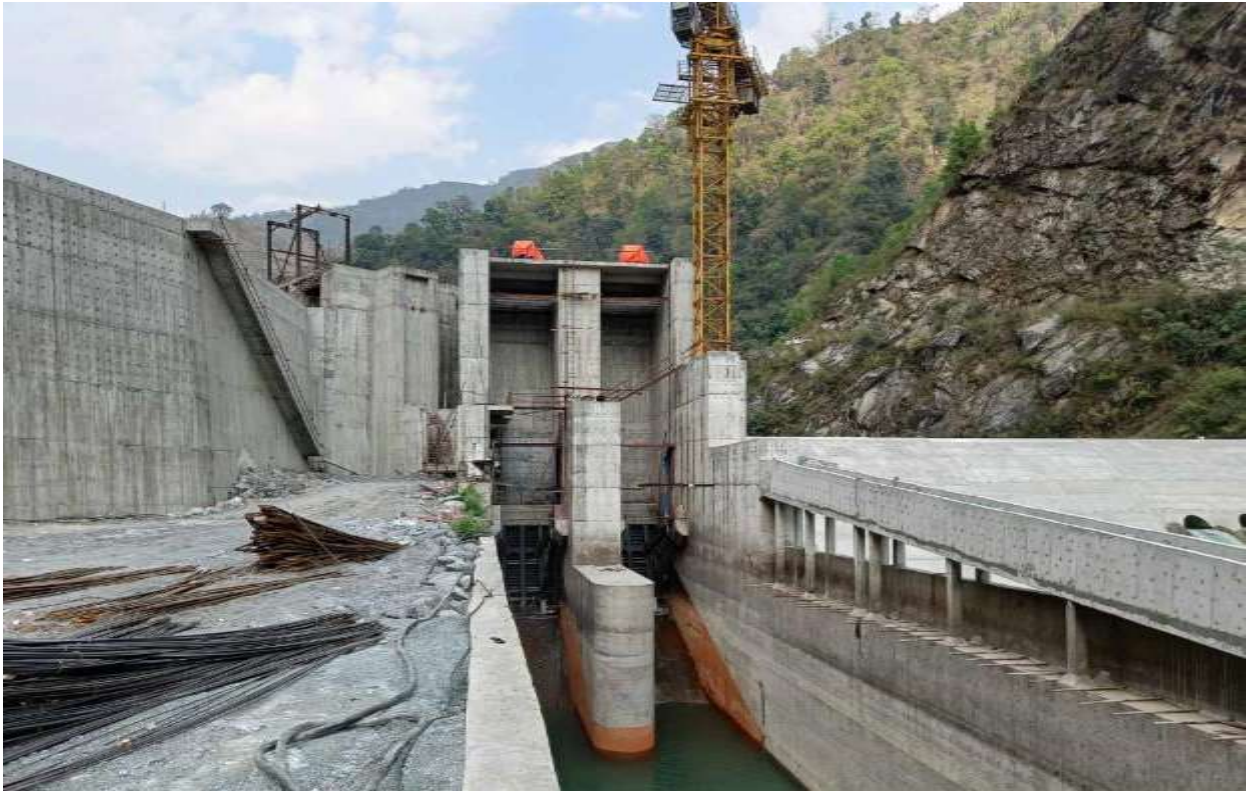
Figure 2-8: Gate installation works at undersluice
