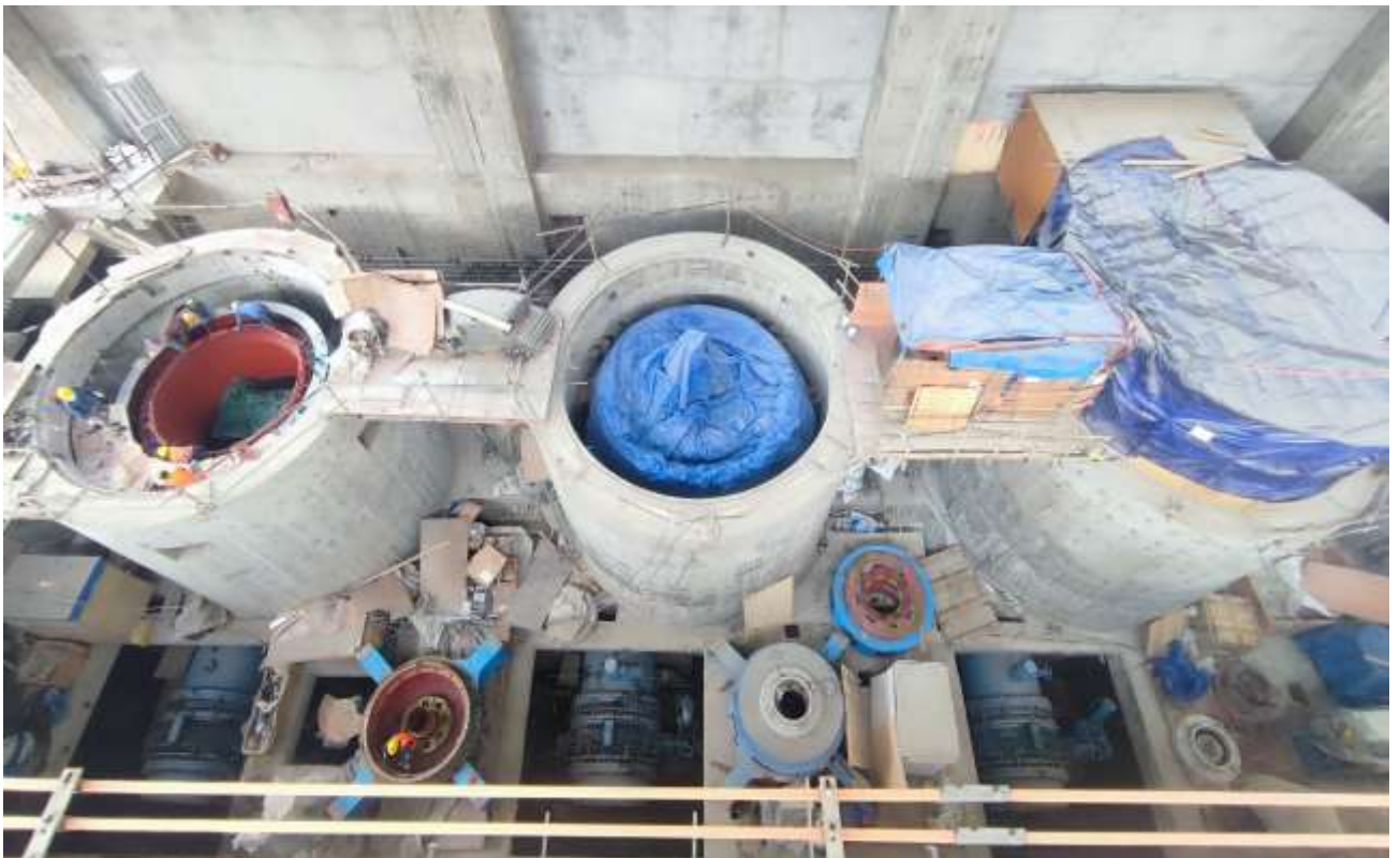
Figure 66: All 4 units M.I.V. lowered to its position
