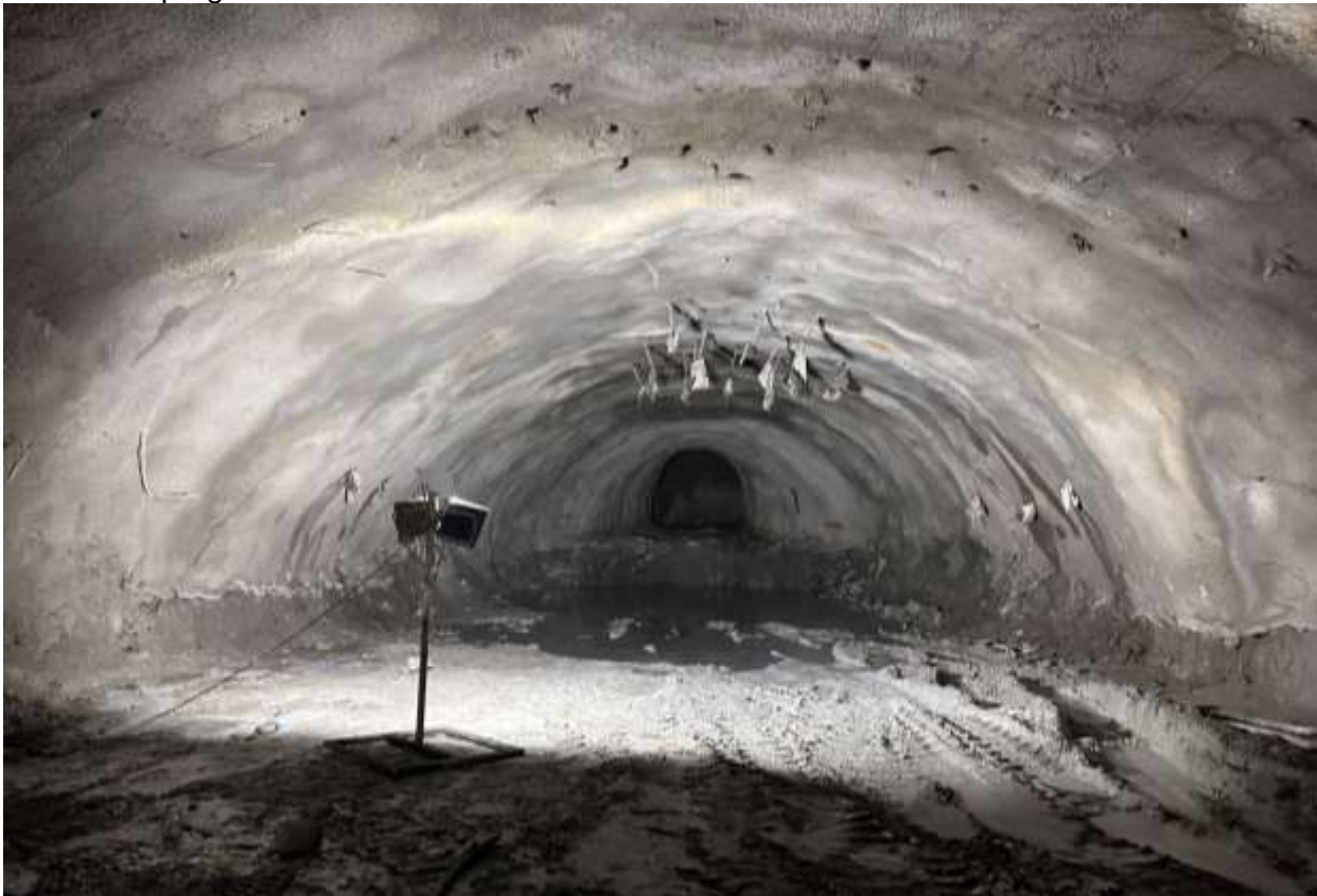
Figure 2-13: A view of SB 03 face
