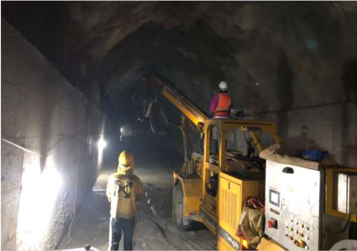
Figure 2-15: Final lining shotcrete works at HRT
