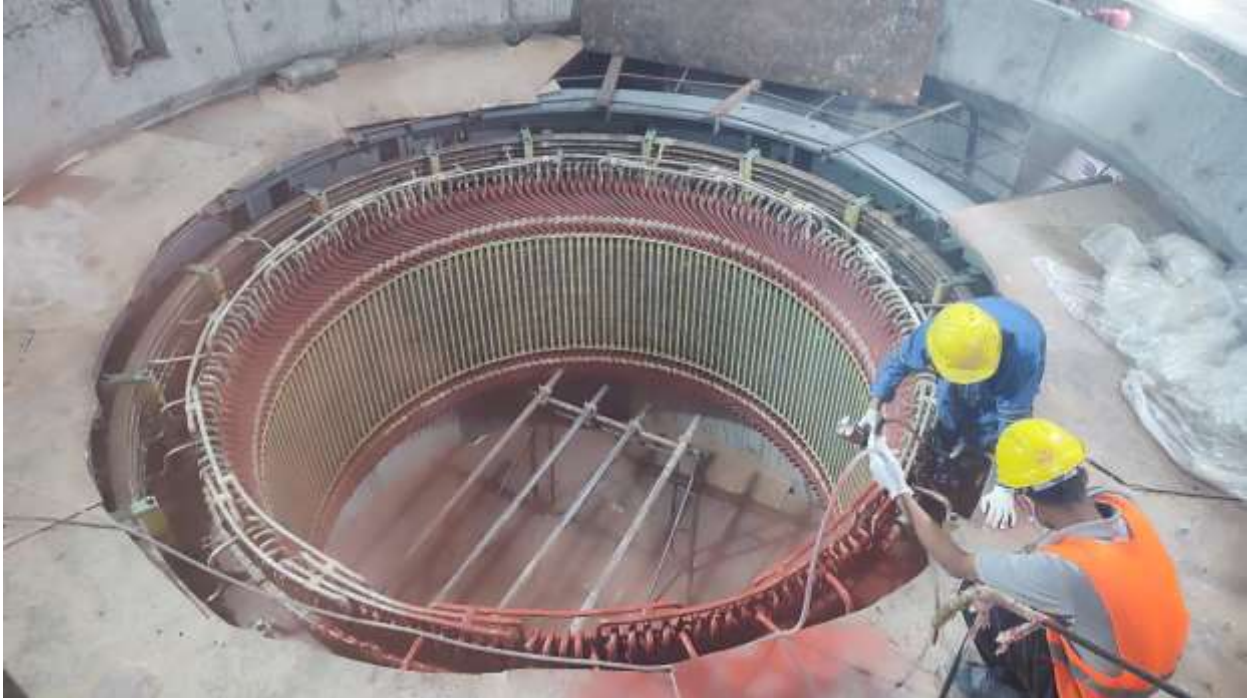
Figure 2-42: Varnish coating of stator coils after brazing work completion
