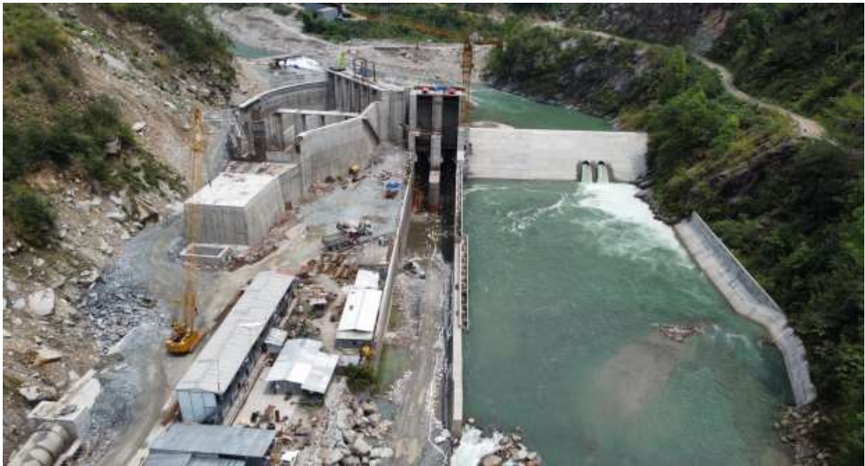
Figure 2-4: Aerial view of Headworks
