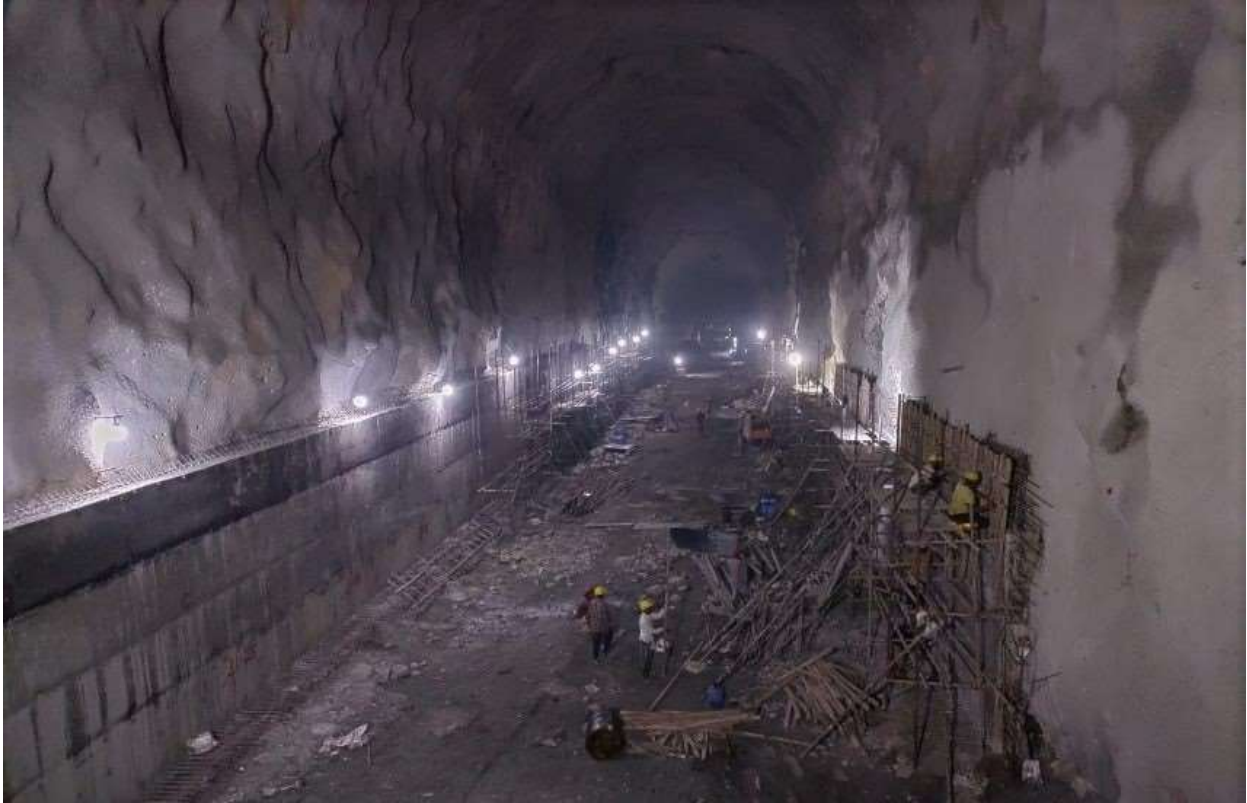
Figure 2-11: A view of concrete lining works being carried out at Settling basin 01
