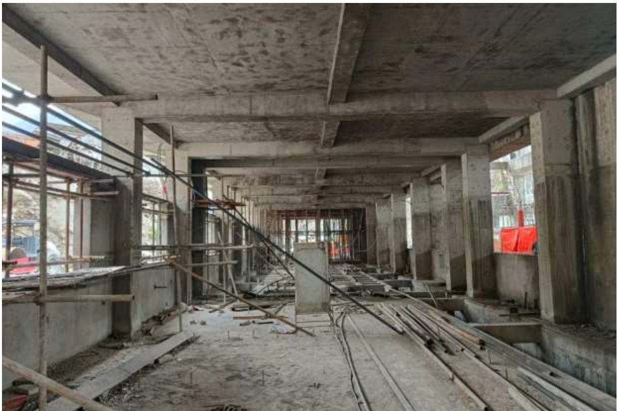
Figure 2-25: A view of auxiliary powerhouse building (control bay)
