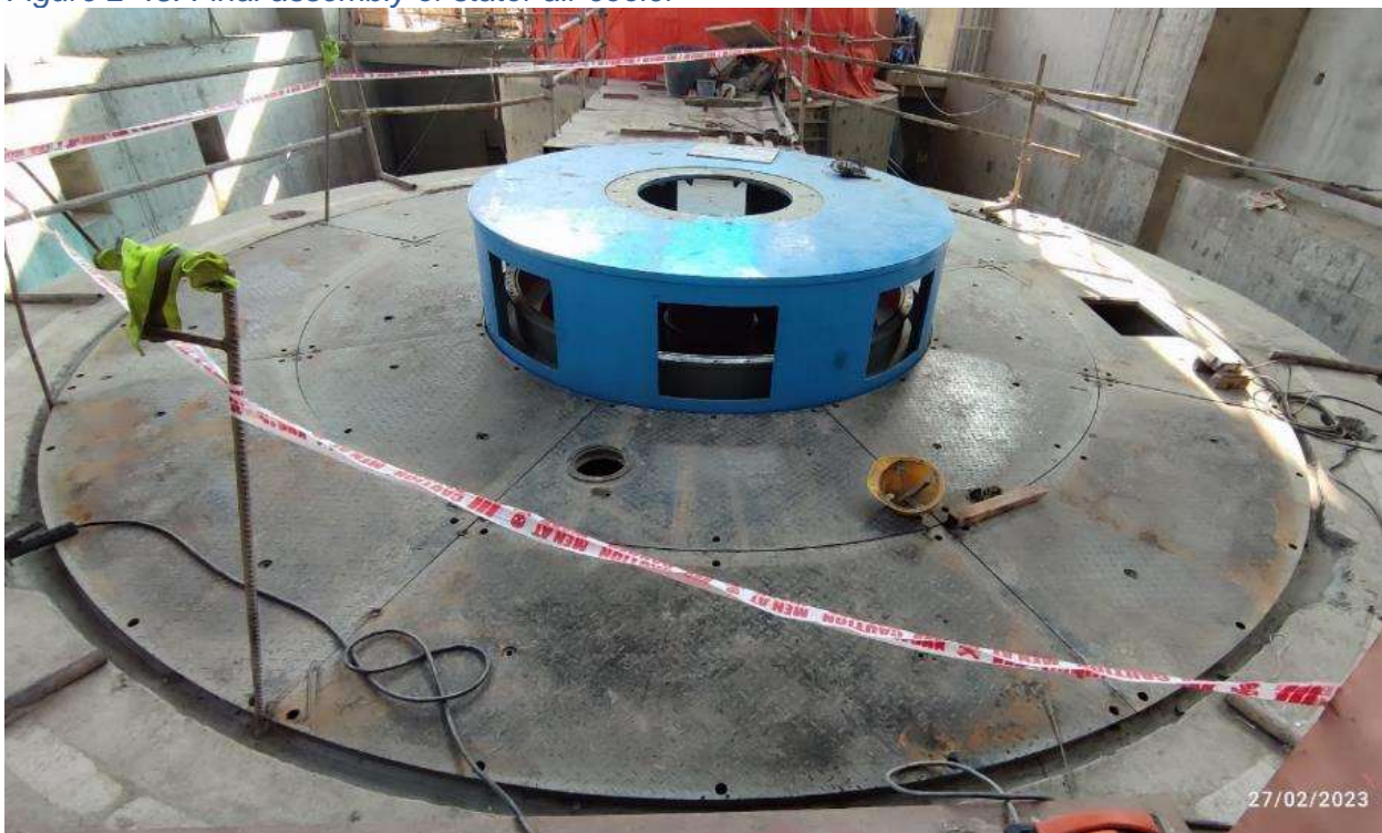
Figure 2-46: Preassembly of generator floor cover plate
