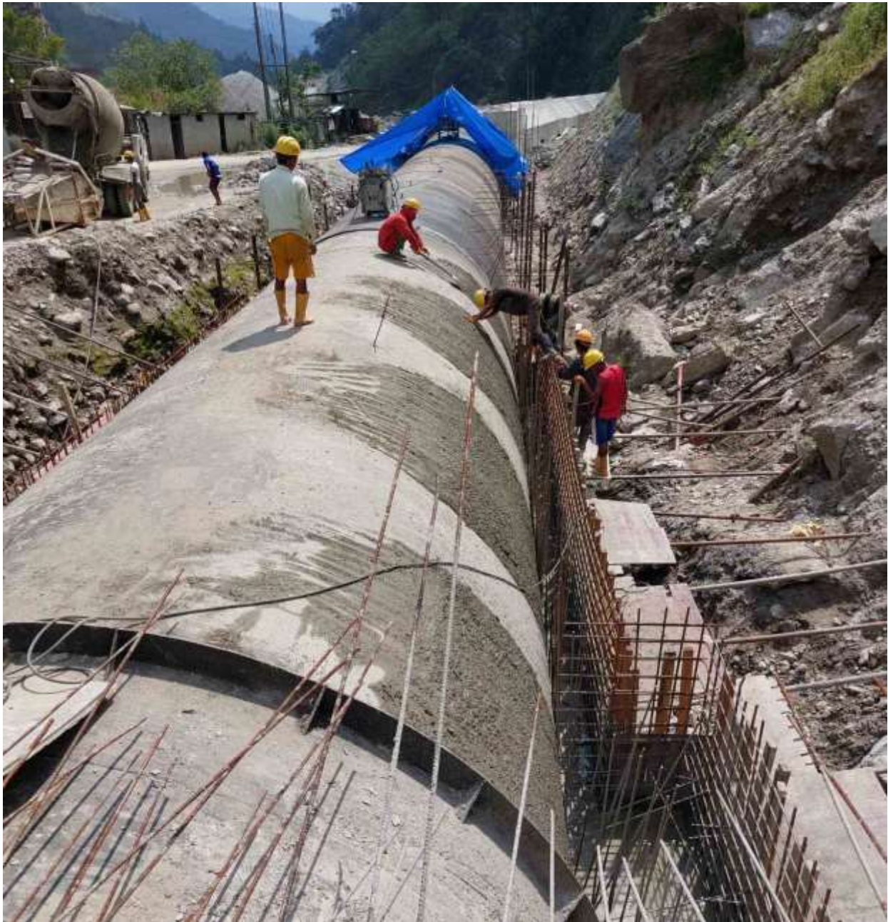
Figure 2-26: Installation of approach pipes at headworks region
