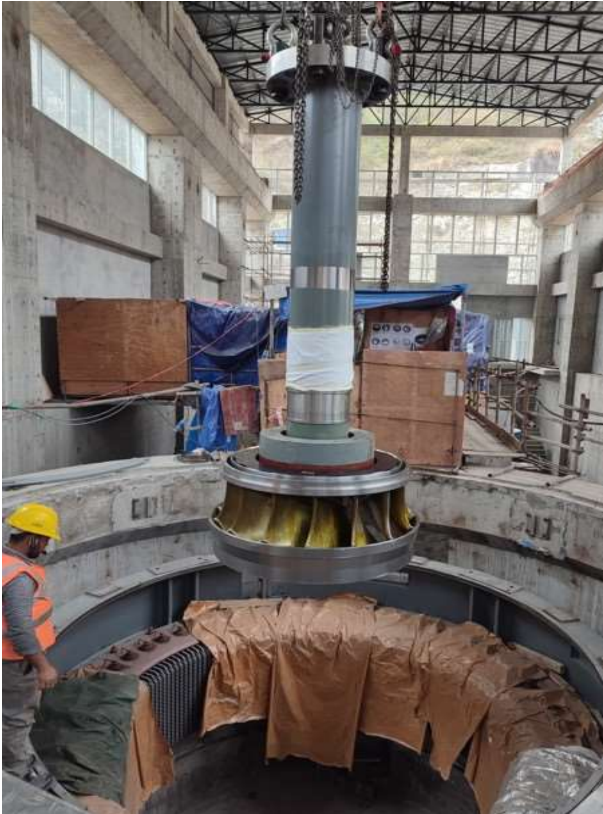
Figure 2-43: Lowering of runner with main shaft in unit 2
