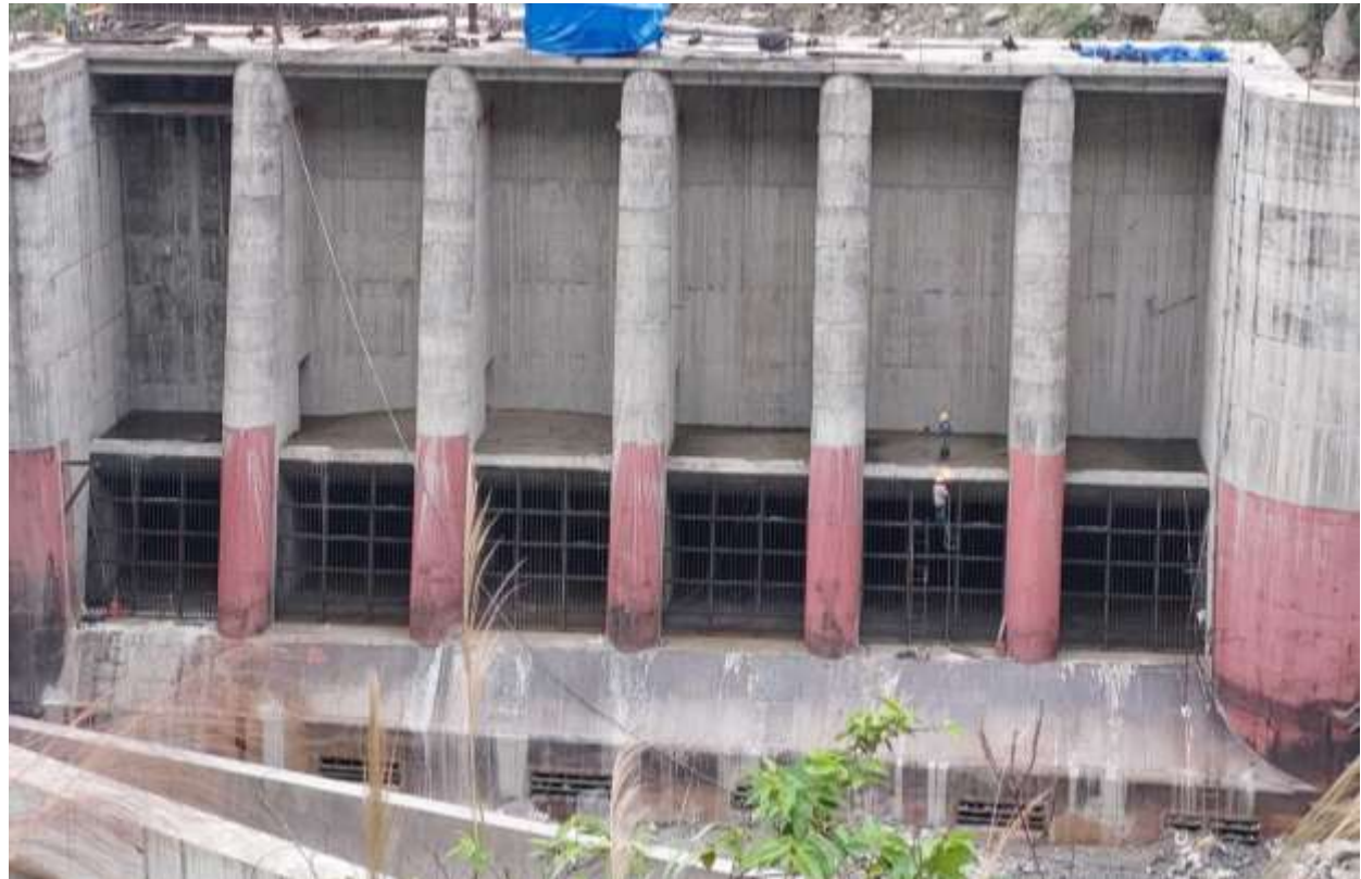
Figure 5: A front view of intake orifices
