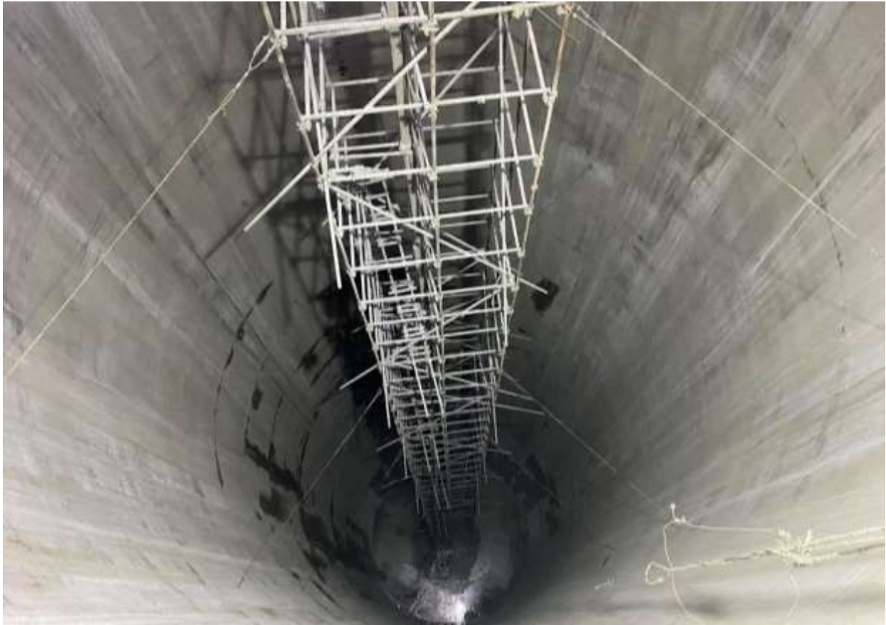
Figure 2-18: A view of surge shaft (Concrete lining completed)
