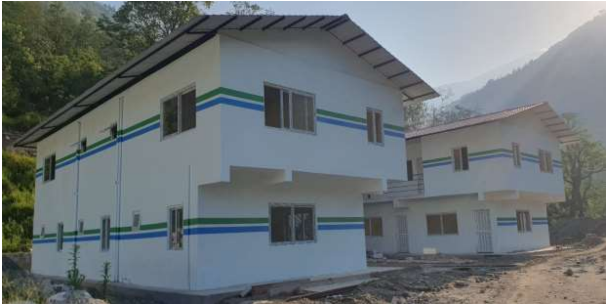
Figure 2: Construction of new camp building at the powerhouse
