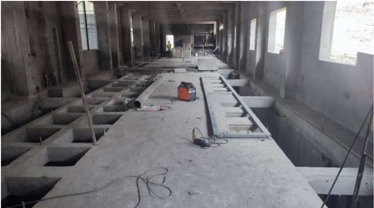
Figure 70: Installation of channels for panel board foundation
