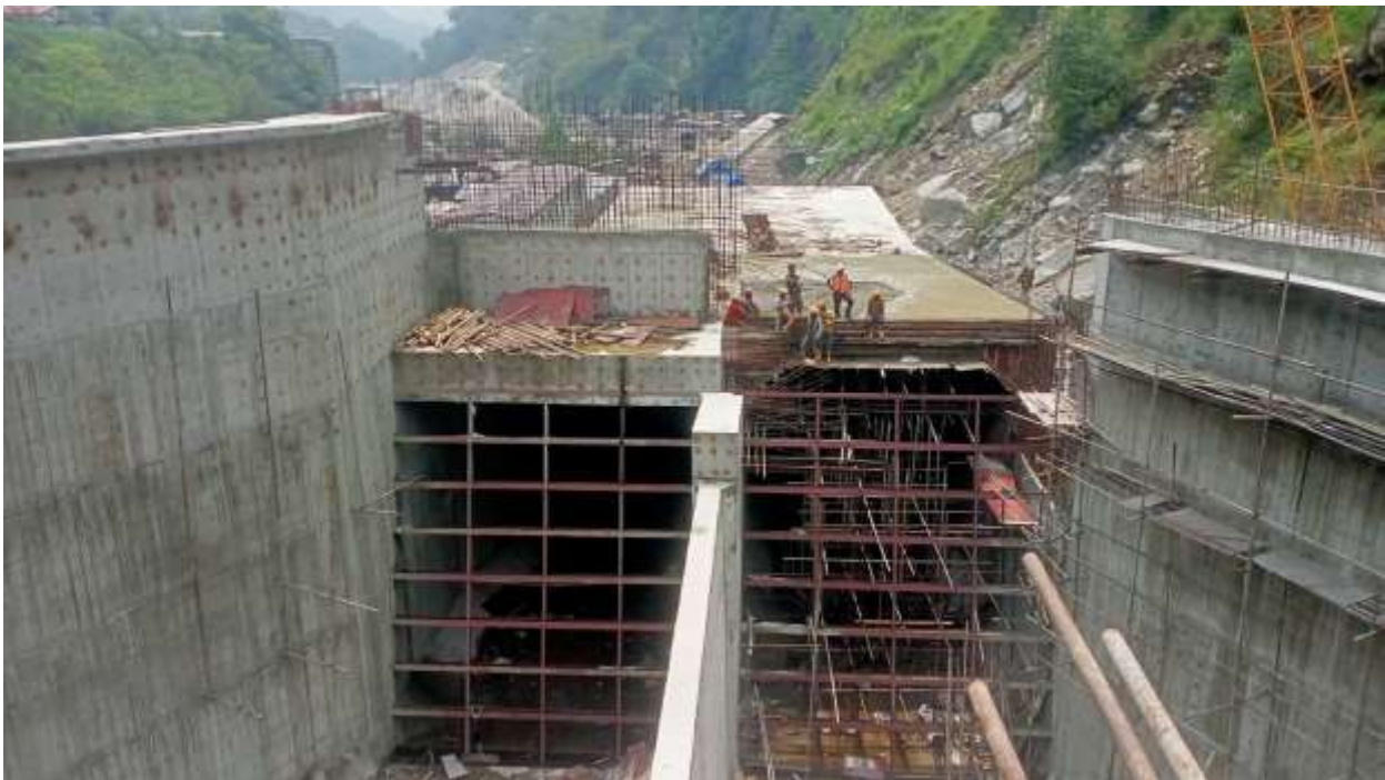
Figure 2-9: Concreting of conveyance tank nearing completion
