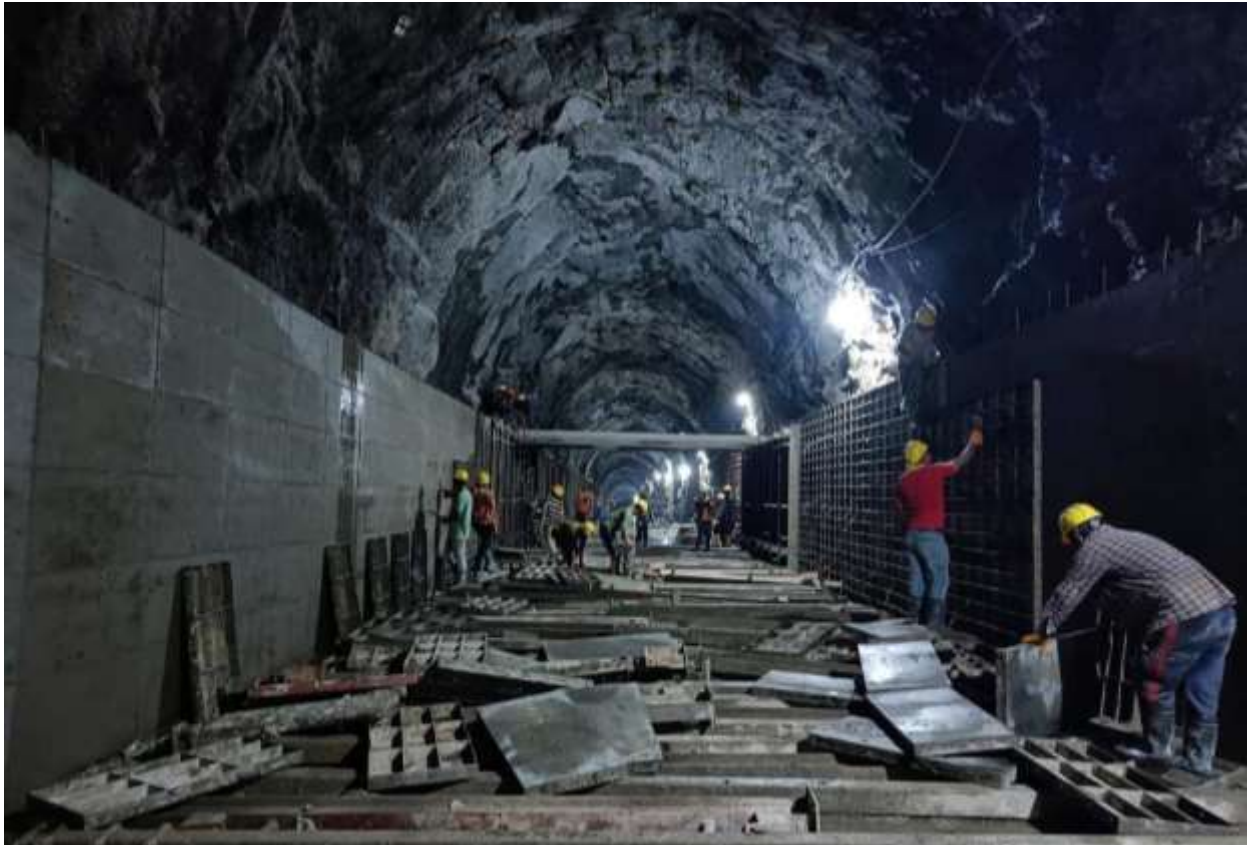
Figure 2-14: A section of HRT with concrete wal lining
