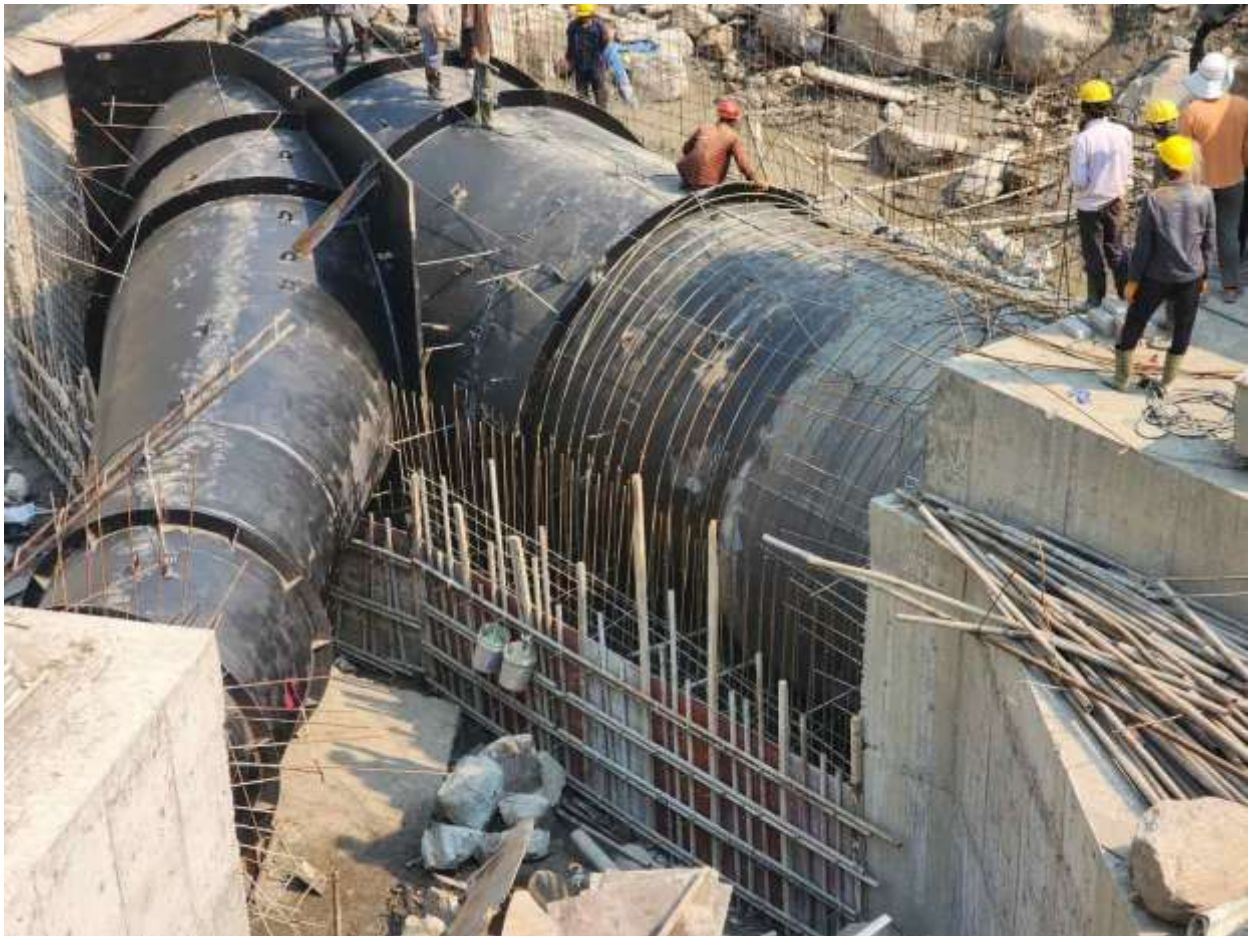
Figure 2-30: Welding work at sickle plate of bifurcation 01
