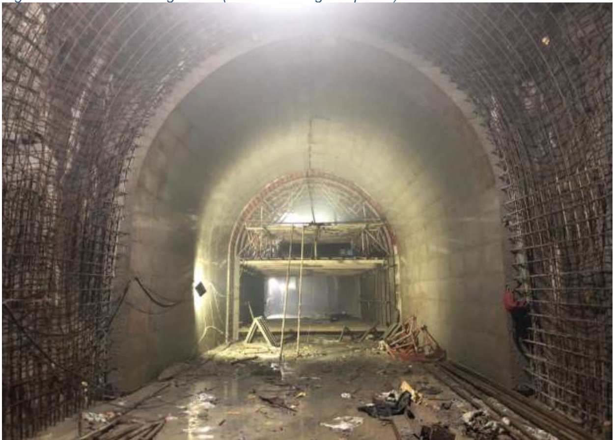
Figure 2-19: Full concrete lining at connecting tunnel to Surge Shaft
