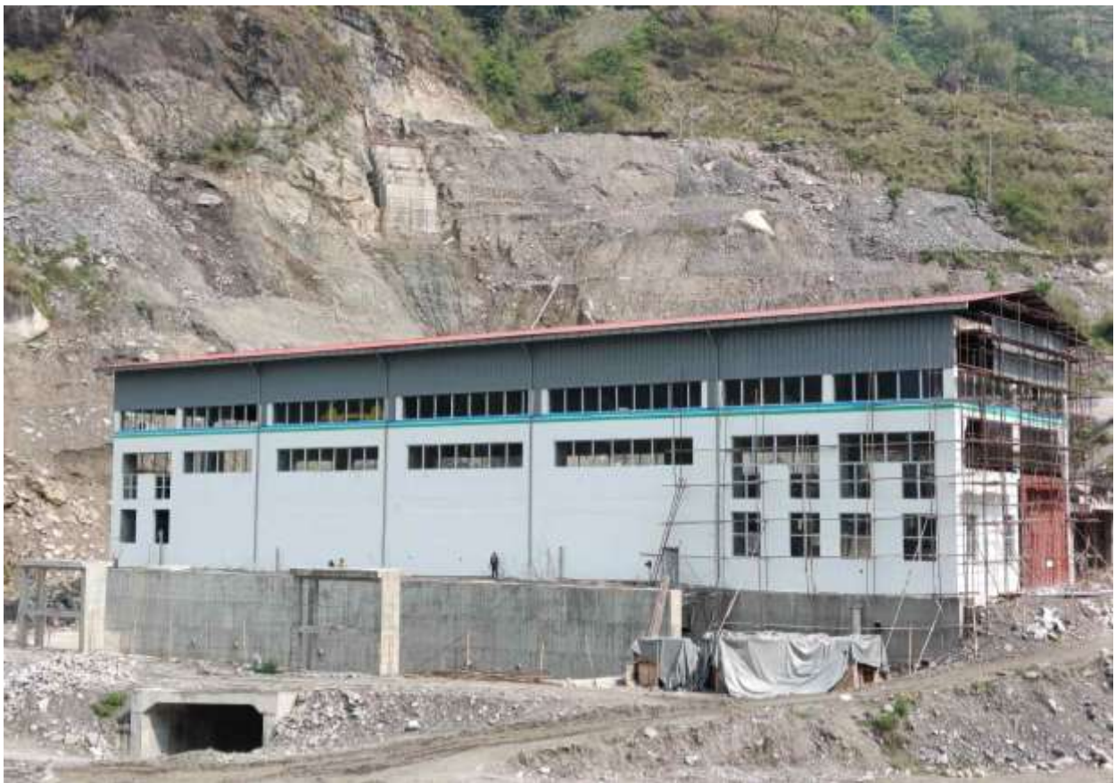
Figure 2-21: A view of Powerhouse from the downstream
