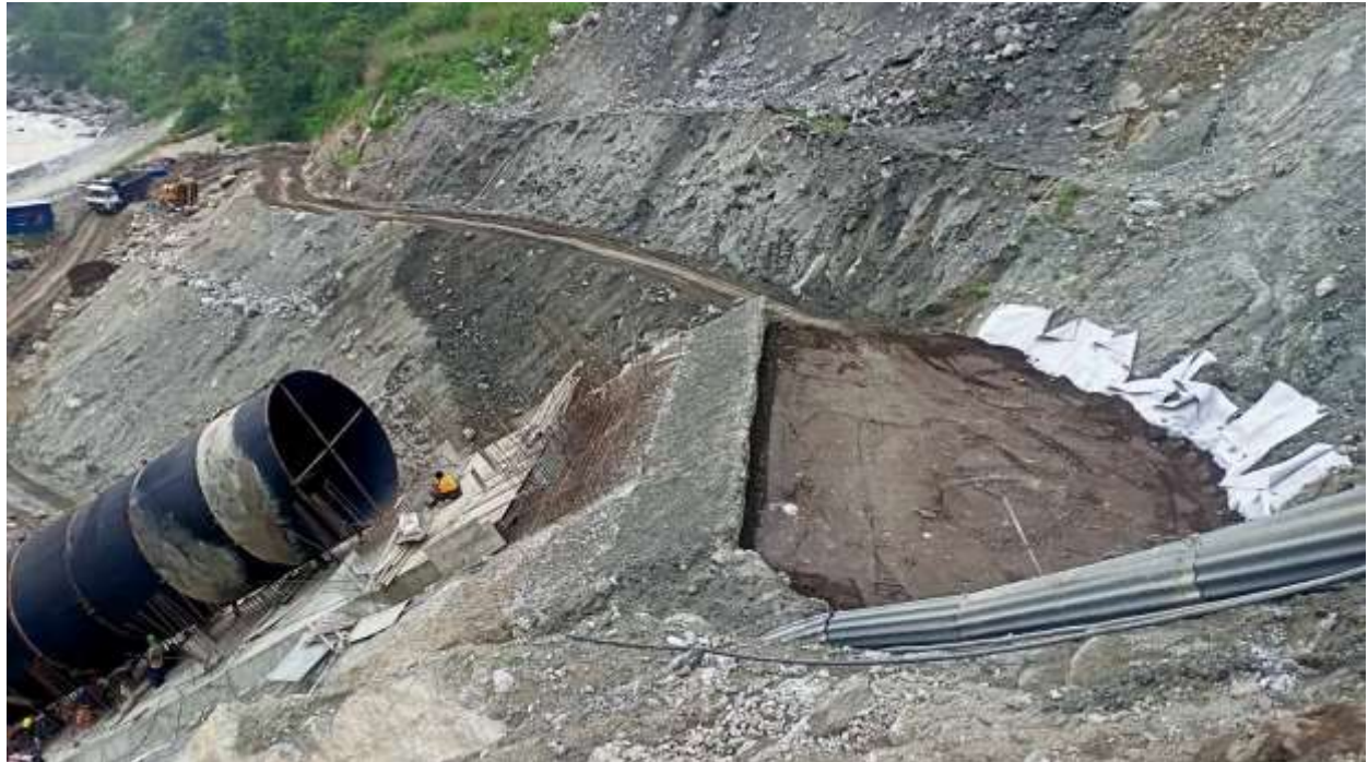
Figure 2-23: Penstock slope stablization works using geogrid (paralink) and macdrain
