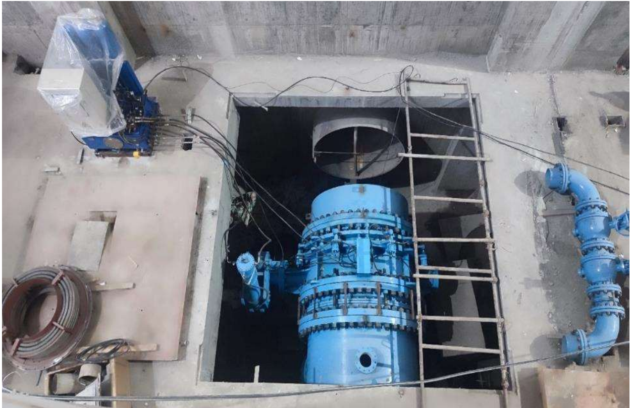
Figure 2-50: Unit 4 MIV lowered to its position
