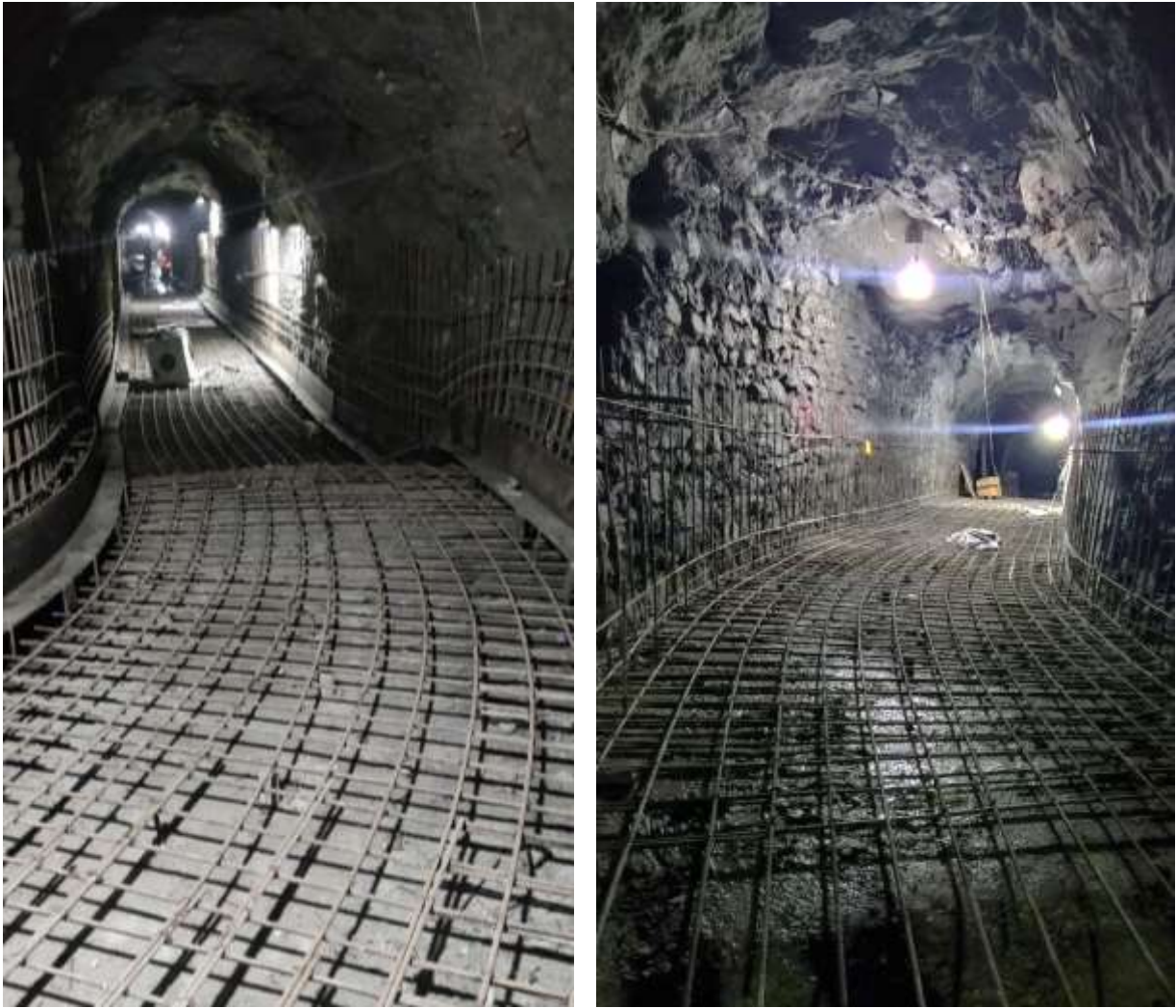
Figure 2-17: A view of rebar layout at the flushing tunnel
