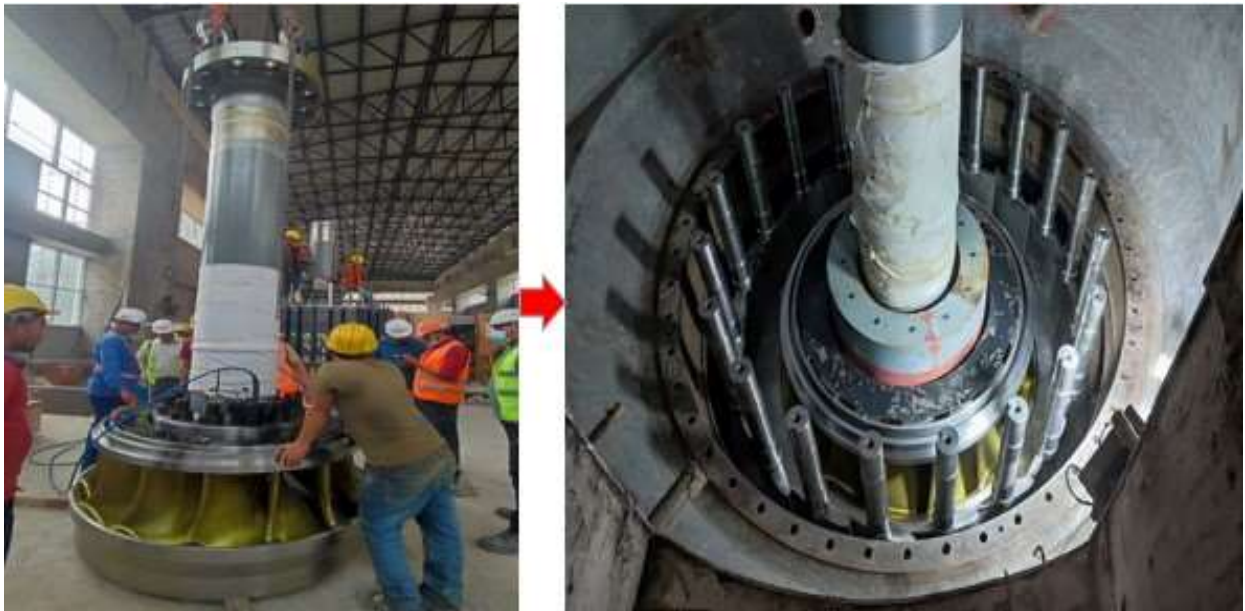
Figure 64: Final assembly of runner with main shaft
