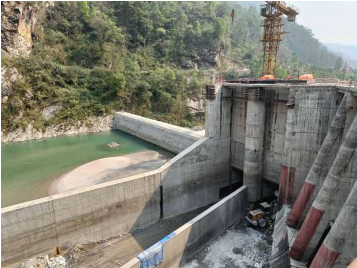
Figure 2-7: A view of weir and undersluice from intake top slab
