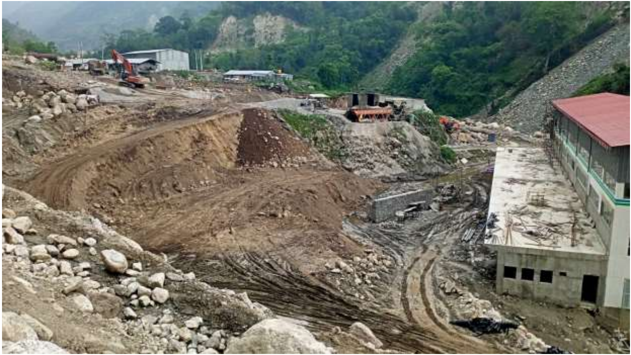
Figure 24: Backfilling of manifold region and excavation of switchyard
