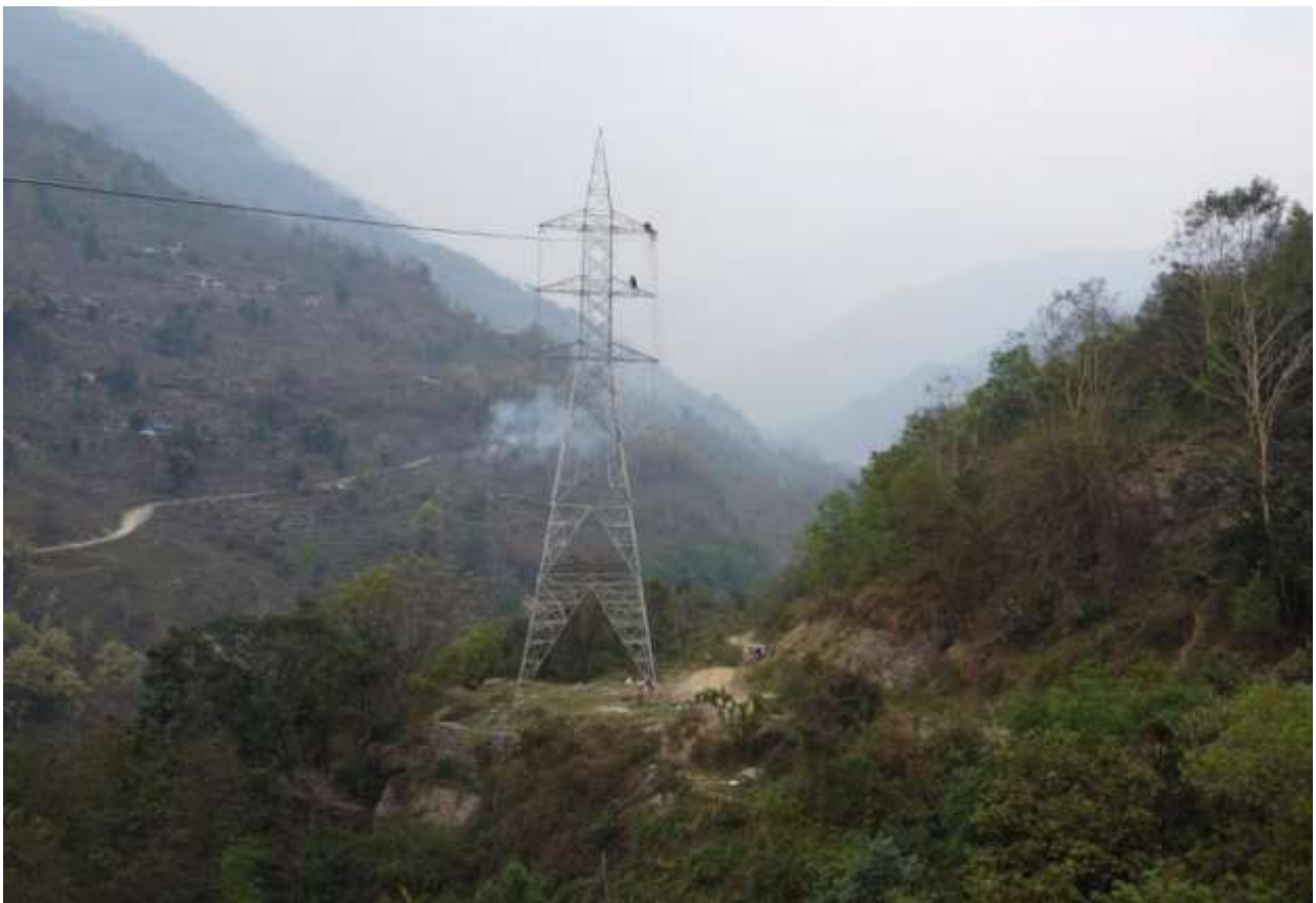
Figure 2-55: A view of stringing works
