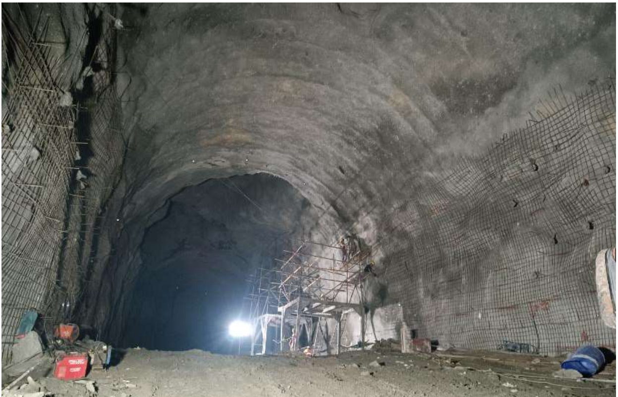
Figure 2-12: Application of wiremesh for shotcrete works
