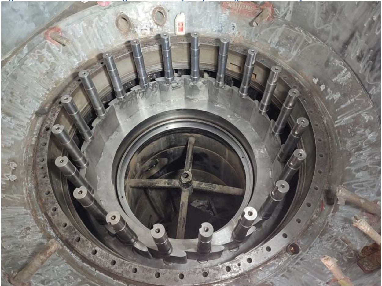
Figure 2-48: Preassembly of bottom ring and guide vane
