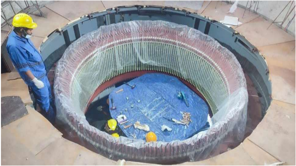
Figure 2-49: Completion of stator winding works
