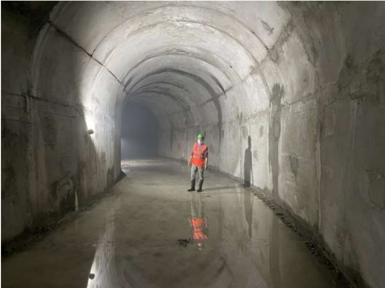
Figure 2-16: A view of full concrete lining works at the connecting tunnel 03
