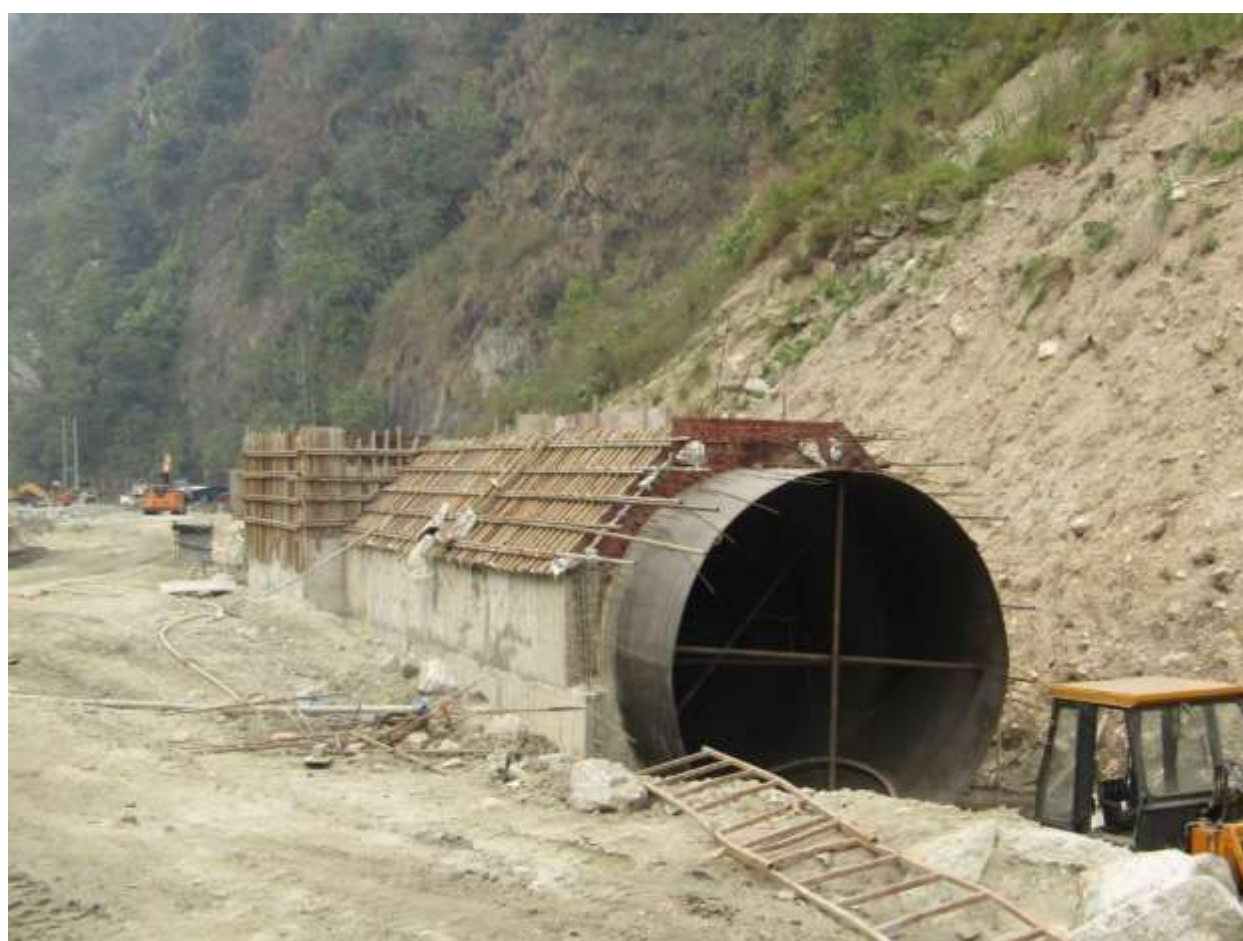
Figure 2-10: Erection of approach pipe
