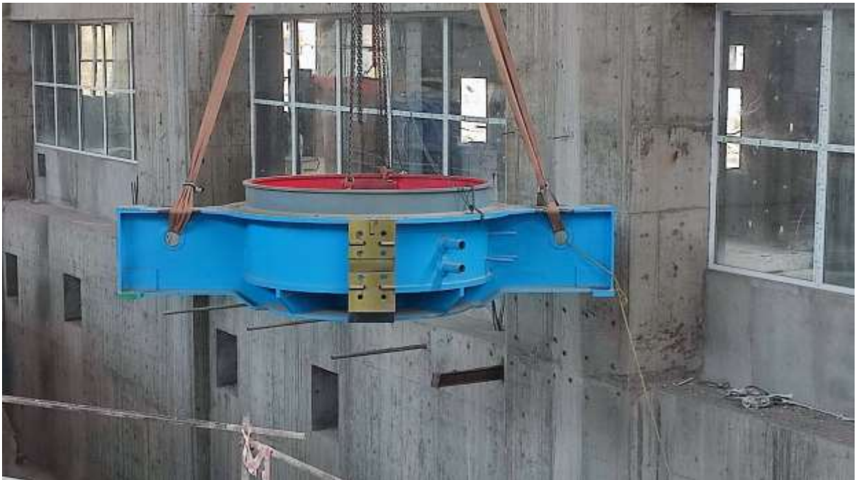
Figure 53: Lowering of upper bracket in unit pit
