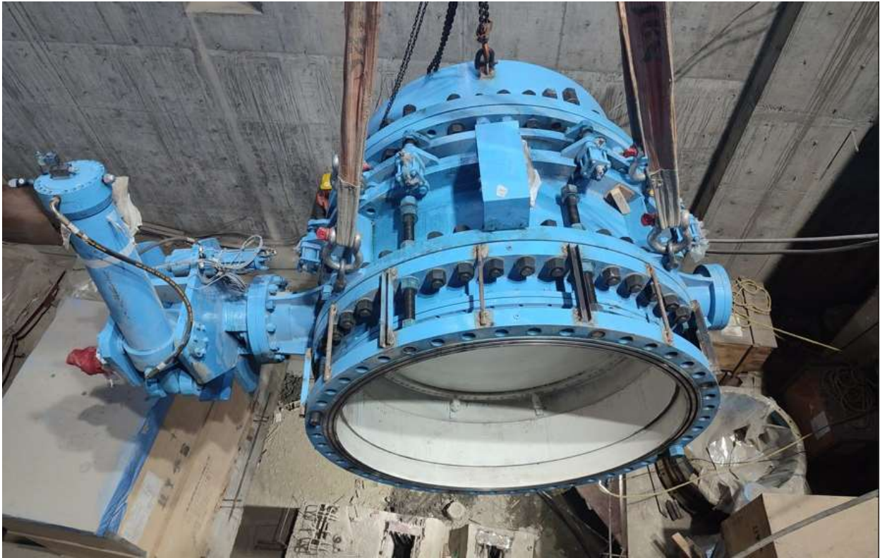
Figure 2-52: Unit 01 MIV lowered in to its position
