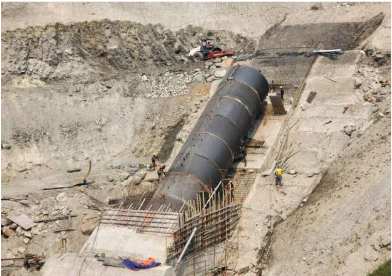
Figure 2-29: Erection of penstock pipe (thickness 30 mm and 28 mm)
