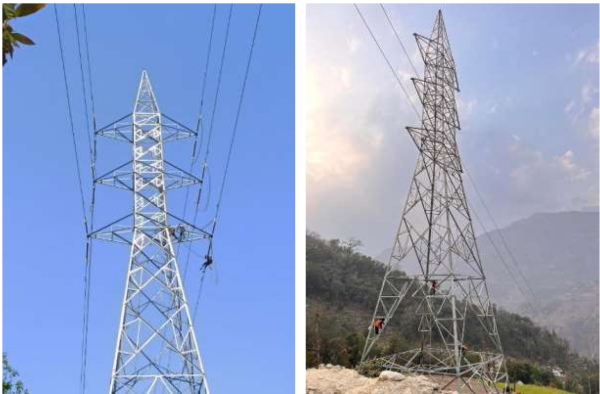
Figure 2-56: Conductor stringing works at various angle points
