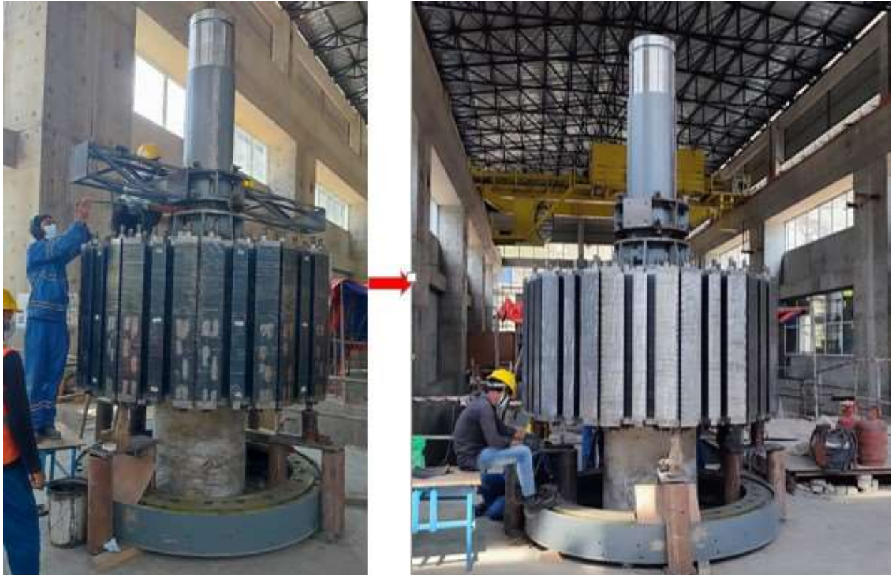
Figure 61: Roundness checking of rotor after yoke punching sheet assembly
