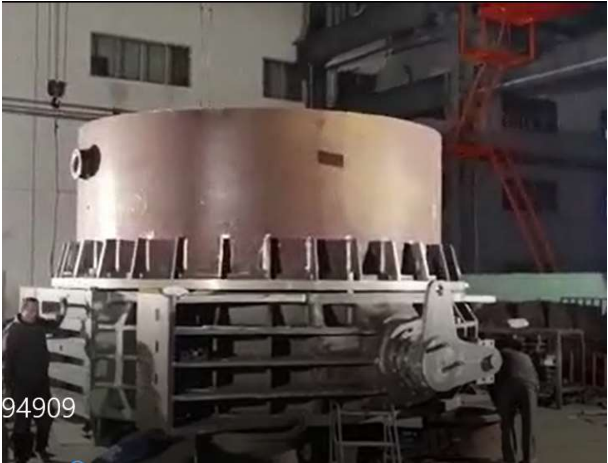
Figure 2-37: PPV being factory preassembled
