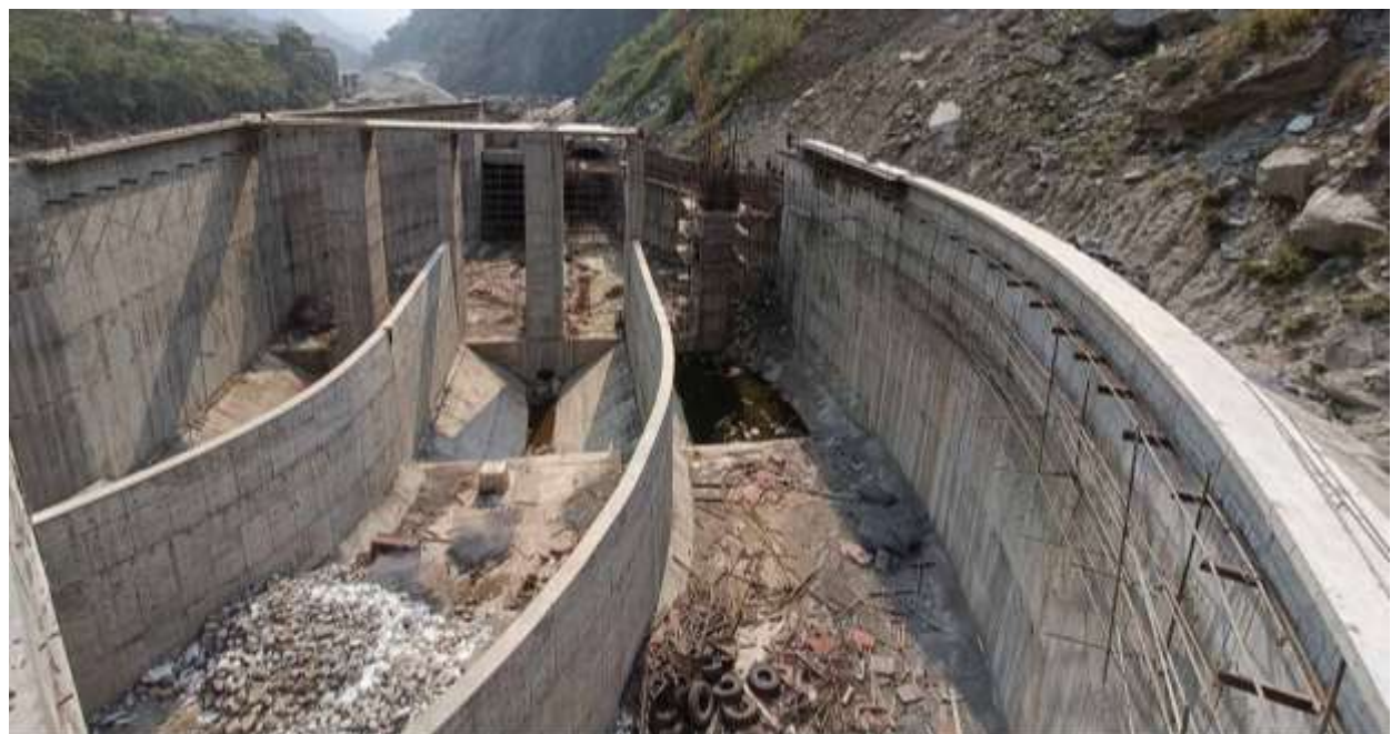
Figure 2-6: Concreting at the hillside wall of intake completed
