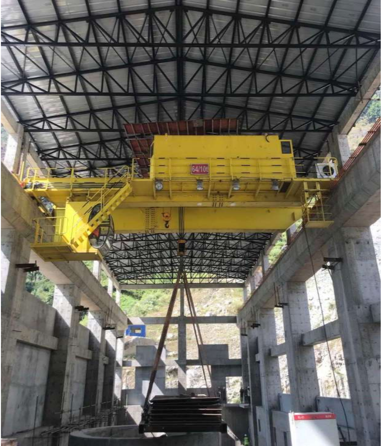
Figure 2-41: Load test of EOT lifting 66 ton and travelling across unit 2
