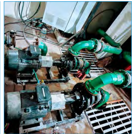
Sump Pit मा Additional Drainage System निर्माण कार्य
