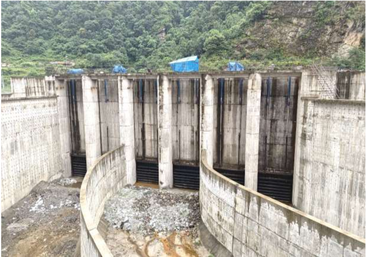
Figure 2-4: A view of intake from downstream and intake canal
