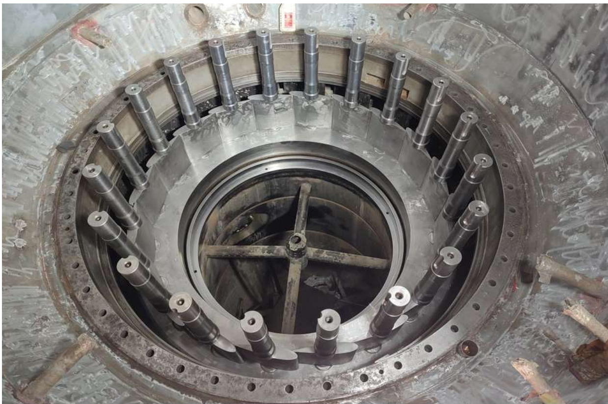
Figure 2-56: Final assembly of bottom ring and guide vane
