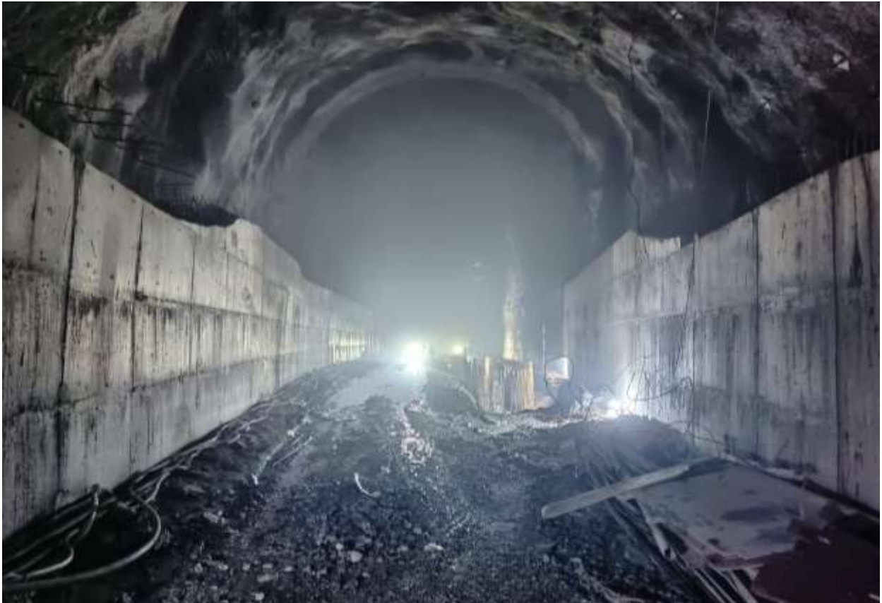
Figure 2-13: Concreting works at the right hopper of settling basin bay 02
