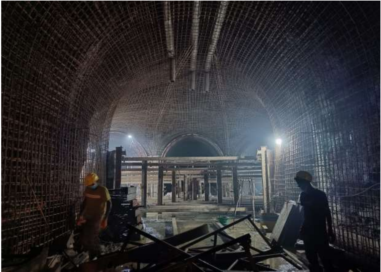
Figure 2-17: Preparation for full lining at the connecting tunnel junction
