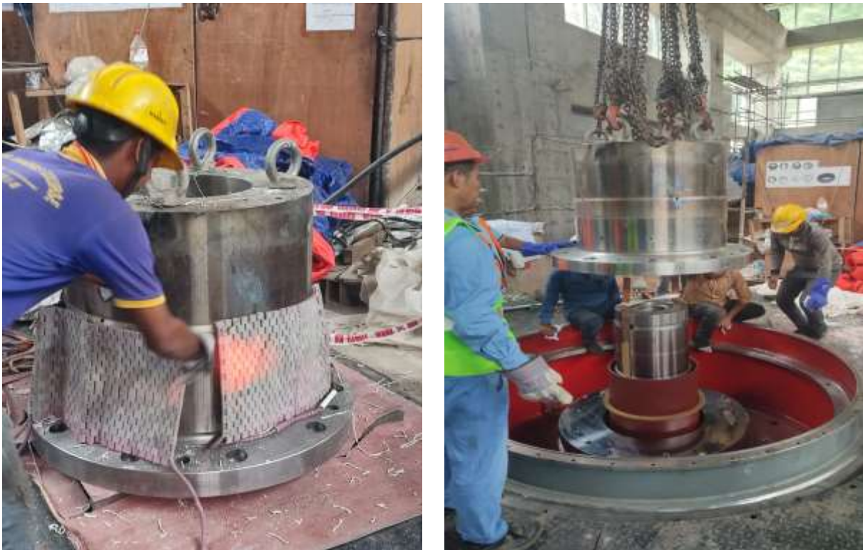
Figure 2-58: Different stages of thrust bearing installation
