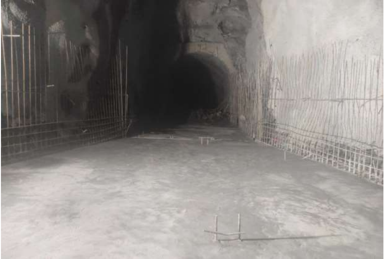
Figure 2-16: Final stage of outlet gate section invert concrete at SB 03
