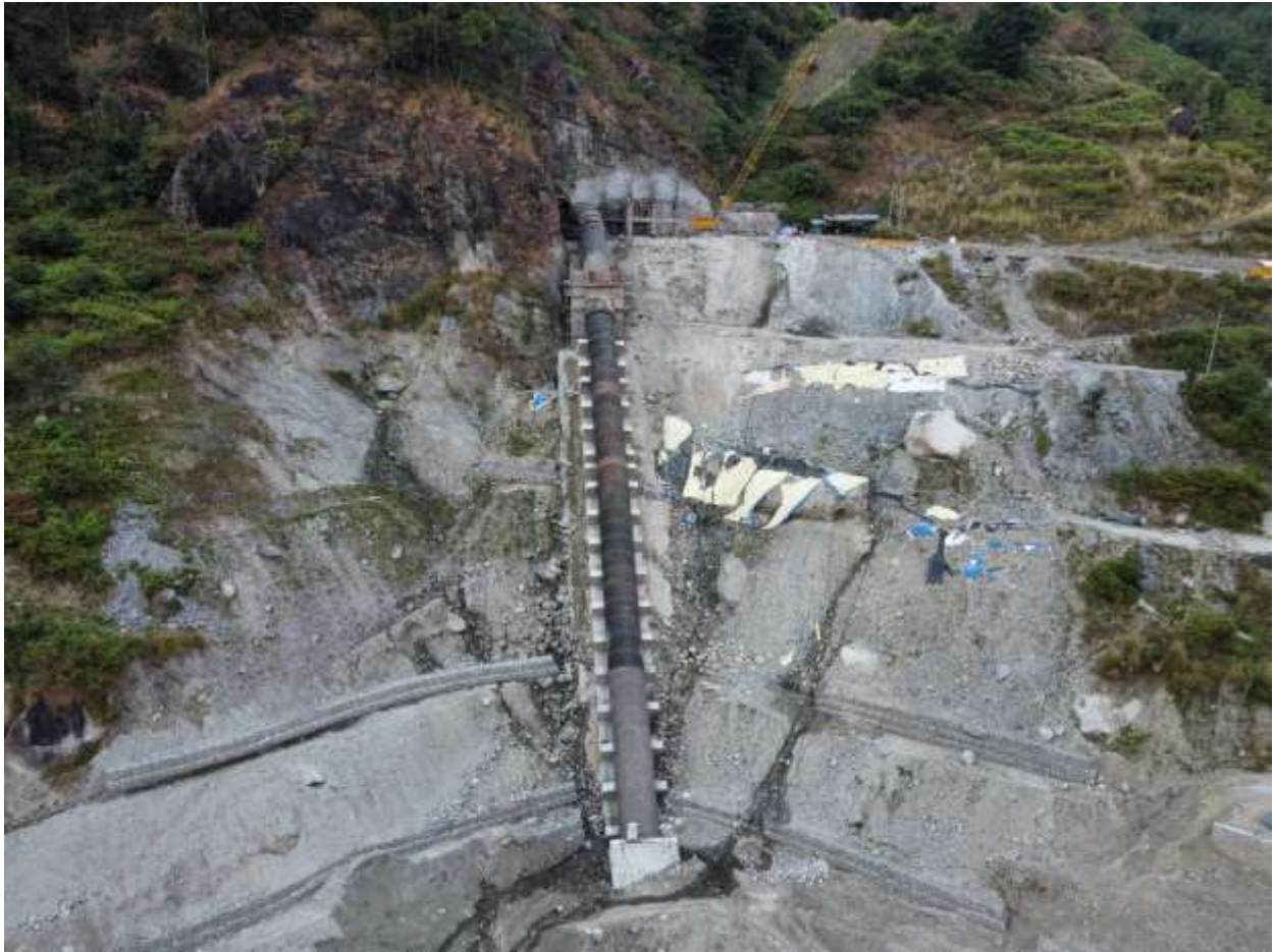
Figure 2-39: Erection of penstock pipes
