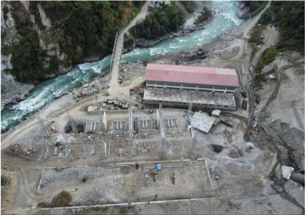
Figure 2-29: Aerial view of powerhouse and switchyard region
