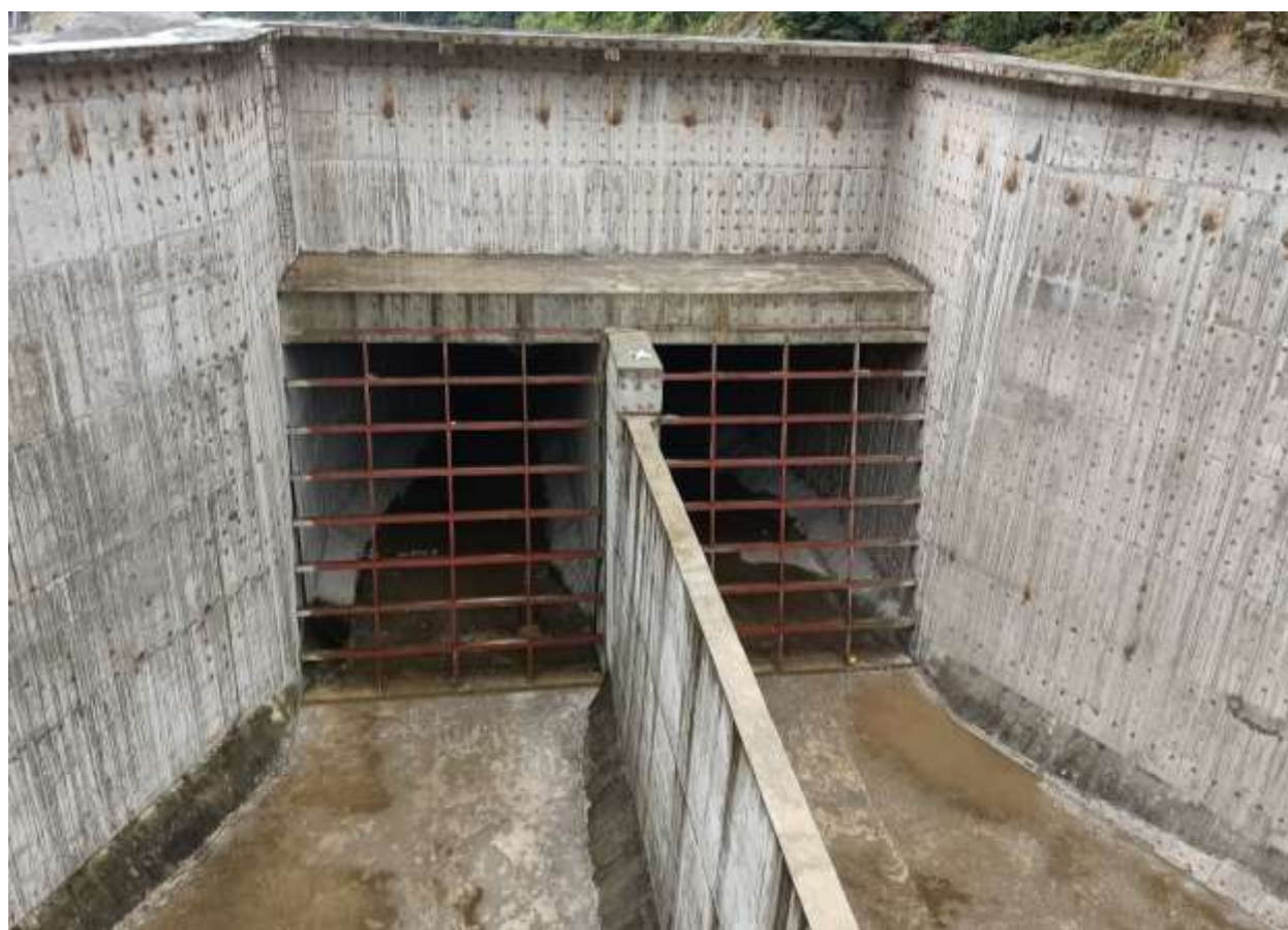
Figure 2-37: Installation of trash rack at the conveyance tank region
