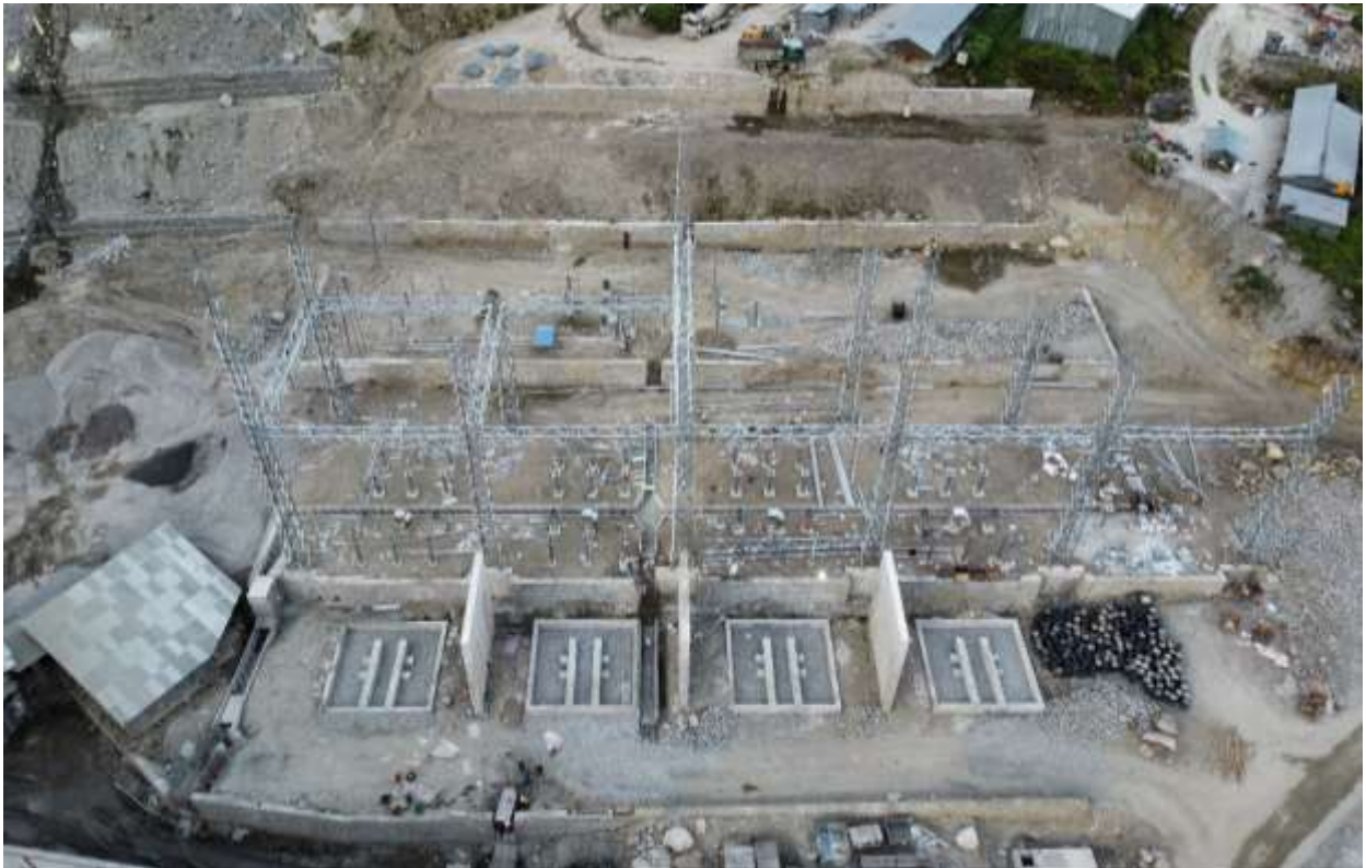
Figure 2-74: Erection of gantry towers at switchyard
