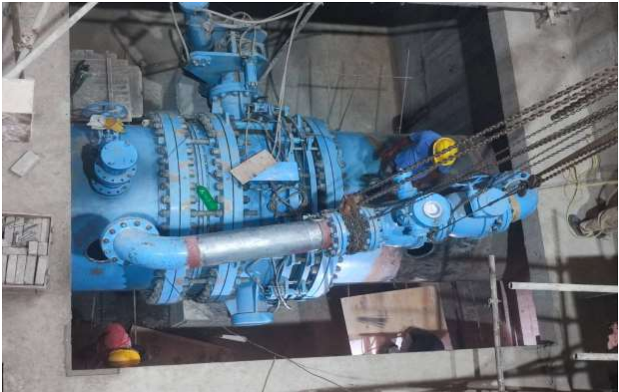
Figure 2-66: Unit 02 bypass valve assembly and erection
