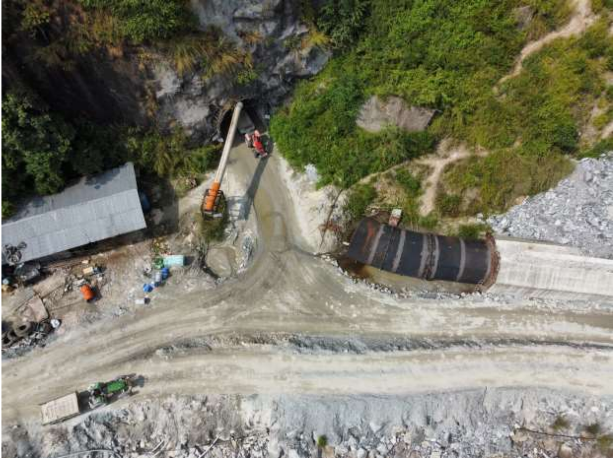
Figure 2-38: Installation of head race bend at the approach pipe section
