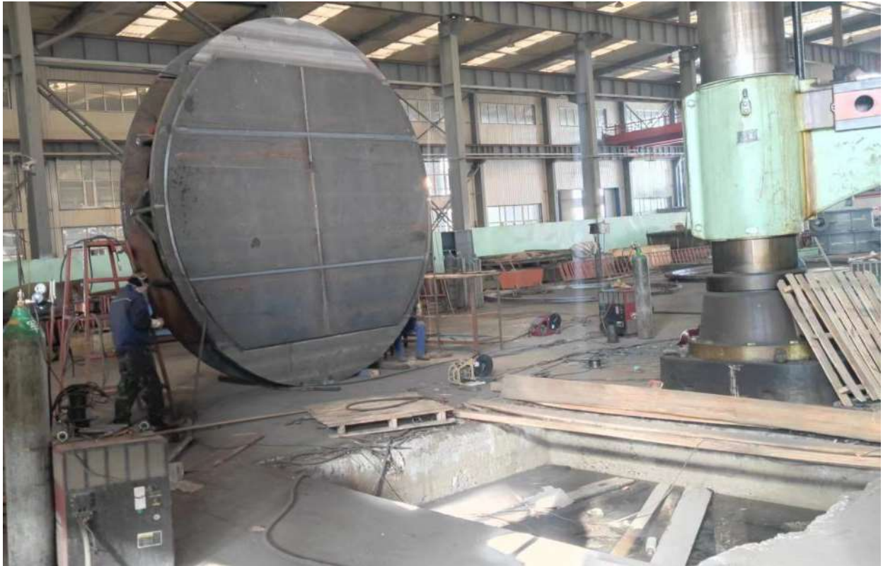
Figure 2-48: PPV disc being welded
