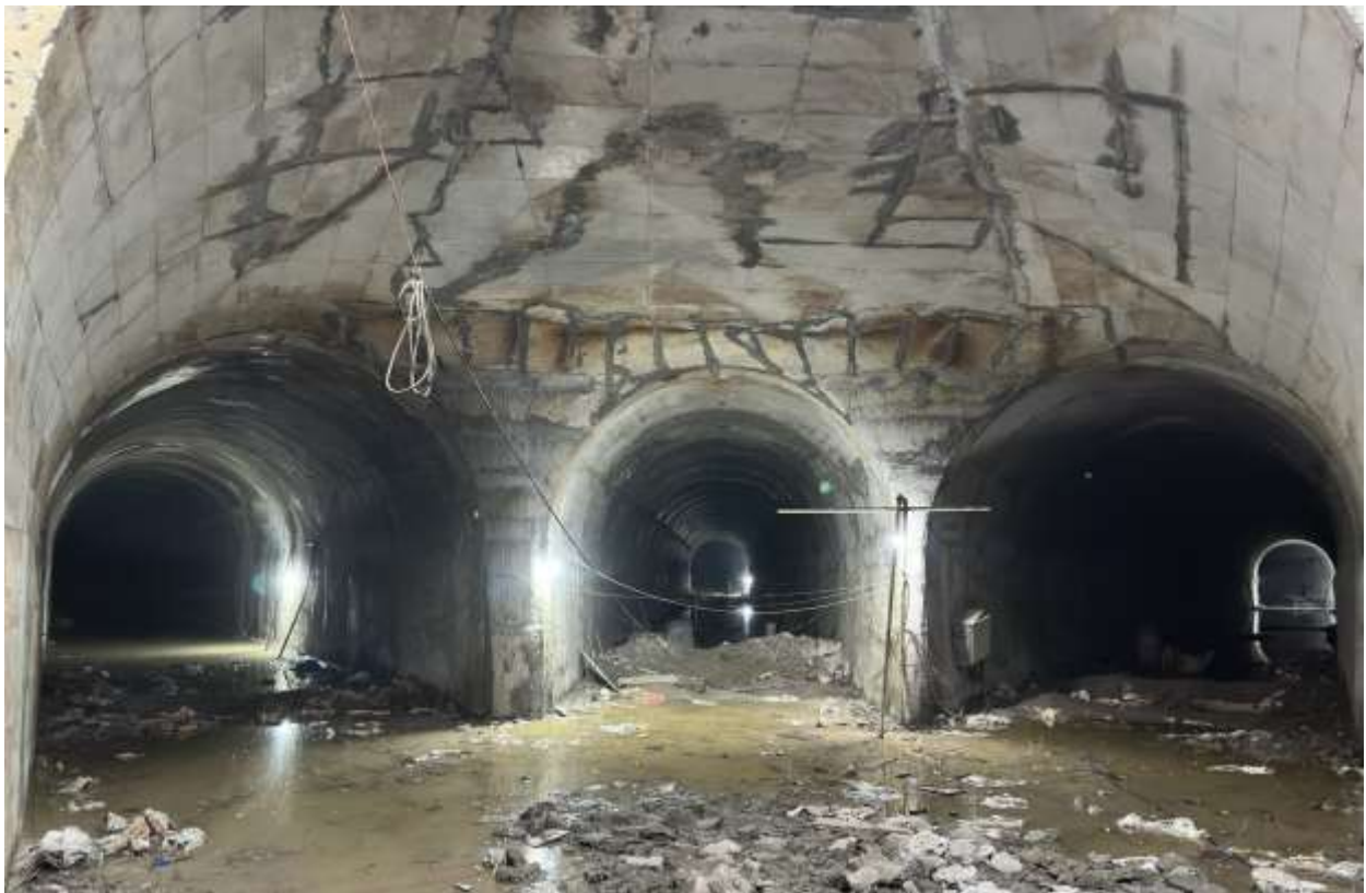
Figure 2-18: Full lining concrete at connecting tunnel junction
