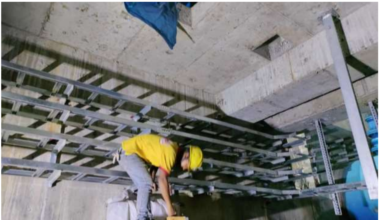
Figure 2-72: Cable tray work under the floor slab of turbine floor
