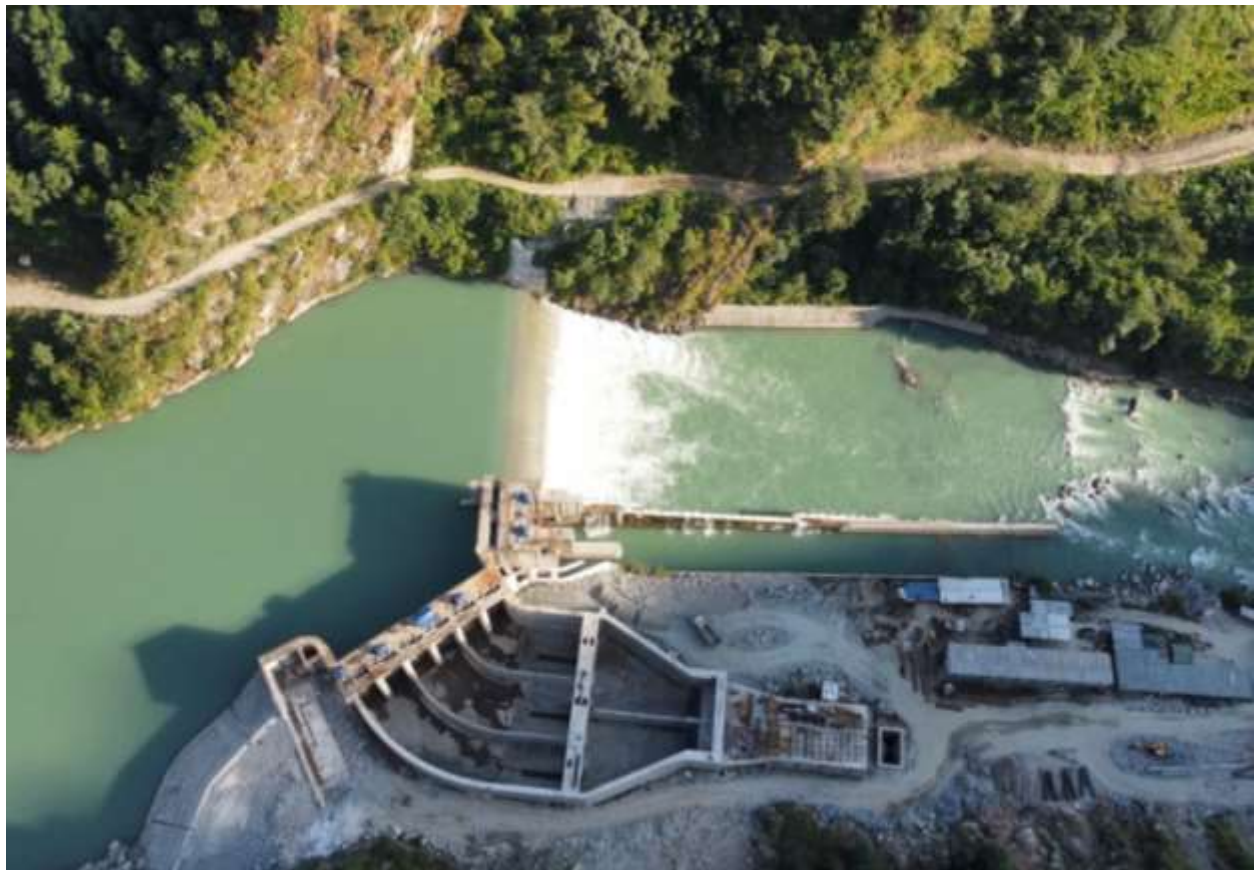
Figure 2-6: An aerial view of weir during monsoon water flow over the ogee crest
