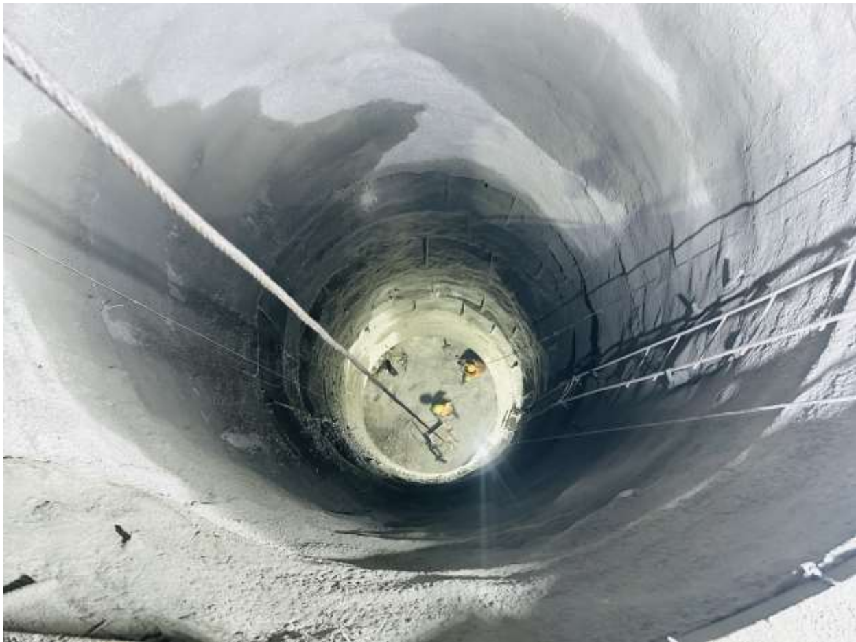
Figure 2-26: Excavation of flushing tunnel 03 in progress
