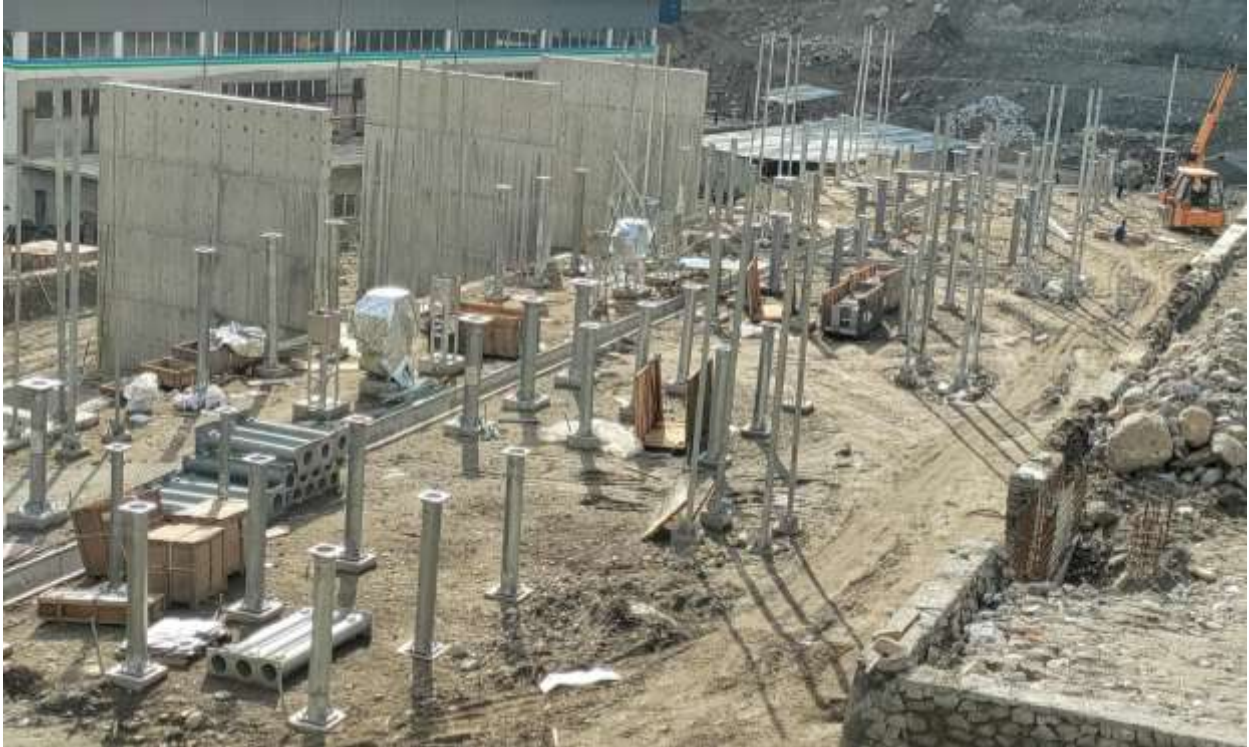
Figure 2-73: Erection of gantry tower and other supporting posts
