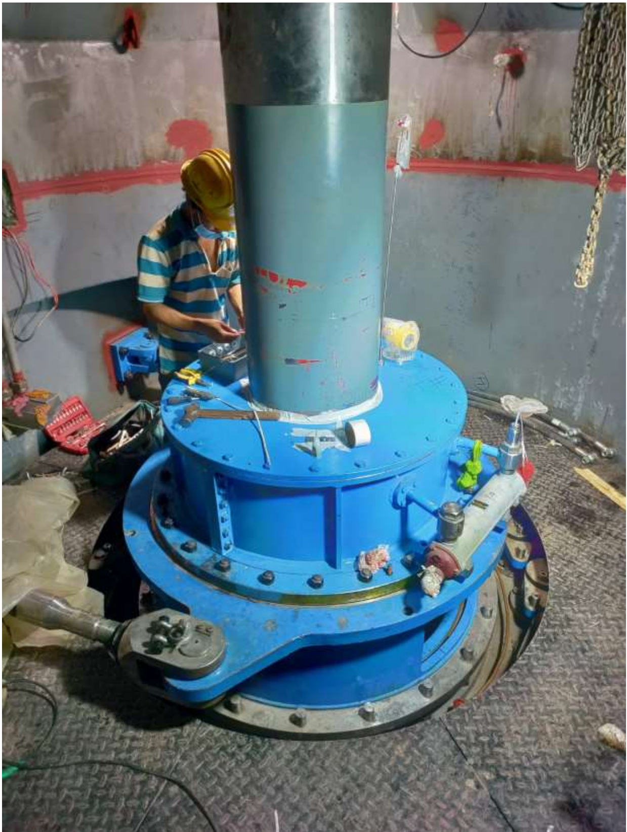
Figure 2-59: Final installation of turbine guide bearing and water regulating mechanism
