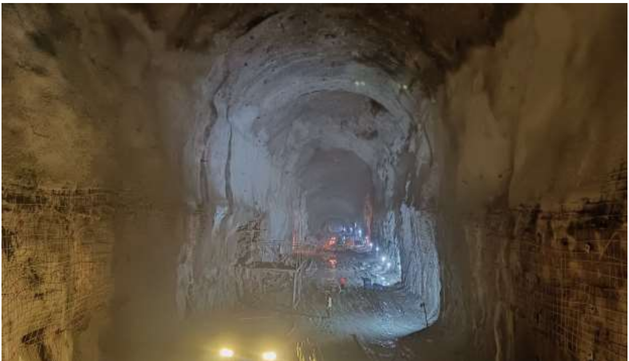
Figure 2-15: A view of SB 03 during installation of final lining wiremesh shotcrete
