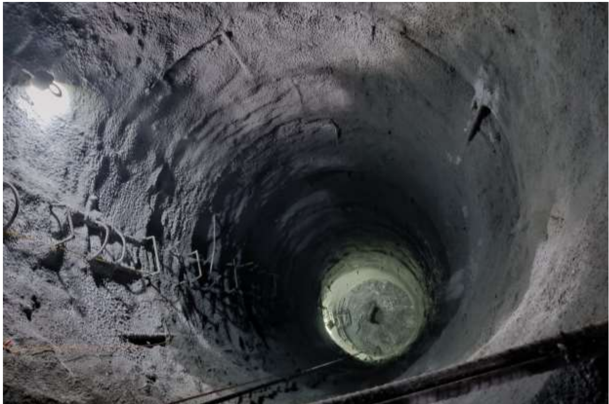
Figure 2-25: Breakthrough of flushing tunnel 04
