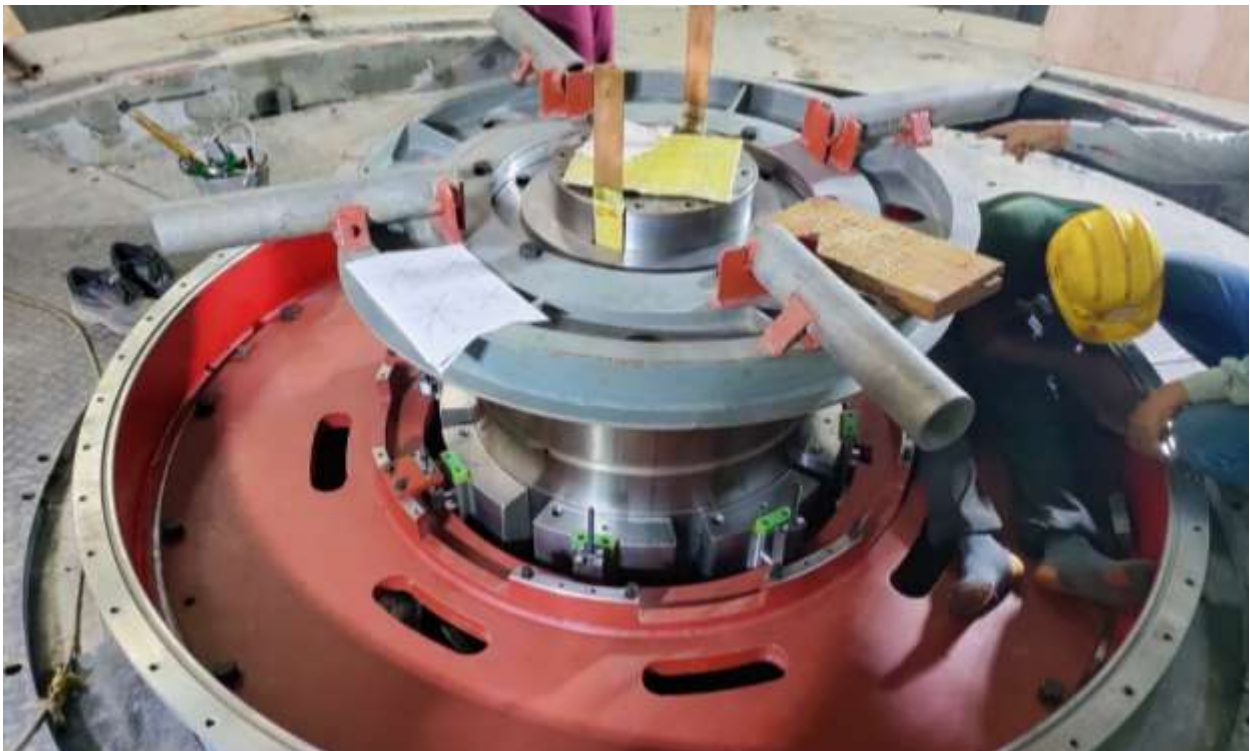
Figure 2-63: Run-out check of shaft
