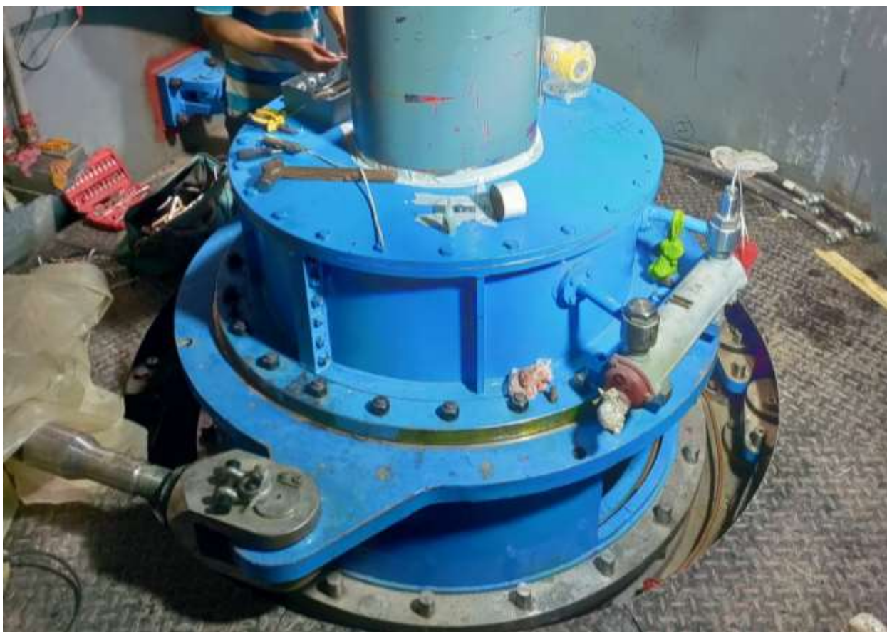
Figure 2-53: Final installation of water guide mechanism along with monitoring sensors
