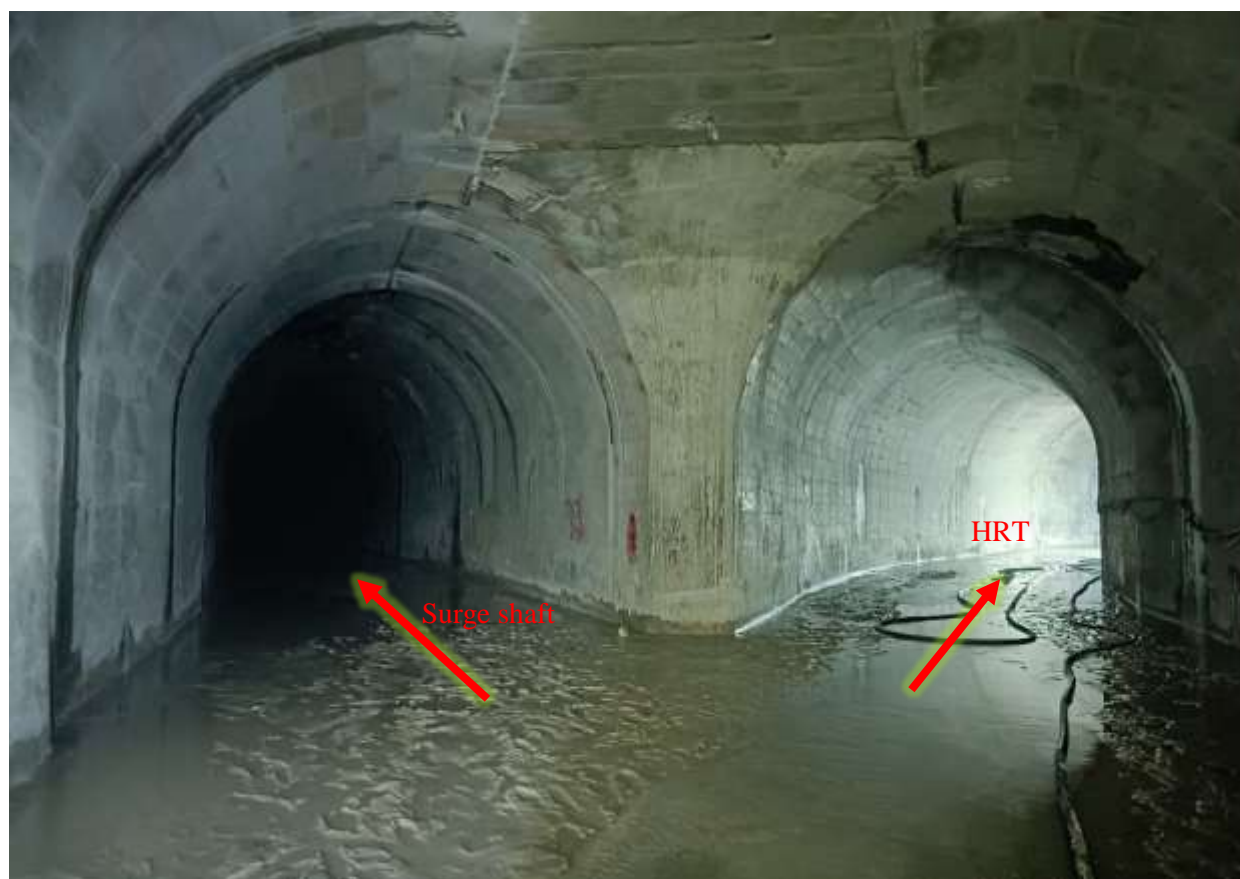
Figure 2-28: Full concrete lining at the junction of connecting tunnel and HRT
