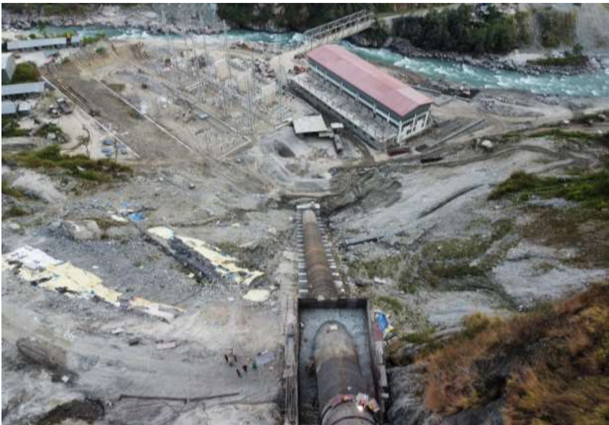
Figure 2-32: A view of penstock alignment, switchyard and powerhouse
