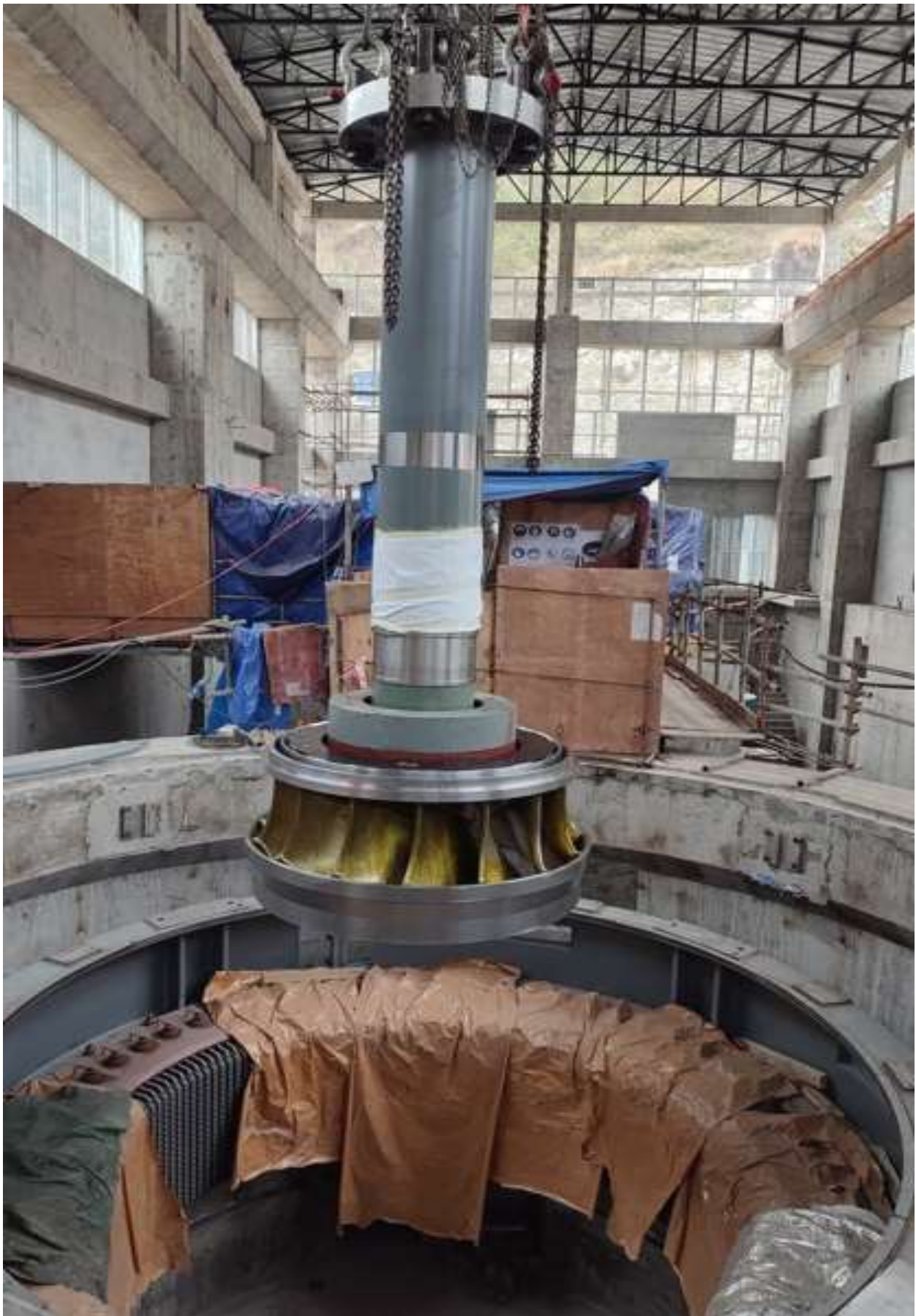
Figure 2-55: Final assembly and lowering of runner with main shaft in unit 2
