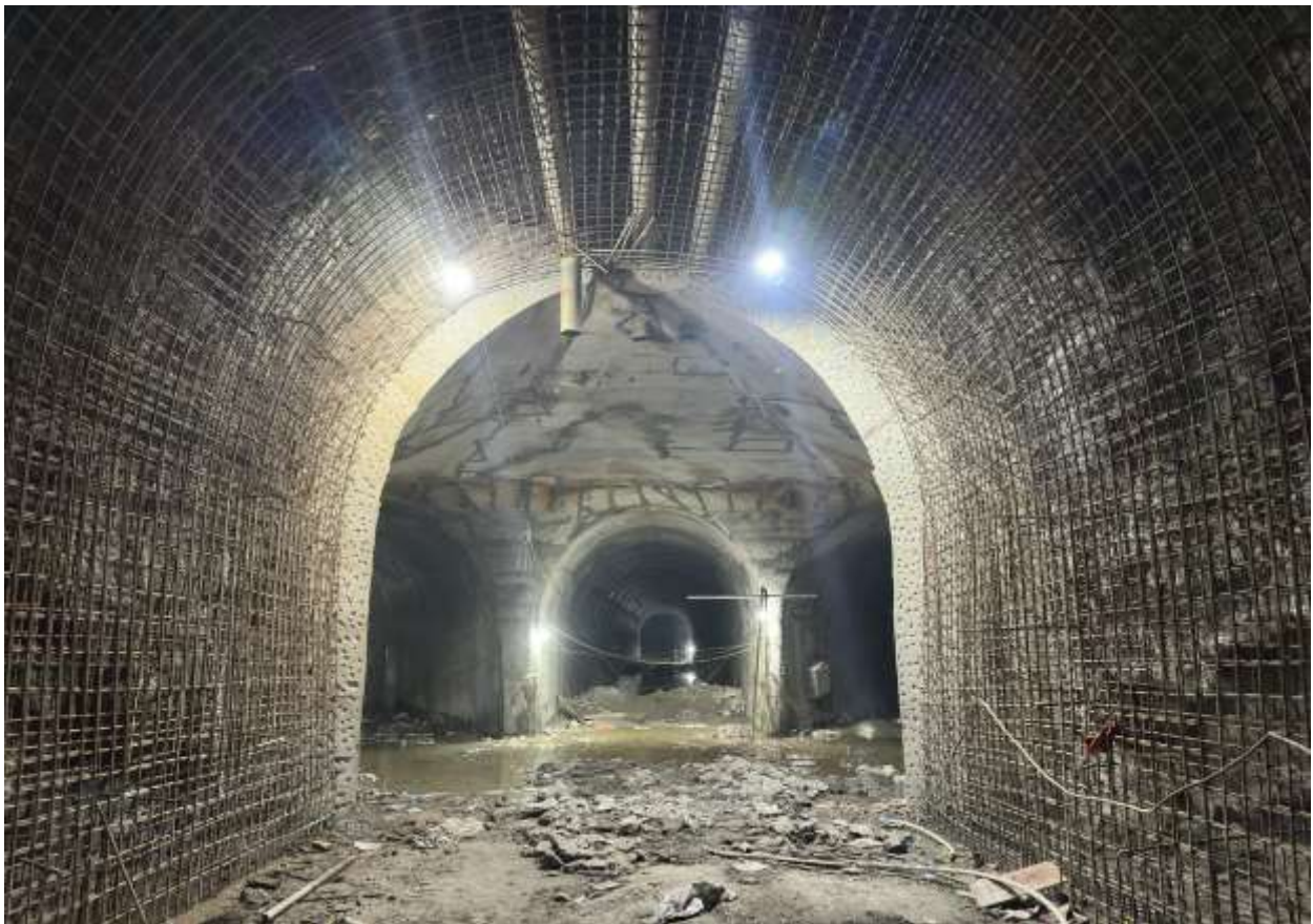
Figure 2-20: Rebar installation at the HRT region
