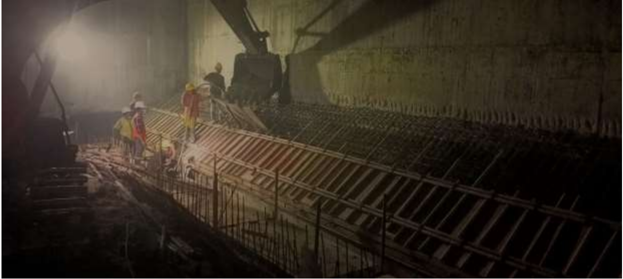
Figure 2-12: Concreting at hopper of SB 02
