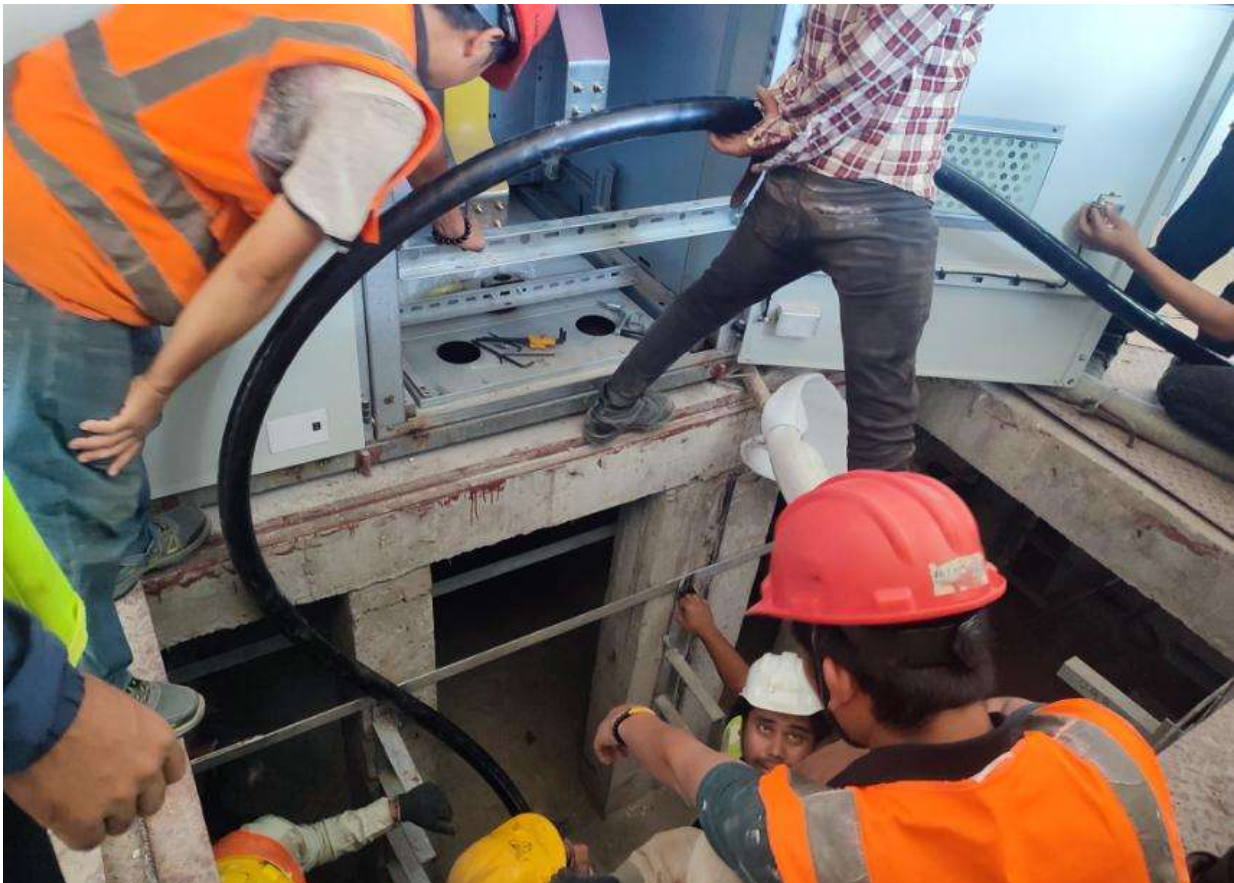
Figure 2-70: Laying of power cables in 11KV switch gear room
