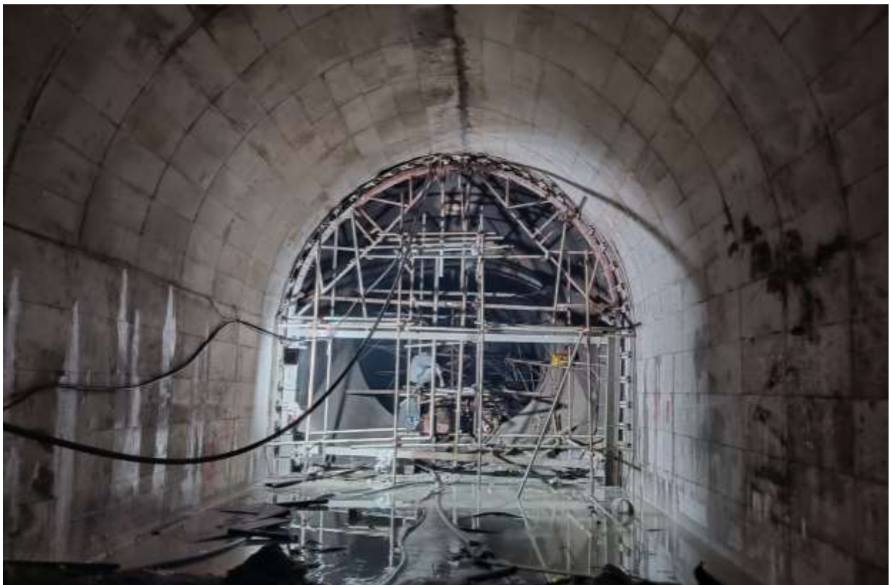
Figure 2-42: Installation of transition pipe at the plug block 01 region
