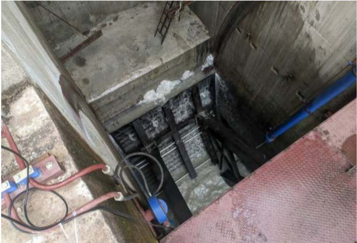
Figure 2-43: Erection of radial gate at undersluice
