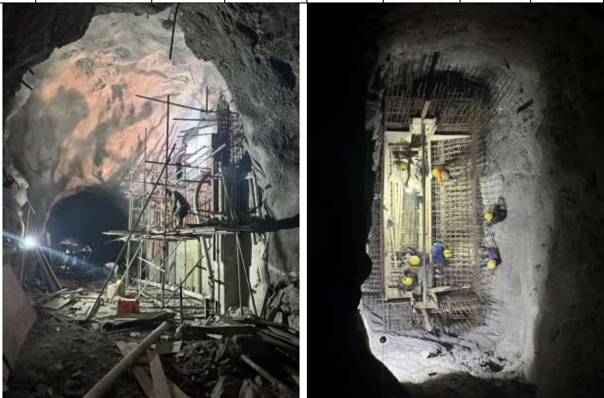
Figure 2-18: Concreting at Inlet gate shaft 01 (left) and Inlet gate shaft 02 (right)
