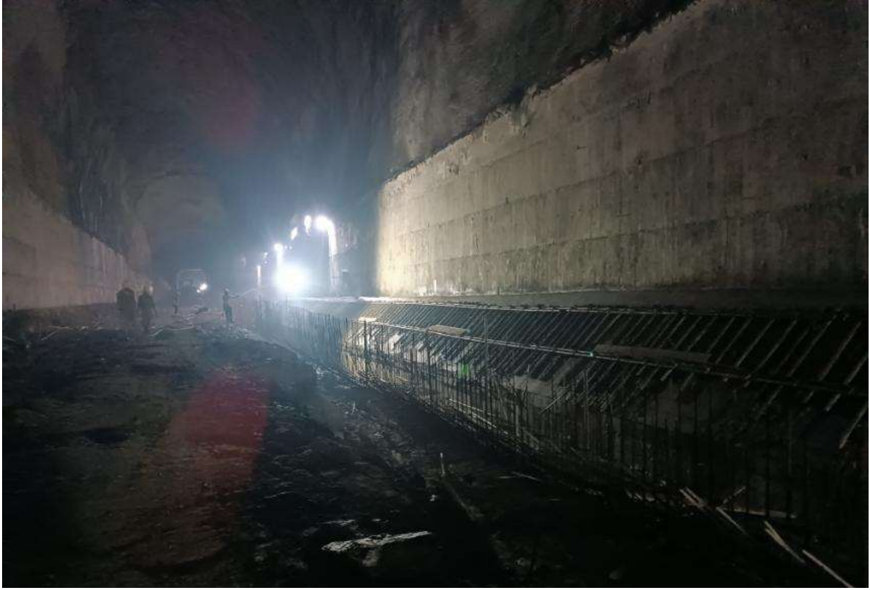
Figure 2-10: A view of SB 01 with completed wall lining and hopper concreting
