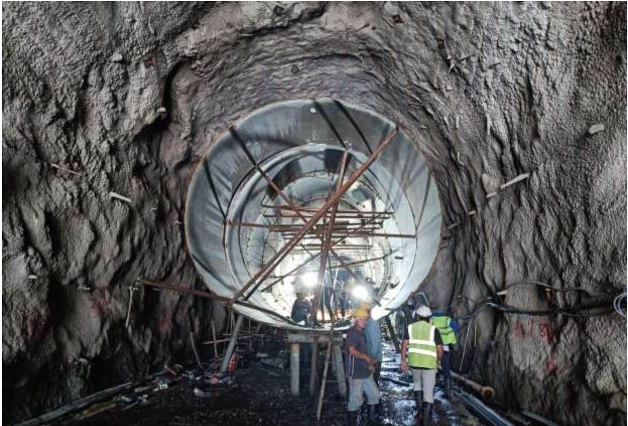
Figure 2-41: Installation of pwnstock pipes inside HRT from outlet region
