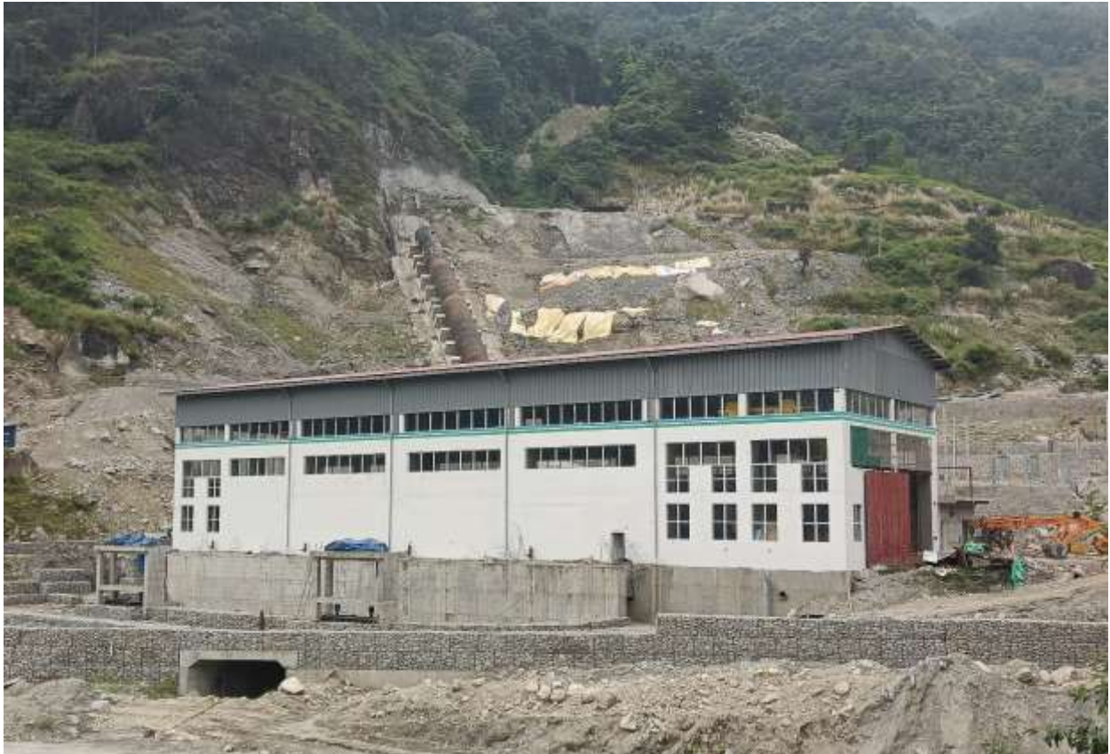
Figure 2-33: A view of powerhouse building
