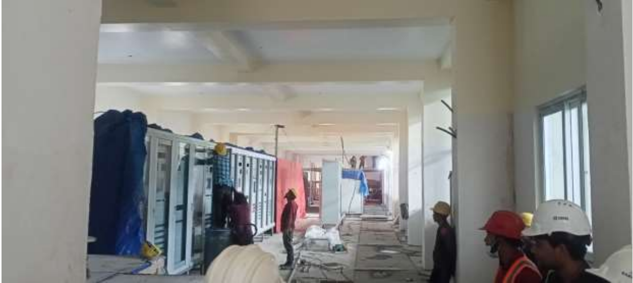
Figure 2-69: Installation of control panels
