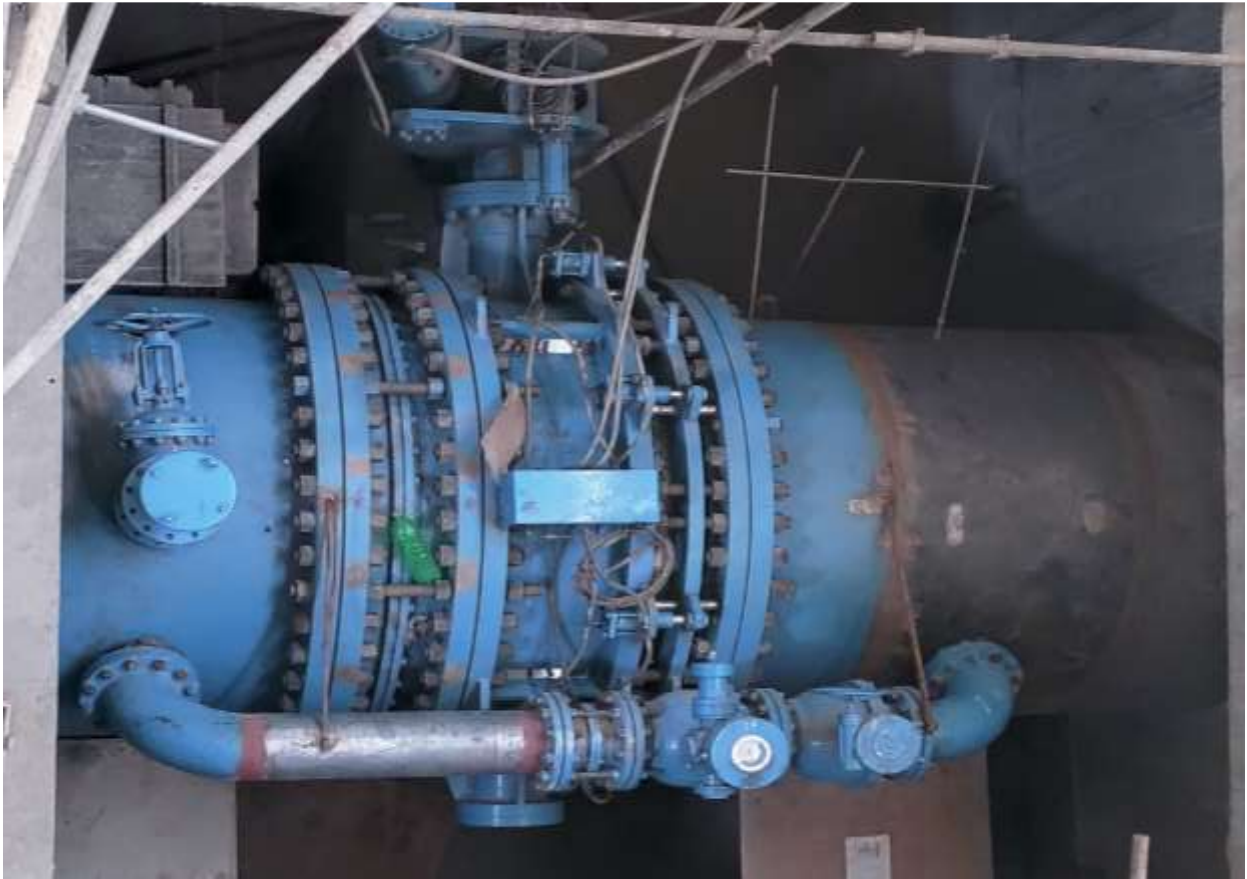
Figure 2-65: Unit 01 bypass valve work
