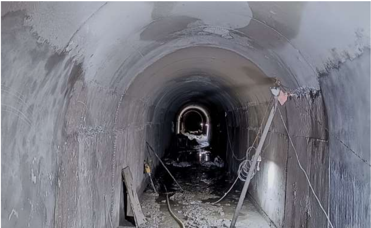
Figure 2-24: A view of full concrete lining at the flushing tunnel
