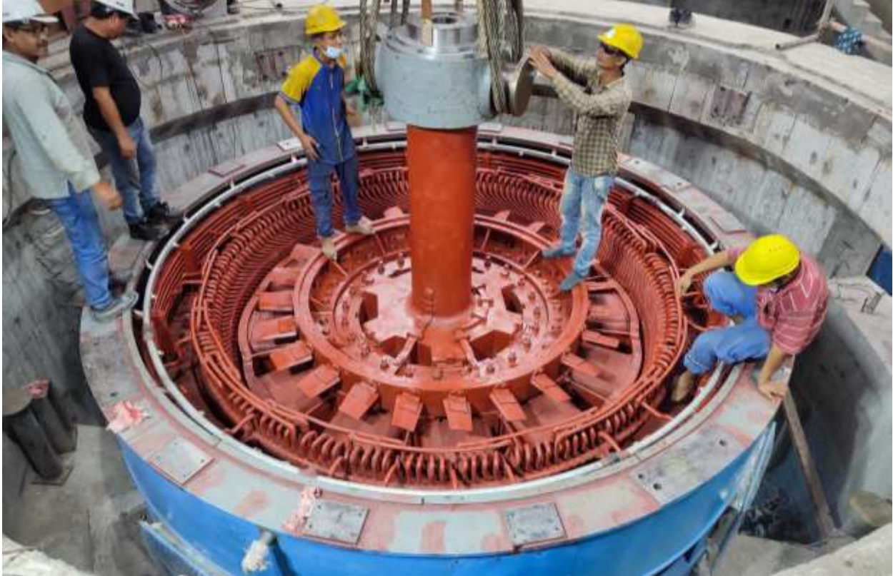
Figure 2-62: Rotor lowering of unit 04
