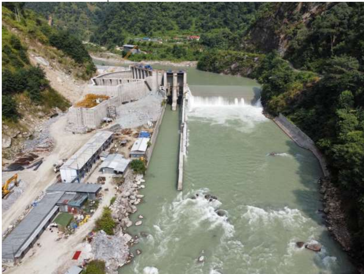
Figure 2-3: Aerial view of Headworks from the downstream
