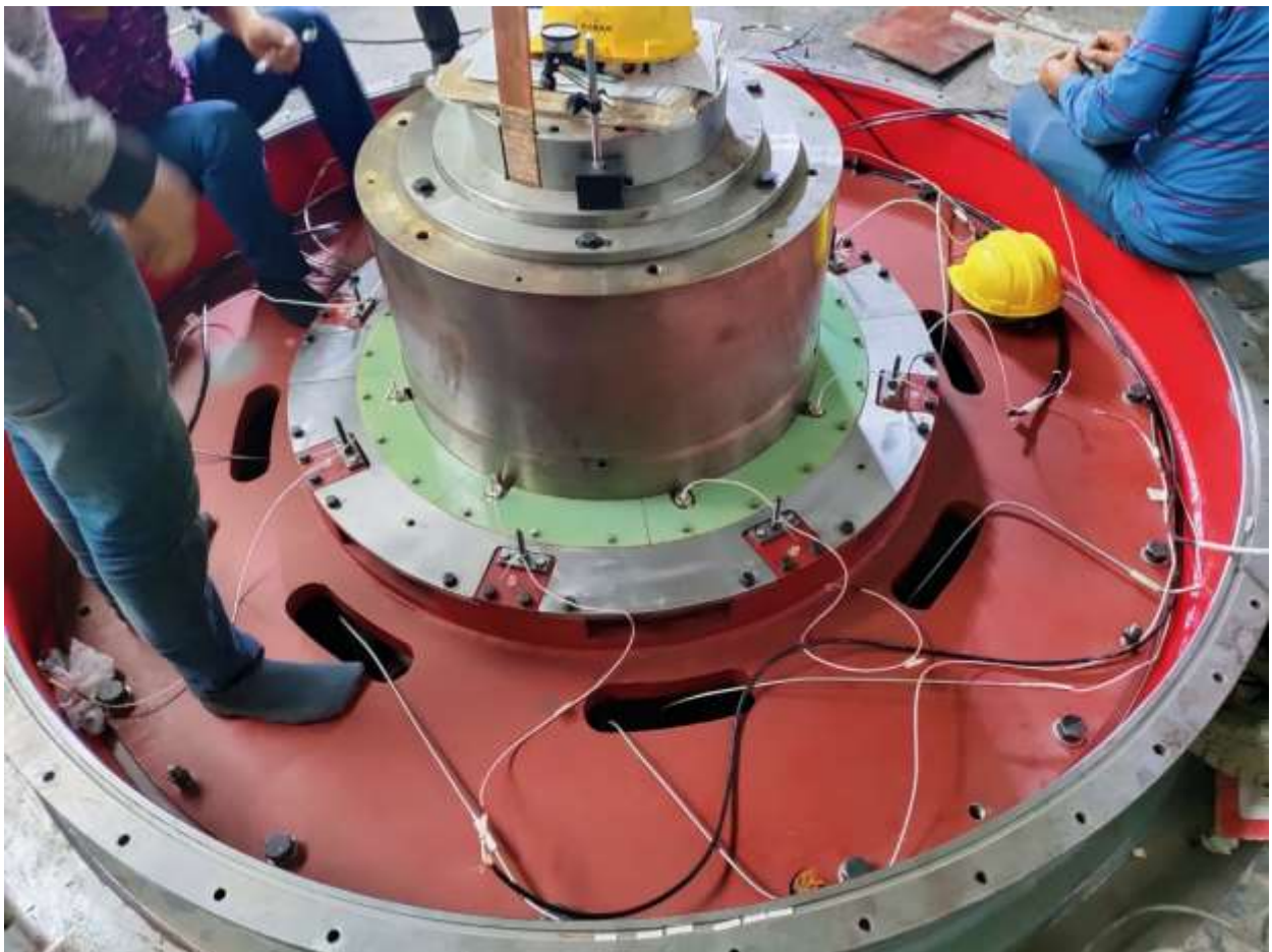
Figure 2-51: Installation of temperature and resistance measuring sensors at thrust bearing
