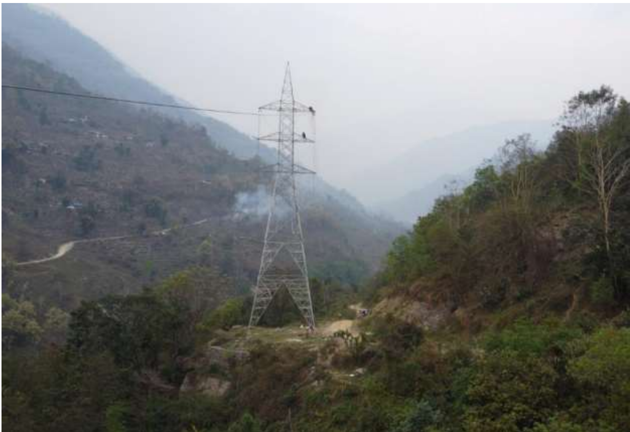
Figure 2-77: A view of stringing works
