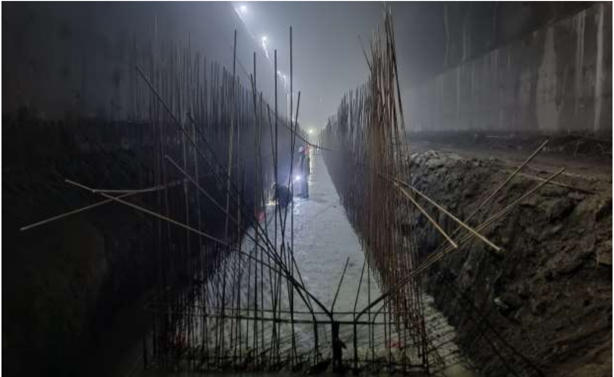
Figure 2-11: A view of concreting at the left hopper of Settling Basin 01
