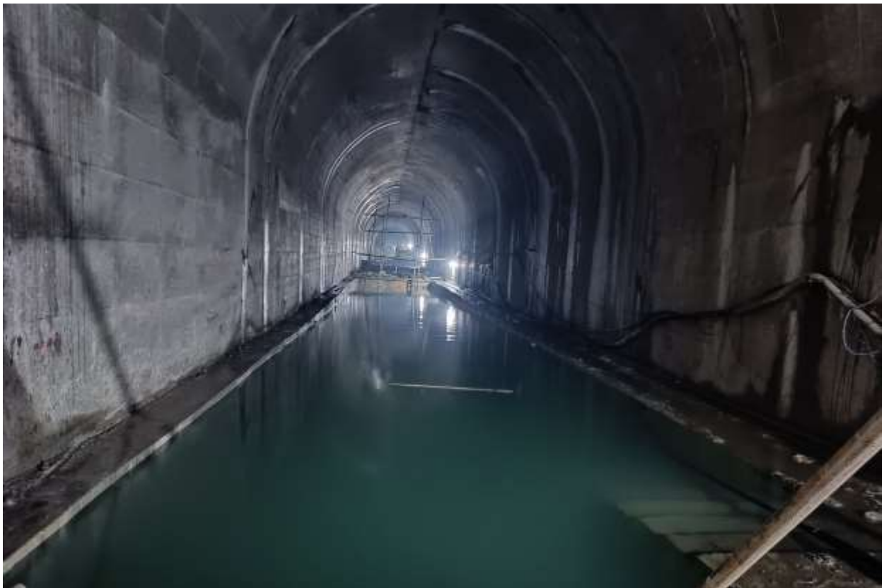
Figure 2-22: A completed section of concrete lining works at rock trap
