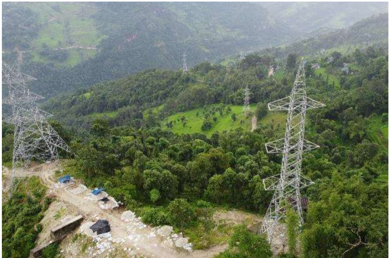
Figure 2-79: Erected last tower at AP24 and tower of NEA (left)
