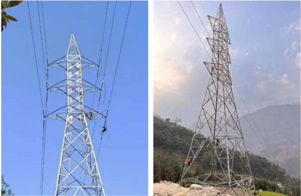
Figure 2-78: Conductor stringing works at various angle points
