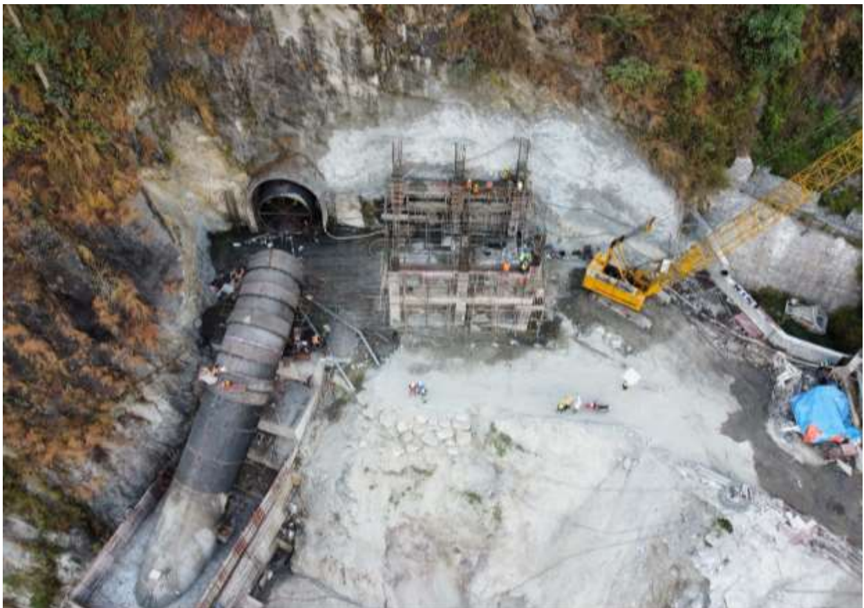
Figure 2-34: Construction of valve house
