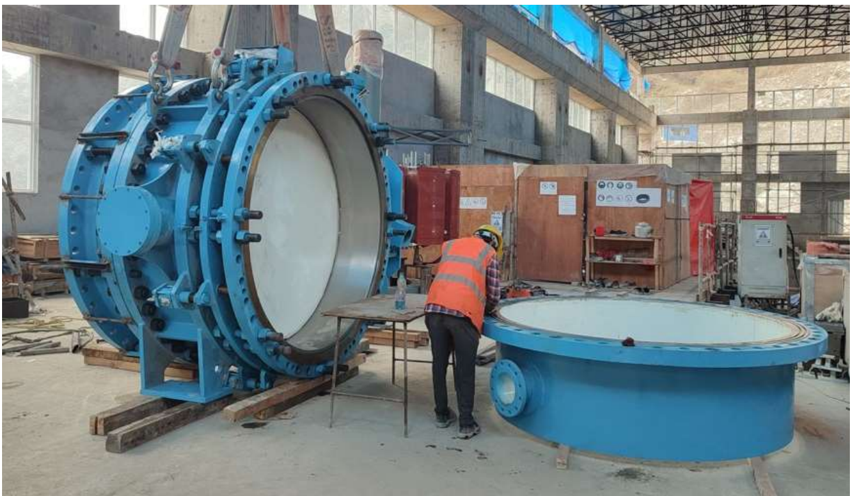
Figure 2-68: MIV assembled at service bay
