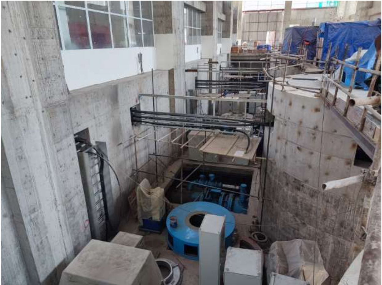
Figure 2-71: Laying of power and control cables in main powerhouse
