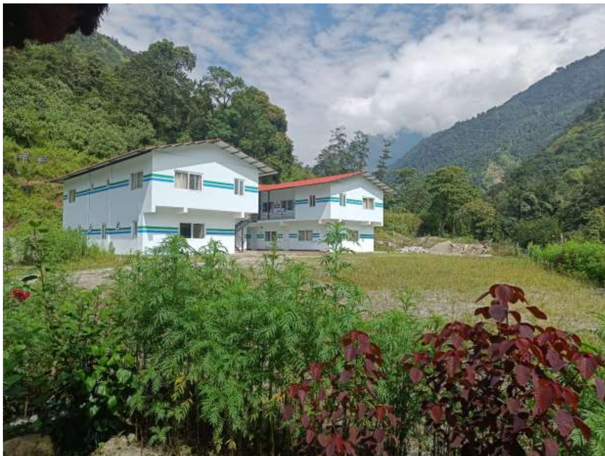
Figure 2-2: Construction of new camp building at the powerhouse
