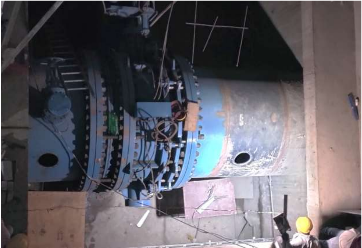
Figure 2-67: Unit 03 preparation for bypass valve erection
