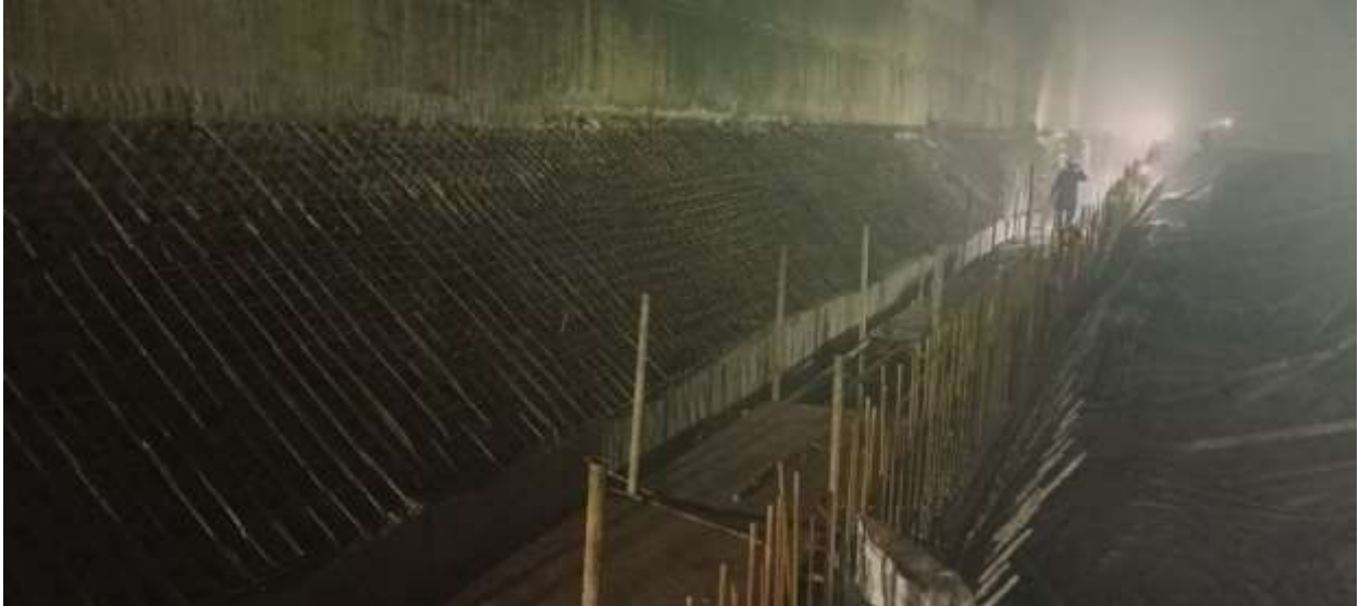
Figure 2-14: Rebar layout of hopper of SB 02
