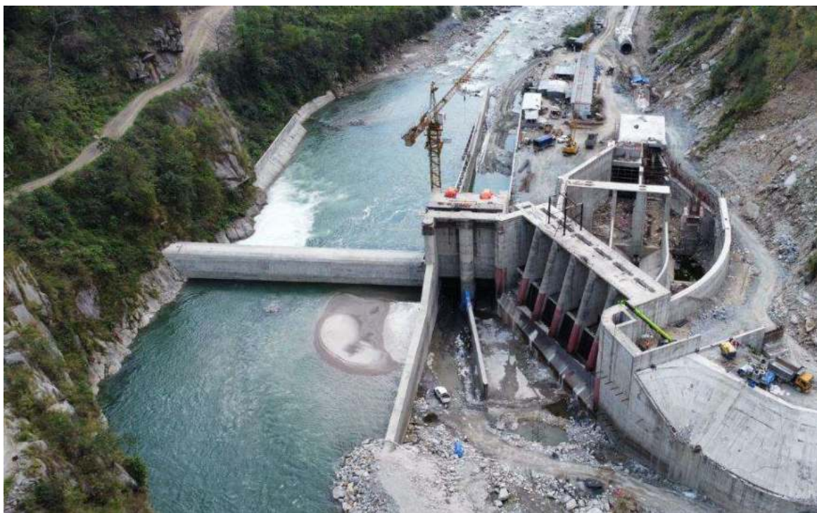
Figure 2-7: Aerial view of headworks from upstream
