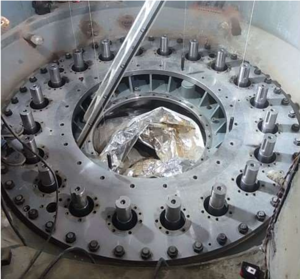
Figure 2-66: Preassembly of head cover
