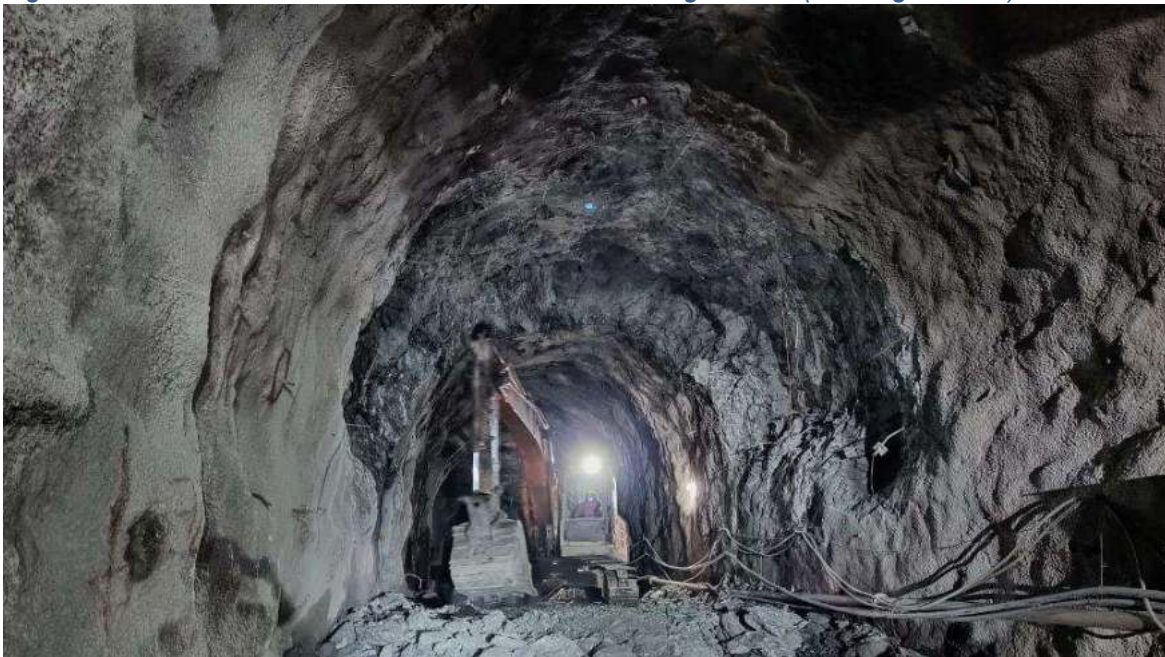
Figure 2-18: Excavation of plug block 01 at HRT outlet region
