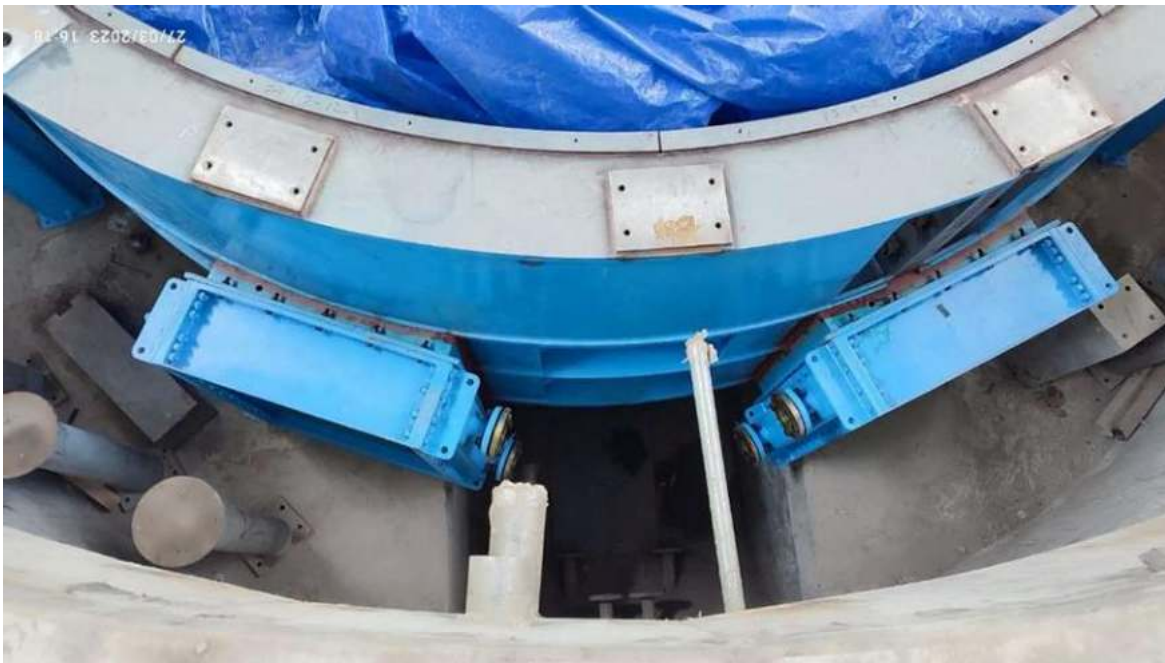
Figure 2-61: Final assembly of stator air cooler
