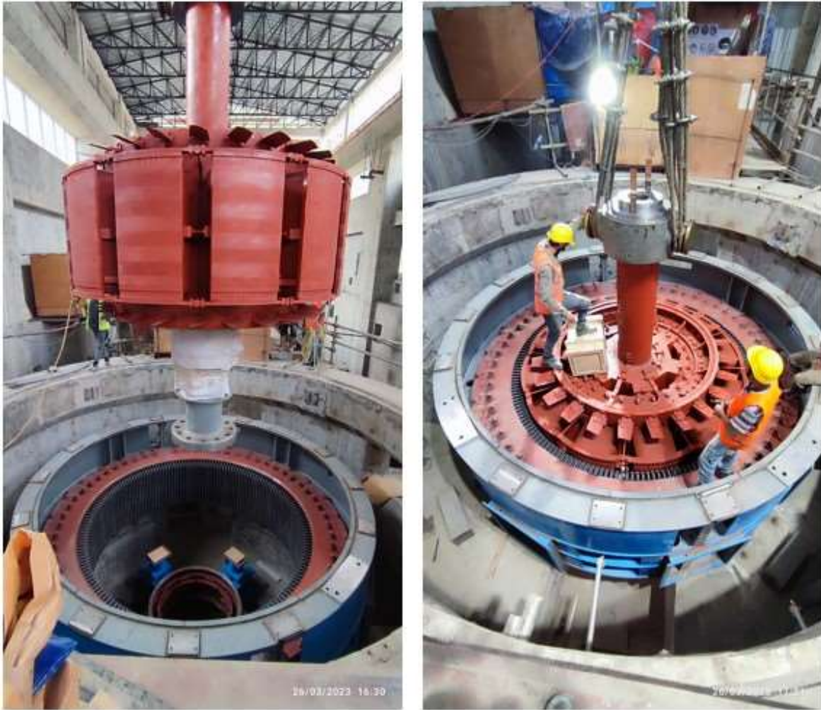
Figure 2-63: Temporary parking of roter of unit 01 at unit 02
