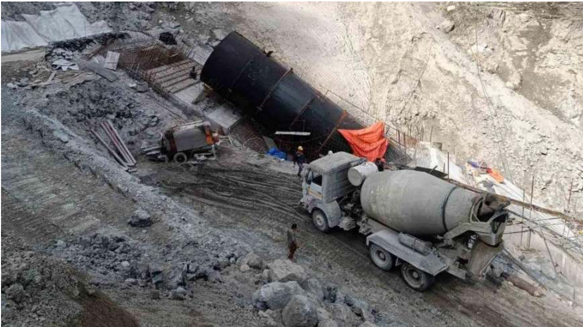
Figure 2-33: A view of erection of penstock pipes (thickness 32 mm)
