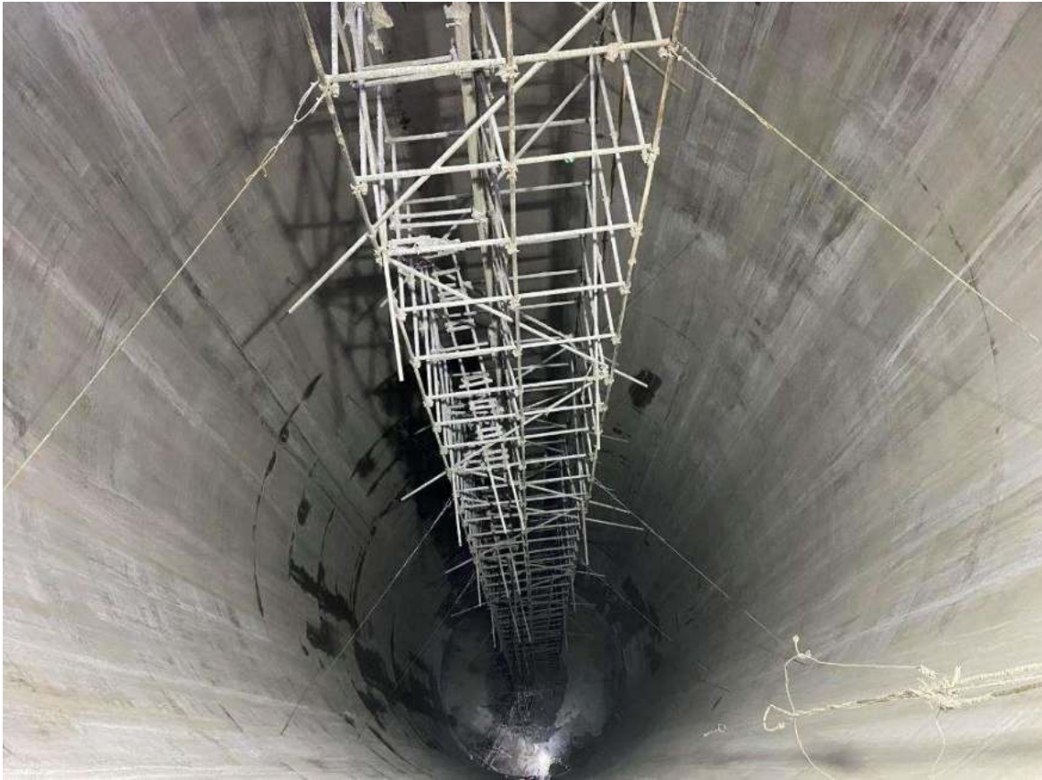
Figure 2-22: A view of surge shaft (Concrete lining completed)
