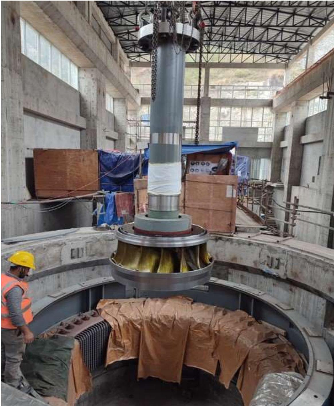
Figure 2-59: Lowering of runner with main shaft in unit 2
