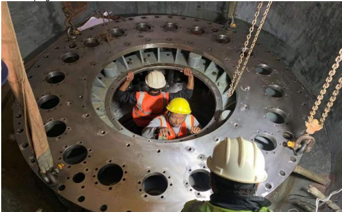
Figure 47: Lowering of headcover in unit 2
