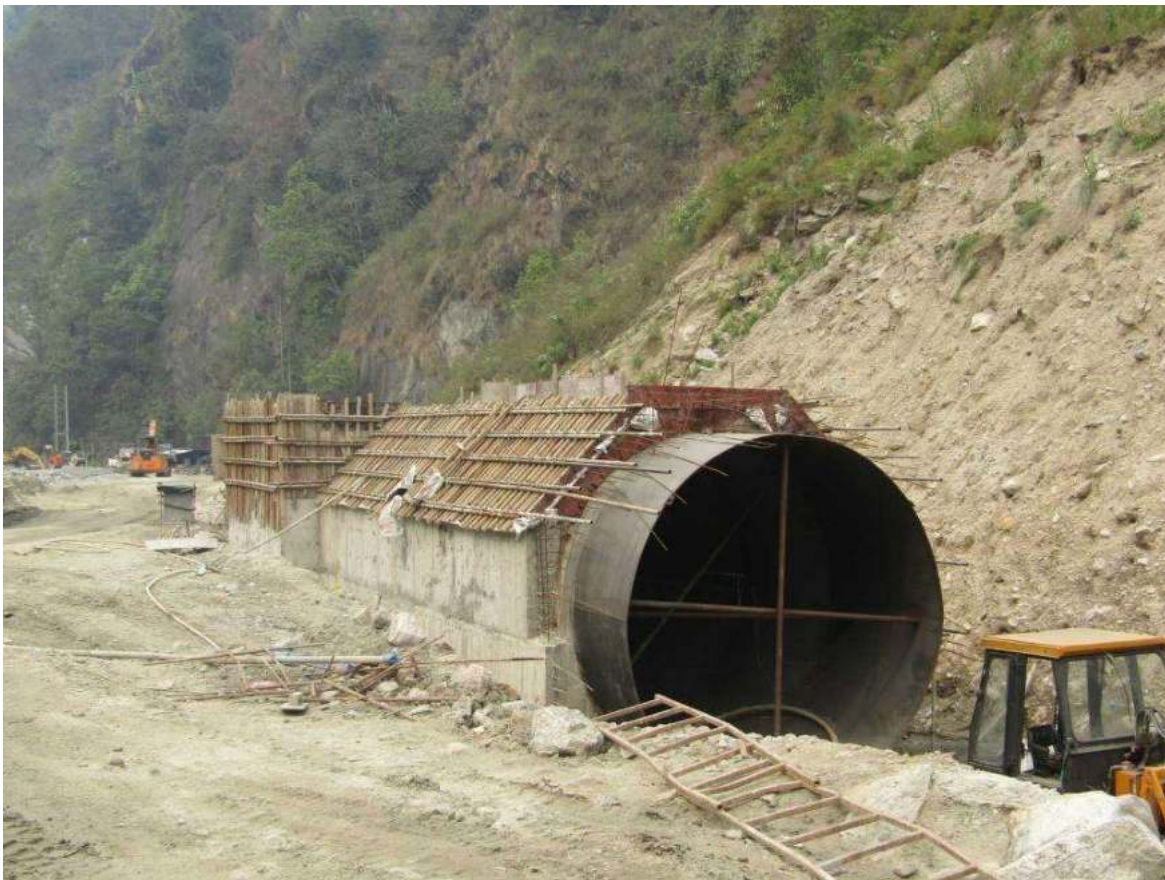
Figure 2-10: Erection of approach pipe
