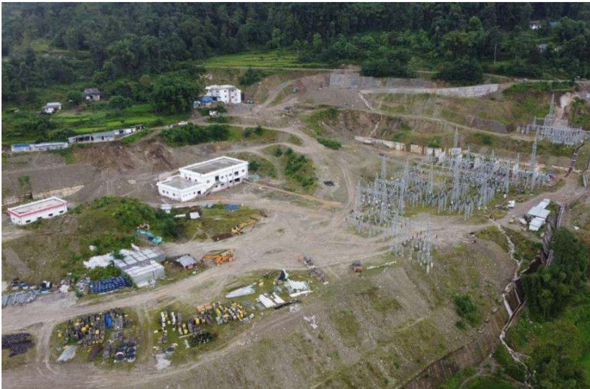
Figure 2-74: An aerial view of Dhunge-sanghu substation (NEA Project)
