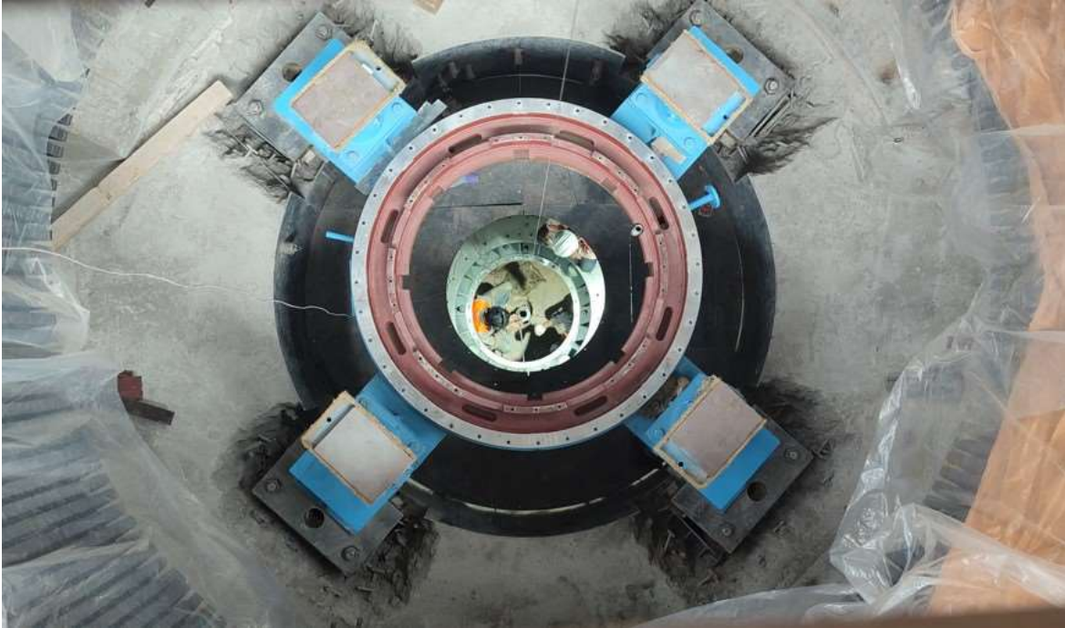
Figure 2-67: Lower bracket placed in to the pit
