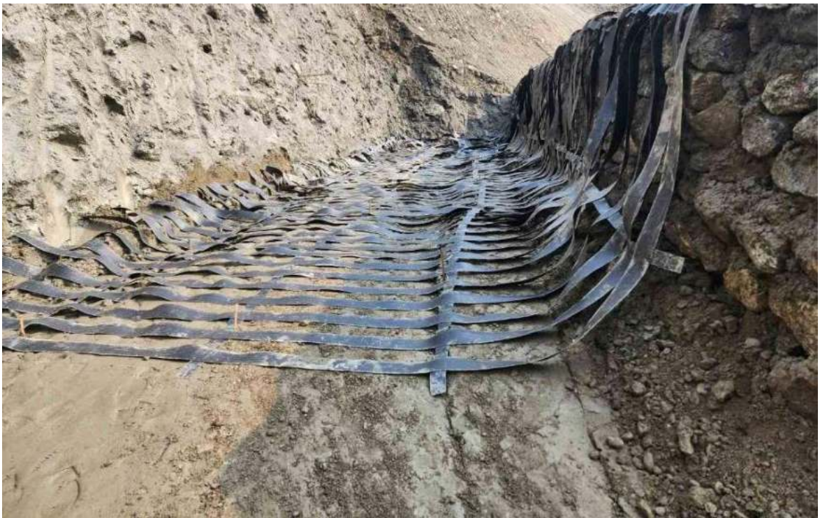
Figure 2-29: Penstock slope stablization using geogrid (paralink)
