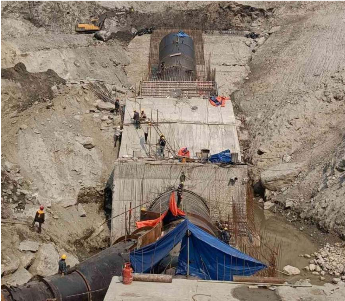
Figure 2-34: Penstock slope stabilization and simultaneous penstock pipe installation
