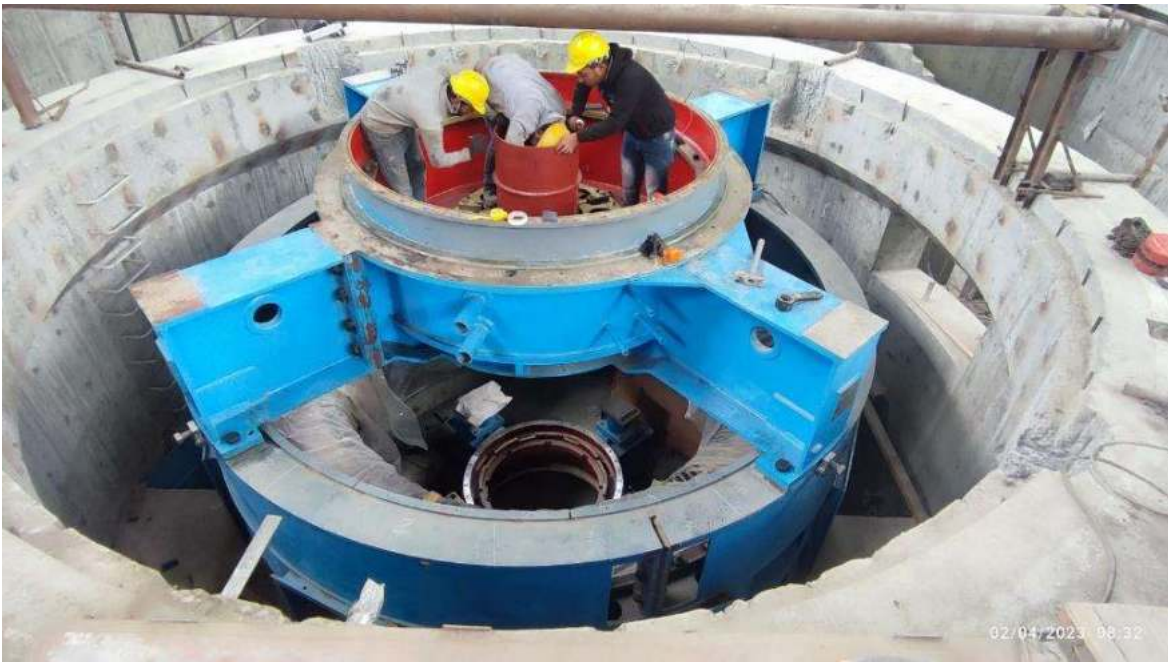
Figure 2-68: Upper bracket lowered in to the pit
