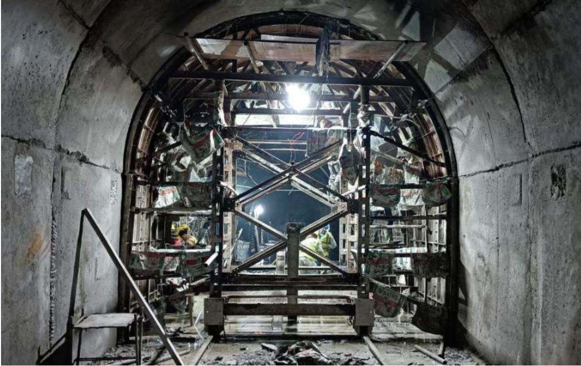
Figure 2-20: Assembling of formwork for full concrete lining at connecting tunnel 03
