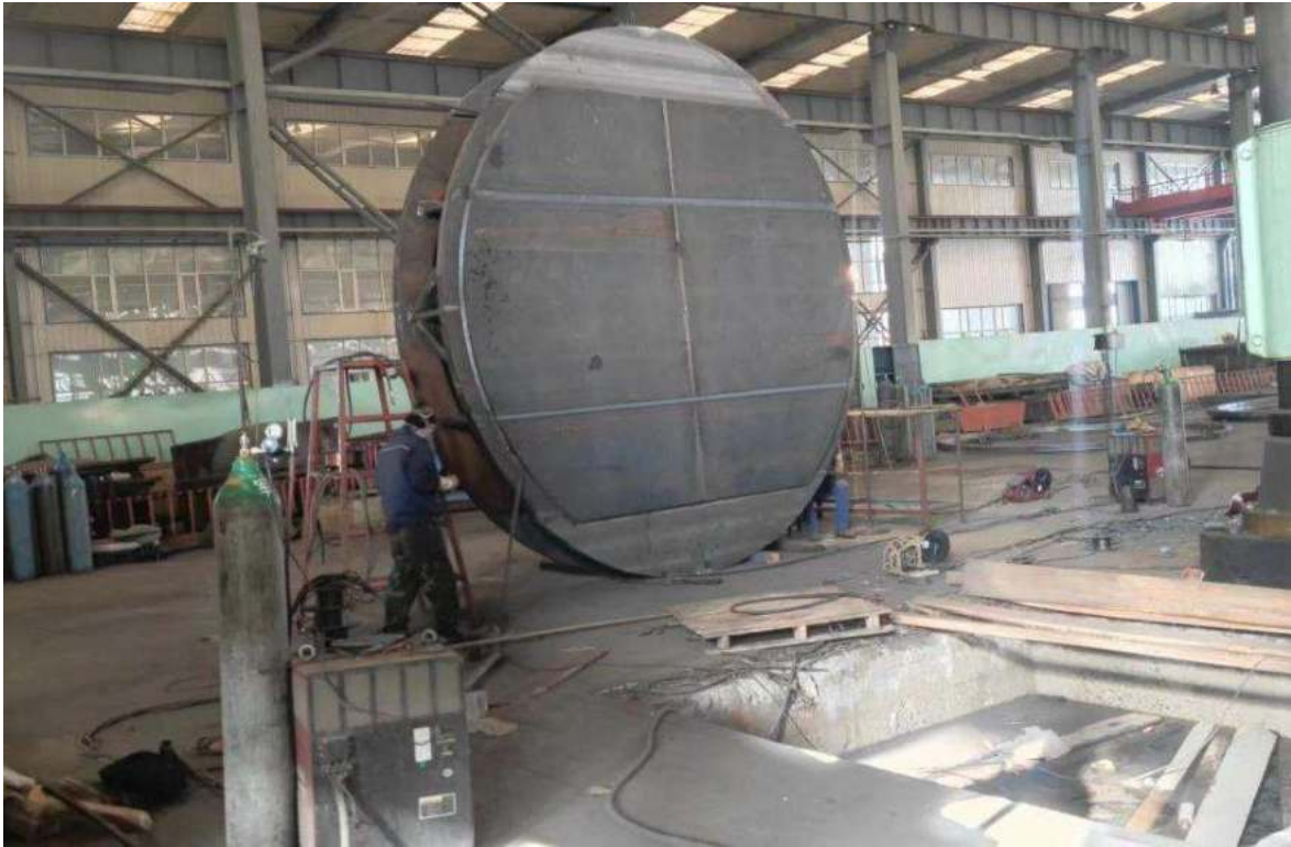
Figure 2-49: PPV disc being welded in a factory in China
