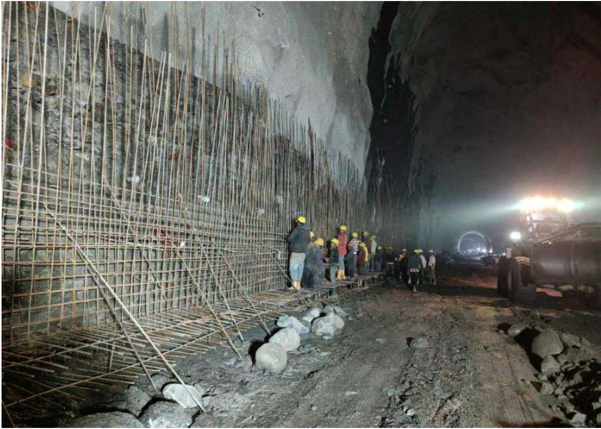
Figure 2-12: Rebar layout at right wall of settling basin 01
