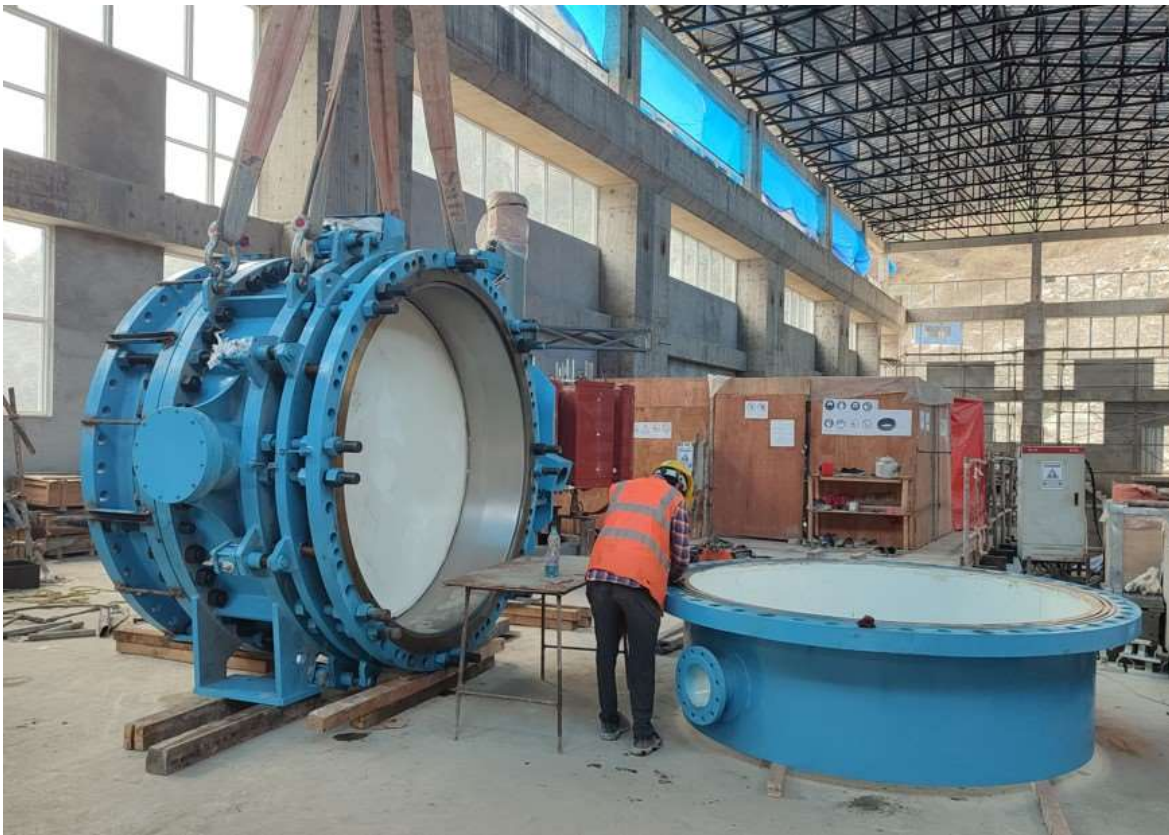
Figure 2-70: Unit 2 MIV assembled at Service bay
