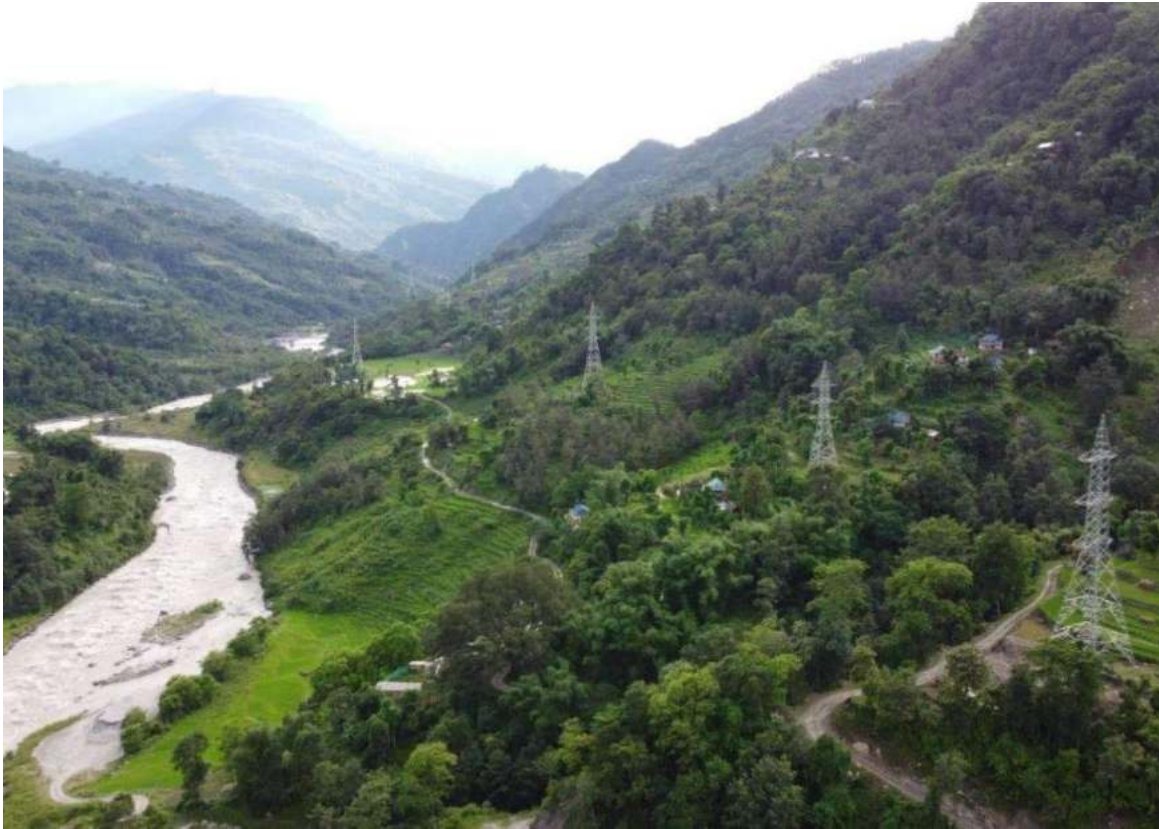
Figure 2-73: View of erected towers from right bank of Tamor
