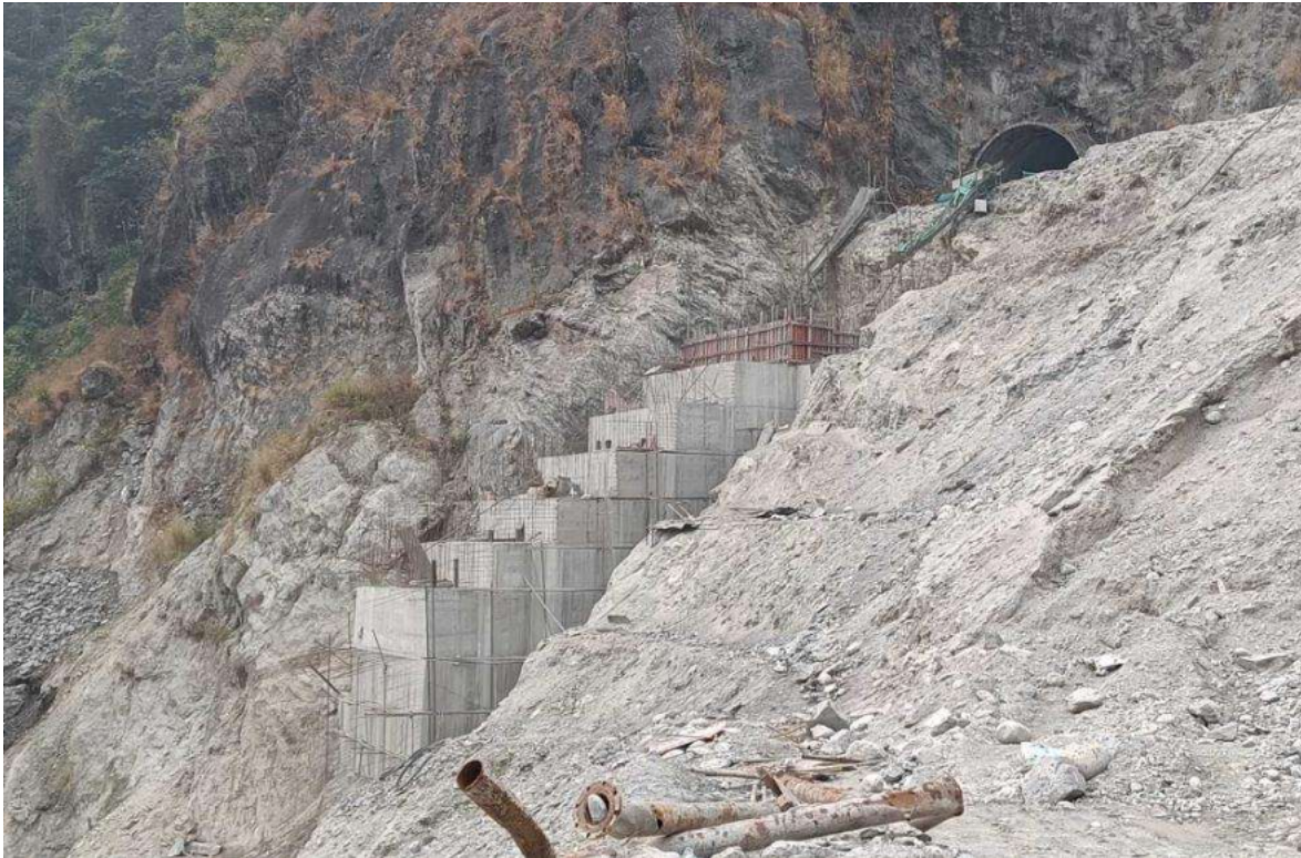
Figure 2-28: Concreting of anchor block
