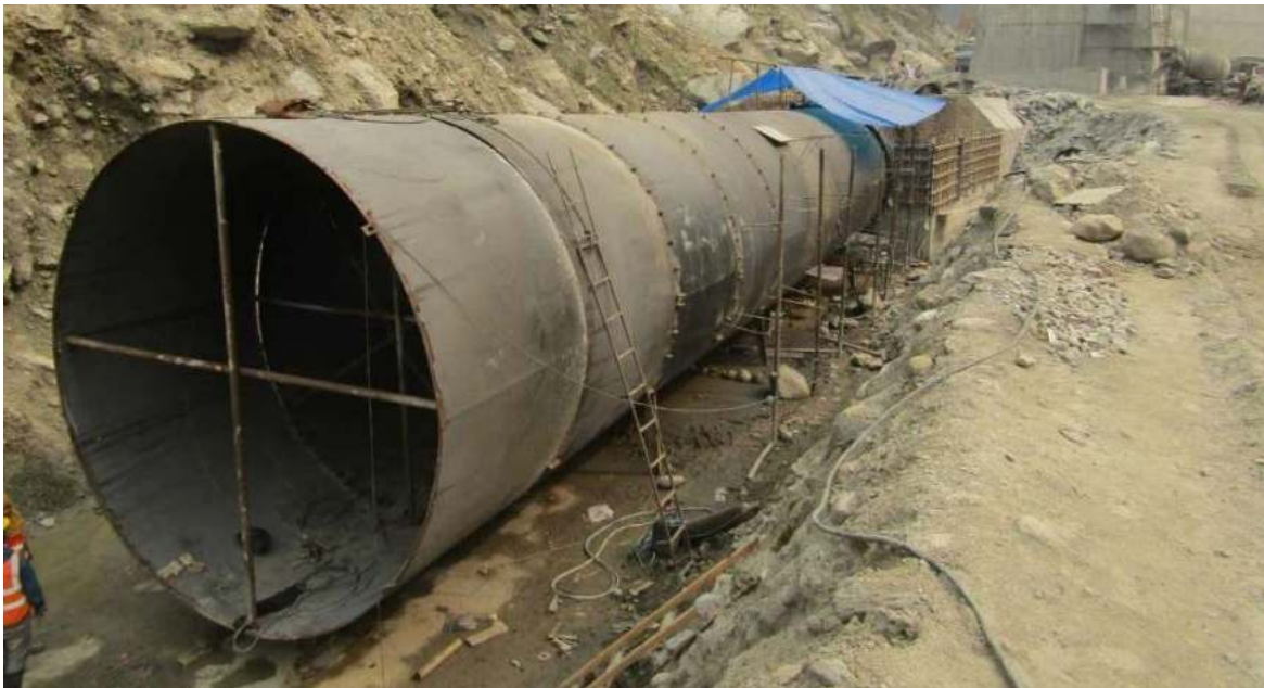
Figure 2-32: Installation of approach pipes at headworks region
