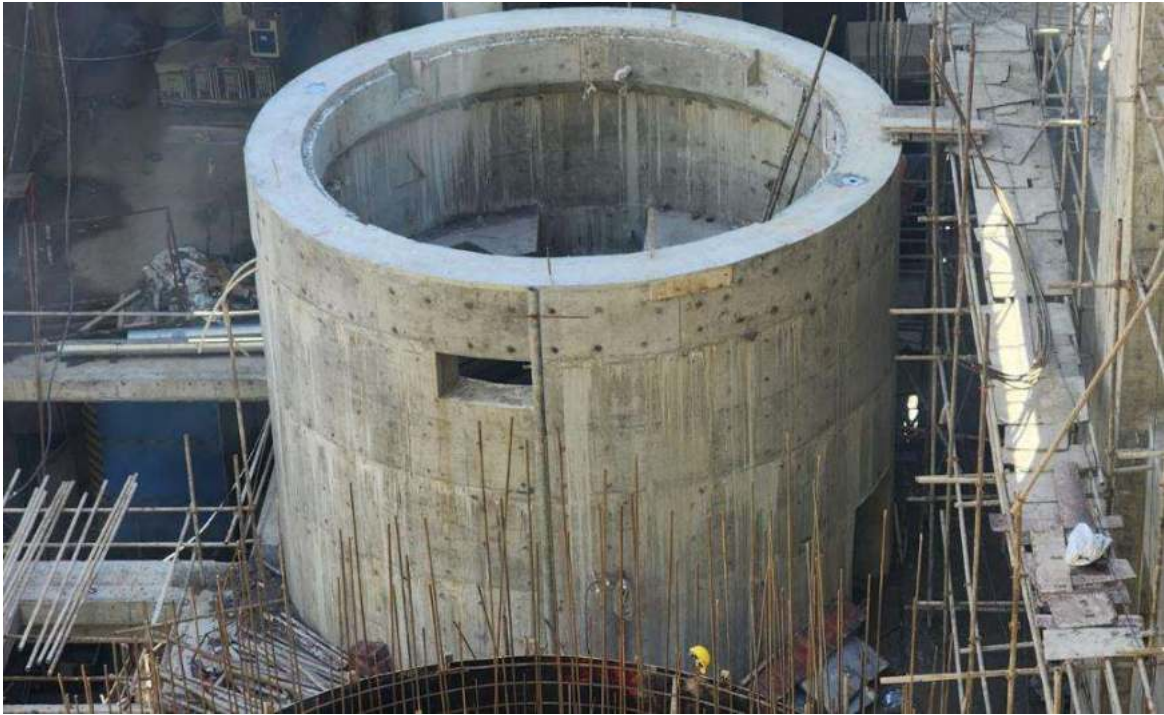
Figure 2-30: Casting of generator casing at unit 01
