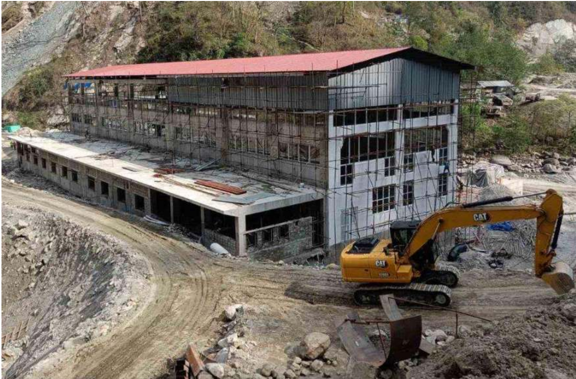
Figure 2-26: A view of Powerhouse and control bay
