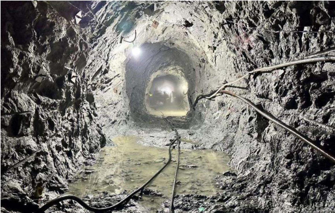
Figure 2-21: A view of invert cleaning works at the flushing tunnel
