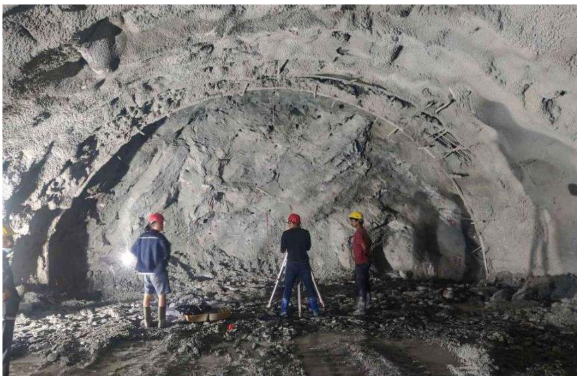
Figure 2-14: Surveying works at SB 03 face
