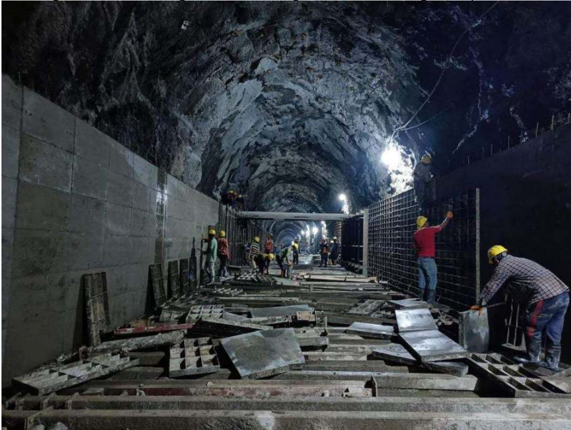
Figure 2-15: A section of HRT with concrete wal lining
