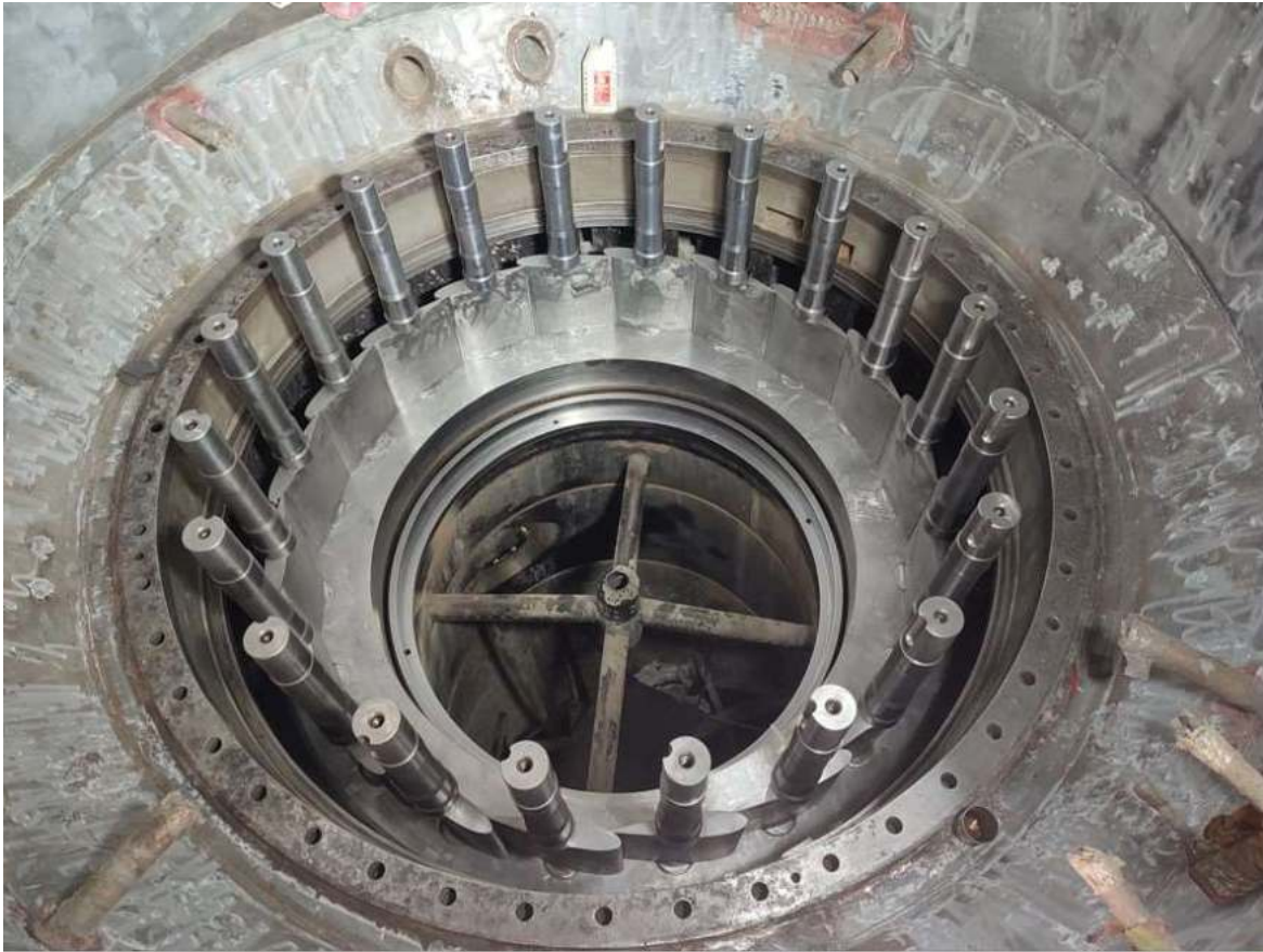
Figure 2-64: Preassembly of bottom ring and guide vane
