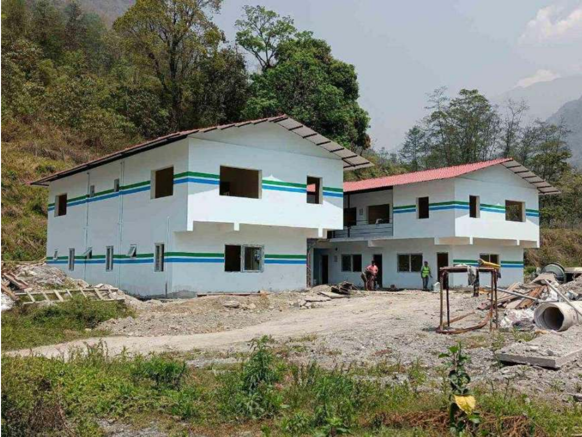
Figure 2: Construction of new camp building at the powerhouse
