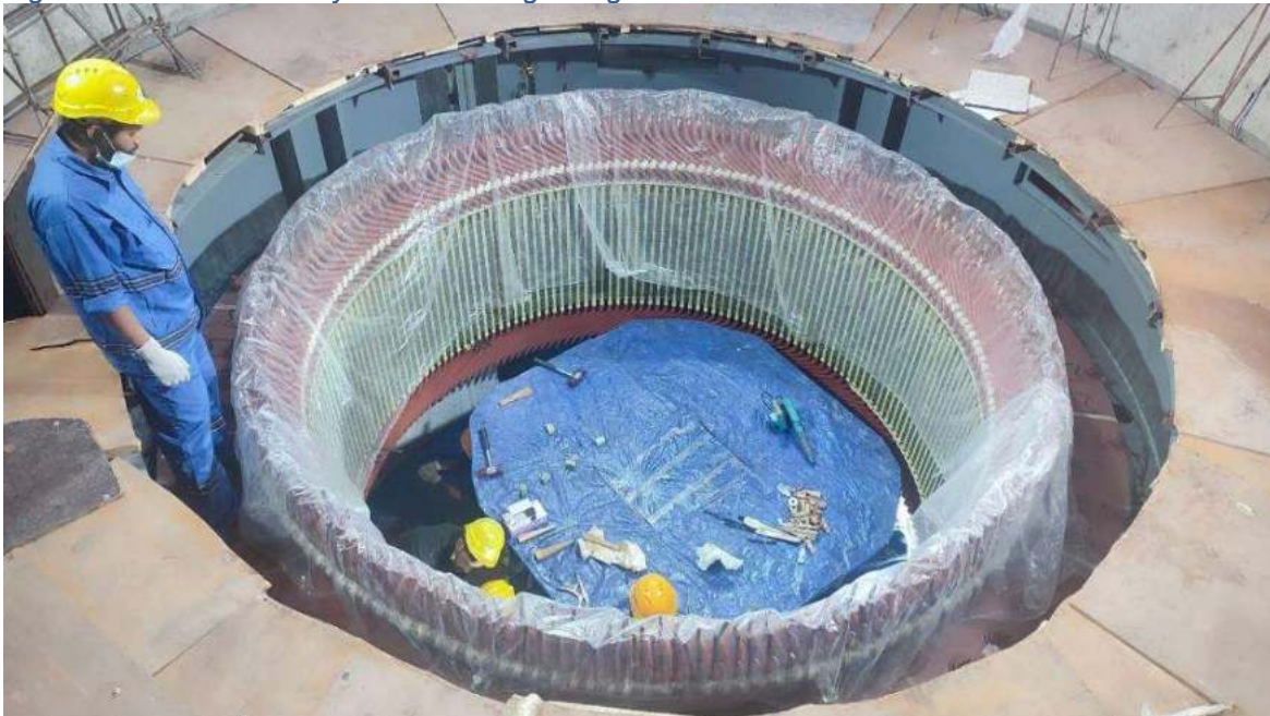
Figure 2-65: Completion of stator winding works
