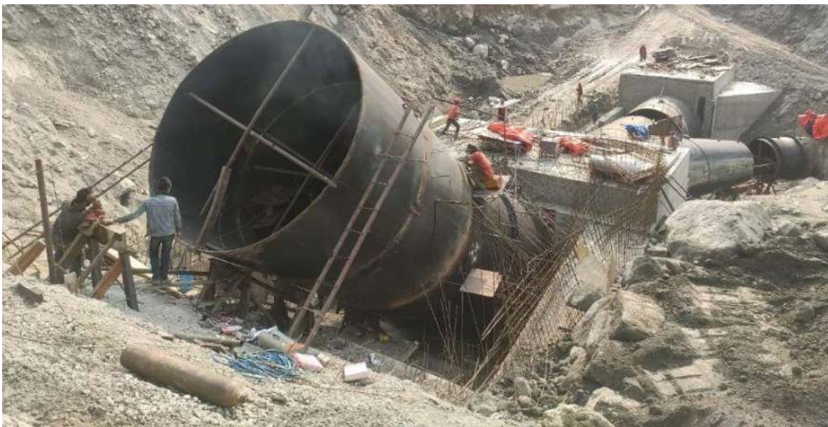
Figure 2-36: Erection of penstock pipe (thickness 30 mm)
