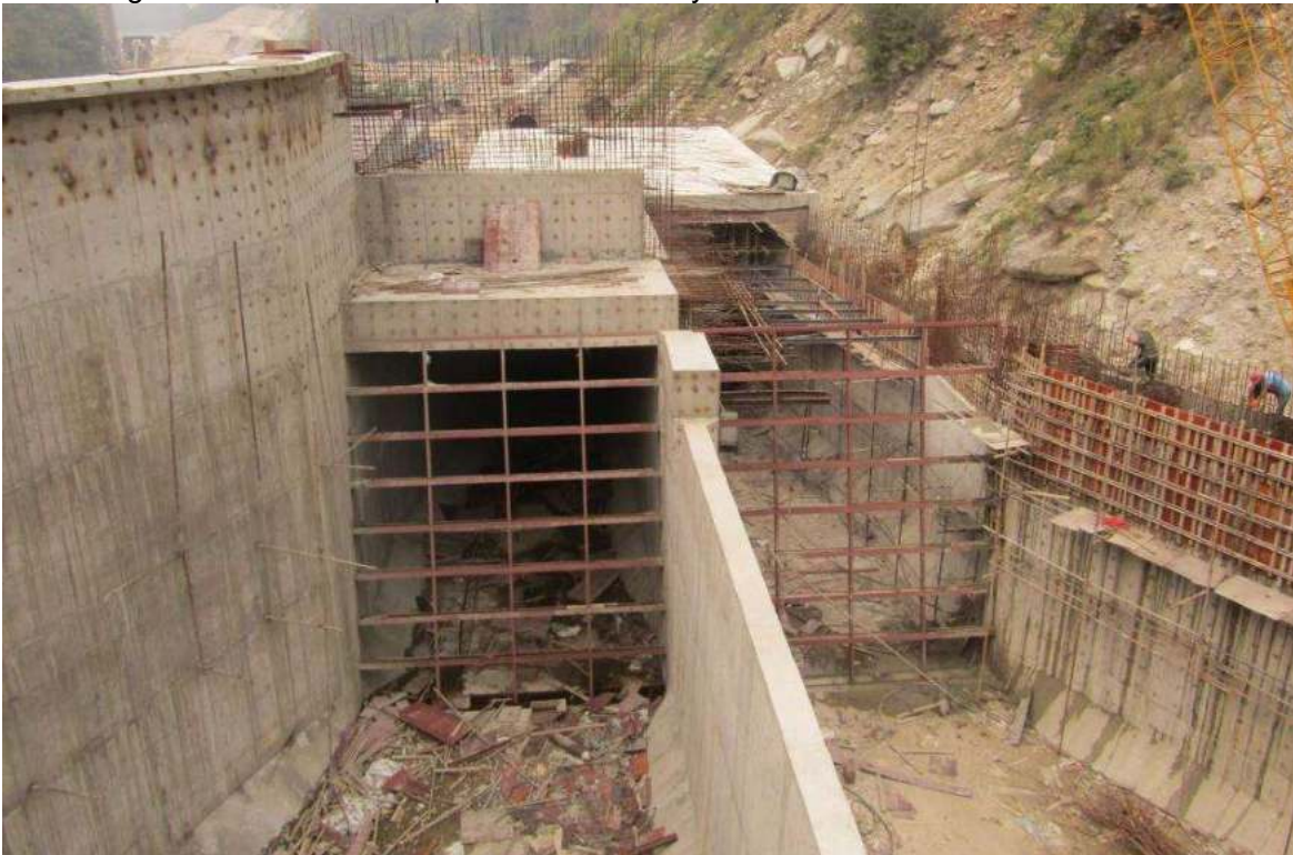
Figure 2-9: Concreting of conveyance tank nearing completion
