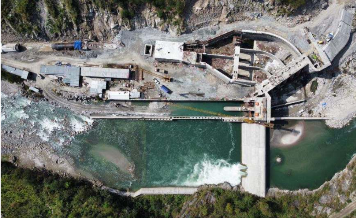
Figure 2-4: Aerial view of Headworks
