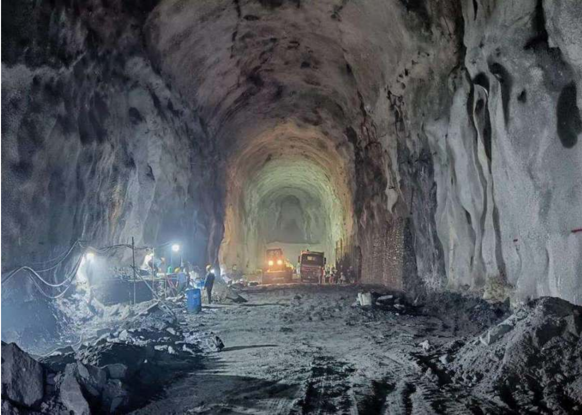
Figure 2-11: A view of stone masonry works at Settling basin 01
