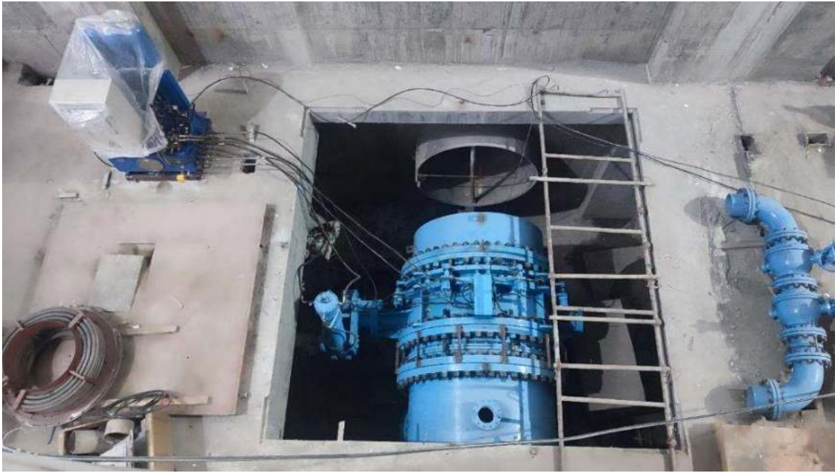
Figure 2-69: Unit 4 MIV lowered to its position
