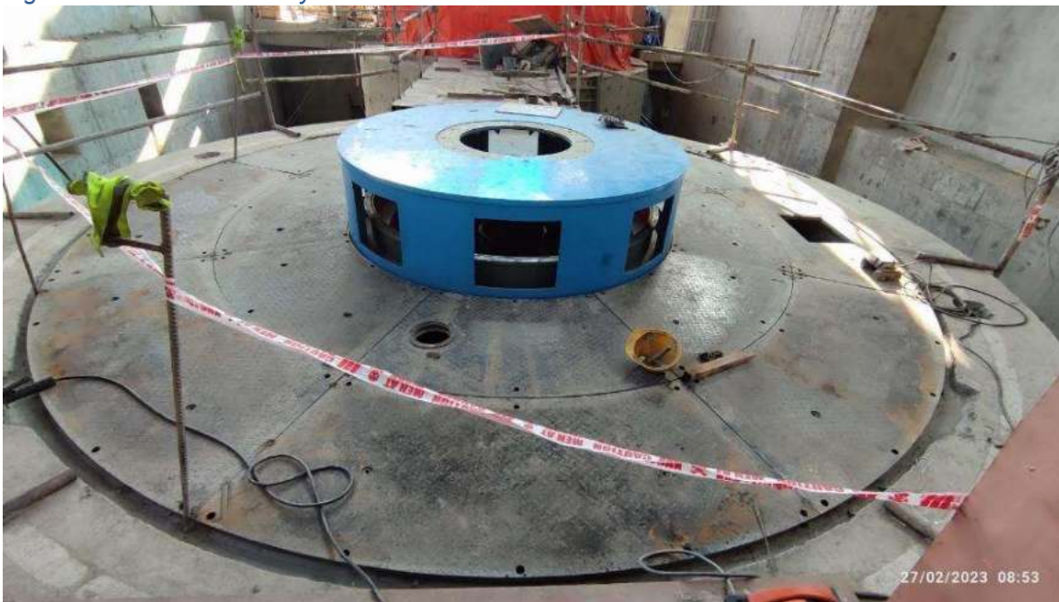
Figure 2-62: Preassembly of generator floor cover plate
