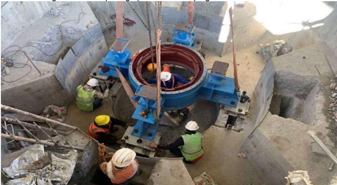
Figure 2-55: Installation of lower bracket in unit 1
