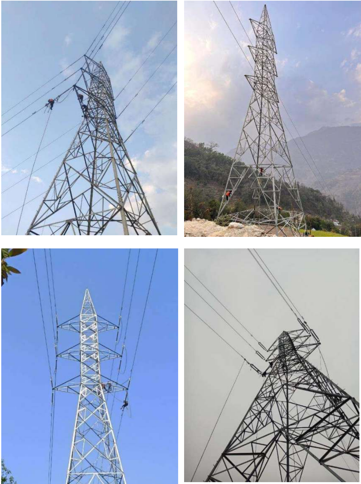
Figure 2-76: Conductor stringing works at various angle points
