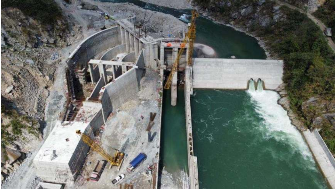
Figure 2-5: Concreting works at gravel trap and conveyance tank
