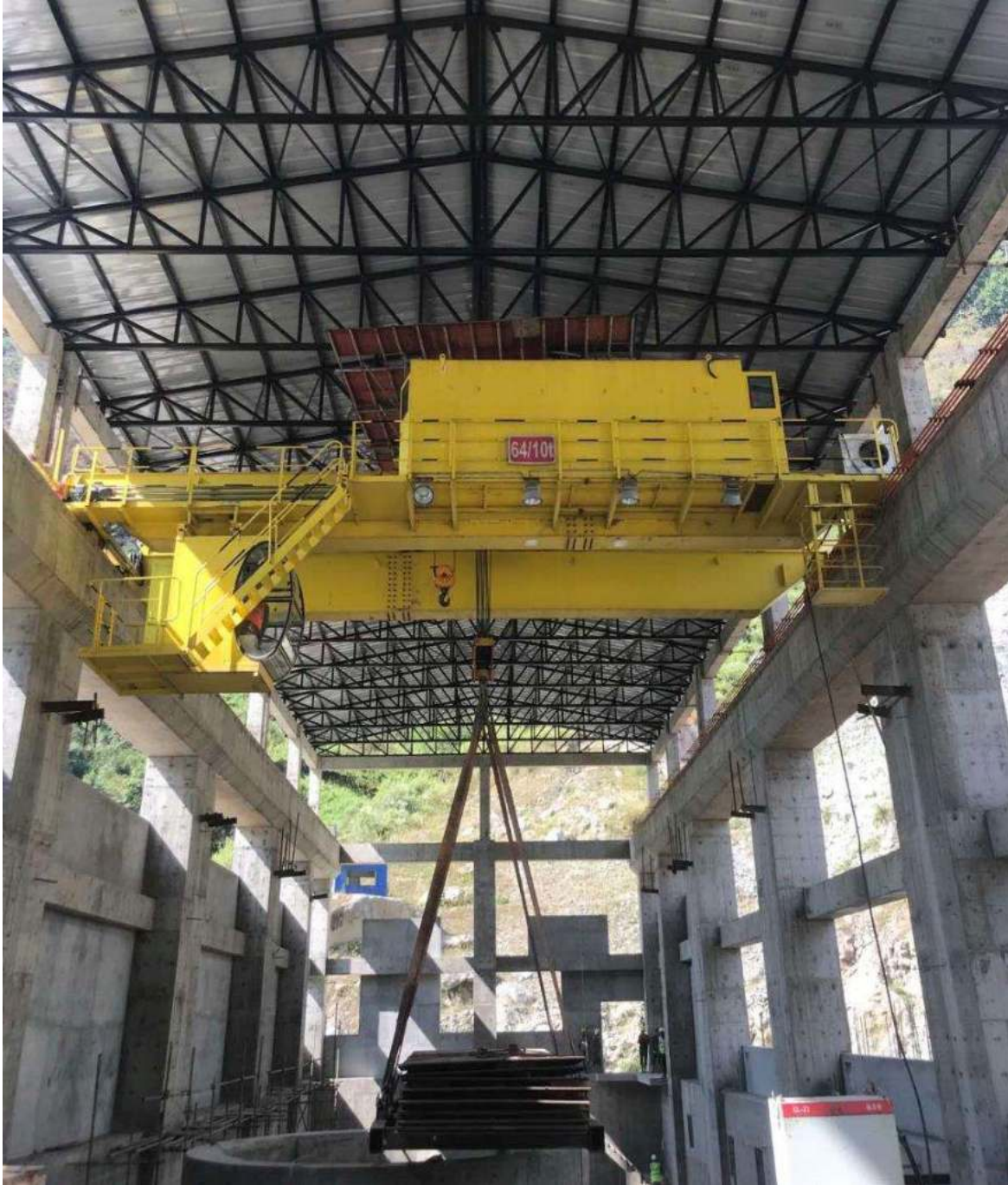
Figure 2-53: Load test of EOT lifting 66 ton and travelling across unit 2
