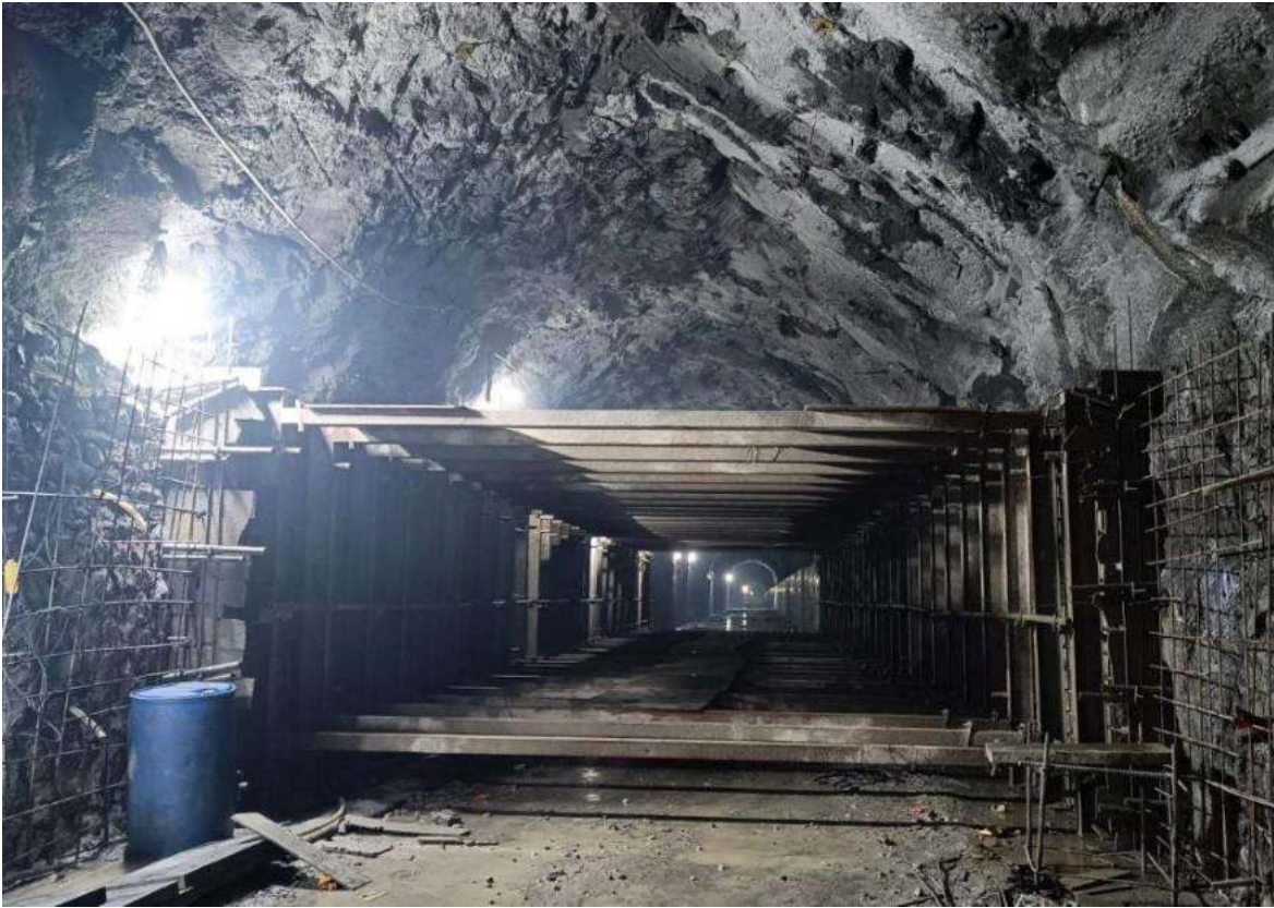
Figure 2-16: Preparation of formwork assembly for concrete wall lining at chainage 1+100
