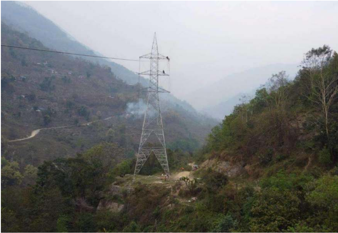
Figure 2-75: A view of stringing works
