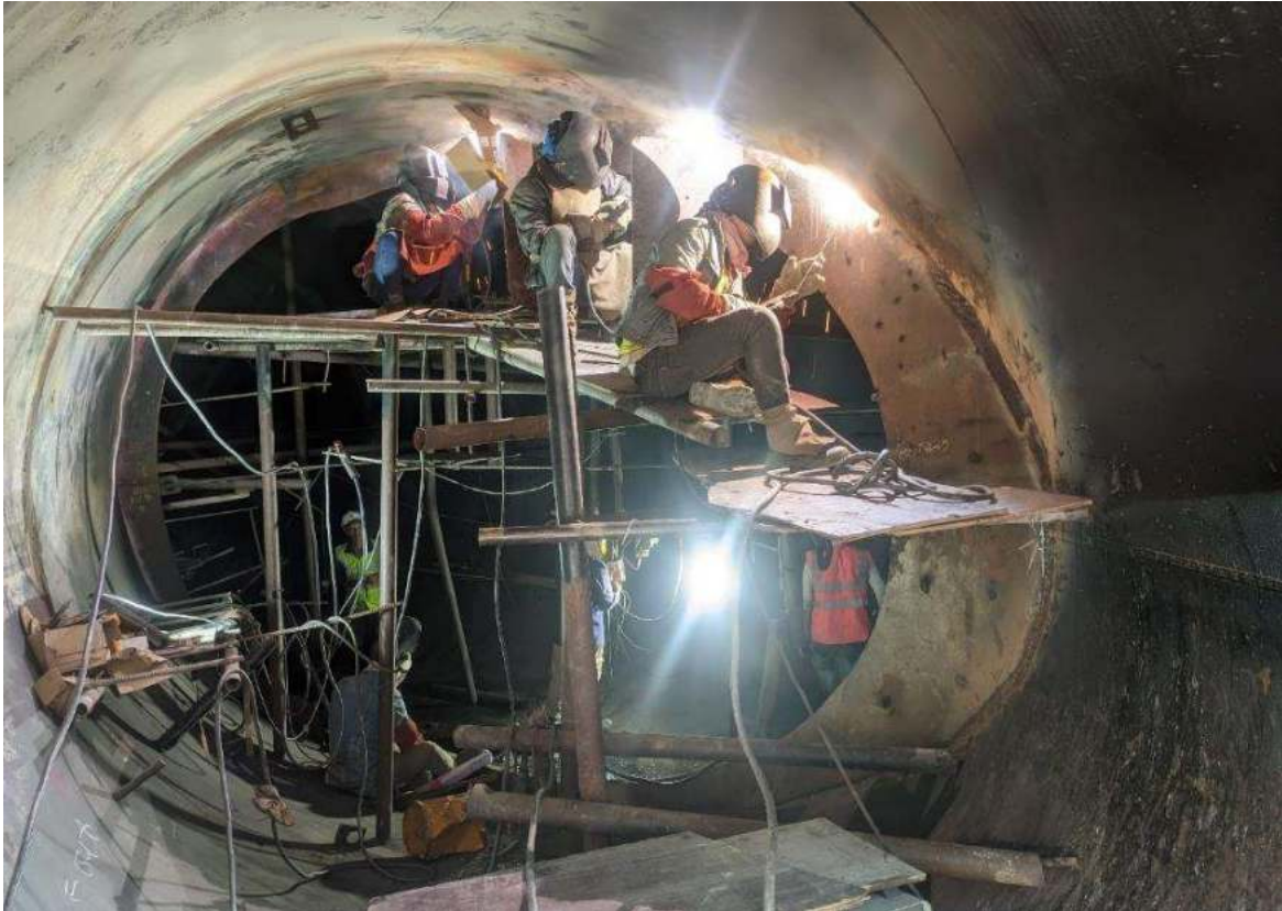
Figure 2-39: Welding work at sickle plate of bifurcation 01
