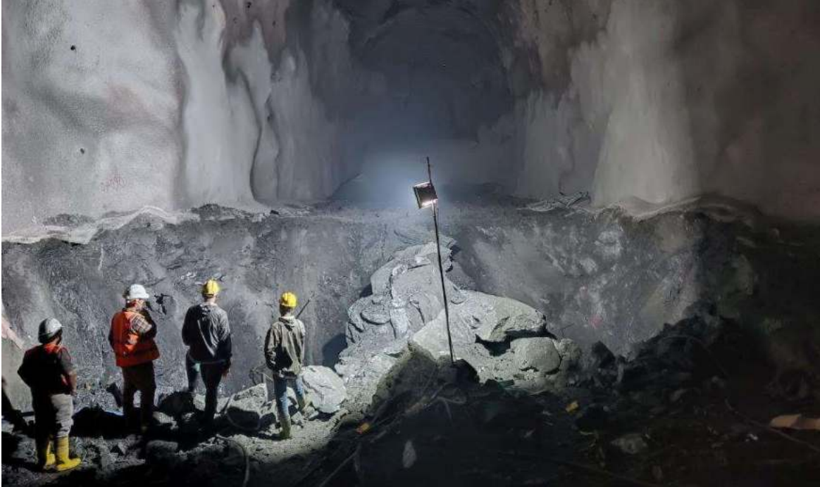
Figure 2-13: Excavation of hooper face
