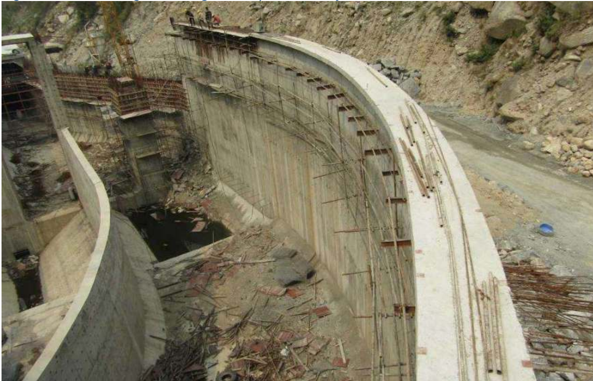
Figure 2-6: Concreting at the hillside wall of intake completed
