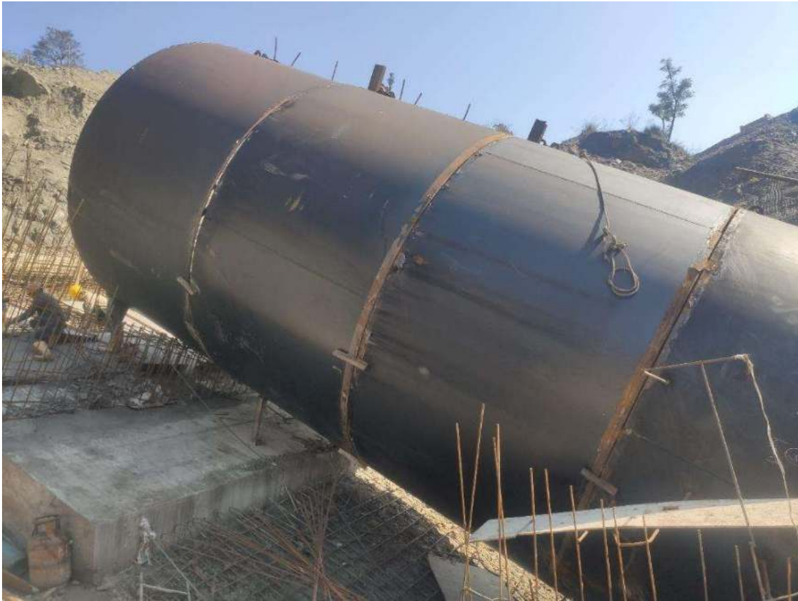
Figure 2-35: Erection of inclined penstock pipe
