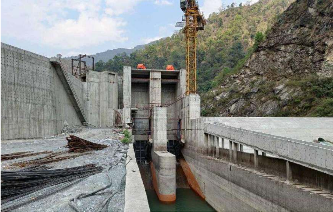
Figure 2-8: Gate installation works at undersluice
