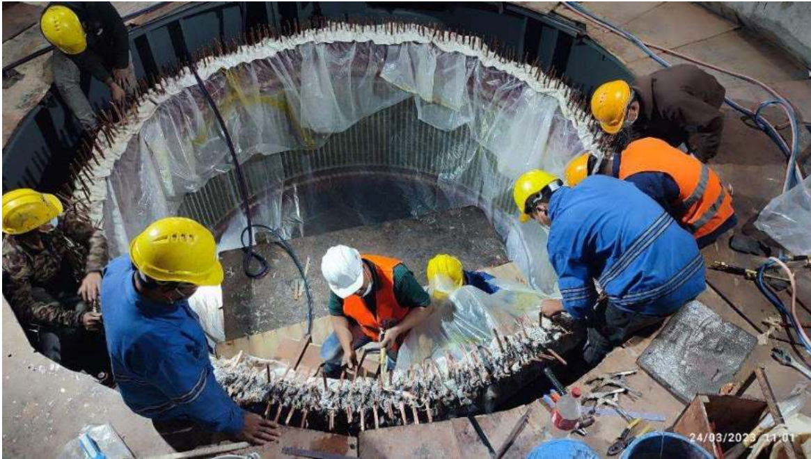
Figure 2-58: Stator coils brazing work after successful completion of Hi-Pot test
