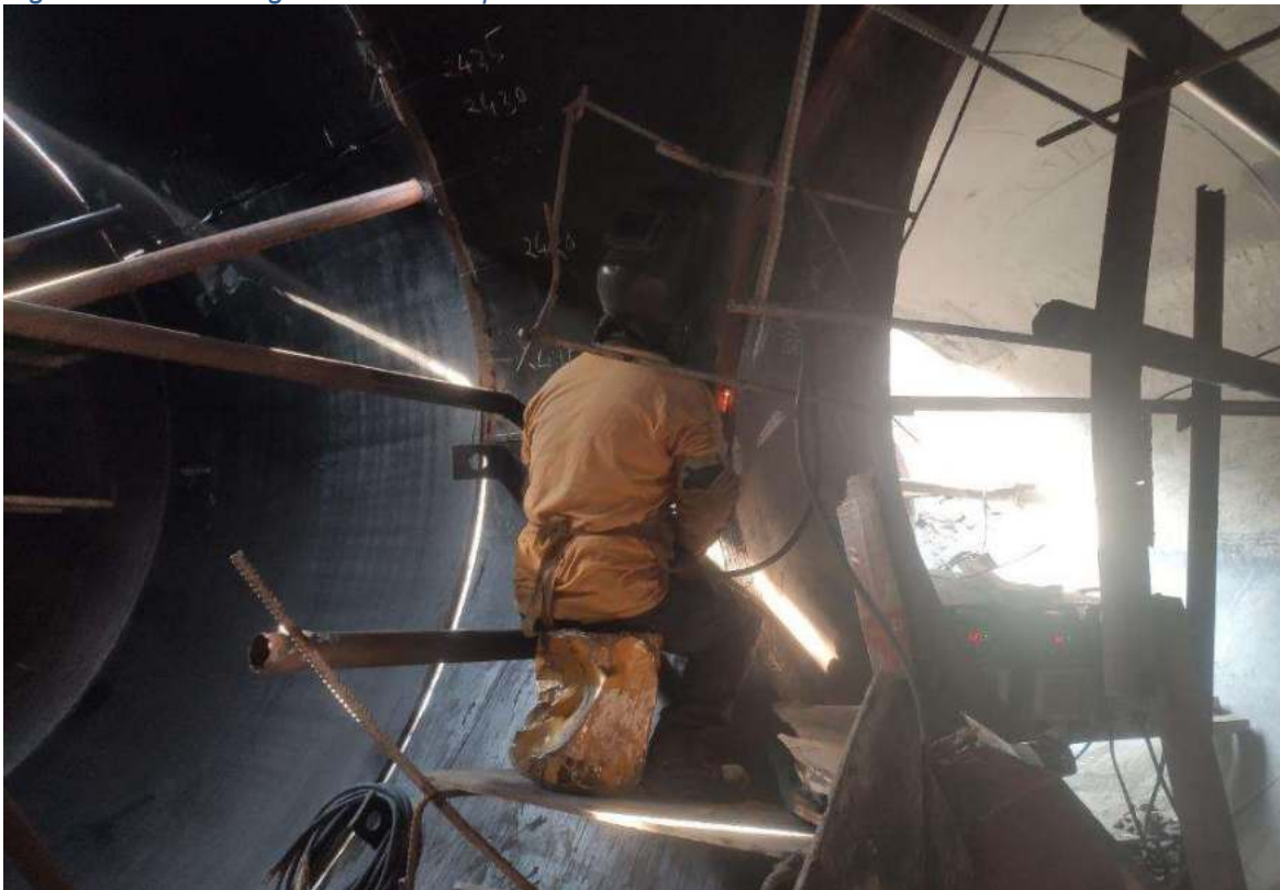
Figure 2-40: Welding at the bifurcation unit 01 at the sickle plate region
