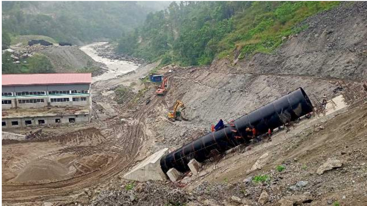
Figure 2-21: Erection of penstock pipes
