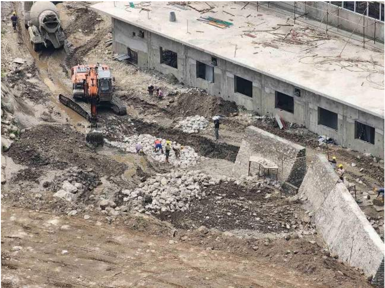
Figure 2-18: Construction of retaining wall at manifold region
