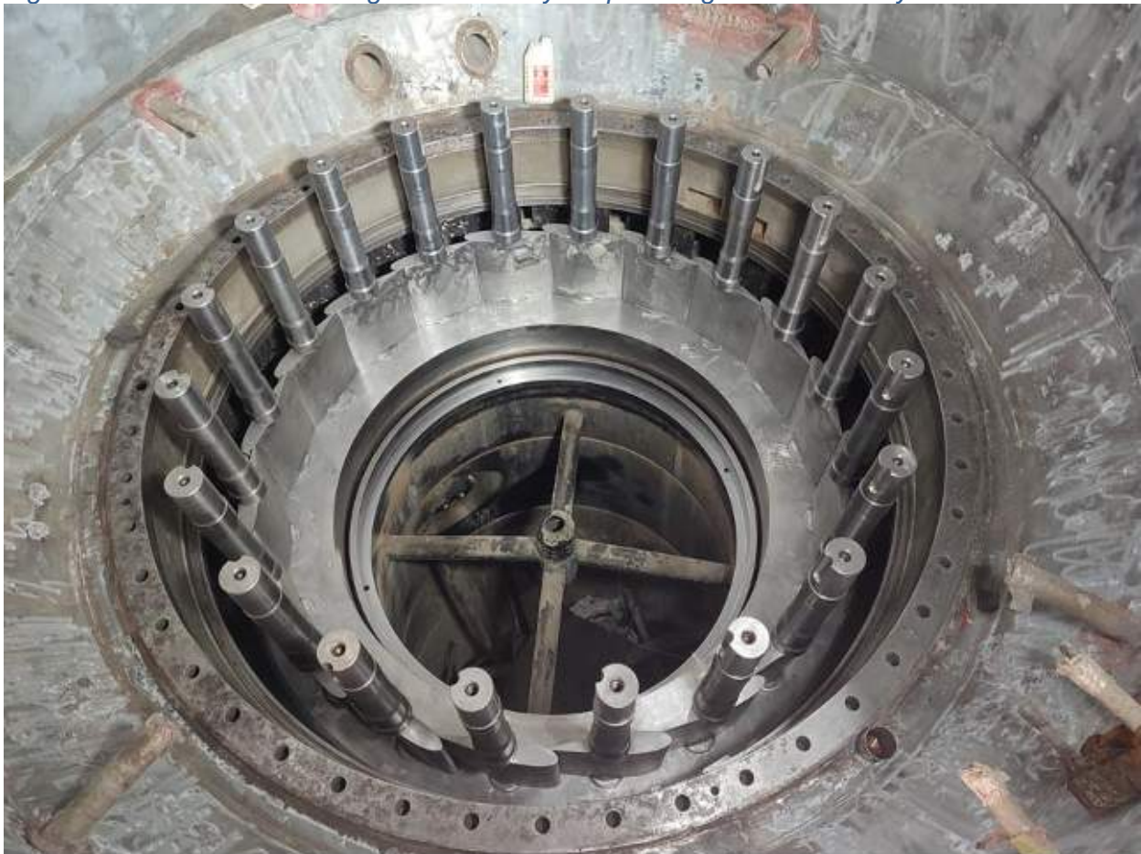
Figure 2-37: Preassembly of bottom ring and guide vane
