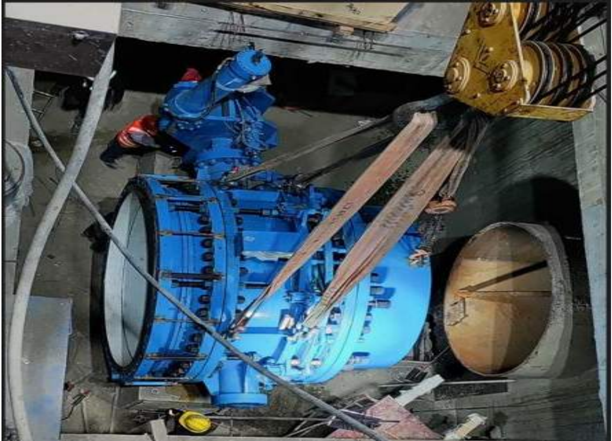
Figure 2-41: Unit 03 MIV lowered in to its position
