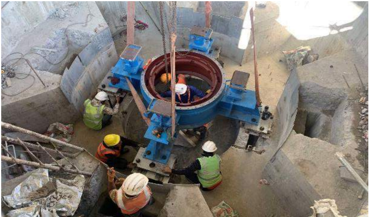
Figure 55: Installation of lower bracket in unit 1
