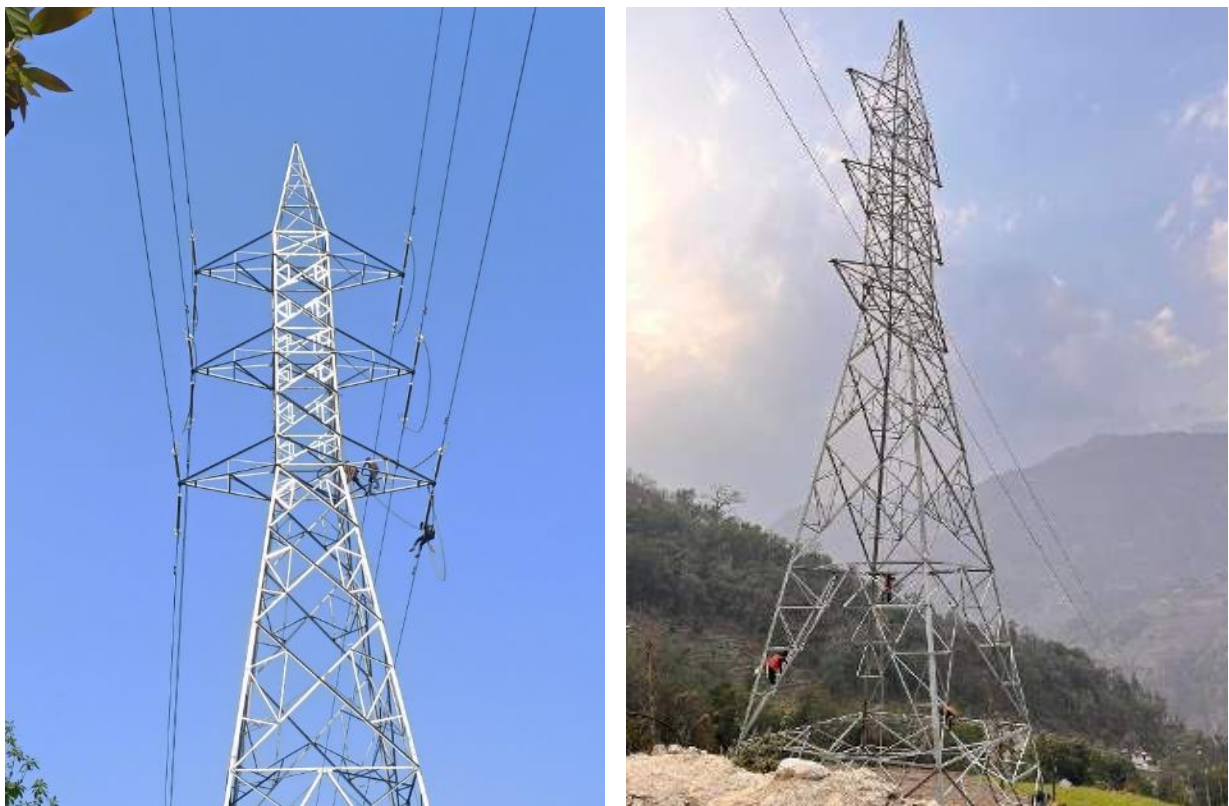
Figure 2-45: Conductor stringing works at various angle points
