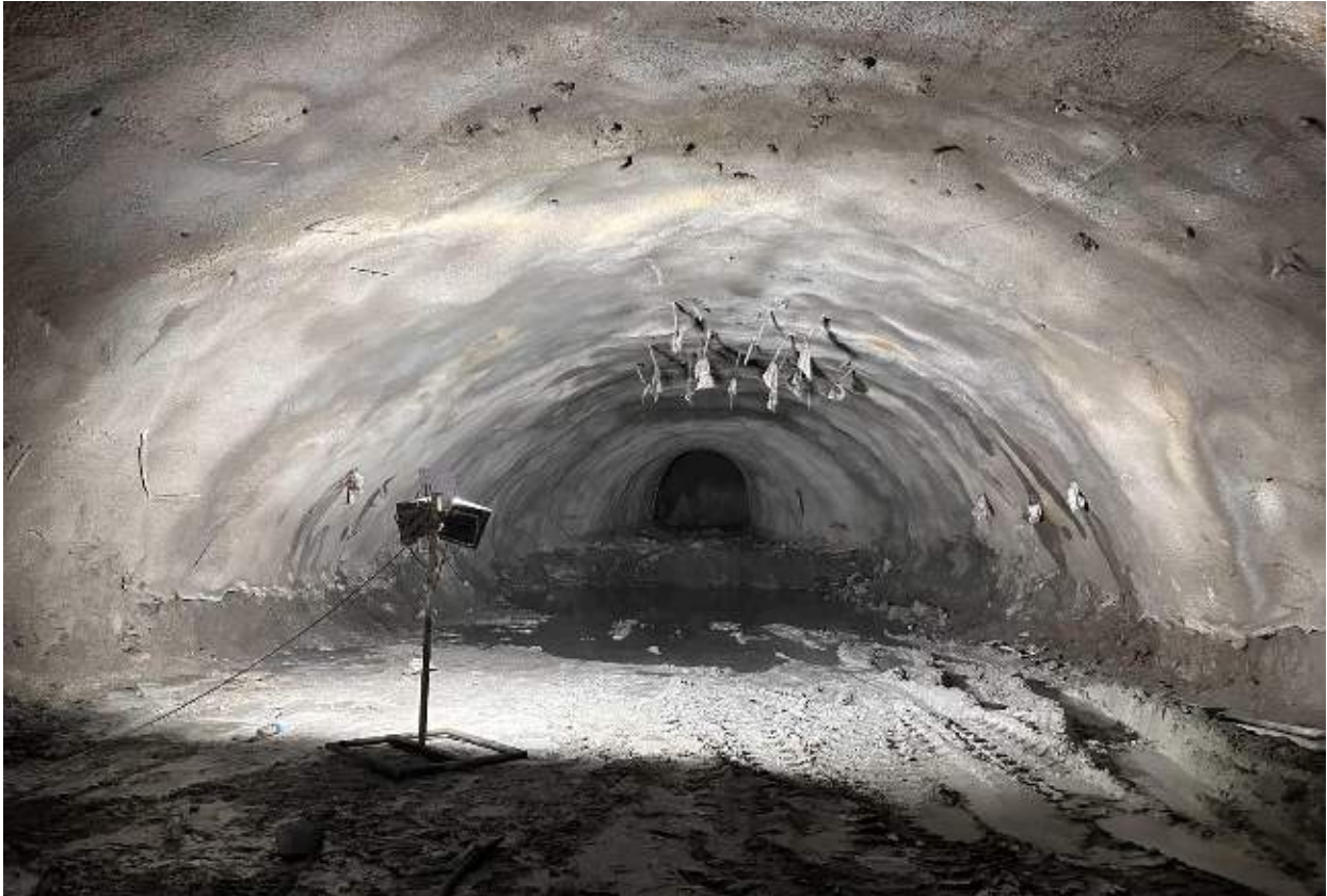
Figure 2-13: A view of SB 03 face
