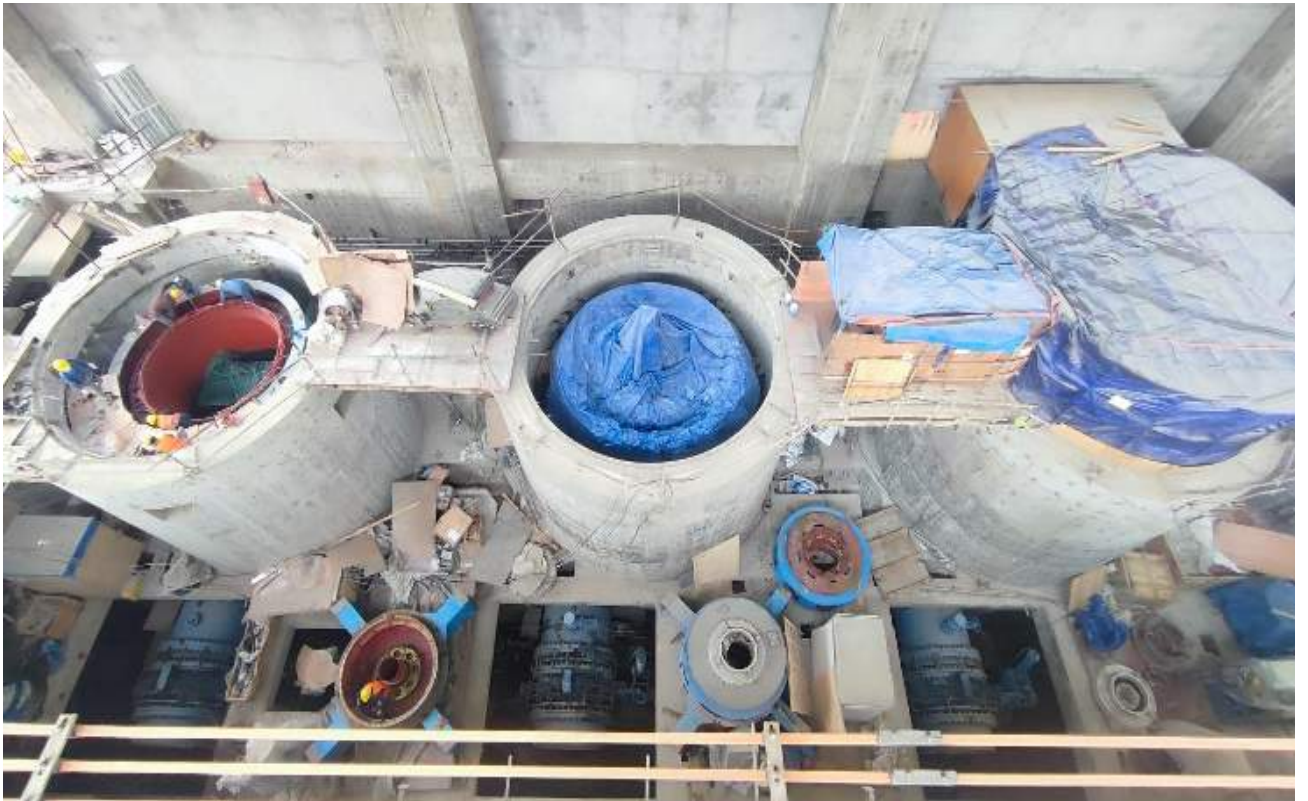
Figure 66: All 4 units M.I.V. lowered to its position
