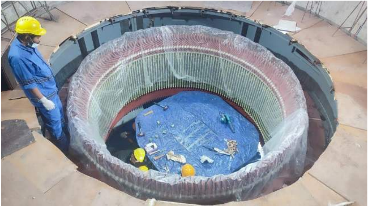
Figure 2-38: Completion of stator winding works
