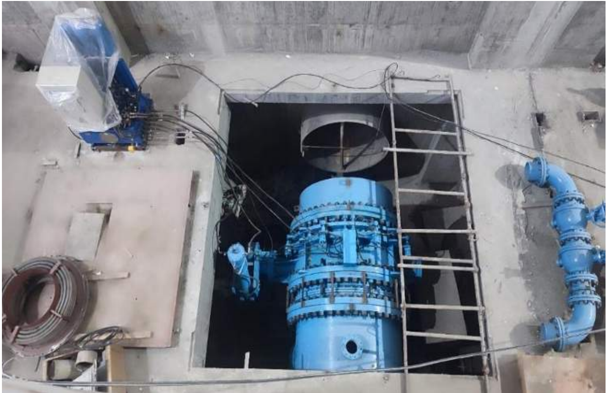
Figure 2-39: Unit 4 MIV lowered to its position
