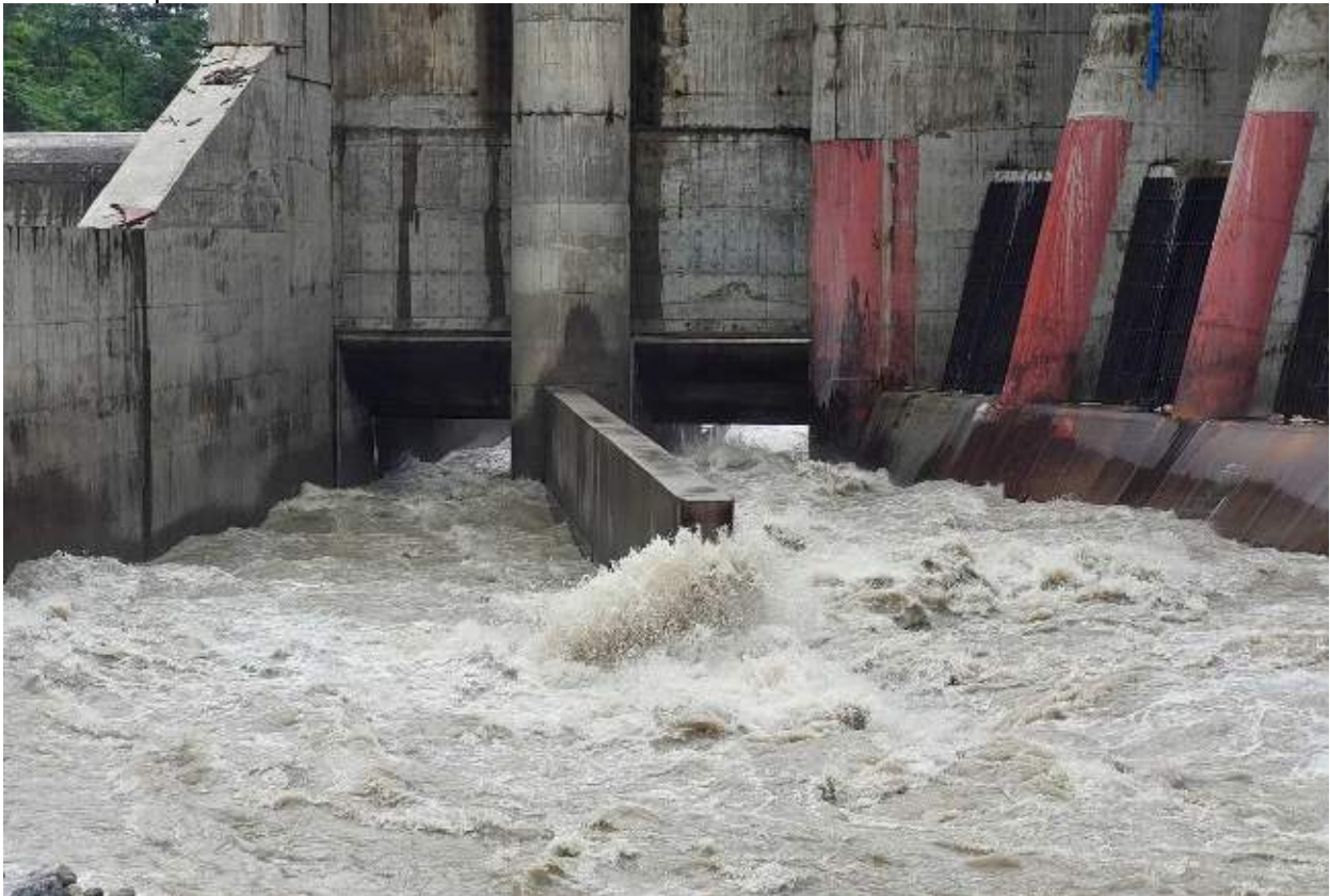
Figure 2-7: Gate installation works at undersluice
