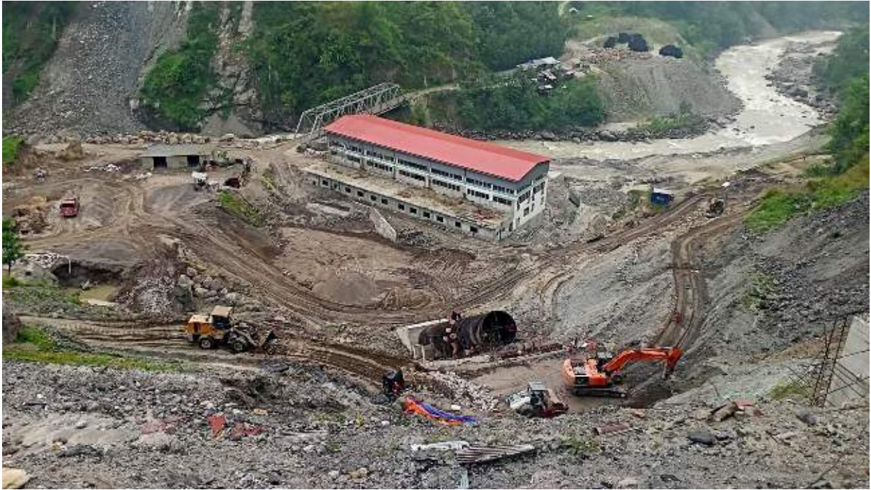
Figure 2-17: A view of backfilling works at the manifold region
