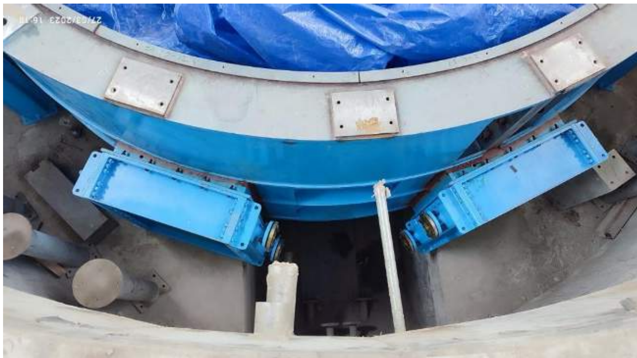
Figure 2-35: Final assembly of stator air cooler
