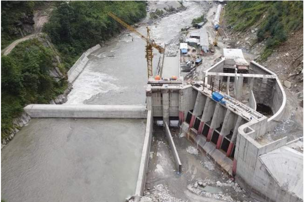
Figure 2-4: Aerial view of Headworks
