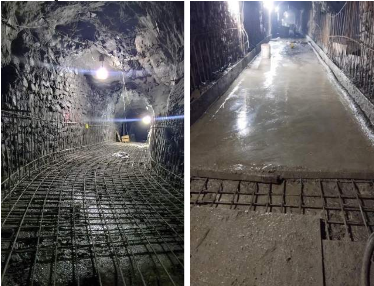
Figure 2-16: A view of rebar layout at the flushing tunnel
