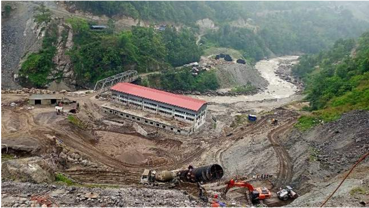
Figure 2-22: Simultaneous work progress with Civil works
