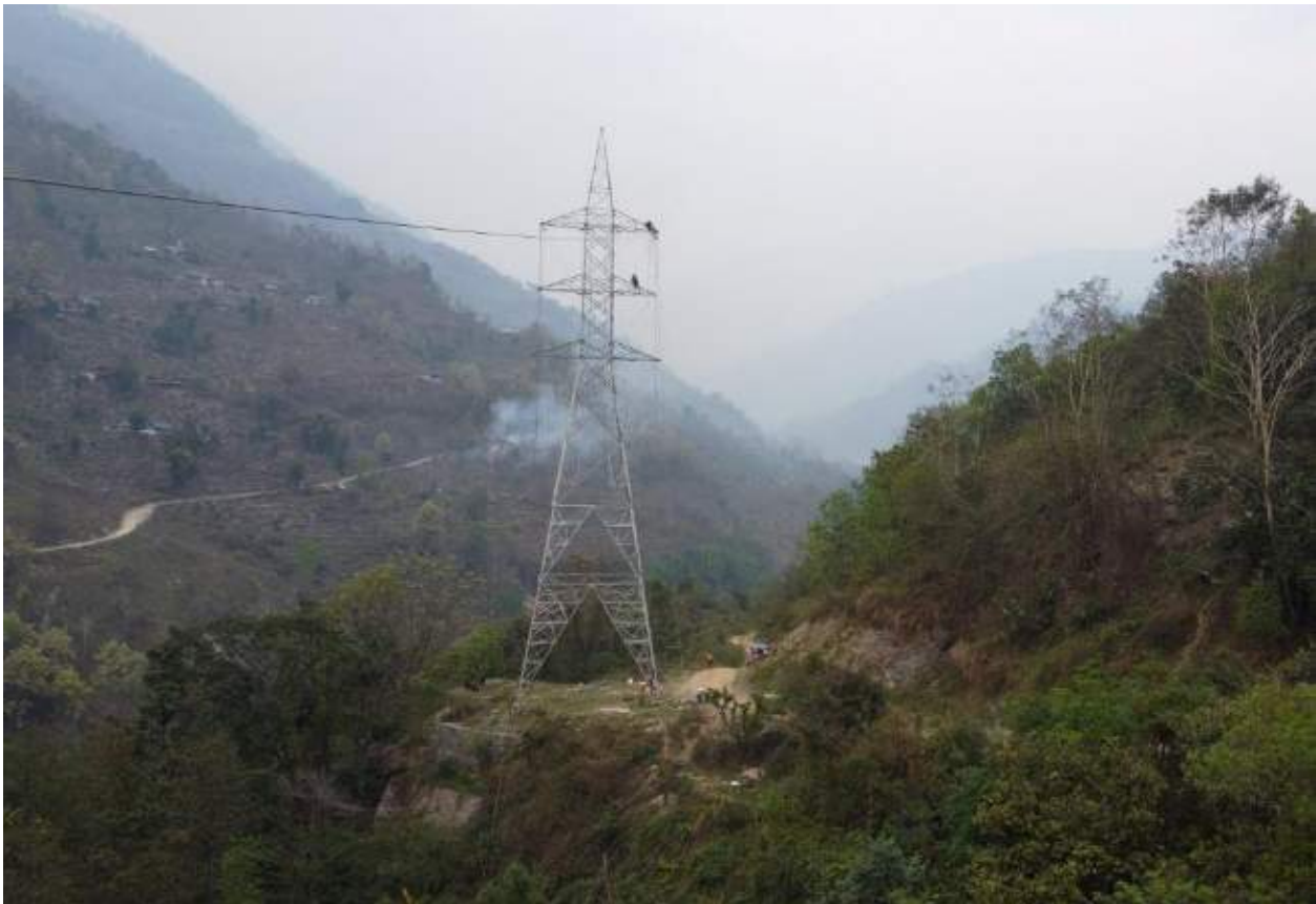
Figure 2-44: A view of stringing works
