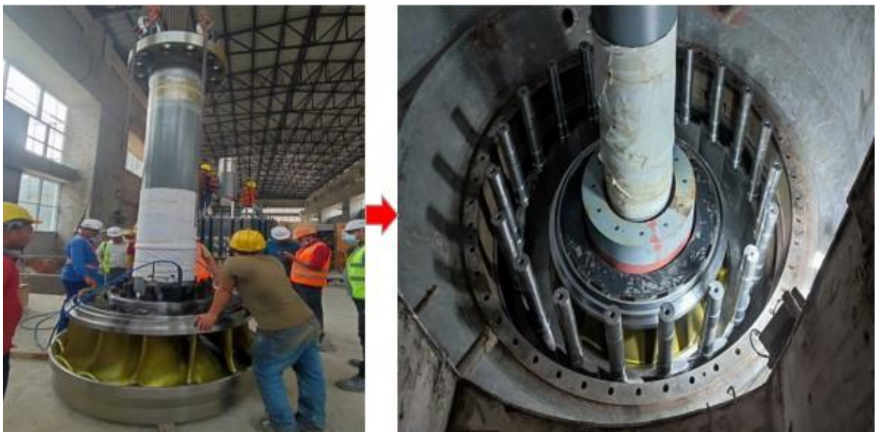
Figure 64: Final assembly of runner with main shaft
