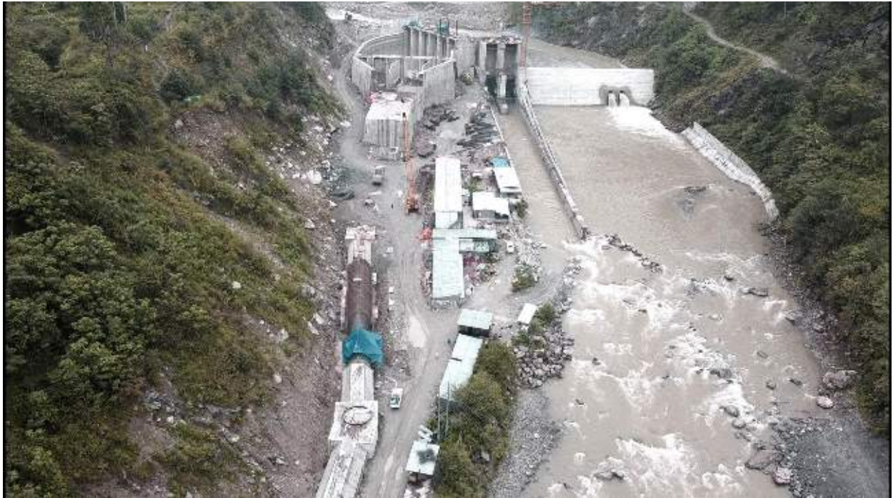
Figure 2-9: Erection of approach pipe
