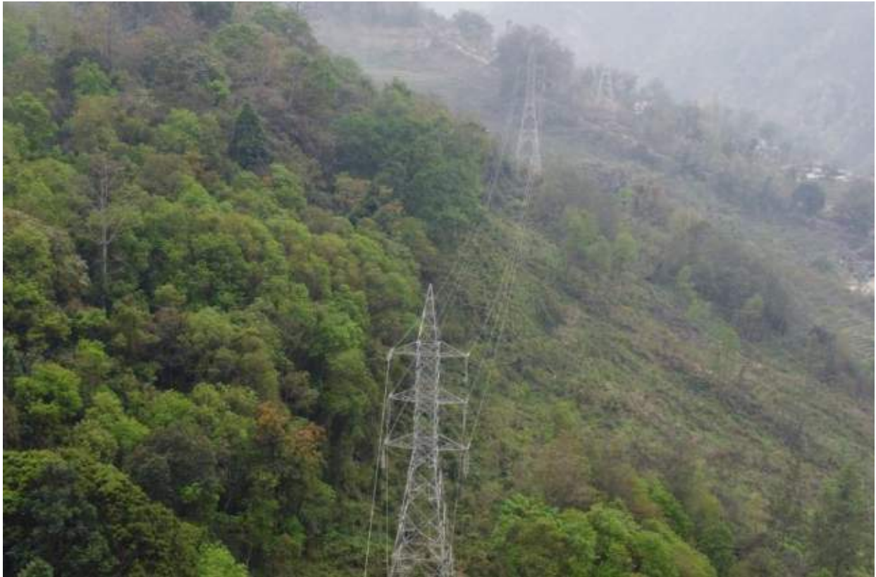
Figure 58: A view of Stringing works completed between two angle points
