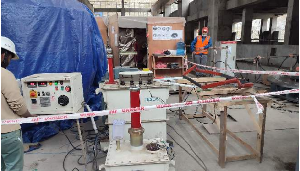
Figure 54: High voltage test of stator coil
