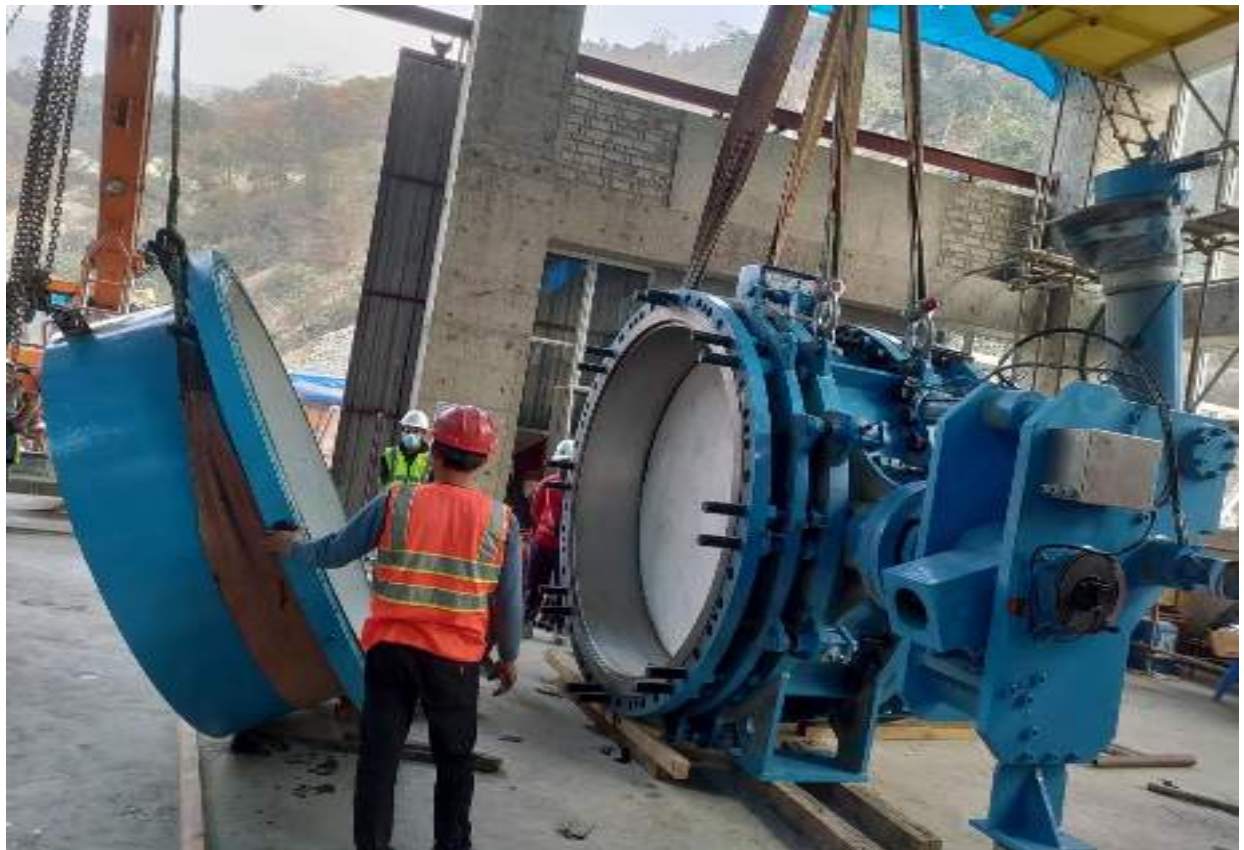
Figure 2-40: Unit 2 MIV assembled at Service bay
