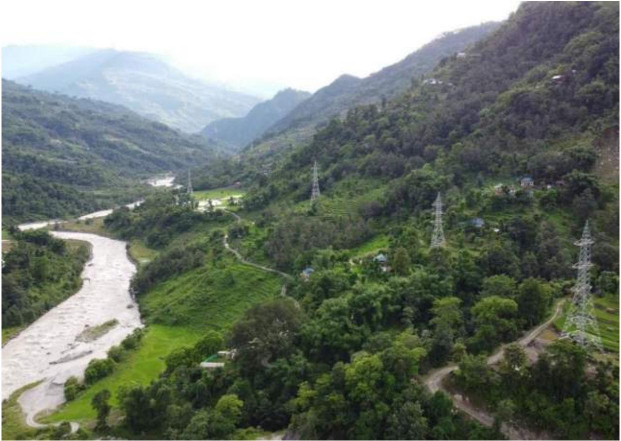
Figure 2-43: View of erected towers from right bank of Tamor
