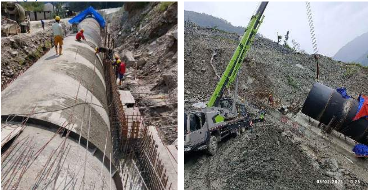
Figure 2-23: Erection of hydraulic hoisting cylinders of radial gate (left) and radial gates of intake side (right)
