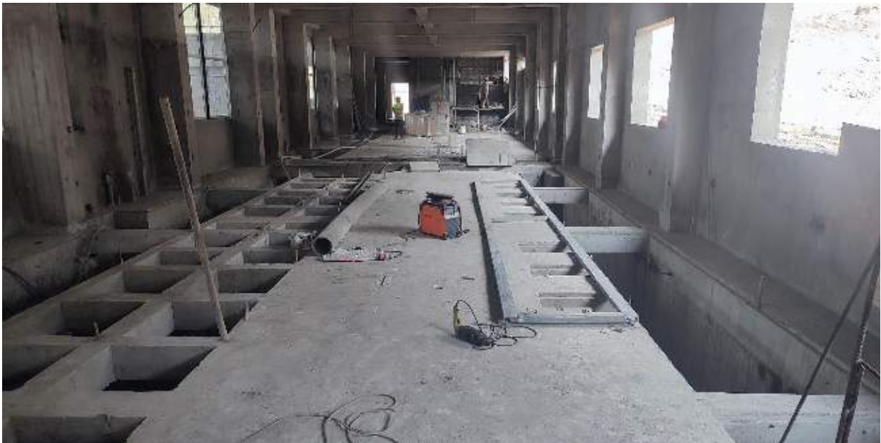
Figure 70: Installation of channels for panel board foundation
