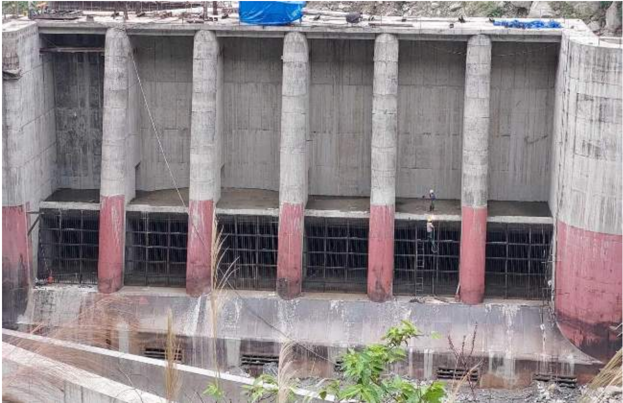
Figure 2-5: A front view of intake orifices
