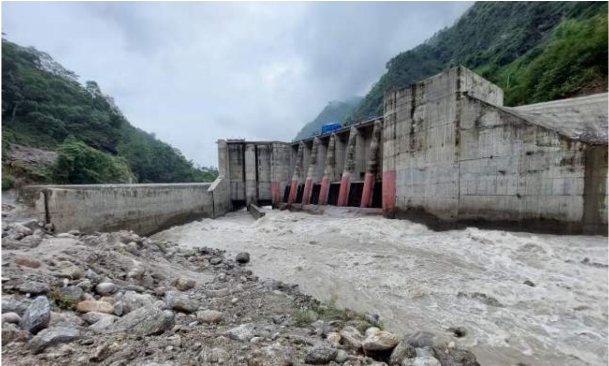
Figure 2-6: A view of weir and undersluice from upstream
