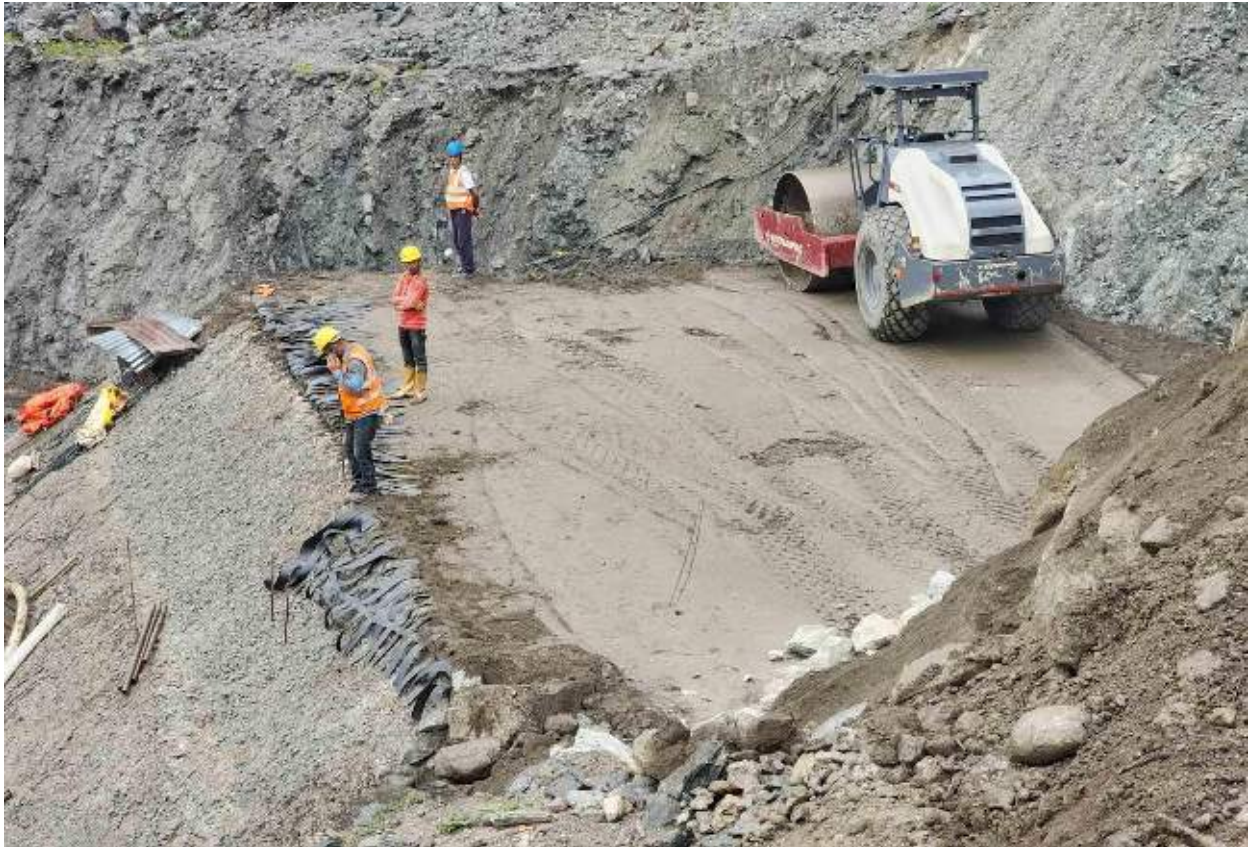
Figure 2-19: Backfilling works along penstock alignment
