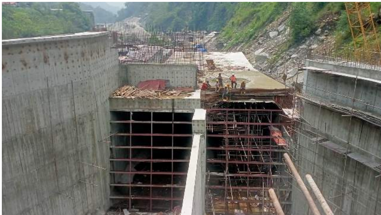
Figure 2-8: Final stage concreting works at the conveyance tank right top slab
