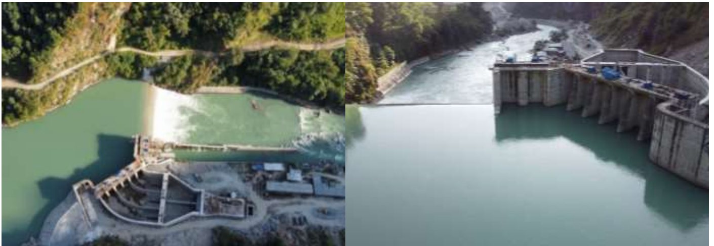
Figure 2-3: An aerial view of weir with flow over the ogee crest (left) and Current view of headworks (right)
