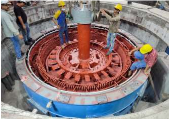
Figure 2-20: Rotor and stator coupling in unit 01 (left) and final installation of water guide mechanism along with monitoring sensors (right)
