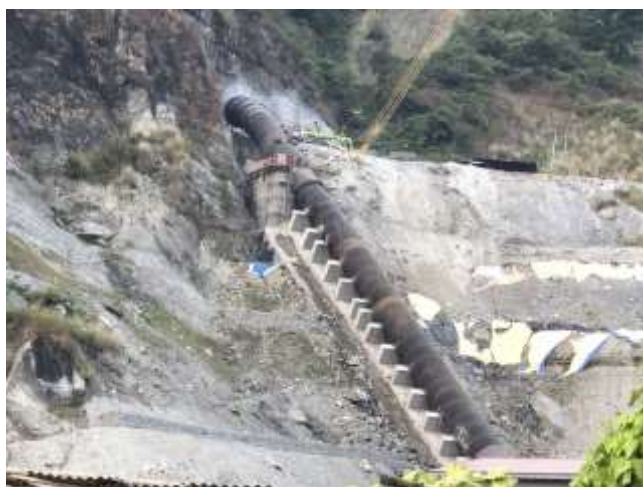
Figure 2-18: Erection of penstock pipes (left) and the PPV locatio (right)
