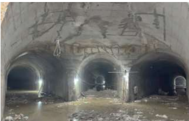
Figure 2-10: Full lining concrete at connecting tunnel junction
