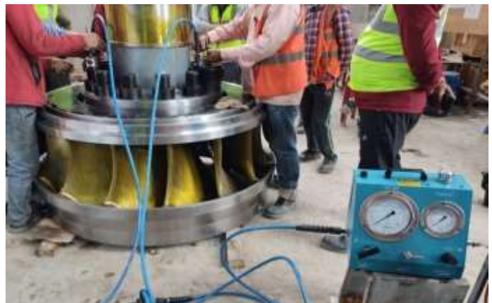
Figure 2-22: Rotor lowering in unit 4 (left) and assembly of runner with main shaft (right)
