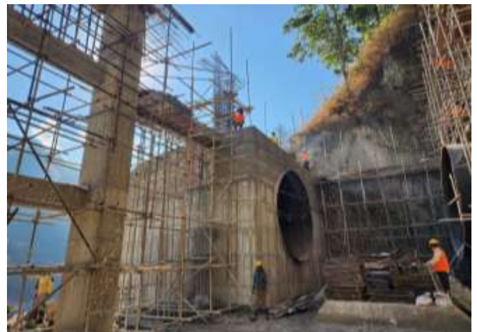
Figure 2-15: A view of switchyard with 4 power transformers positioned (left) and construction of anchor block and valve house (right)
