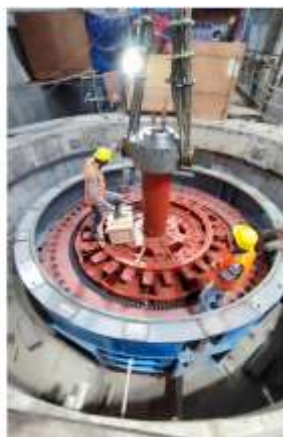
Figure 2-22: Rotor lowering in unit 4 (left) and assembly of runner with main shaft (right)
