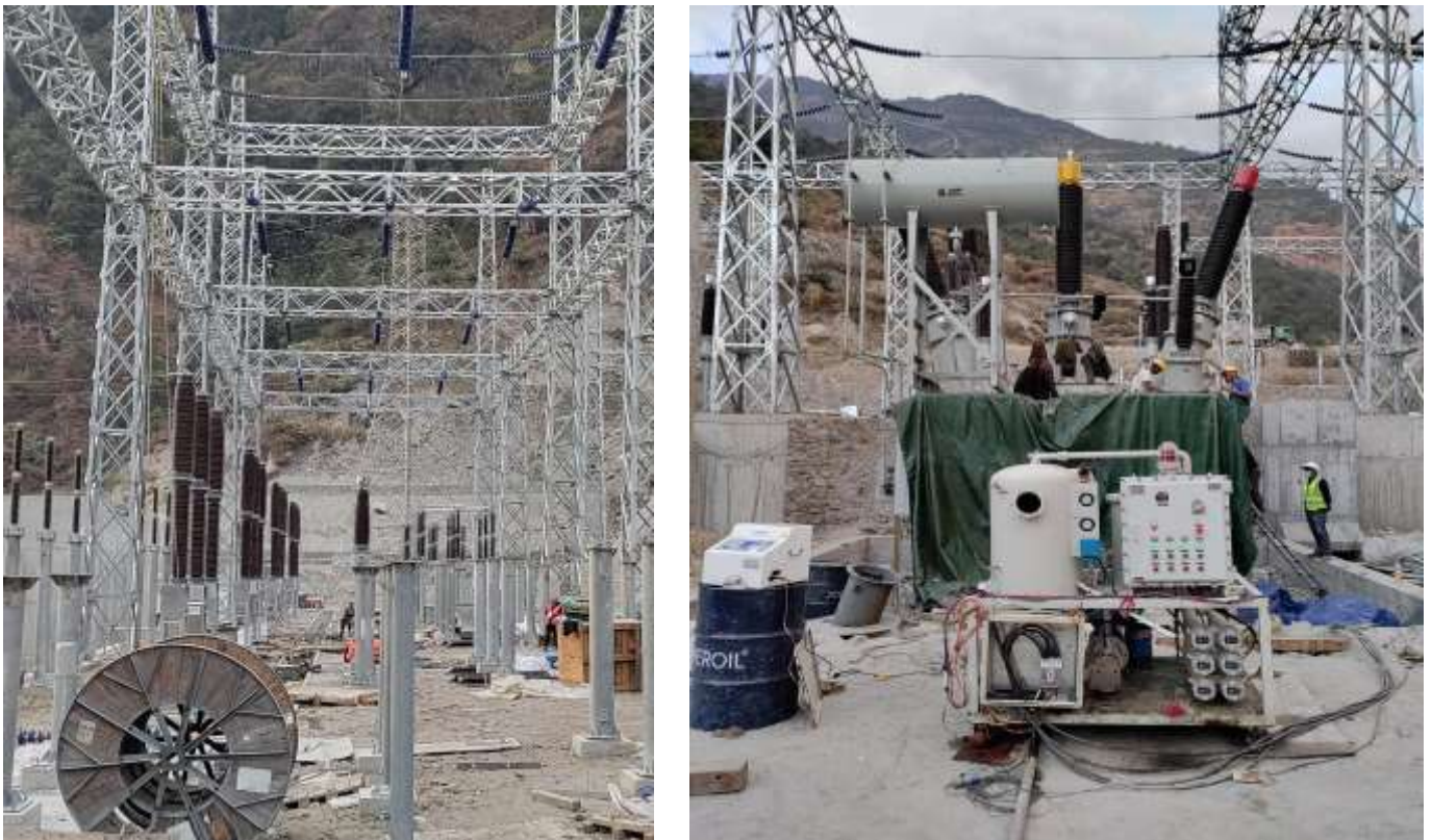
Figure 2-25: Erection of gantry towers and final assembly of Transformer at switchyard
