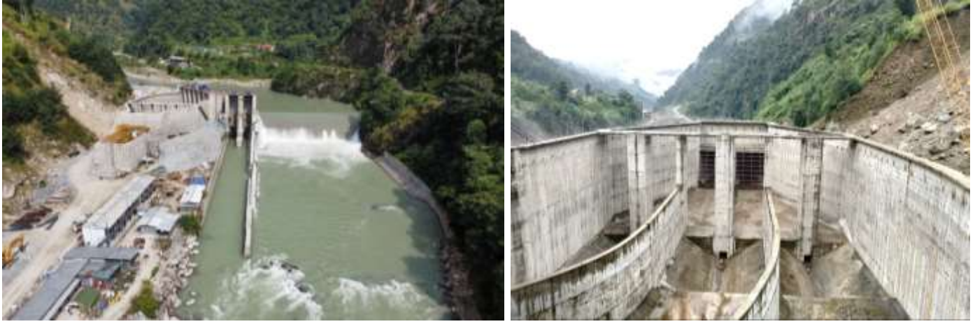
Figure 2-2: Aerial view of Headworks from the downstream (left) and A view of gravel trap and conveyance tank from upstream (right)
