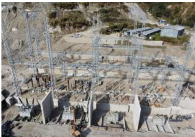
Figure 2-15: A view of switchyard with 4 power transformers positioned (left) and construction of anchor block and valve house (right)
