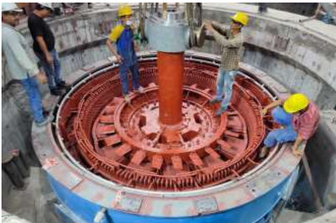
Figure 2-23: Rotor lowering of unit 04 (left) and Unit 02 MIV valve assembly and erection (right)
