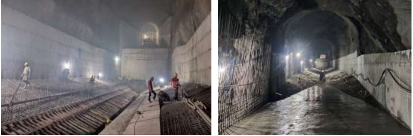
Figure 2-9: A view of SB 03 during concrete works
