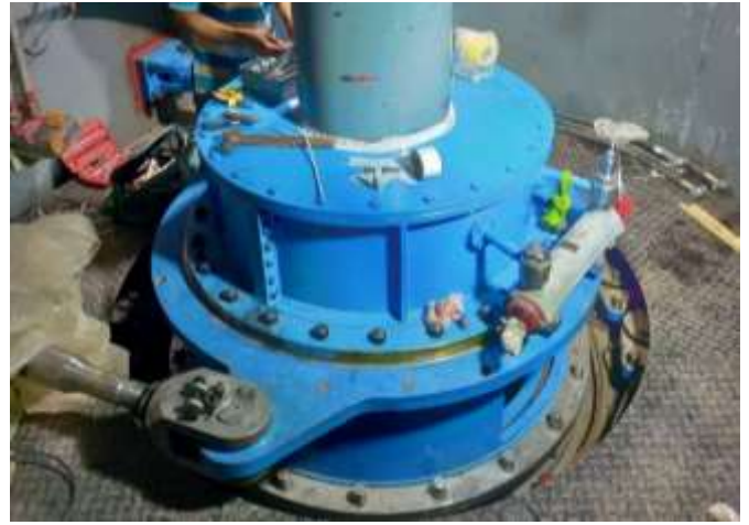
Figure 2-20: Rotor and stator coupling in unit 01 (left) and final installation of water guide mechanism along with monitoring sensors (right)
