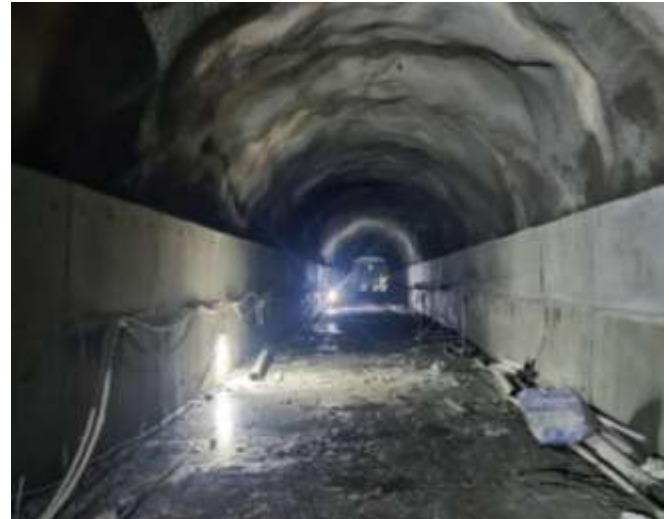
Figure 2-8: A view of SB 02 after the completion of concreting works (left) and a view of approach tunnel 02 (right)
