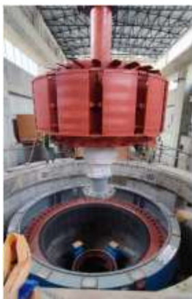
Figure 2-22: Rotor lowering in unit 4 (left) and assembly of runner with main shaft (right)
