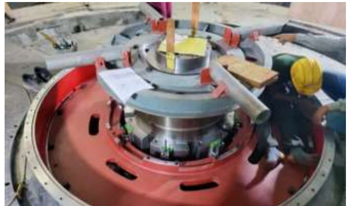
Figure 2-21: Brazing and lacing work of stator coils in Unit 02 (left) and run-out check of shaft Unit 03 (right)
