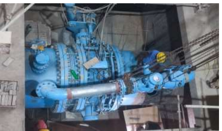
Figure 2-23: Rotor lowering of unit 04 (left) and Unit 02 MIV valve assembly and erection (right)
