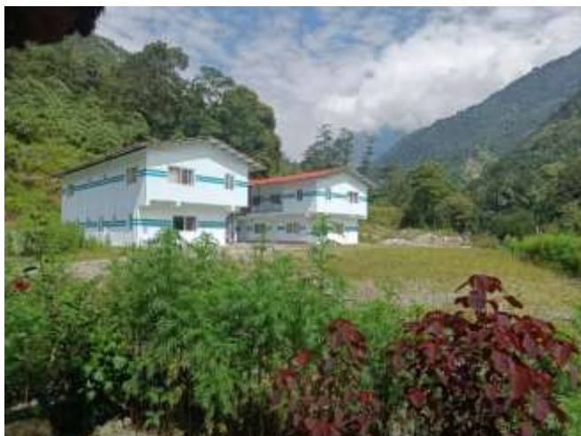
Figure 2-1: Construction of new residential camp building at the powerhouse
