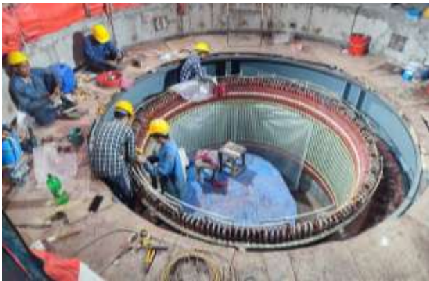
Figure 2-21: Brazing and lacing work of stator coils in Unit 02 (left) and run-out check of shaft Unit 03 (right)
