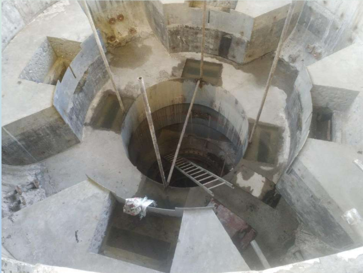
Generator casing at Unit 02
