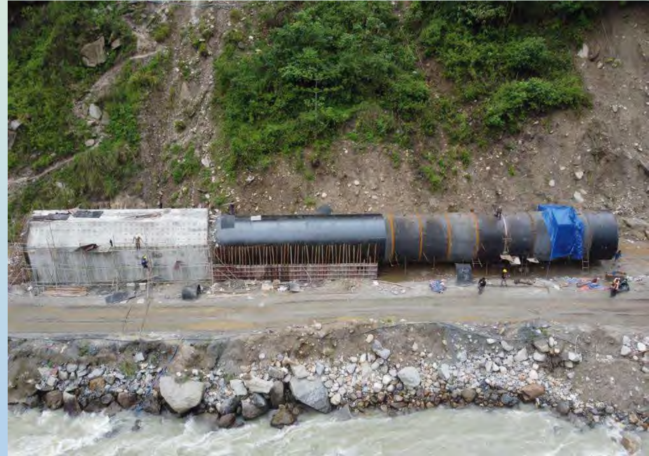
Erection of approach pipes
