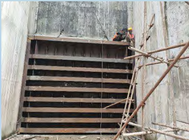
Erection work at Unit 1 of Intake Gate
