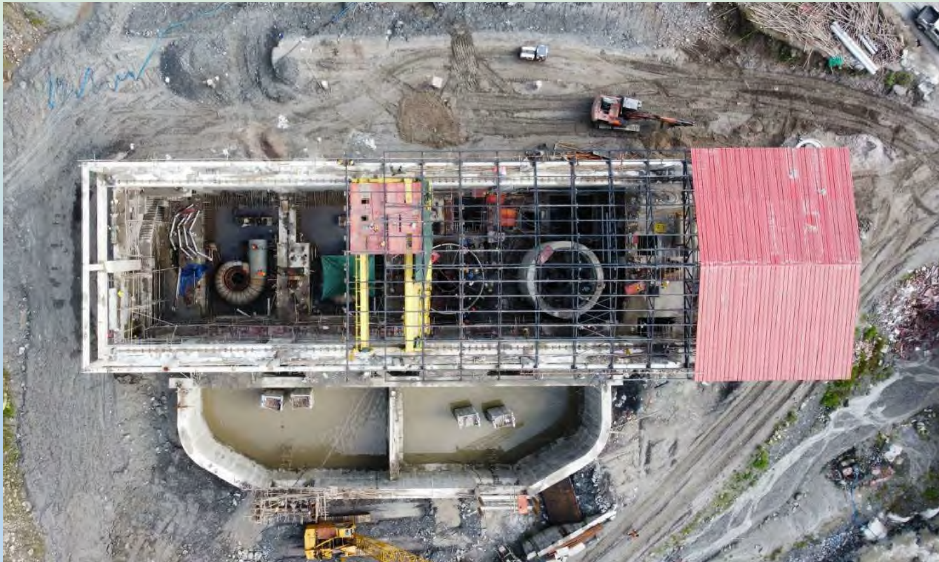
An aerial view of Powerhouse after installation of spiral casing
