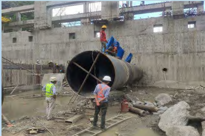
Erection work(Unit 1) (Dia: 2.0 m and thk: 20 mm)
