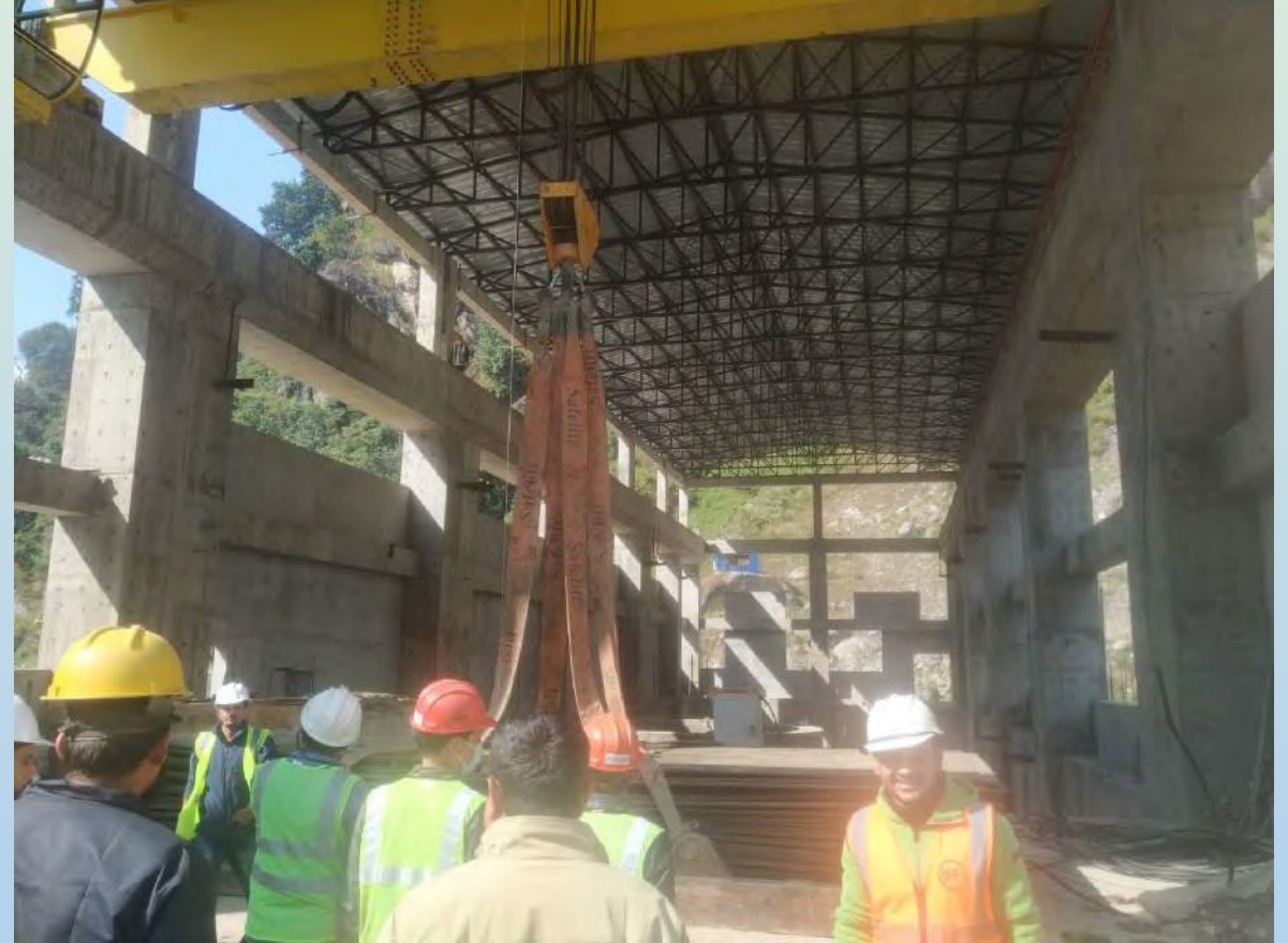
Static load testing of EOT crane
