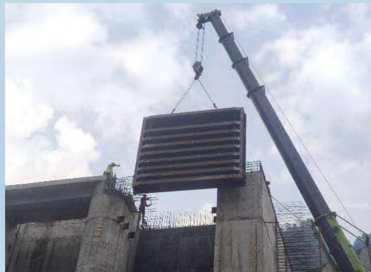
Erection of Intake gate
