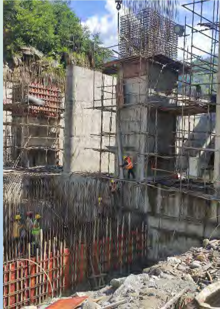
Erection of air vent pipe at gravel flushing Unit 3 (Dia. 200 mm)
