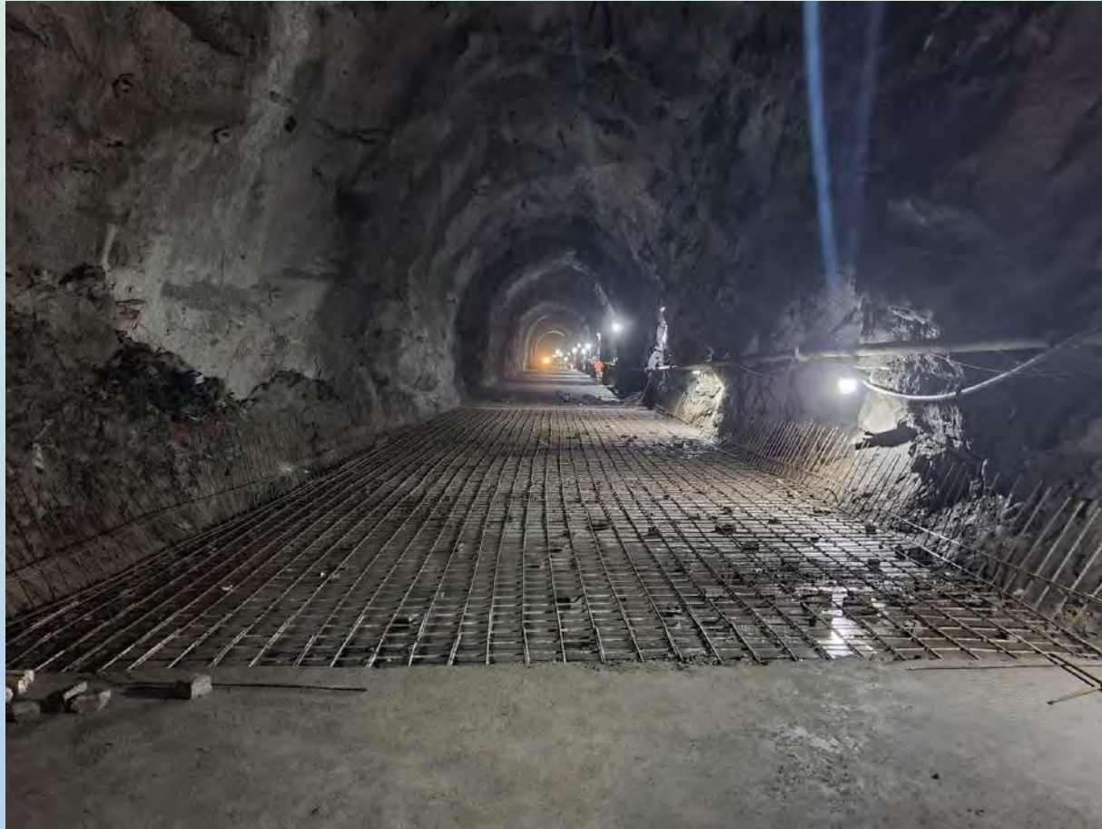
Invert lining works at HRT
