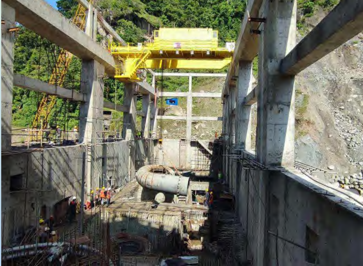
EOT crane being commissioned with the medium load
