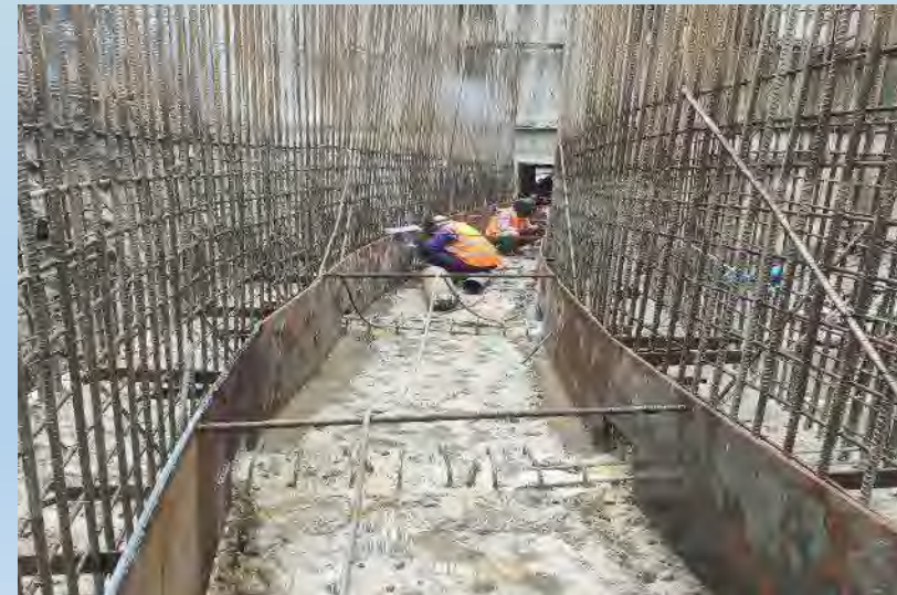
Steel lining works at gravel flushing culvert (thk: 12 mm)
