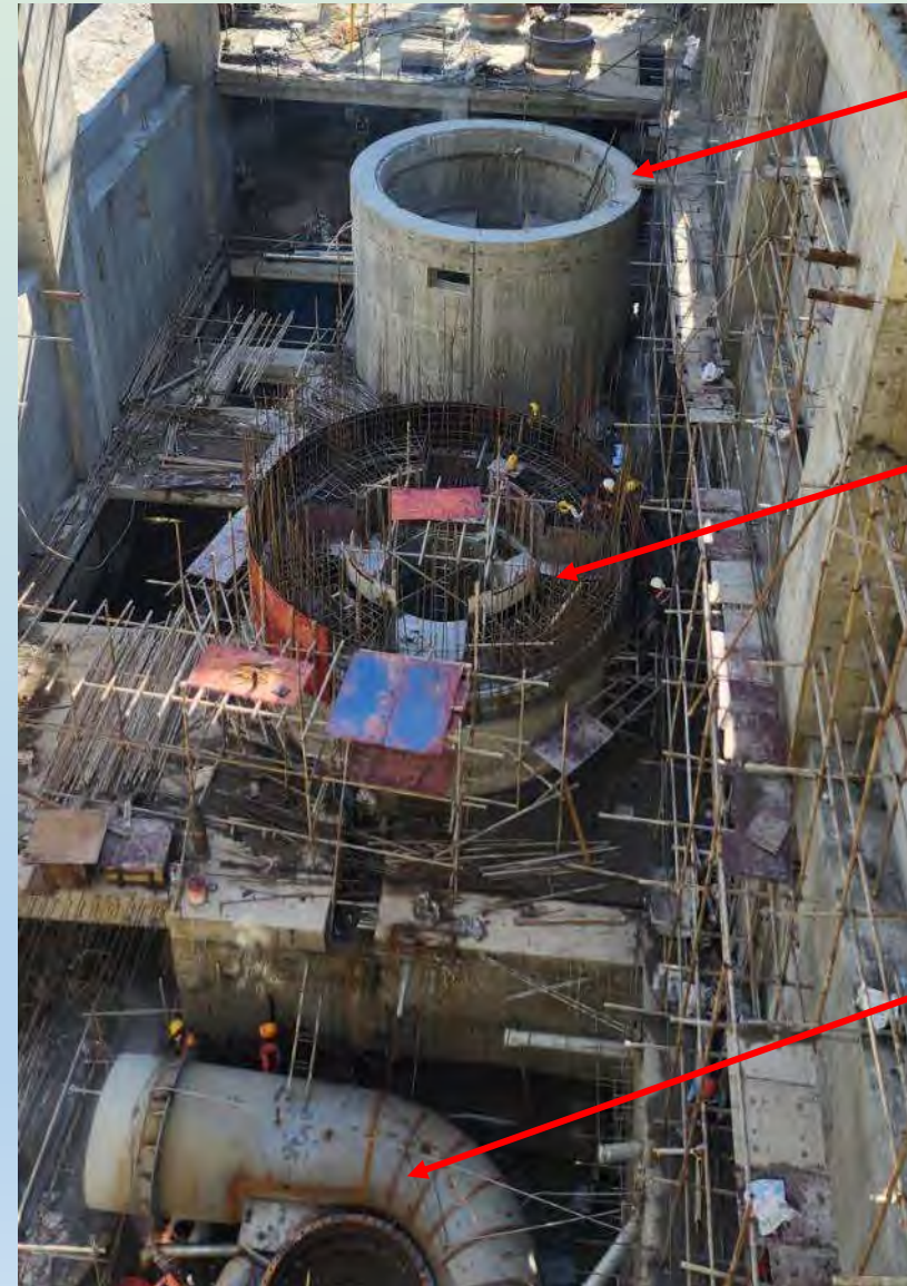
Unit 01 (Generator casing)
