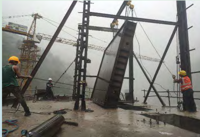
Lifting of intake gate Unit 2 for erection
