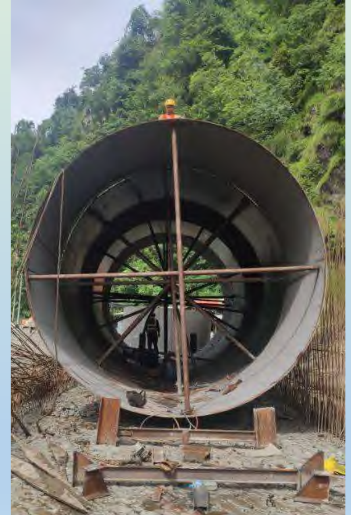
Erection of approach pipe and simultaneous concreting
