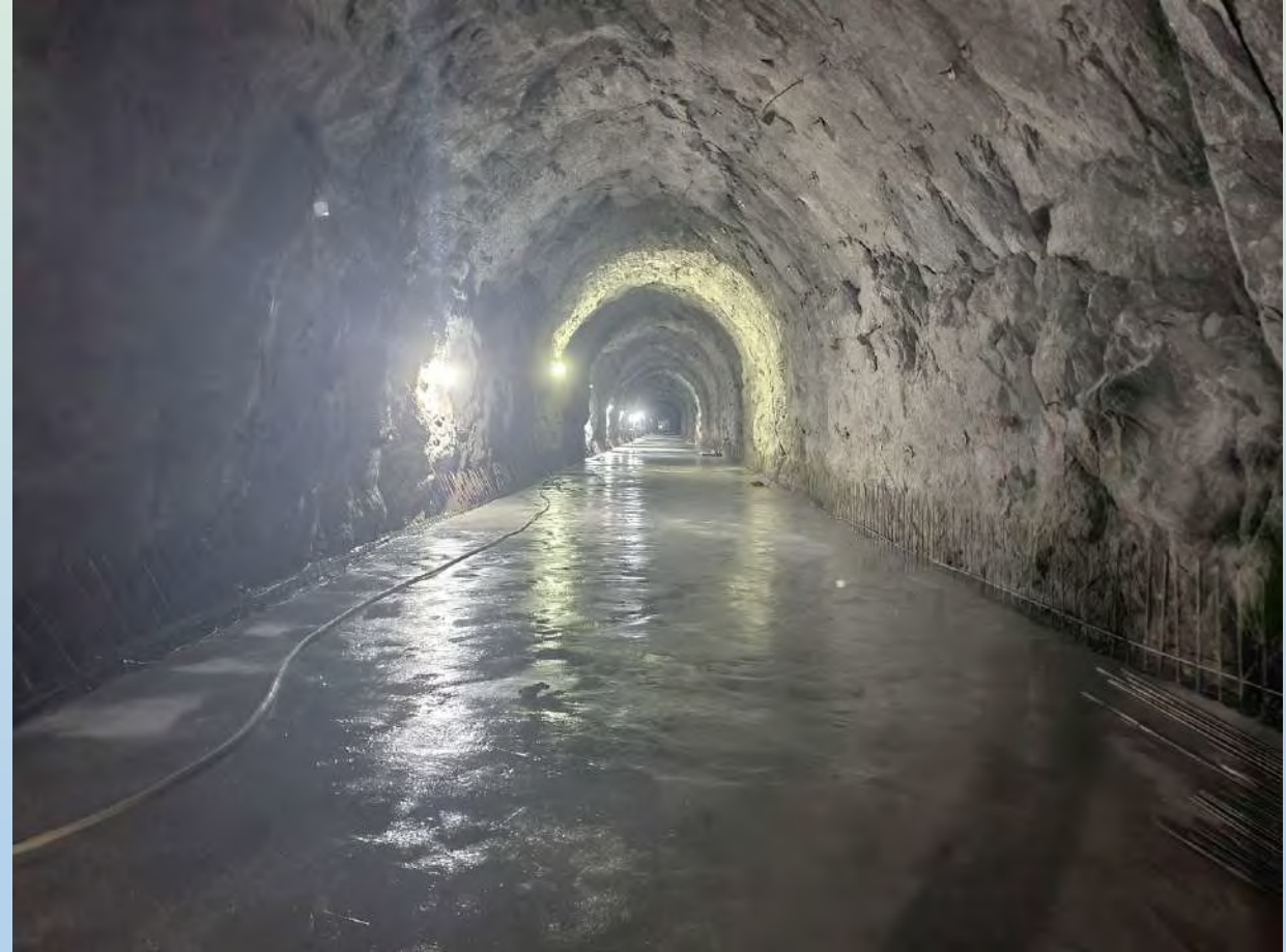
Invert lining works at HRT
