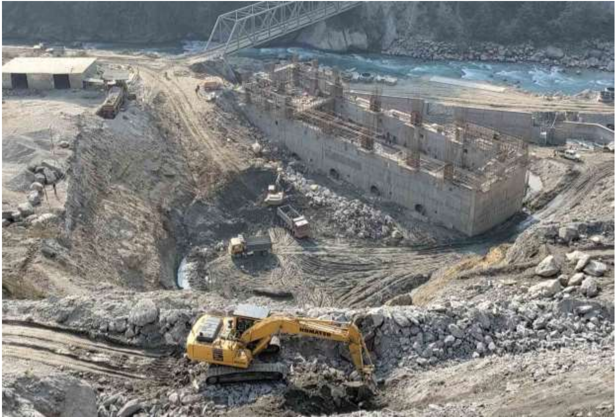
Figure 24: View of excavation works for penstock
