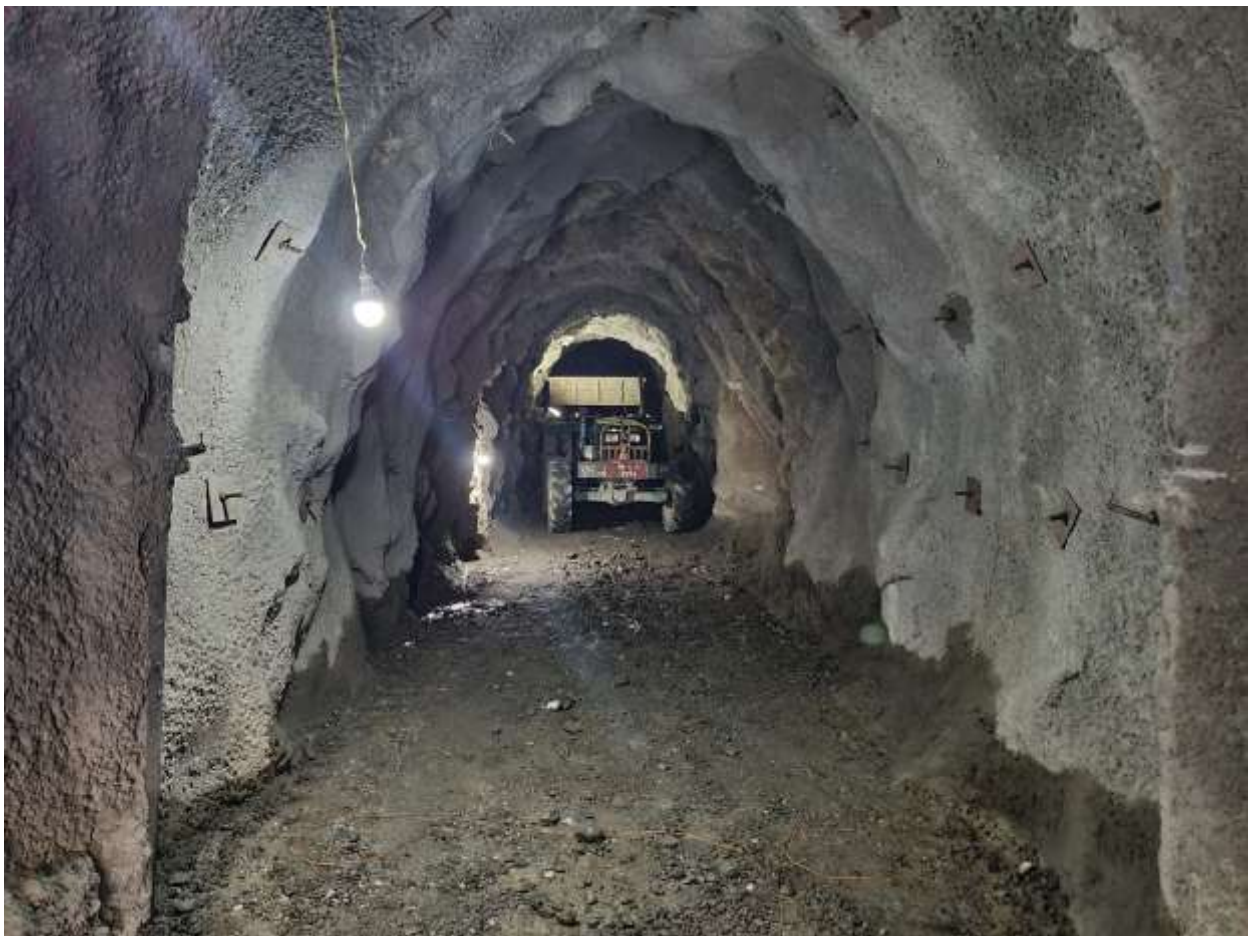
Figure 20: Excavation works at flushing tunnel
