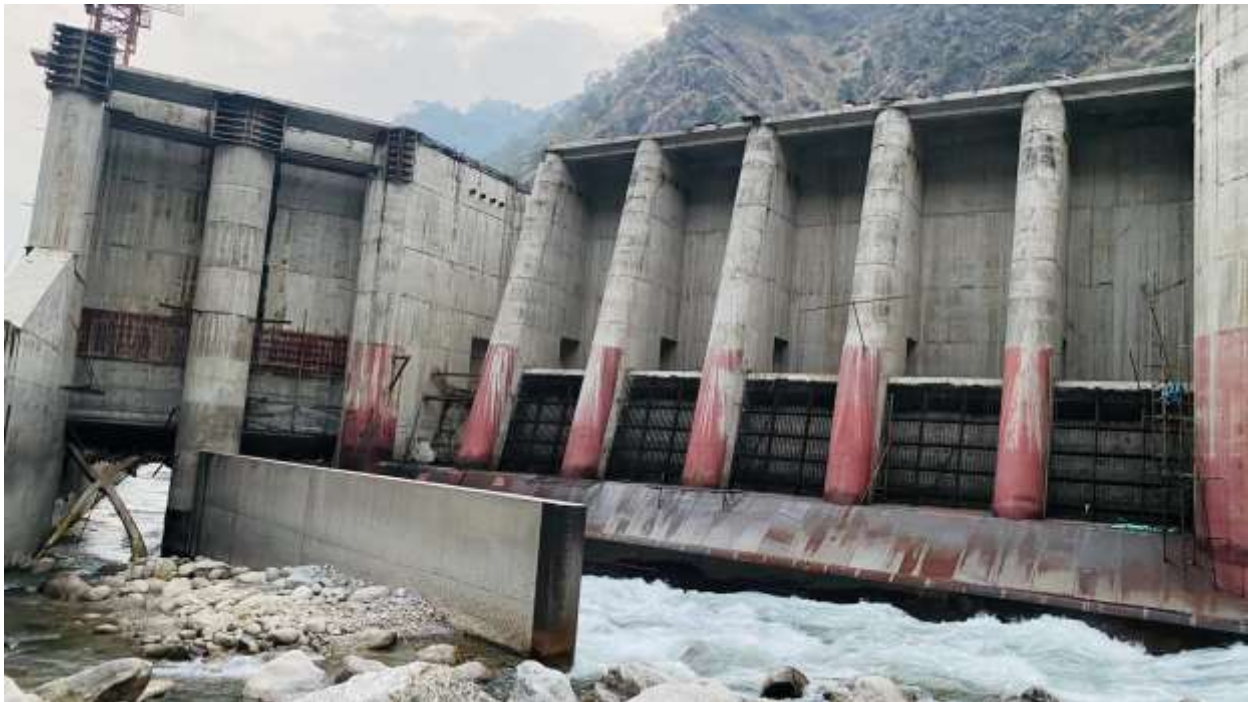
Figure 8: Intake and Undersluice section from upstream
