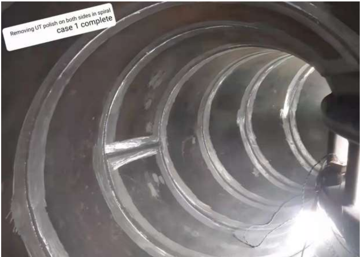
Figure 52: Surface being readied for Ultrasonic test
