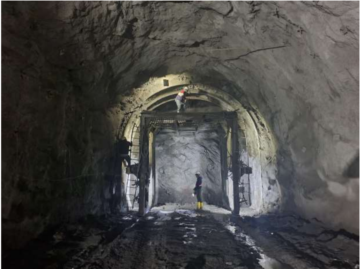
Figure 21: A view of HRT from Outlet
