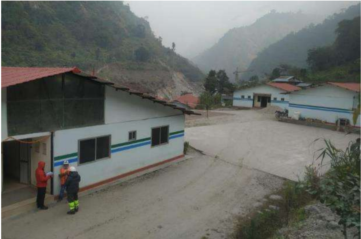
Figure 5: Employer's residential camp at Headworks (Simle)
