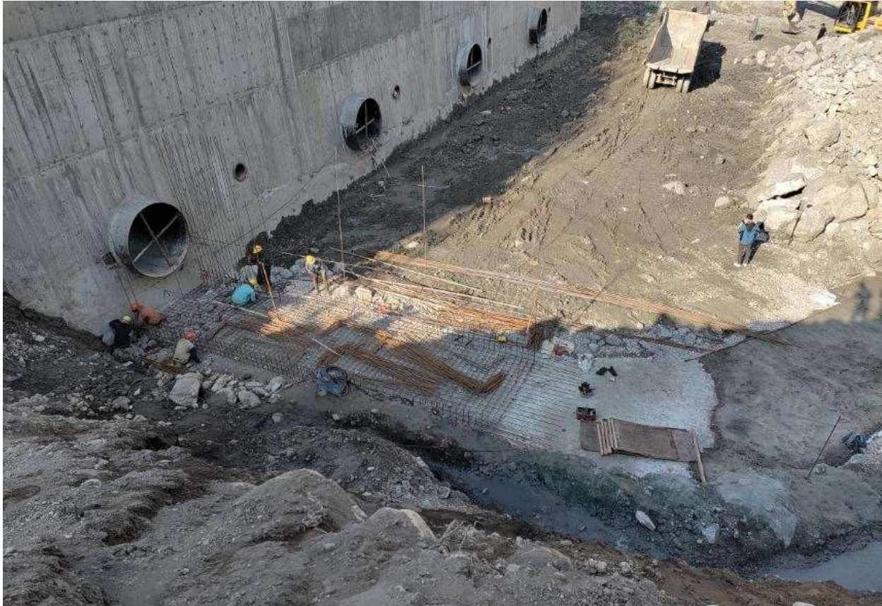
Figure 25: Concreting works for the installation of branch pipes of penstock
