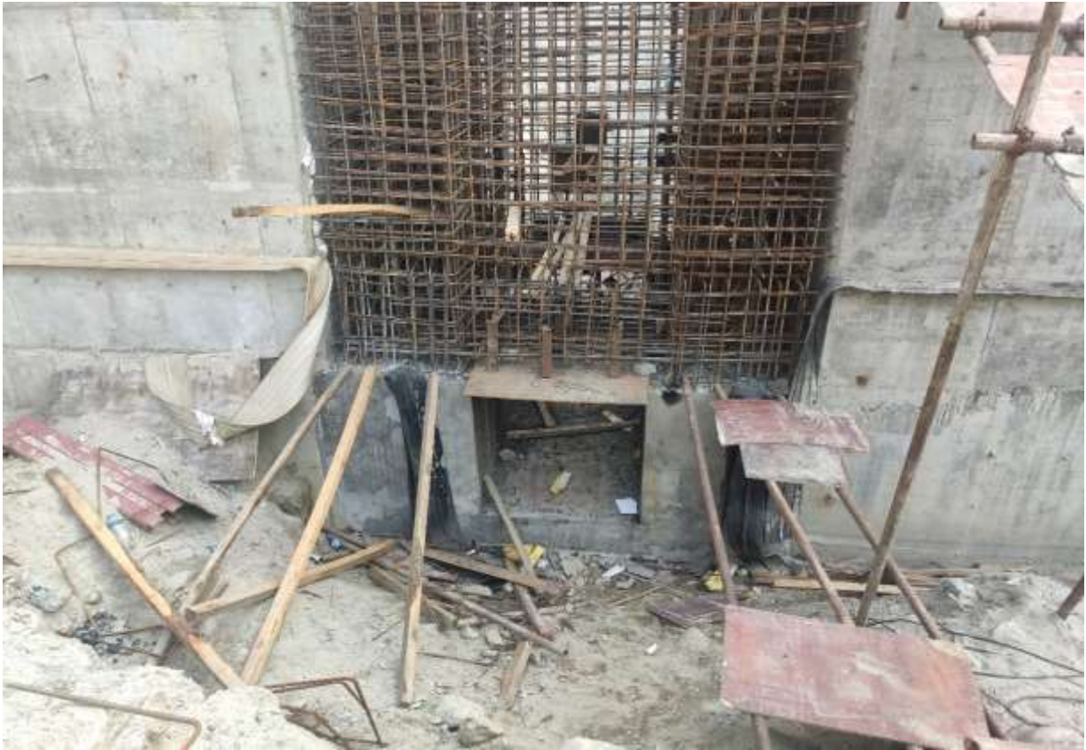
Figure 37: Completion of gated section 2 at gravel flushing culvert
