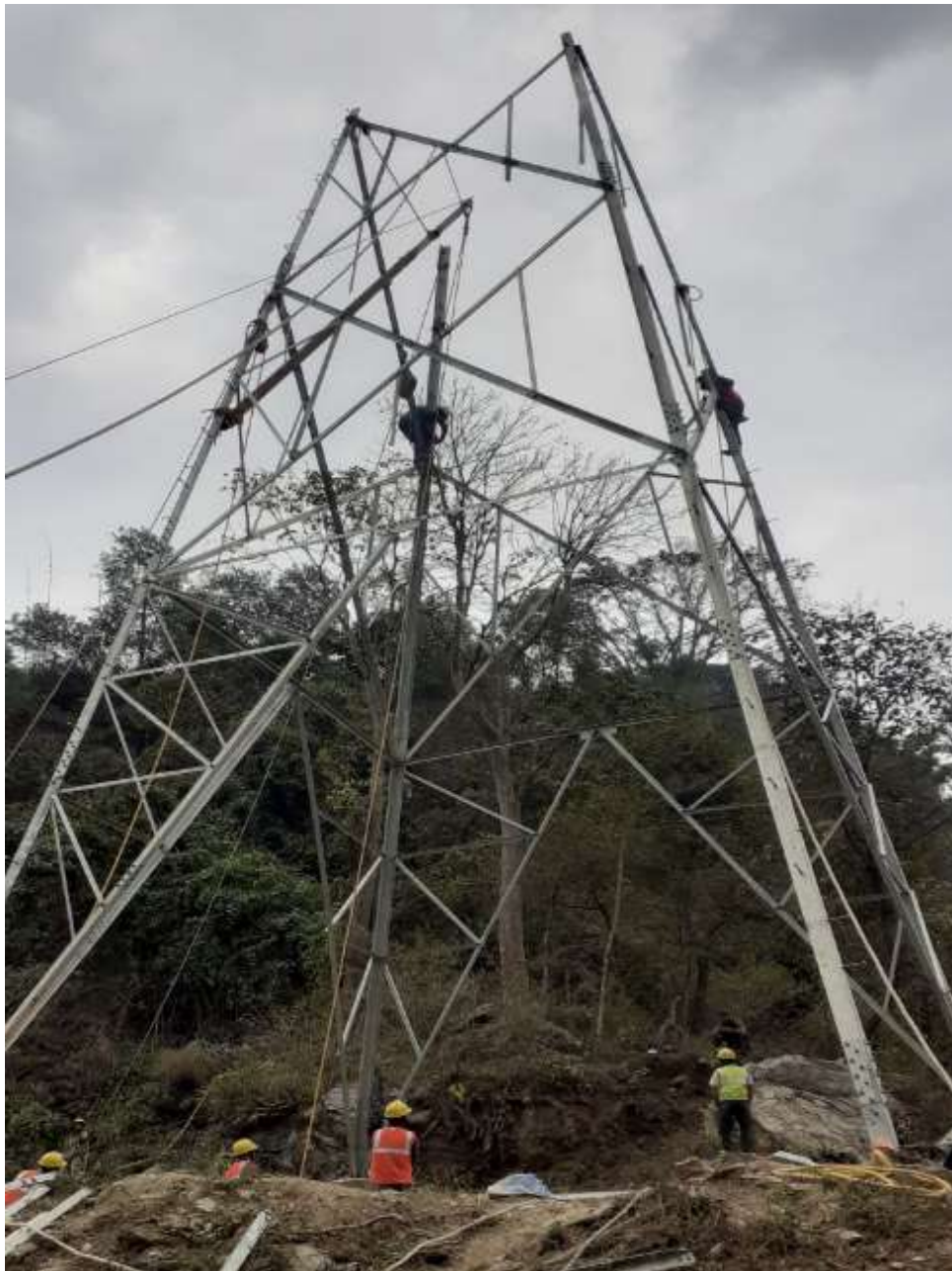
Figure 55: Tower erection works ongoing at AP16
