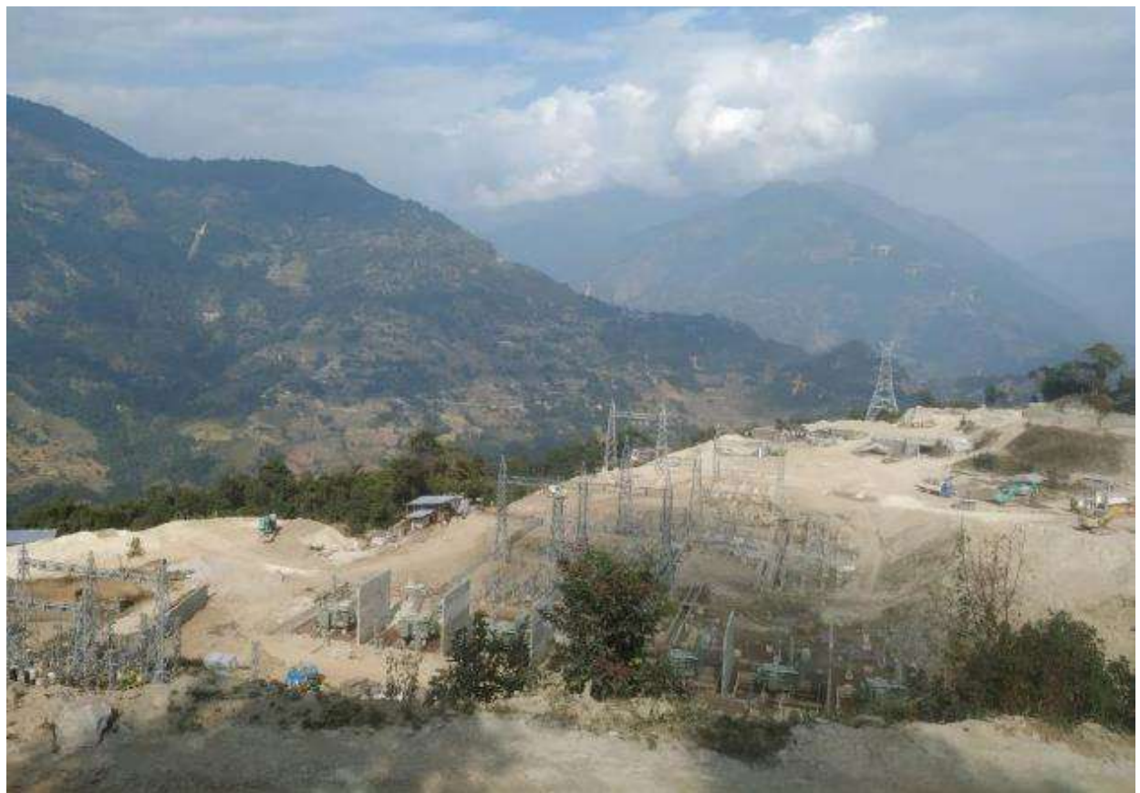
Figure 50: Dhunge-Sanghu substation (NEA Project)
