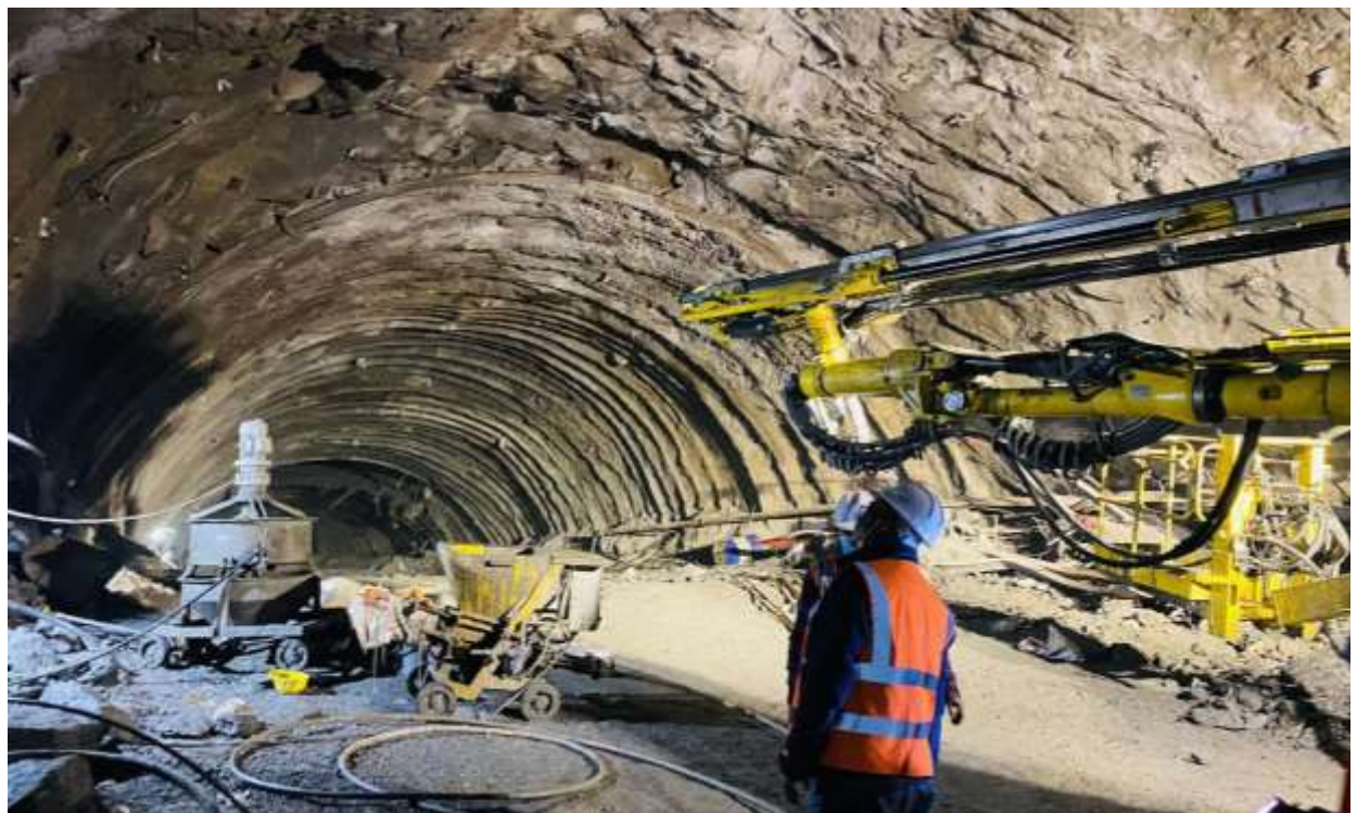
Figure 18: Face drilled by Boomer at SB 01
