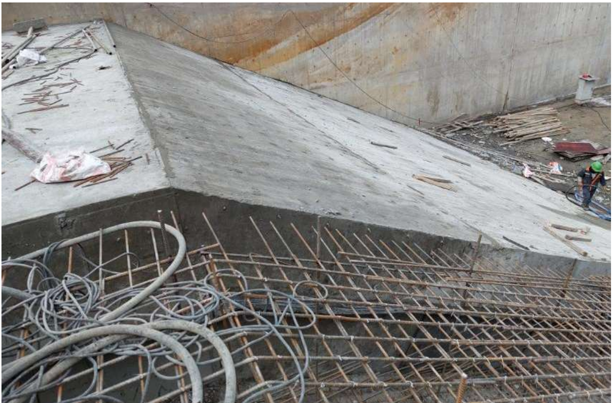
Figure 15: Ongoing Reinforcement works at jumping apron of stilling basin
