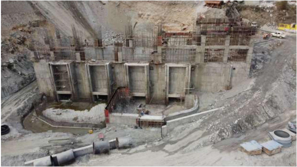
Figure 28: An aerial view of Powerhouse
