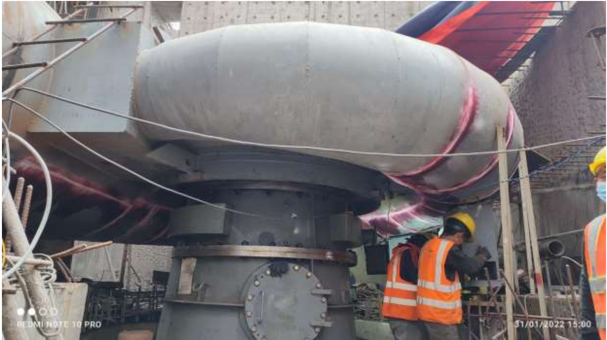
Figure 50: DPT test of welded segments of Spiral case
