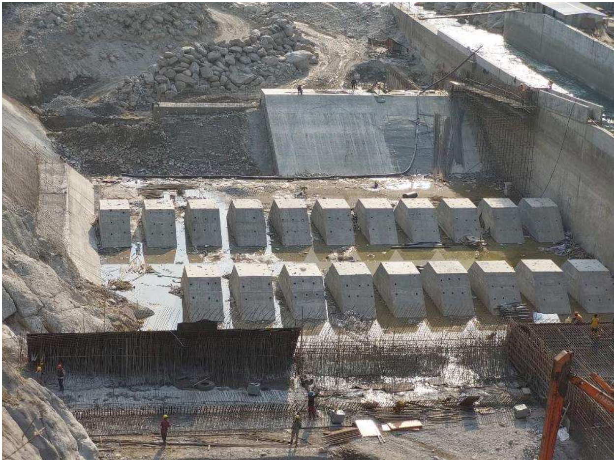
Figure 11: Reinforcement works at weir main body
