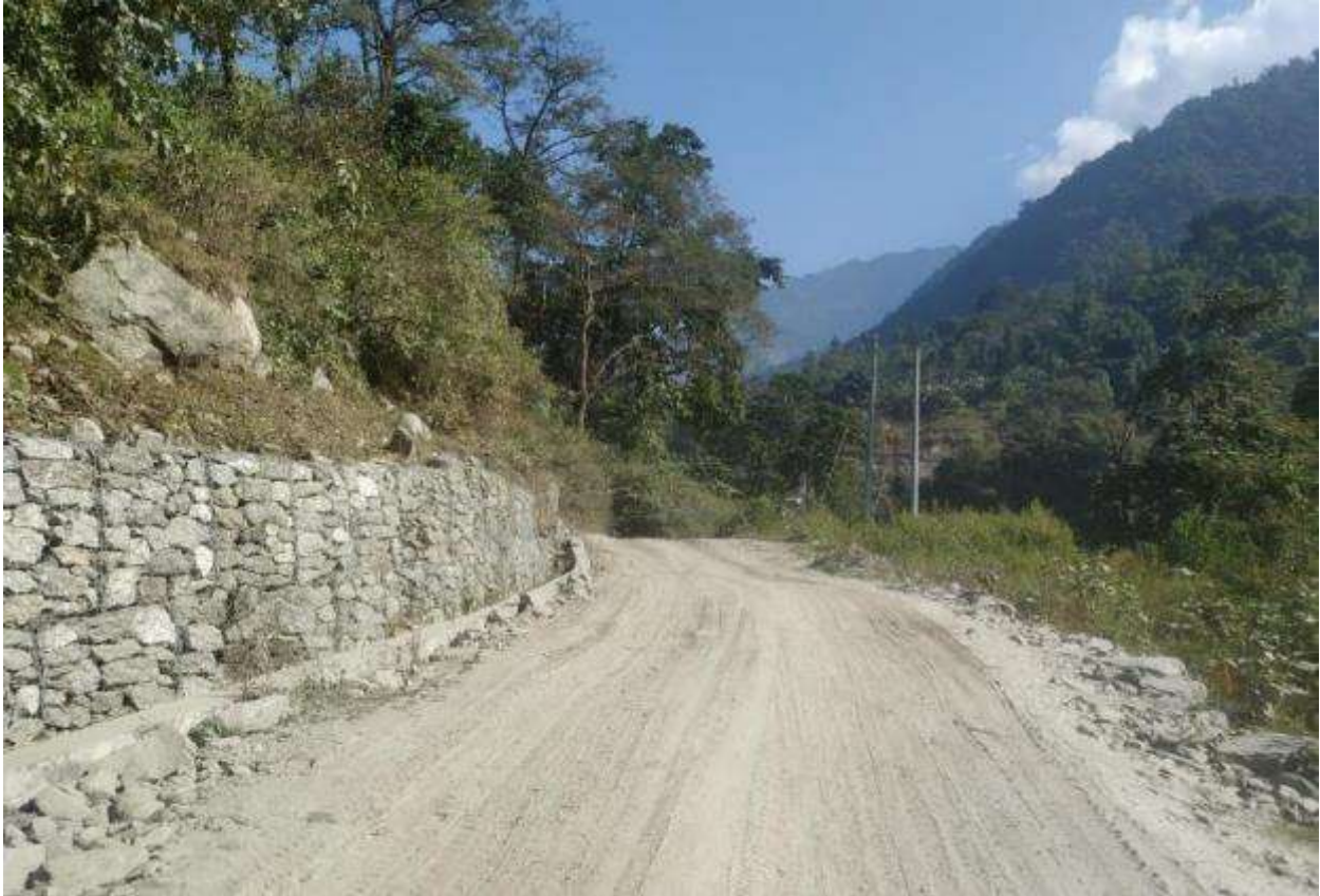
Figure 3: Gabion wall construction at new access road from Mitlung to Thumba
