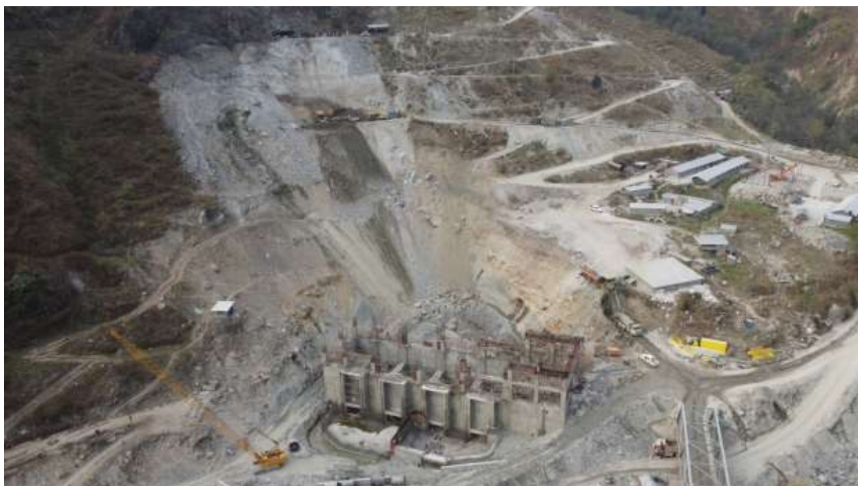
Figure 30: Bird's eye view of construction works at Penstock area
