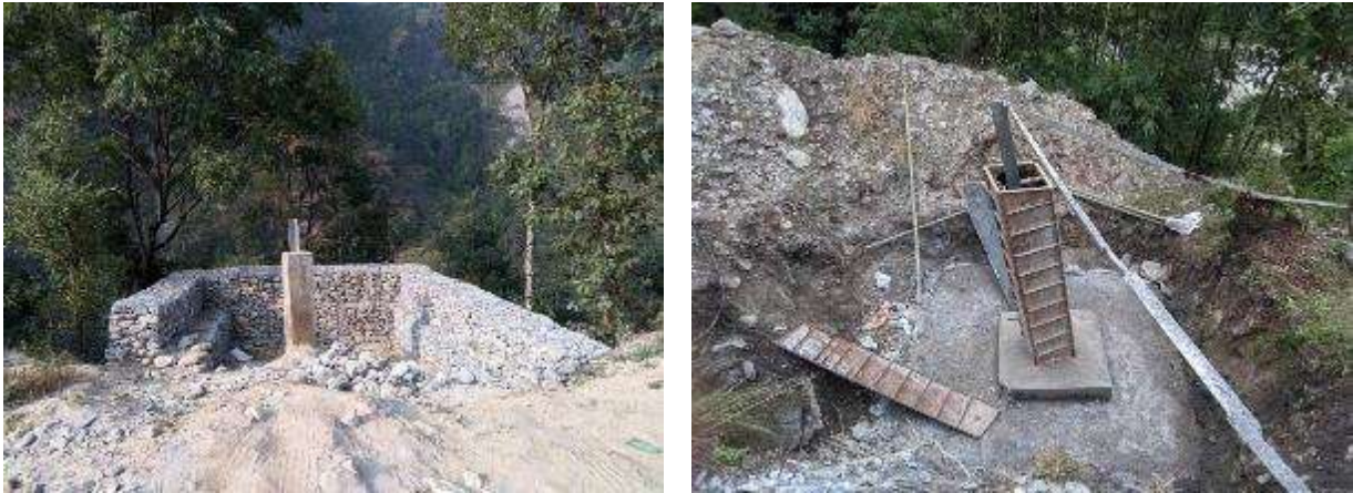
Figure 49: Stub erection and foundation works
