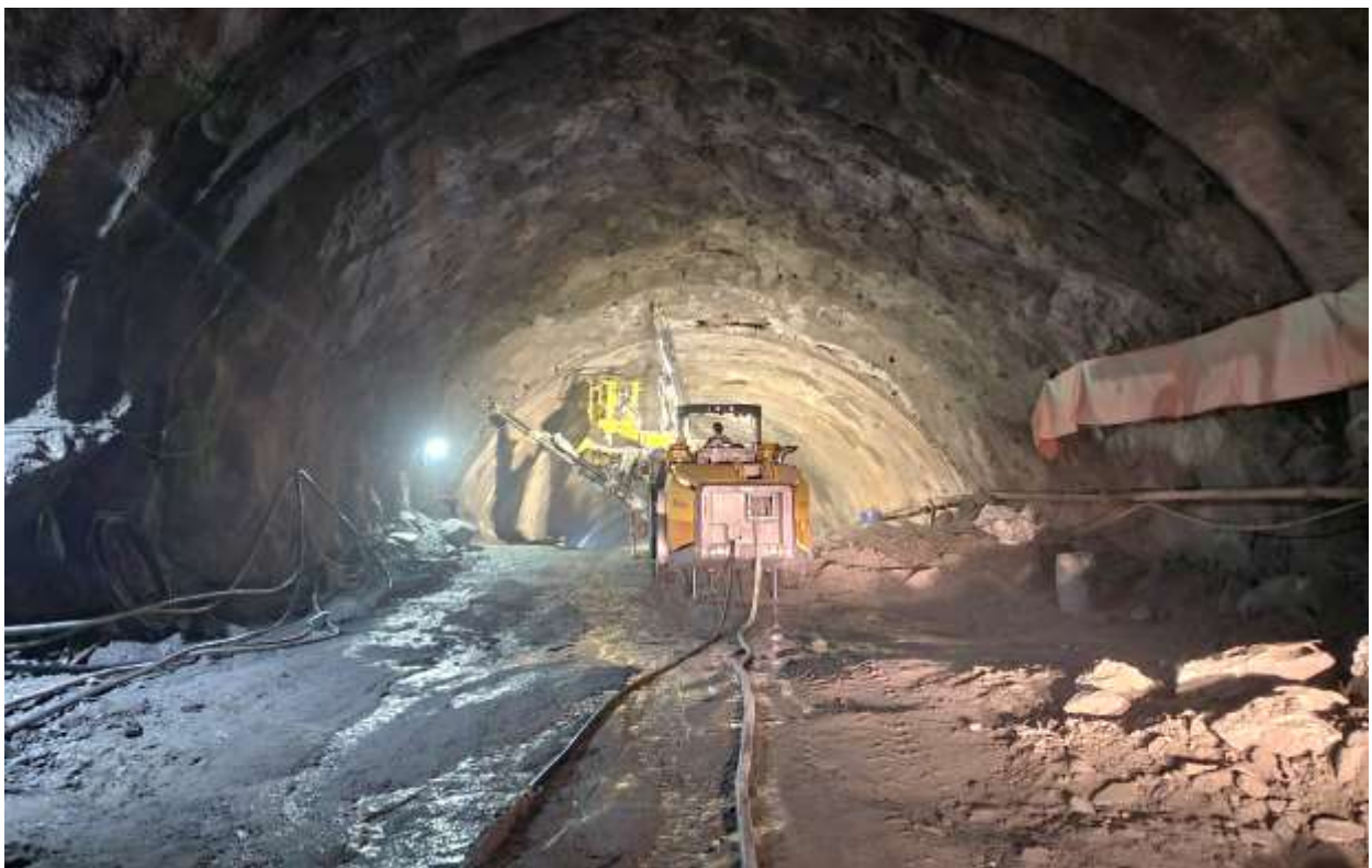
Figure 22: Drilling works at SB for rock bolts installation
