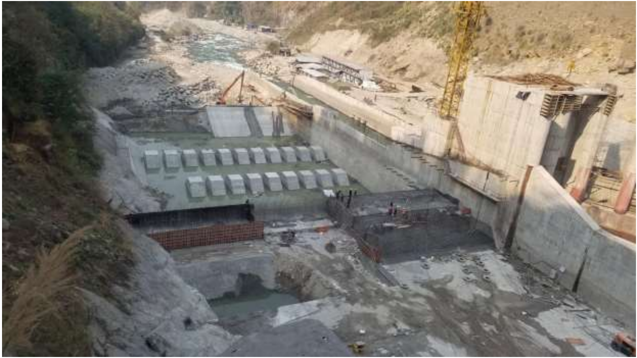
Figure 12: Aerial view of concreting works at stilling basin and weir body
