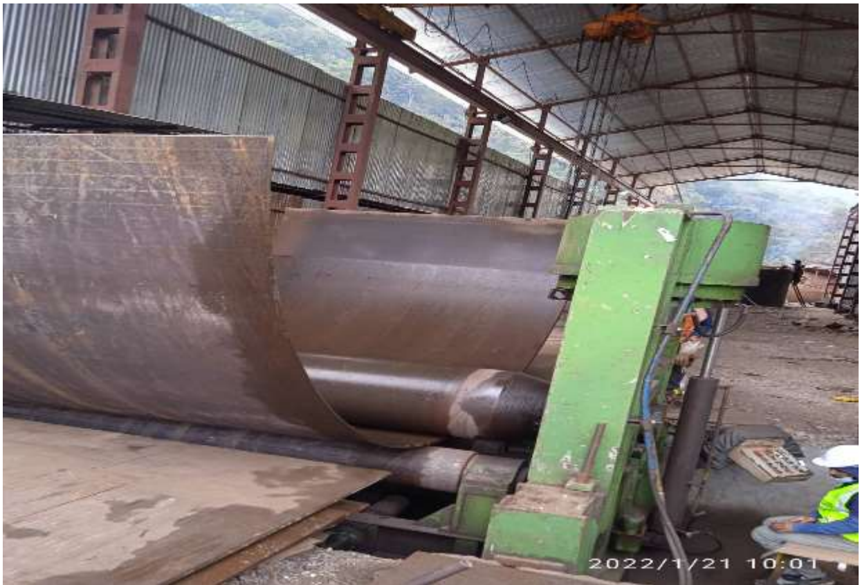
Figure 35: Rolling of penstock pipe
