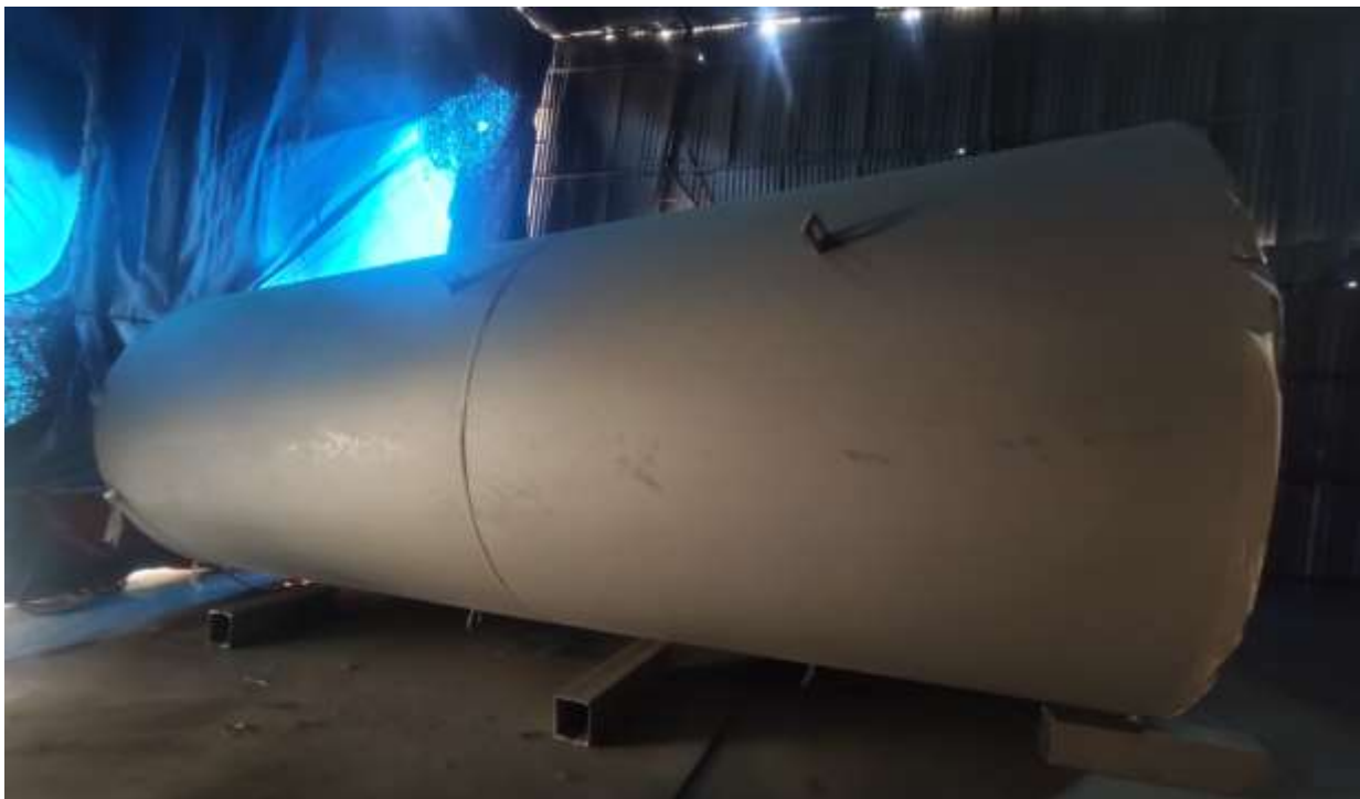
Figure 34: Bifurcation Unit 1 part 2 after applying primer coating
