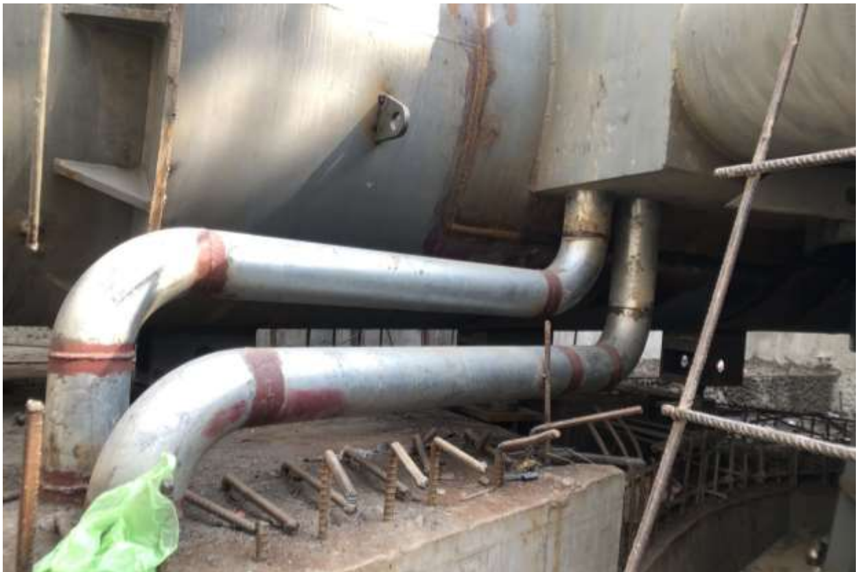
Figure 53: Nose drain of Spiral case
