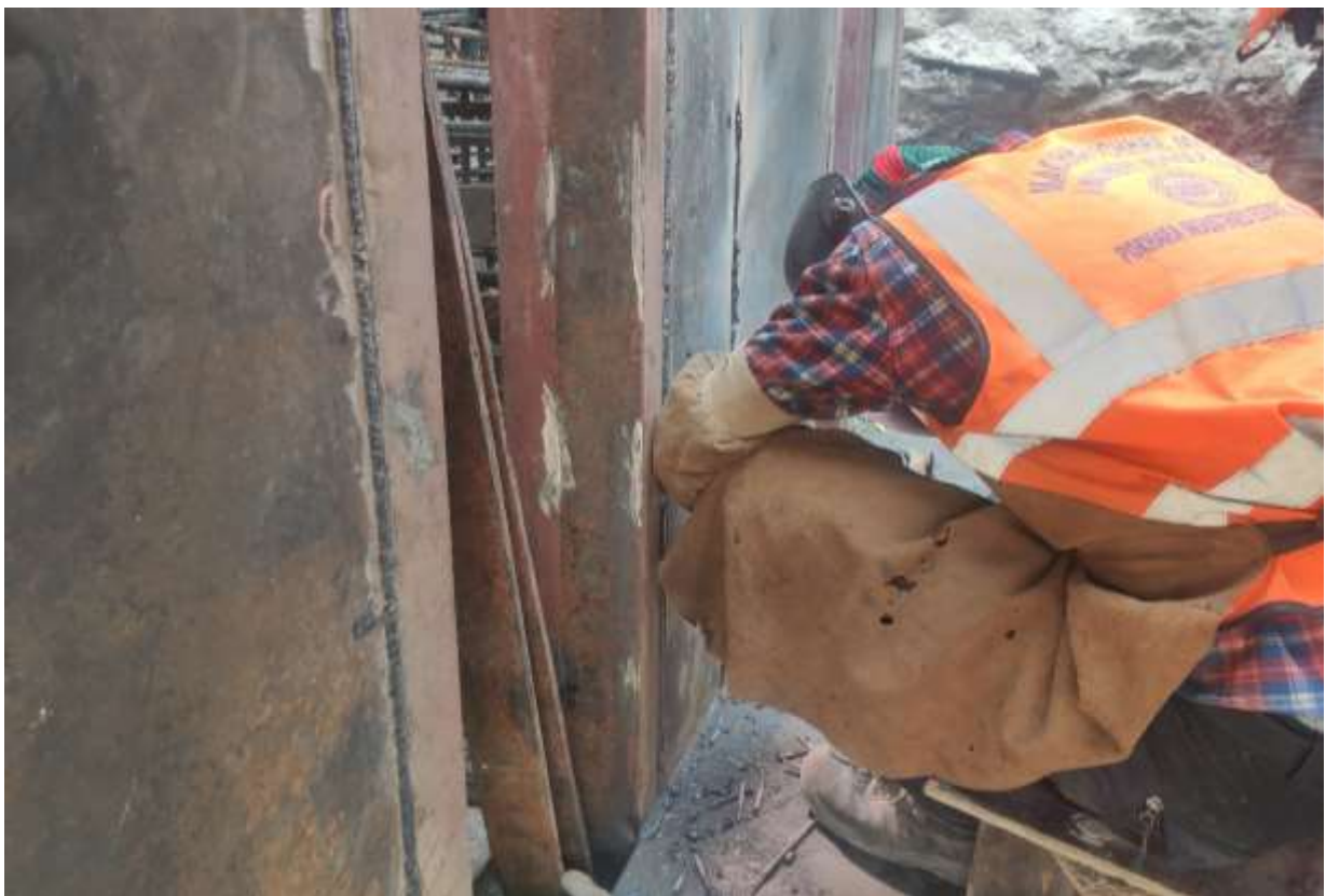
Figure 36: Erection and welding of steel lining at gravel flushing section
