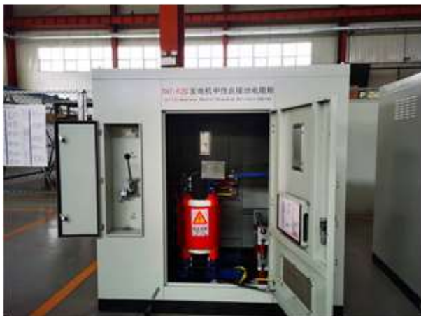
Figure 47: Neutral grounding panel
