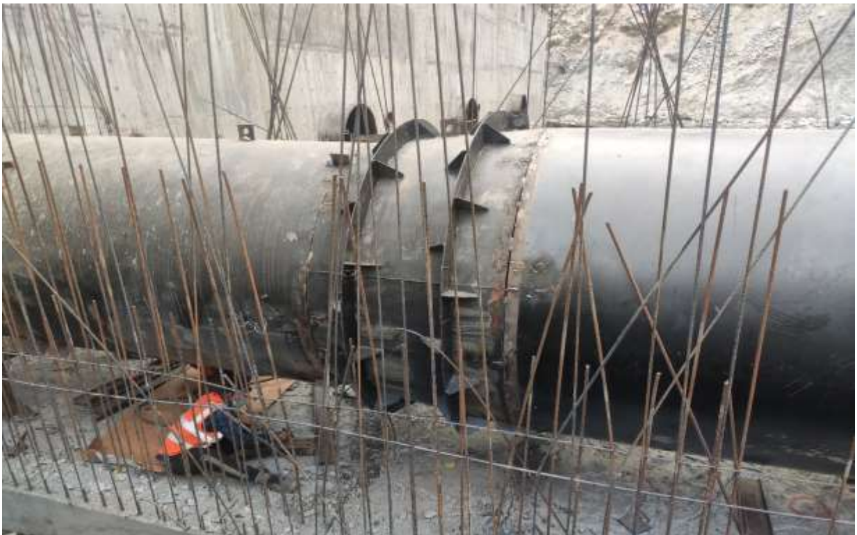
Figure 38: Position adjustment of branch pipes of penstock
