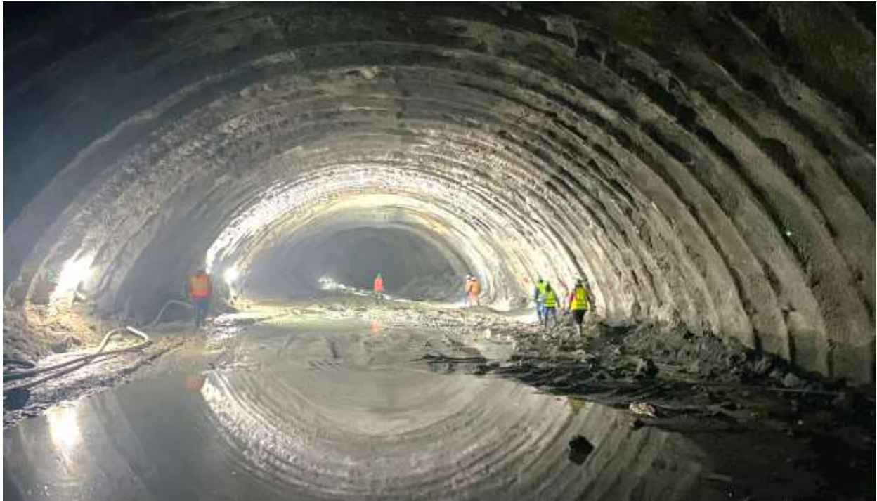
Figure 19: Breakthrough at Connecting Tunnel junction (SB-02)
