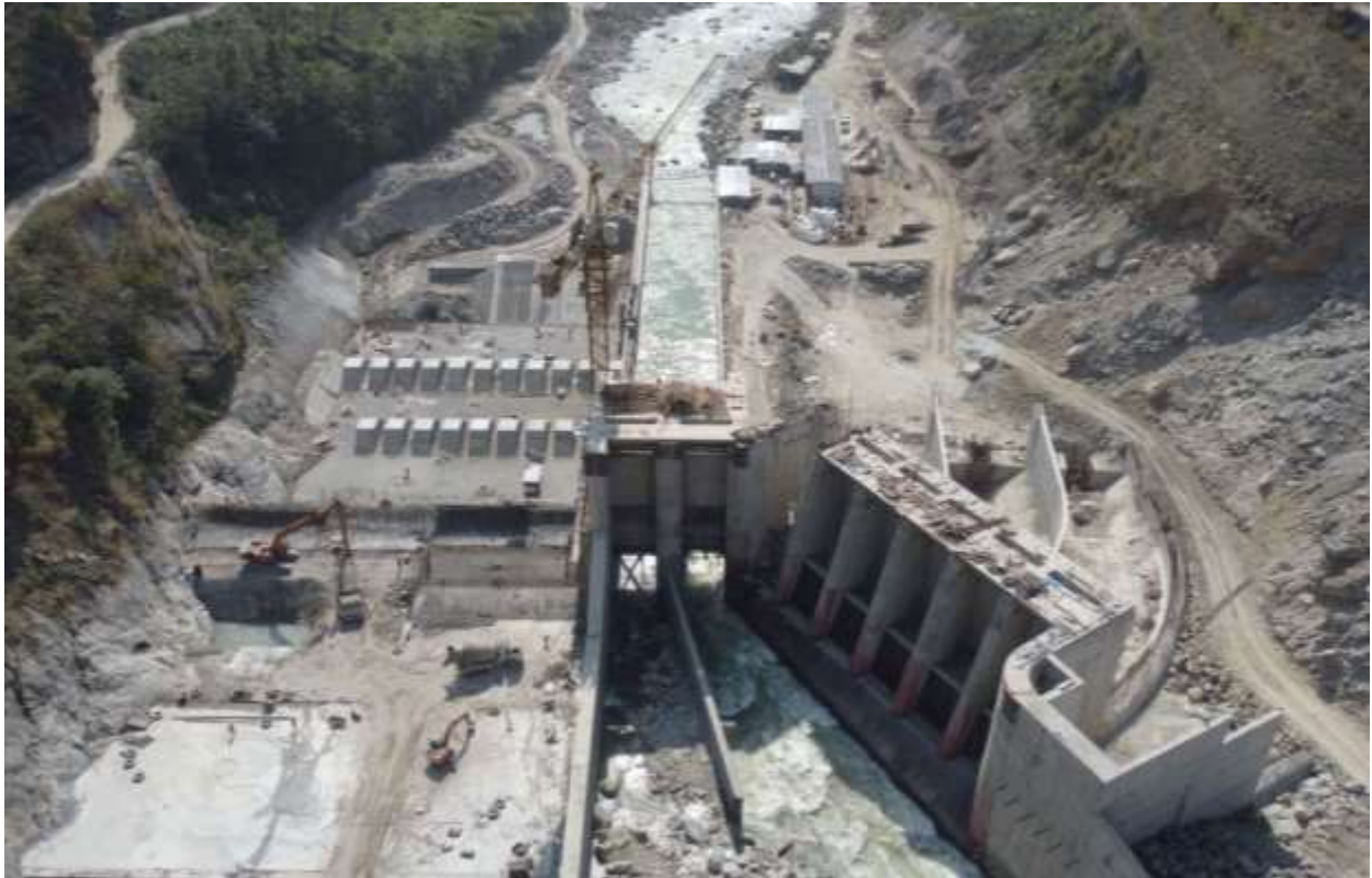
Figure 10: Headworks (A view of Undersluice and weir stilling basin from upstream)
