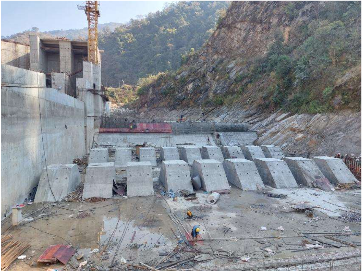
Figure 14: Completed concreting works at baffle blocks
