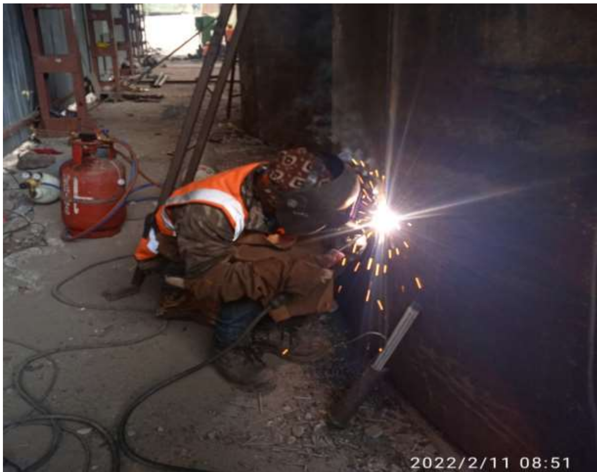
Figure 32: Welding of pipes at HM workshop
