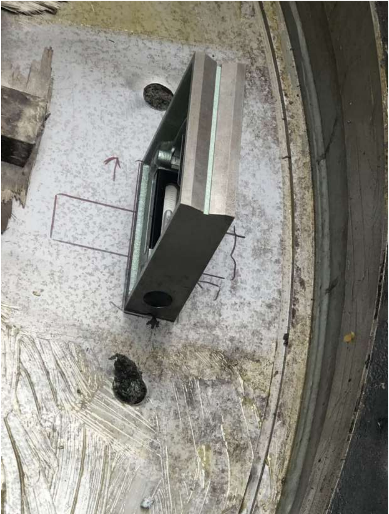
Figure 49: Labeling work of bottom ring plate
