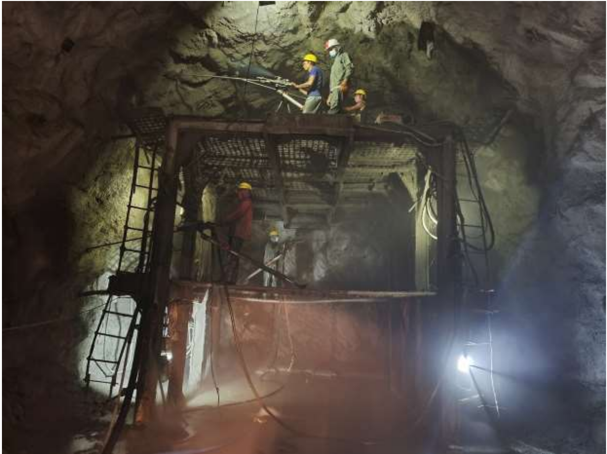
Figure 17: Rock support works at HRT from adit
