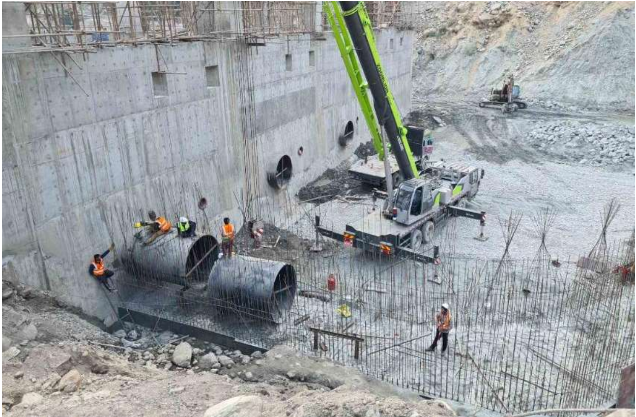
Figure 33: Installation of penstock pipes (branch pipes)
