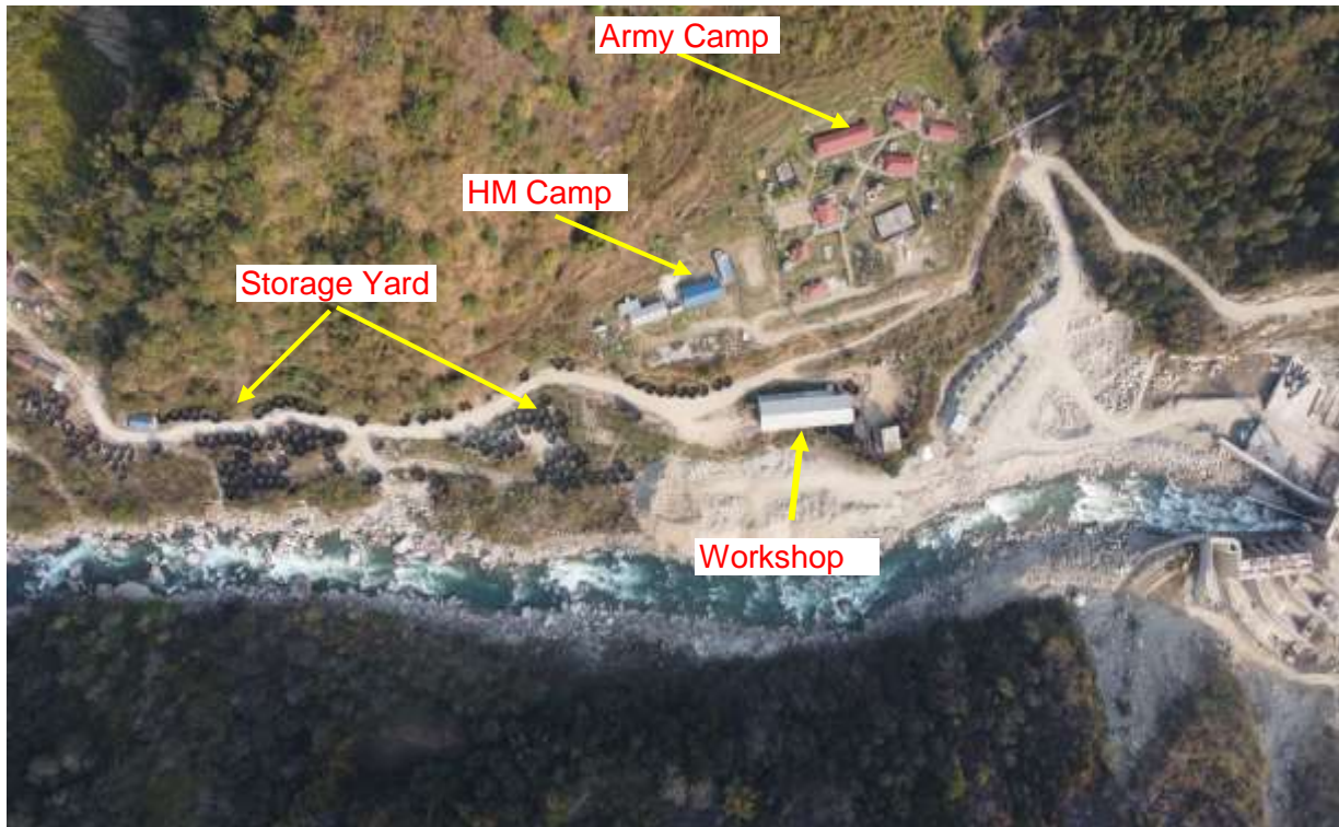
Figure 31: Aerial view of HM Camp, storage yard, workshop and Army camp
