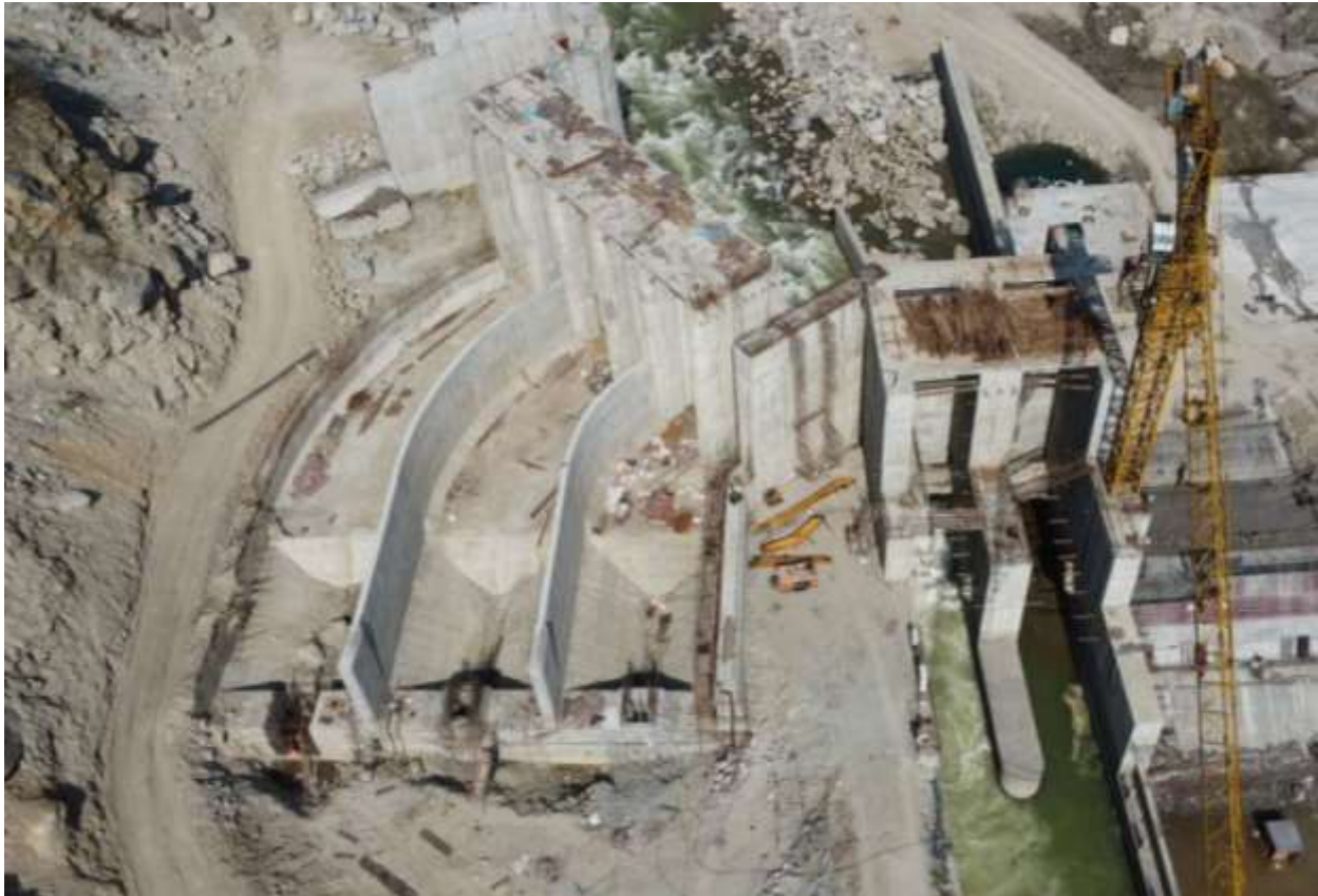
Figure 9: A aerial view of Gravel trap
