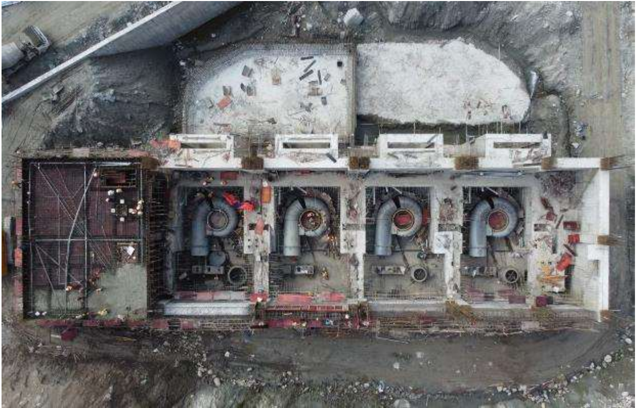
Figure 26: Top view of powerhouse
