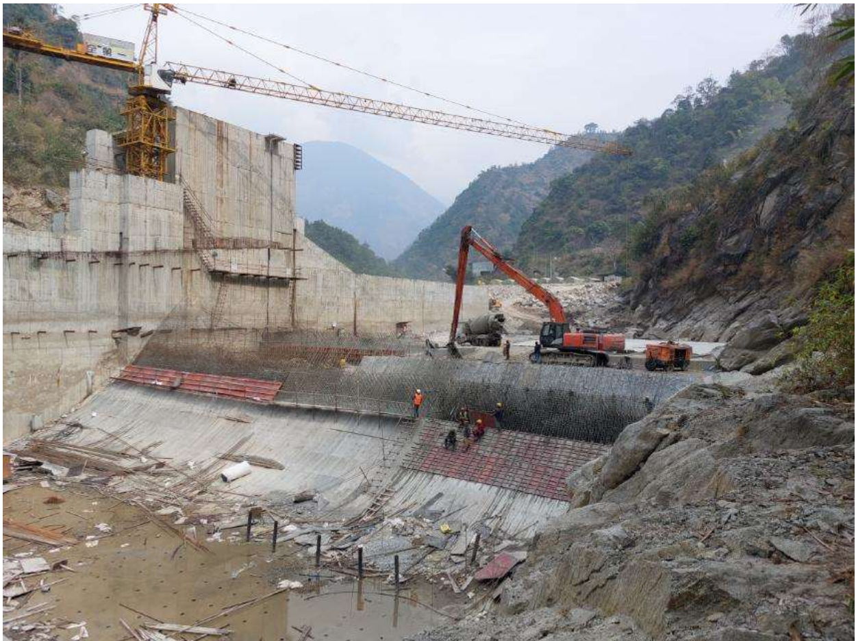
Figure 13: Ongoing reinforcement works of downstream slope of weir body
