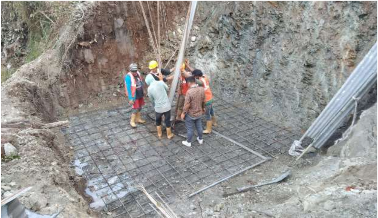
Figure 56: Rebar installation work of leg at AP24
