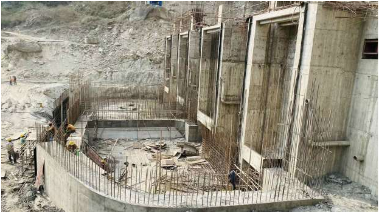
Figure 29: Reinforcement works at Tailrace culvert Panel 01 & 02
