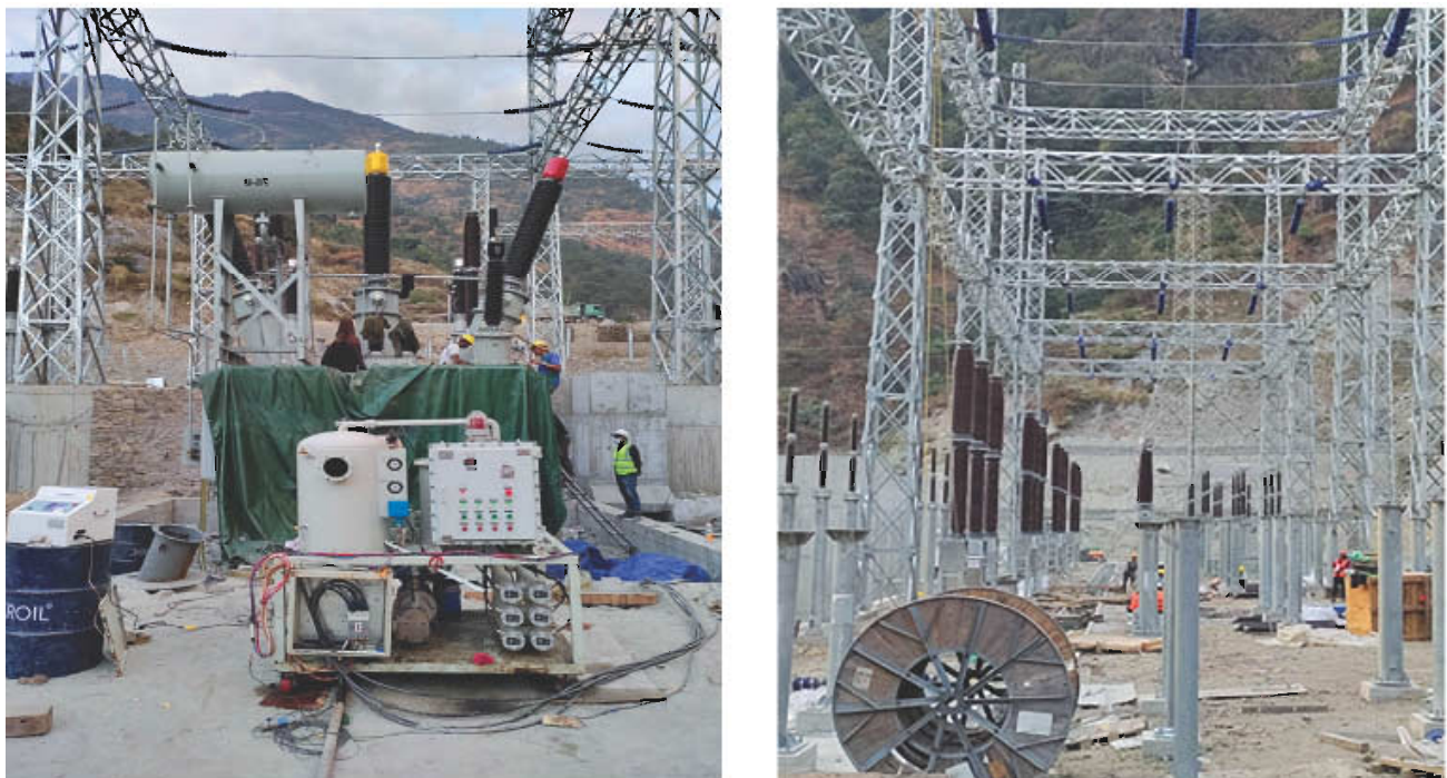
Figure 2.25: Erection of gantry towers and final assembly of Transformer at switchyard
