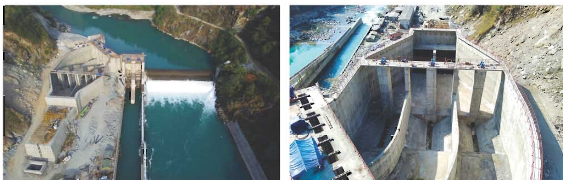
Figure 2.2: Aerial view of Headworks from the downstream (left) and A view of gravel trap and conveyance tank from upstream (right)
