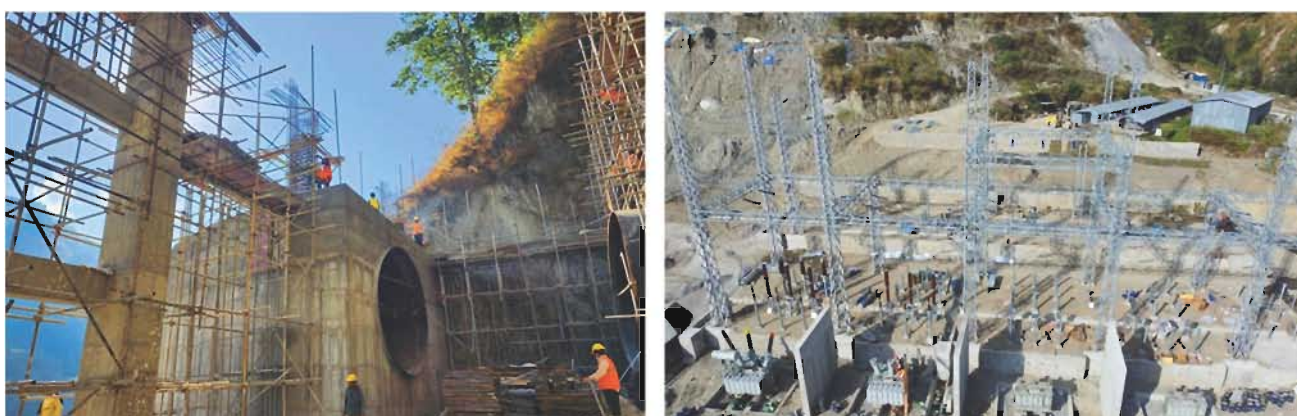
Figure 2.15: A view of switchyard with 4 power transformers positioned (left) and construction of anchor block and valve house (right)
