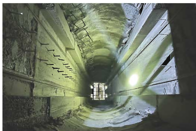
Concrete lining at Flushing gate shaft
