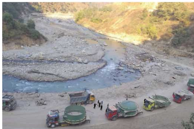
Penstock Protection Valve Transportation
