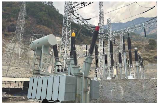
Transformer final assembly at switchyard
