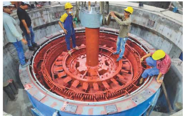
Figure 2.23: Rotor lowering of unit 04 (left) and Unit 02 MIV valve assembly and erection (right)
