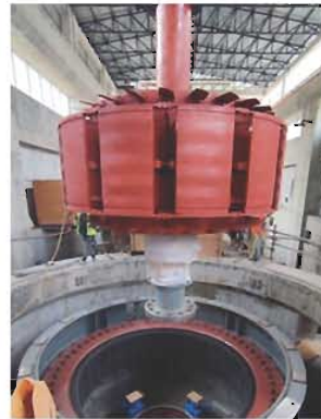
Figure 2.22: Rotor lowering in unit 4 (left) and assembly of runner with main shaft (right)
