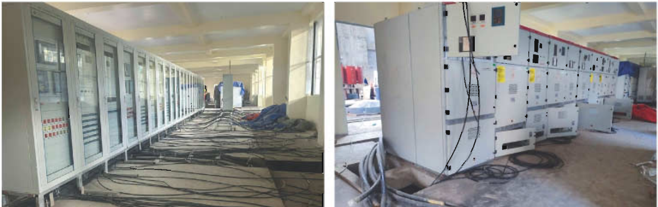
Figure 2.24: Laying of control cables in control room (left) and laying of power and control cables in 11kV switchgear room (right)
