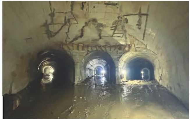
Figure 2.10: Full lining concrete at connecting tunnel junction
