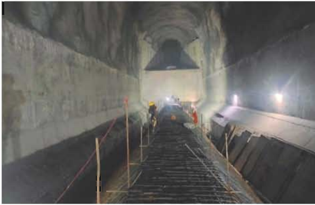
Figure 2.7: A view of rebar layout and concreting works at SB 01
