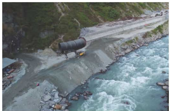
Approach pipes installation at Headworks
