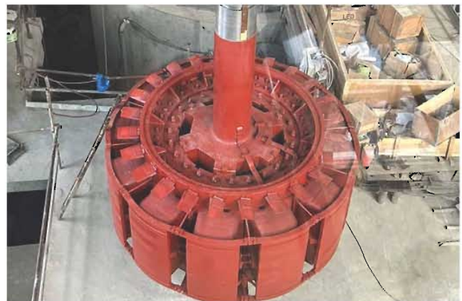
Rotor assembly at service bay
