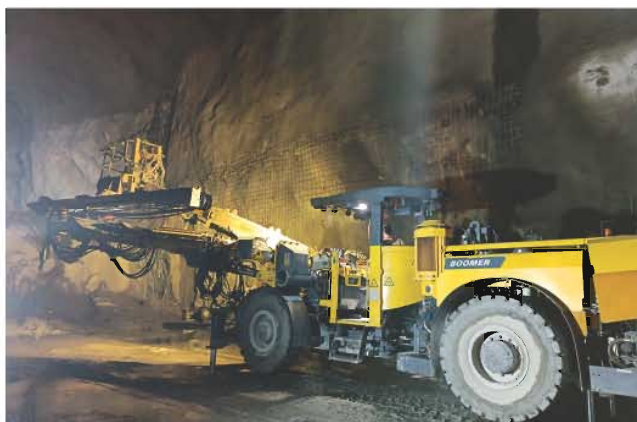
Drilling works using Boomer
