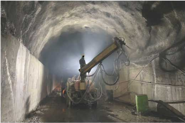
Shotcreting at HRT using Robotic shotcrete machine
