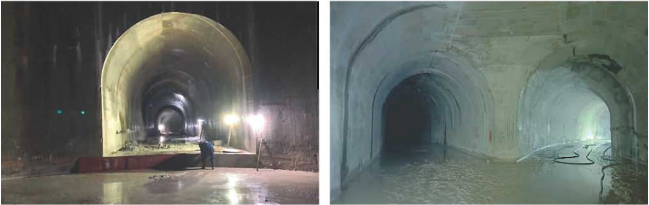
Figure 2.13: A view of full lining concrete at connecting tunnel (left) and the junction of connecting tunnel and HRT (right)
