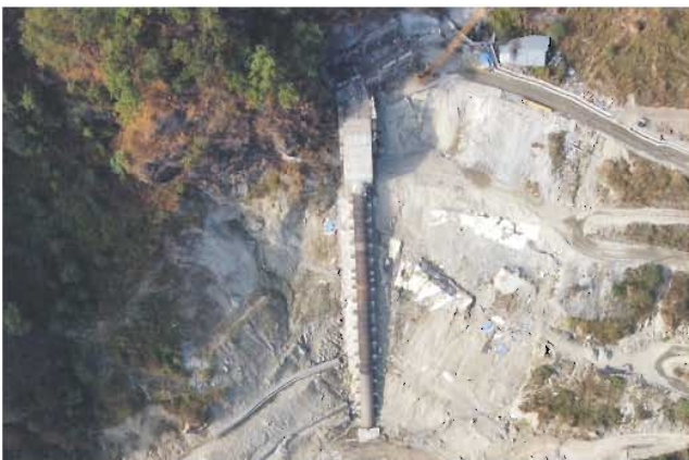
Aerial view of valve house, anchorblock and penstock pipes
