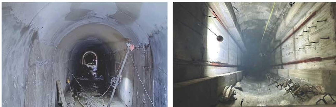
Figure 2.12: A view of full concrete lining at the flushing tunnel (left) and Concreting works at flushing shaft 'A' (right)
