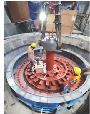
Figure 2.22: Rotor lowering in unit 4 (left) and assembly of runner with main shaft (right)
