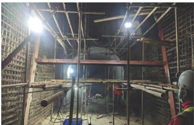
Figure 2.17: Erection of trashrack frame and gate embedded parts at SB Outlet Gate-3 (left) and installation of head race bend (right)
