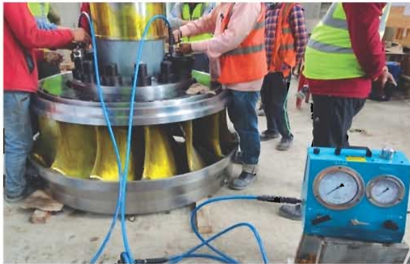
Figure 2.22: Rotor lowering in unit 4 (left) and assembly of runner with main shaft (right)
