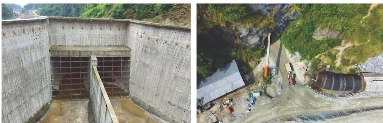
Figure 2.4: A view of conveyance tank (left) and Approach pipes installation completed upto inlet portal (right)
