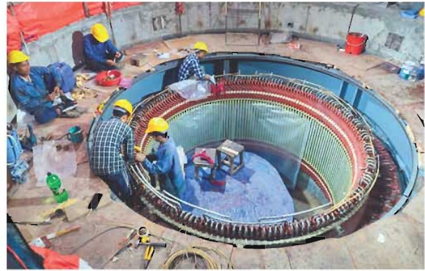
Figure 2.21: Brazing and lacing work of stator coils in Unit 02 (left) and run-out check of shaft Unit 03 (right)
