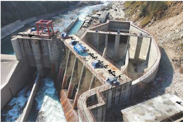
Aerial view of undersluice, intake and gravel trap
