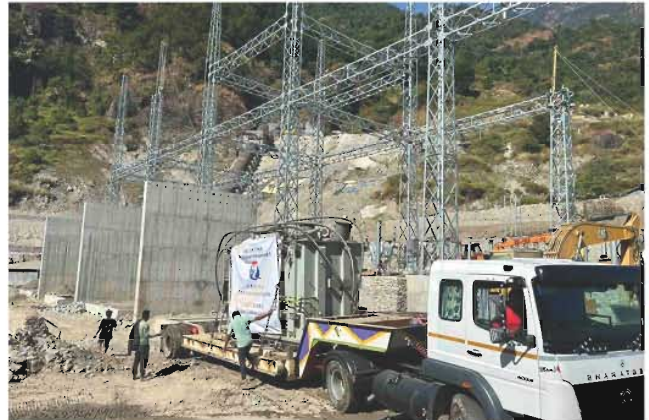
Transportation of Power Transformers)
