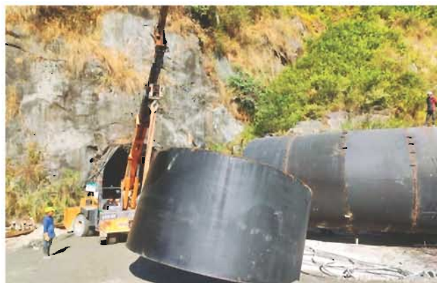
Figure 2.17: Erection of trashrack frame and gate embedded parts at SB Outlet Gate-3 (left) and installation of head race bend (right)
