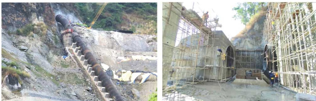
Figure 2.18: Erection of penstock pipes (left) and the PPV location (right)
