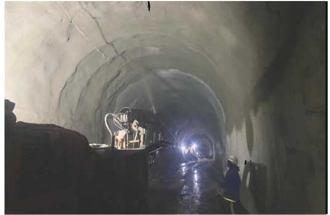
Shotcreting at HRT using Robotic shotcrete machine
