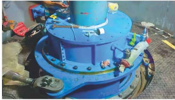
Figure 2.20: Rotor and stator coupling in unit 01 (left) and final installation of water guide mechanism along with monitoring sensors (right)
