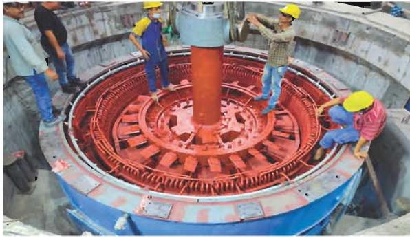
Figure 2.20: Rotor and stator coupling in unit 01 (left) and final installation of water guide mechanism along with monitoring sensors (right)
