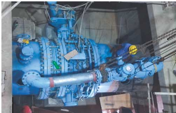
Figure 2.23: Rotor lowering of unit 04 (left) and Unit 02 MIV valve assembly and erection (right)
