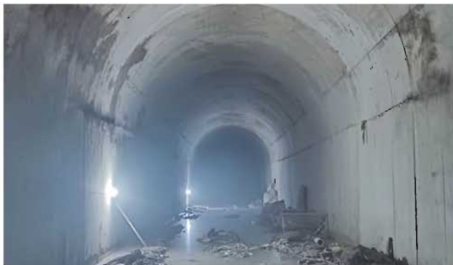
Figure 2.11: A section of HRT with concrete full lining from the adit region (left) and A completed section of rock trap (right)
