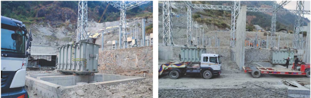
Figure 2.26: Power transformers placed at its position (left) and unloading of power transformers at the switchyard region (right)
