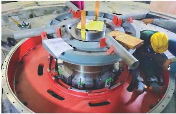
Figure 2.21: Brazing and lacing work of stator coils in Unit 02 (left) and run-out check of shaft Unit 03 (right)
