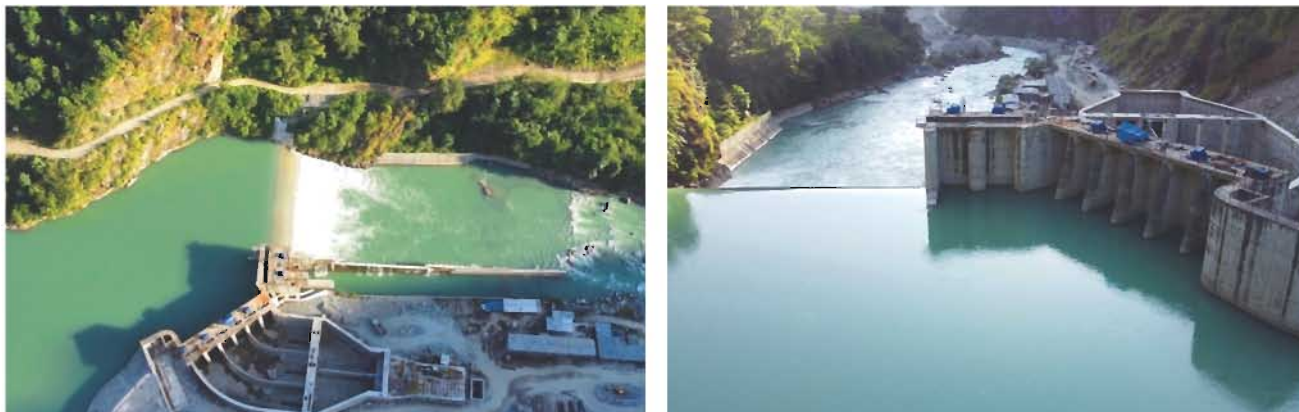
Figure 2.3: An aerial view of weir with flow over the ogee crest (left) and Current view of headworks (right)
