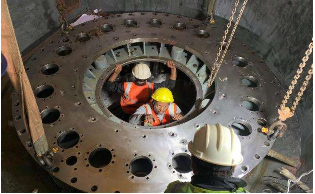
Figure 47: Lowering of headcover in unit 2
