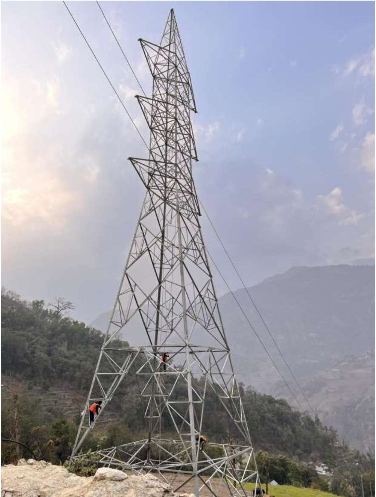
Figure 2-76: Conductor Stringing preparation work ongoing between AP21 and AP 22
