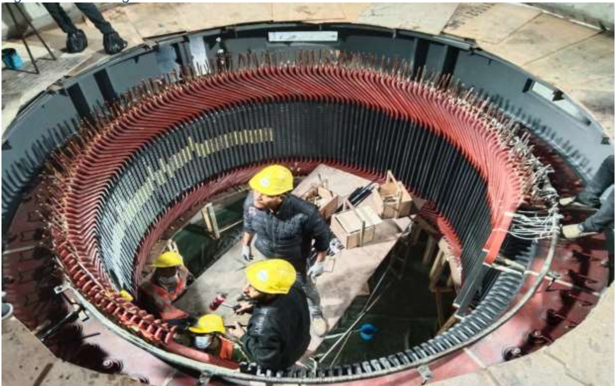
Figure 63: Stator winding works at near completion stage
