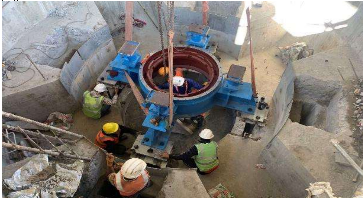
Figure 2-58: Installation of lower bracket in unit 1
