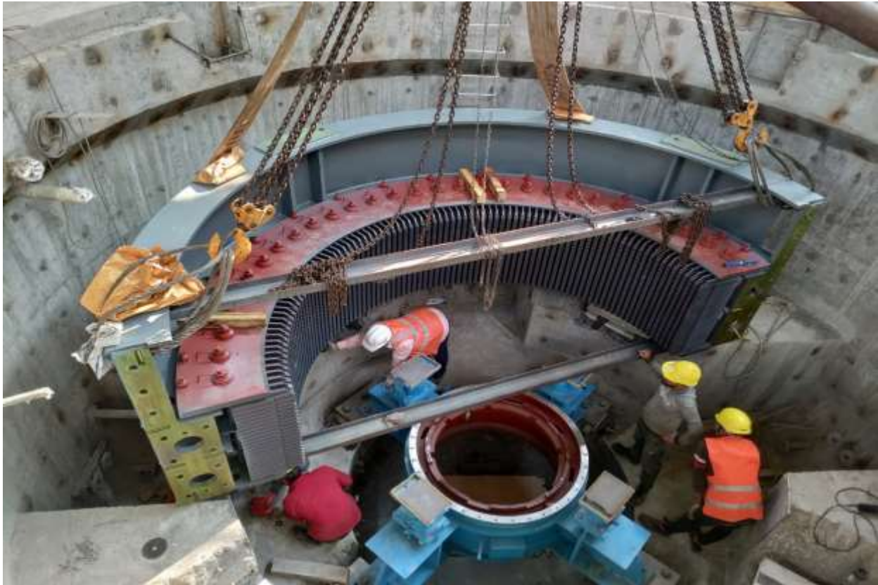
Figure 65: Lowering of split stator into the pit
