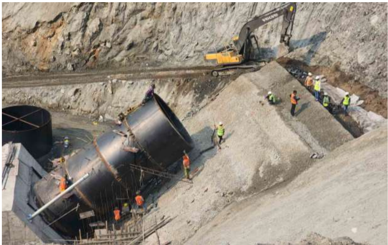
Figure 2-36: Penstock slope stabilization and simultaneous penstock pipe installation
