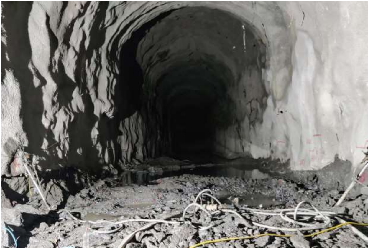
Figure 2-21: A view of excavation of Settling basin 02 (Completed up to hooper level)
