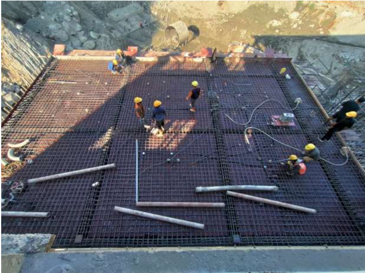
Figure 69: Imbedded parts and pipes of Control room slab
