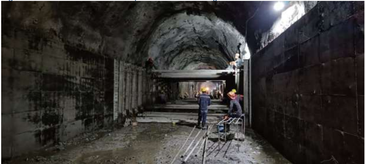
Figure 2-15: Preparation of formwork assembly for concrete wall lining at chainage 1+500
