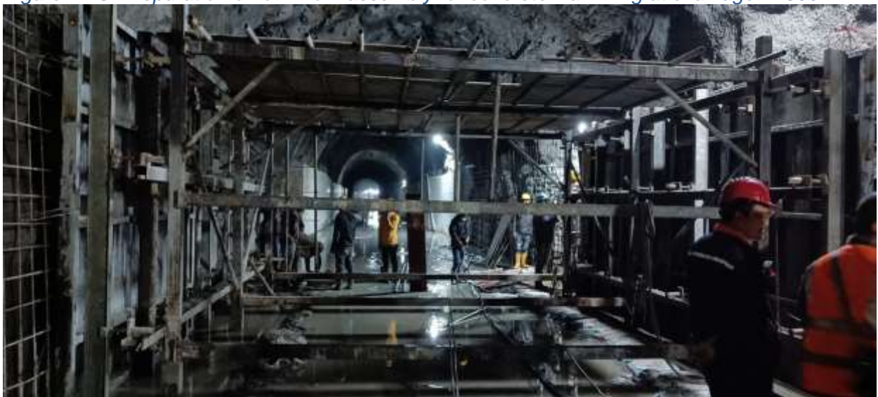
Figure 2-16: Preparation of formwork assembly for concrete wall lining at chainage 2+100
