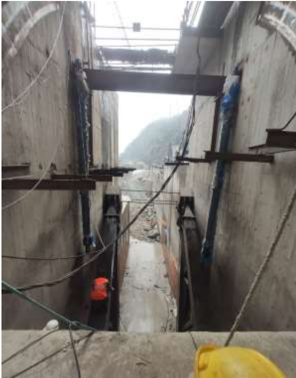
Figure 2-45: Hoisting Cylinders placed in position along with the Bush (left) and Conveyance tank right side trashrack frame (right)
