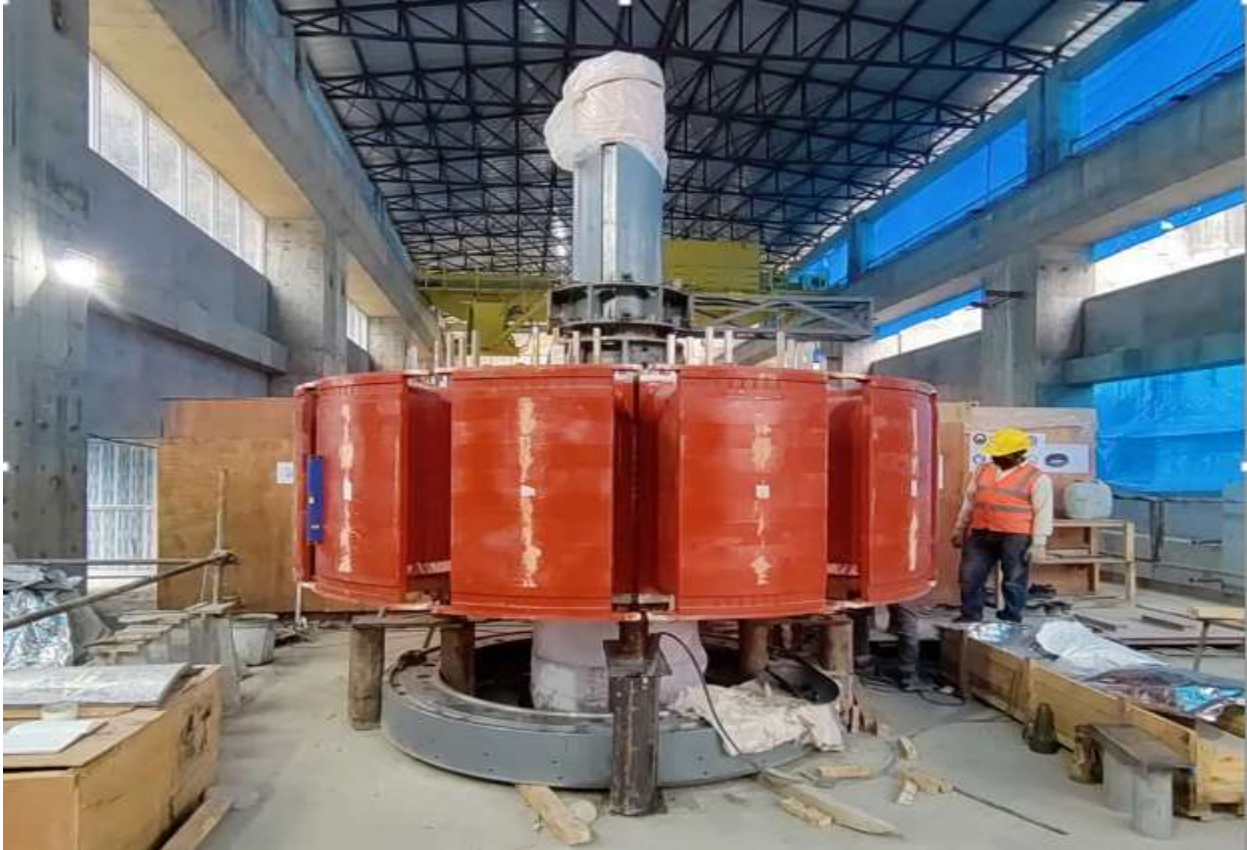
Figure 2-59: Rotor assembly at near completion stage
