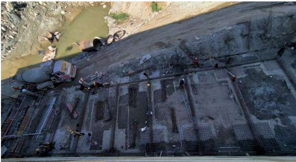
Figure 68: Imbedded parts and pipes at the bottom slab of Control room
