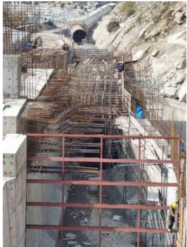
Figure 2-12: Erection of approach pipe (left) and rebar layout at conveyance tank region (right)
