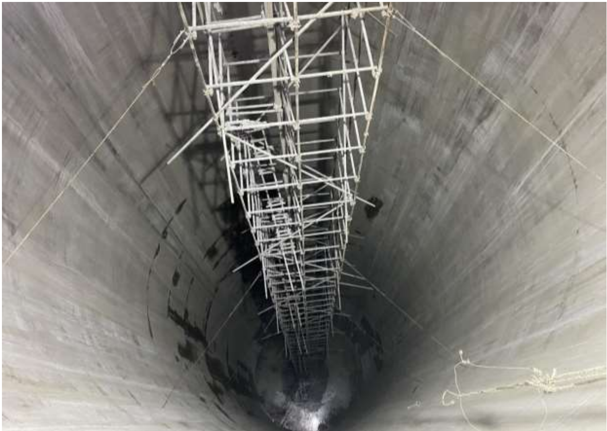
Figure 2-13: A view of surge shaft (Concrete lining completed)
