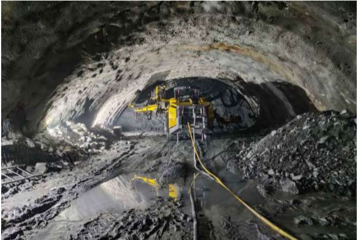
Figure 2-23: A view of drilling for face excavation of SB 03 using boomer
