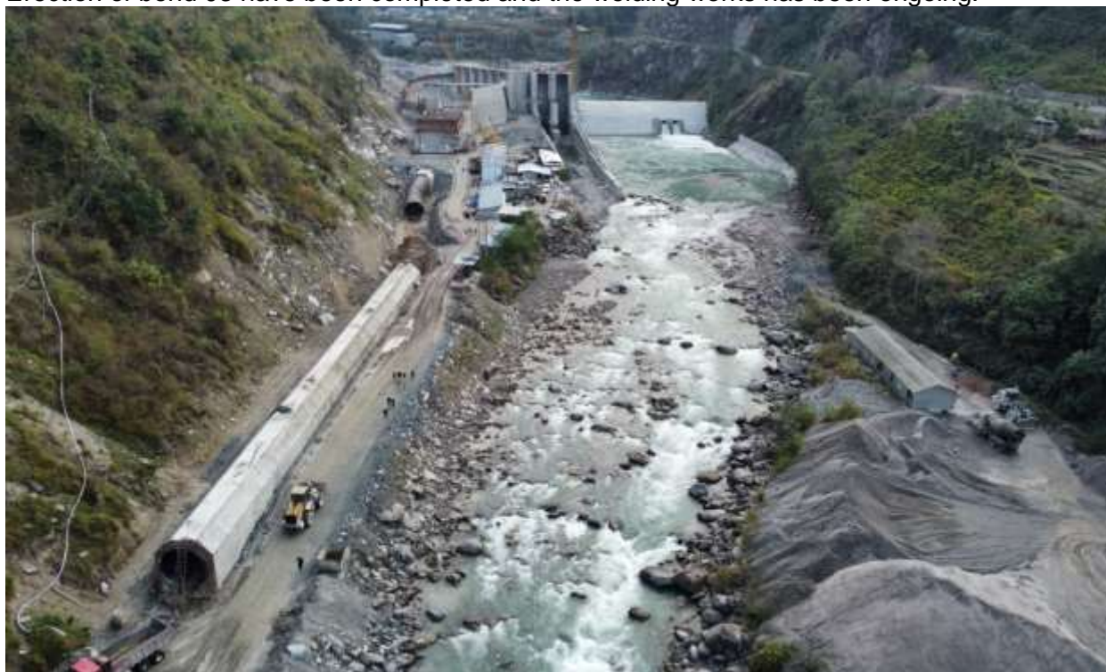
Figure 2-34: Installation of approach pipes at headworks region
