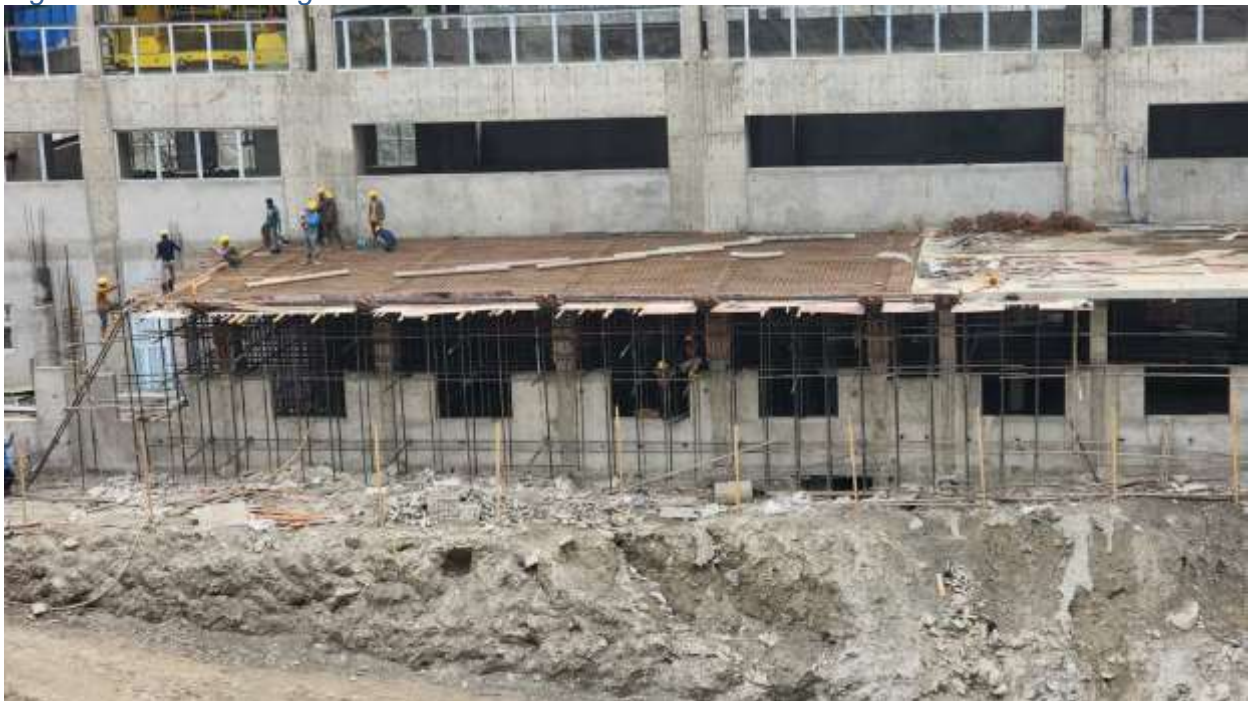
Figure 2-28: Concreting works at auxiliary powerhouse (control bay)
