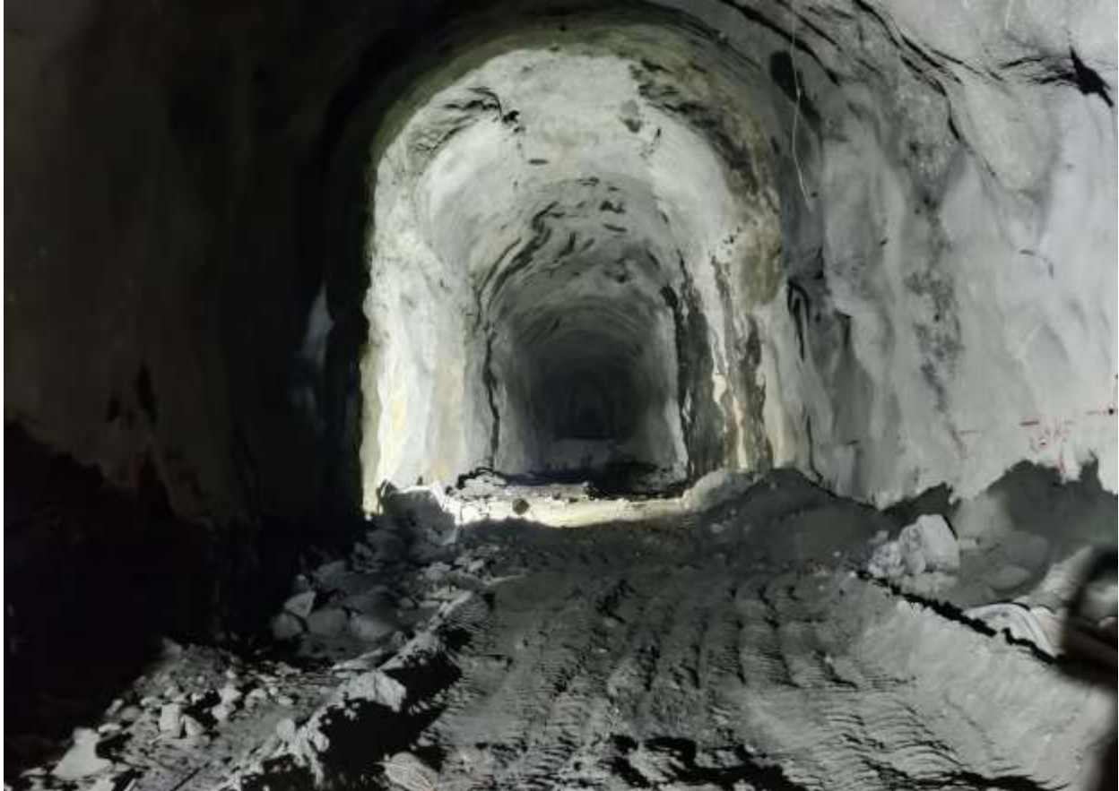
Figure 2-20: A view of excavation of Settling basin 01 (Completed up to hooper level)
