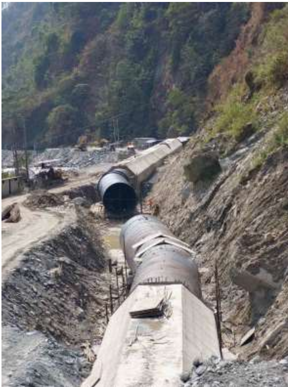
Figure 2-12: Erection of approach pipe (left) and rebar layout at conveyance tank region (right)
