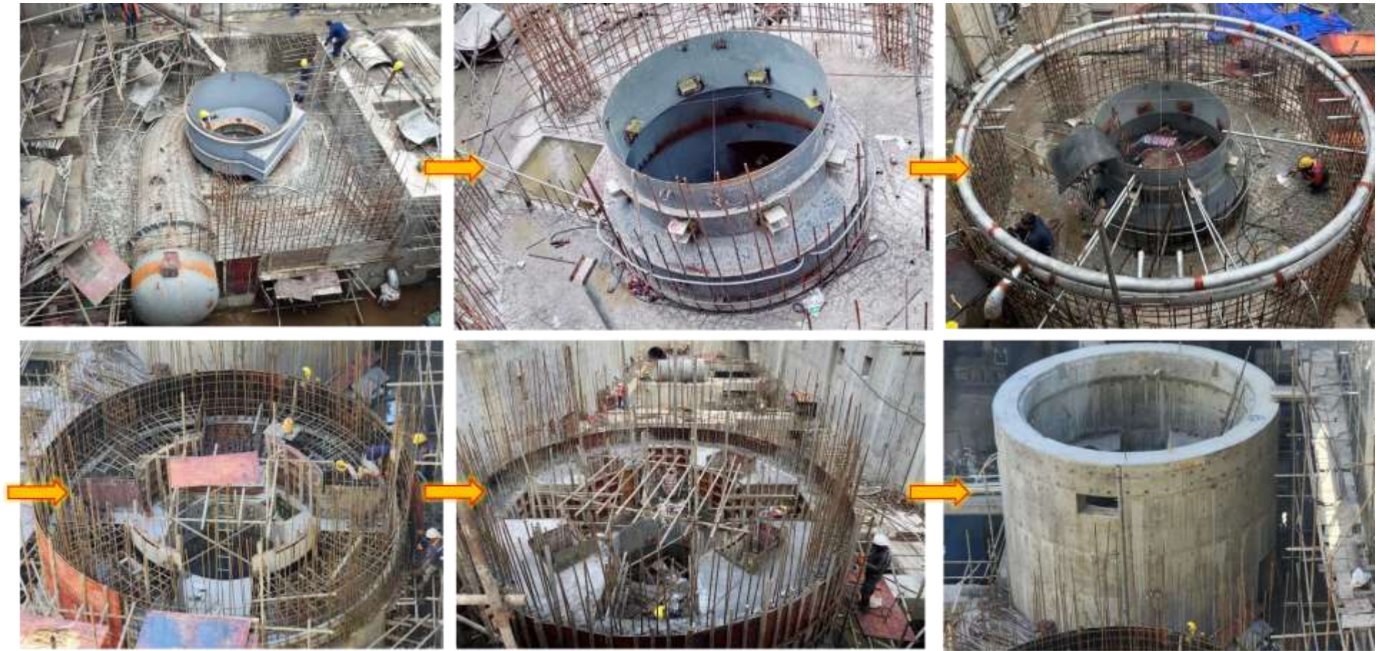
Figure 2-33: Progress of interface concrete works (Spiral case installation, pit liner installation, ventilation and heat exchange pipes and generator casing)
