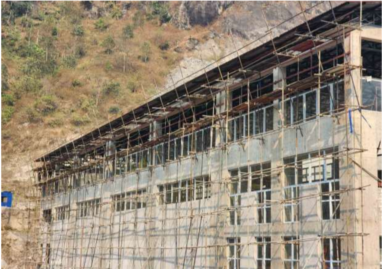
Figure 2-25: A view of Powerhouse from the downstream (installation of cladding)
