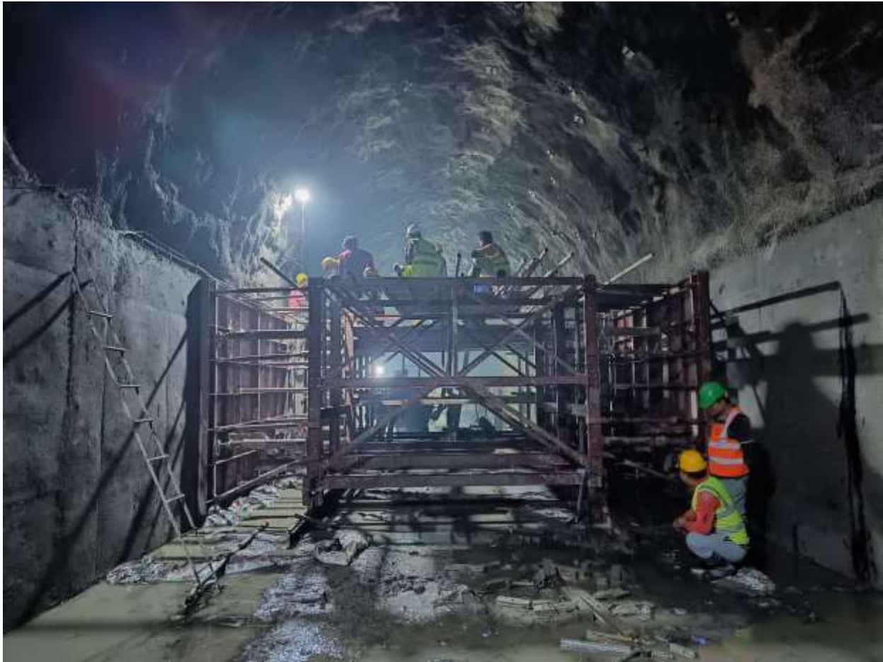
Figure 2-17: Mechanical formwork for partial concrete lining at HRT (chainage 2+100)
