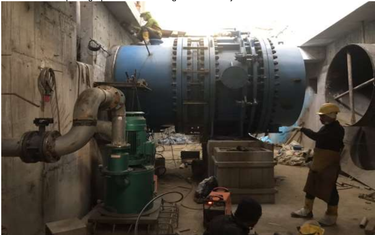
Figure 66: Unit 2 MIV lowered to its position
