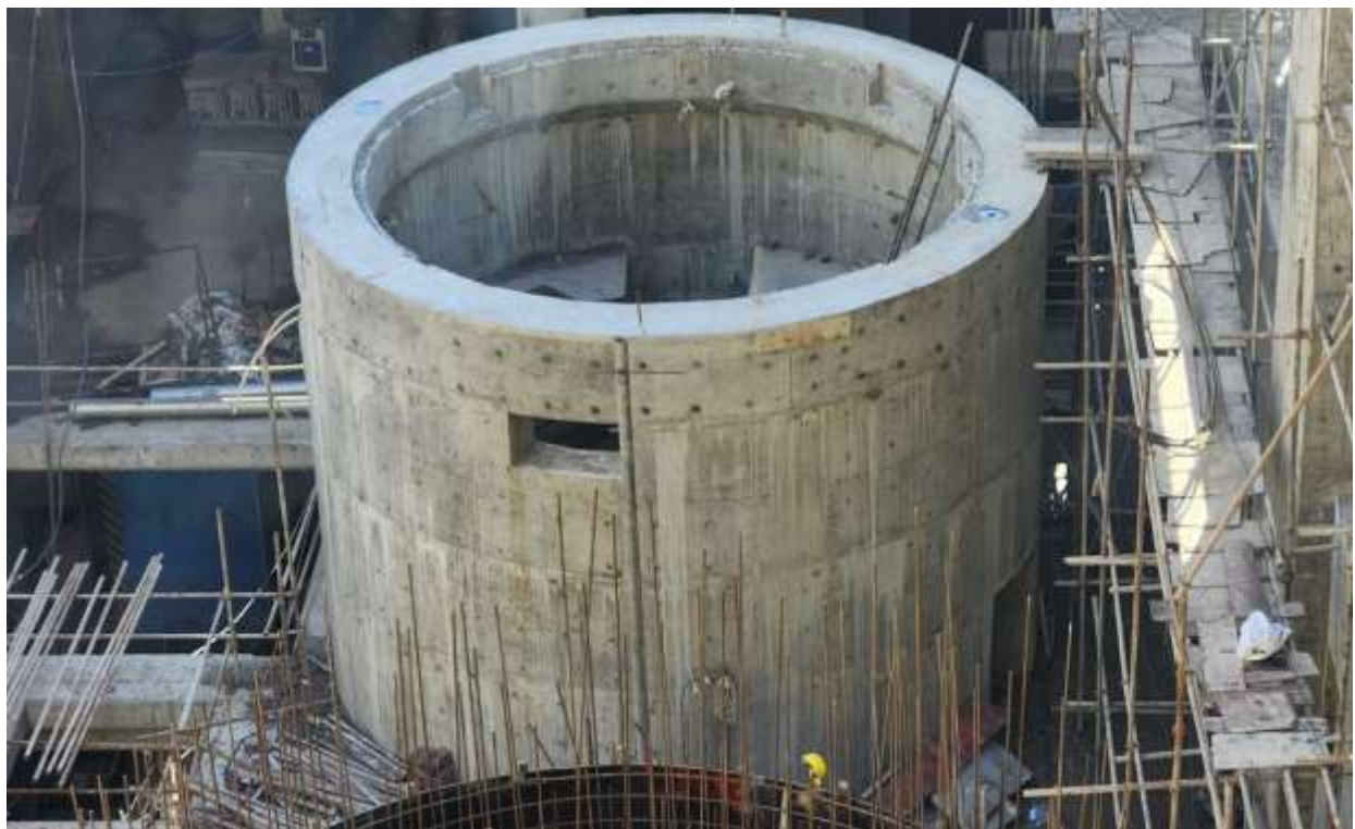
Figure 2-32: Casting of generator casing at unit 01
