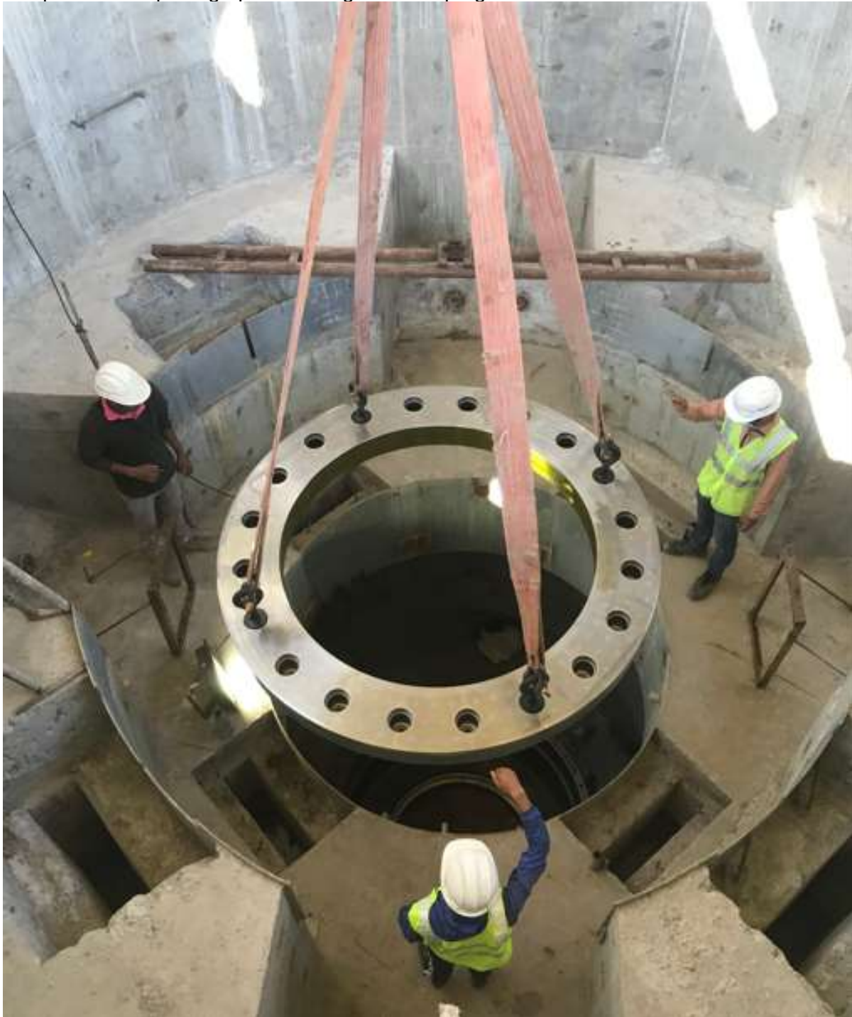
Figure 64: Bottom ring being lowered into the pit
