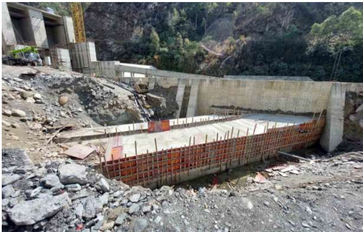
Figure 2-10: Gravel flushing culvert
