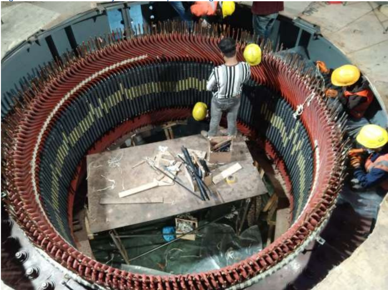
Figure 2-60: Stator winding works at near completion stage
