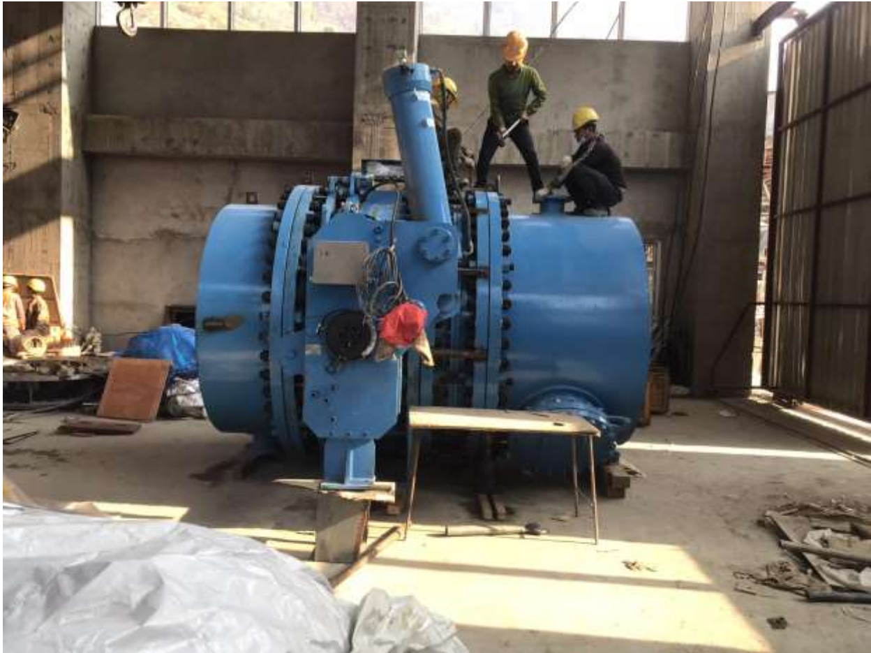
Figure 67: Unit 3 MIV assembled at Service bay
