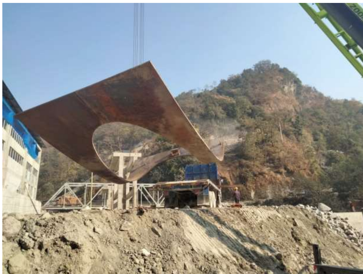
Figure 2-41: Erection of sickle plate for bifurcation 01
