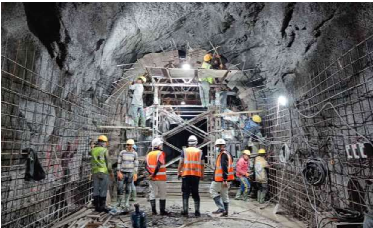
Figure 2-18: Assembling of formwork for full concrete lining at connecting tunnel 03
