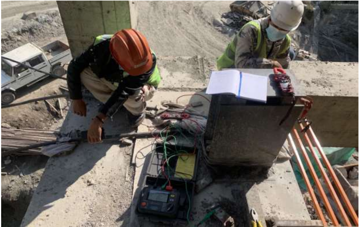
Figure 2-57: Insulation Resistance of EOT's busbar
