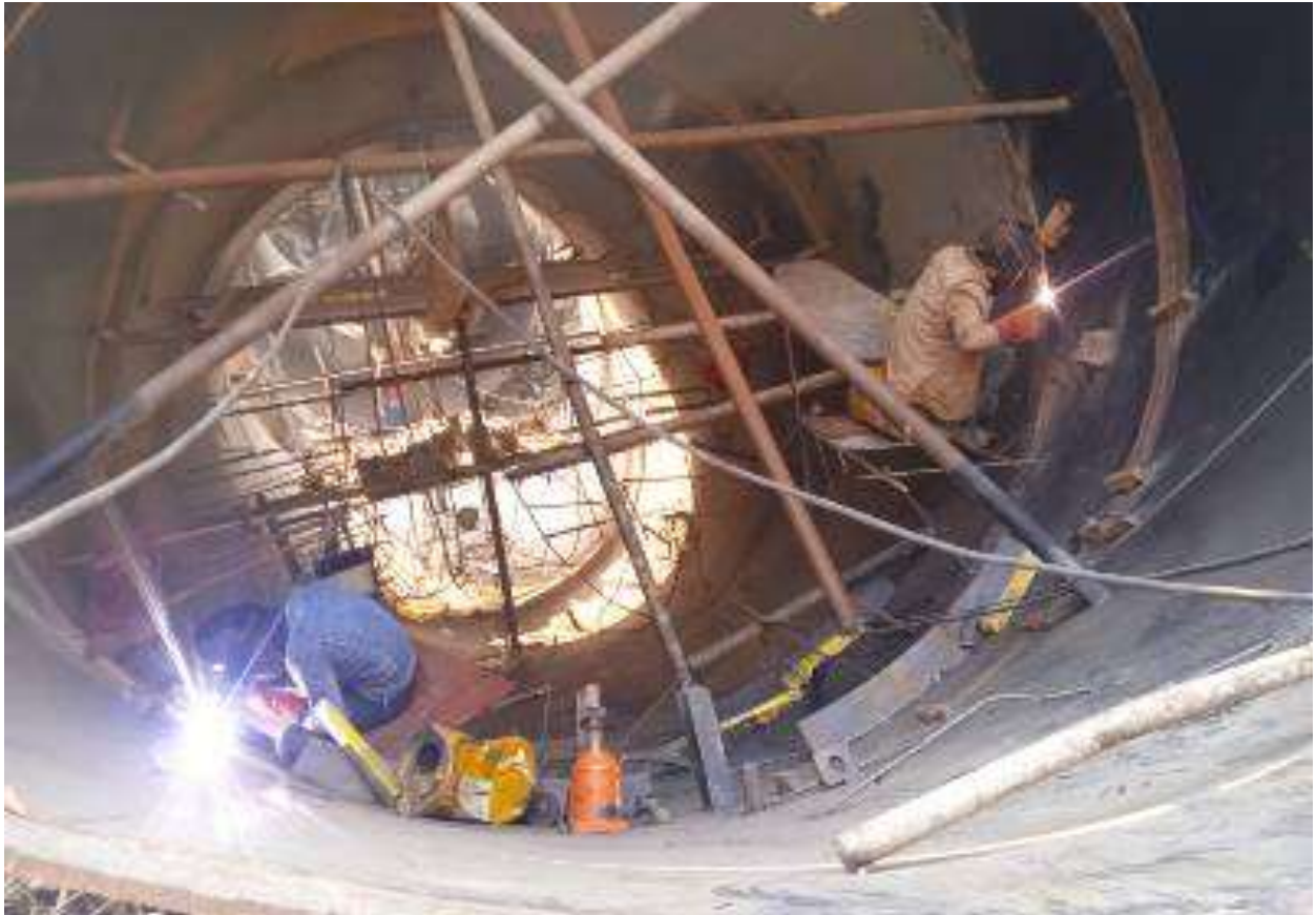
Figure 2-37: Welding work ongoing inside incline pipe at powerhouse
