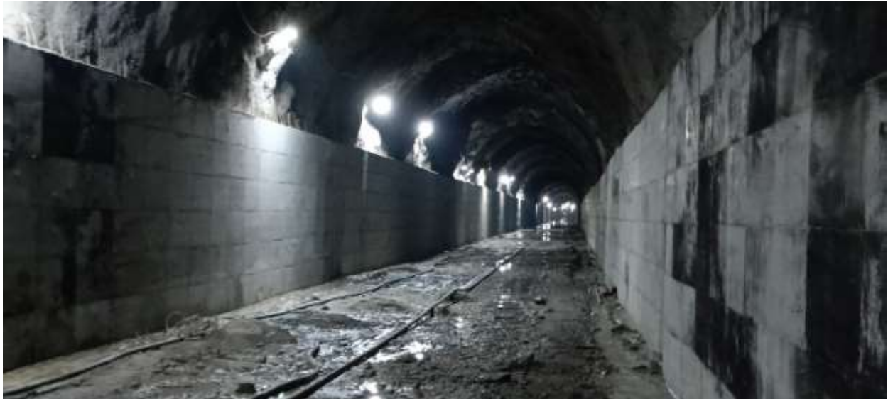
Figure 2-14: A section of HRT with partial concrete lining
