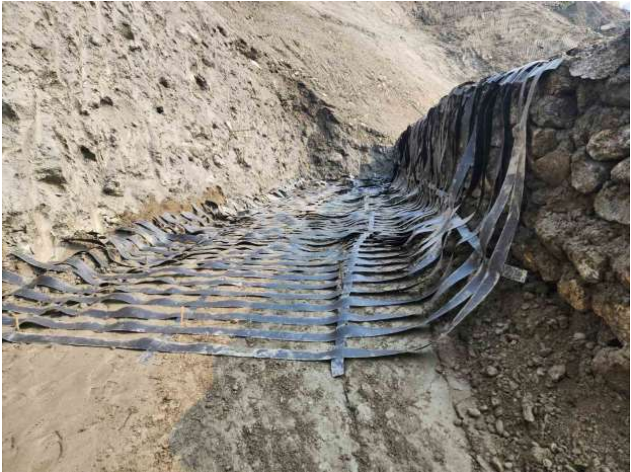
Figure 2-29: Penstock slope stablization using geogrid (paralink)
