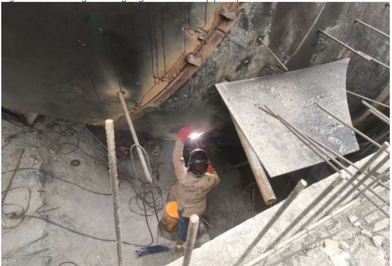
Figure 2-38: Welding work at pipe of dia 4.5 m and thk 32 mm from outside
