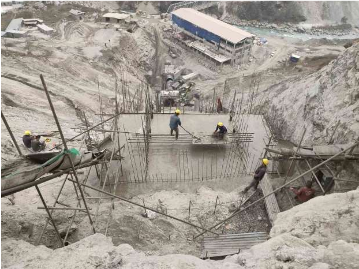
Figure 2-27: Concreting of anchor block
