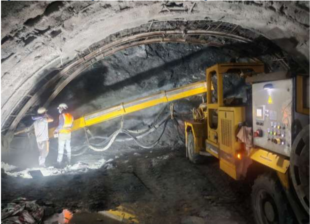
Figure 2-24: Application of shotcrete on the left crown of SB 03 using robotic shotcrete machine
