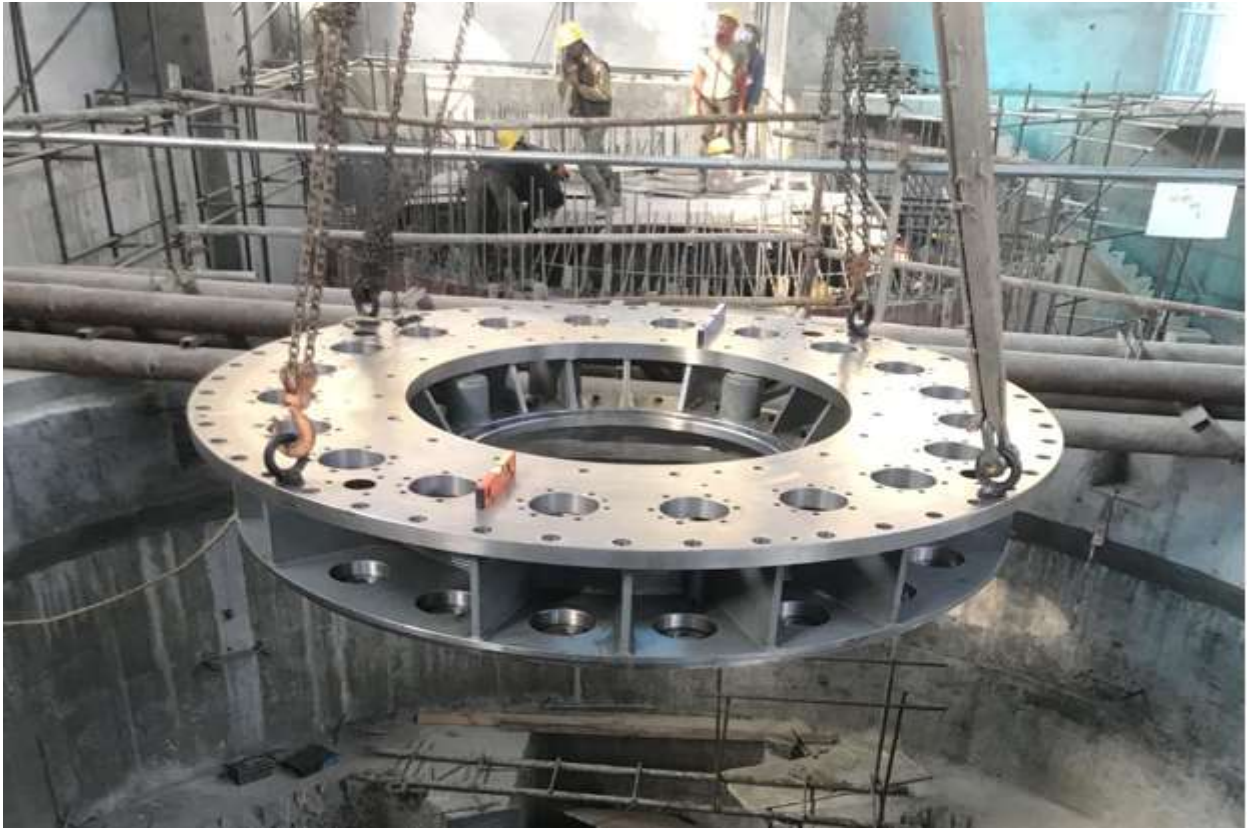
Figure 62: Lowering of Head cover
