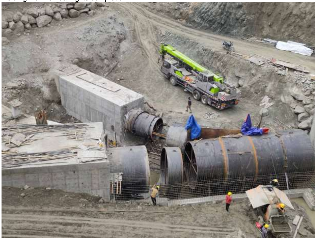
Figure 2-40: Erection of bifurcation unit 01
