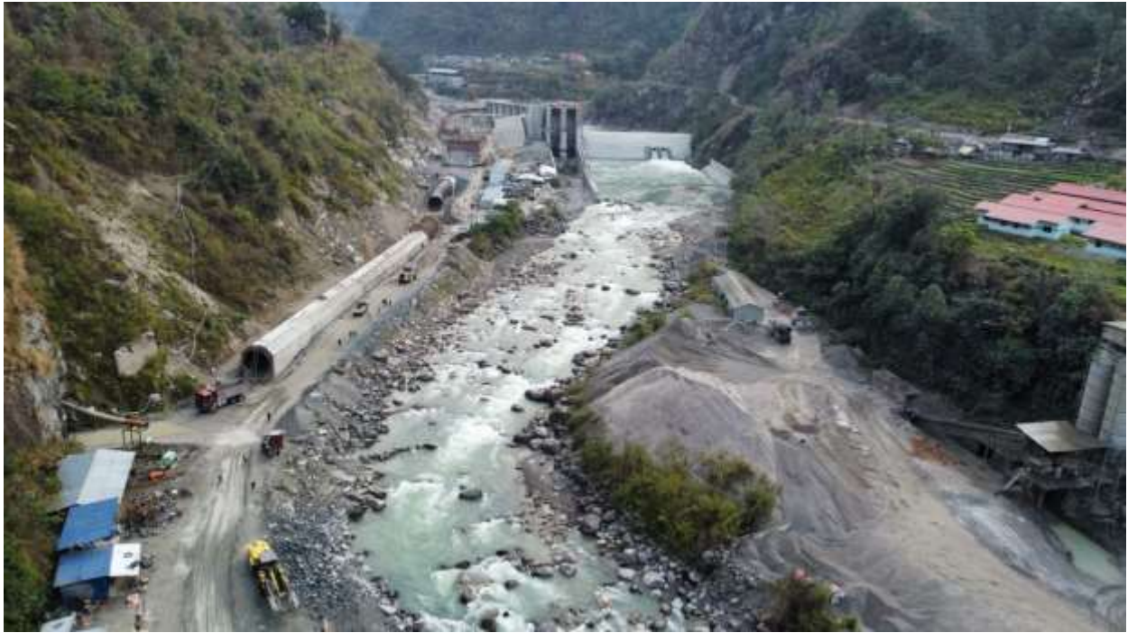
Figure 2-11: Erection of concrete encased approach pipe
