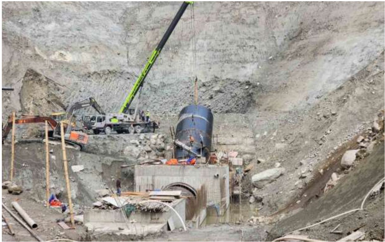
Figure 2-35: A view of erection of penstock pipe (thickness 32 mm)
