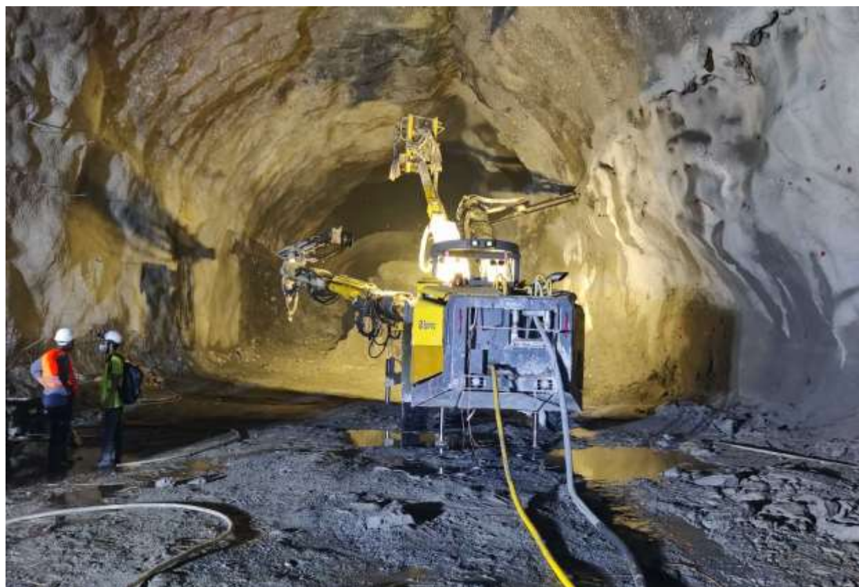
Figure 2-17: Final stage of rock bolt installation works
