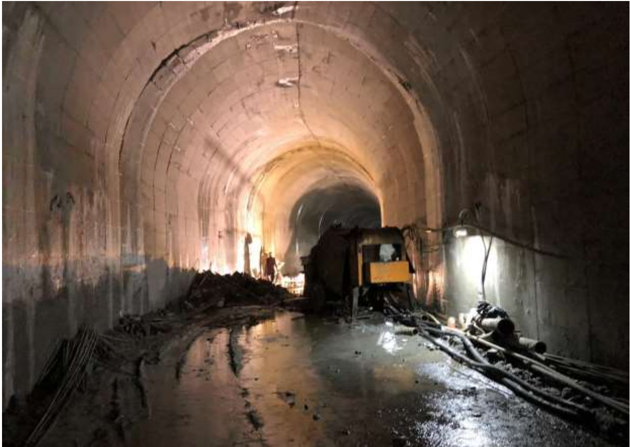
Figure 2-19: Full lining section at HRT bends
