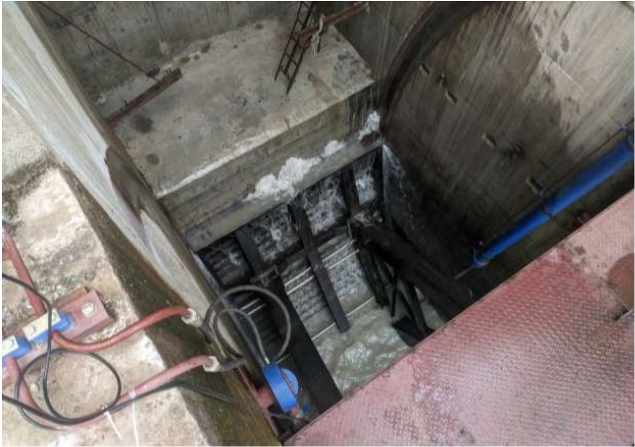
Figure 2-37: Erection of radial gate at undersluice
