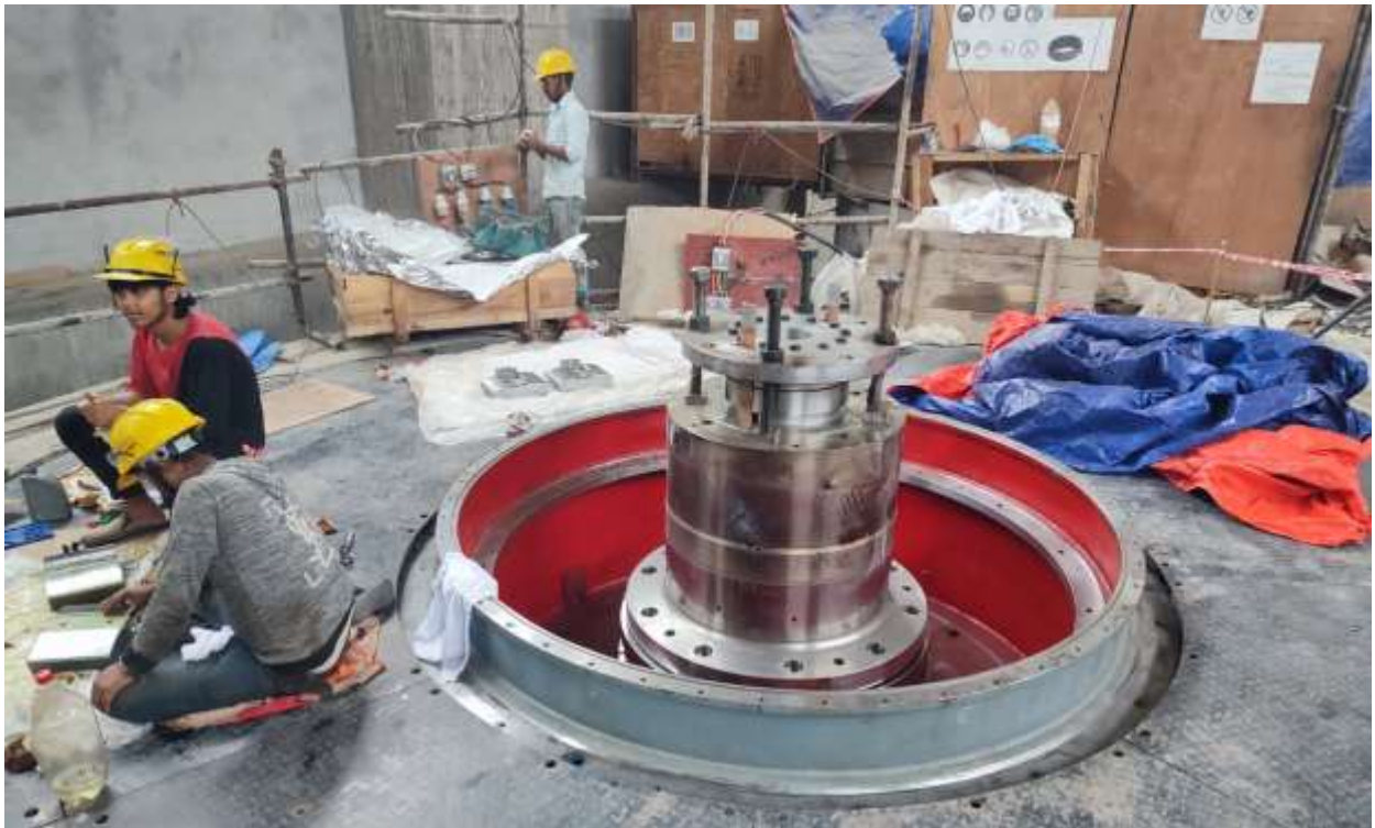
Figure 2-53: Overview of thrust bearing
