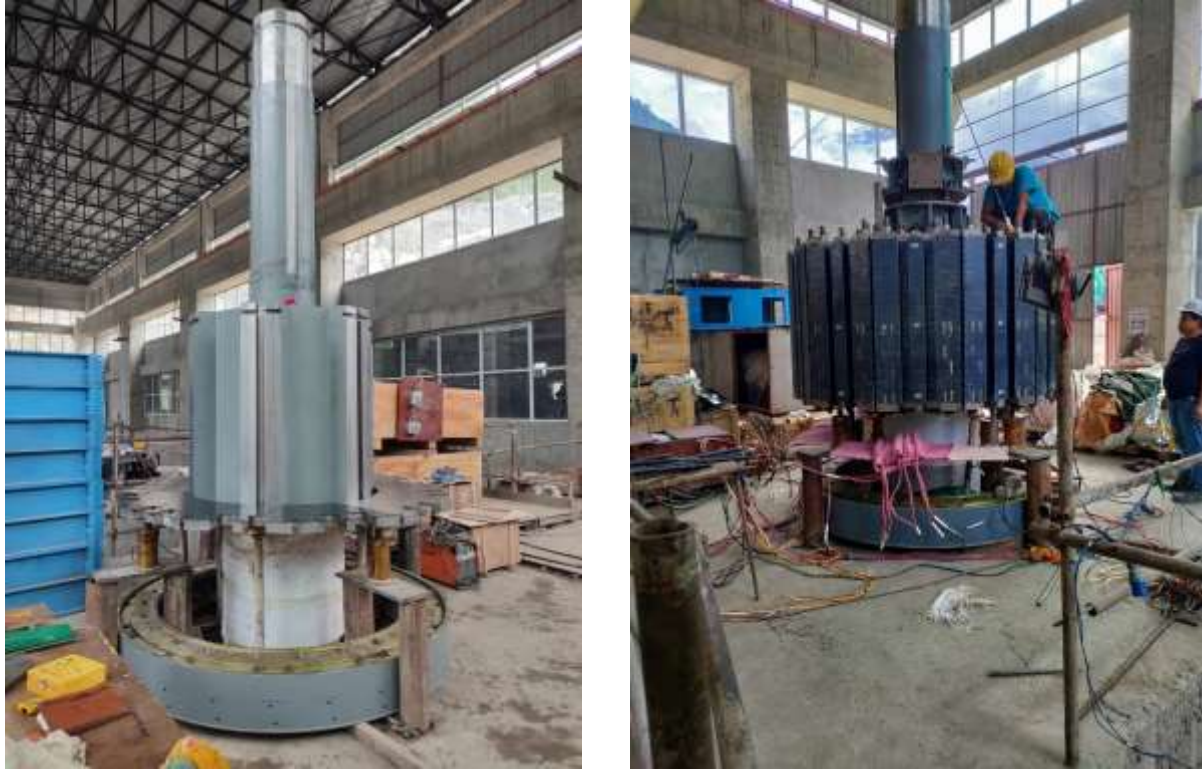
Figure 2-56: Different stages of rotor assembly
