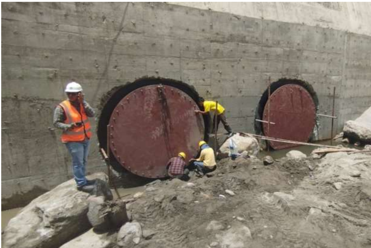
Figure 2-38: Plugging of openings at weir
