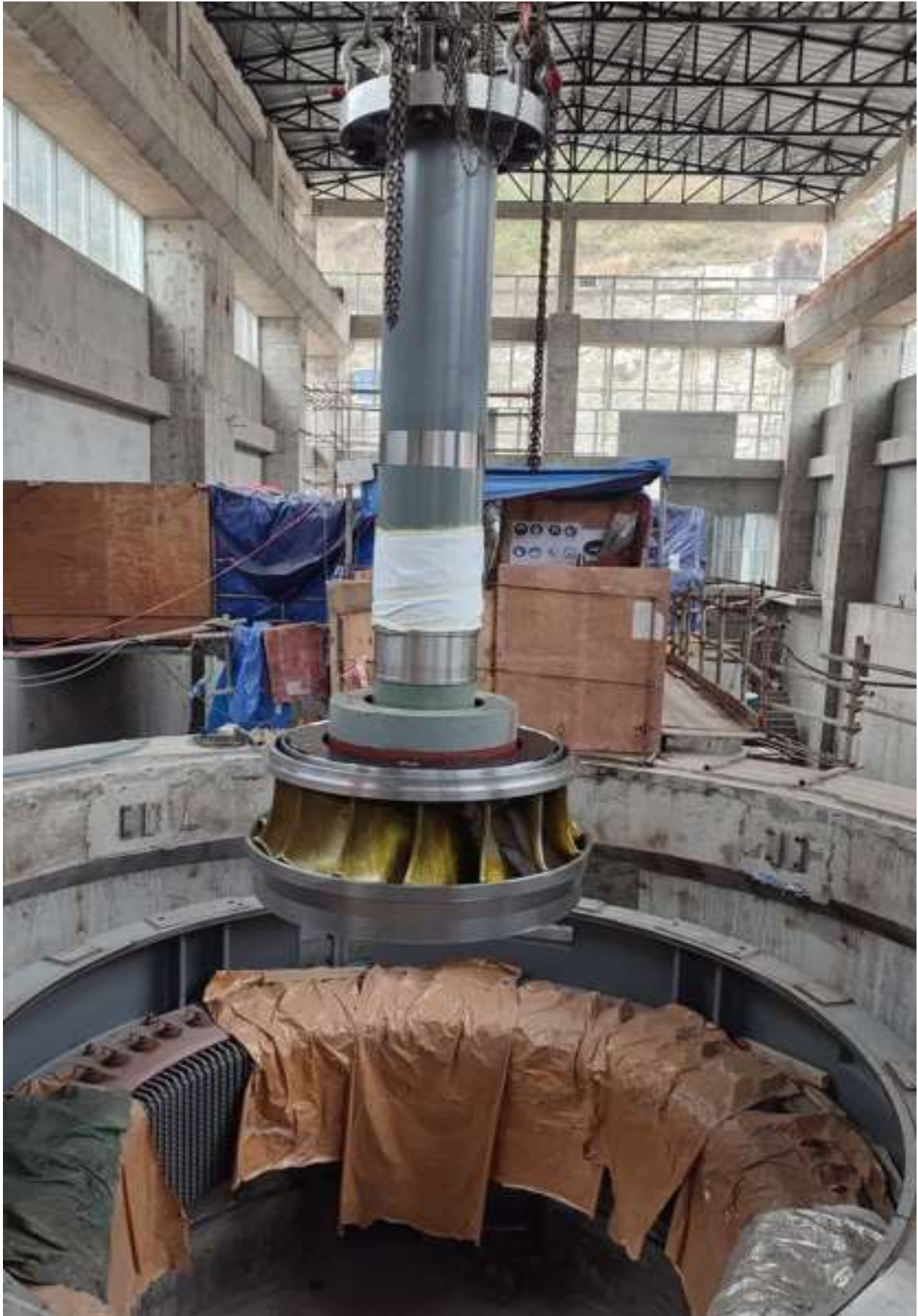
Figure 2-51: Final assembly and lowering of runner with main shaft in unit 2
