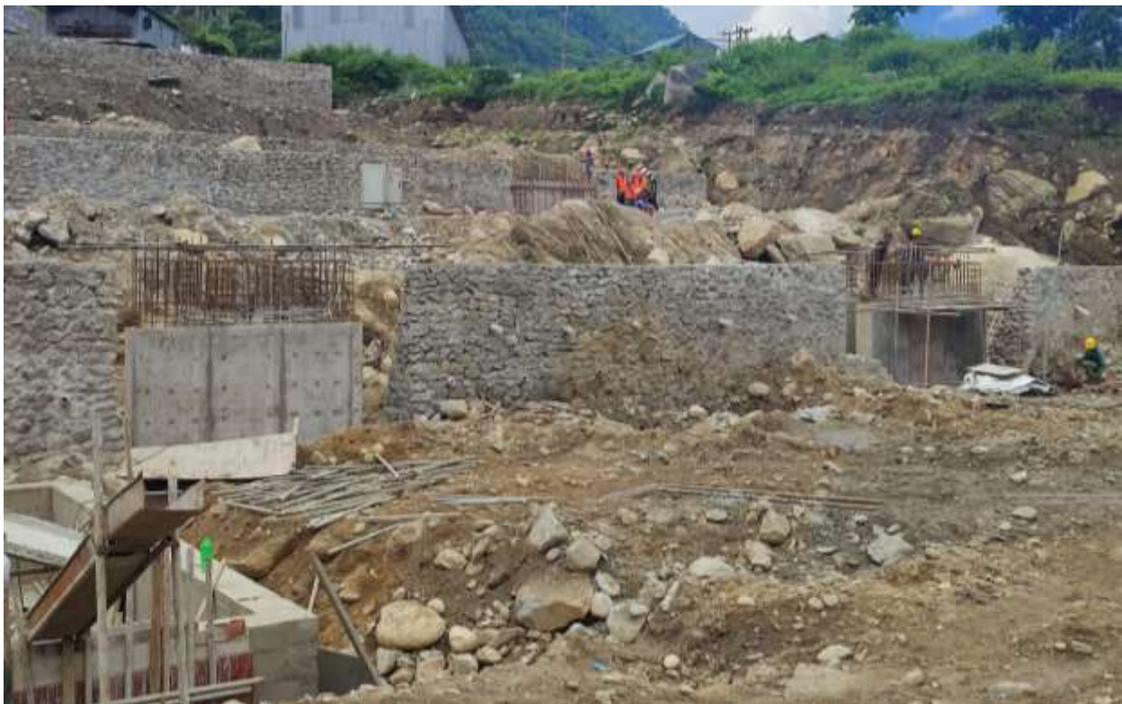
Figure 2-67: Gantry foundation
