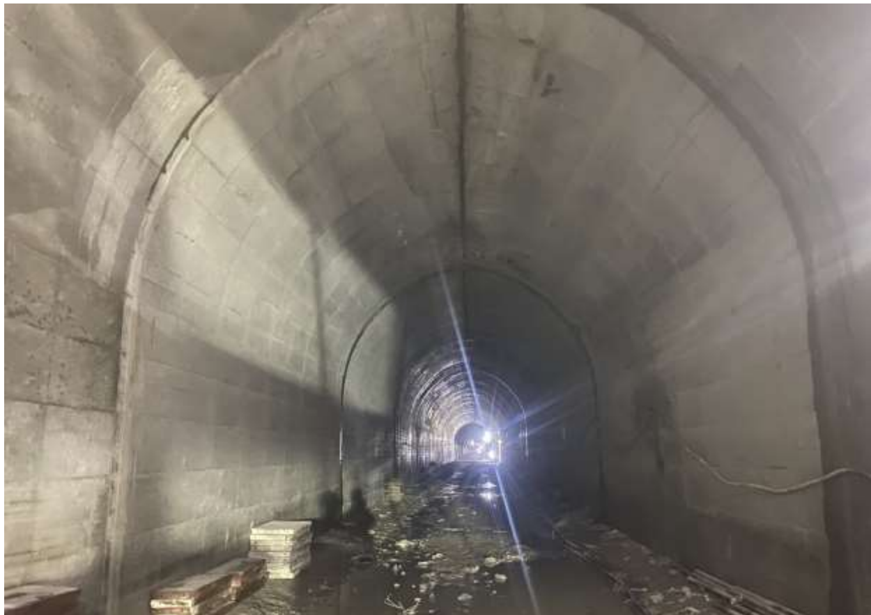
Figure 2-18: A section of HRT with concrete full lining
