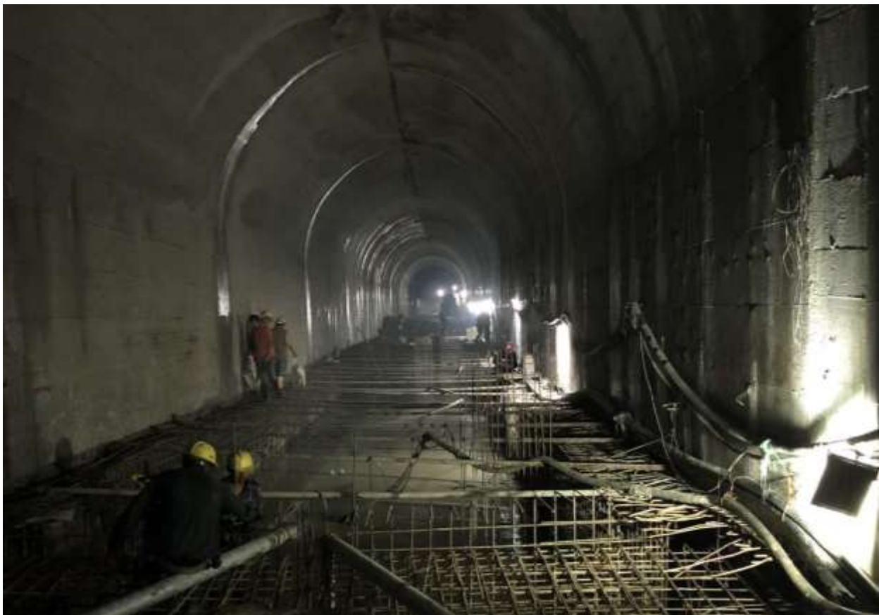
Figure 2-20: Concrete lining works at rock trap
