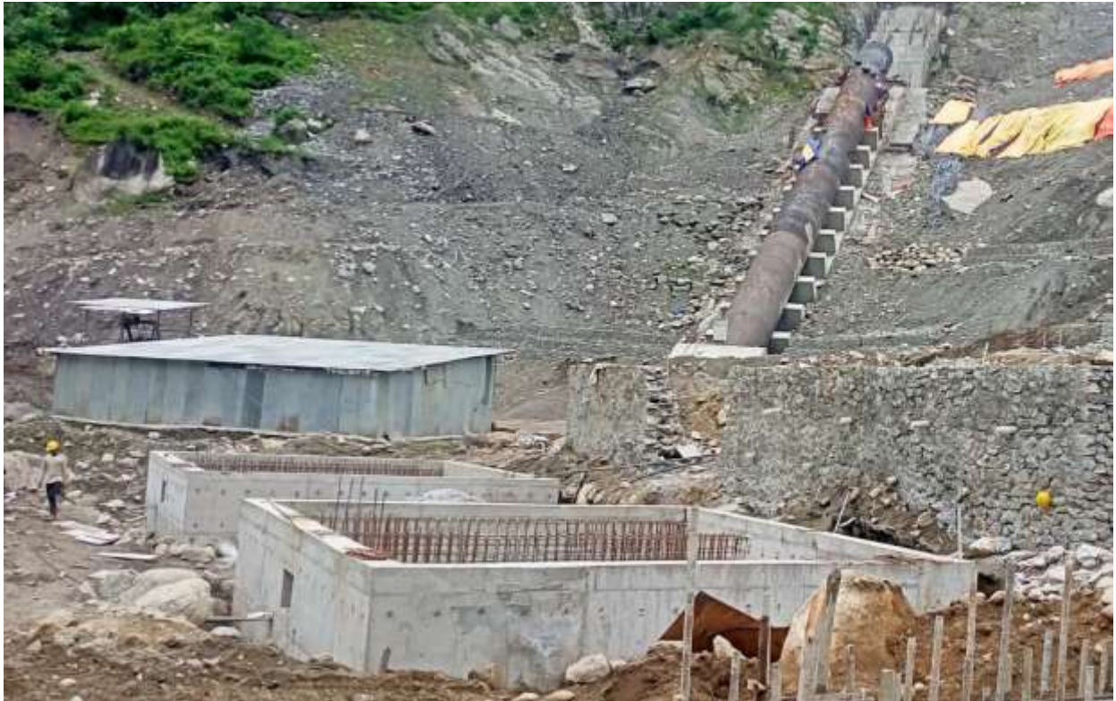
Figure 2-32: Construction of transformer foundation
