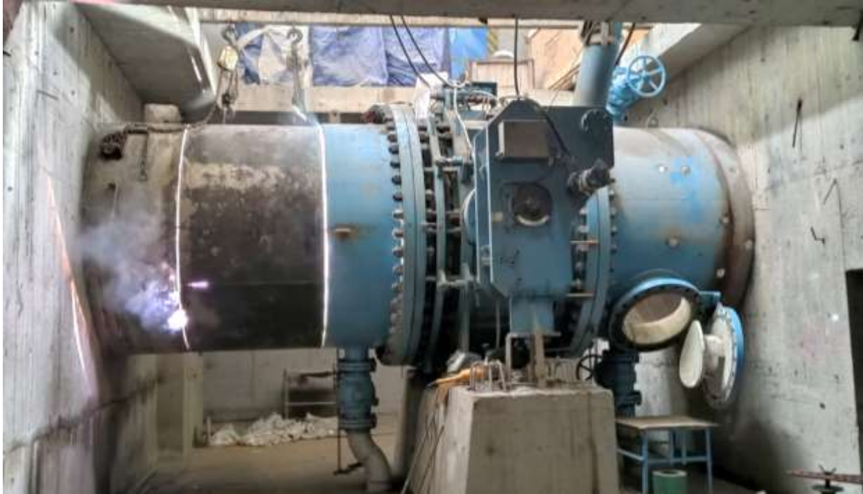
Figure 2-57: Unit 01 cut piece erection and welding
