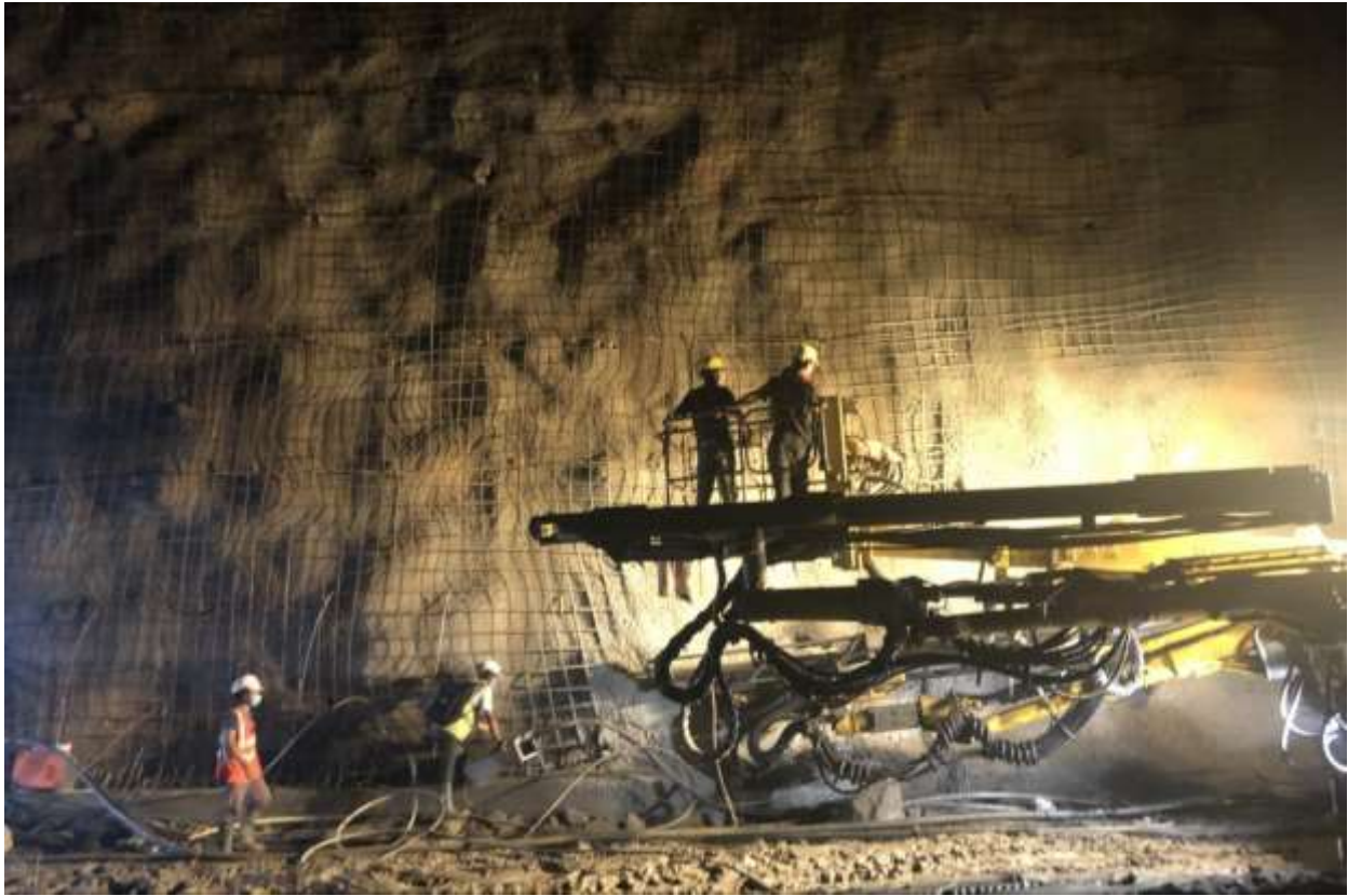
Figure 2-12: A view of wire mesh shotcrete work at Settling Basin 01
