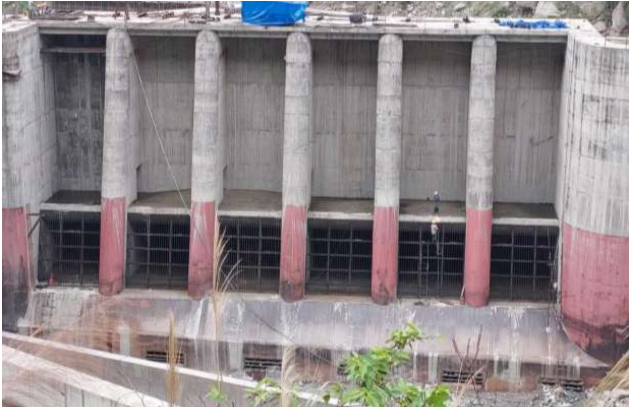
Figure 2-4: A front view of intake orifices
