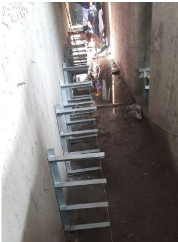
Figure 2-61: Installation of cable support bracket and control panel base
