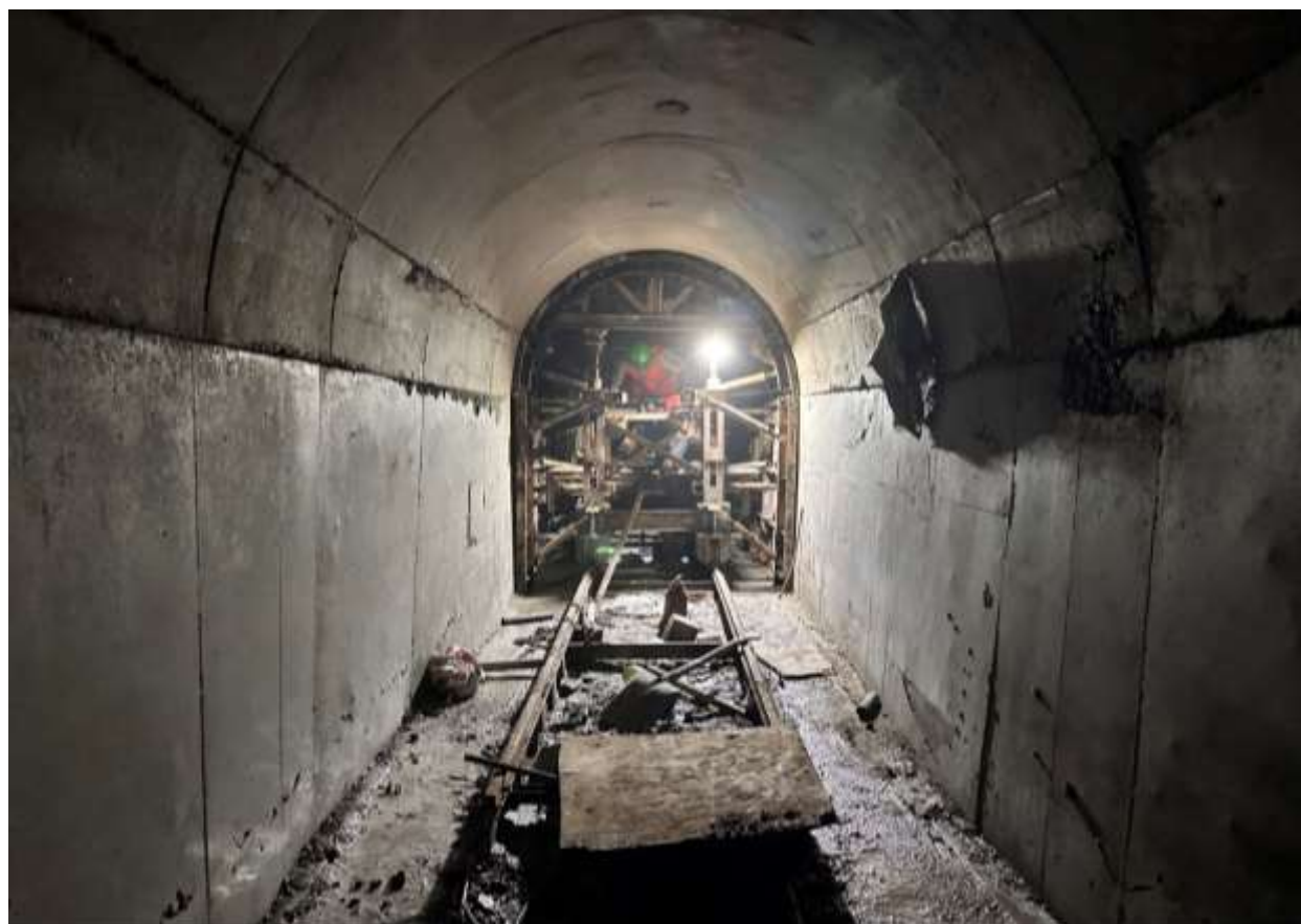
Figure 2-25: A view of full concrete lining at the flushing tunnel
