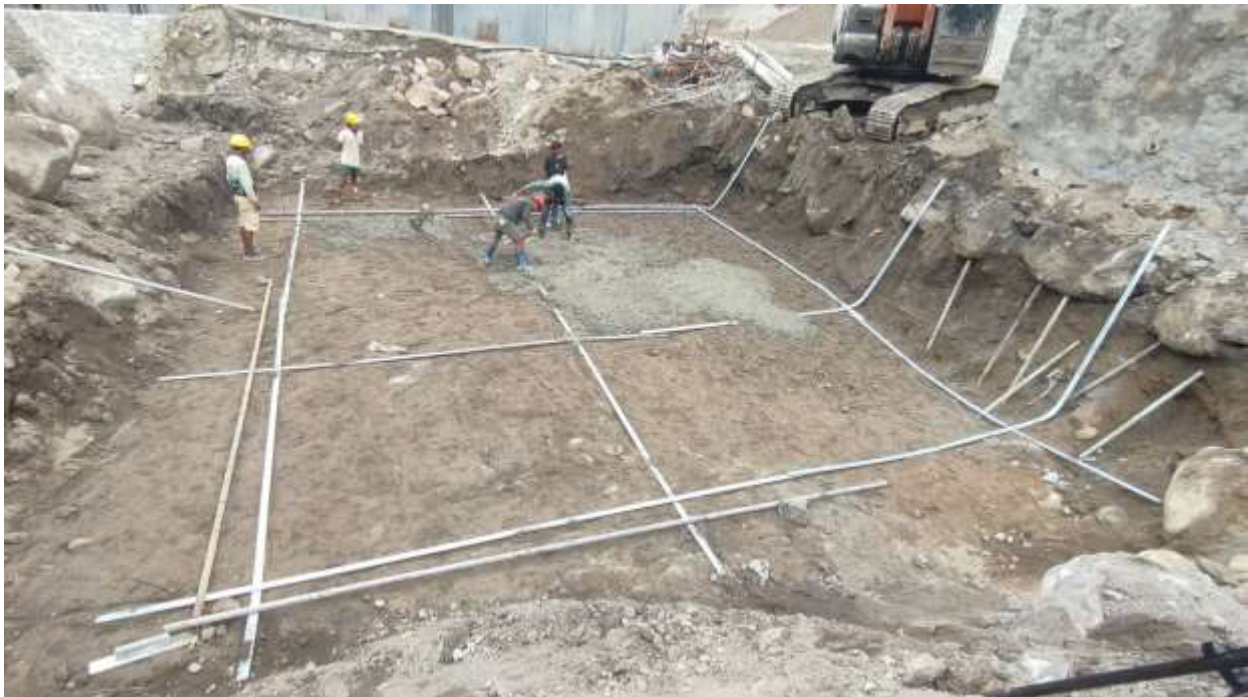
Figure 2-63: Laying of earthing plates for transformer foundation
