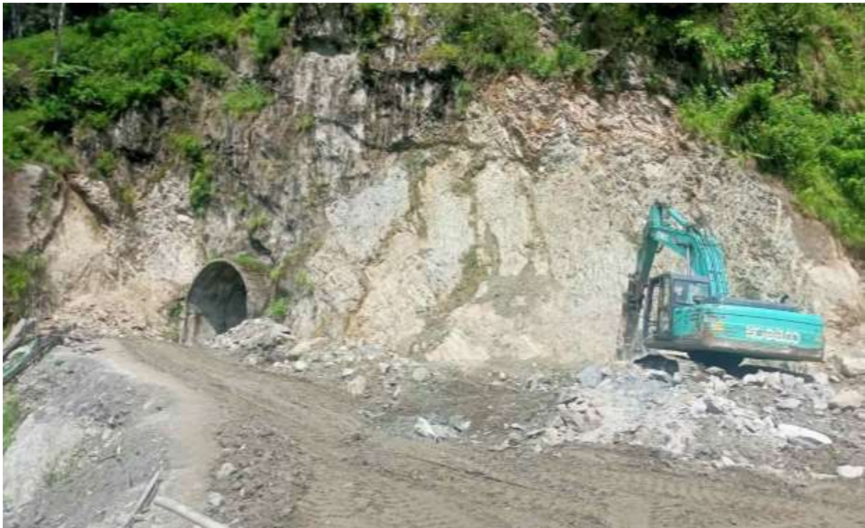
Figure 2-31: Excavation of valve house region
