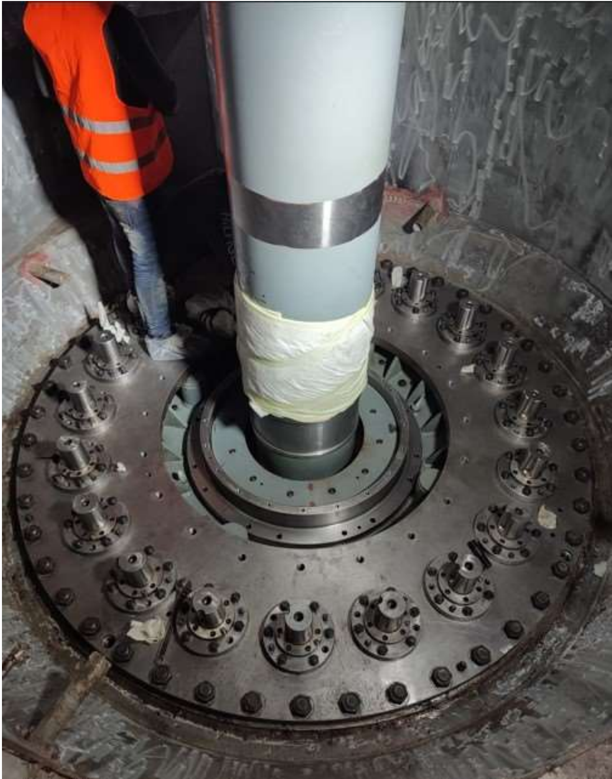
Figure 2-50: Final assembly of bottom ring, guide vane, head cover and main shaft with runner
