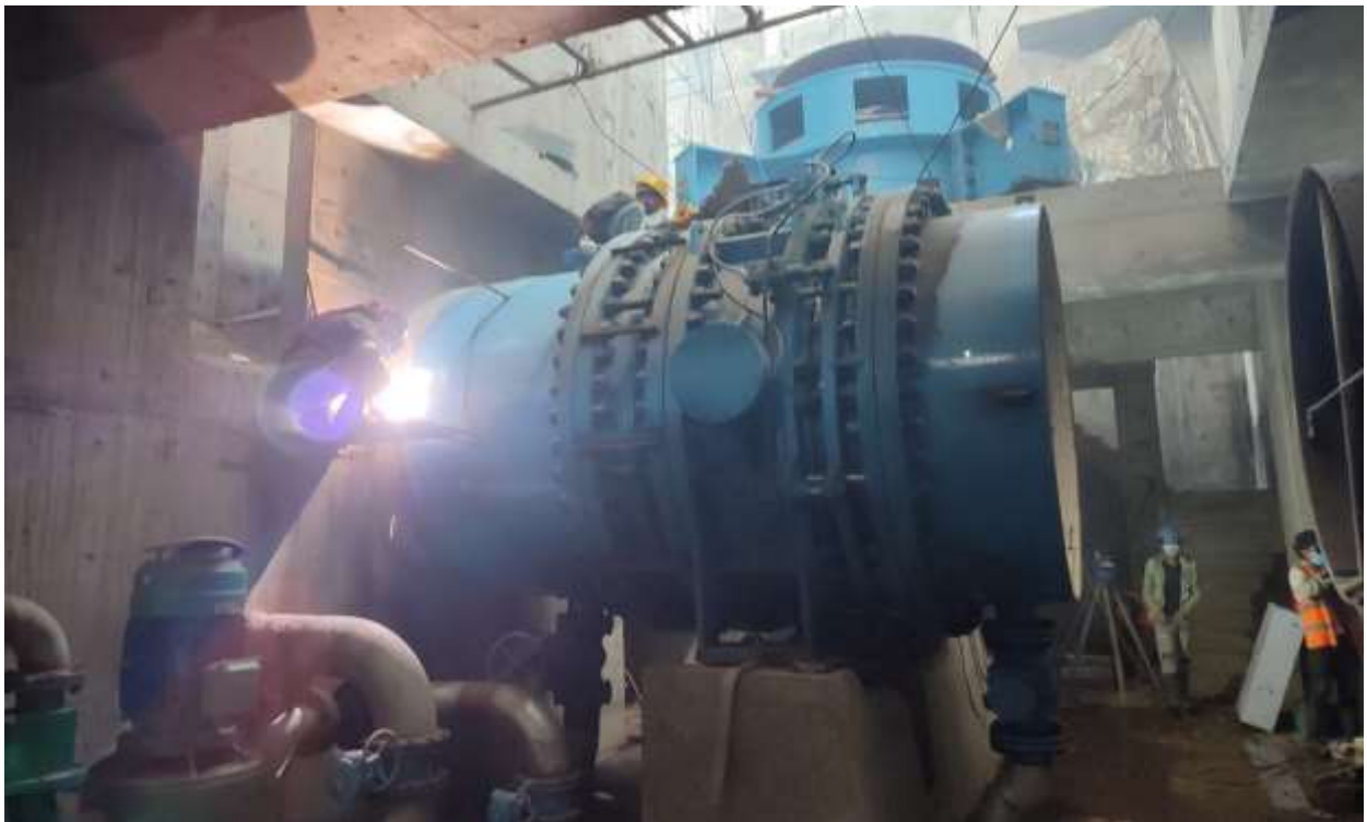
Figure 2-60: Unit 04 downstream side welding
