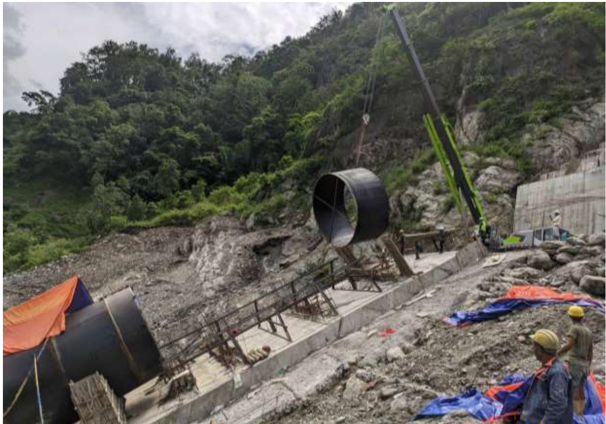
Figure 2-35: Erection of penstock pipes
