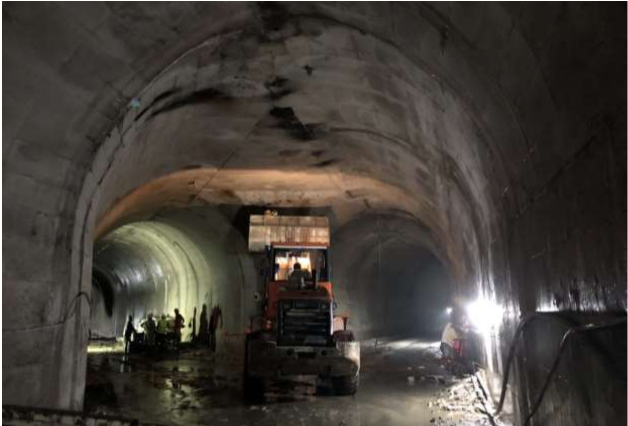
Figure 2-23: Full concrete lining at the junction of connecting tunnel and HRT
