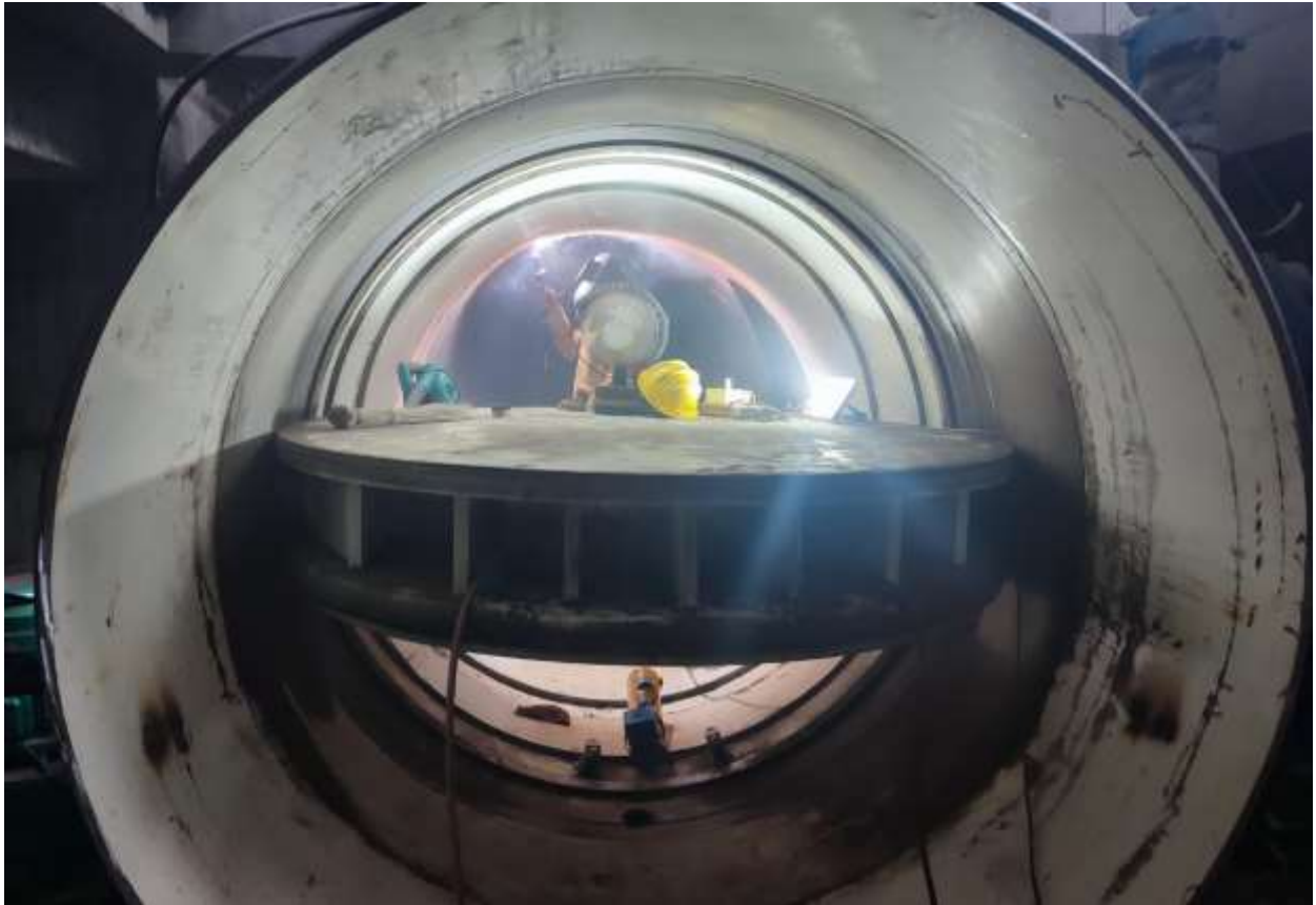
Figure 2-59: Unit 03 downstream side welding
