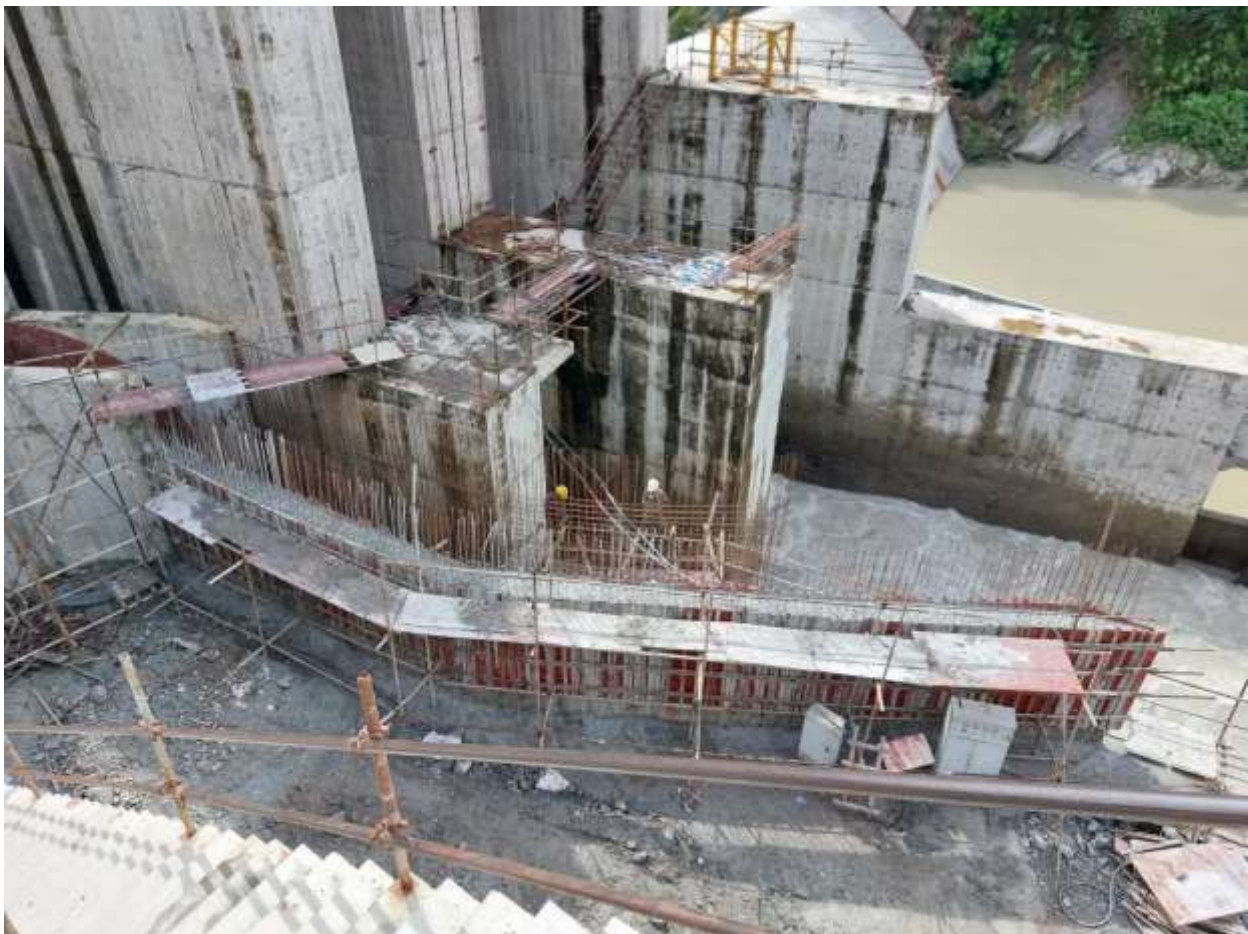
Figure 2-11: Construction of bed load sluice culvert
