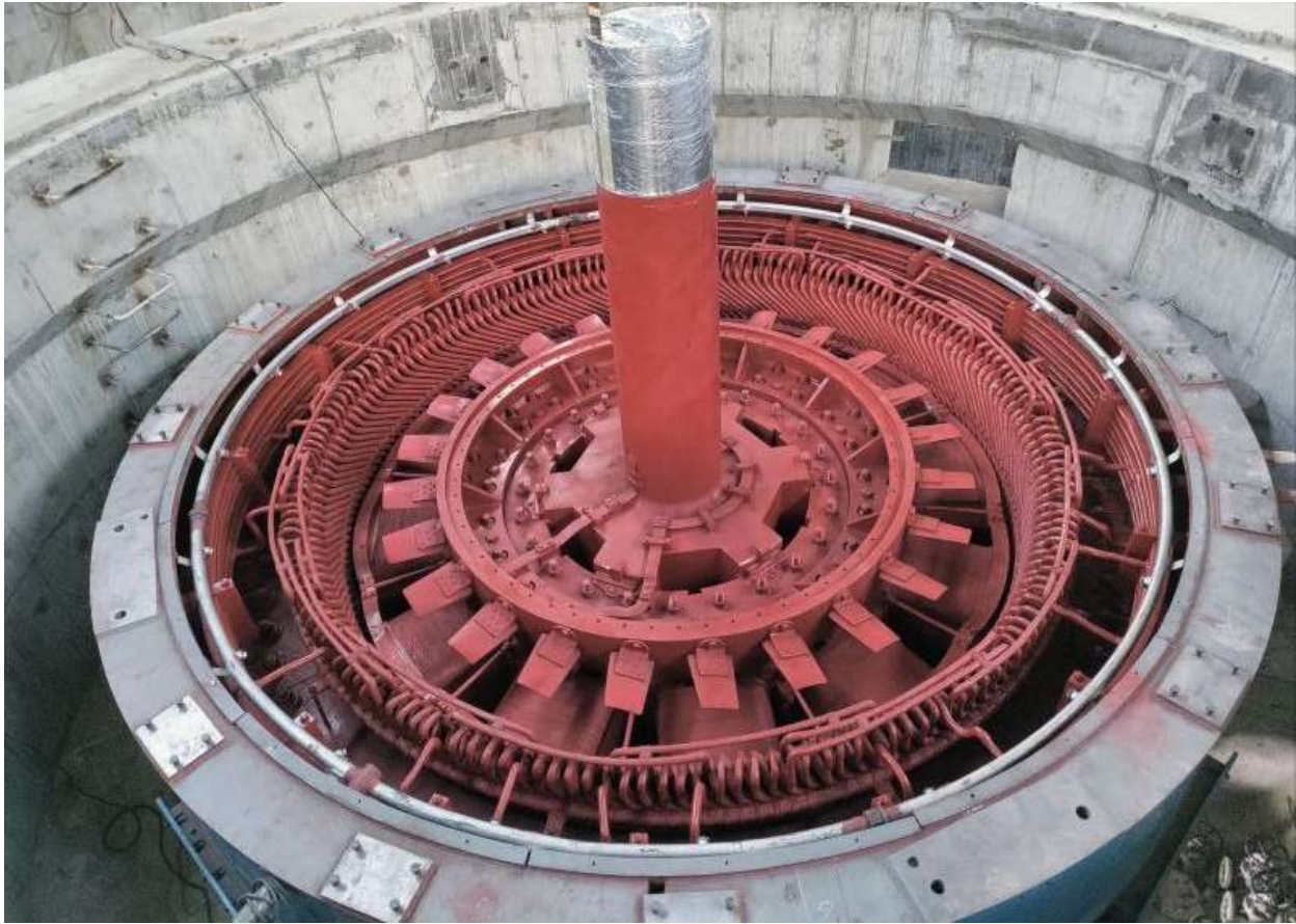
Figure 2-46: Rotor and stator coupling in unit 01
