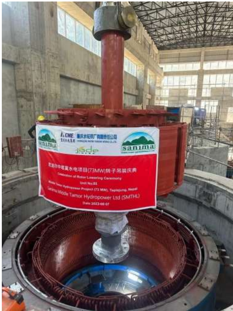
Figure 2-44: Rotor lowering at unit 01
