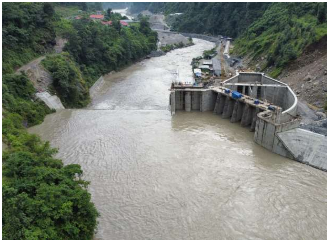
Figure 2-3: Aerial view of Headworks during closing of gates
