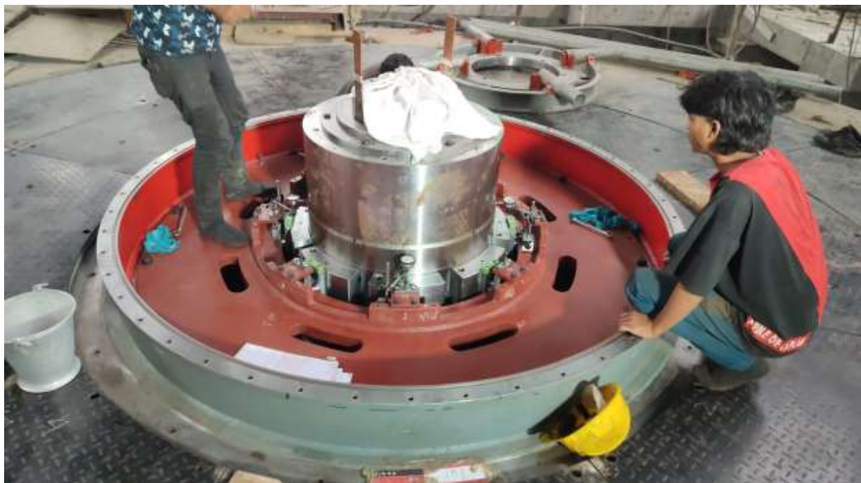
Figure 2-45: Alignment check after thrust and guide bearing installation
