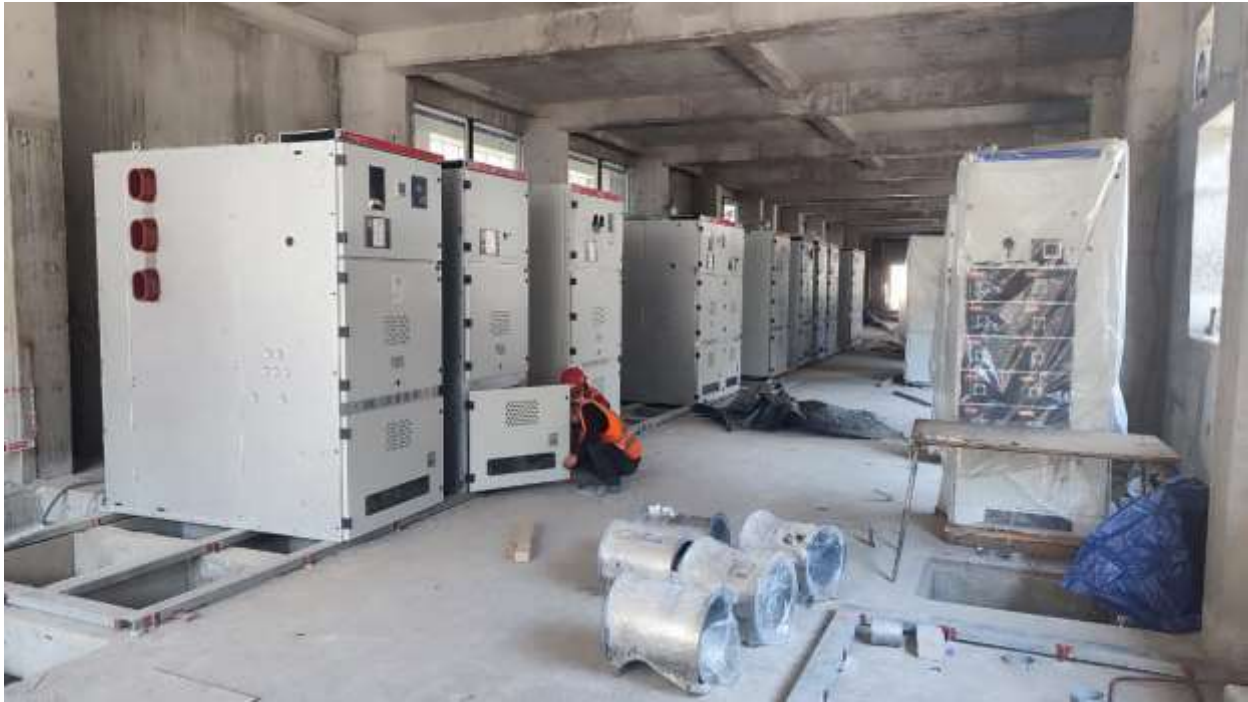
Figure 70: Installation of 11 kV switchgear panels
