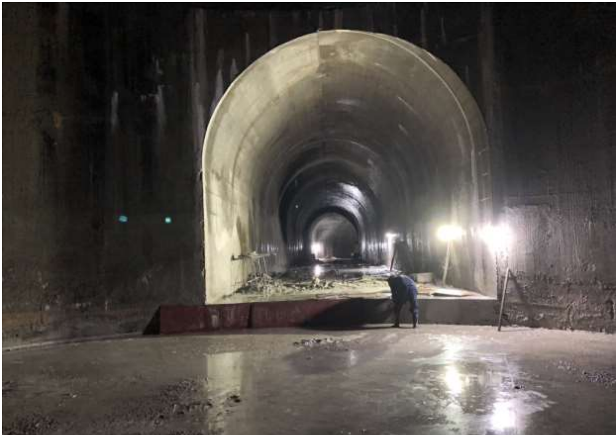
Figure 2-22: A view of full lining concrete at connecting tunnel of Surge Shaft
