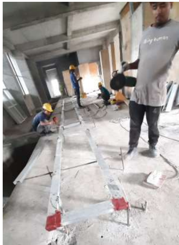
Figure 2-61: Installation of cable support bracket and control panel base
