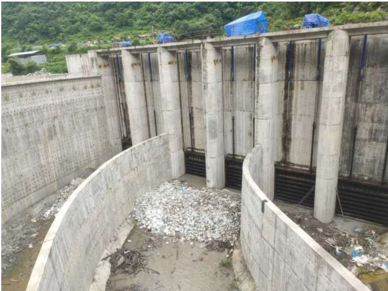
Figure 2-5: A view of intake from downstream and intake canal
