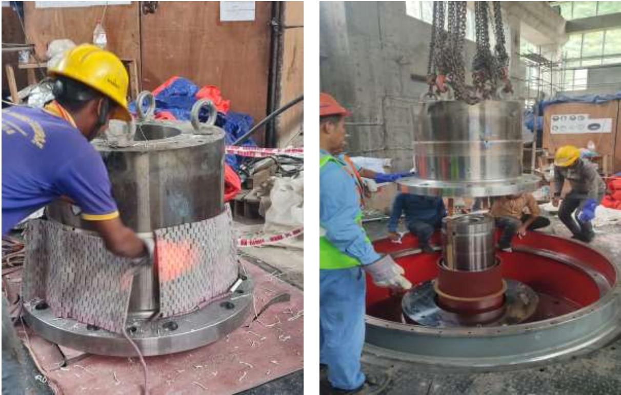
Figure 61: Different stages of thrust bearing installation
