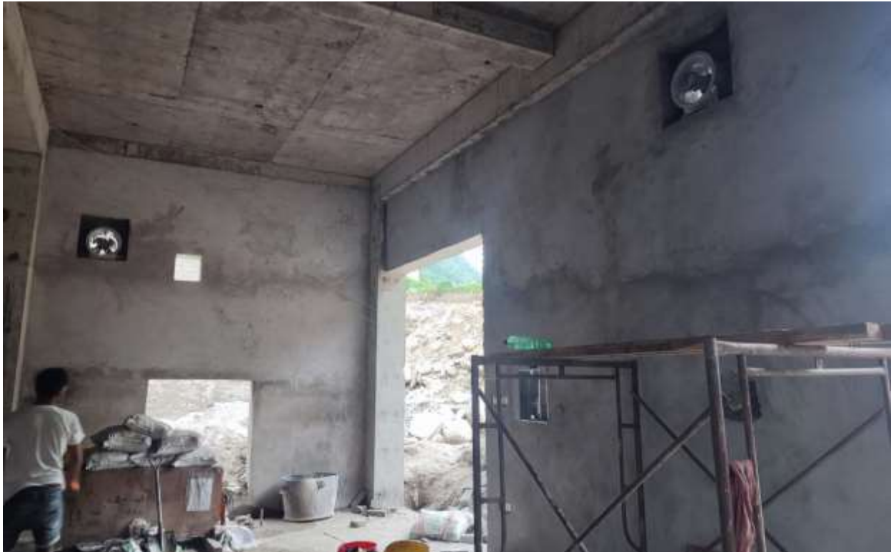
Figure 2-62: Installation of ventilating fans
