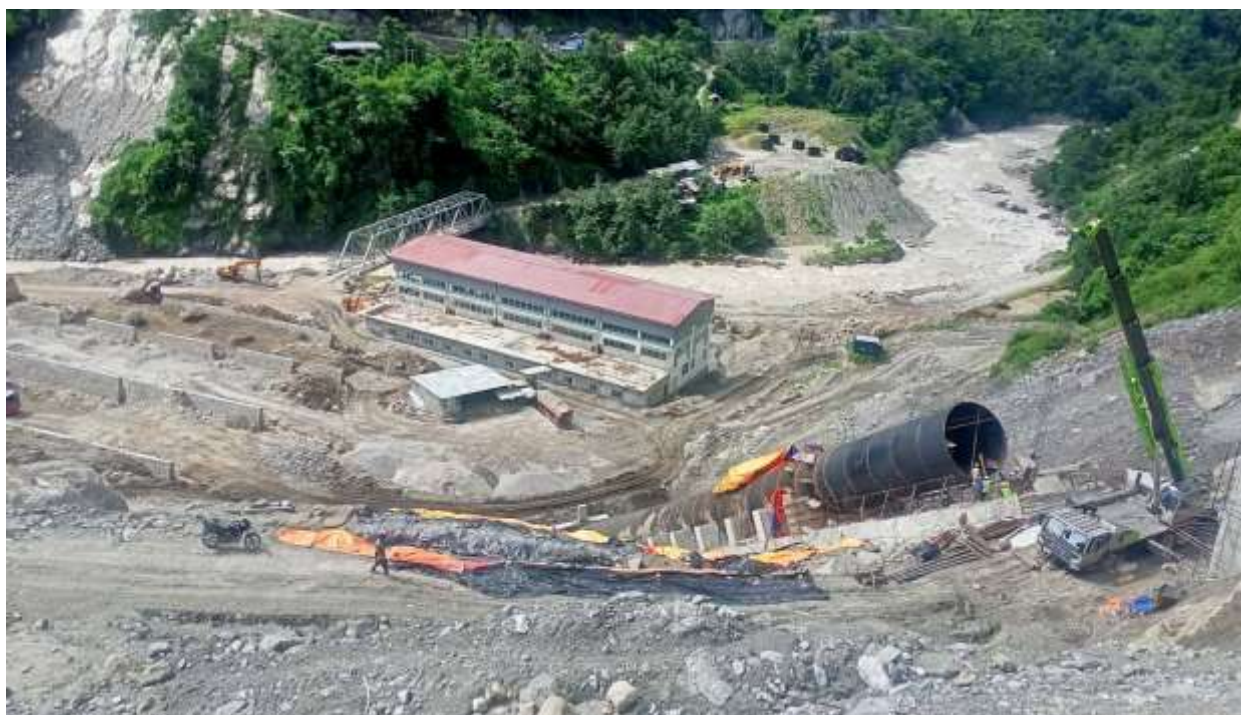
Figure 2-27: A view of backfilling works at the manifold region
