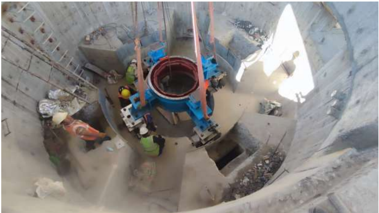
Figure 2-49: Preassembly of Lower bracket
