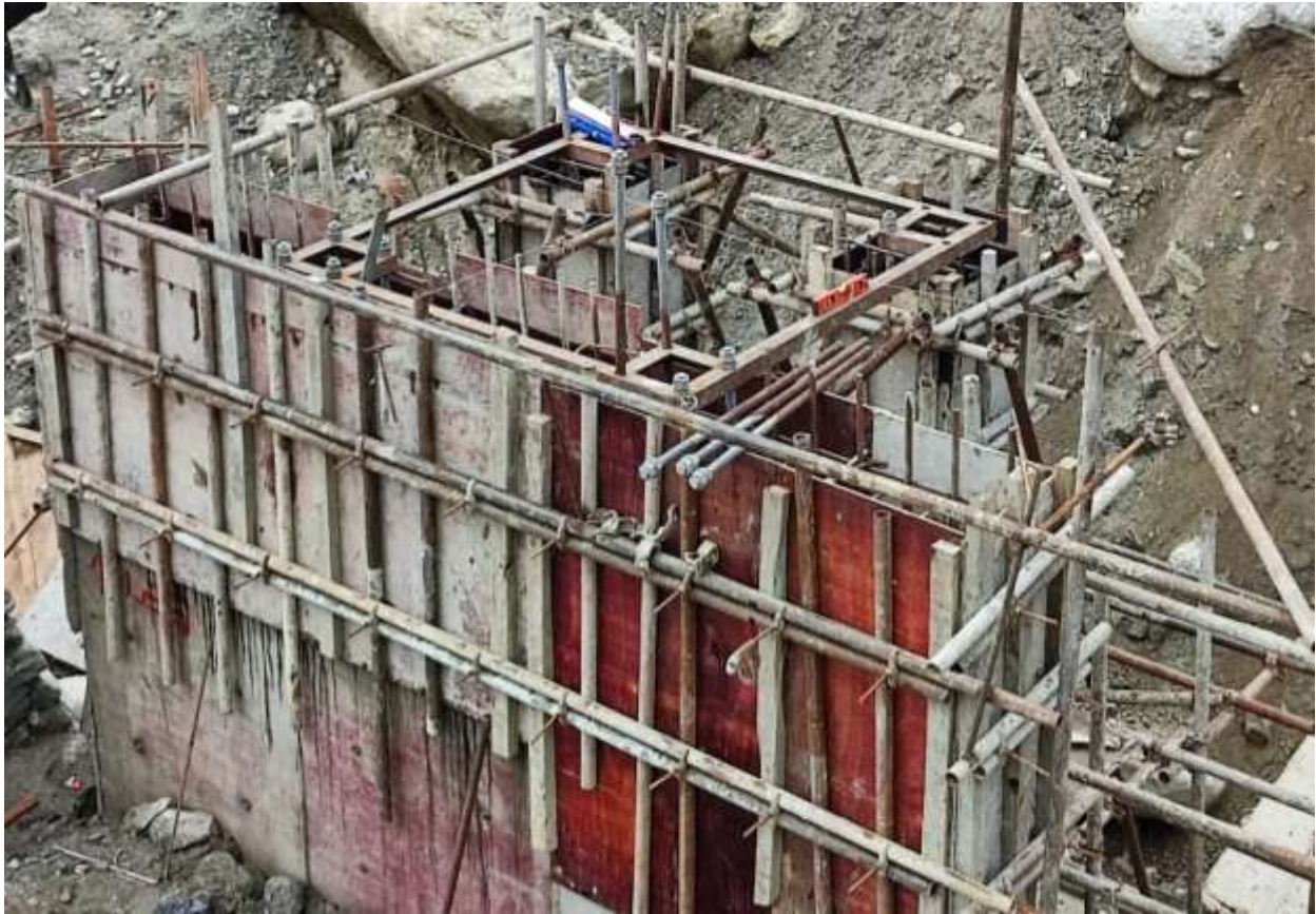
Figure 2-66: Anchor bolt fixing for gantry foundation
