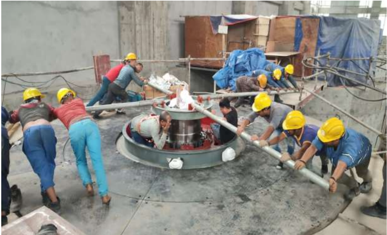
Figure 54: Run out check after shaft coupling
