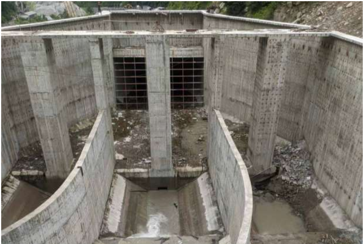
Figure 2-8: A view of gravel trap and conveyance tank
