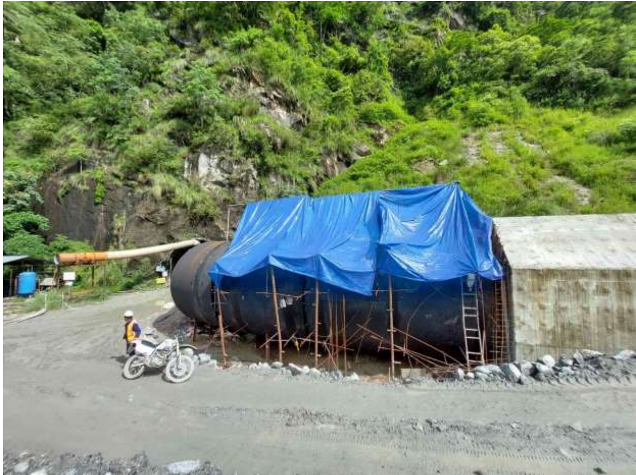
Figure 2-34: Installation of head race bend
