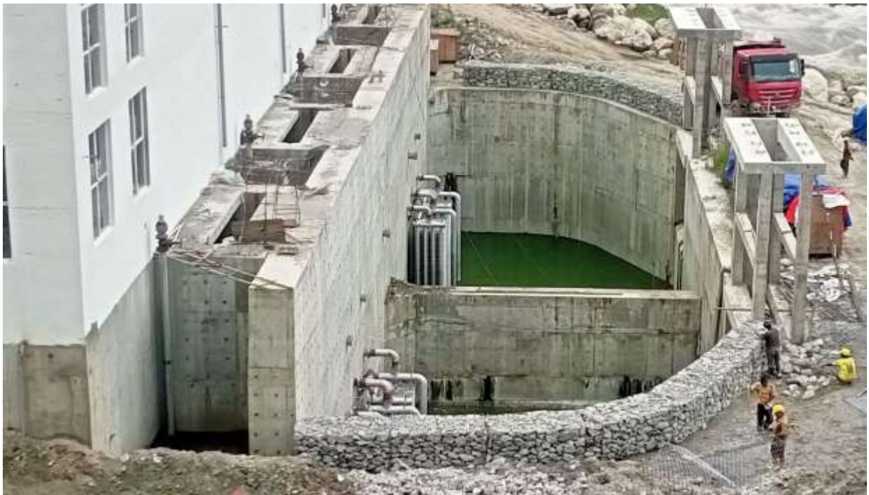
Figure 2-33: A view of gabion works under going at tailrace chamber region
