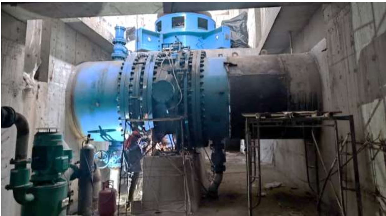
Figure 2-58: Unit 02 cut piece erection
