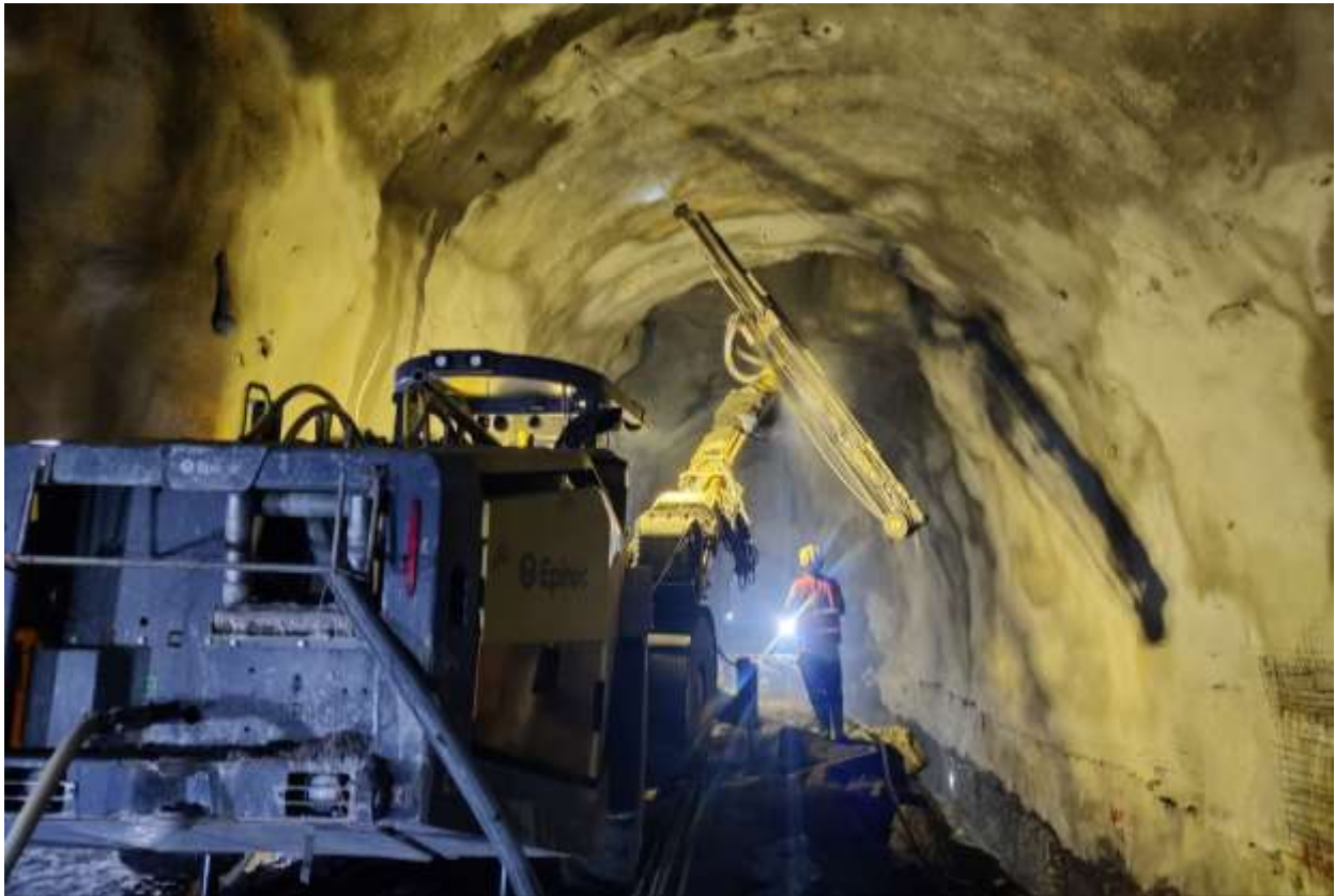
Figure 2-16: Additional Rock bolt installation in SB 03
