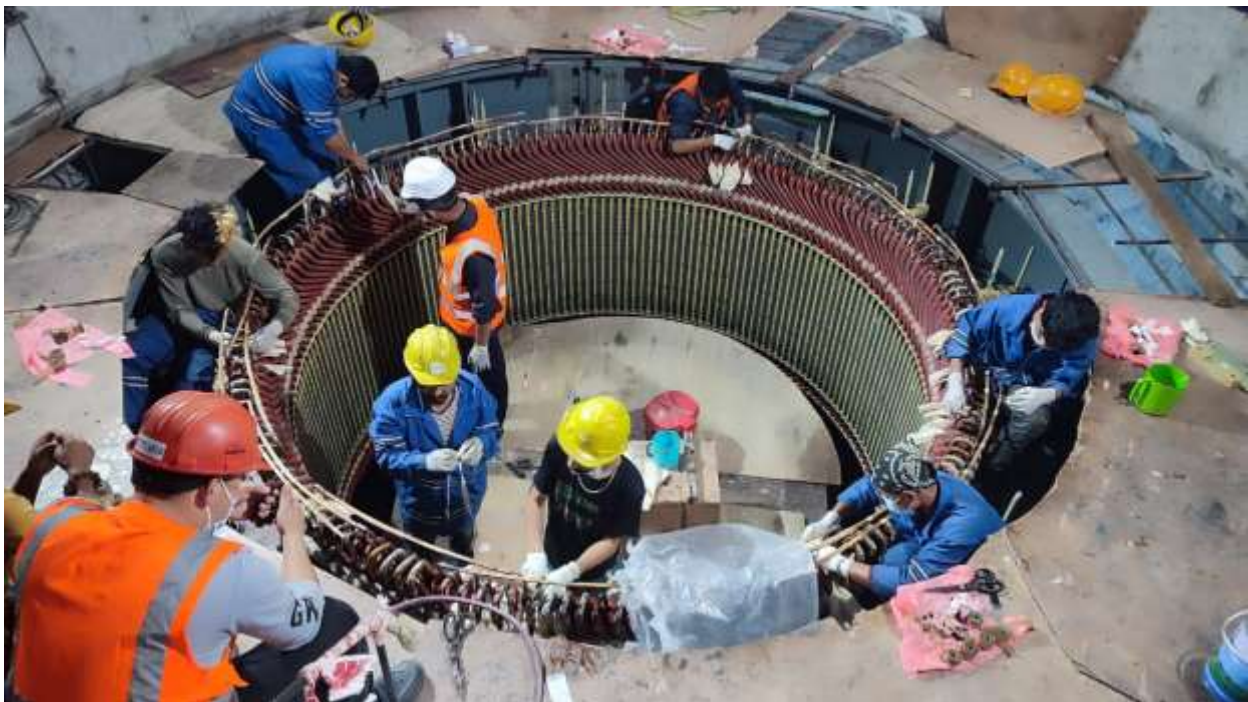
Figure 64: Brazing and insulating work of stator coils
