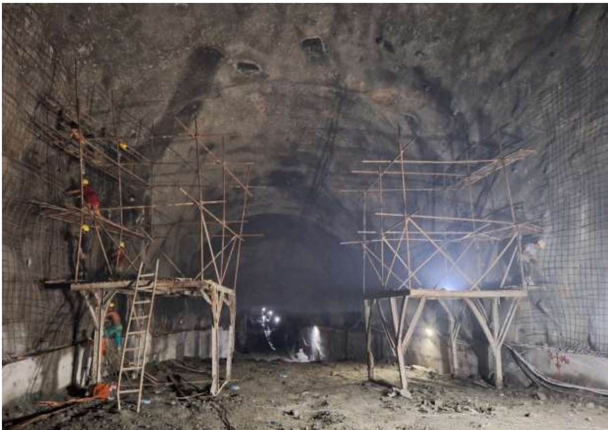
Figure 2-13: A view of wire mesh shotcrete work at Settling Basin 01s
