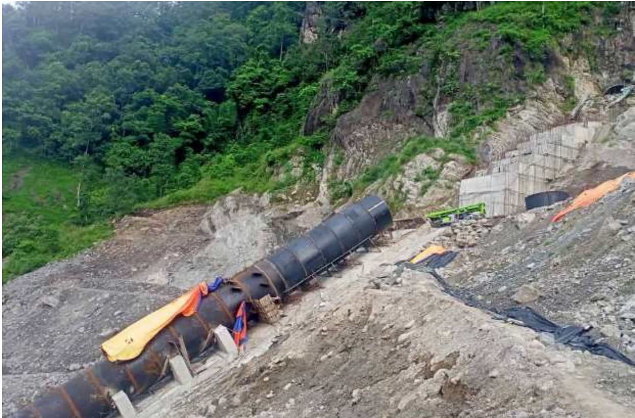
Figure 2-30: Final stage of penstock stabilization works
