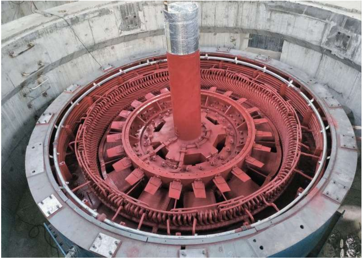
Figure 2-41: Rotor and stator coupling
