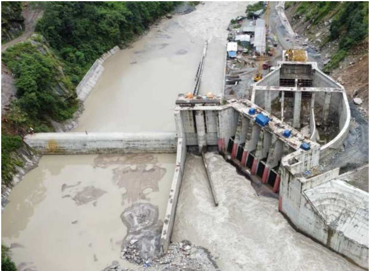
Figure 2-4: Aerial view of Headworks
