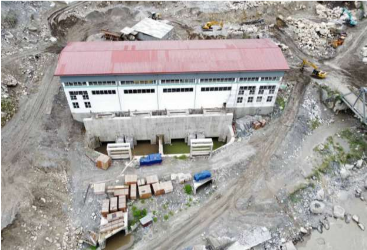
Figure 2-26: A view of powerhouse main building from the downstream
