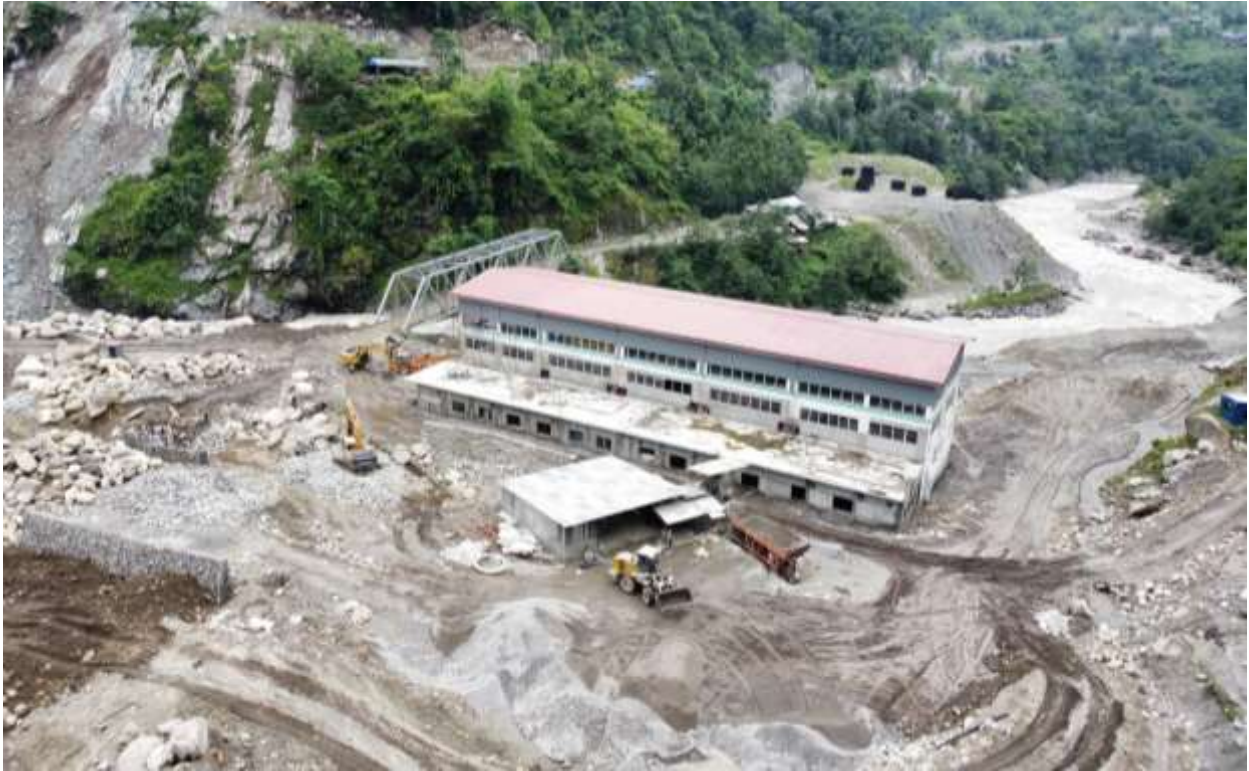
Figure 2-22: A view of backfilling works at the manifold region
