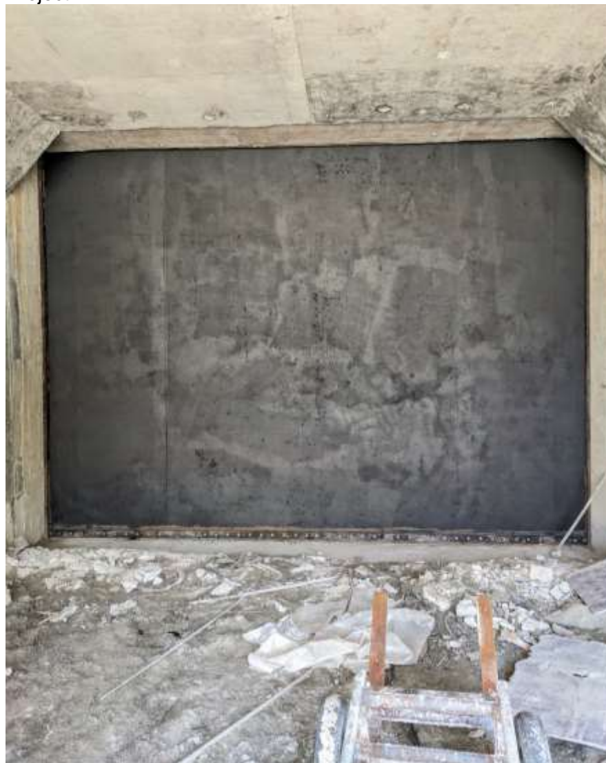
Figure 2-31: Erection of vertical gate at intake
