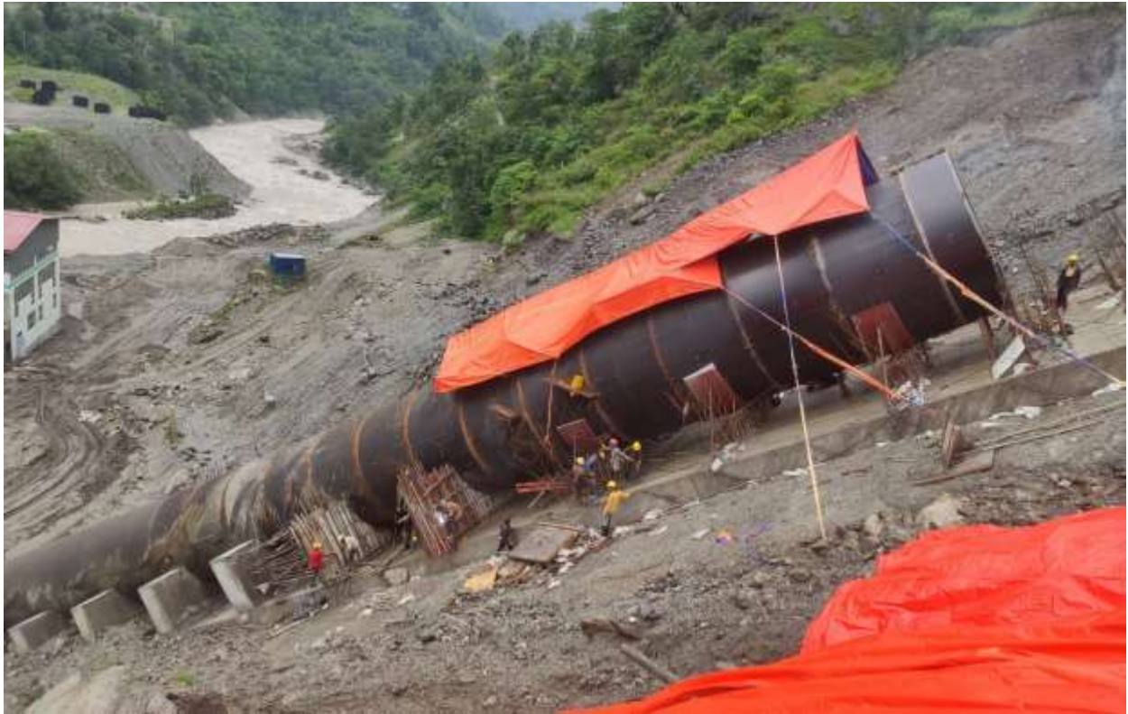
Figure 2-29: Erection of penstock pipes
