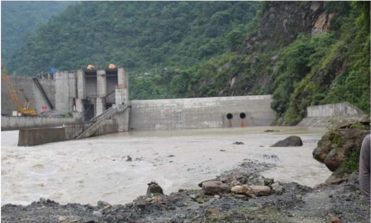
Figure 2-6: A view of weir from upstream
