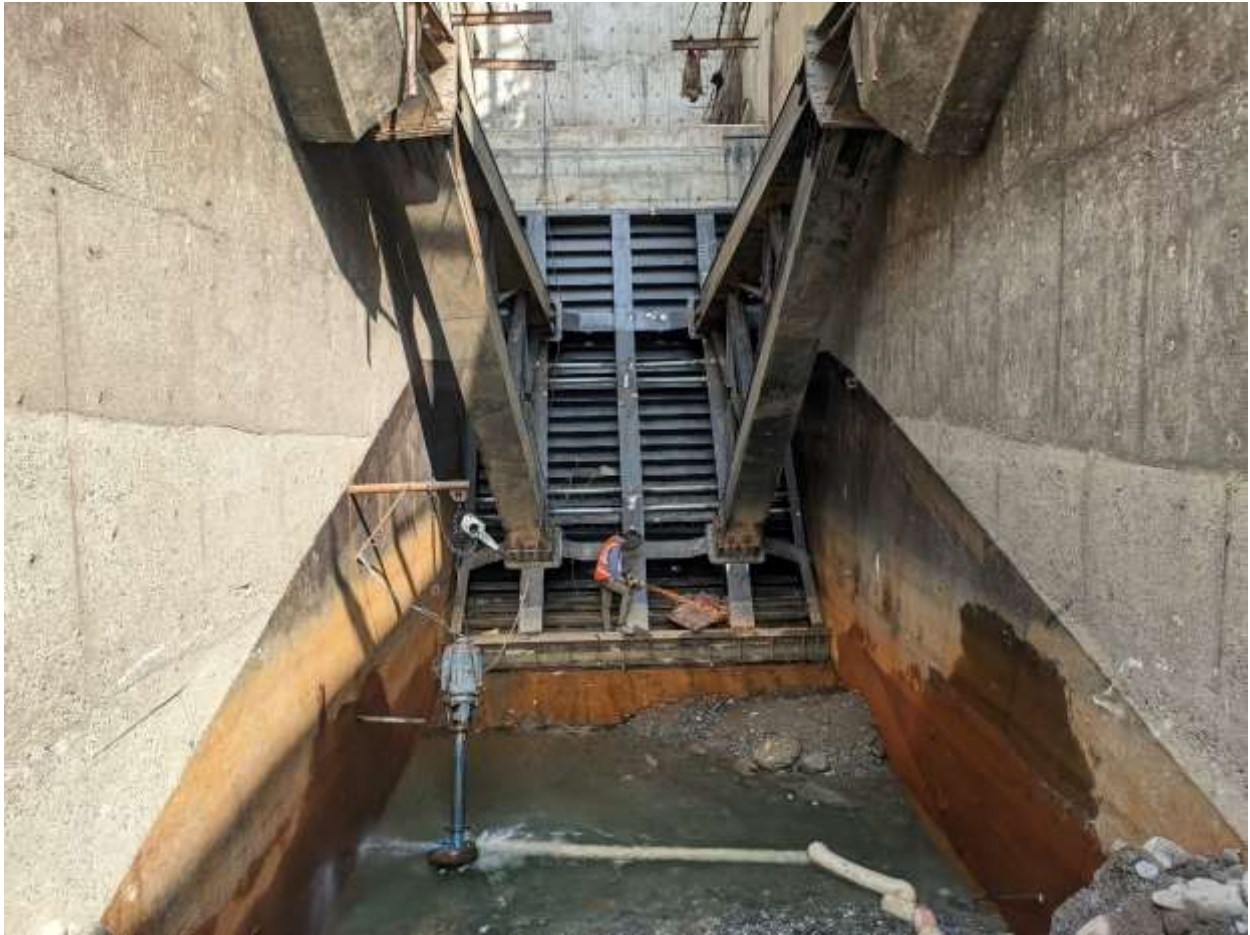
Figure 2-32: Erection of radial gate at undersluice
