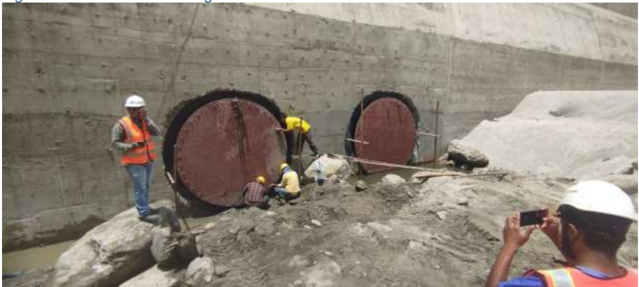
Figure 2-33: Plugging of openings at weir
