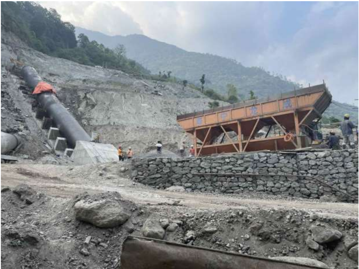
Figure 2-23: Shifting of batching plant over manifold region
