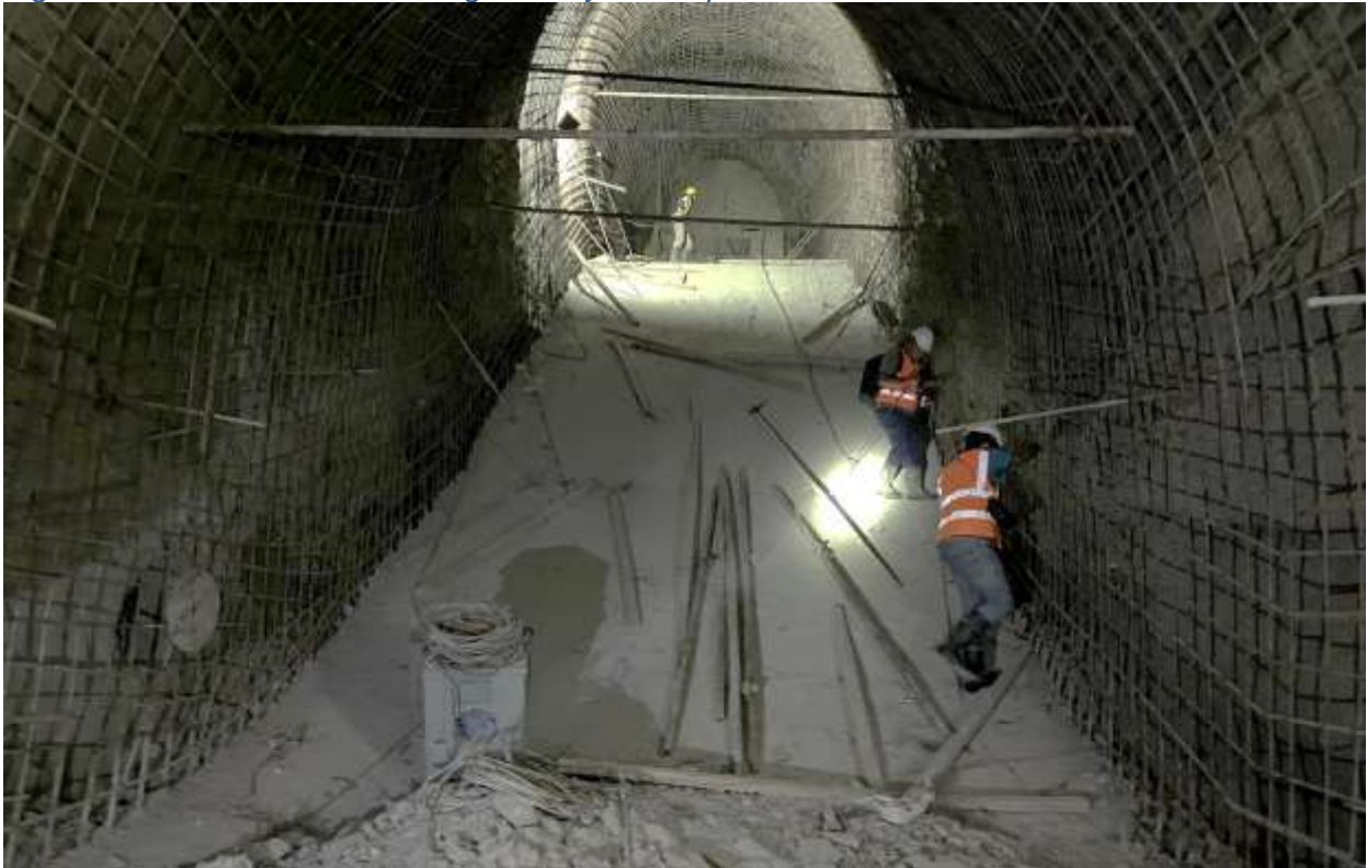
Figure 2-19: Concreting at connecting tunnel slope
