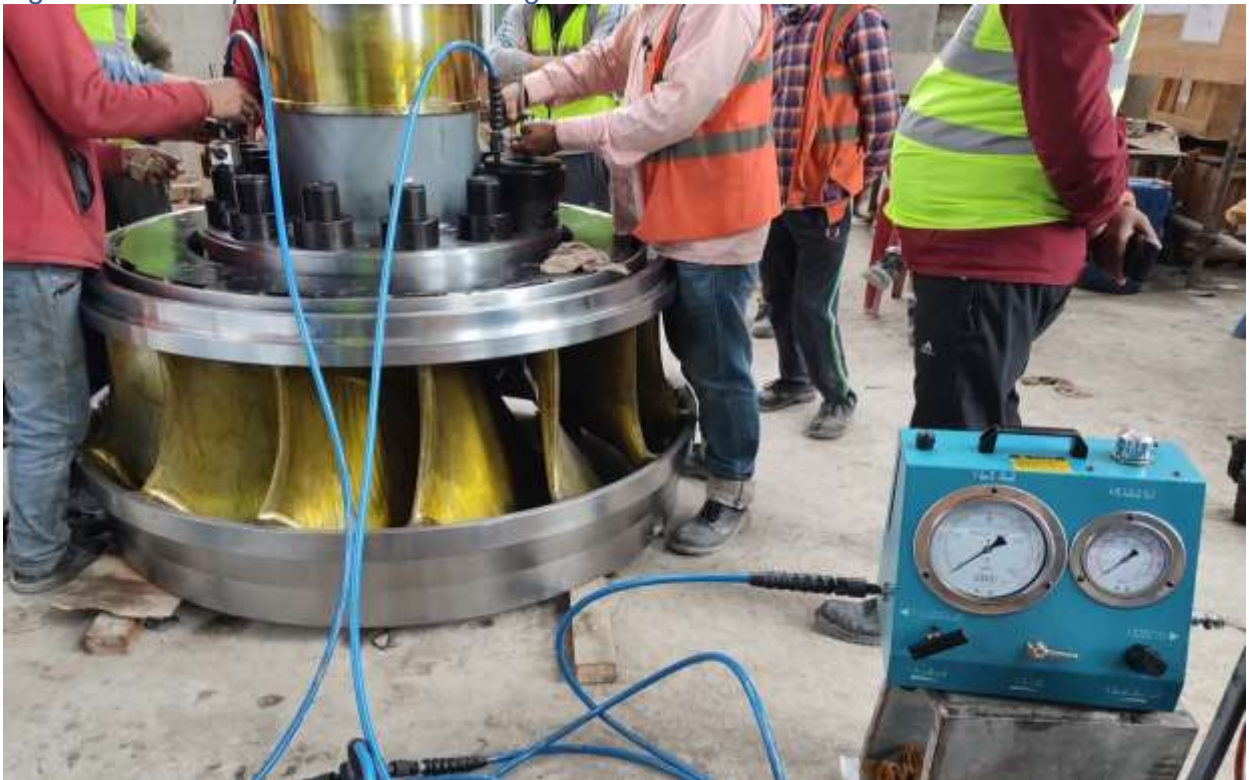
Figure 2-46: Assembly of runner with main shaft
