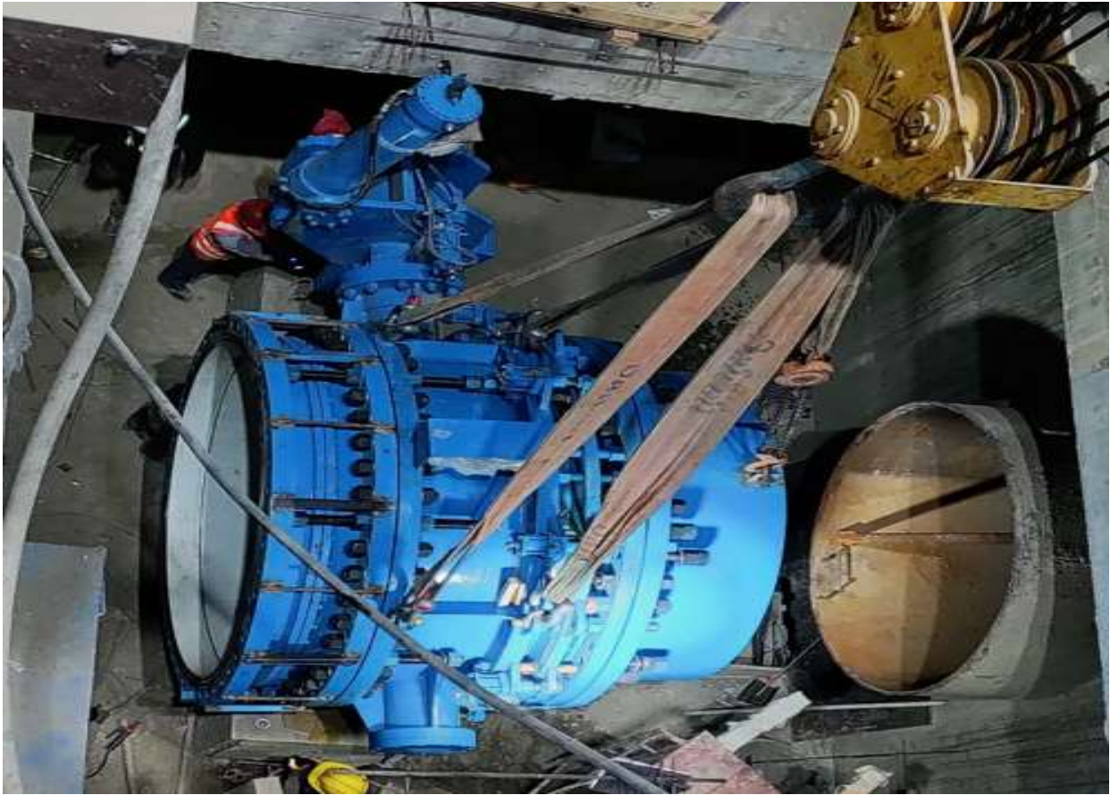
Figure 2-49: Unit 03 MIV lowered in to its position
