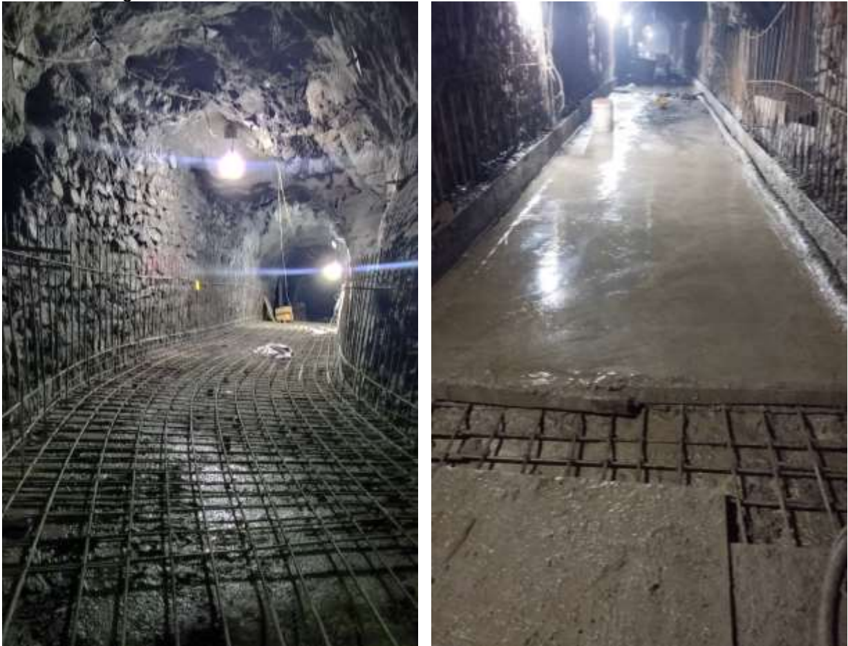
Figure 2-21: A view of rebar layout at the flushing tunnel
