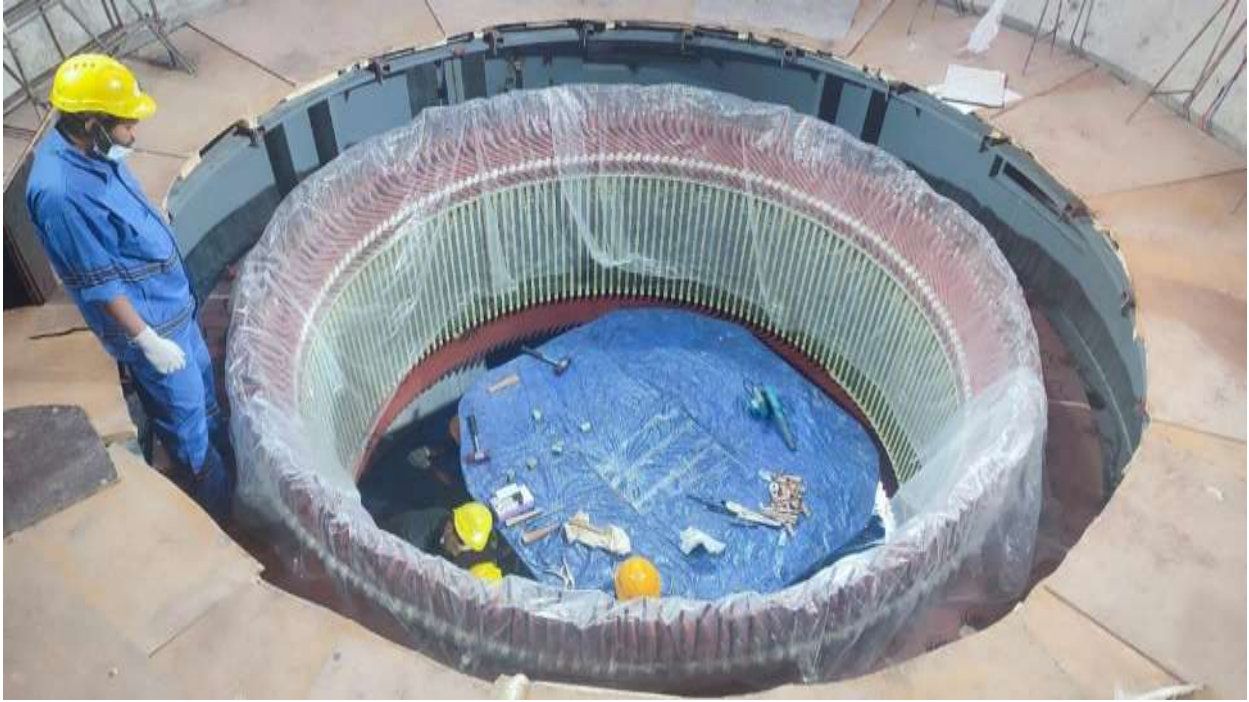
Figure 2-45: Completion of stator winding works
