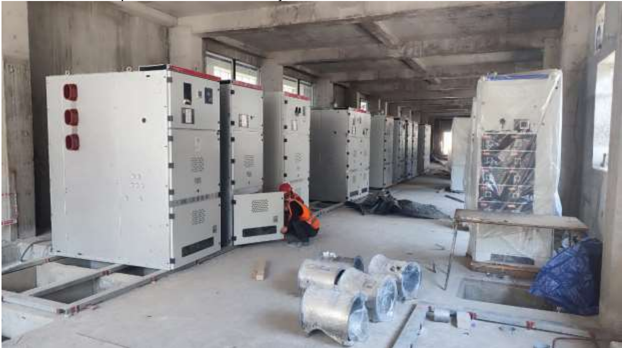
Figure 70: Installation of 11 kV switchgear panels
