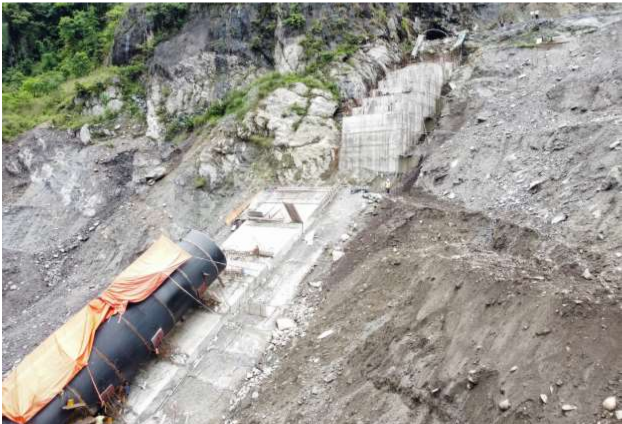
Figure 2-25: Penstock stabilization works
