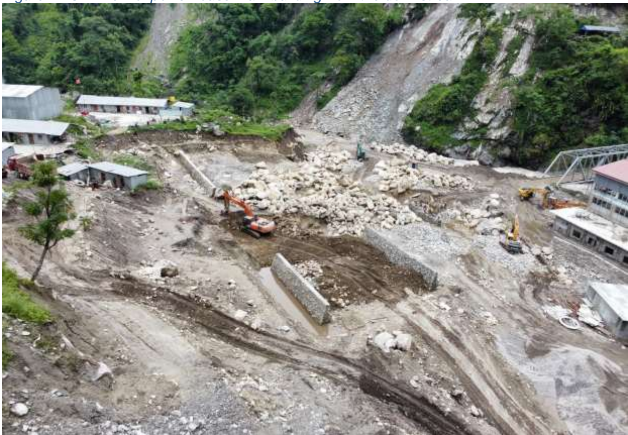
Figure 2-27: Excavation works at the switchyard area
