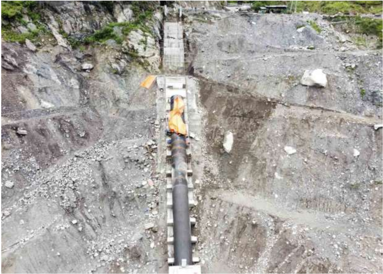
Figure 2-24: Penstock installation works
