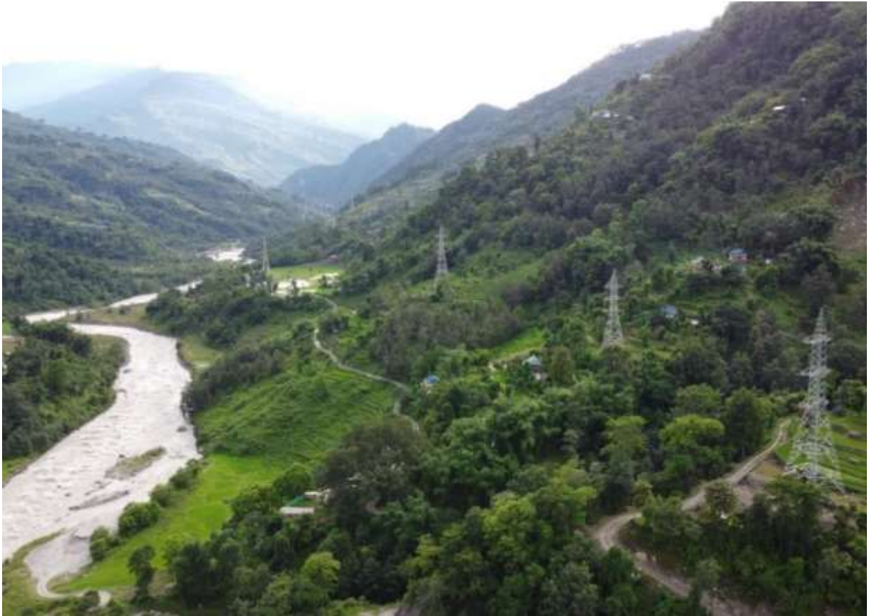
Figure 2-53: View of erected towers from right bank of Tamor
