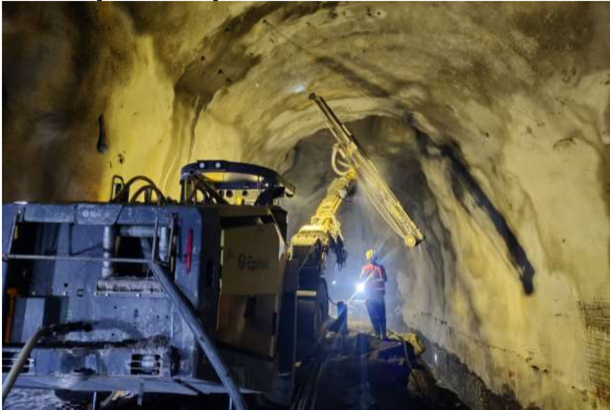
Figure 2-14: Additional Rock bolt installation in SB 03
