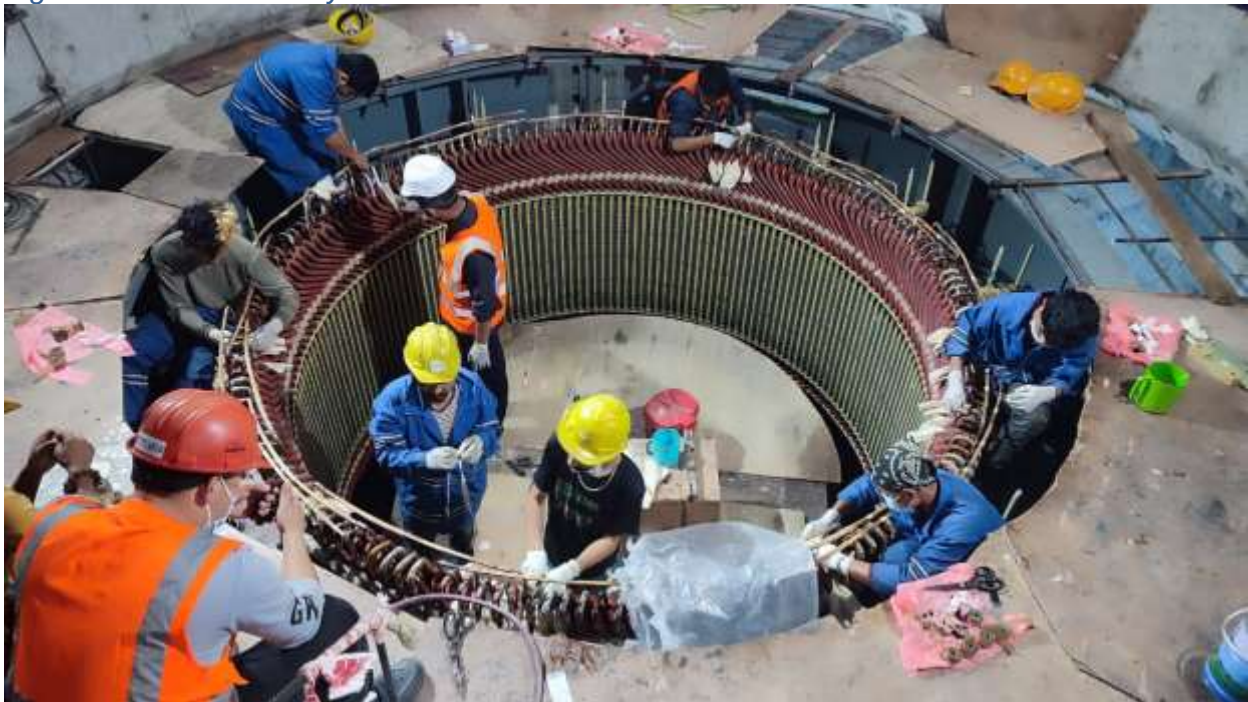
Figure 65: Stator coil insulation work
