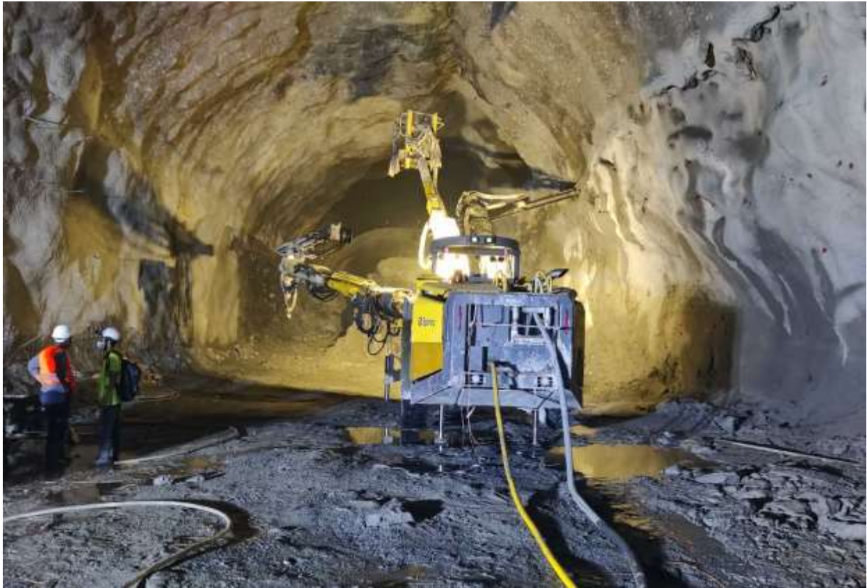
Figure 2-15: Final stage of rock bolt installation works
