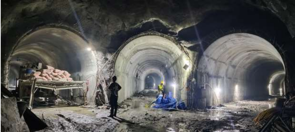
Figure 2-18: A view of connecting tunnel junction point
