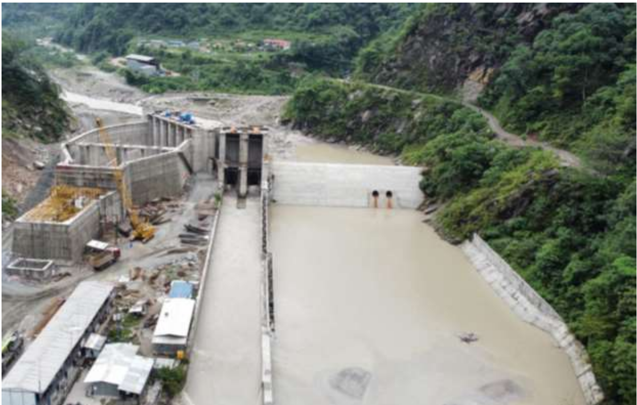
Figure 2-10: A view of headworks from the downstream
