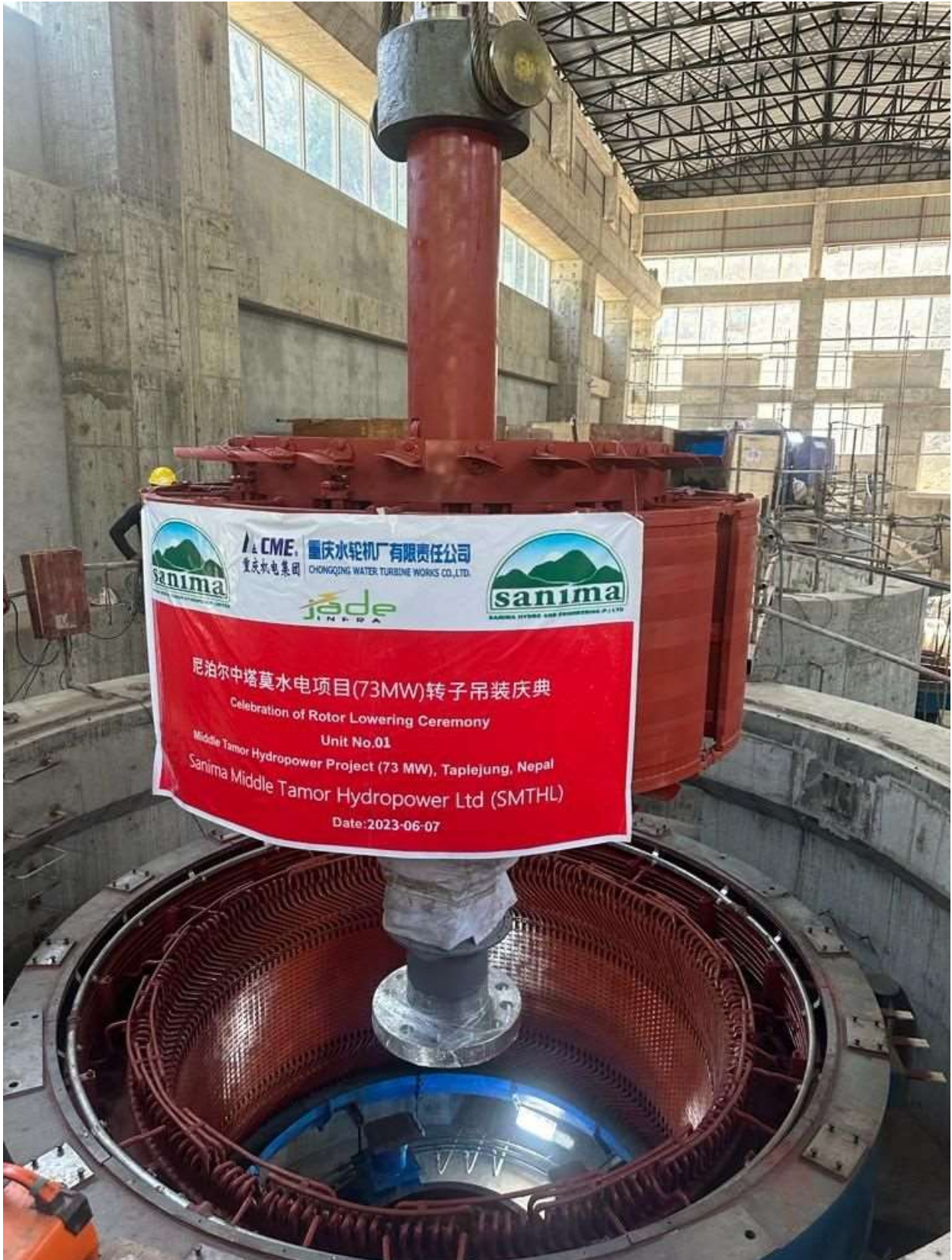
Figure 2-40: Rotor lowering at unit 01
