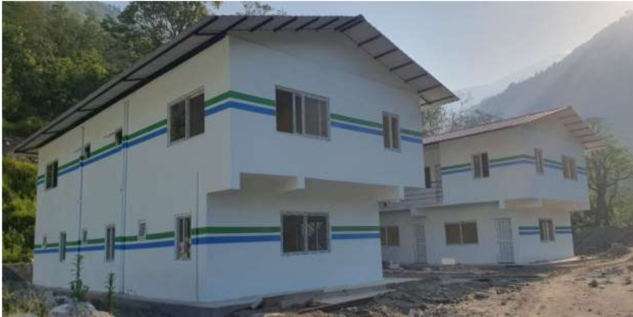
Figure 2-2: Construction of new camp building at the powerhouse
