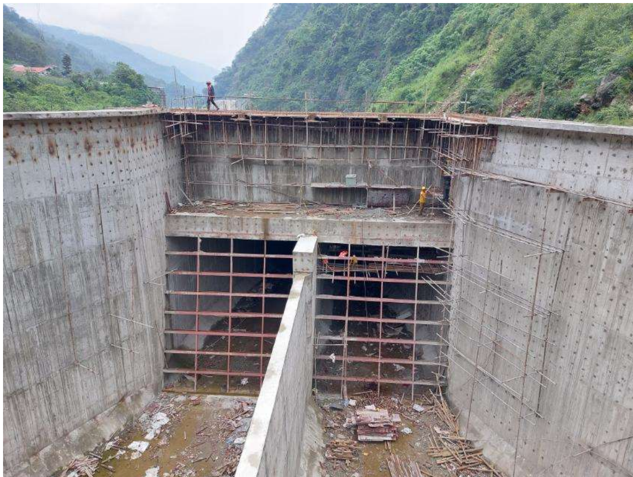
Figure 2-8: Final stage concreting works at the conveyance tank right top slab
