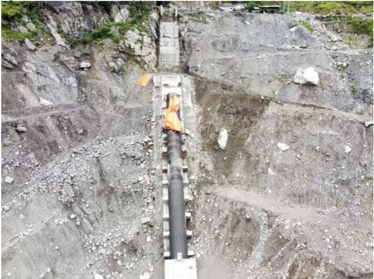
Figure 2-30: Simultaneous work progress with Civil works
