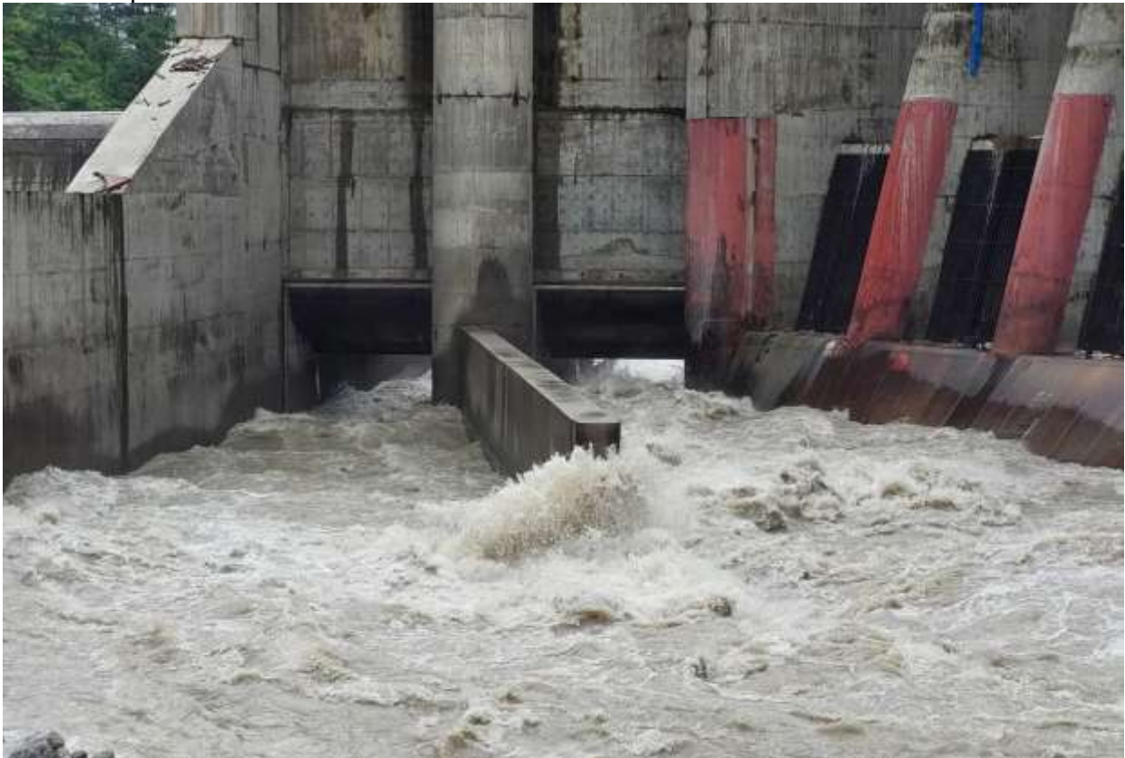
Figure 2-7: Gate installation works at undersluice
