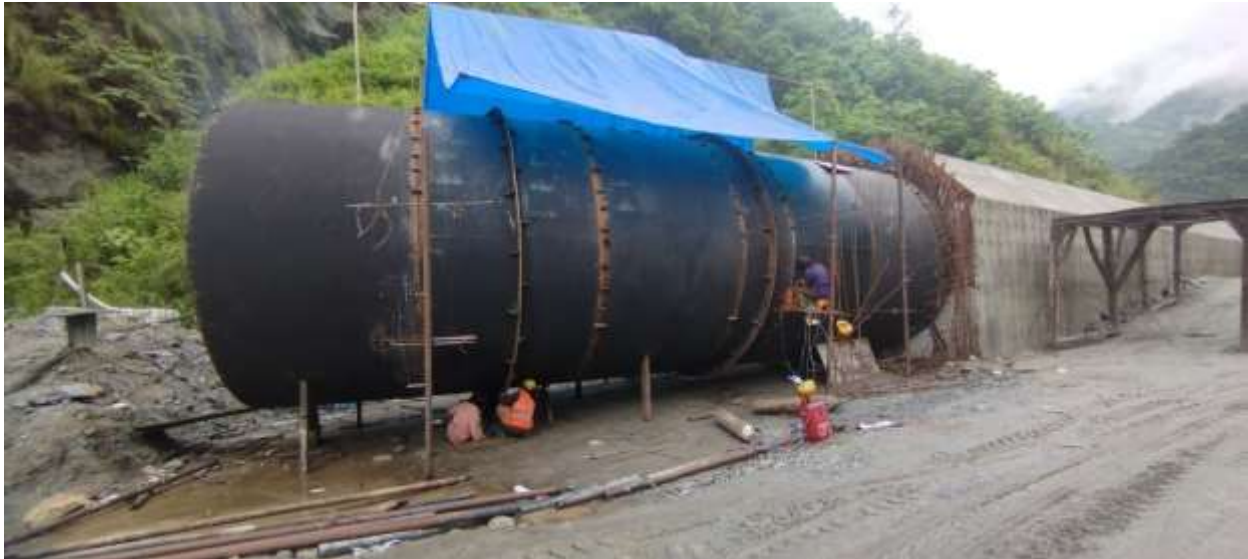
Figure 2-28: Installation of head race bend
