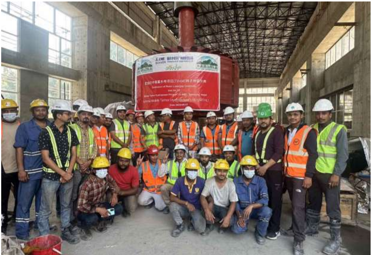
Figure 55: Rotor lowering at unit 1 on June 07, 2023
