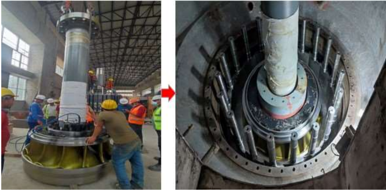
Figure 64: Final assembly of runner with main shaft
