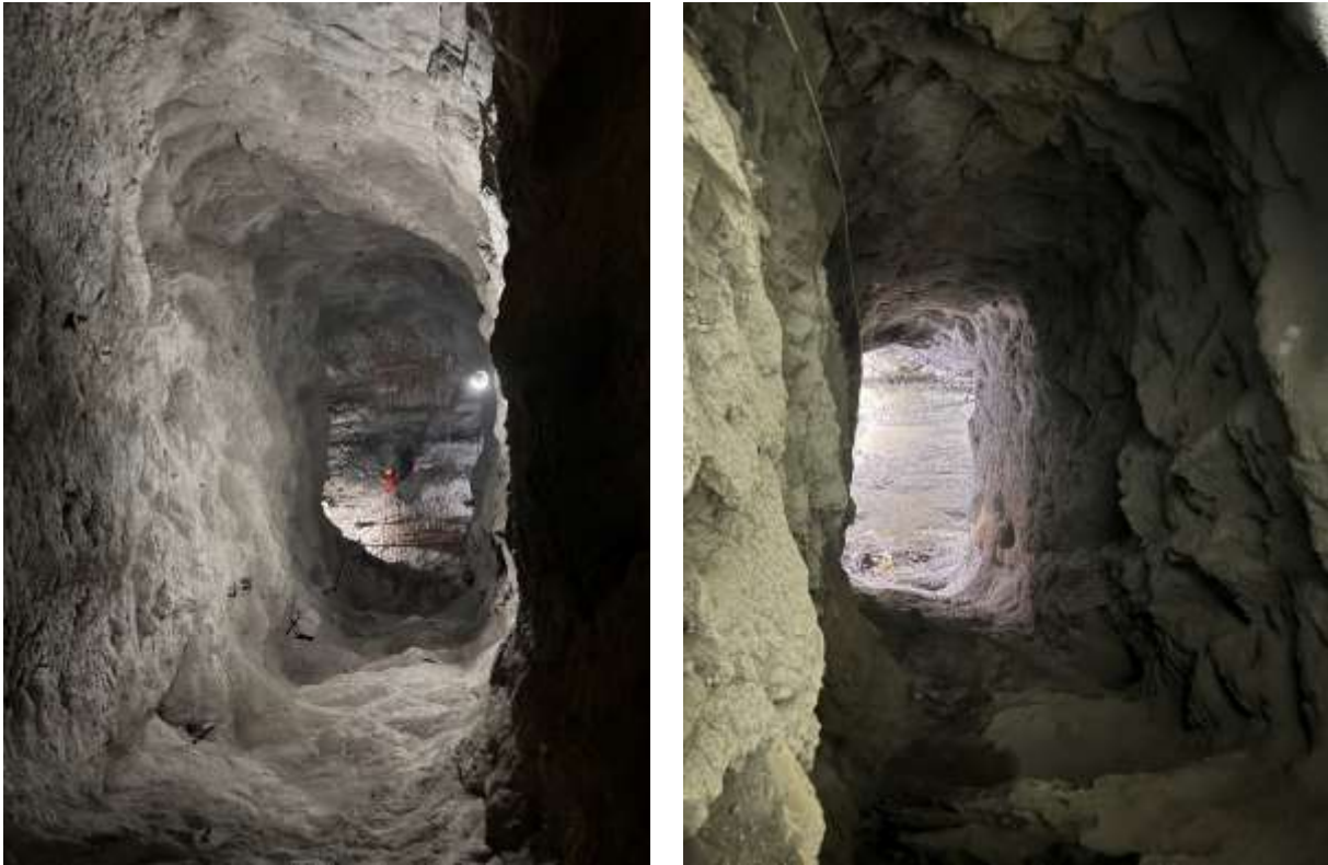
Figure 2-18: Inlet gate shaft 01 (left) and Inlet gate shaft 02 (right)
