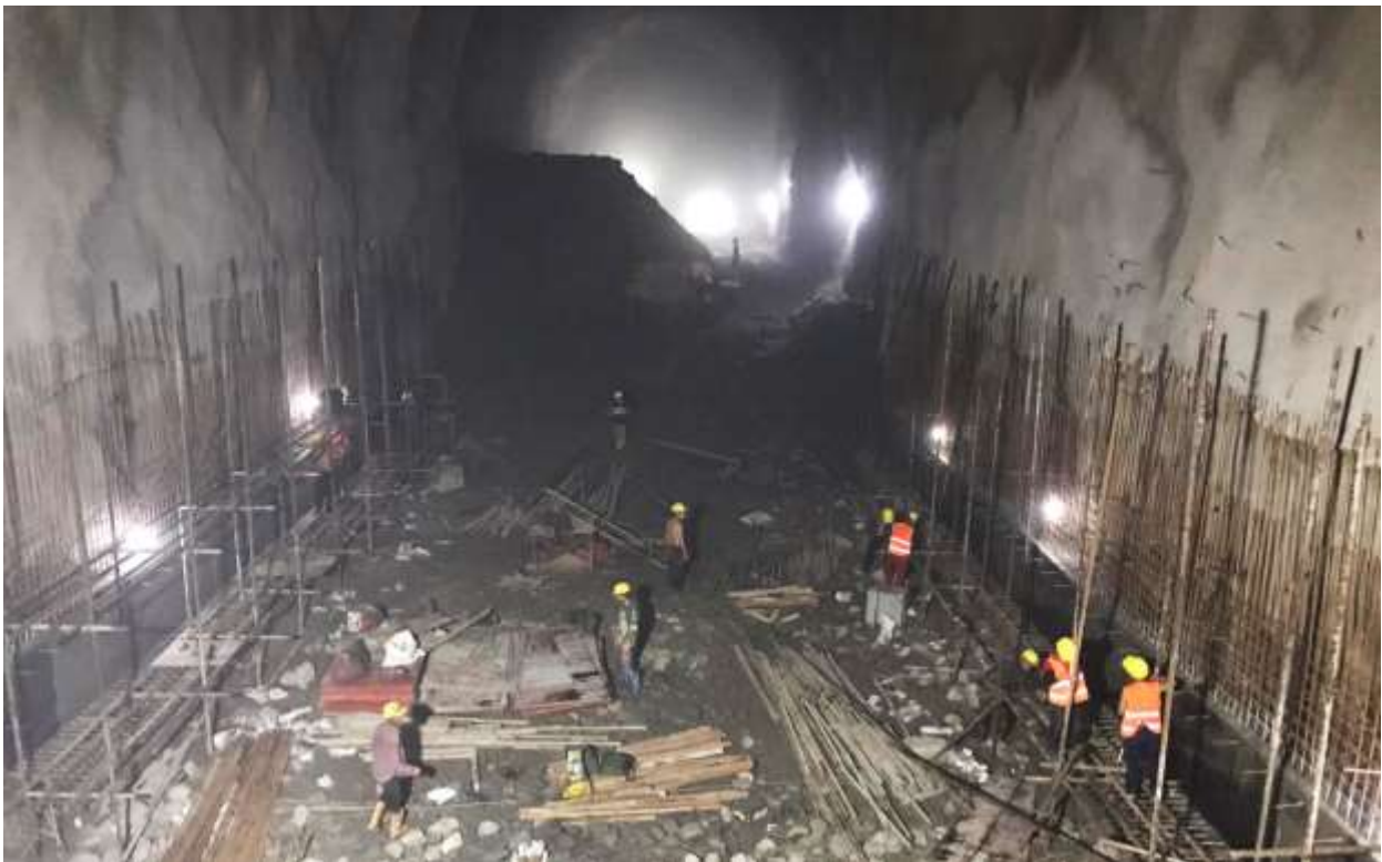
Figure 2-12: Concreting works at the settling basin bay 02 walls
