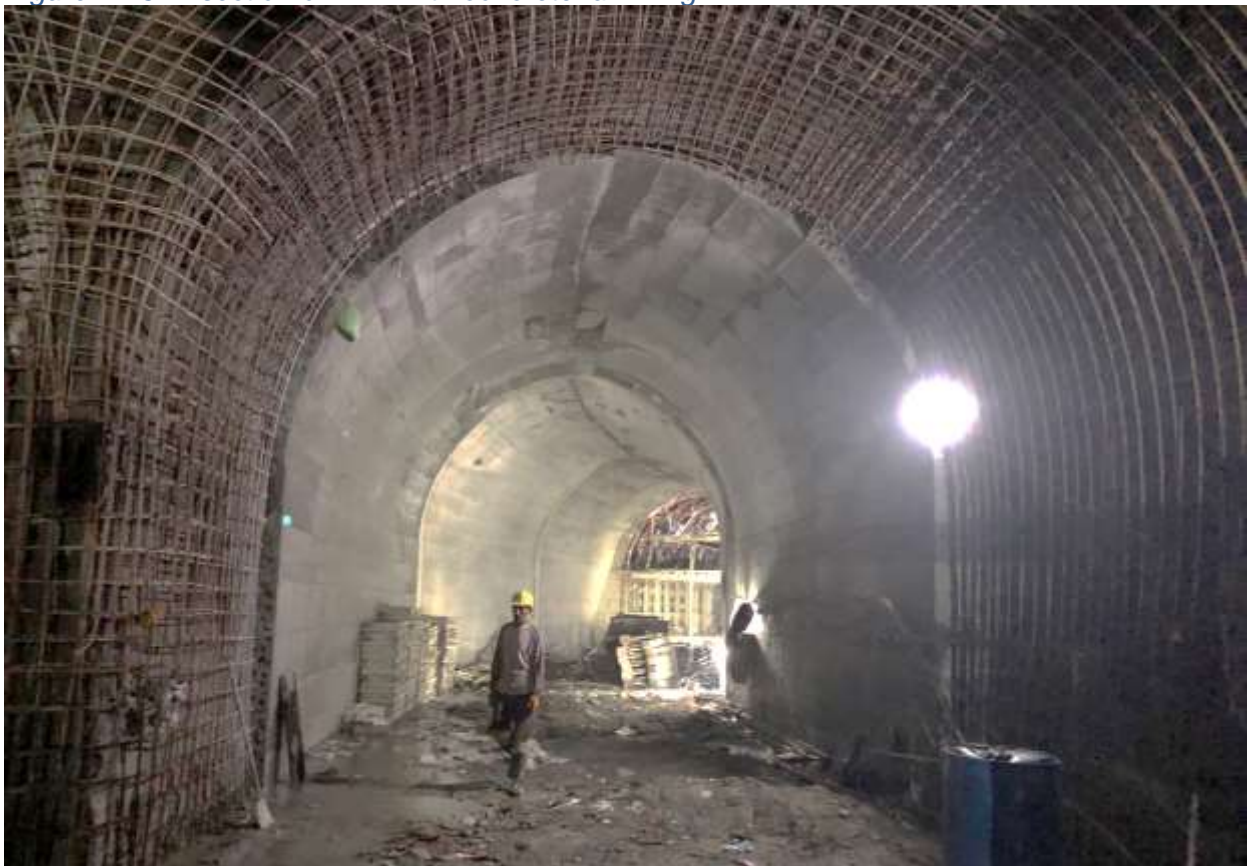
Figure 2-17: Full lining section at HRT bends
